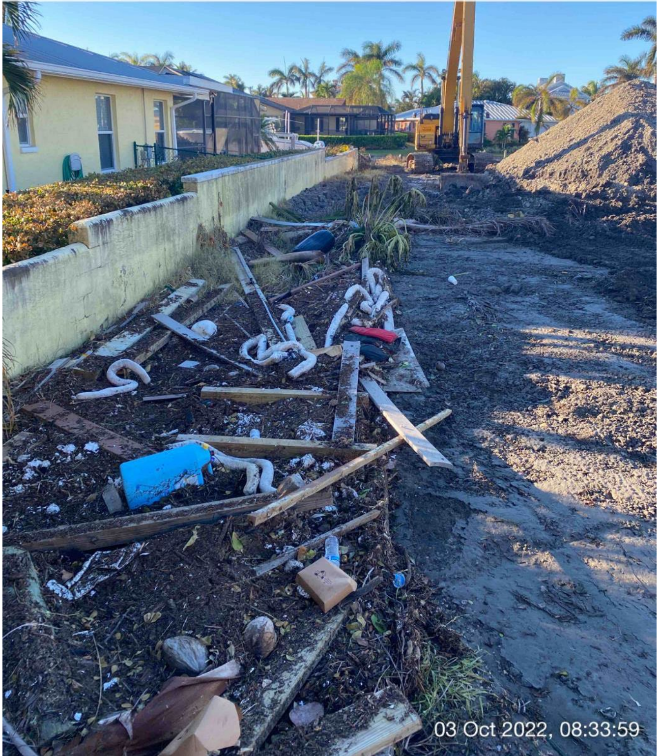
Debris washed up to east side of 1300 Curlew Avenue
