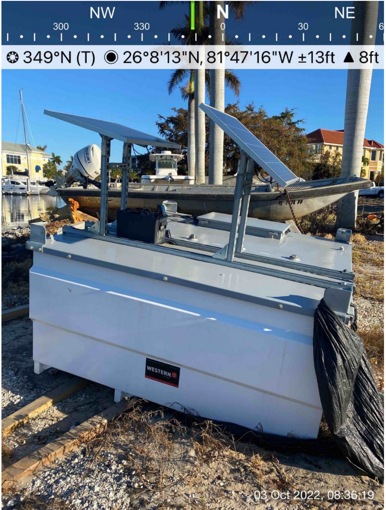
Support frame broken and large fuel cube buried into ground at southwest corner of 1300 Curlew Avenue
