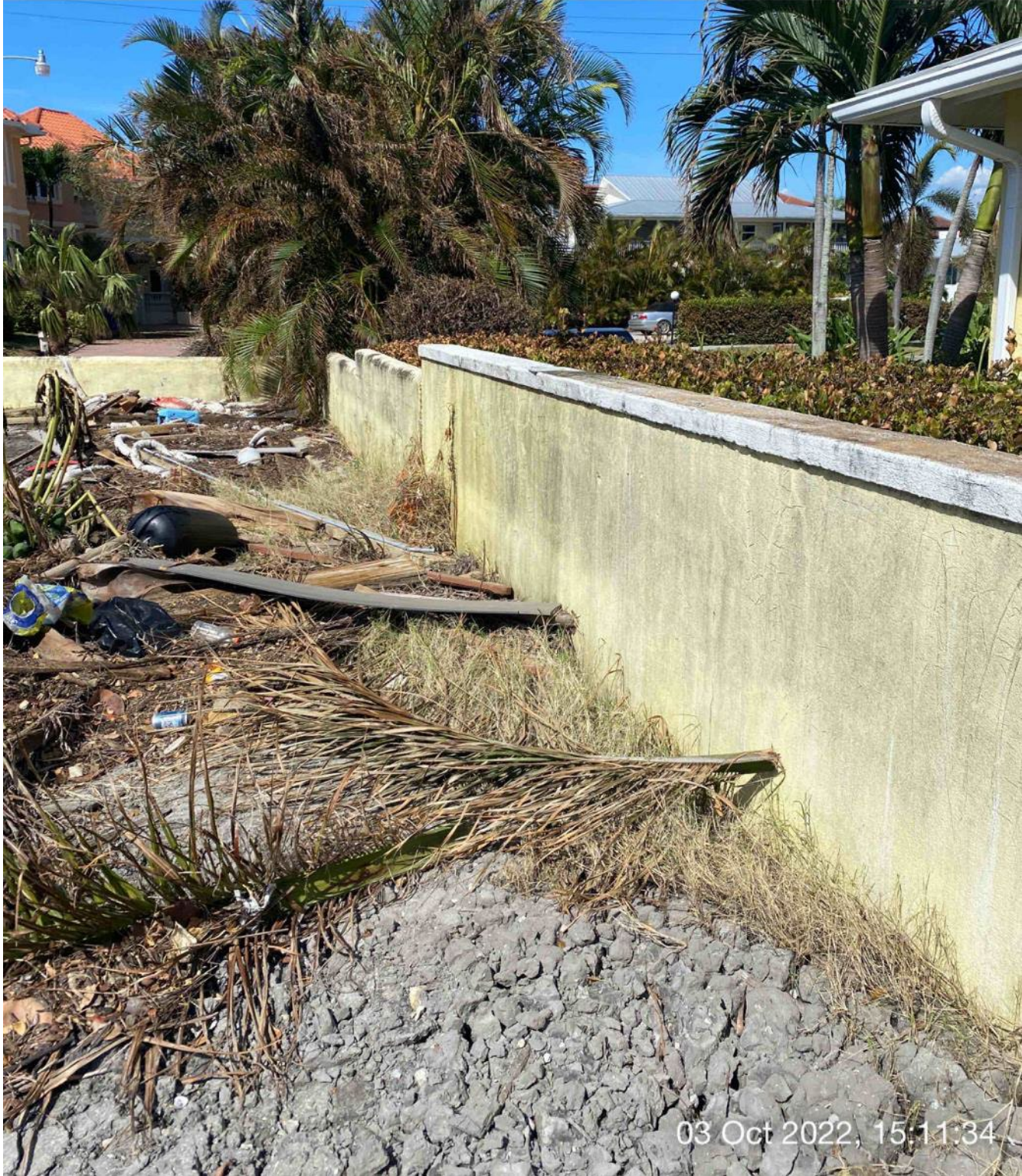
Debris and high water mark on east side wall at 1300 Curlew Avenue
