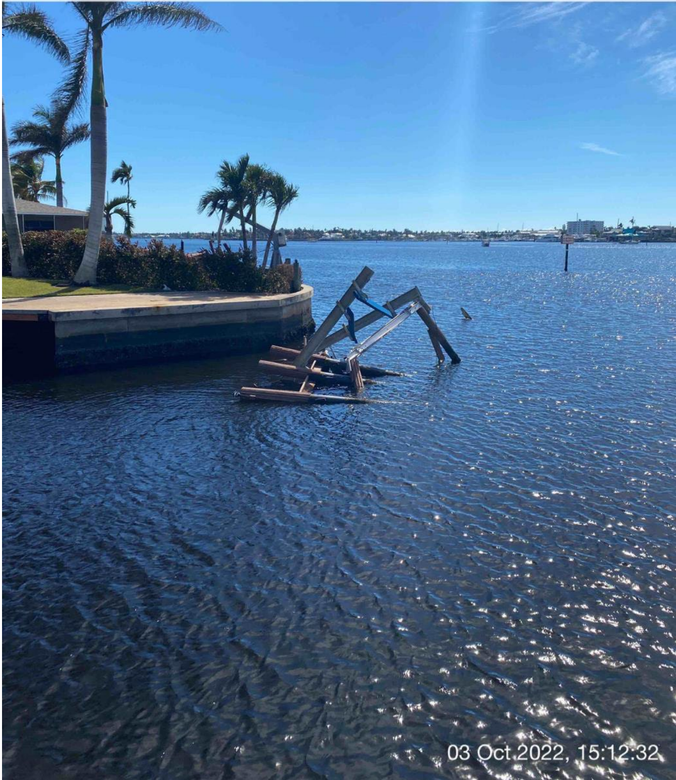
Destroyed dock section and boat lift in Canal CC-CC station 1+00
