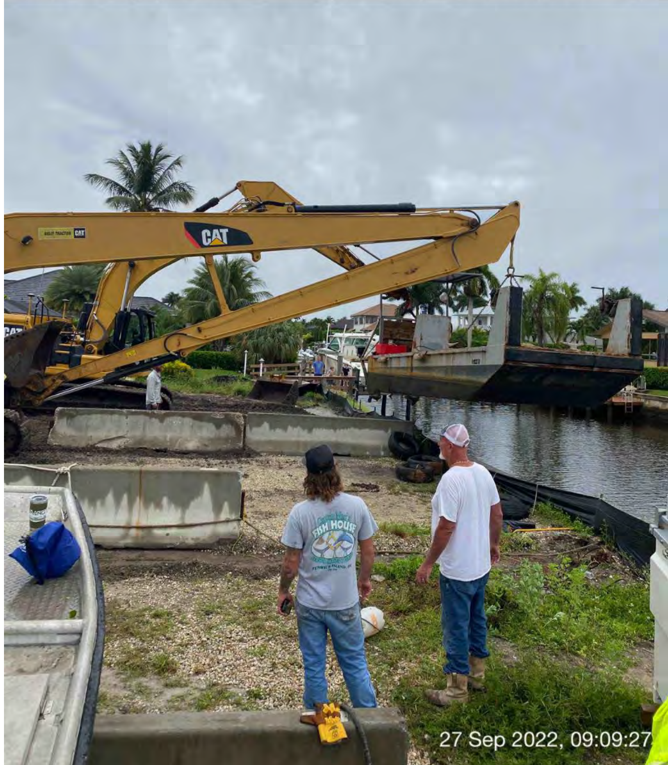
323 and 326 excavators lifting push boat out of Canal CC-CC and onto jersey barriers at 1300 Curlew Avenue
