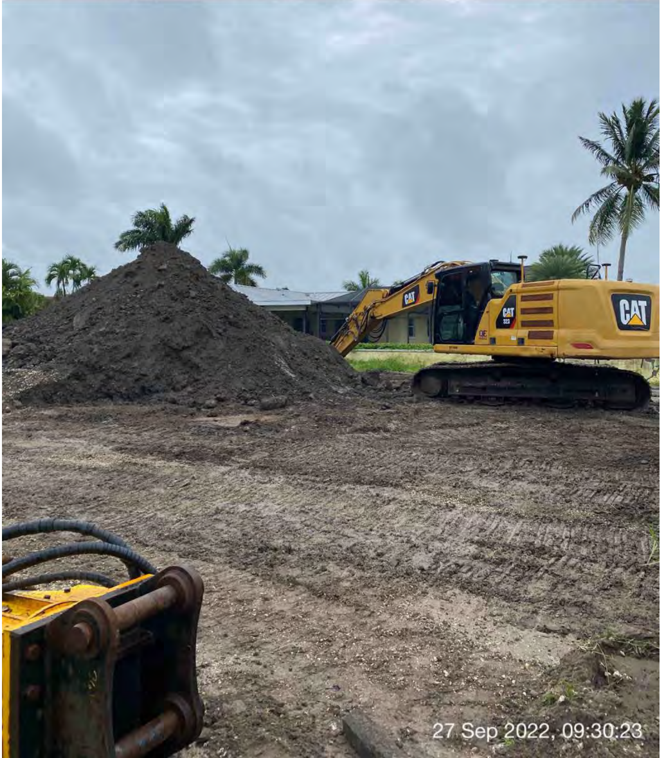
323 excavator and removed material on site at 1300 Curlew Avenue
