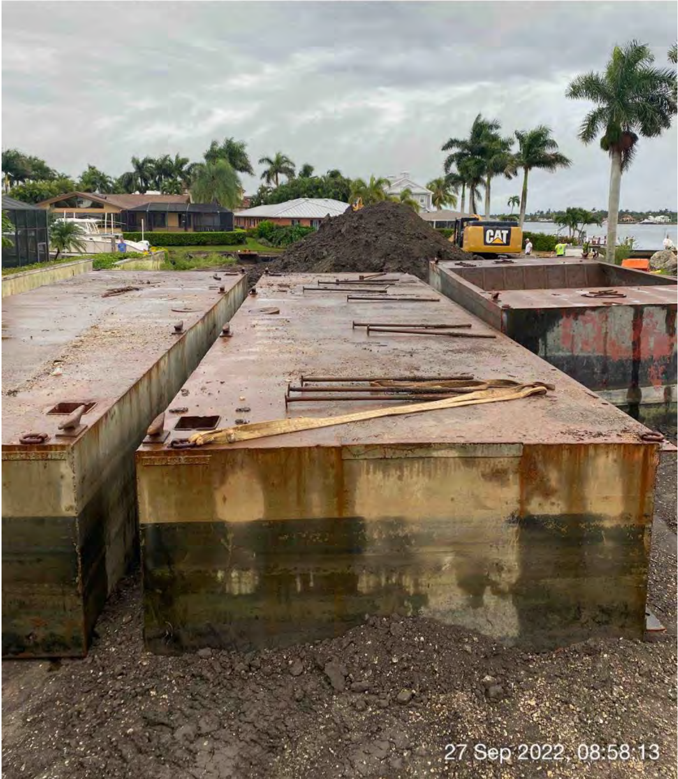
Two barge sections and hopper on site at 1300 Curlew Avenue
