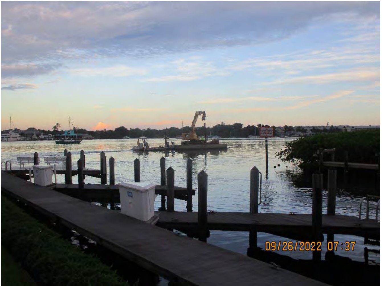
Barge heading out of Canal W-W mouth back towards 1300 Curlew Ave.
