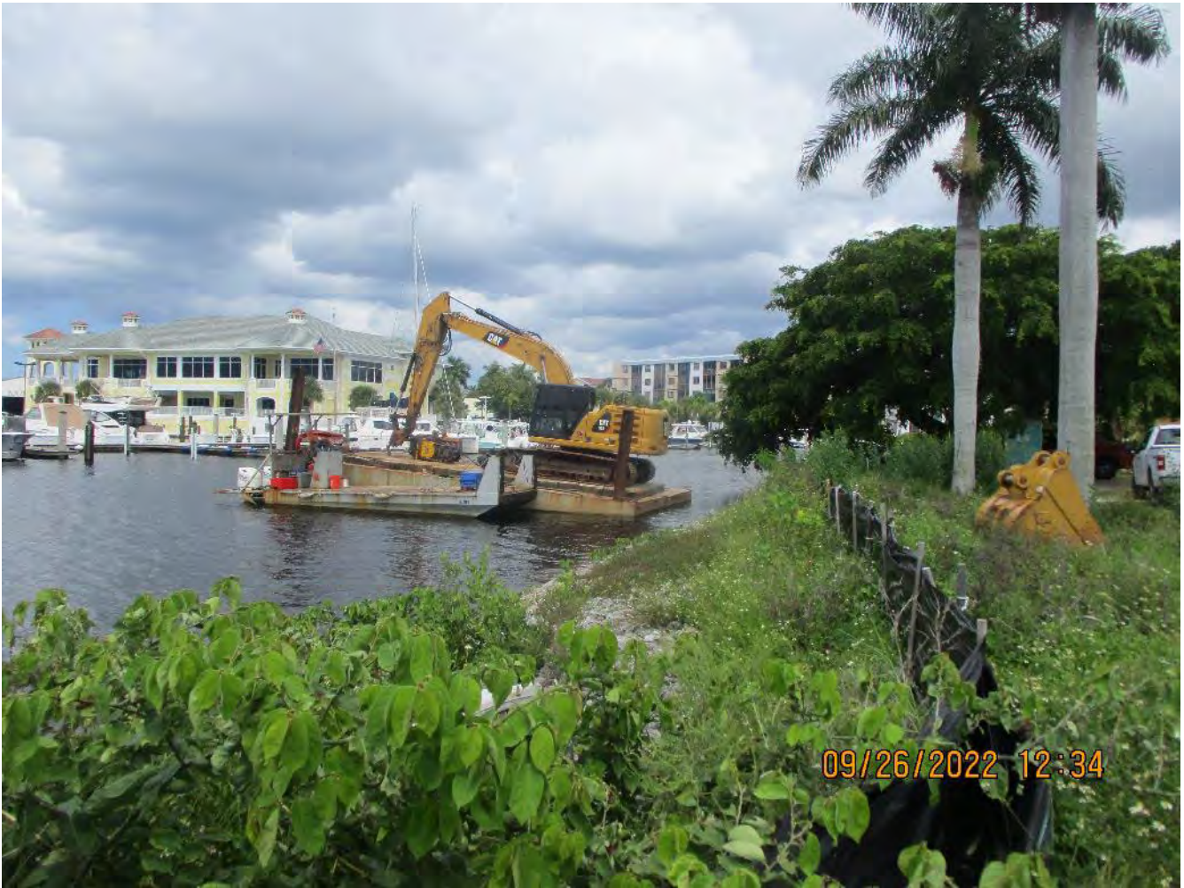
Excavator walk off area to Curlew Ave staging location
