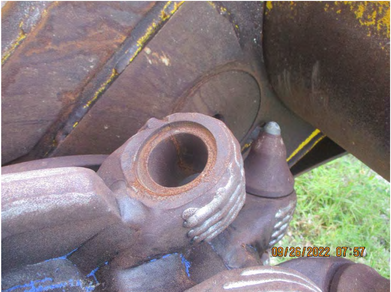
Cracked cutting tooth sleeve
