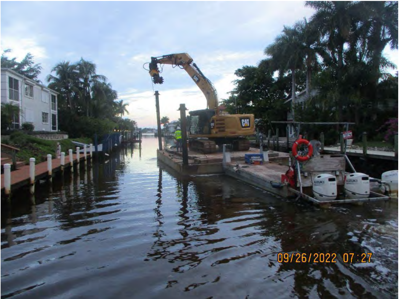
Barge/excavator/push boat leaving staged area at approx. station 13+00 (Canal W-W)
