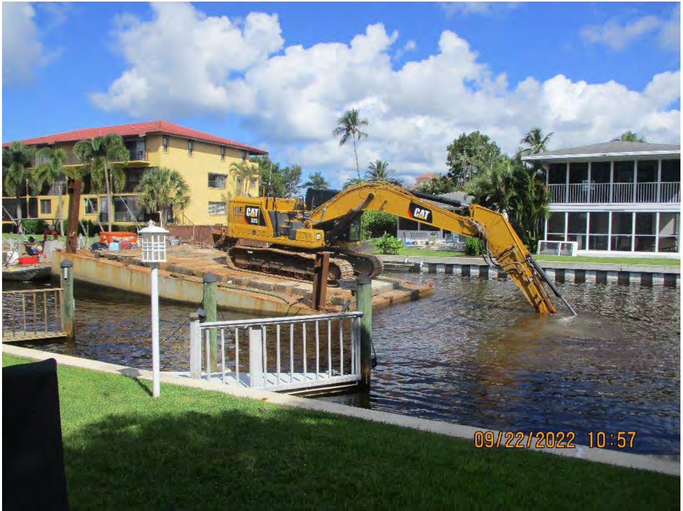
Canal W-W bottom grinding in progress (approx. sta. 10+50)
