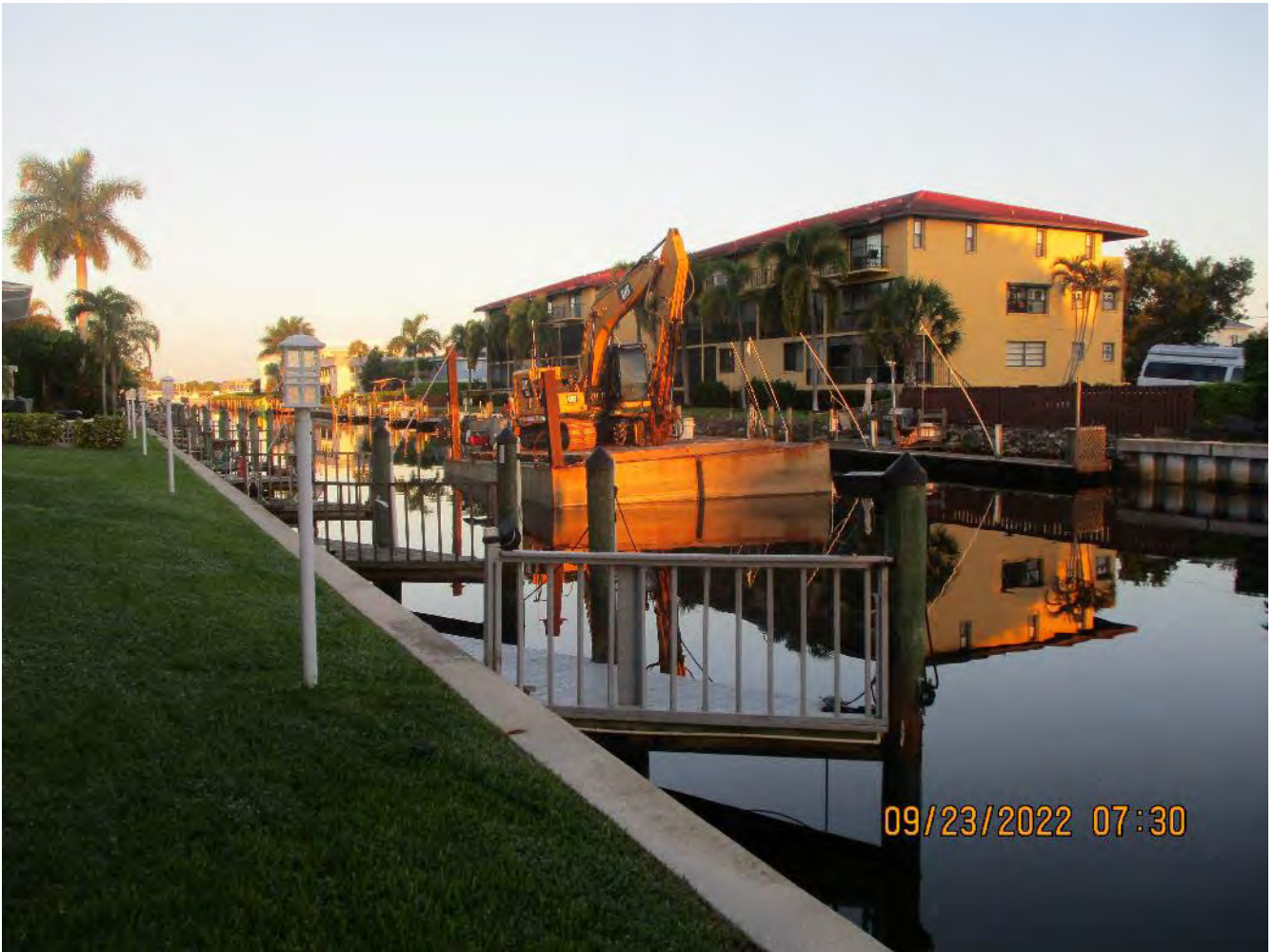
Barge/excavator/push boat staged at approx. station 10+00 (Canal W-W)
