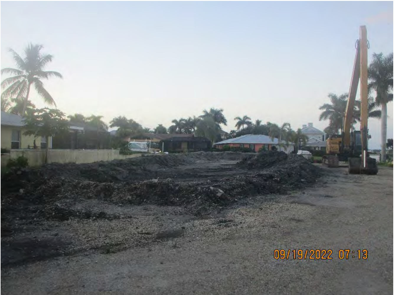
Current status of 1300 Curlew Ave project stockpile/staging area
