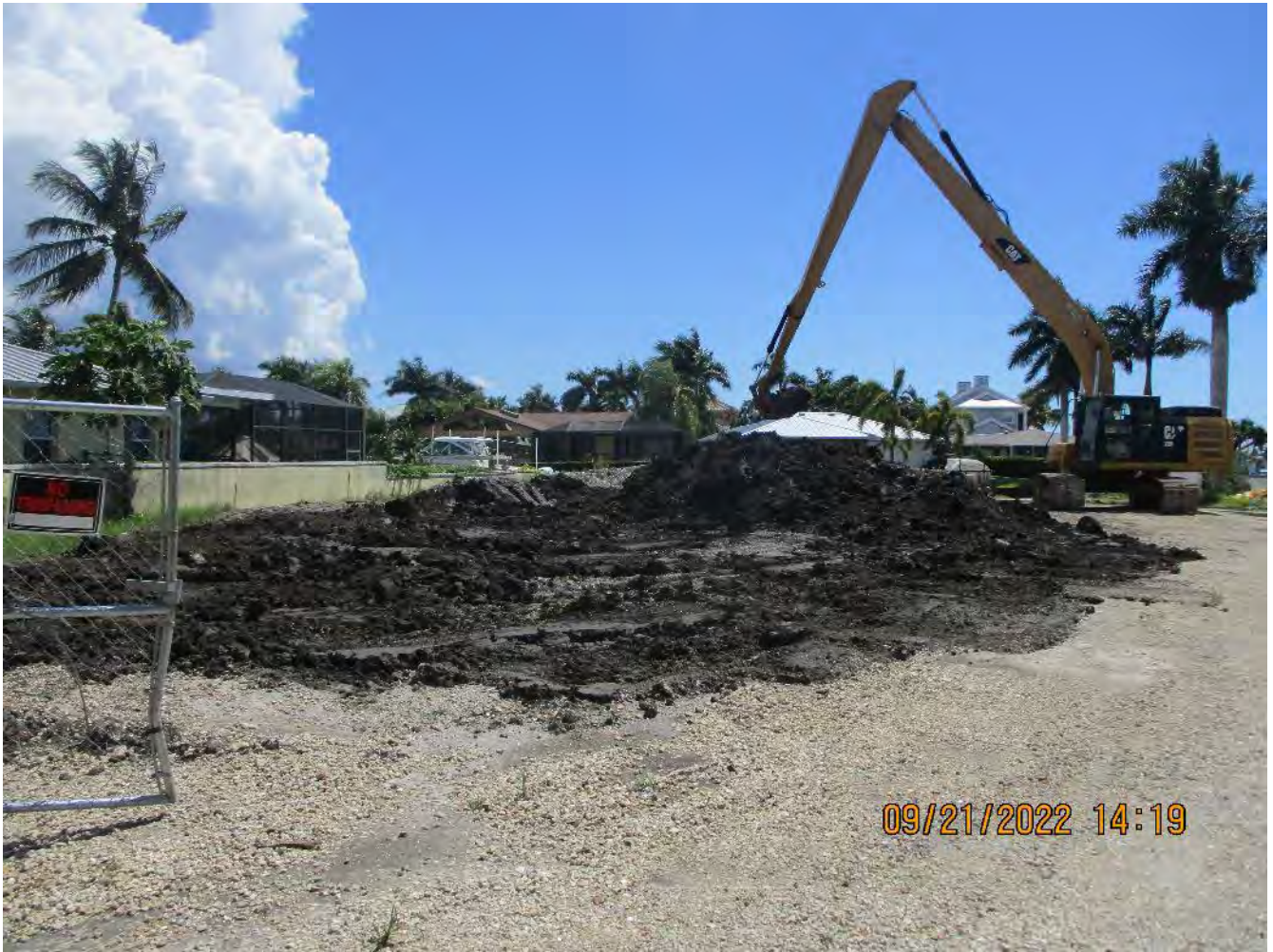
Long stick excavator stockpiling previously dredged material (1300 Curlew Ave. location)
