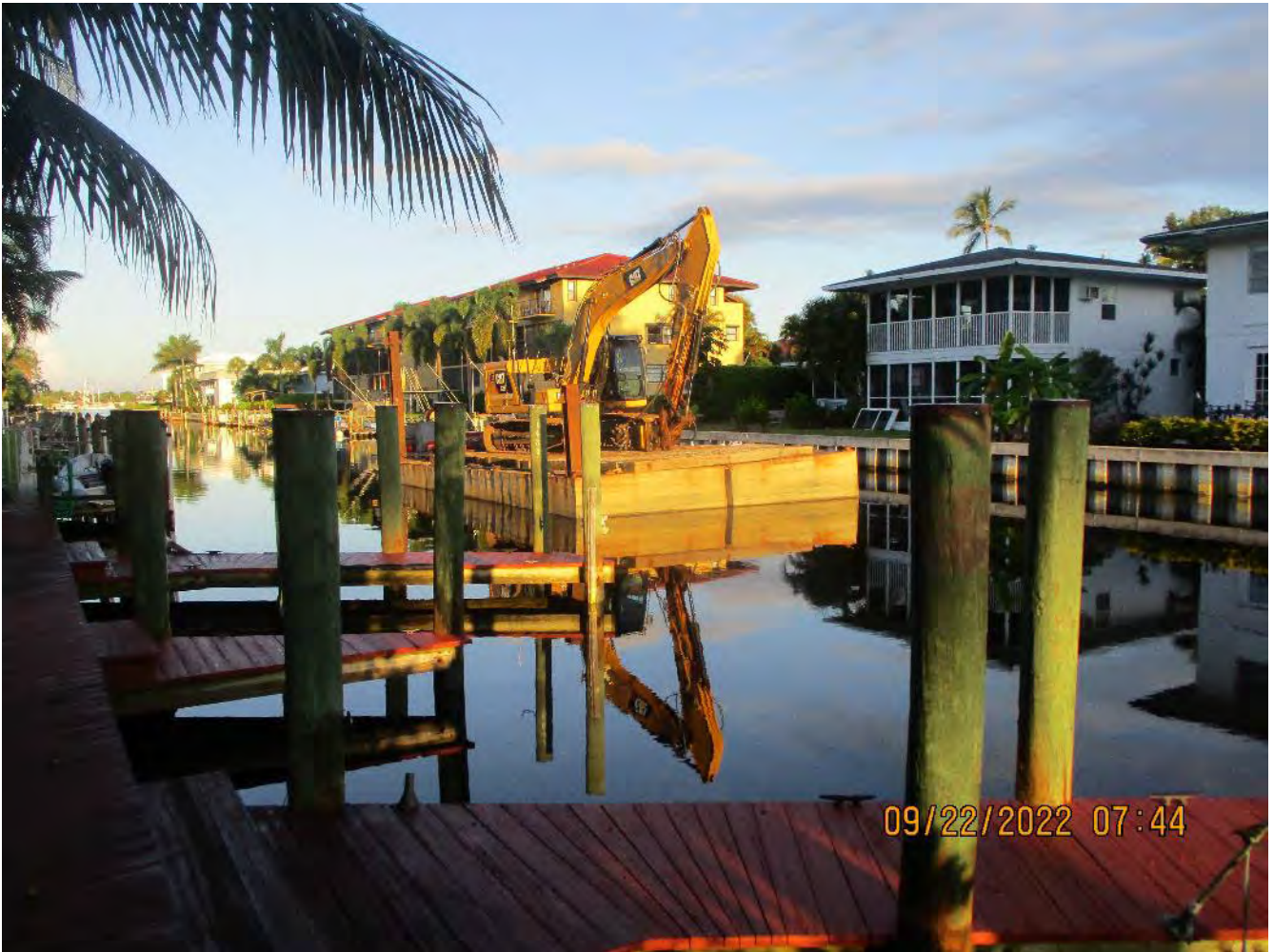
Barge/excavator/push boat staged at approx. station 10+75 (Canal W-W)
