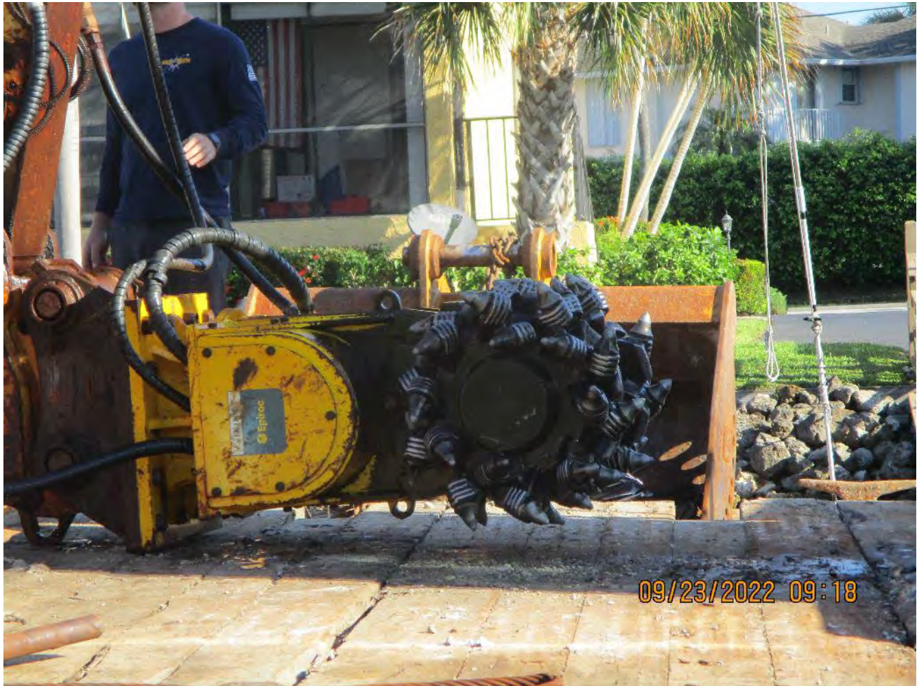
Contractor examining grinding attachment/excavator boom areas
