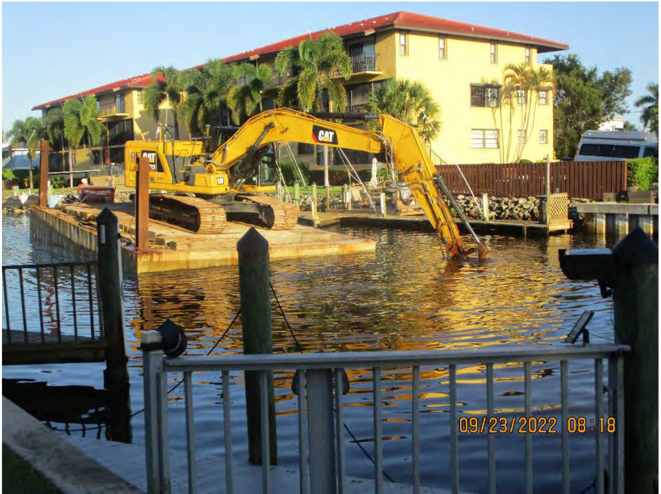
Start of canal bottom grinding (Canal W-W, approx. station 10+00)
