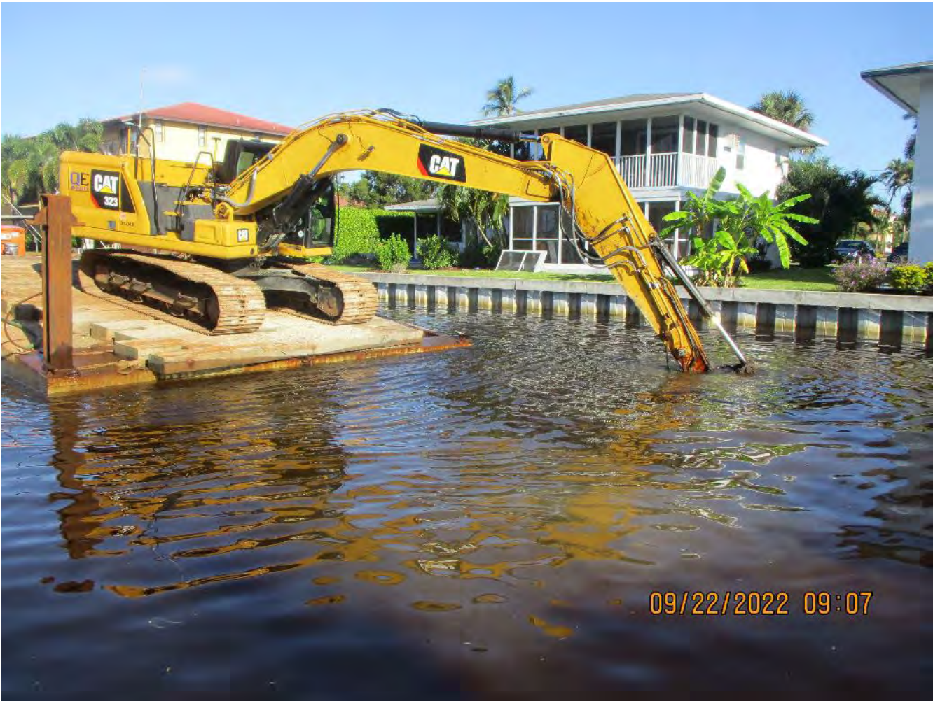
Canal W-W bottom grinding in progress (approx. station 10+75)
