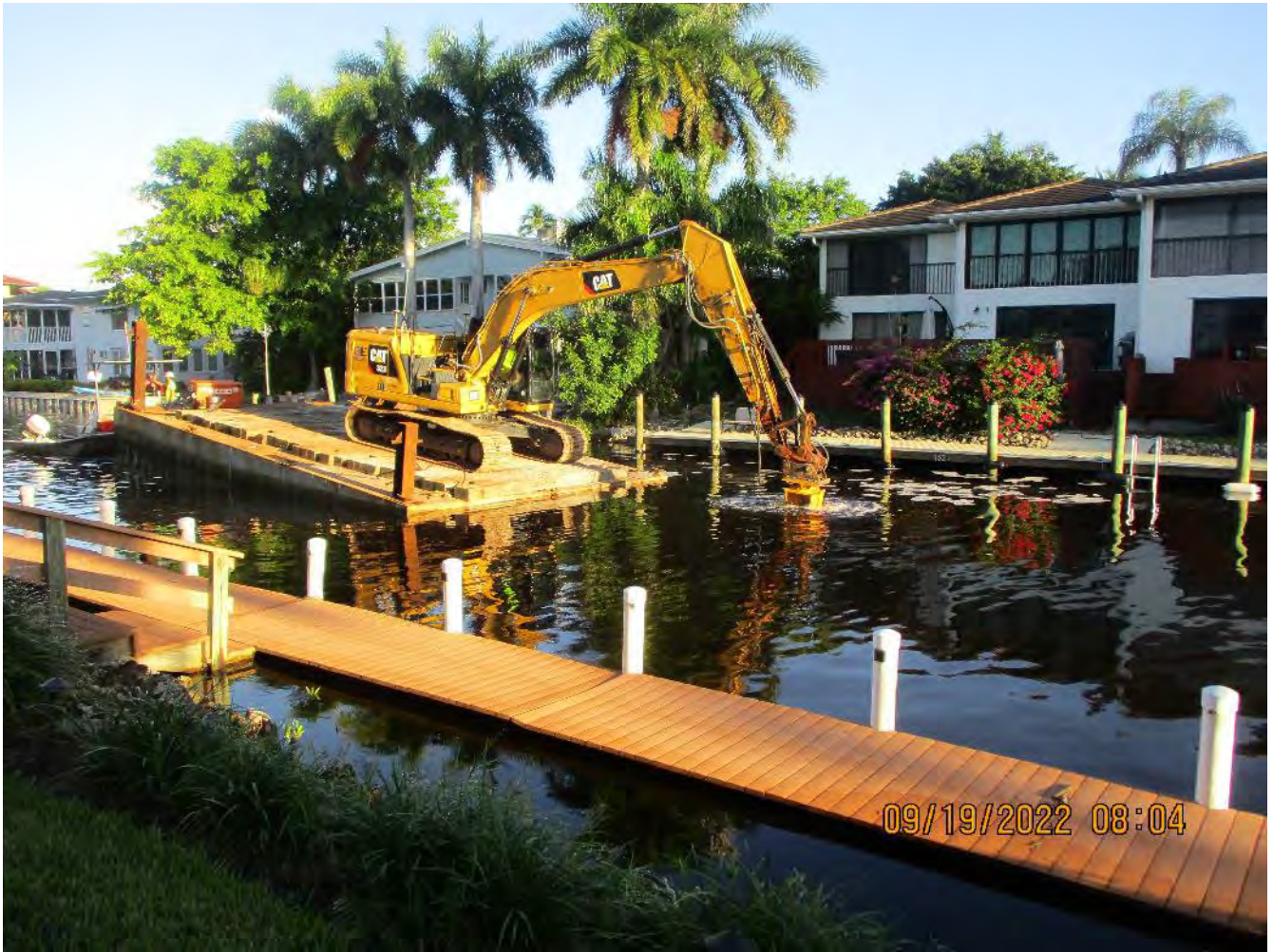
Start of today's canal bottom grinding (Canal W-W, approx. station 13+00)
