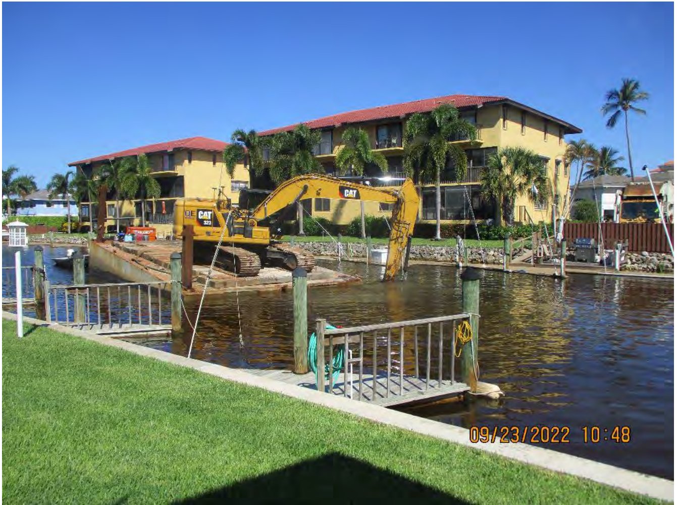
Canal W-W bottom grinding in progress (approx. station 9+60)
