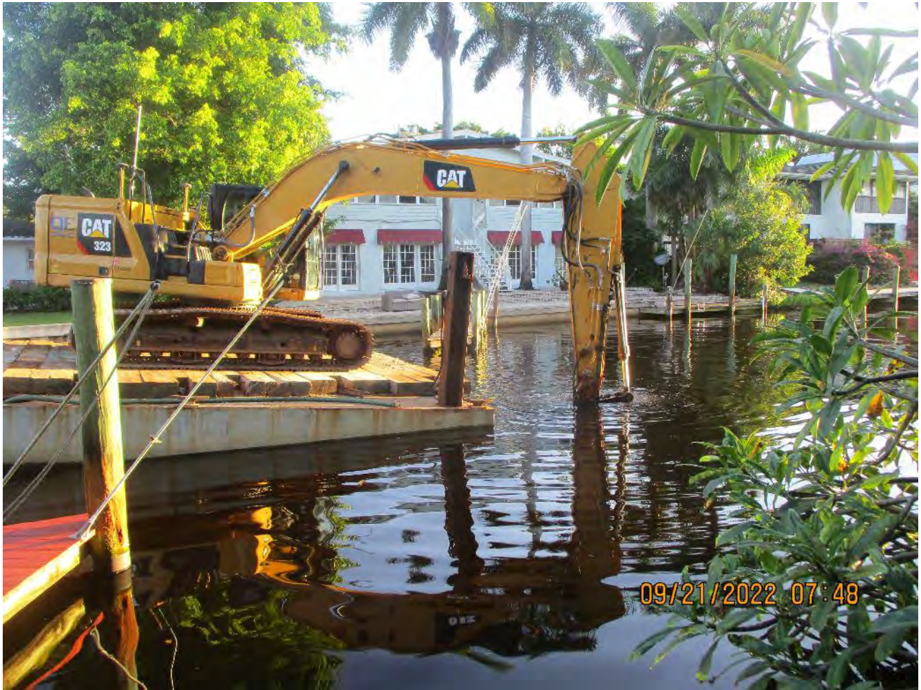
Start of canal bottom grinding (Canal W-W, approx. station 11+50)
