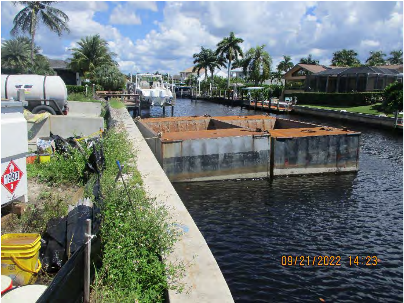
Staged hoppers (2) at Canal CC-CC approx. station 2+00 location
