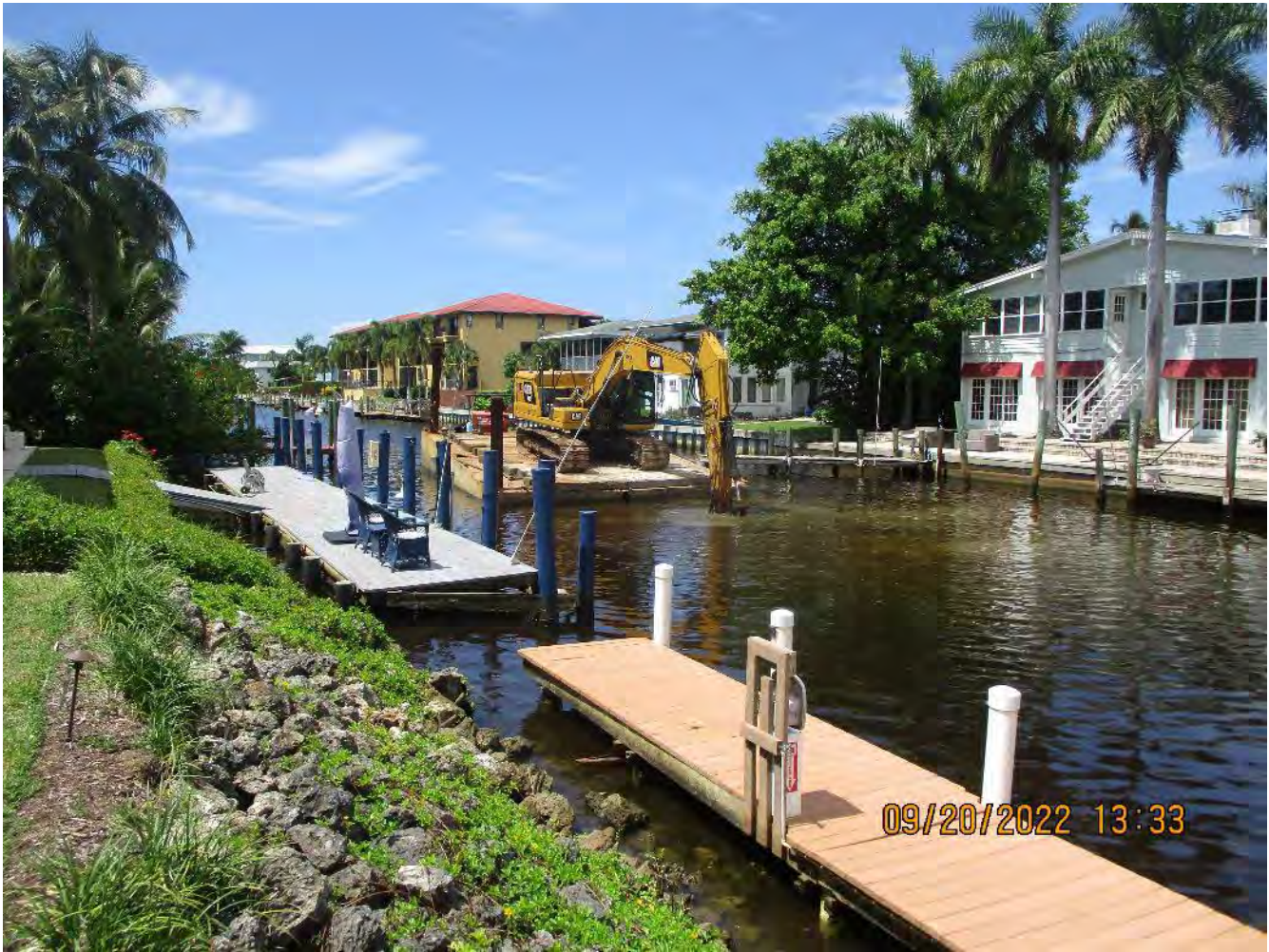
Canal W-W bottom grinding in progress (approx. sta. 12+00)
