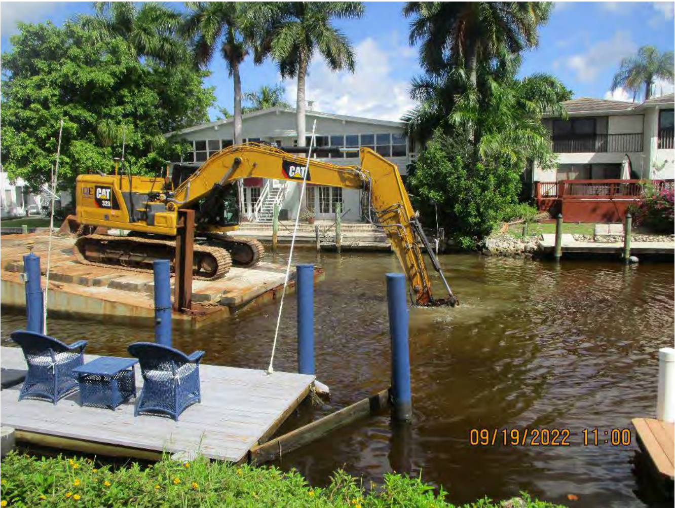
Canal W-W bottom grinding in progress (approx. station 12+50)
