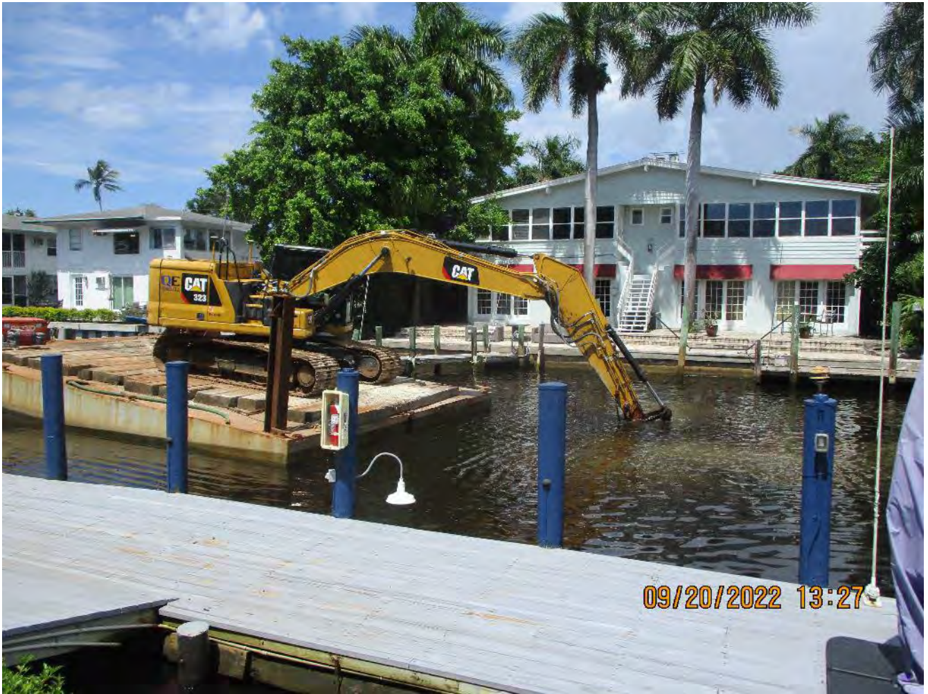
Canal W-W bottom grinding resumes at approx. station 12+00 (Canal W-W)
