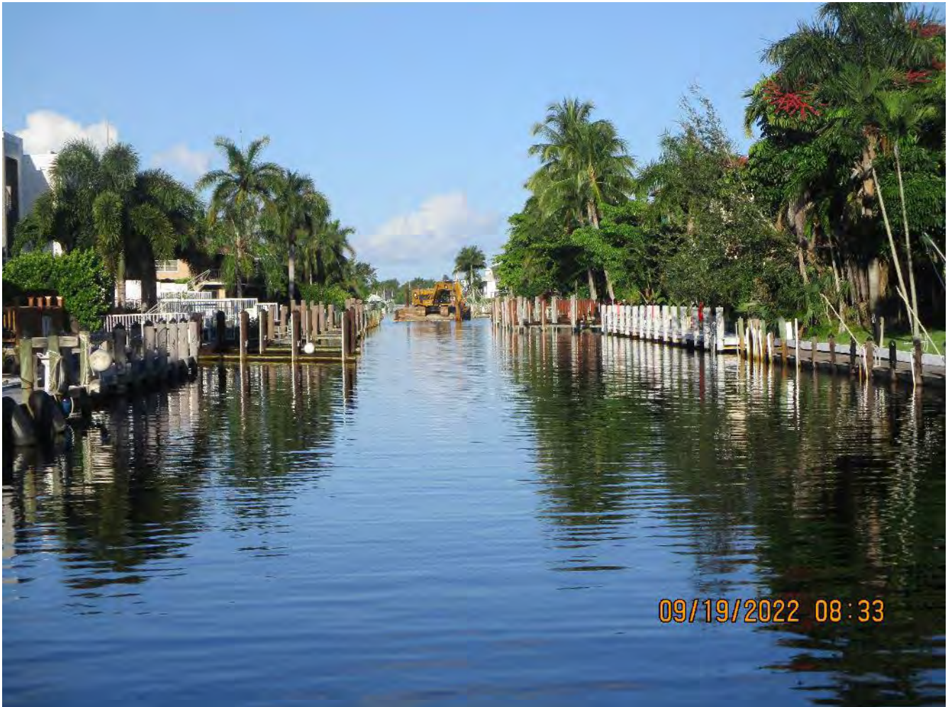
Canal bottom grinding at approx. station 13+00 (Canal W-W)
