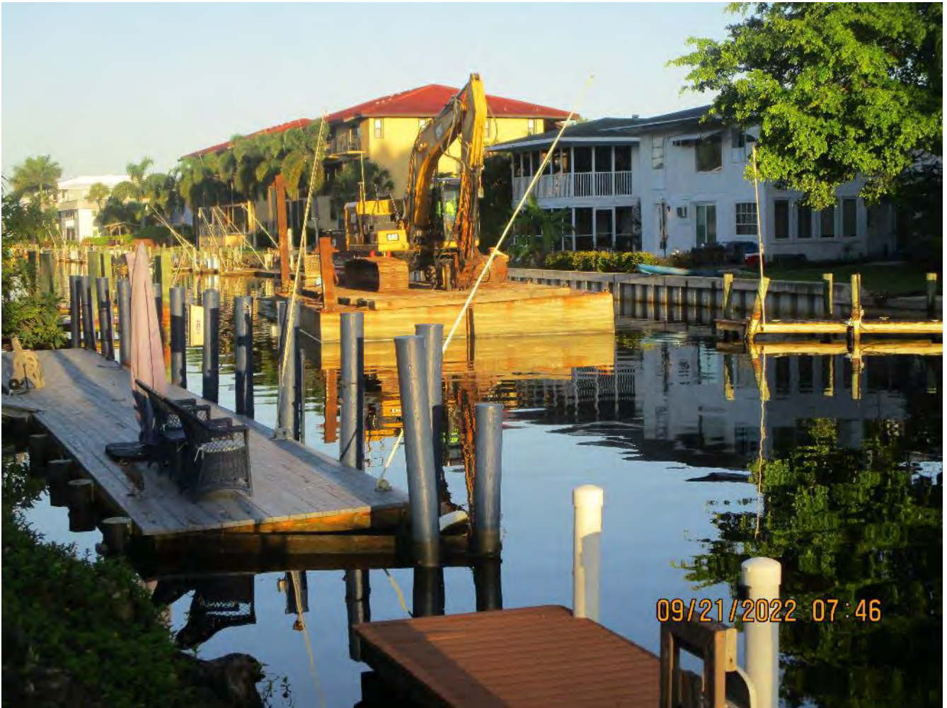
Barge/excavator/push boat staged at approx. station 11+50 (Canal W-W)
