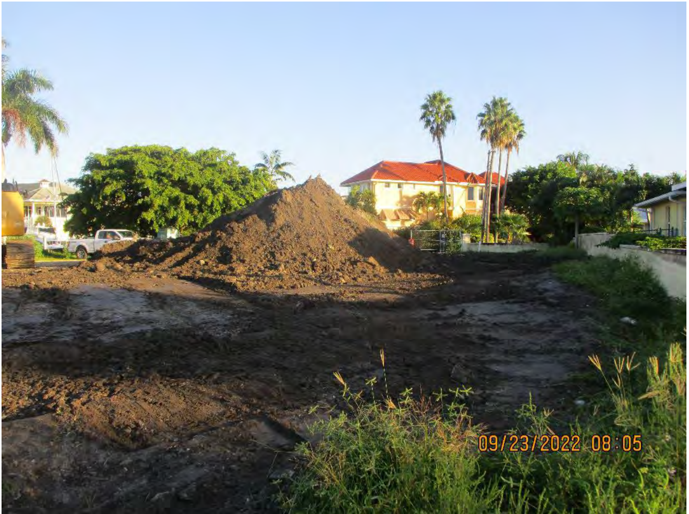
Current status of 1300 Curlew Ave project stockpile area
