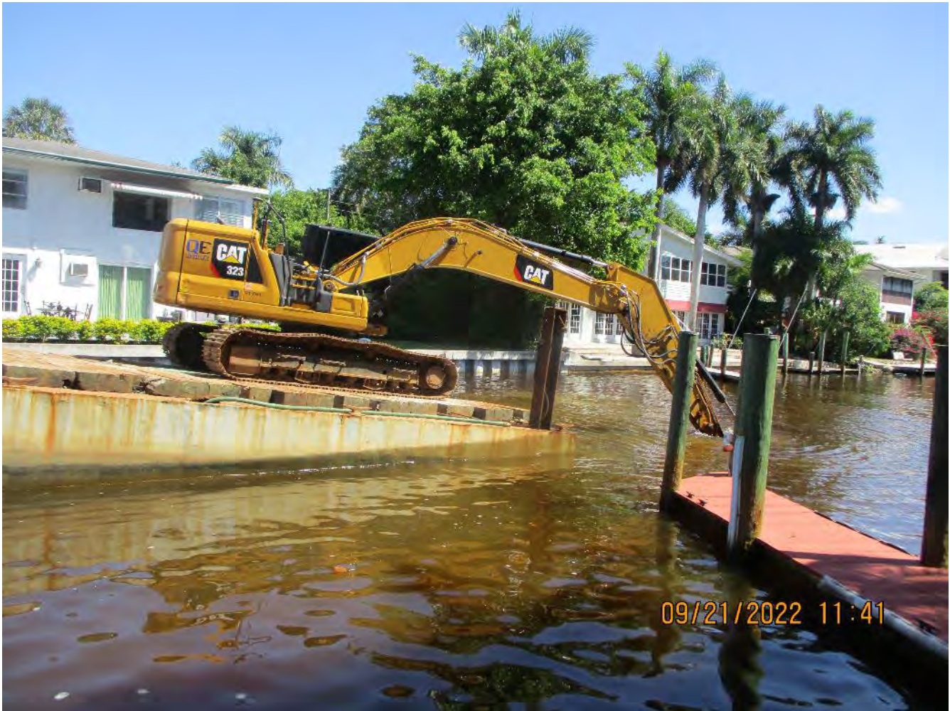
Canal W-W bottom grinding in progress (approx. station 11+25)
