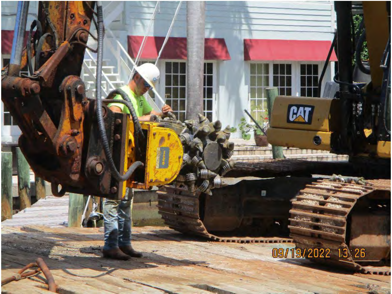
Periodic grinding drum/teeth maintenance in progress
