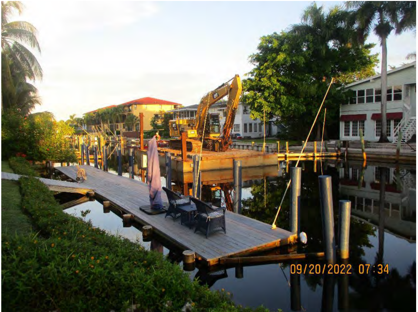
Barge/excavator/push boat staged at approx. station 12+00 (Canal W-W)
