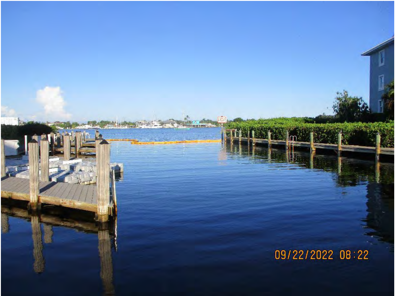
Turbidity curtain in place at mouth of Canal W-W
