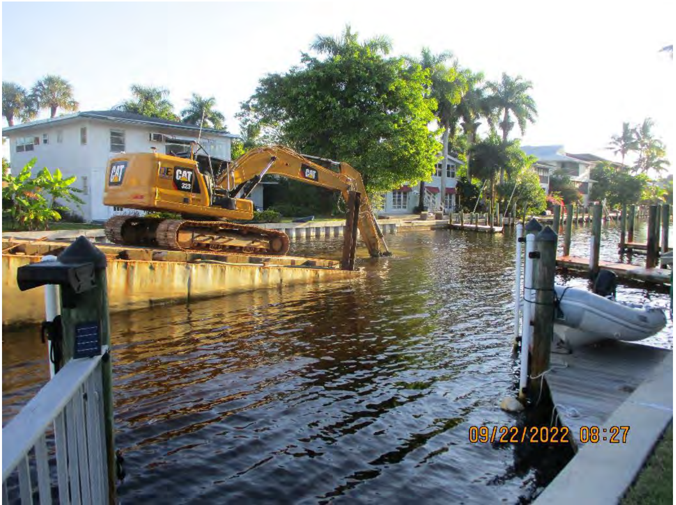
Start of canal bottom grinding (Canal W-W, approx. station 10+75)
