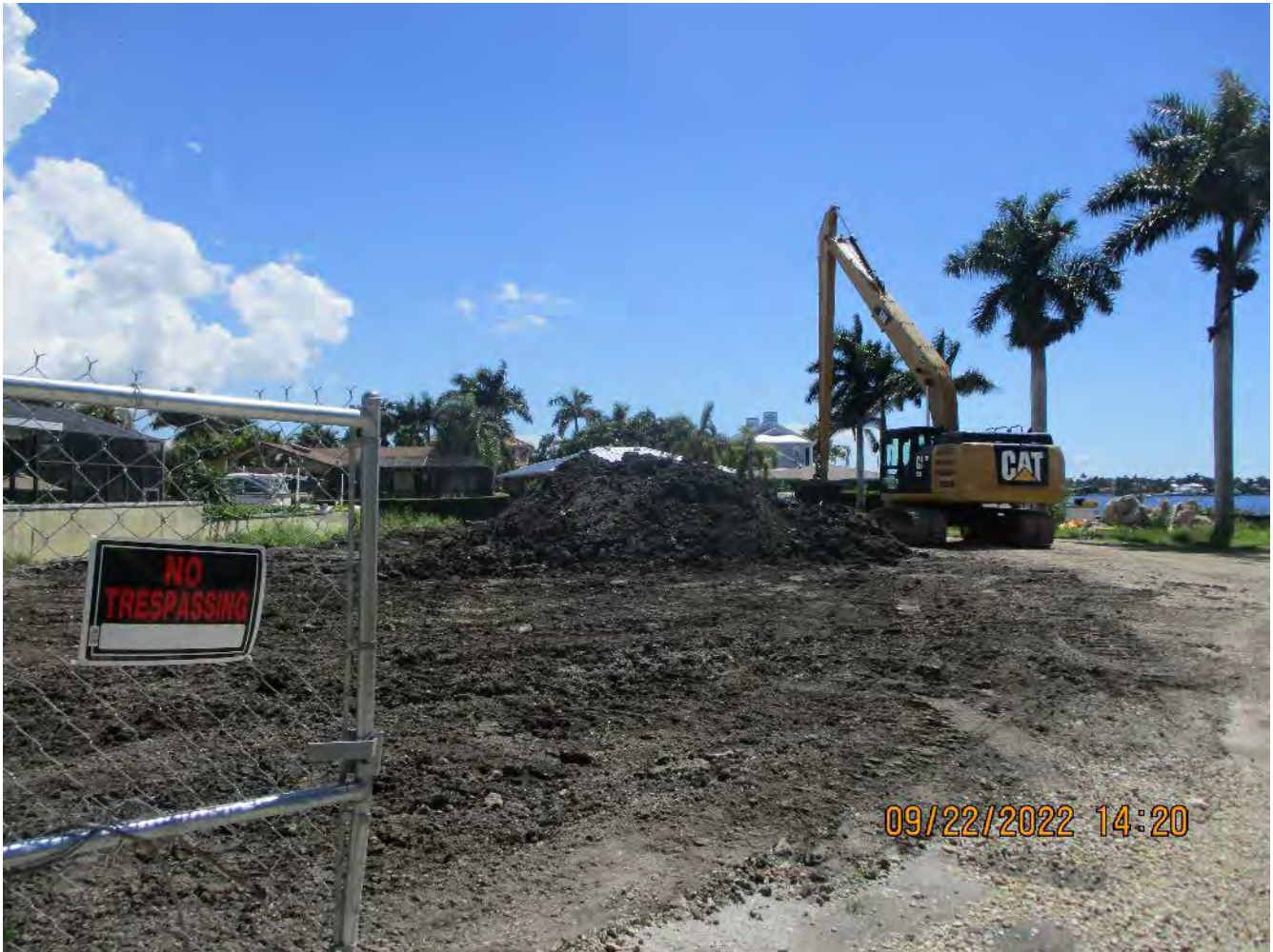
Current status of project 1300 Curlew Ave. staging/stockpile area
