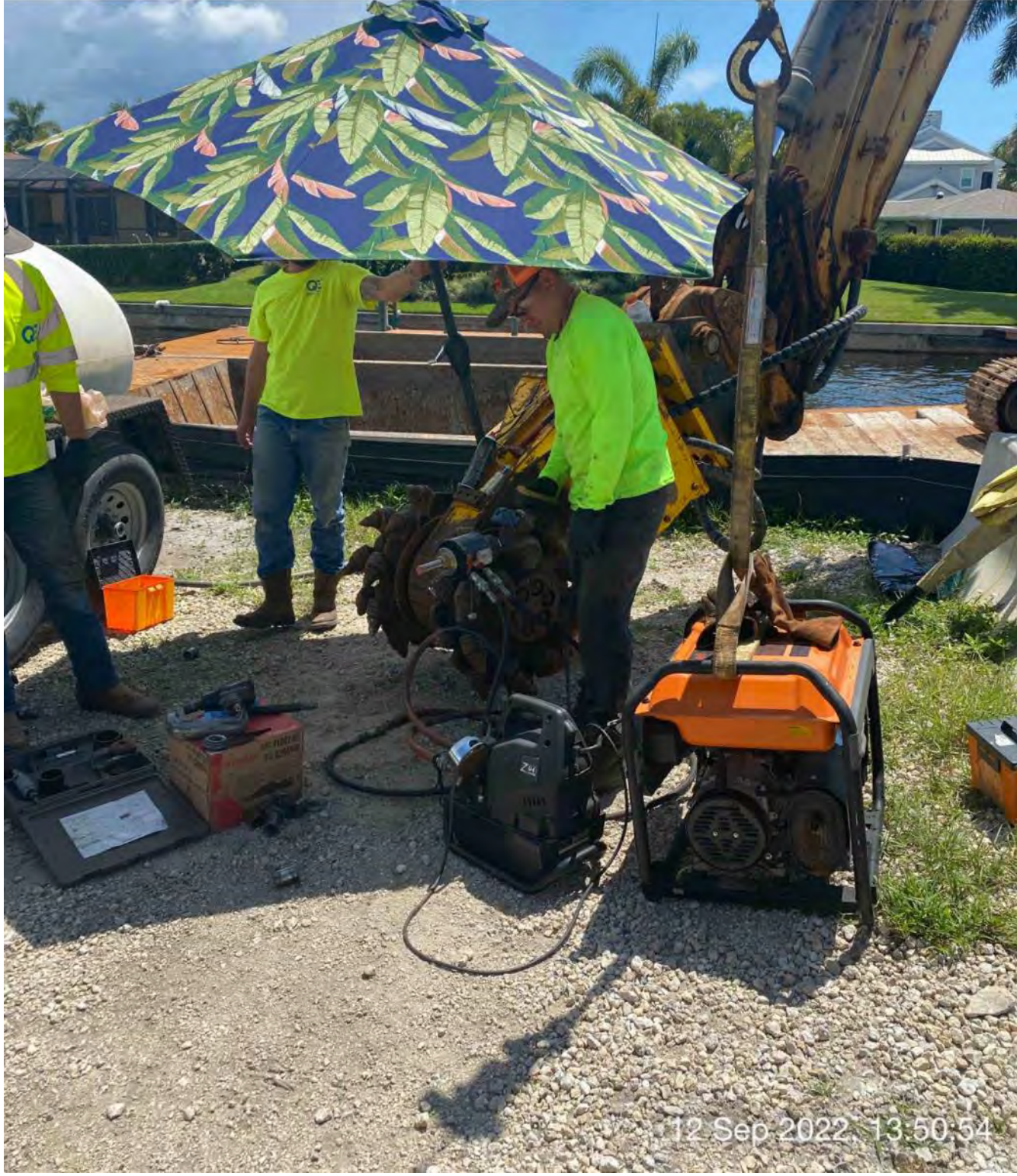
Mechanic removing, fixing, and replacing teeth sleeves on Epiroc grinder
