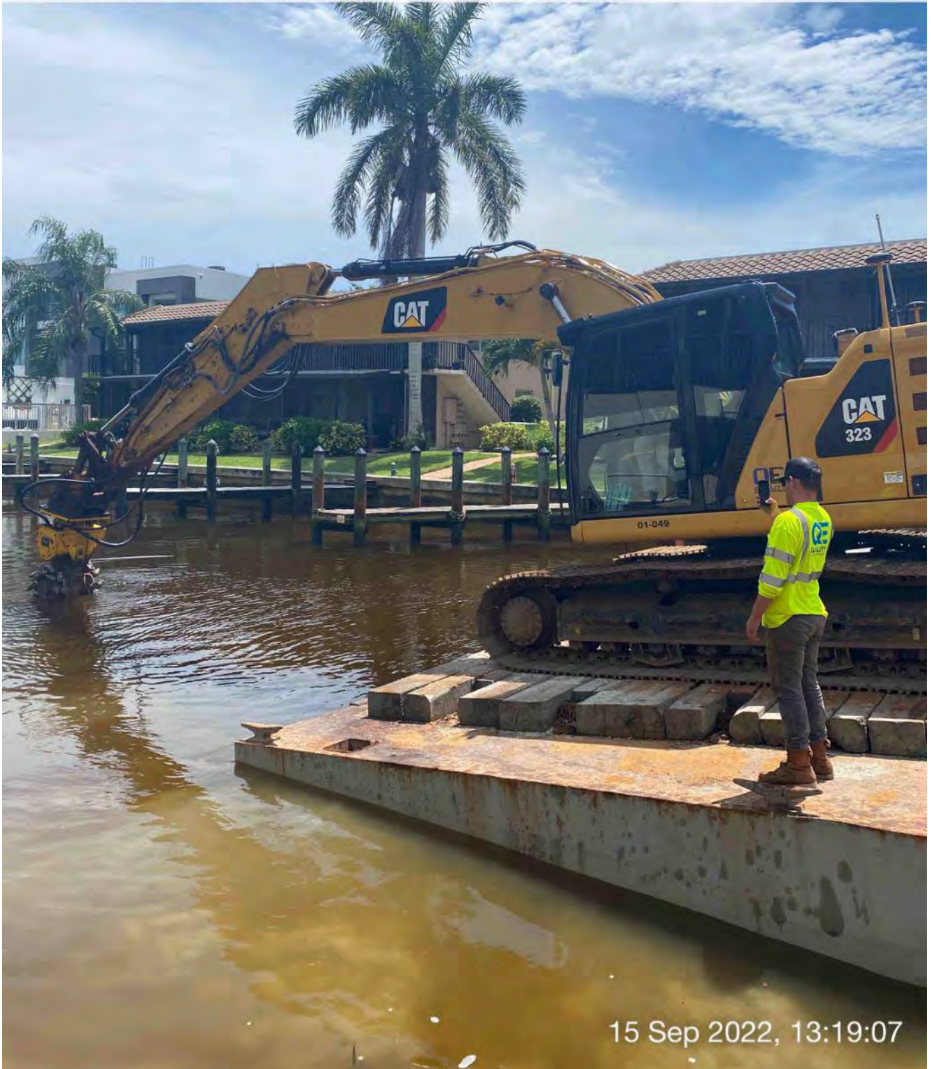
323 excavator grinding rock at station 13+50
