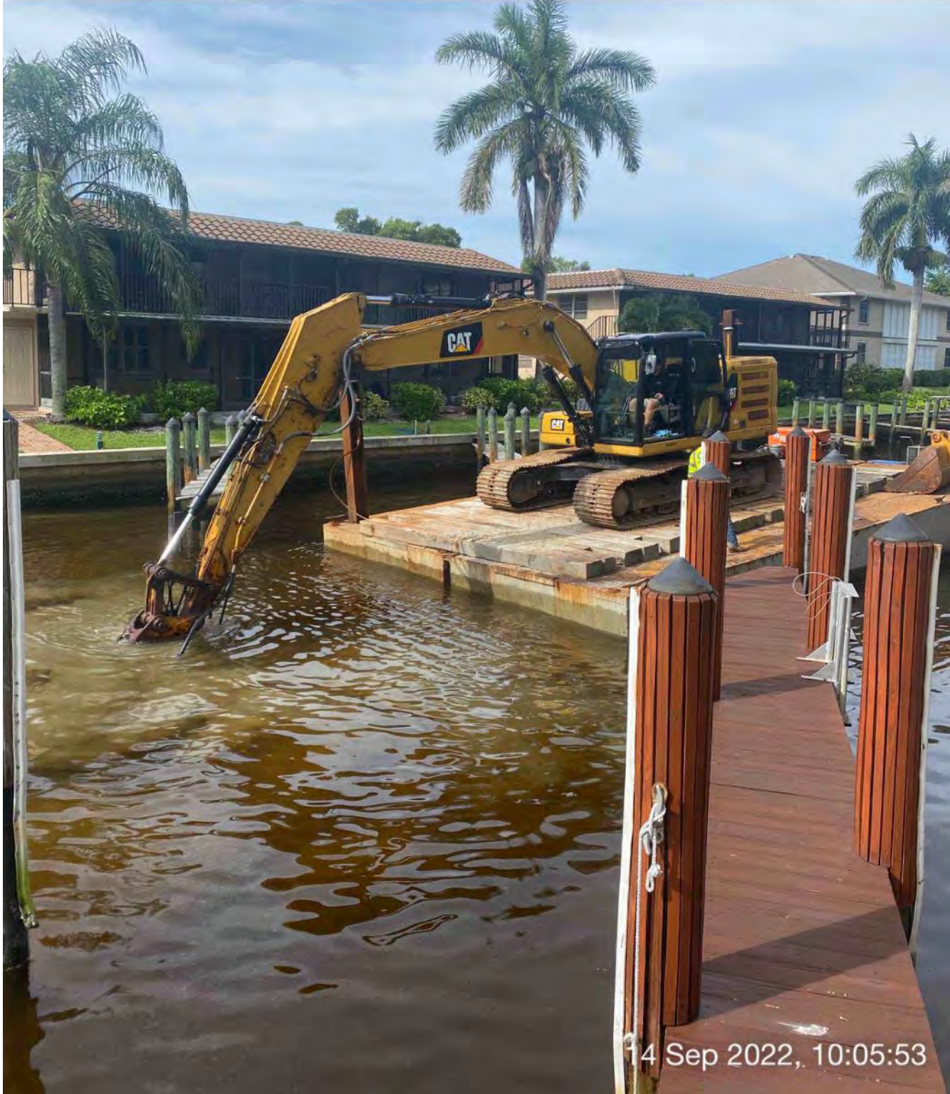
323 excavator grinding rock at station 14+75
