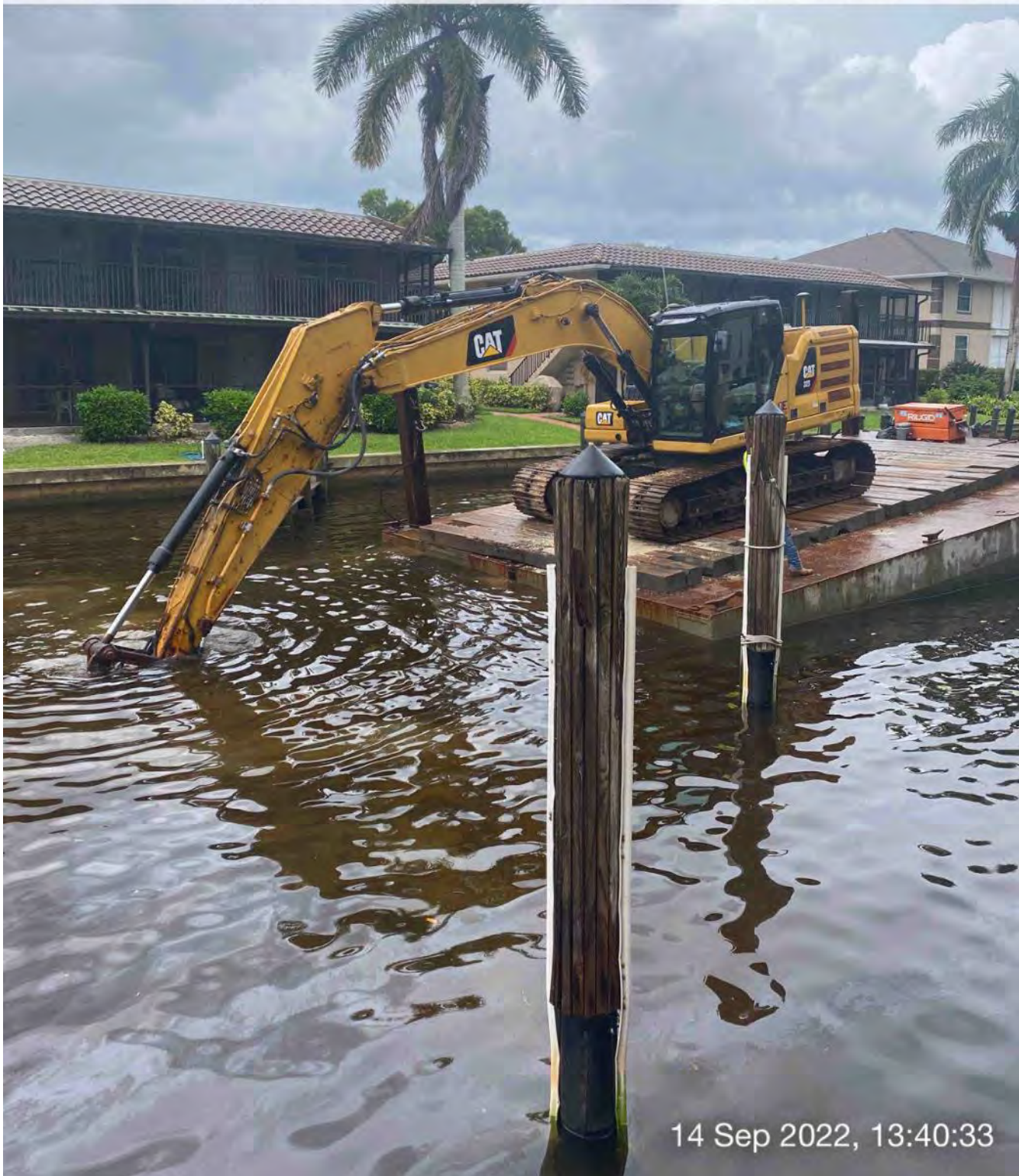
323 excavator grinding rock at station 14+25
