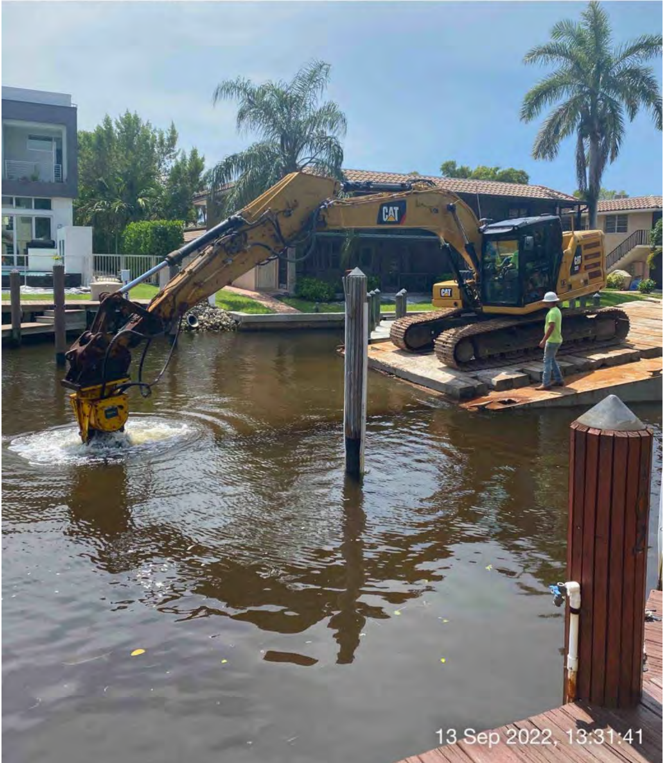
323 excavator grinding rock at station 14+75
