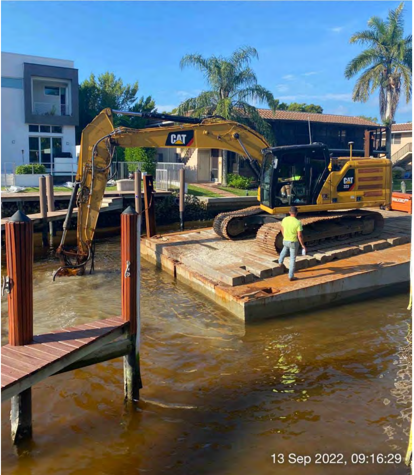
323 excavator grinding rock at station 15+25
