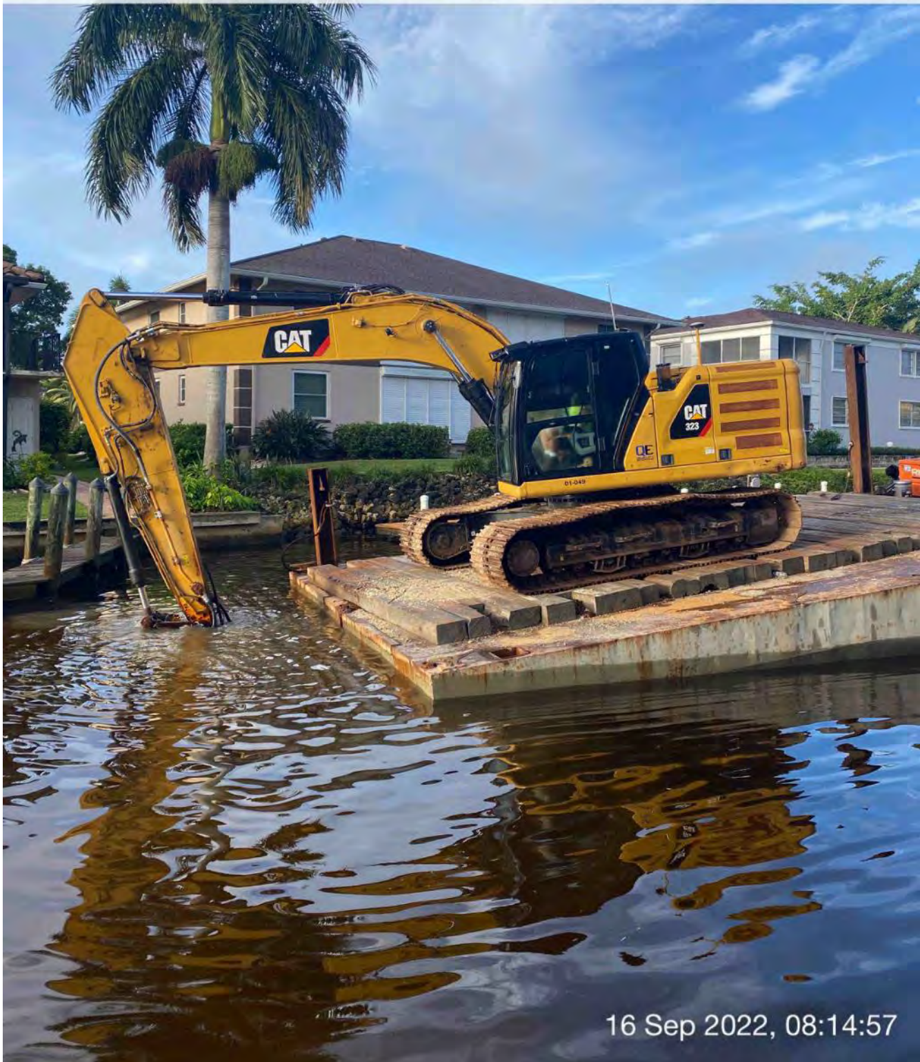
323 excavator grinding rock at station 13+25
