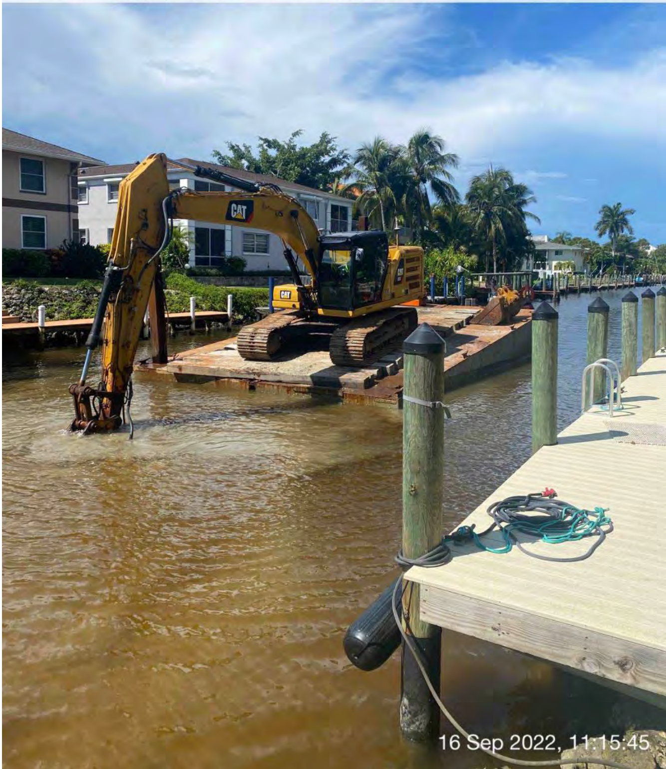
323 excavator grinding rock at station 13+00
