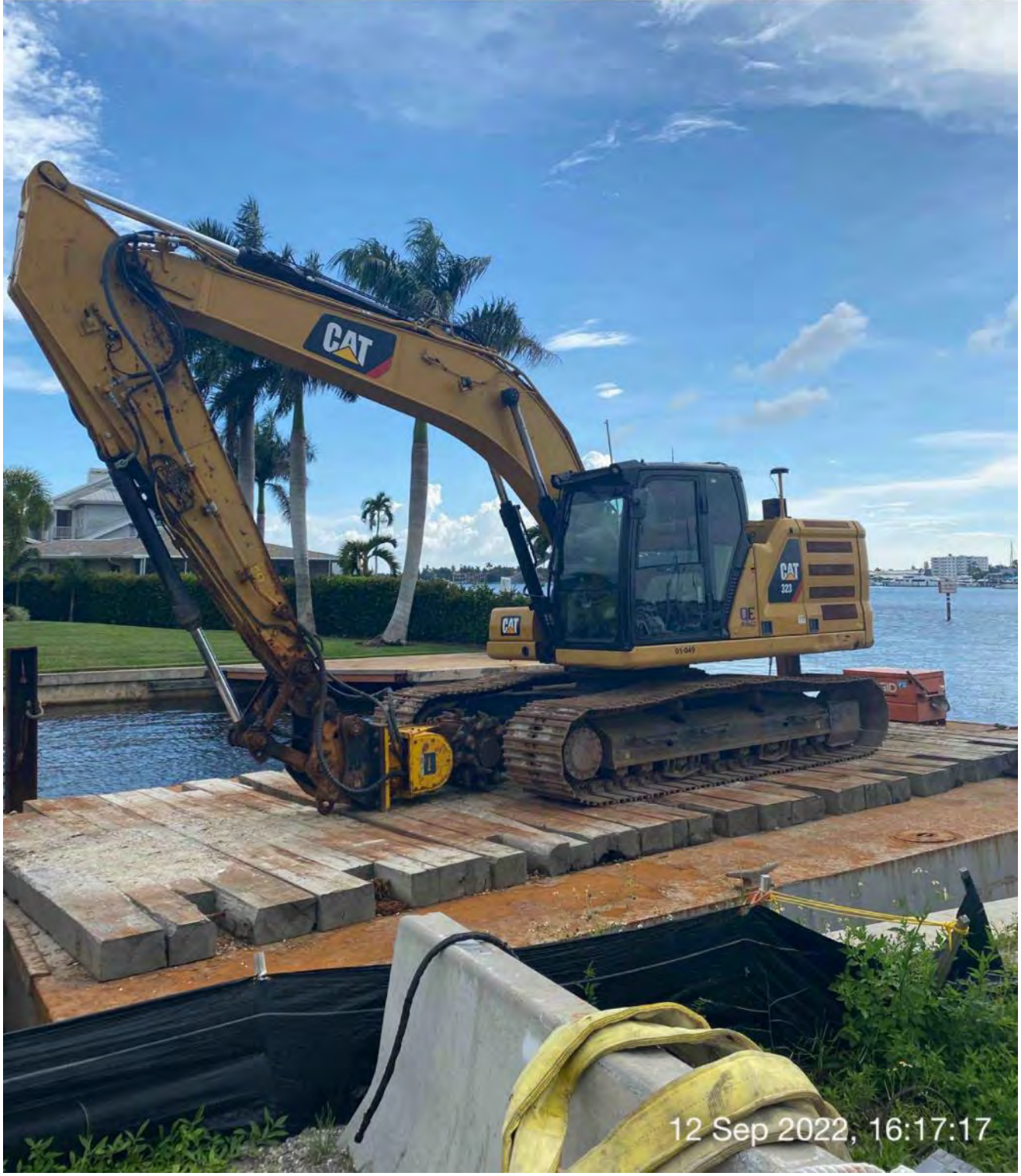
323 excavator on barge at station 1+00 in Canal CC-CC
