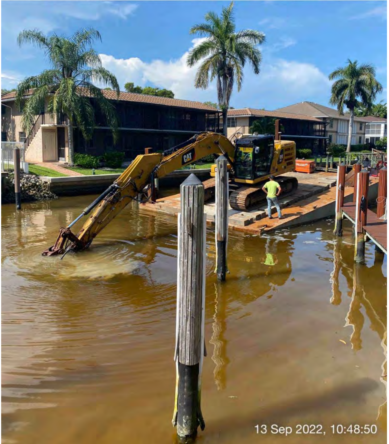
323 excavator grinding rock at station 15+00
