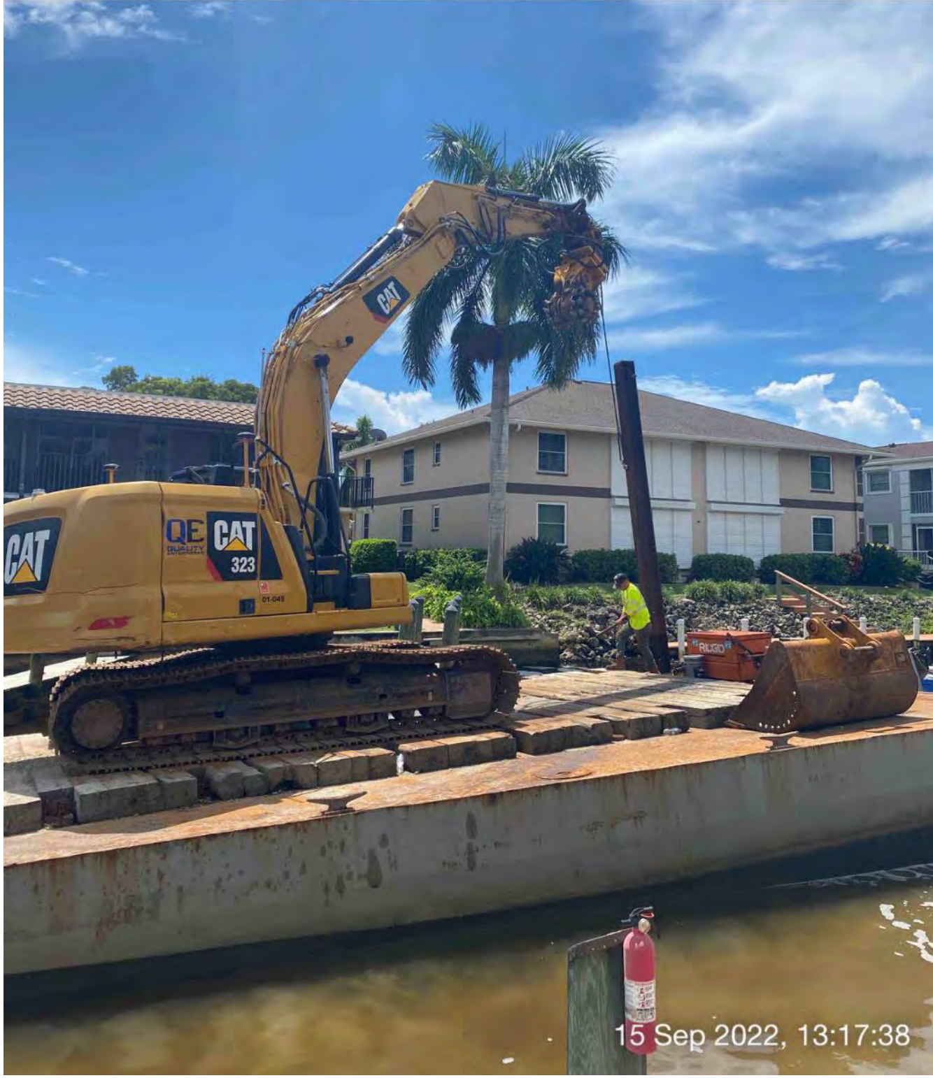
323 excavator lifting spud to allow push boat to mobilize barge at station 13+75
