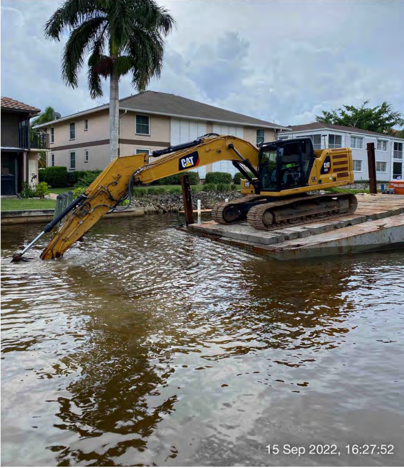
323 excavator grinding rock at station 13+25
