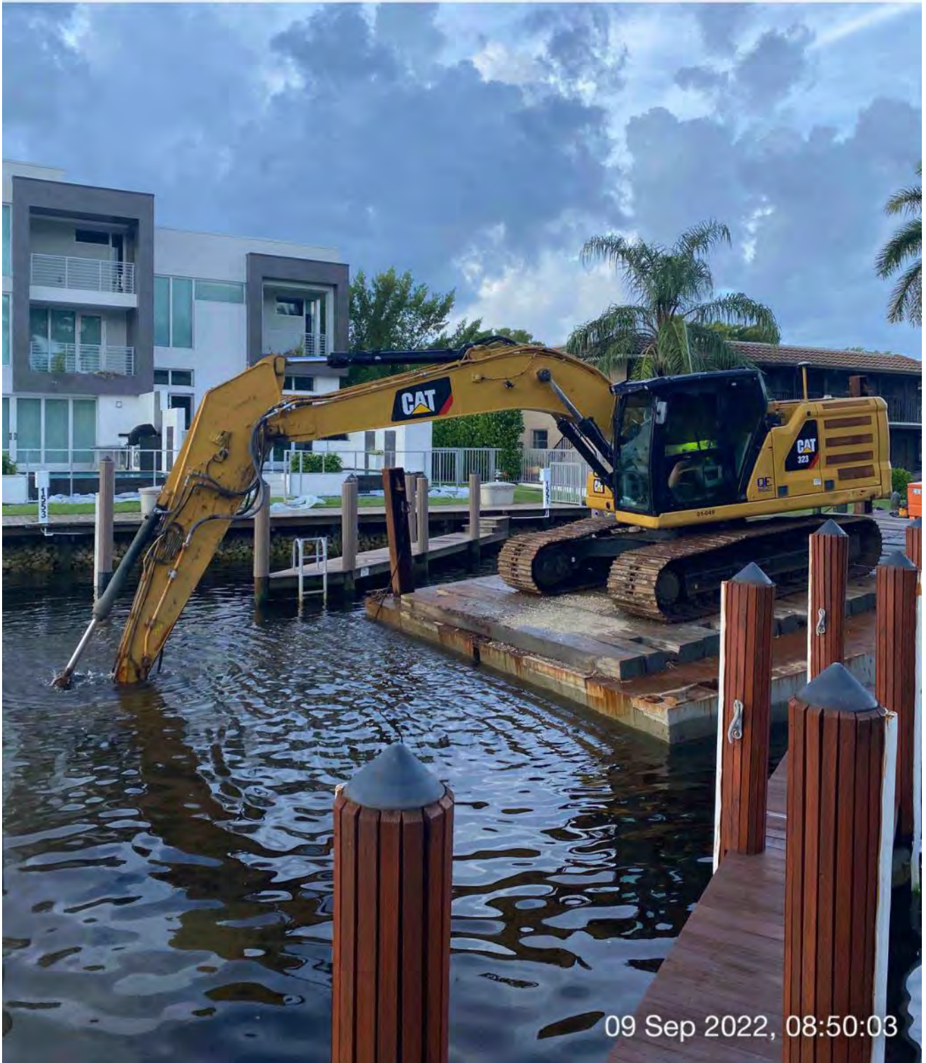
323 excavator grinding rock at station 15+50
