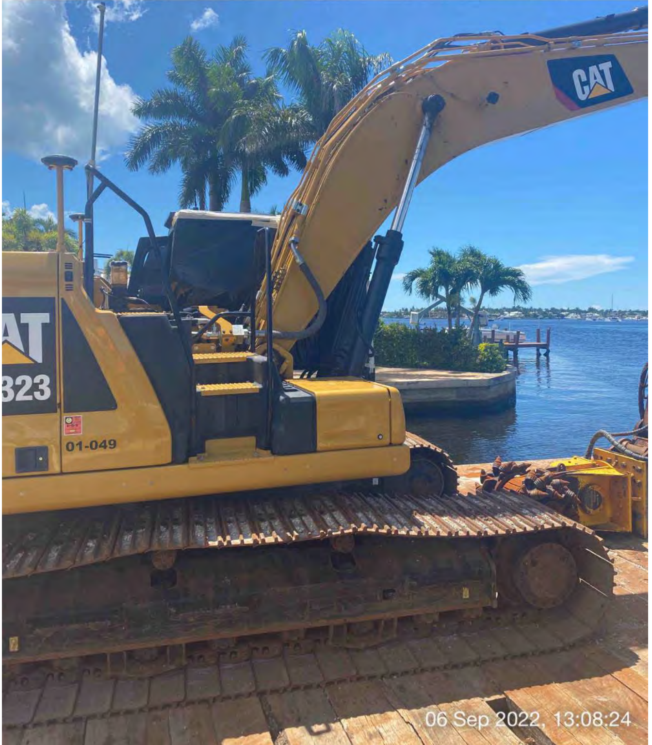
323 excavator on barge in Canal CC-CC at station 1+00
