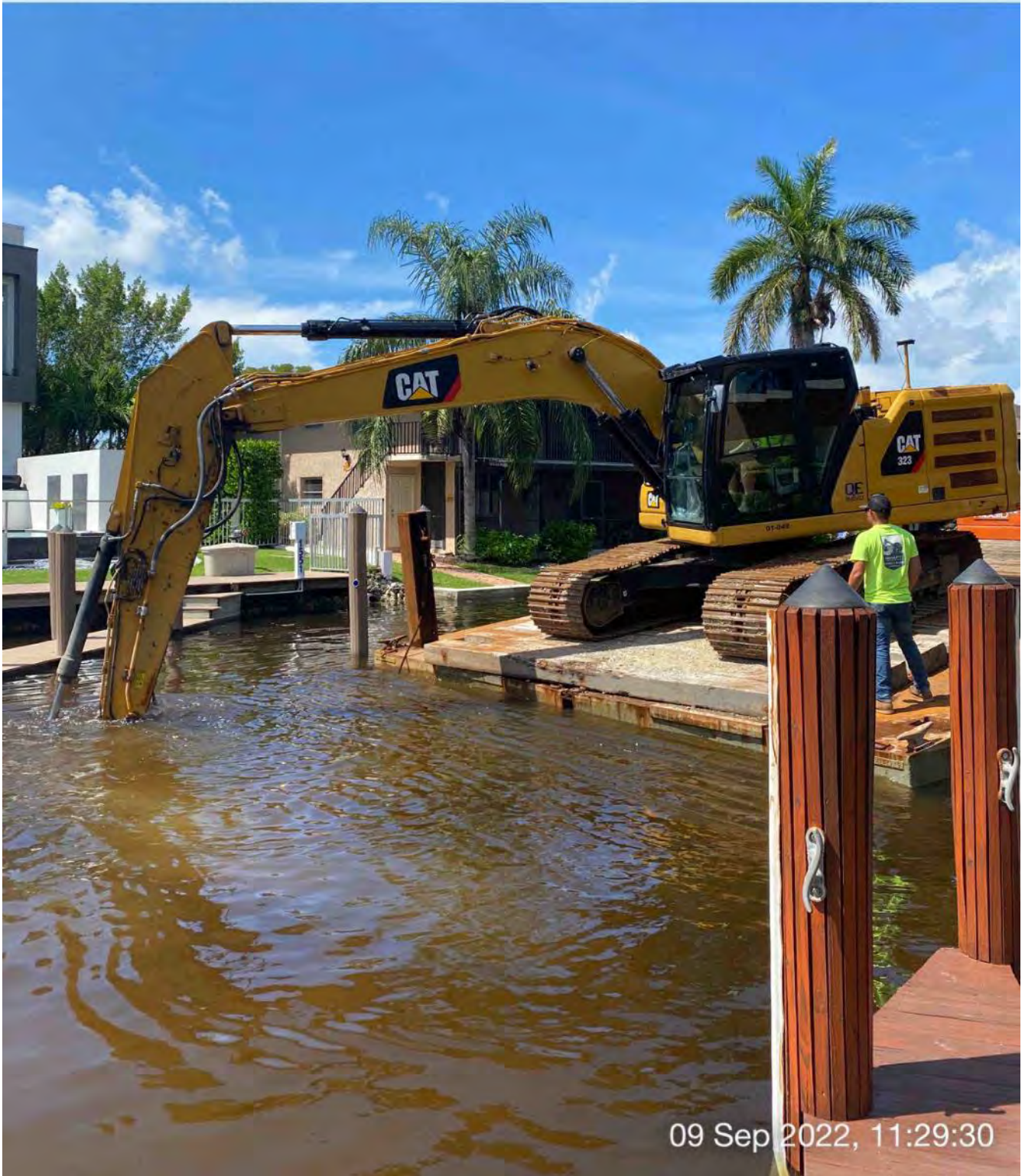
323 excavator grinding rock at station 15+00
