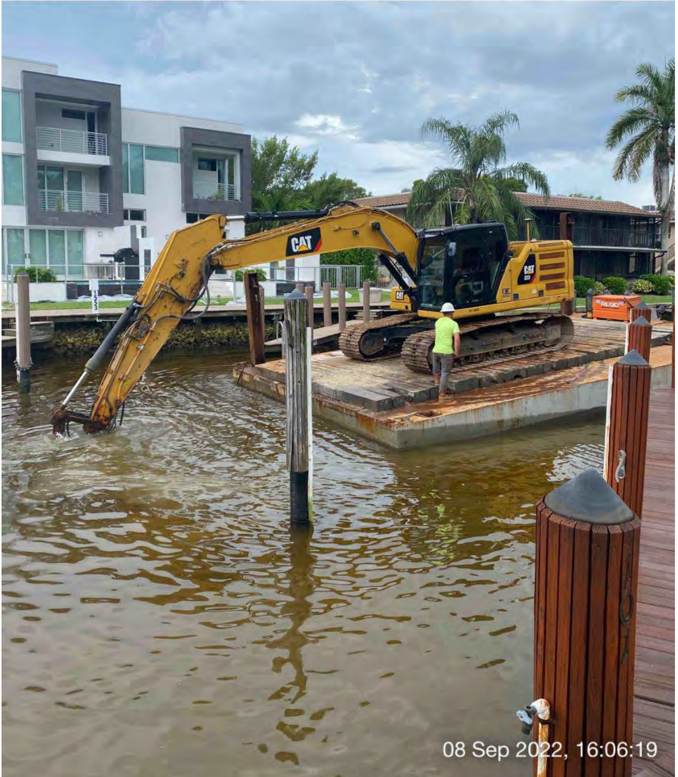
323 excavator grinding rock at station 15+50
