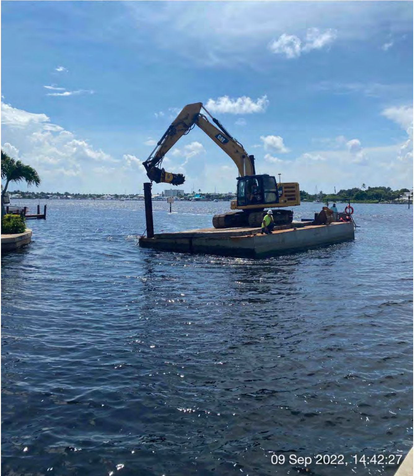
Push boat transporting 323 excavator and barge back to Canal CC-CC
