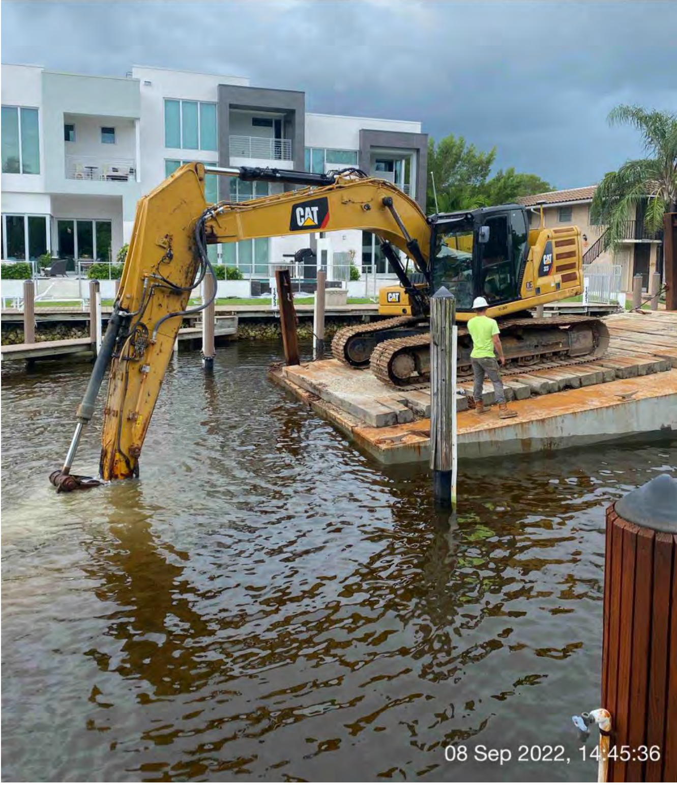
323 excavator grinding rock at station 16+00
