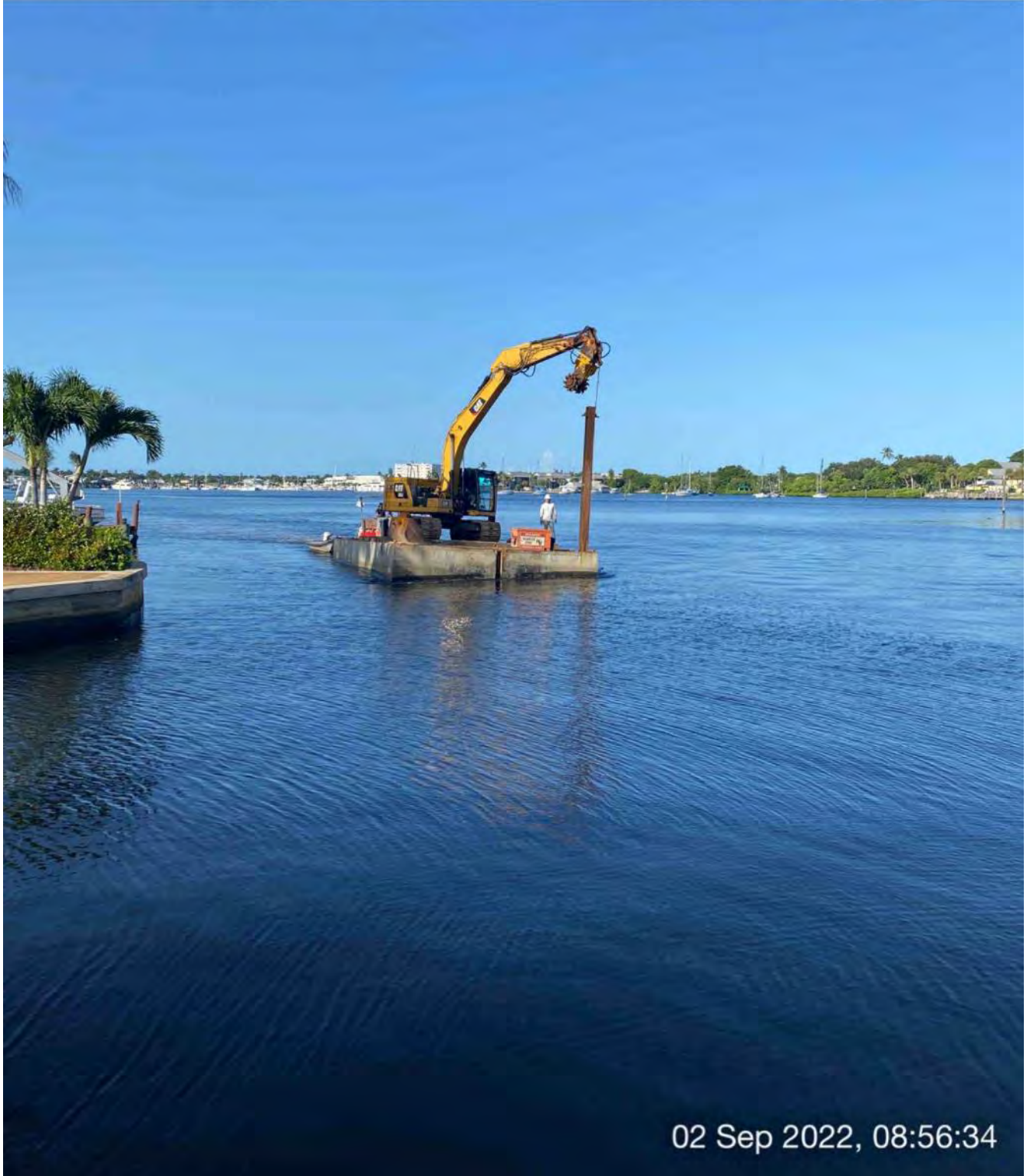
323 excavator lifting spud to allow push boat to transport barge from Canal W-W to Canal CC-CC
