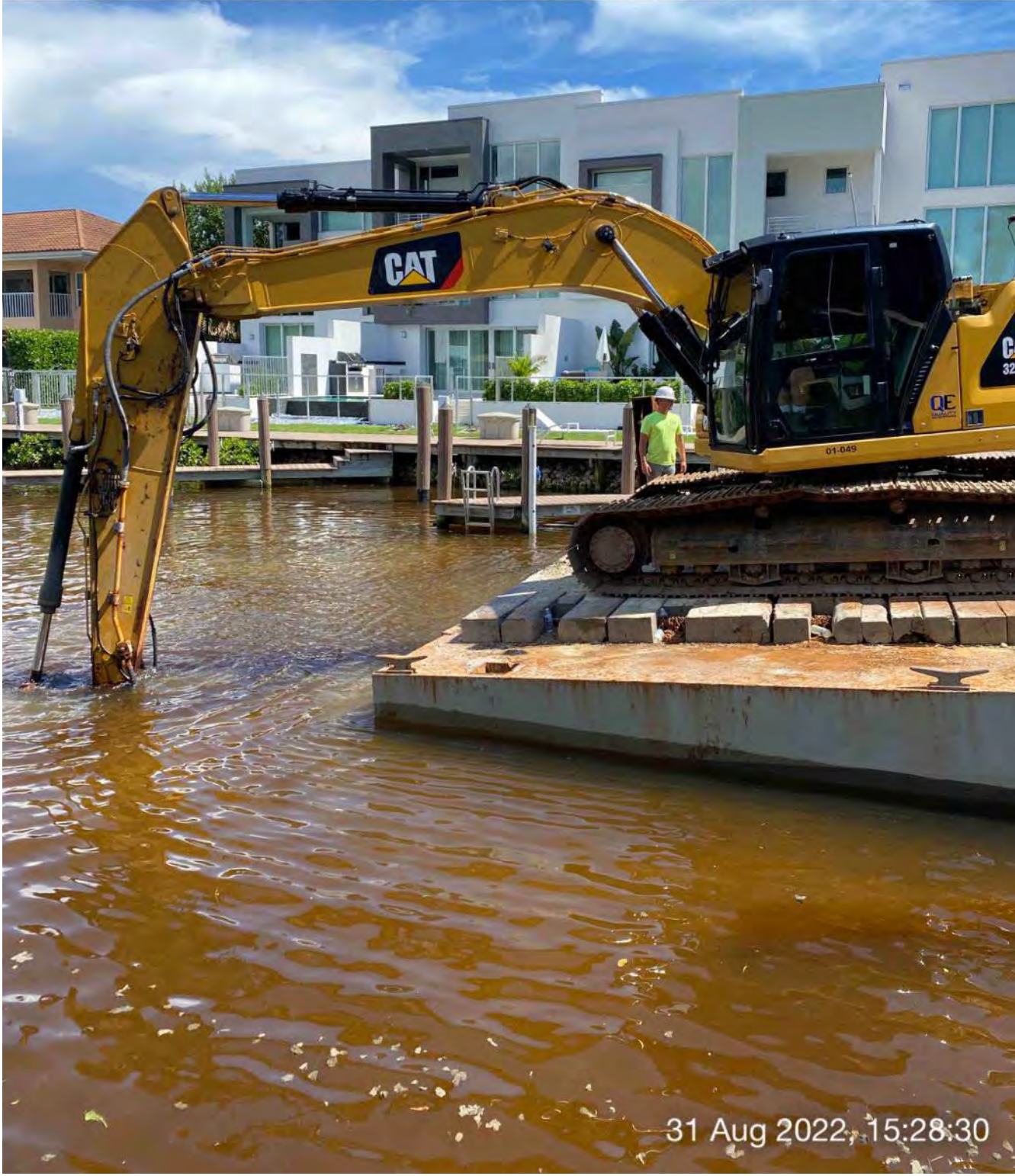
323 excavator grinding rock at station 15+75
