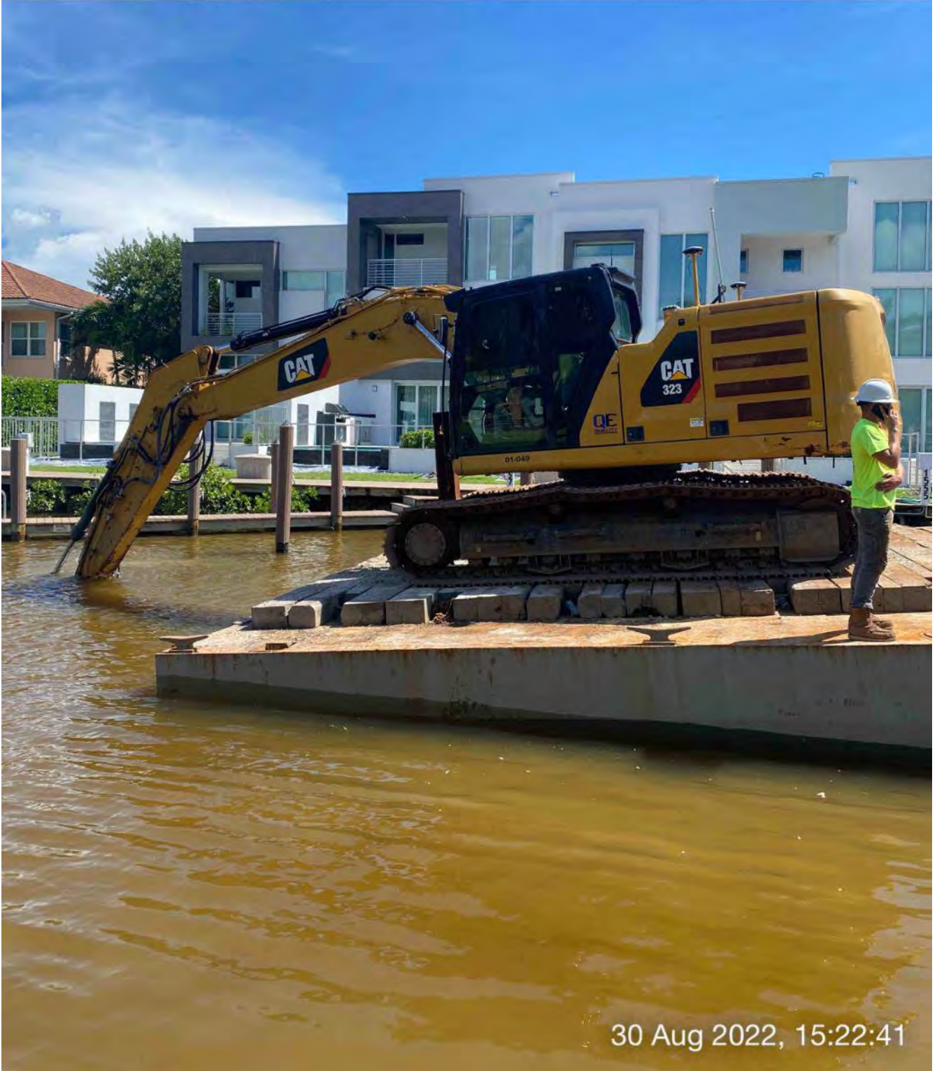
323 excavator grinding rock at station 16+00
