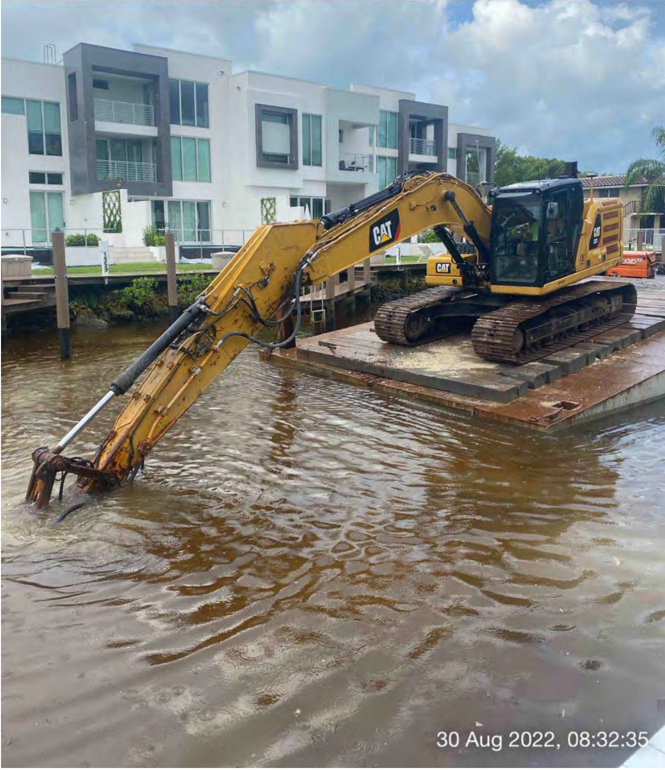
323 excavator grinding rock at station 16+50
