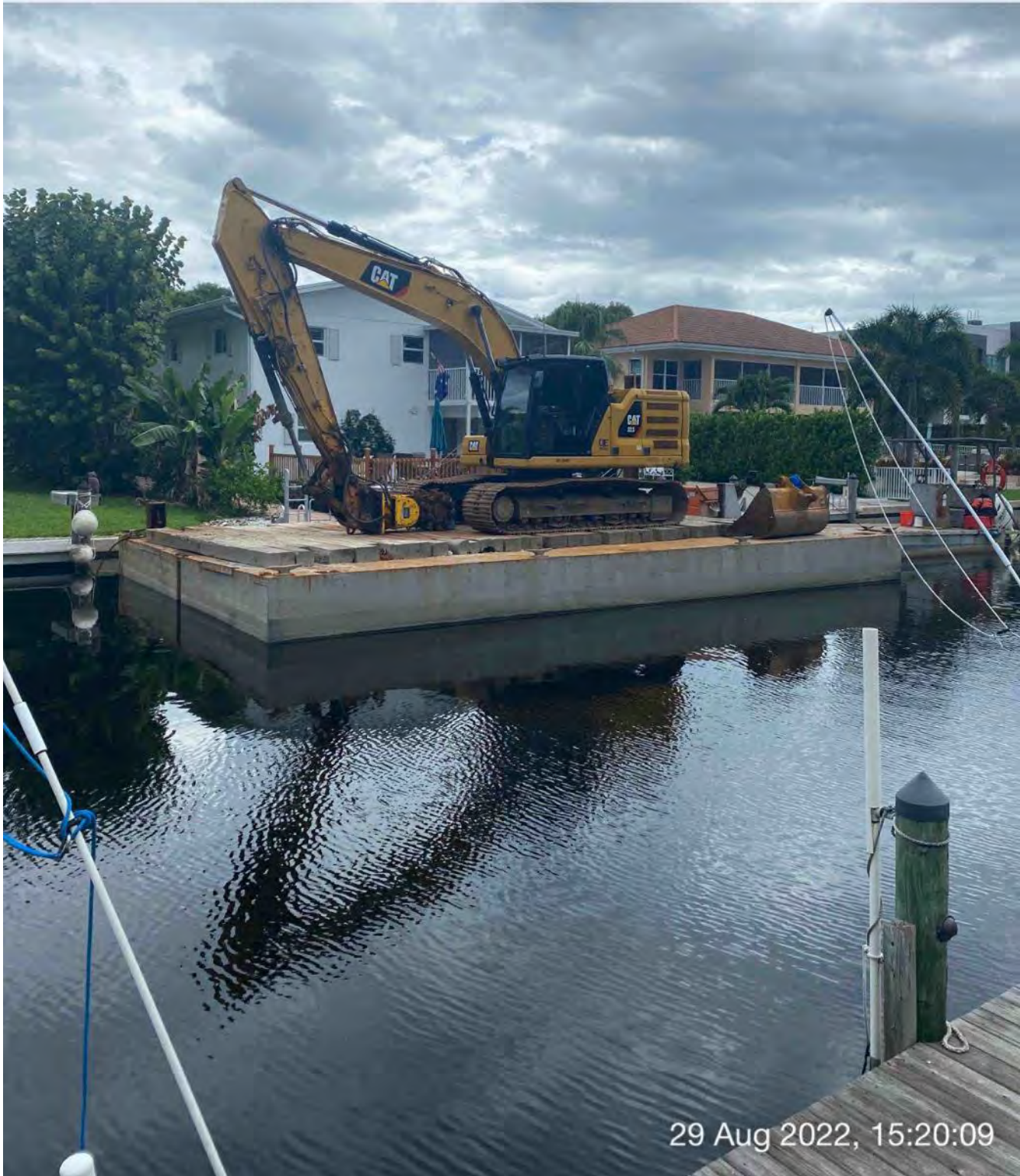
Barge, 323 excavator, and push boat at station 18+25 in Canal W-W
