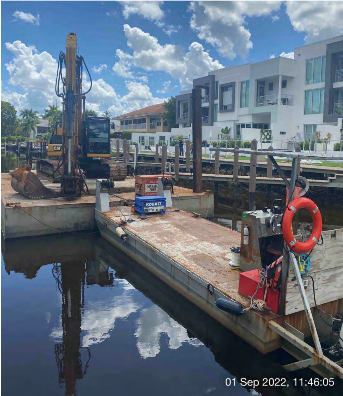
Barge, 323 excavator, and push boat staged in Canal W-W at station 16+00
