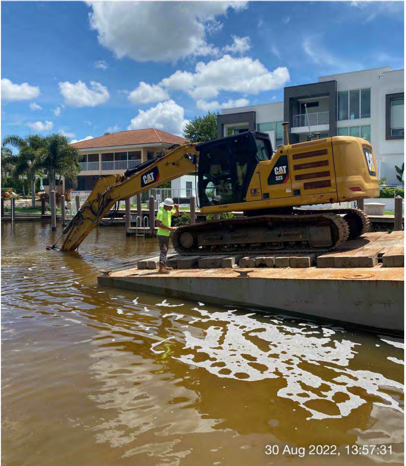
323 excavator grinding rock at station 16+00
