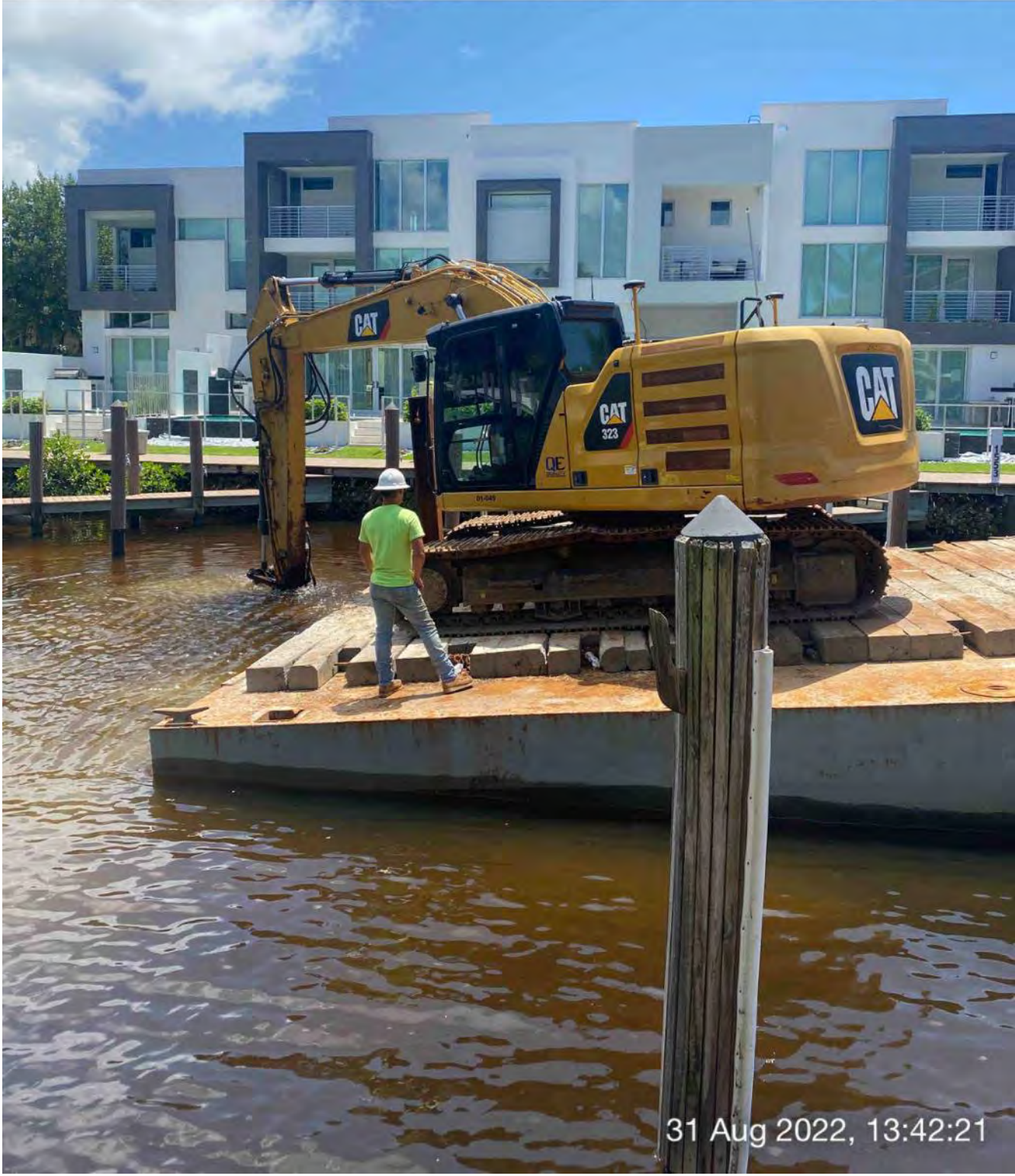
323 excavator grinding rock at station 16+00
