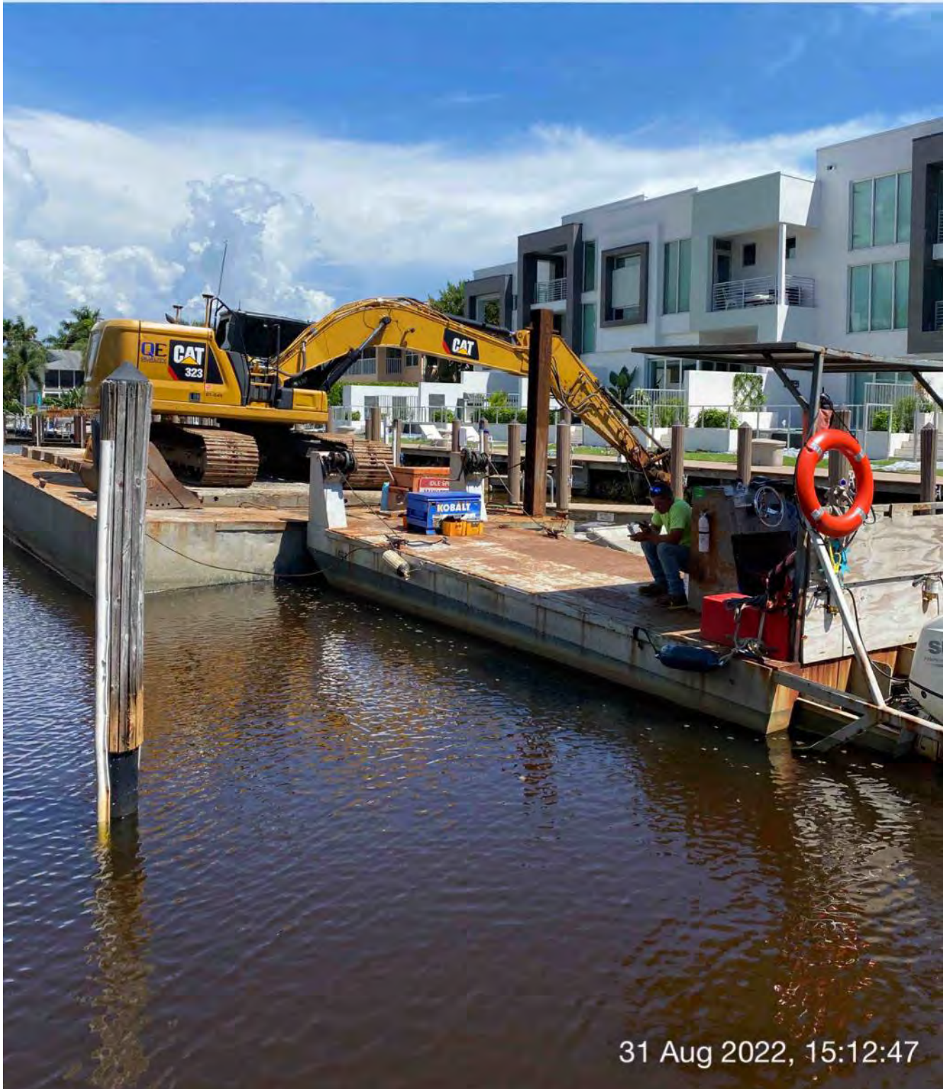
323 excavator tilting barge so that contractor can pump water out from bottom of barge
