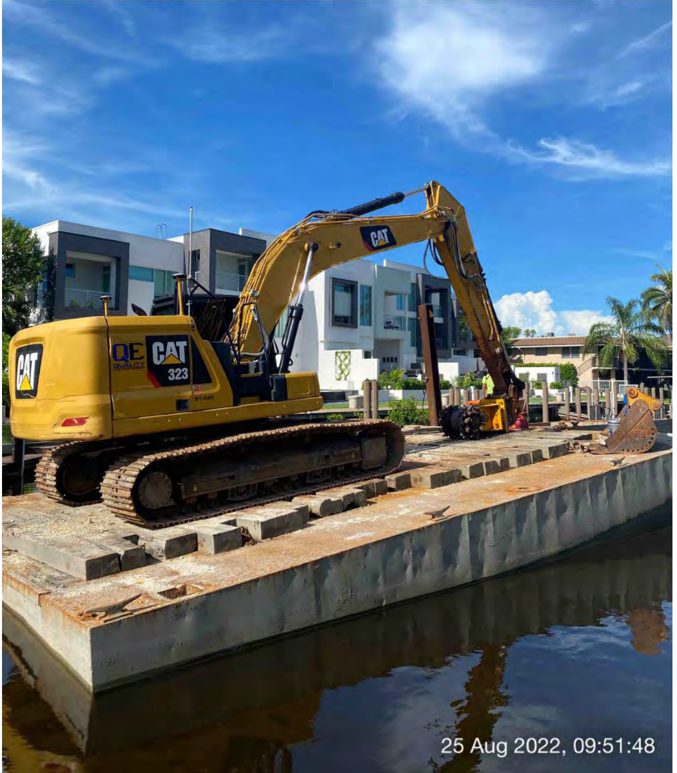
323 excavator and Epiroc grinder on barge at station 16+75
