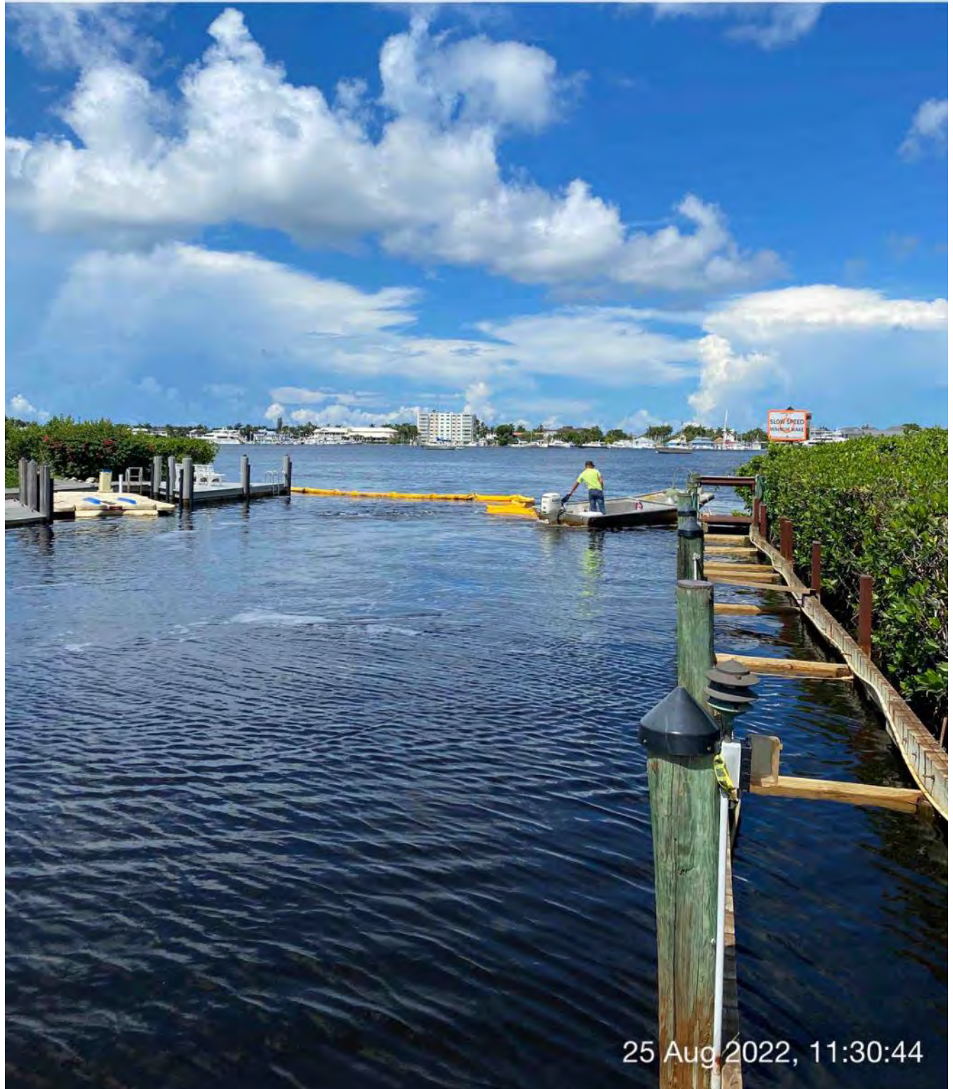
Contractor using support boat to install turbidity curtain across the mouth of Canal W-W
