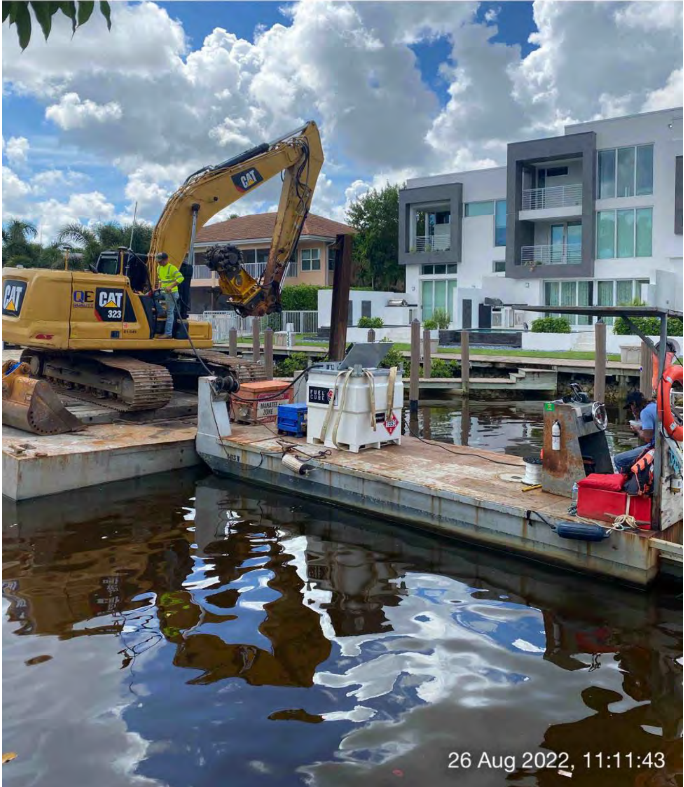
Contractor using small fuel cube to refuel 323 excavator at station 16+25
