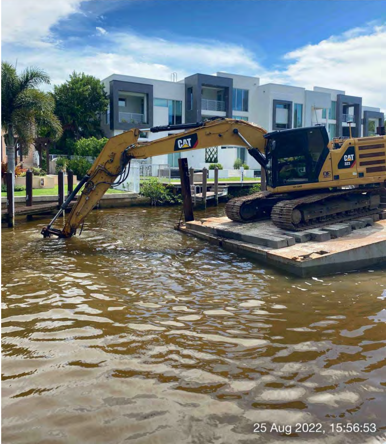
323 excavator grinding rock at station 16+50
