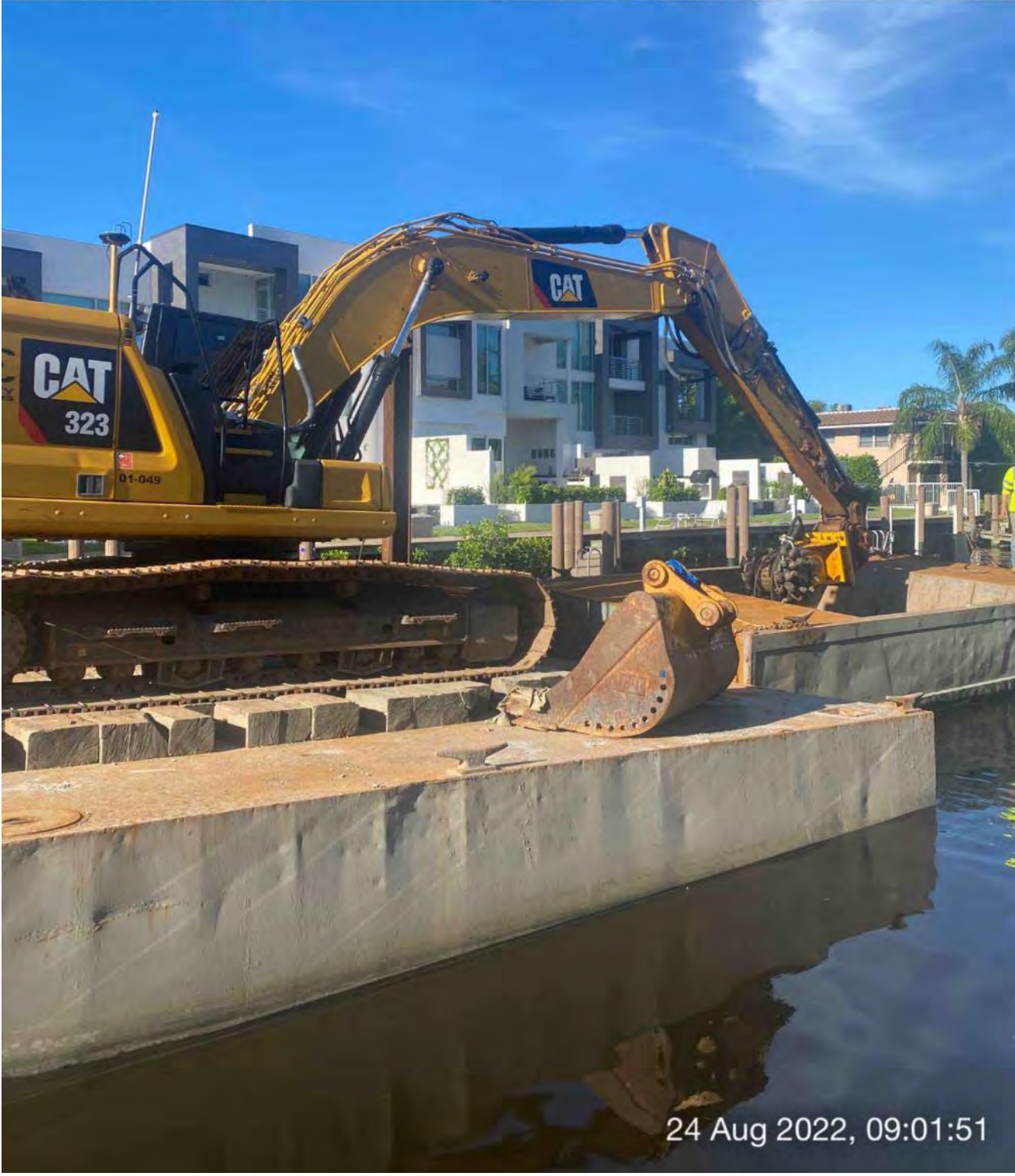
323 excavator placing Epiroc grinder in hopper in Canal W-W
