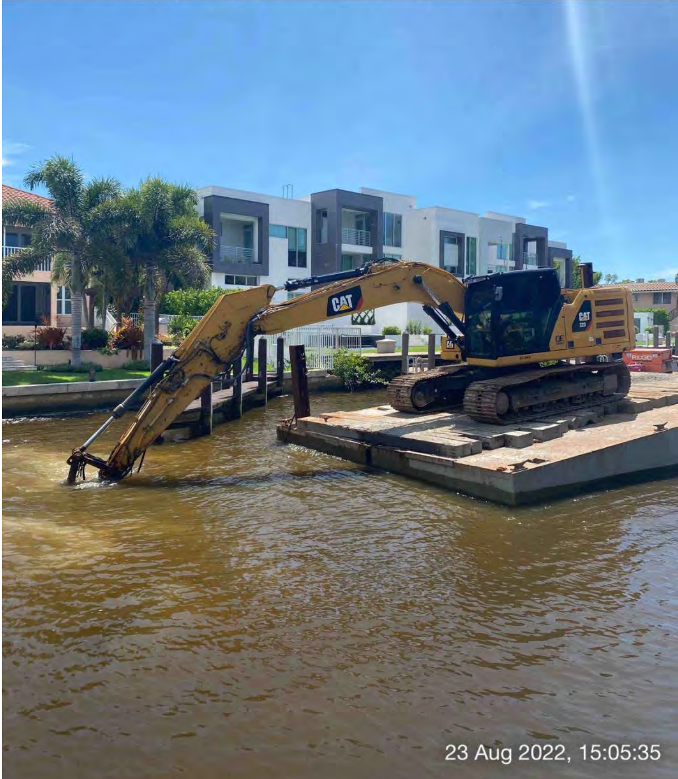
323 excavator grinding rock at station 16+75
