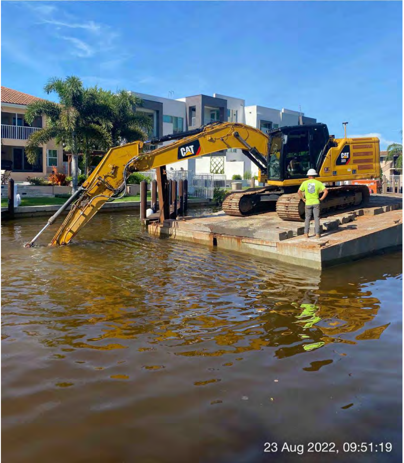
323 excavator grinding rock at station 17+00
