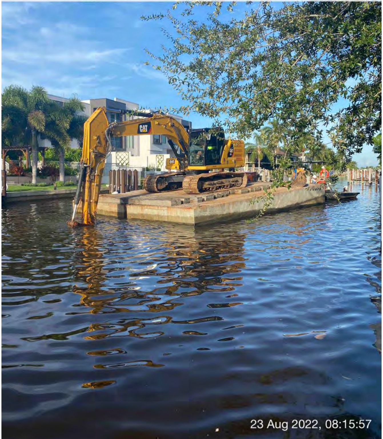
323 excavator grinding rock at station 17+00
