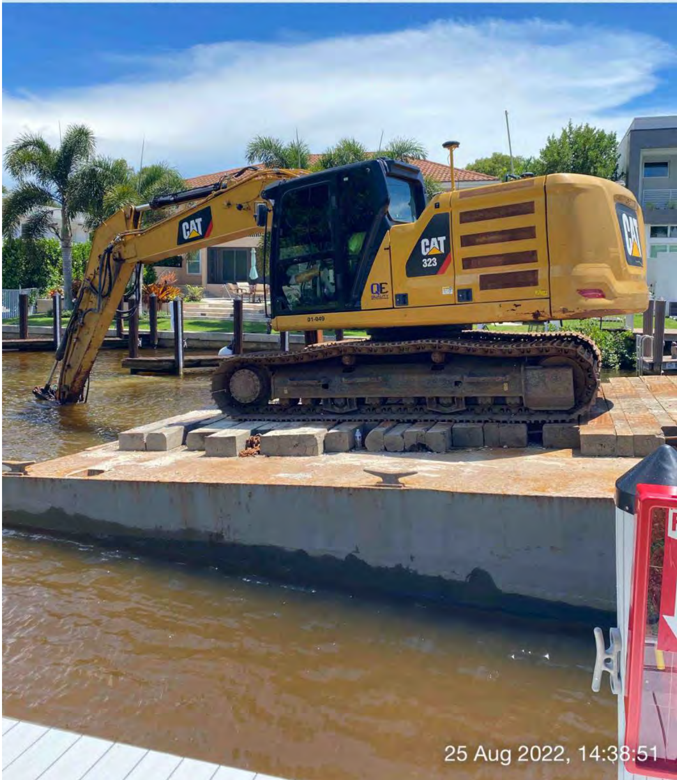
323 excavator grinding rock at station 16+50
