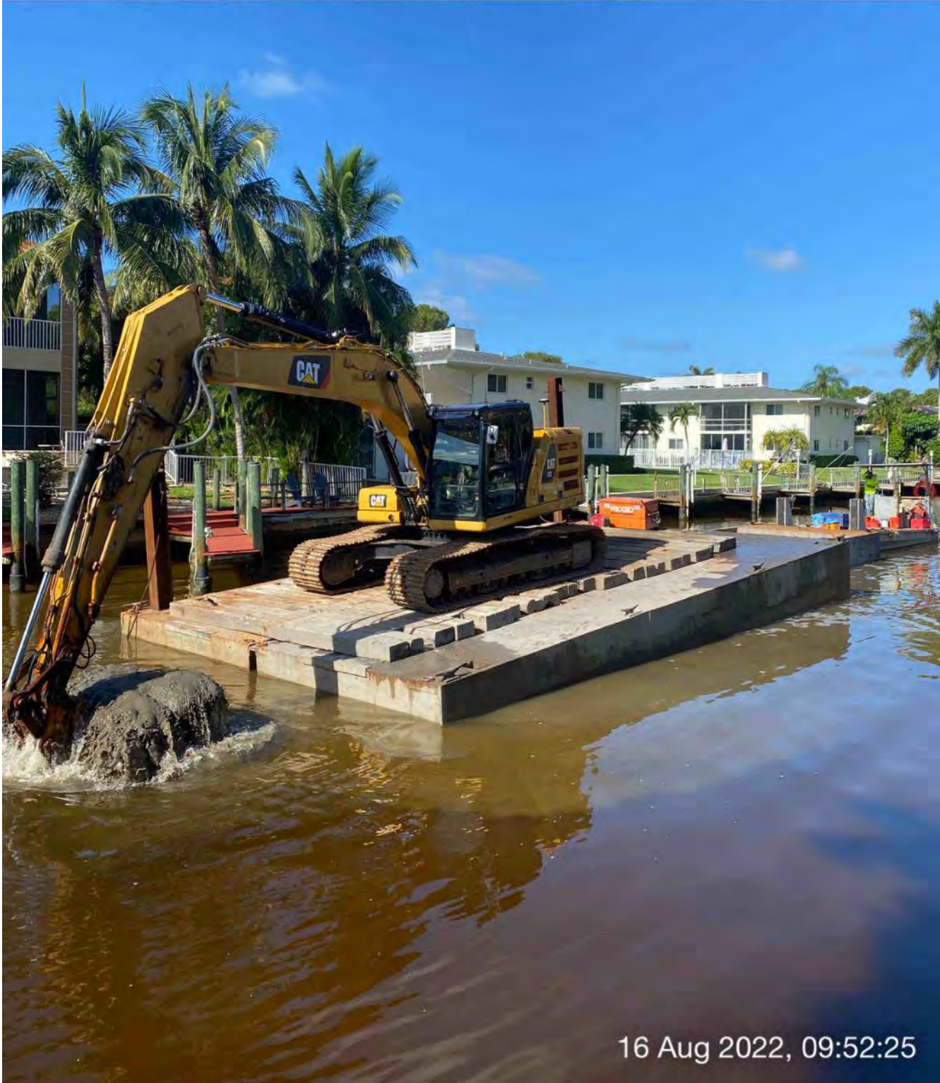
323 excavator removing material from station 11+50
