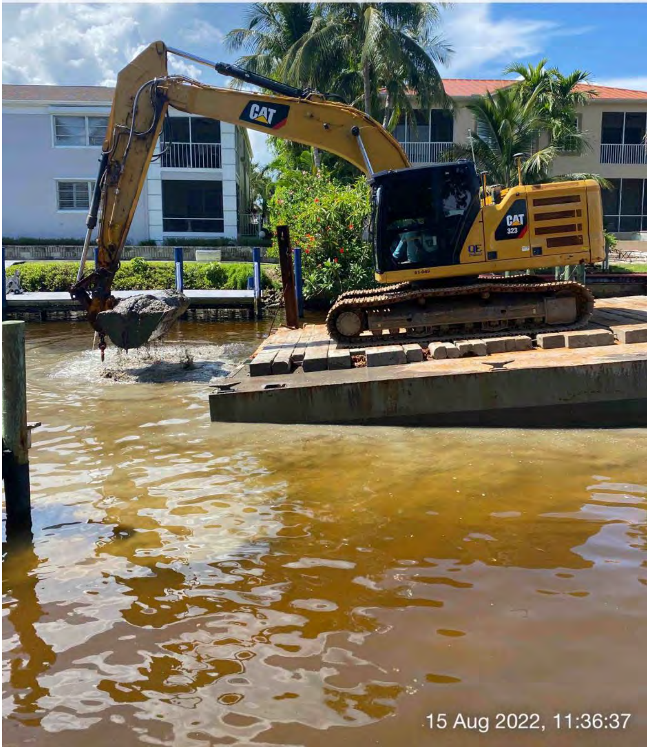
323 excavator removing material from station 11+75
