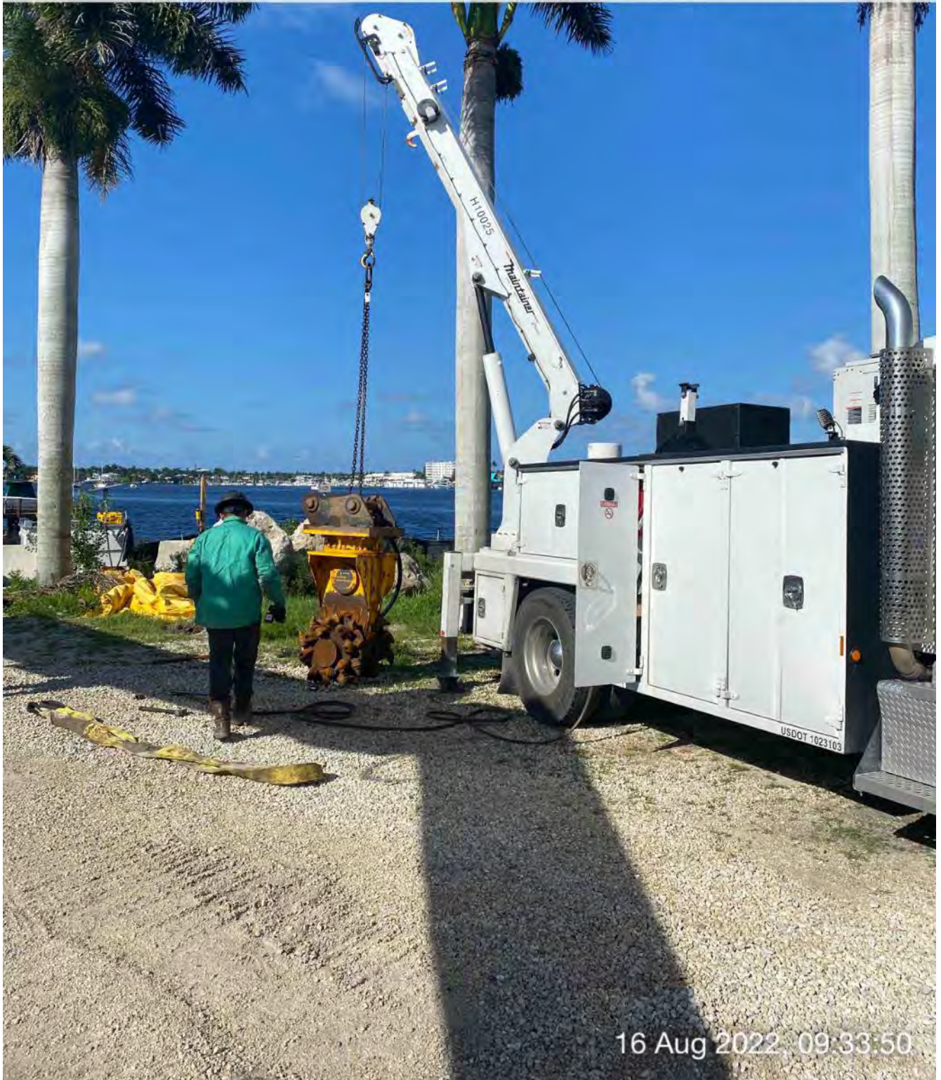
Mechanic lifting Epiroc grinder with utility truck crane
