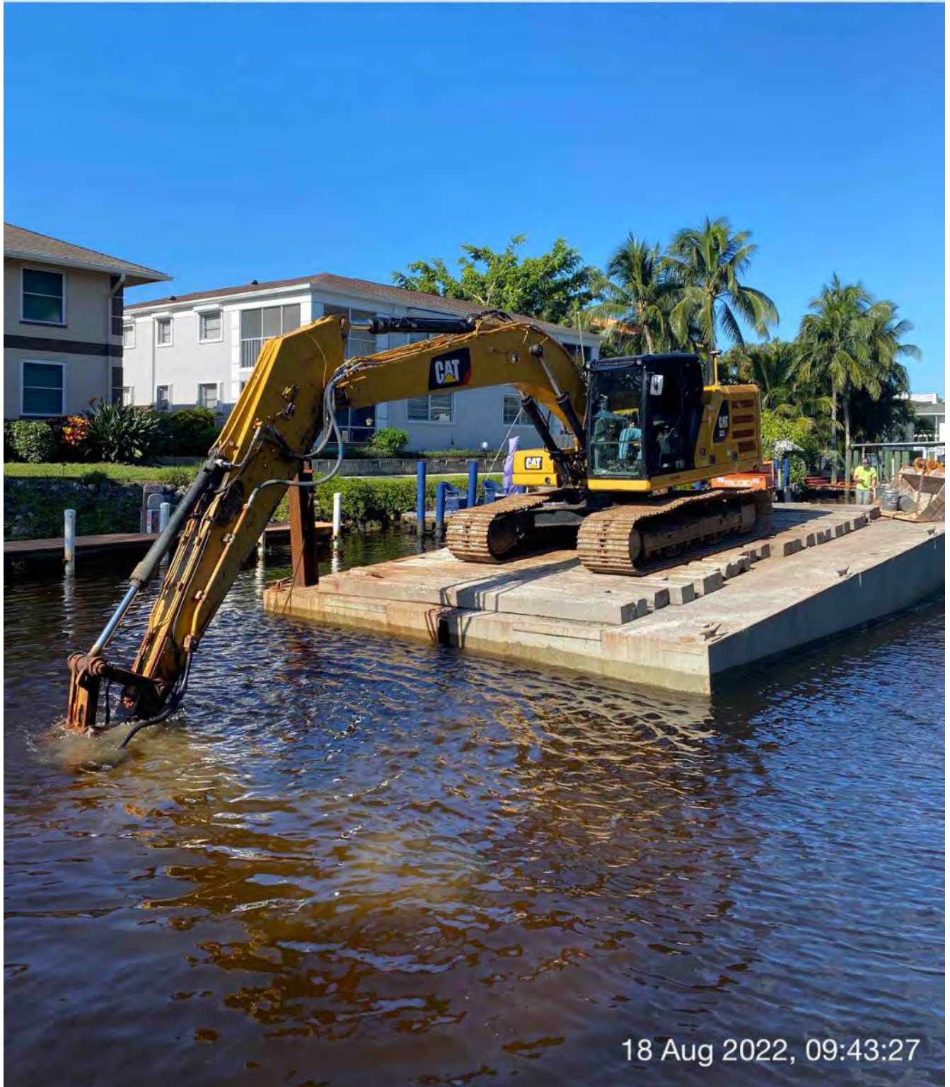
323 excavator grinding rock at station 13+00
