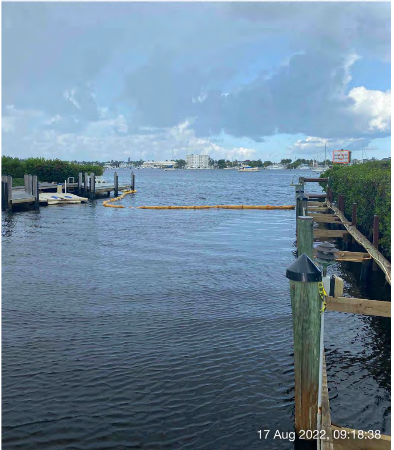
Turbidity curtain installed across the mouth of Canal W-W
