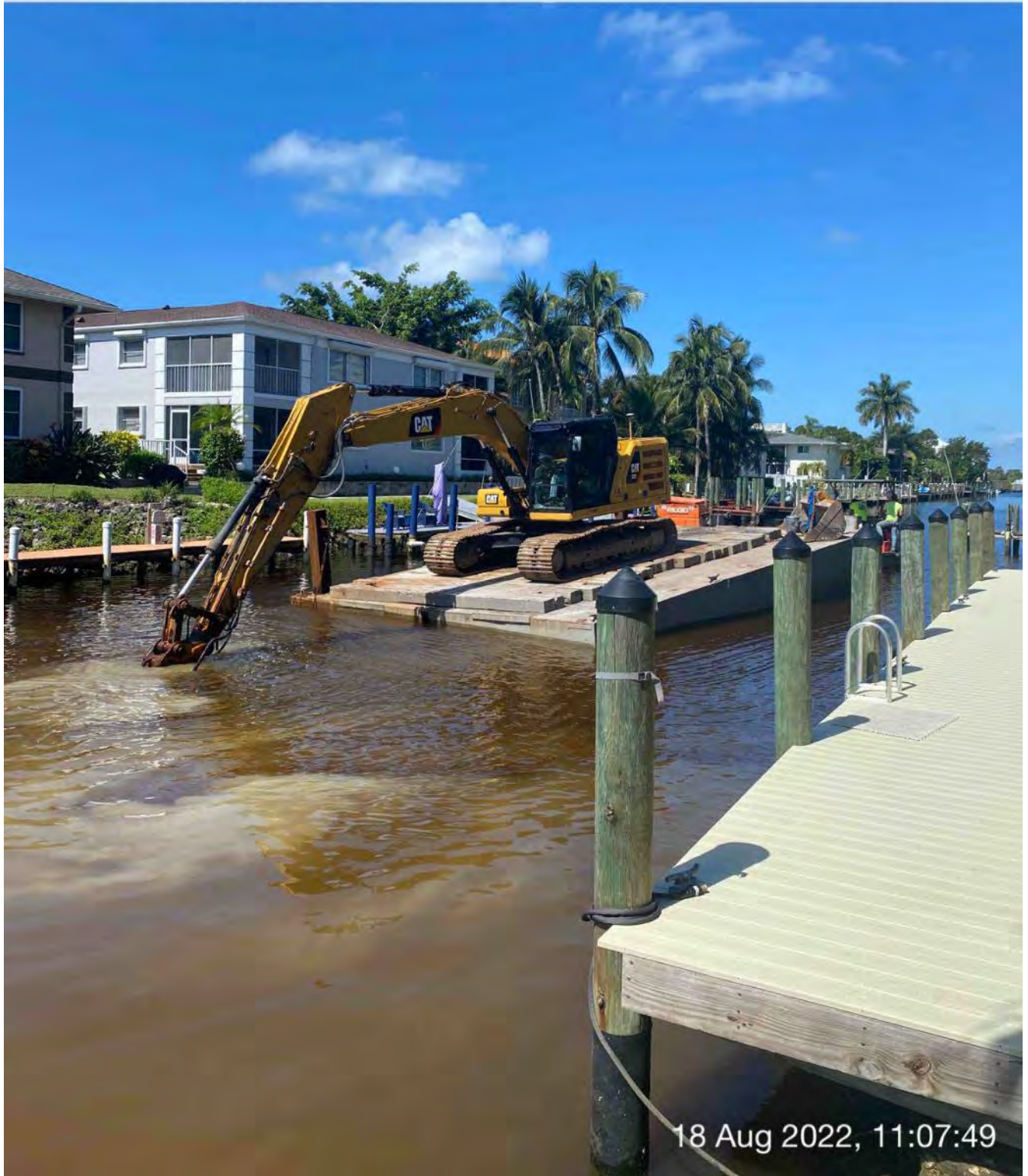
323 excavator grinding rock at station 13+50
