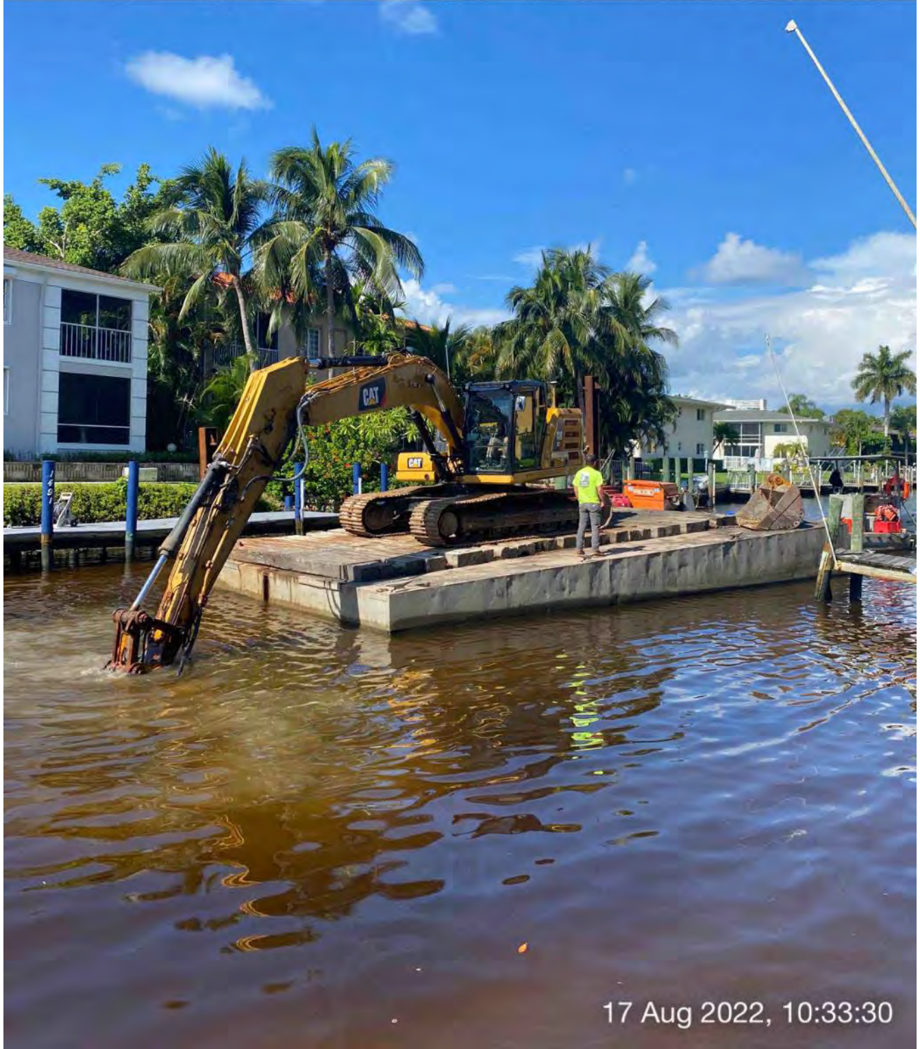
323 excavator grinding rock at station 12+00
