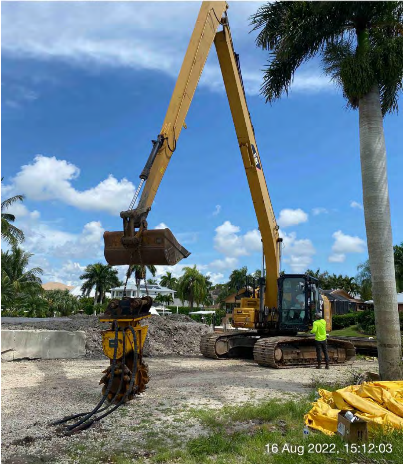
326 excavator transporting Epiroc grinder from site at 1300 Curlew Avenue to hopper
