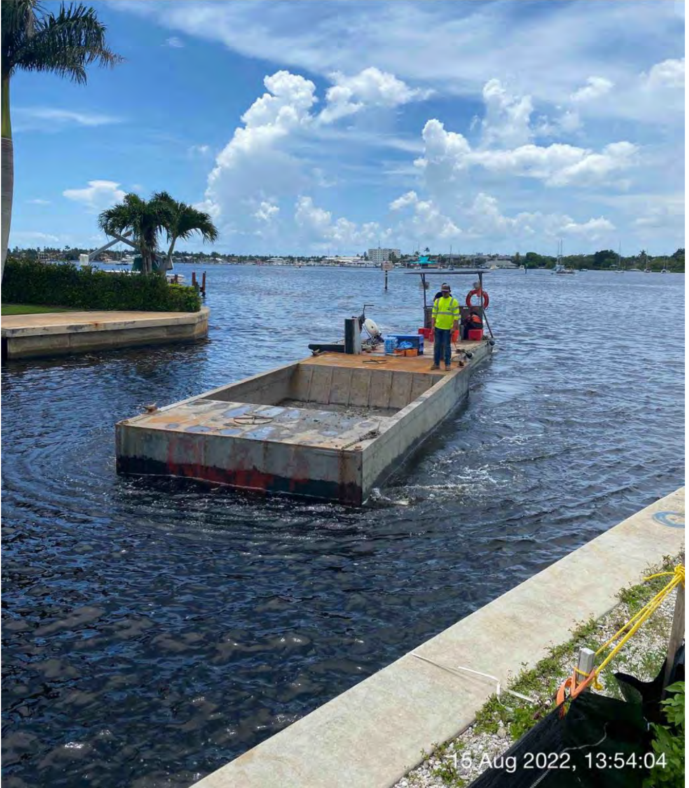
Push boat transporting full hopper of removed material from Canal W-W to Canal CC-CC
