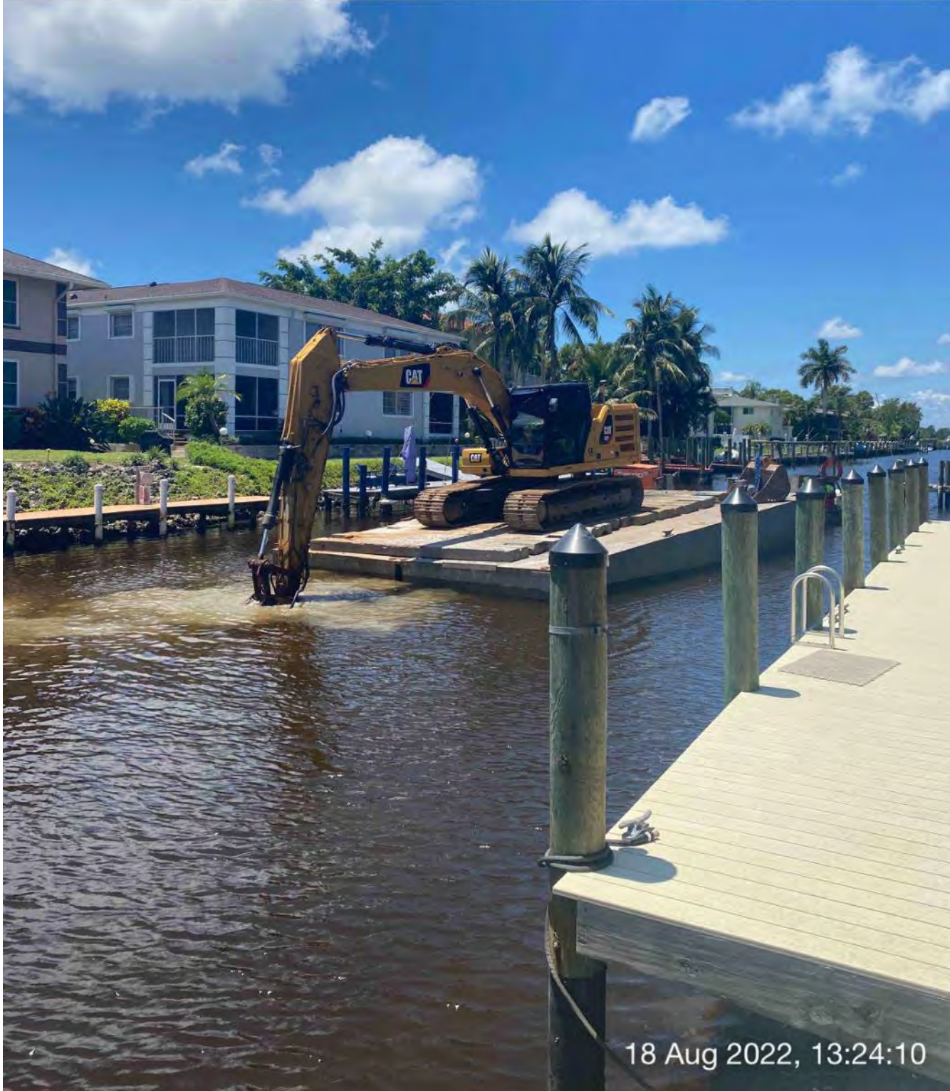
323 excavator grinding rock at station 13+50
