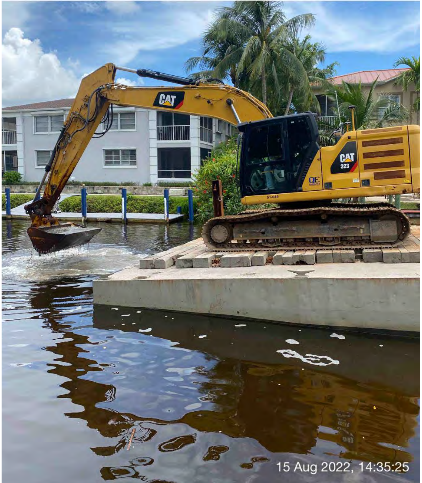
323 excavator removing material from station 12+25
