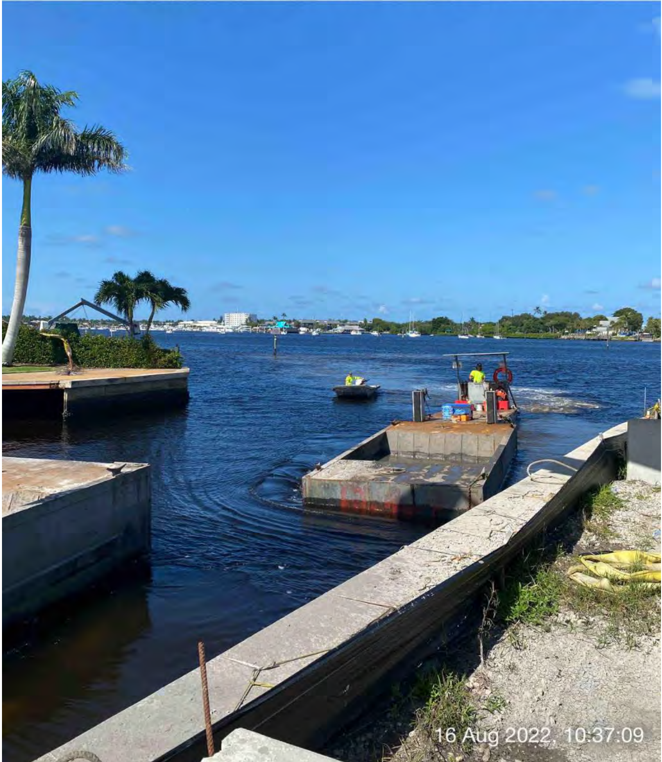
Push boat dropping off full hopper of removed material in Canal CC-CC
