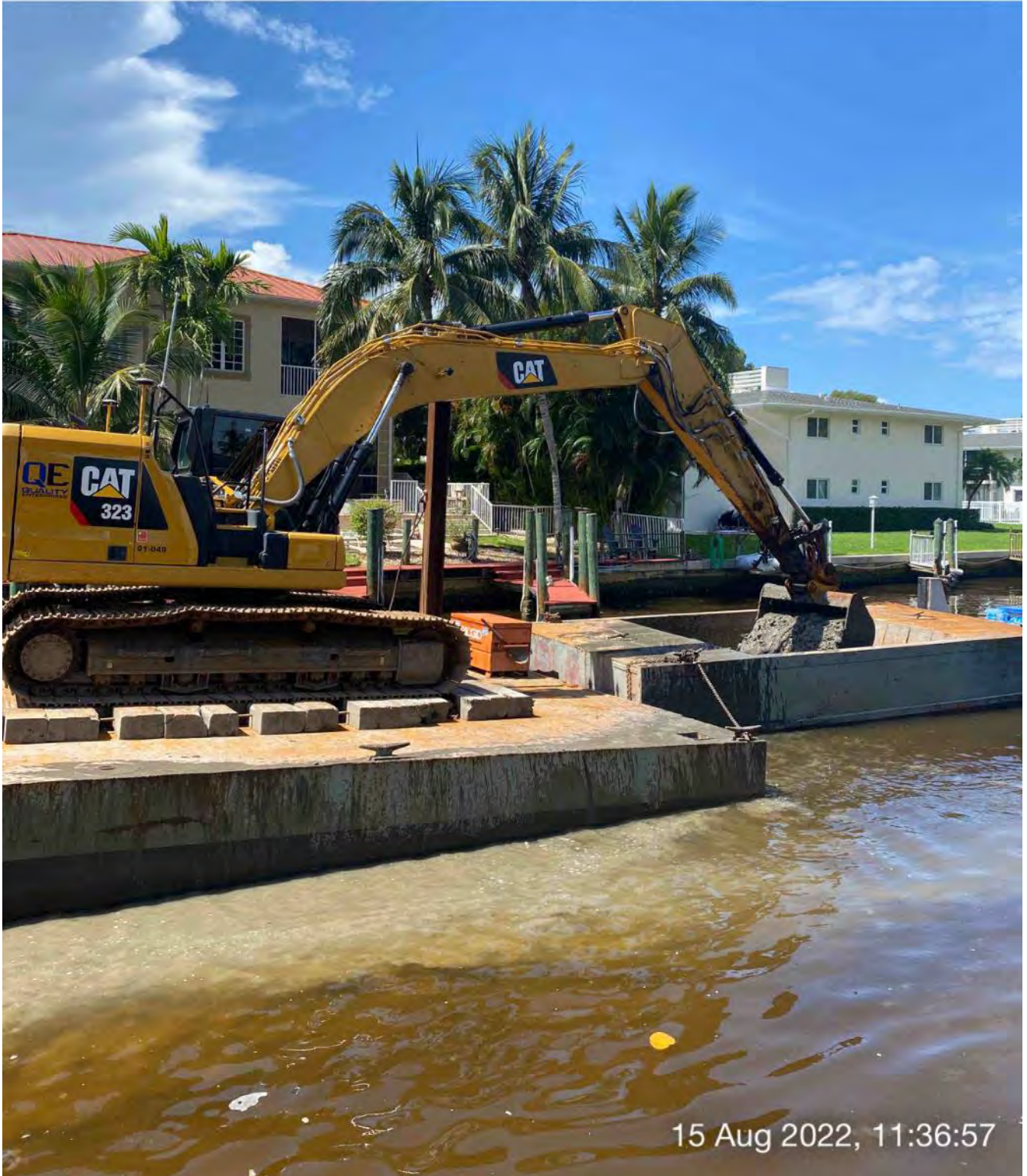
323 excavator removing material from station 11+75 and transferring to hopper
