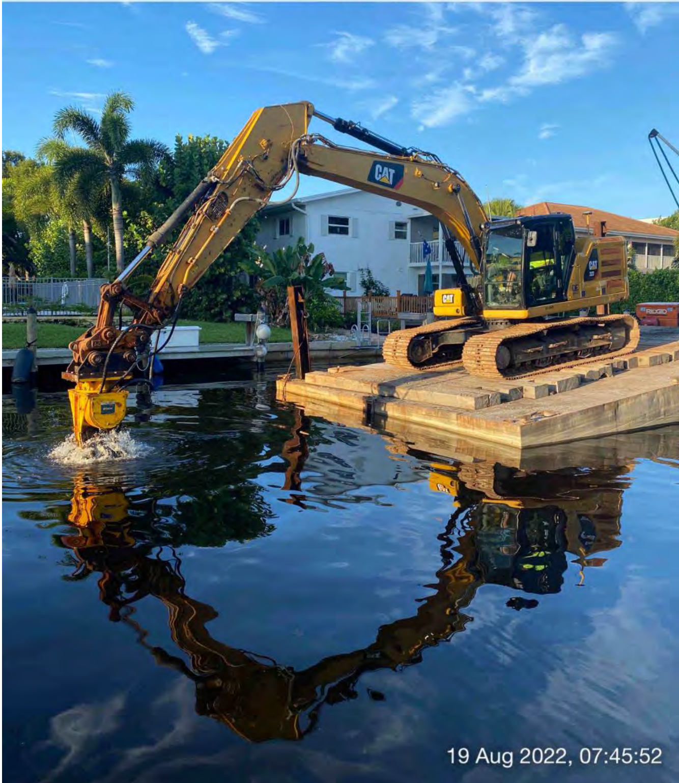
323 excavator grinding rock at station 18+25
