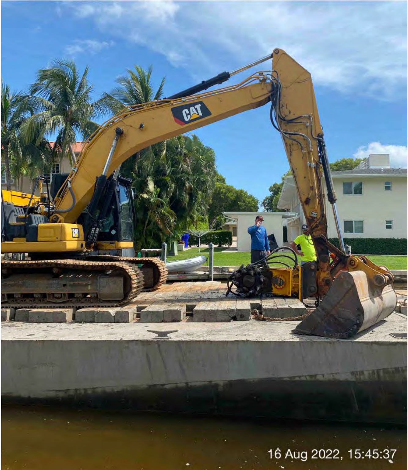
Contractor installing Epiroc grinder attachment on 323 excavator
