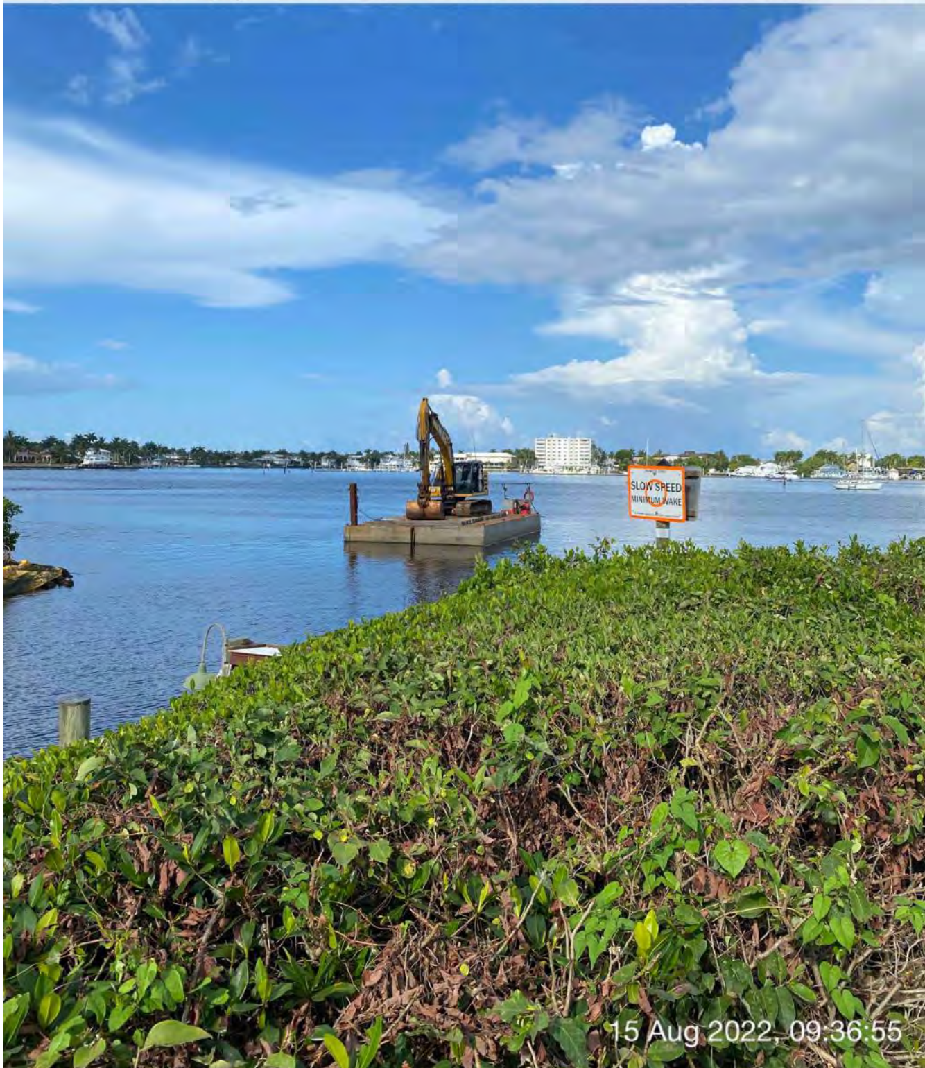
323 excavator and barge at station 0+00
