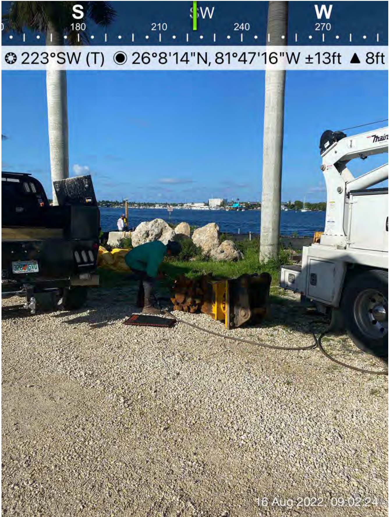
Mechanic welding Epiroc grinder on site at 1300 Curlew Avenue
