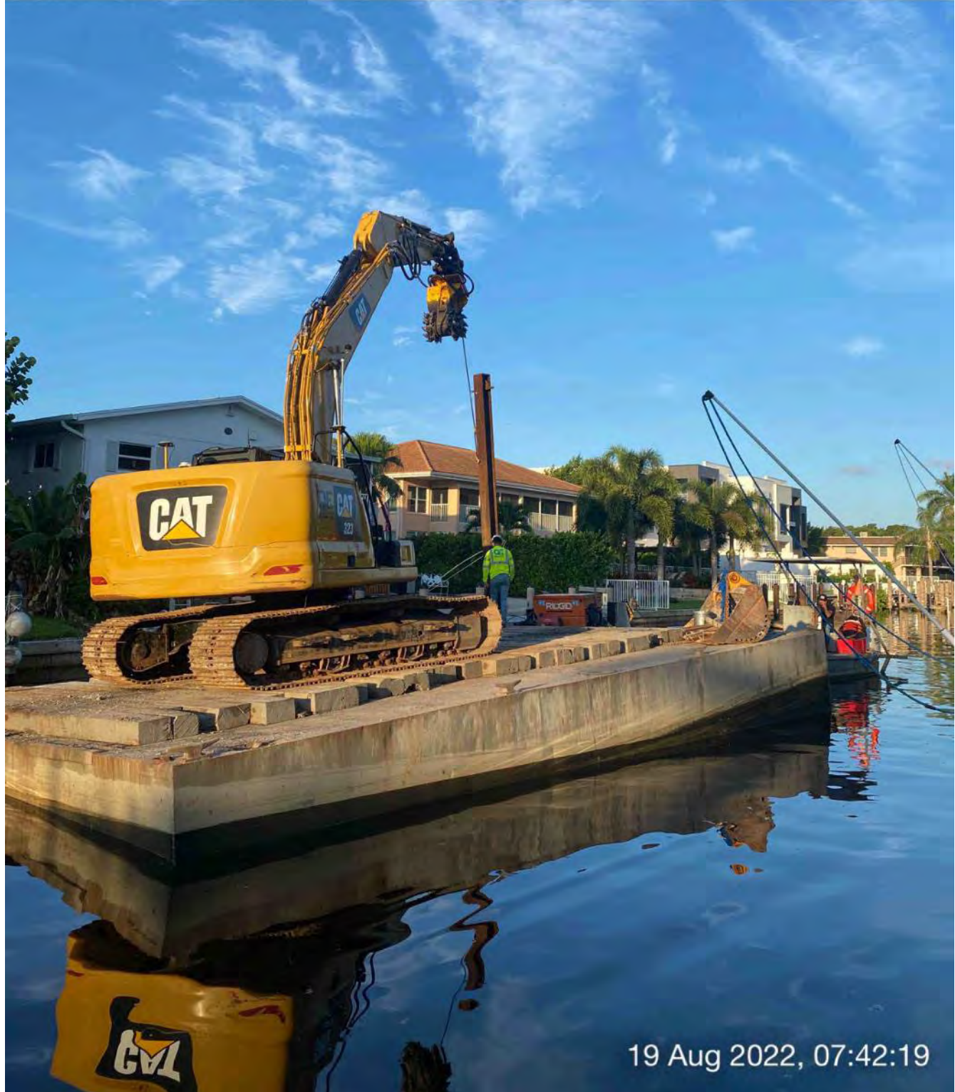
323 excavator lifting spud to allow push boat to mobilize barge at station 18+25
