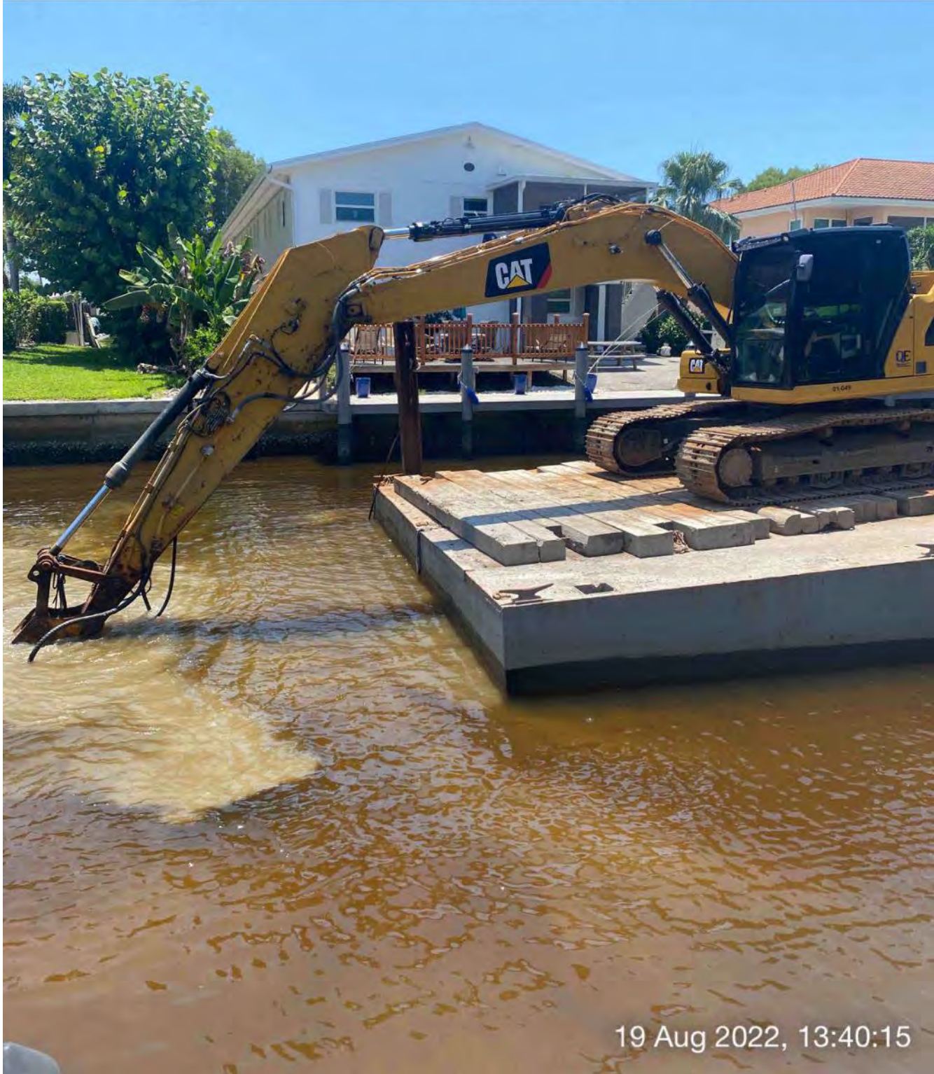
323 excavator grinding rock at station 18+00
