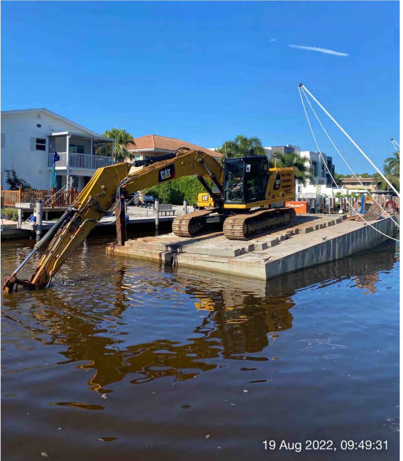
323 excavator grinding rock at station 18+25
