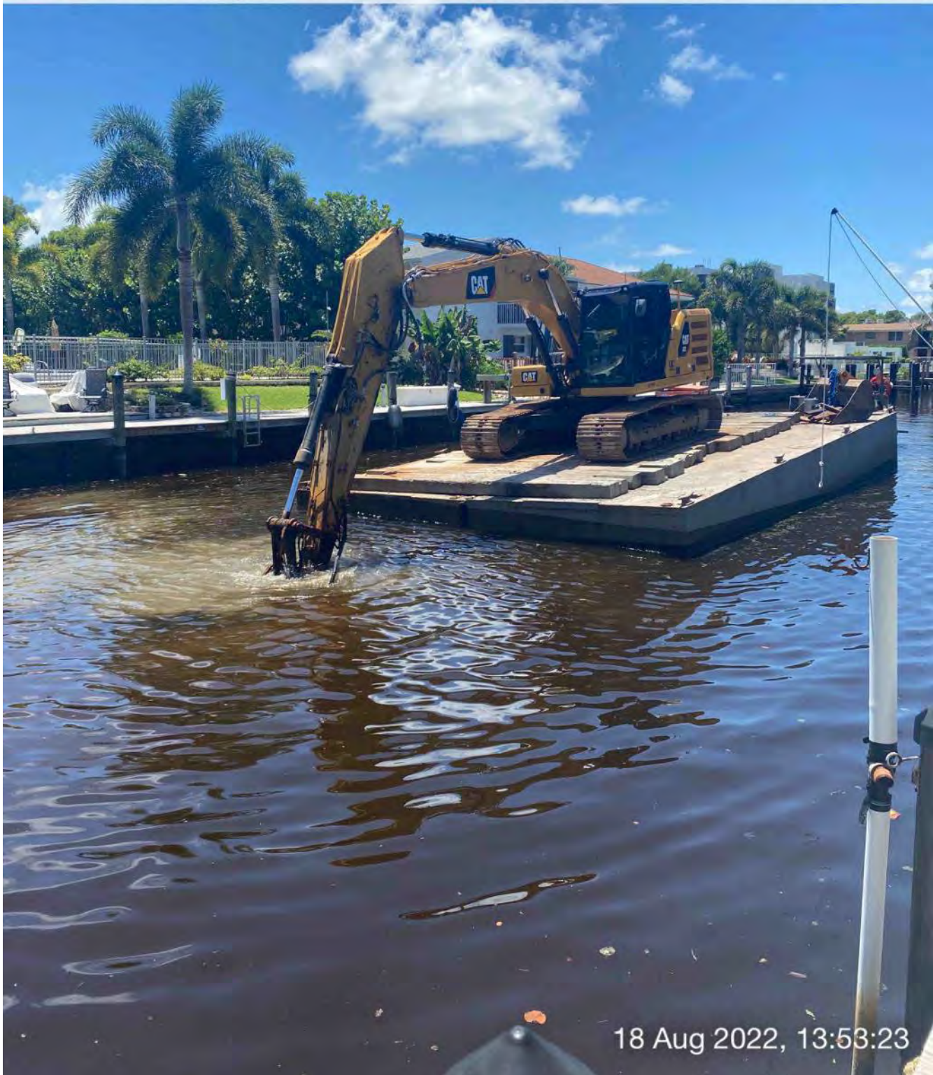
323 excavator grinding rock at station 18+75
