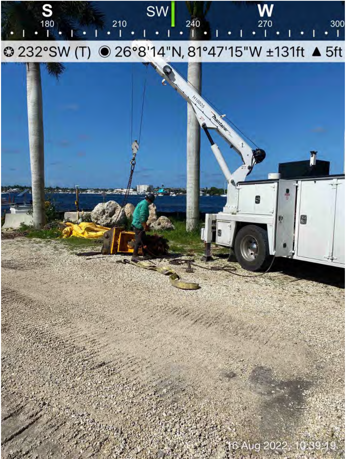
Mechanic replacing sleeves on Epiroc grinder on site at 1300 Curlew Avenue
