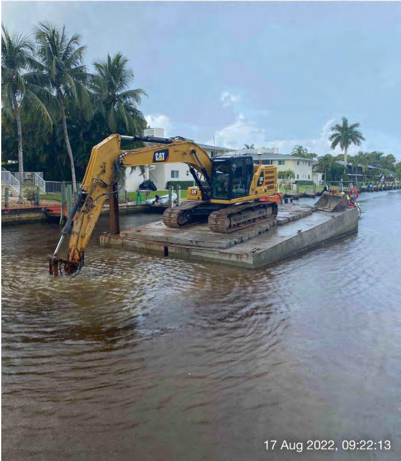
323 excavator grinding rock at station 11+50
