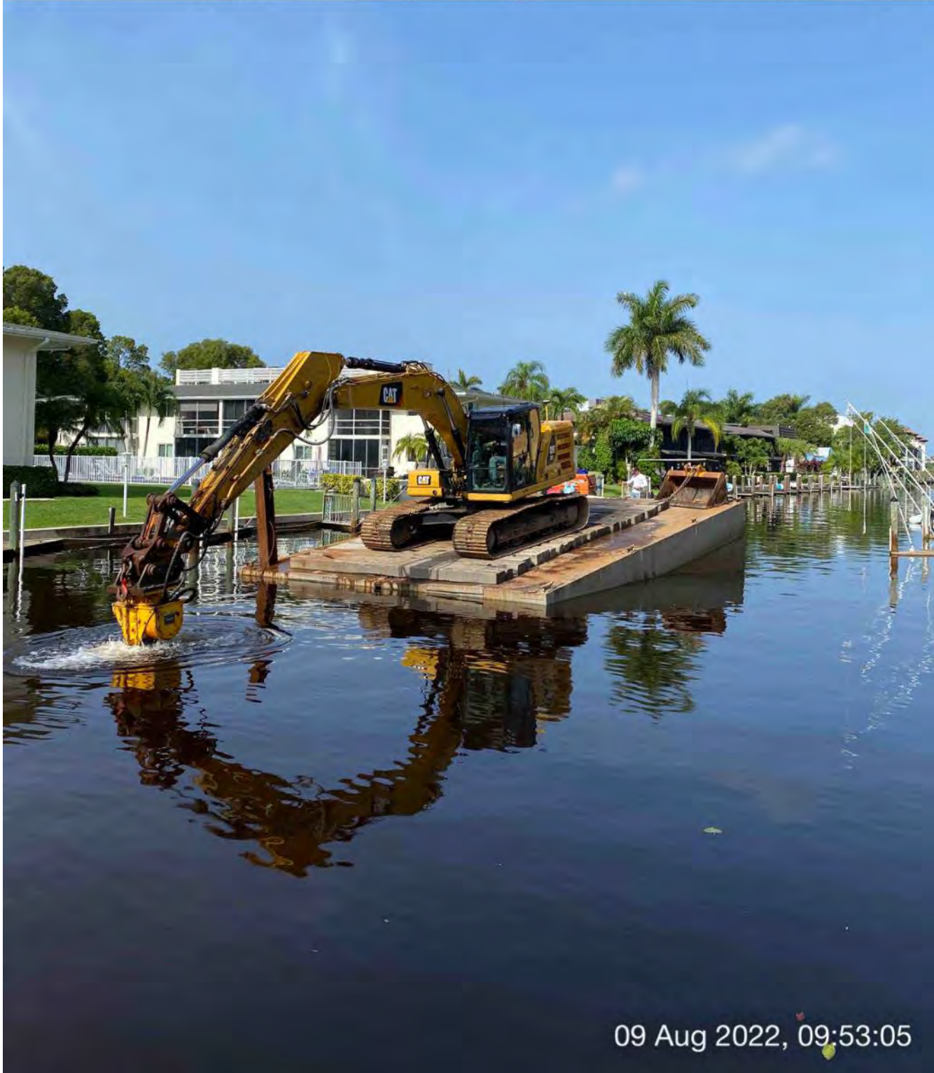
323 excavator grinding rock at station 10+00
