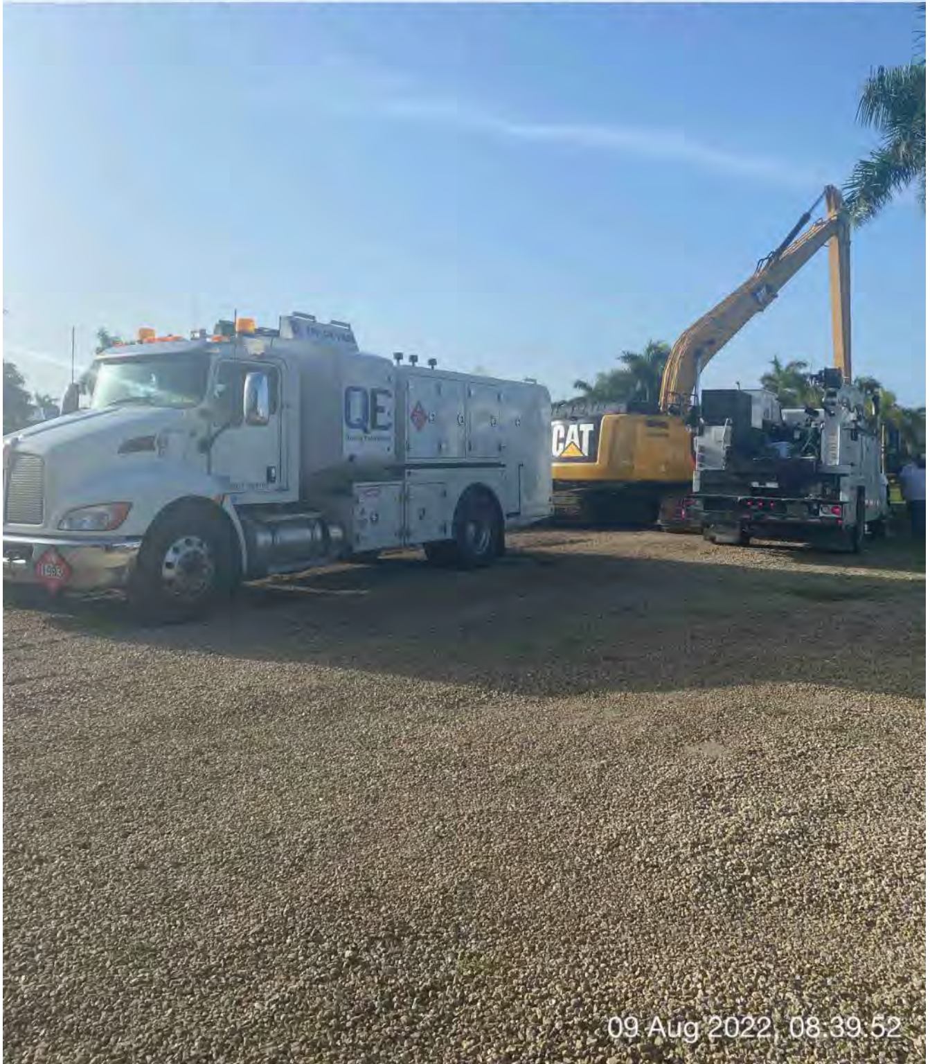
Fuel truck and utility truck on site at 1300 Curlew Avenue
