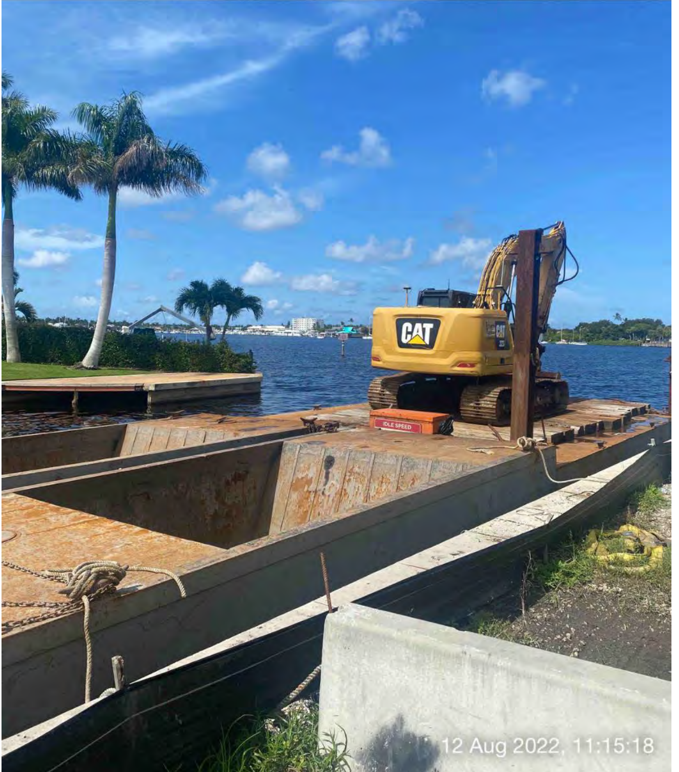
323 excavator, barge, and 2 hoppers staged in Canal CC-CC between stations 1+00 and 1+50
