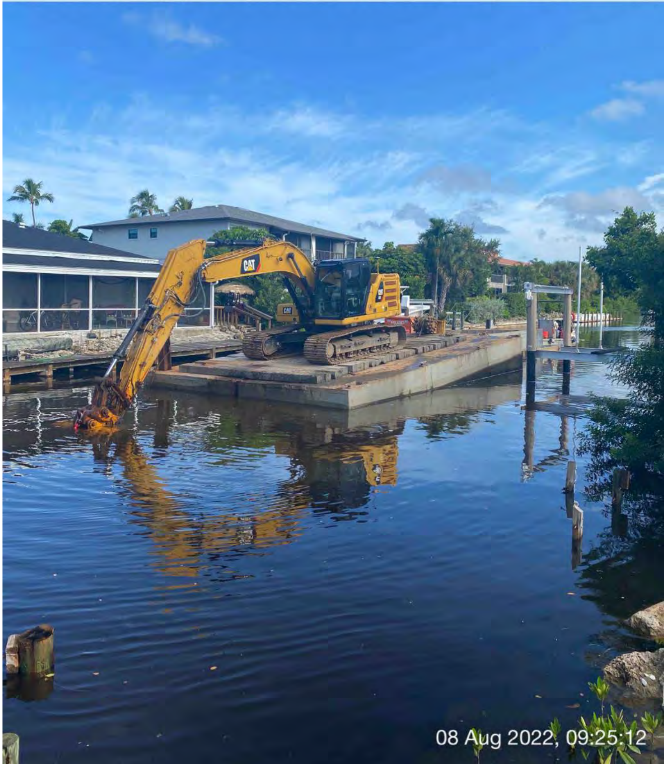
323 excavator checking elevations and removing material from station 4+00 in Canal AA-AA
