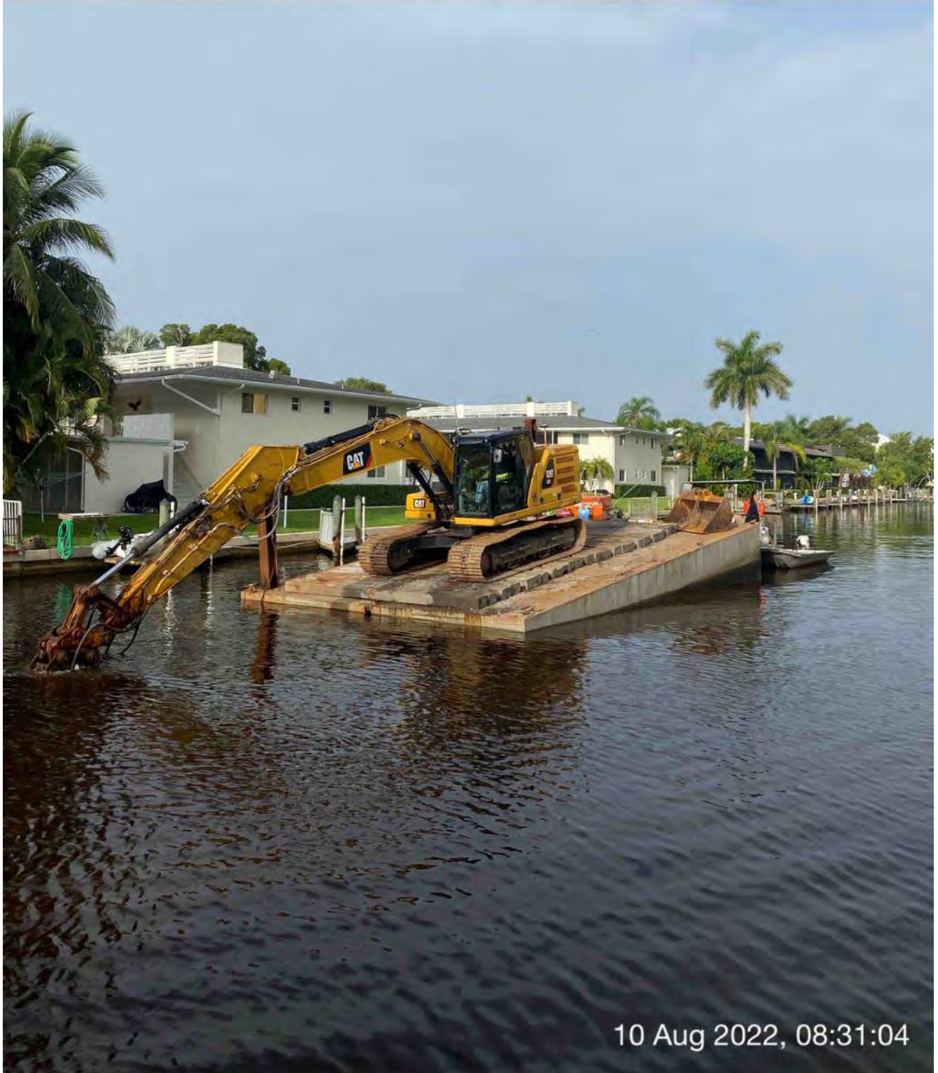
323 excavator grinding rock at station 11+00
