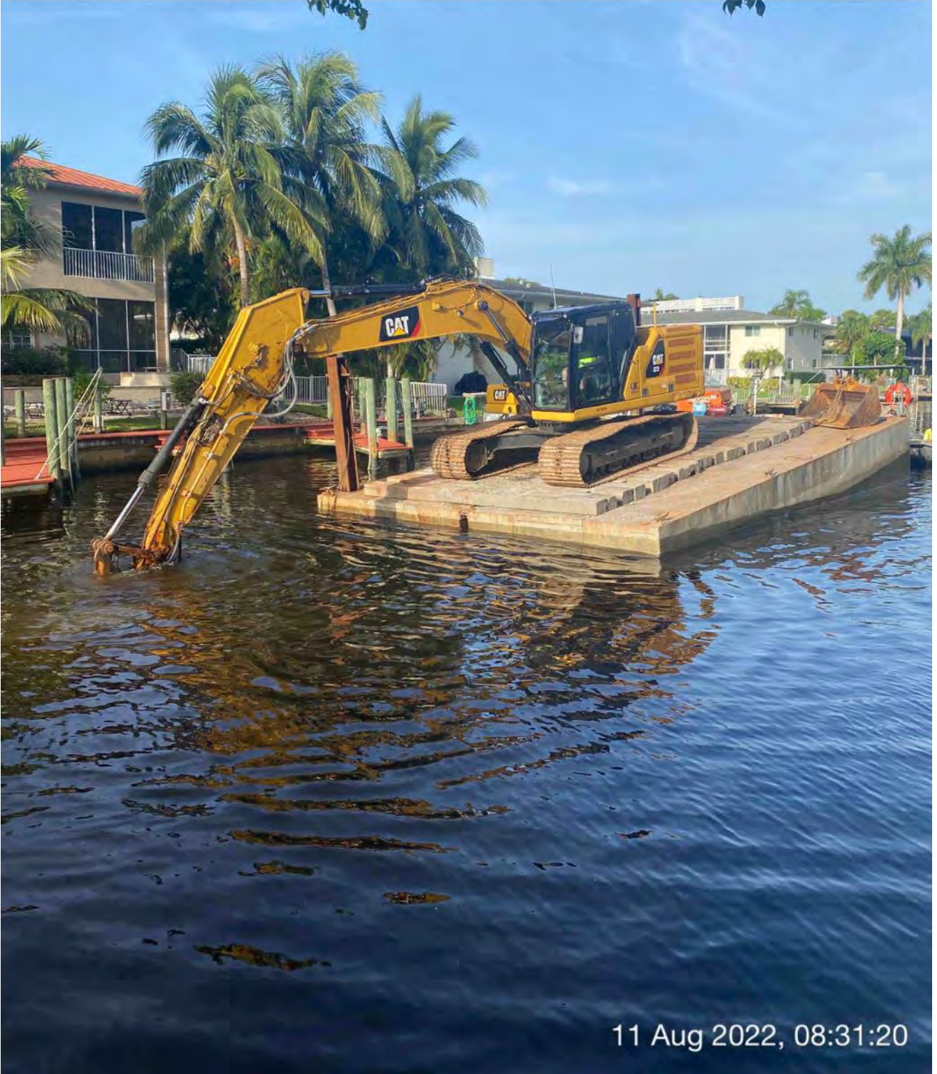
323 excavator grinding rock at station 11+25
