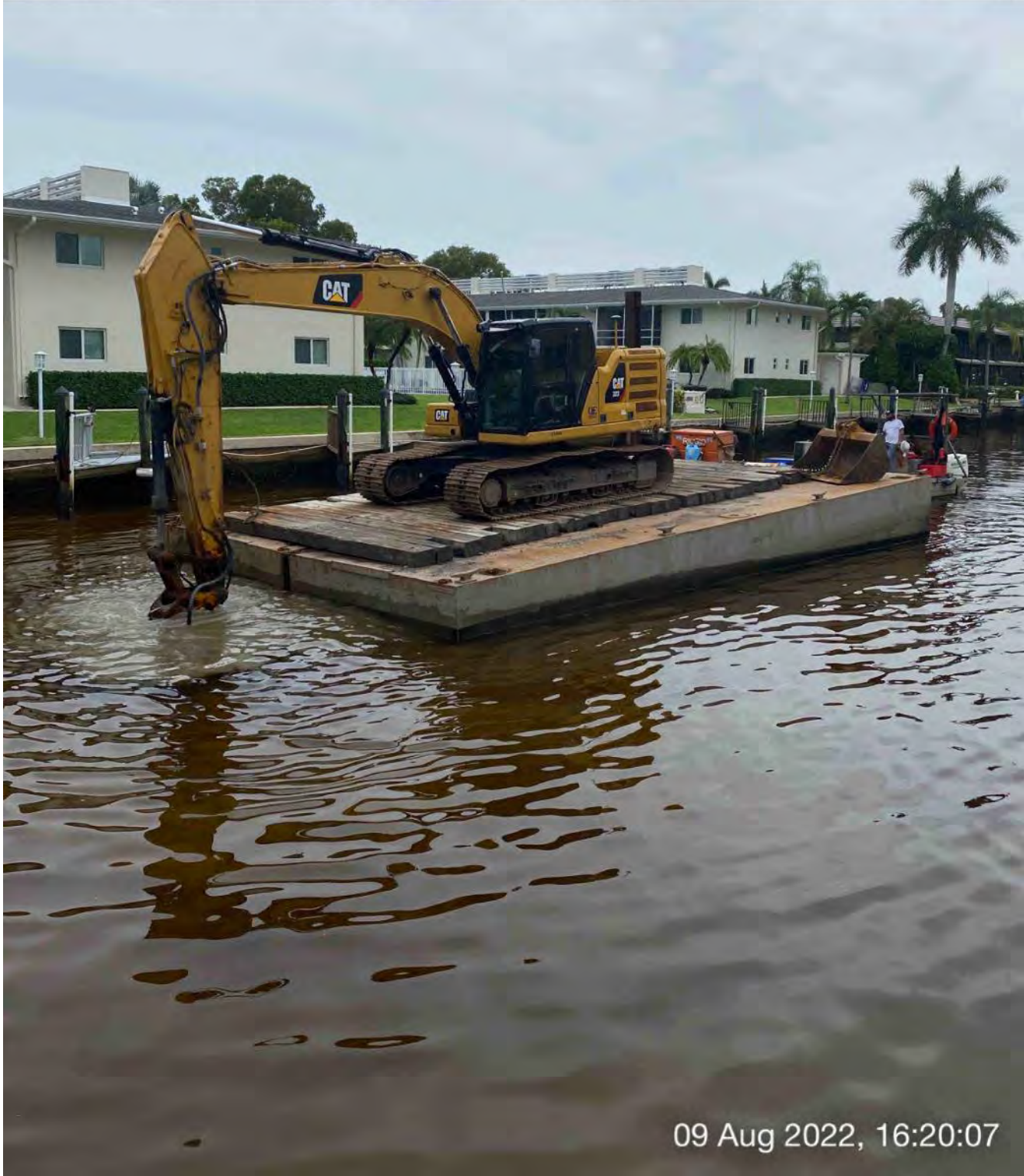
323 excavator grinding rock at station 11+00
