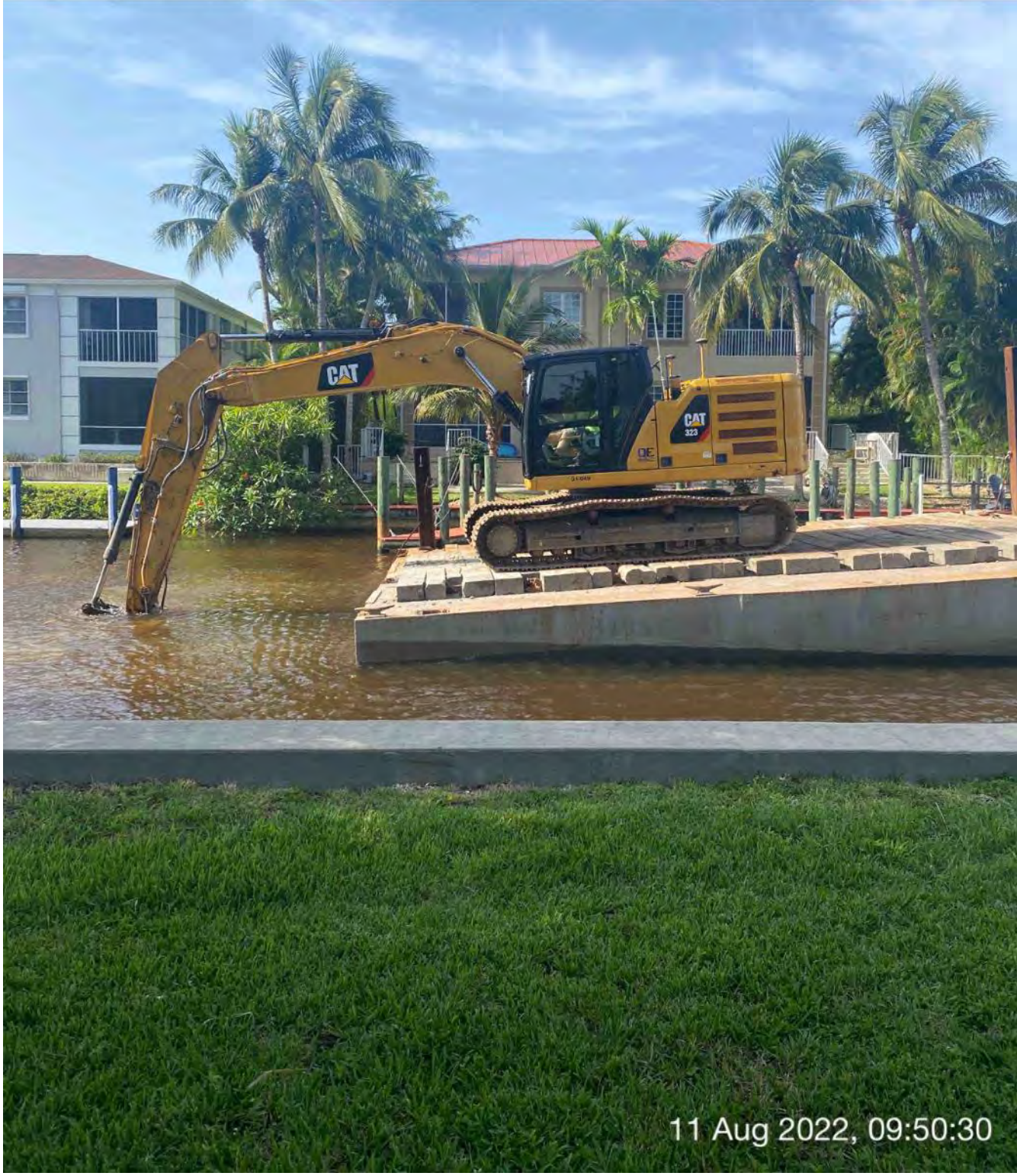
323 excavator grinding rock at station 11+50
