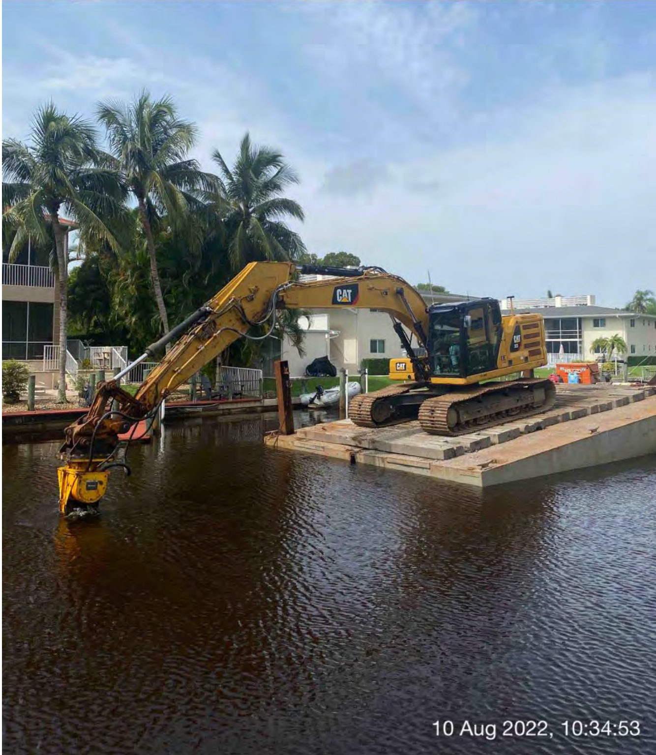
323 excavator grinding rock at station 11+00
