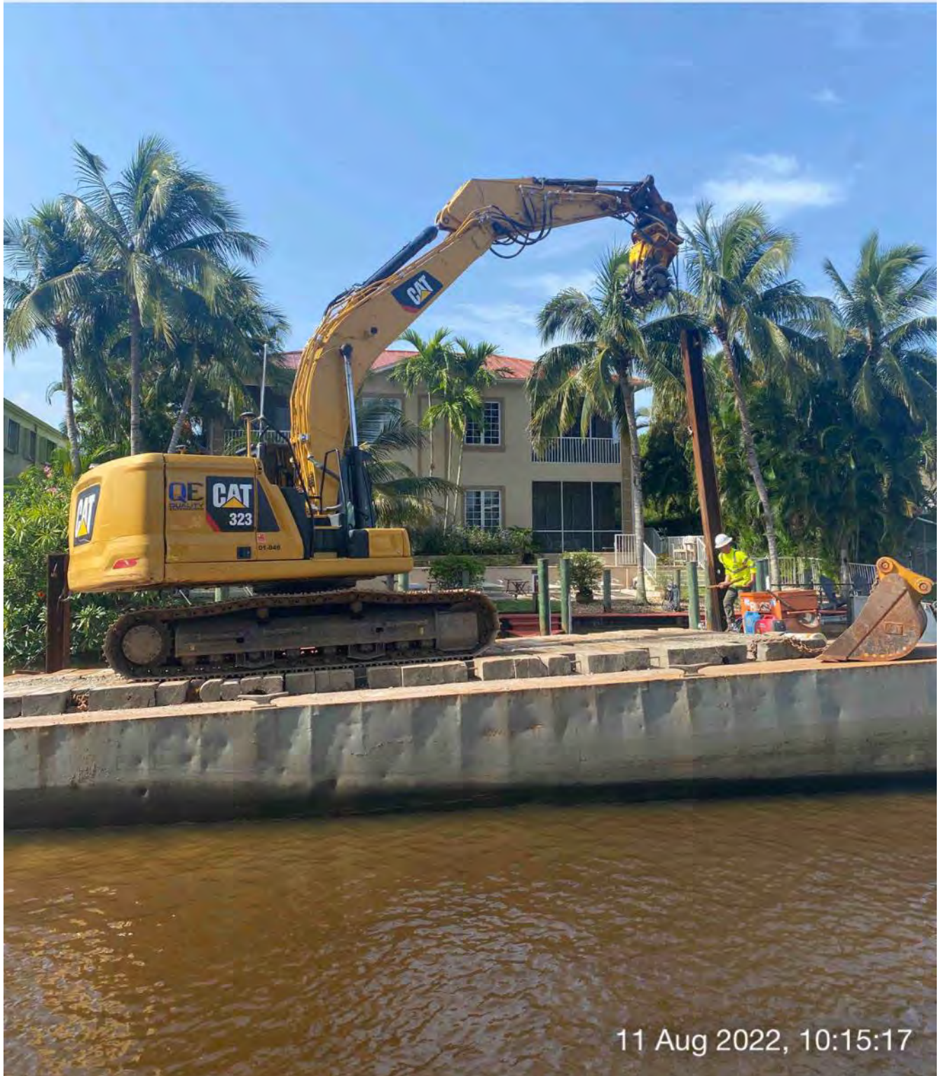
323 excavator lifting spud to allow push boat to mobilize barge at station 11+25
