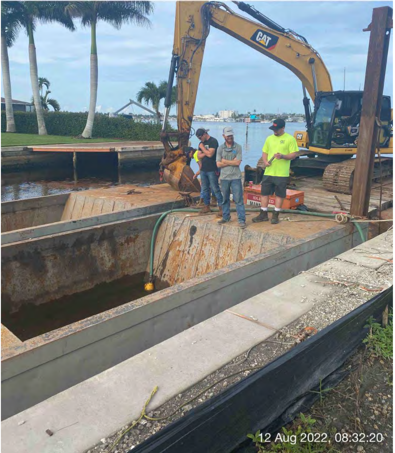
Contractor pumping water out from hoppers in Canal CC-CC station 1+50
