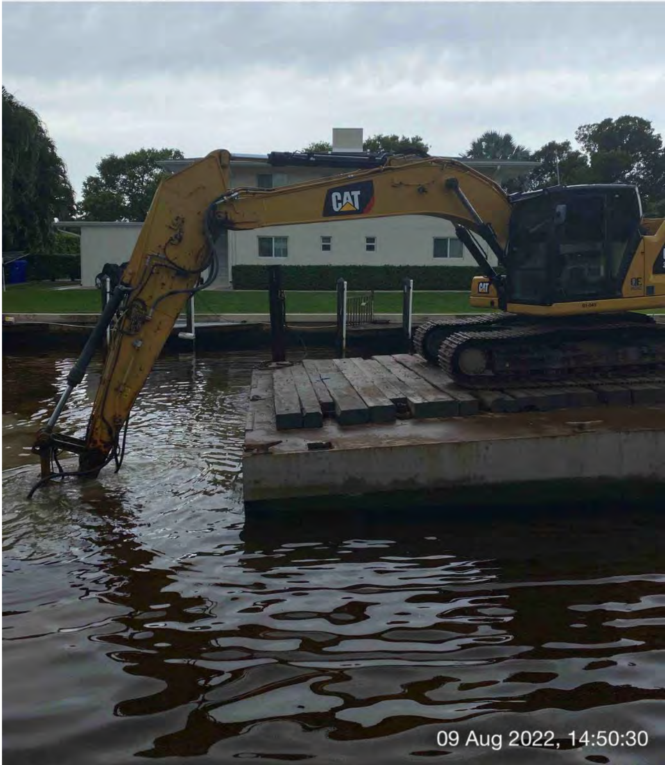
323 excavator grinding rock at station 10+50
