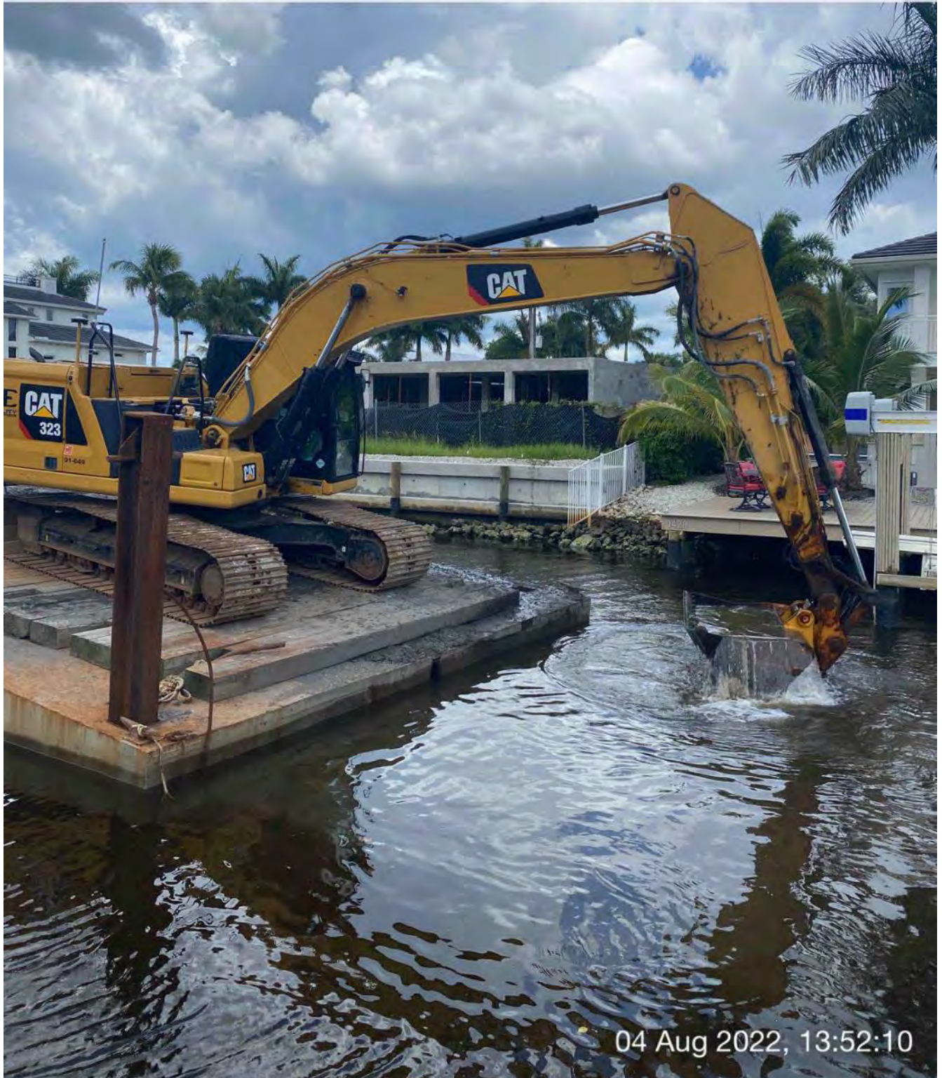
323 excavator removing material from station 4+50 in Canal X-X
