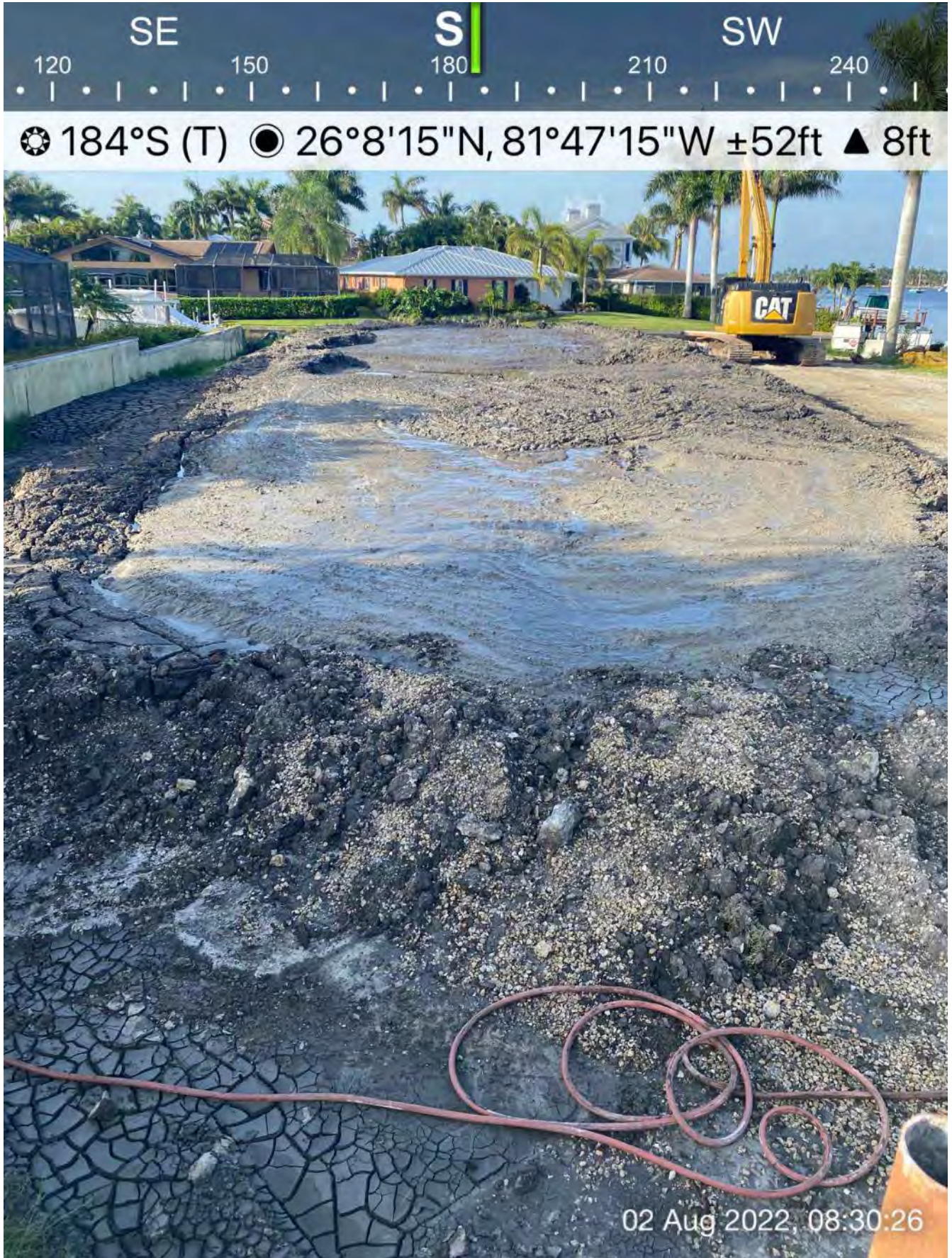
Removed material at dewatering site at 1300 Curlew Avenue
