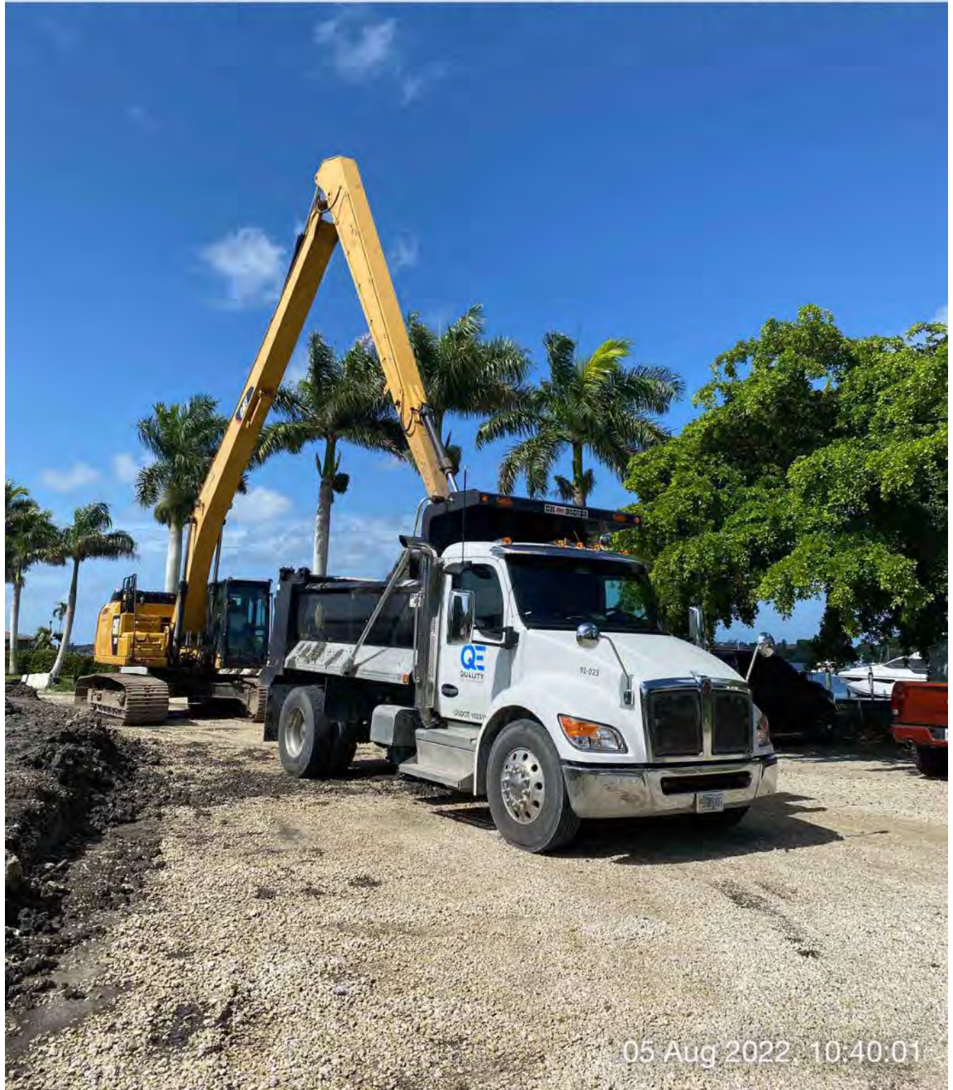
326 excavator transferring removed material from dewatering site to dump truck bed at 1300 Curlew Avenue
