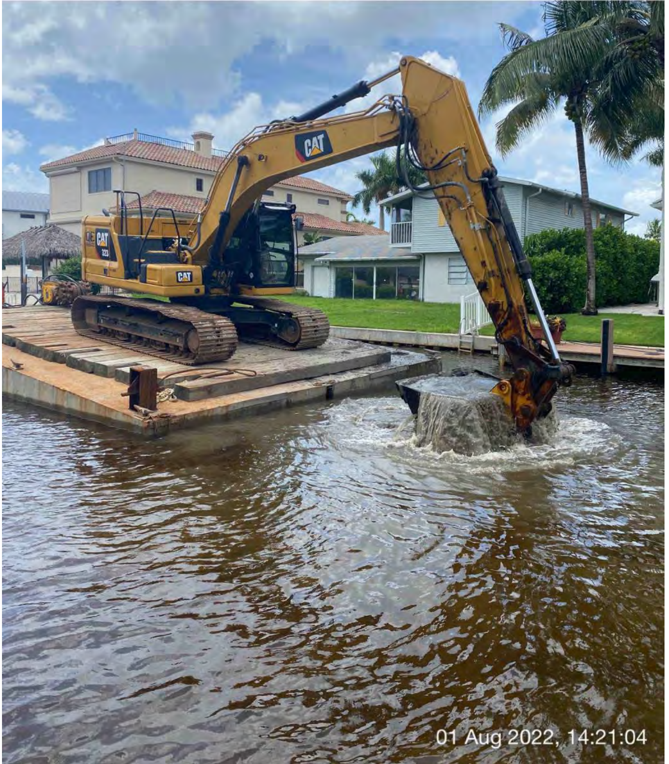
323 excavator removing material from station 3+50
