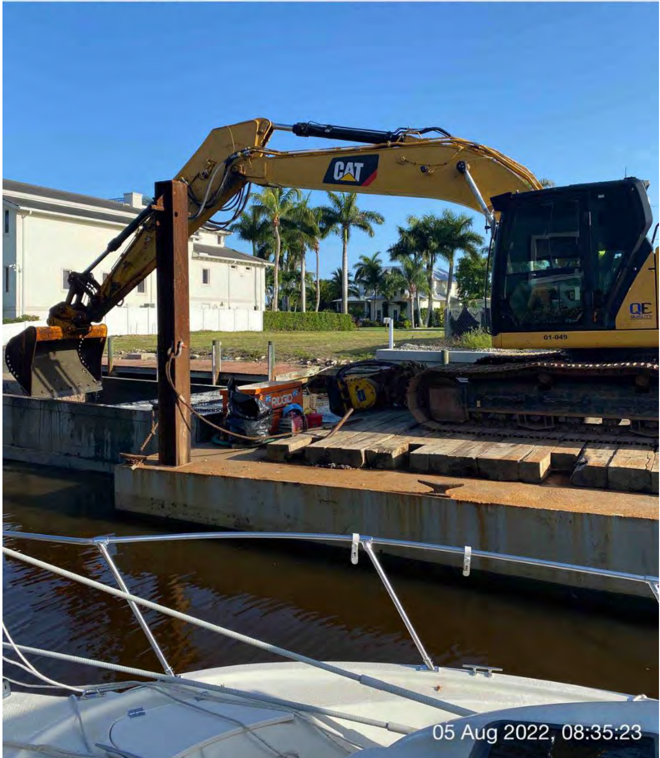
323 excavator removing material from station 4+00 and transferring to hopper
