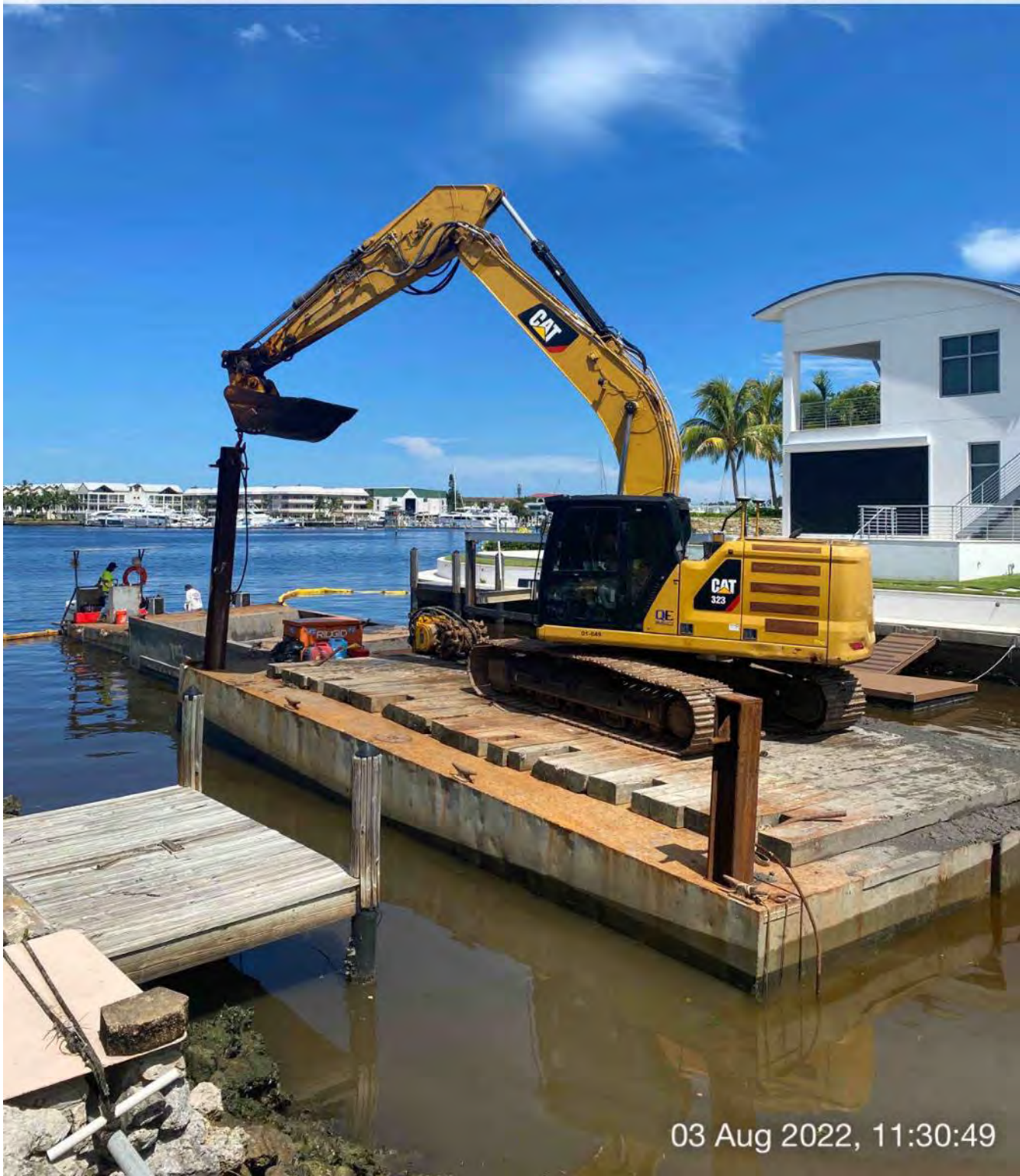
323 excavator lifting spud to allow push boat to mobilize barge at station 2+00
