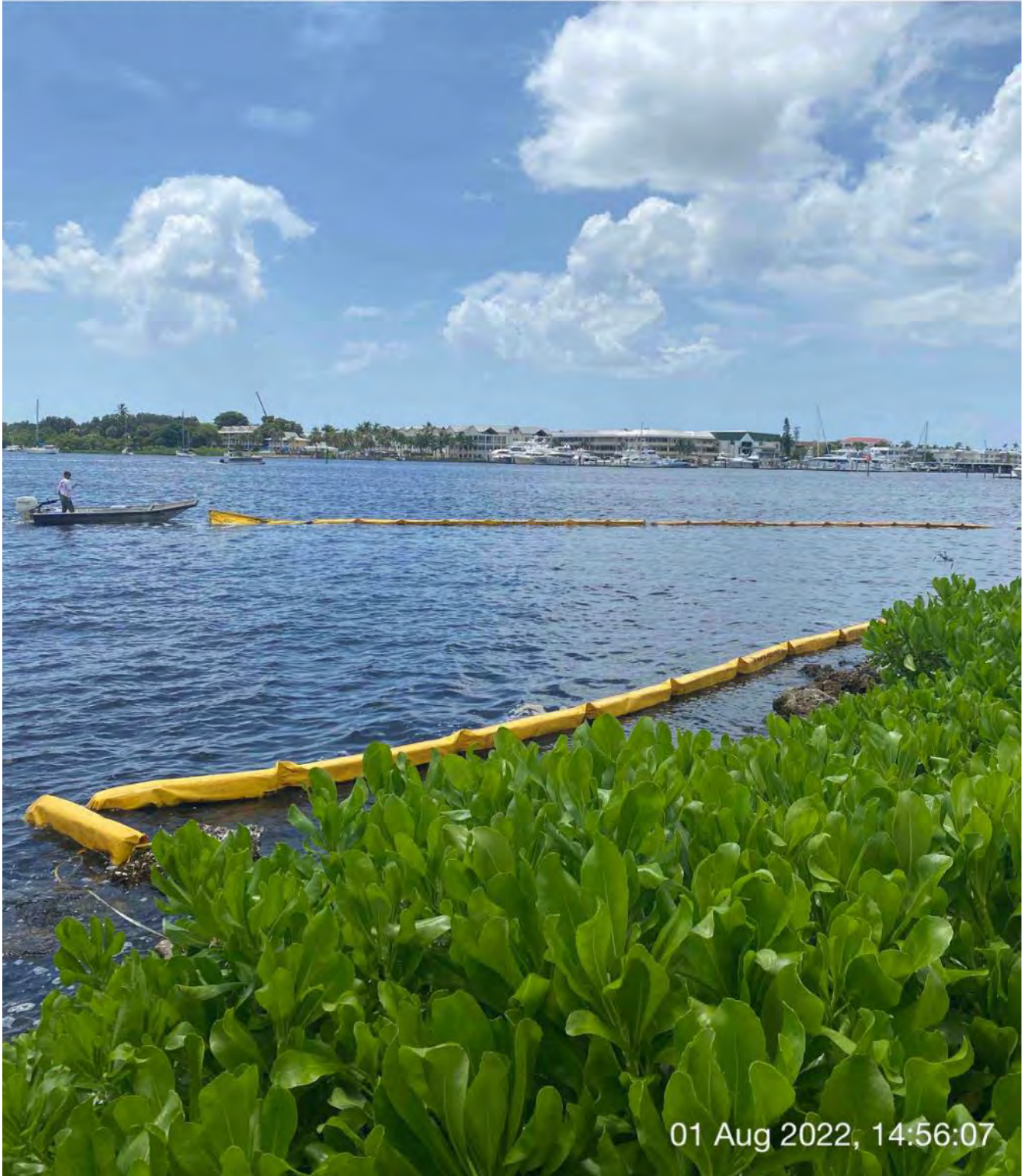
Support boat opening turbidity curtain to allow push boat to exit Canal BB-BB
