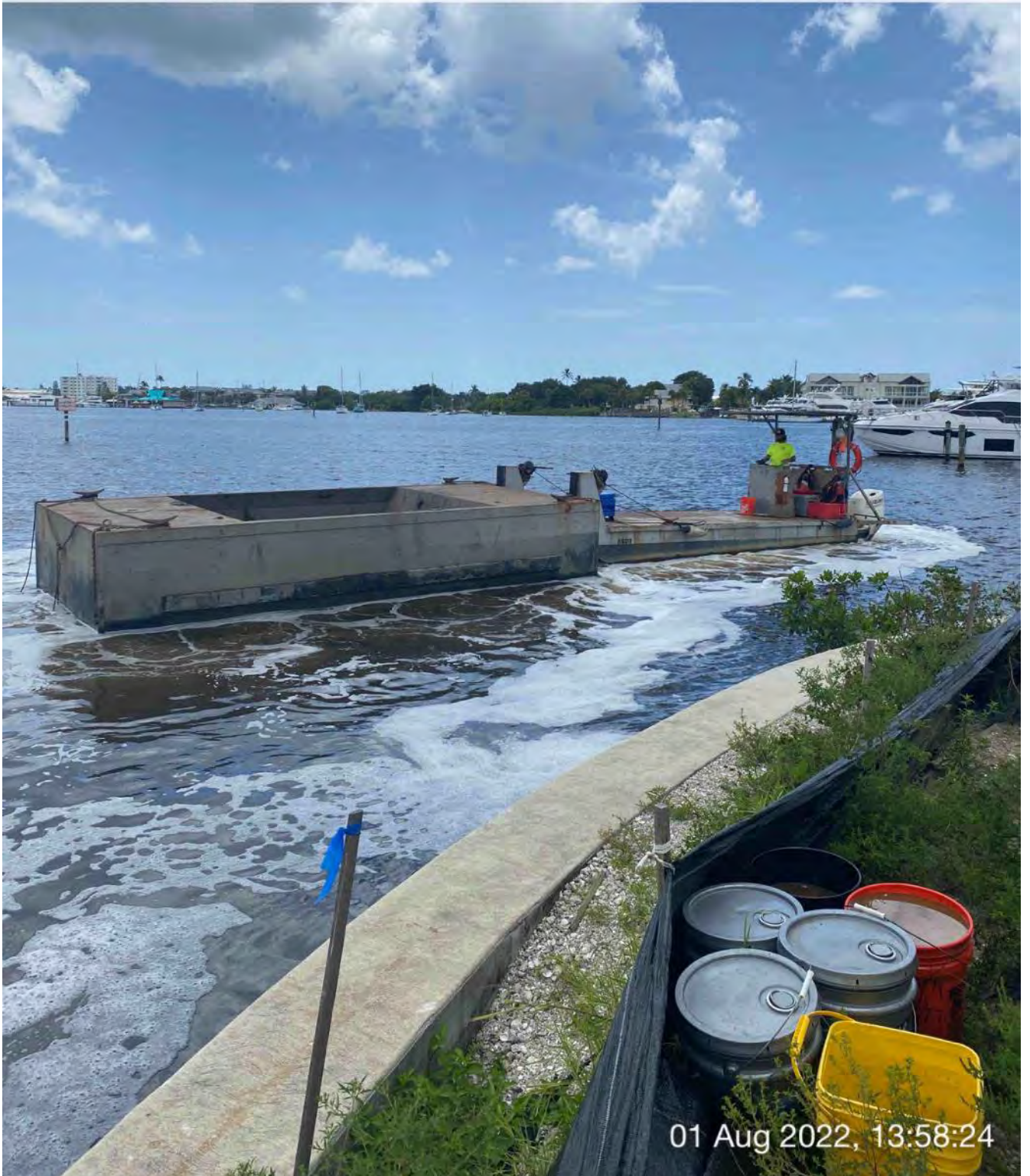
Push boat transporting empty hopper from Canal CC-CC to Canal BB-BB
