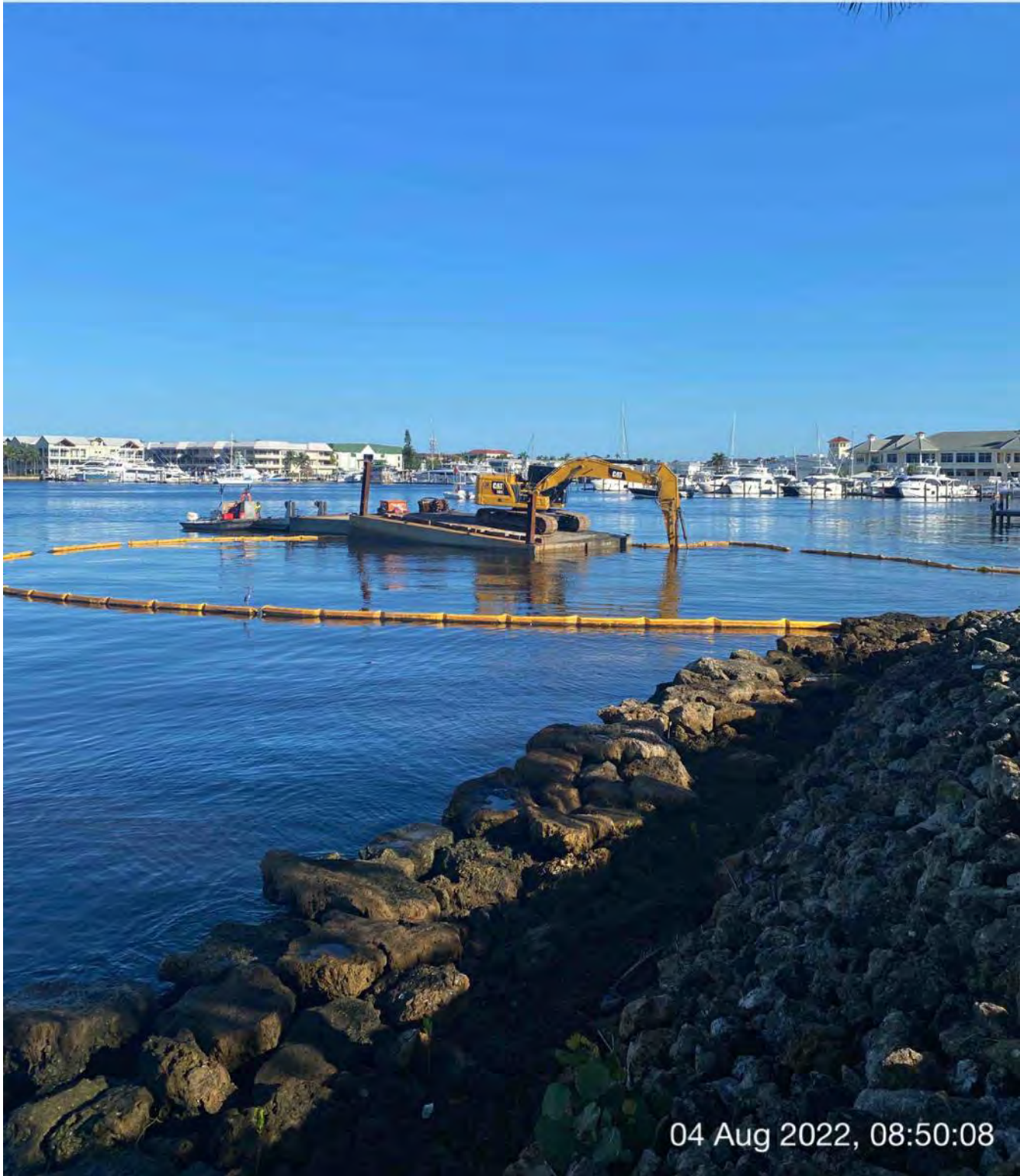
323 excavator removing material from station 0+50 in Canal BB-BB
