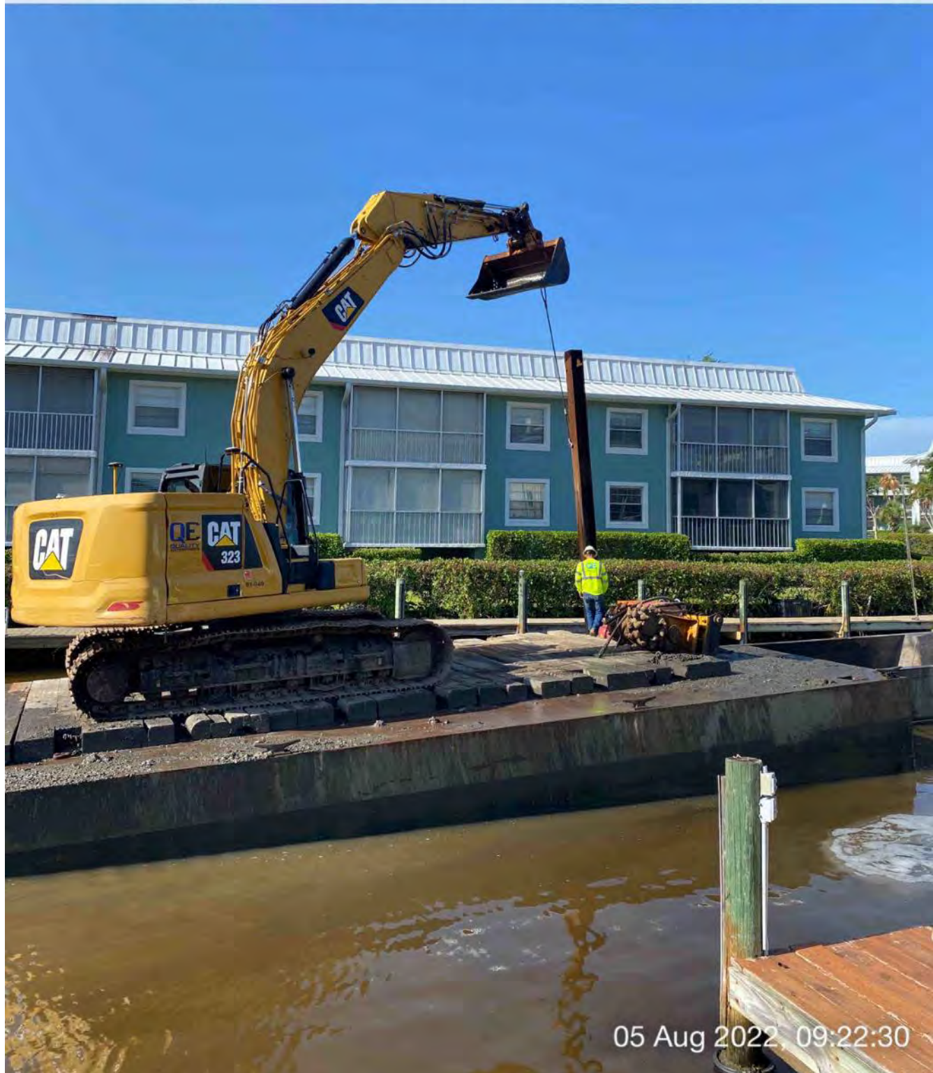
323 excavator lifting spud to allow push boat to mobilize barge at station 3+50
