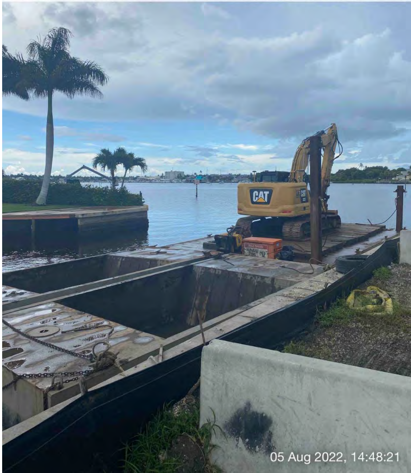
Barge, 323 excavator, and 2 hoppers staged in Canal CC-CC between stations 1+00 and 2+00
