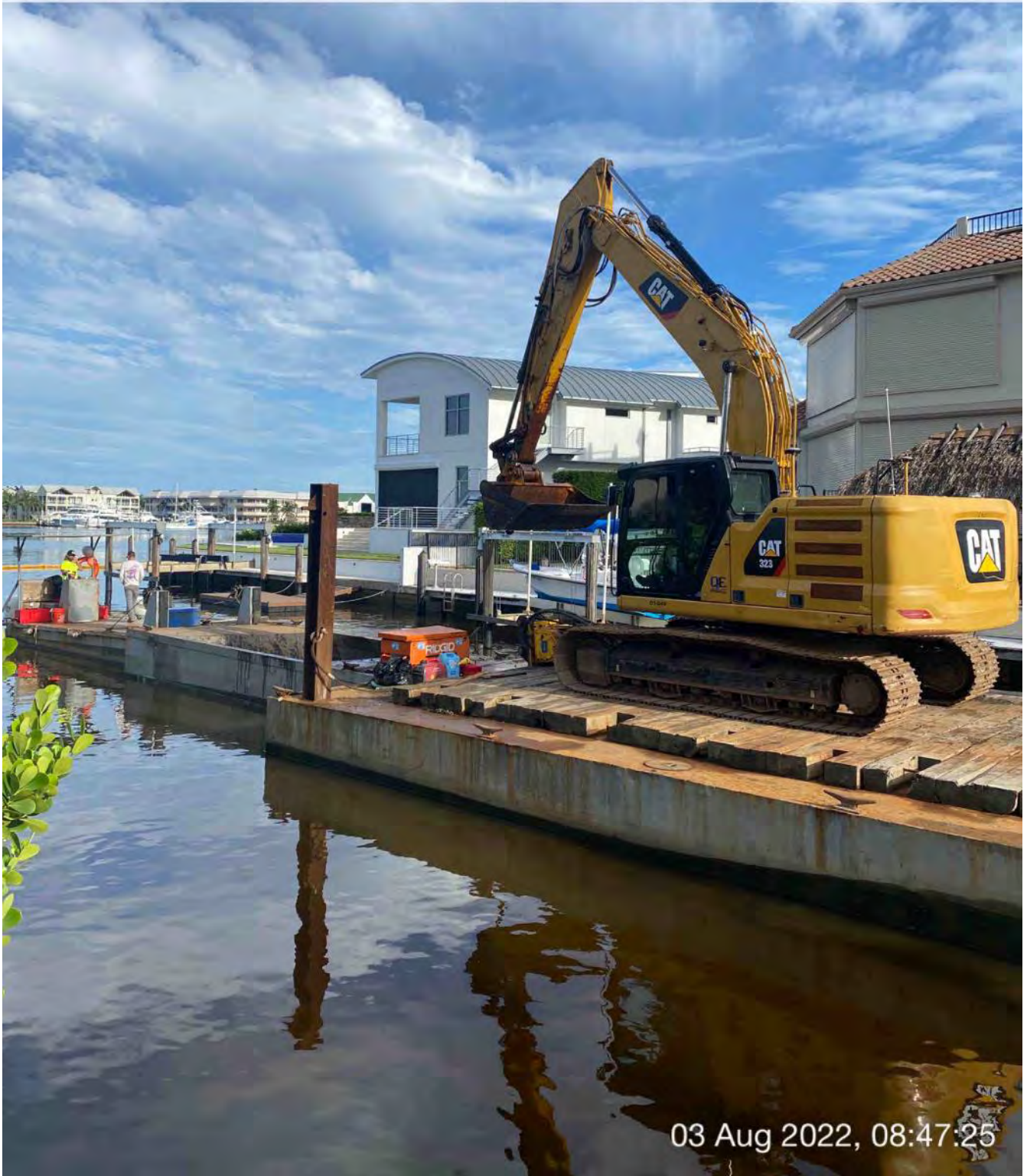
Barge, 323 excavator, hopper, and push boat between stations 2+00 and 3+00
