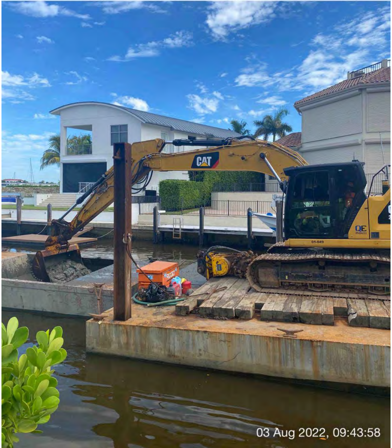
323 excavator removing material from station 3+00 and transferring to hopper
