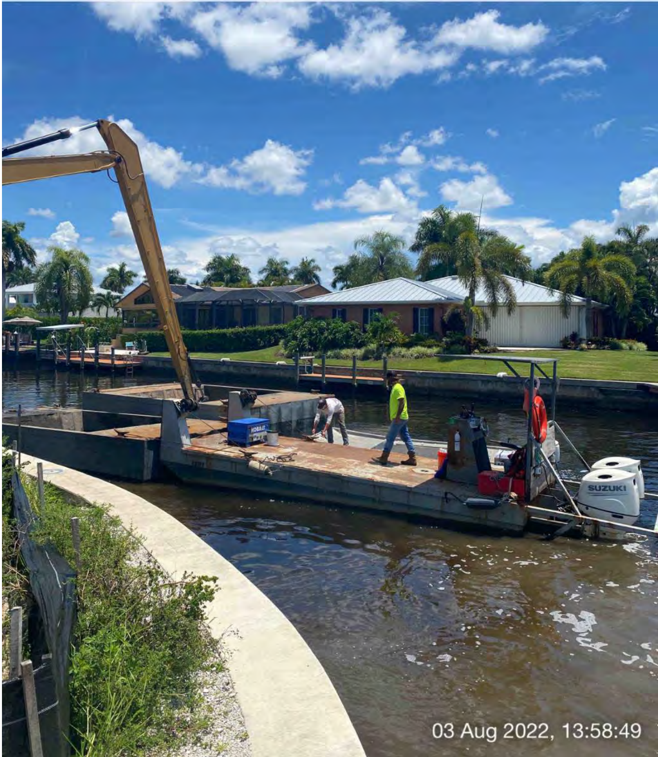
Push boat dropping off full hopper of removed material in Canal CC-CC
