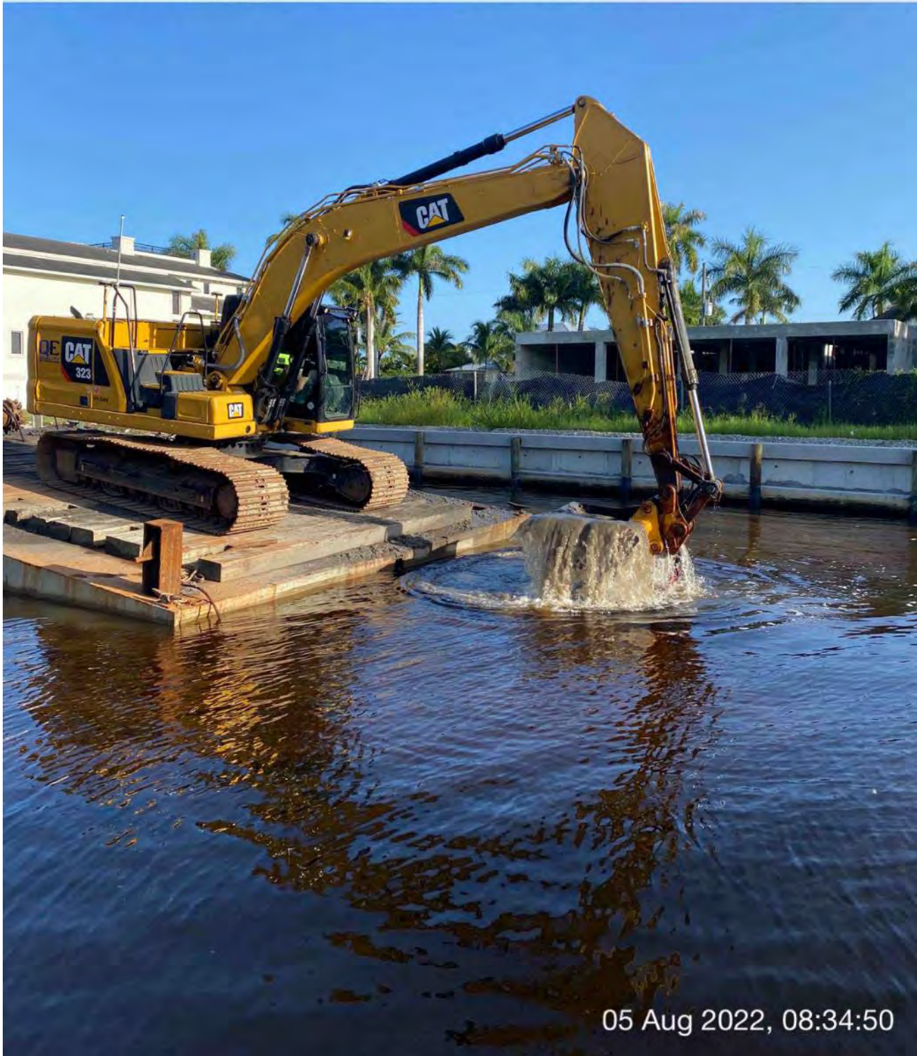
323 excavator removing material from station 4+00
