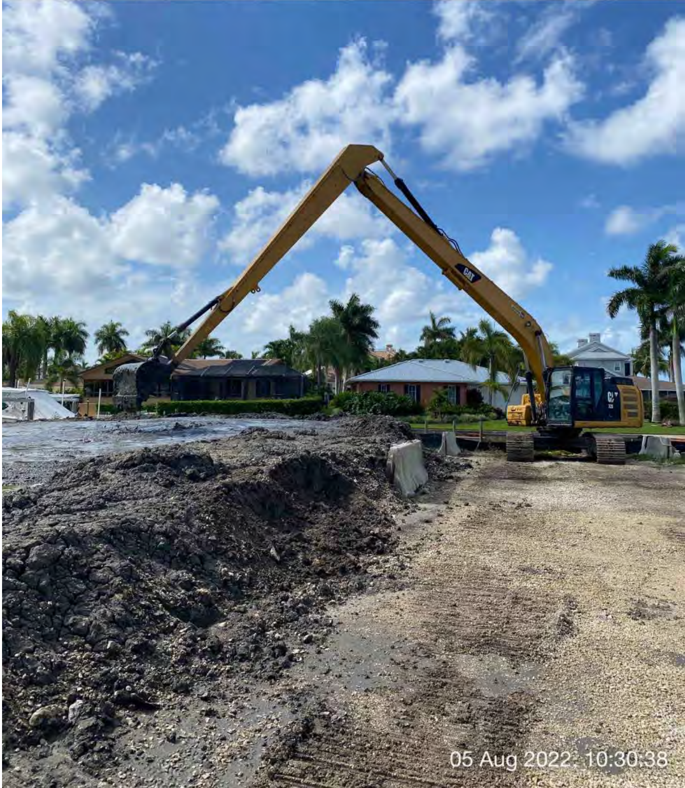
326 excavator transferring removed material from hopper to dewatering site at 1300 Curlew Avenue
