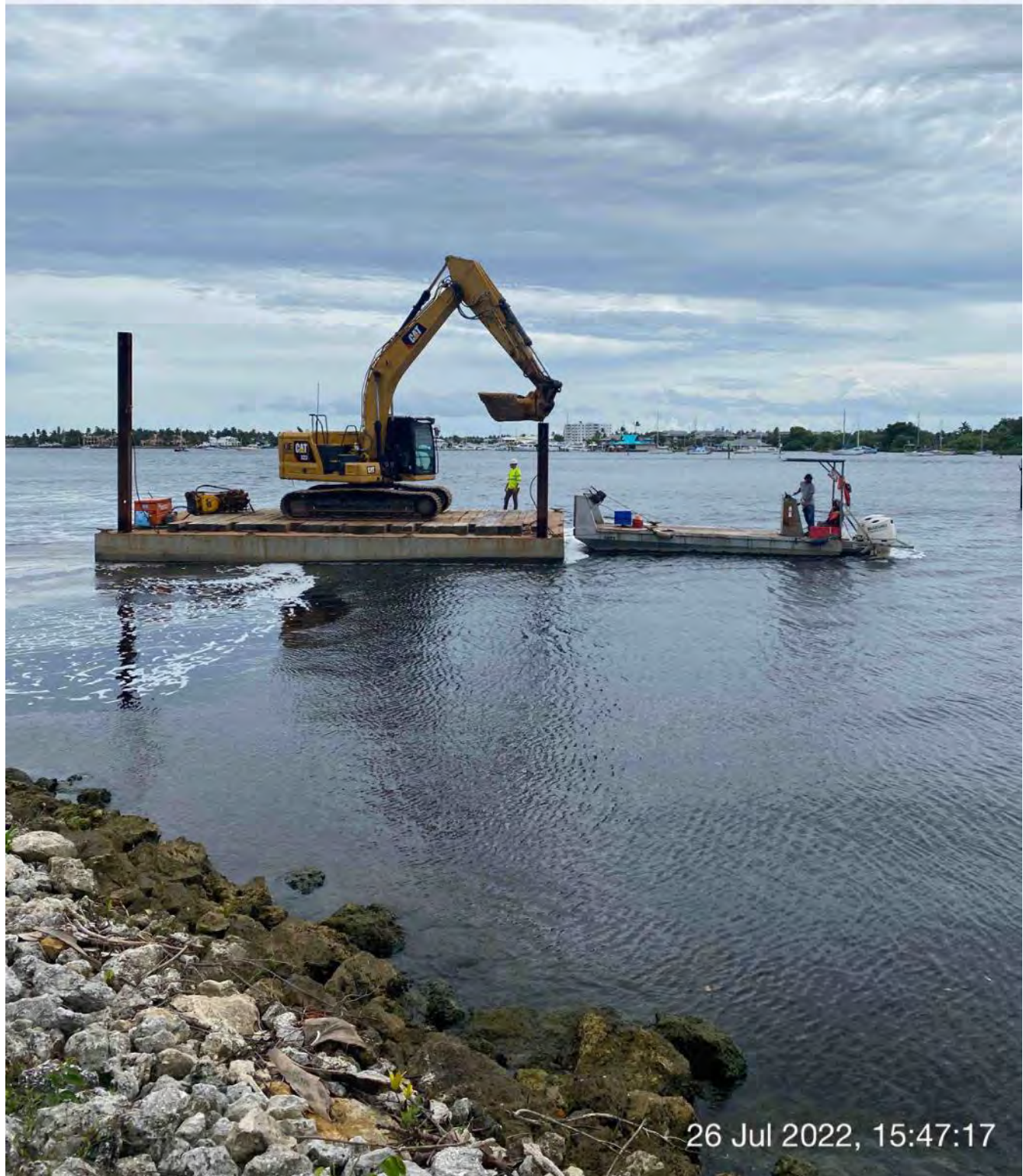
323 excavator lifting spud to allow push boat to transport barge from Canal CC-CC to Canal BB-BB
