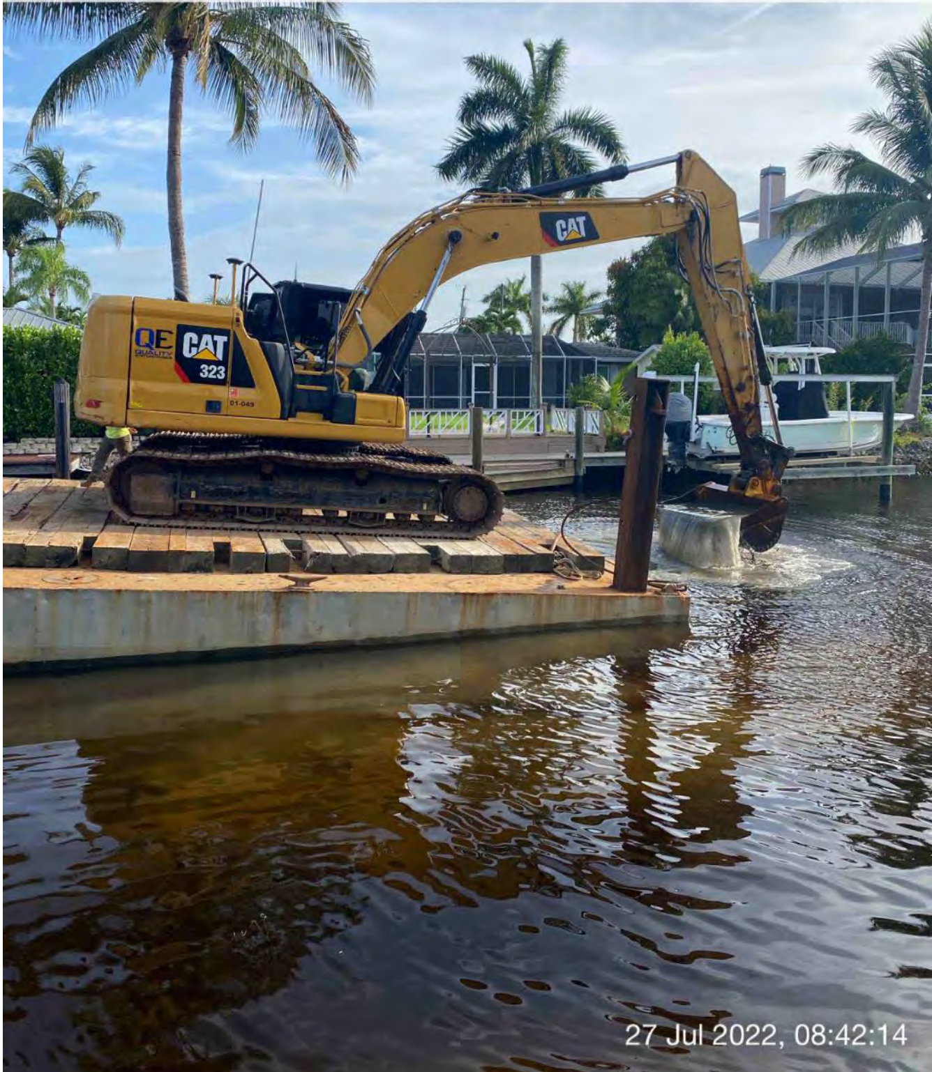
323 excavator removing material from station 8+50
