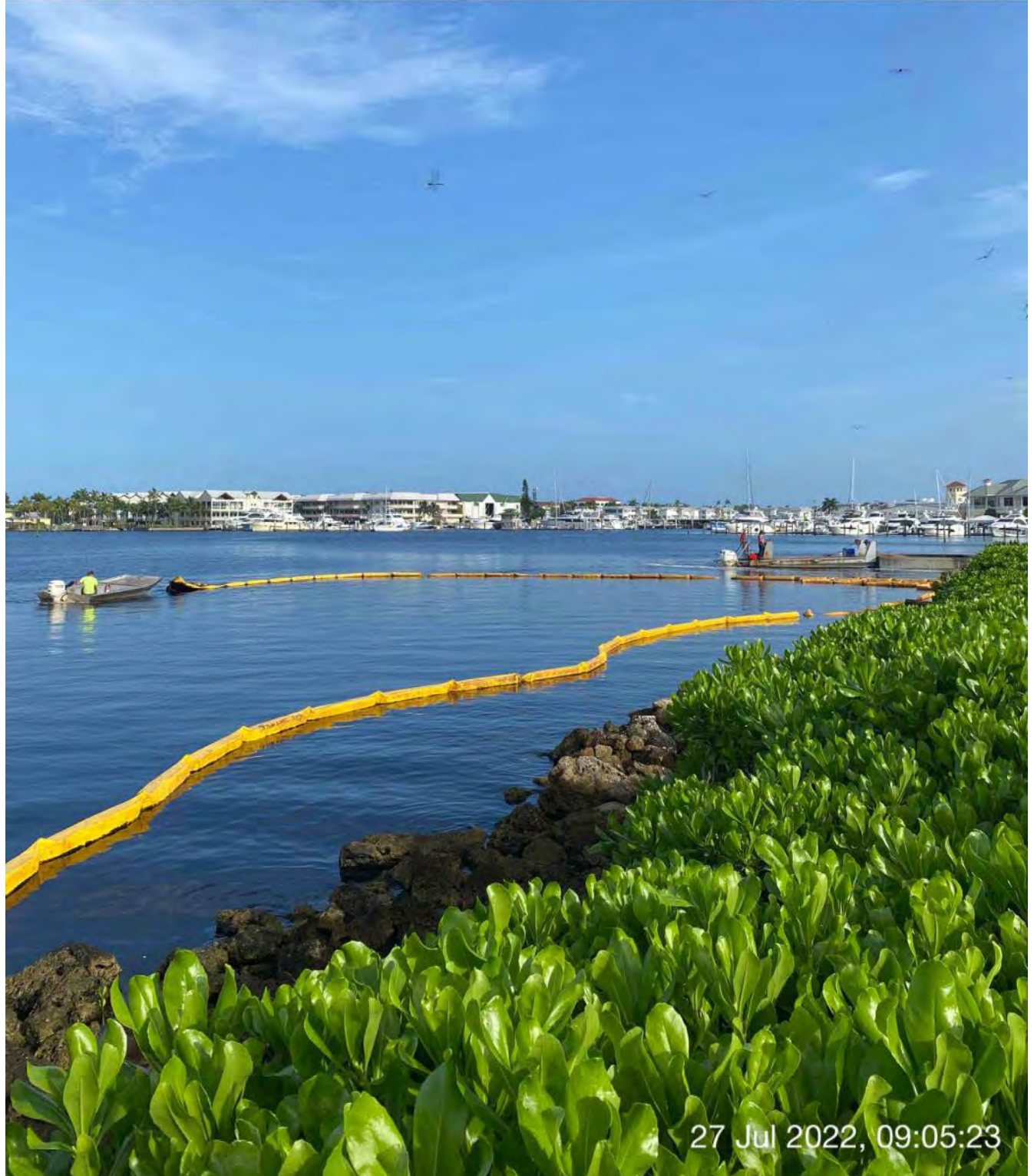
Support boat opening turbidity curtain to allow push boat to transport hopper from Canal BB-BB to Canal CC-CC
