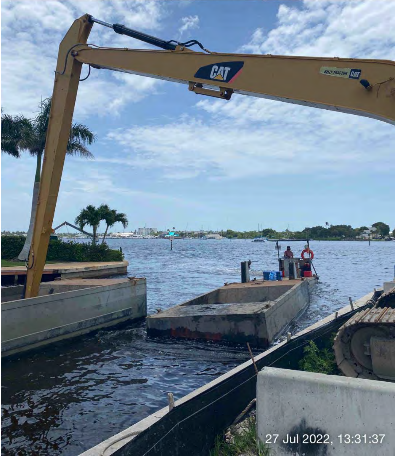
Push boat dropping off full hopper of removed material in Canal CC-CC and picking up empty hopper
