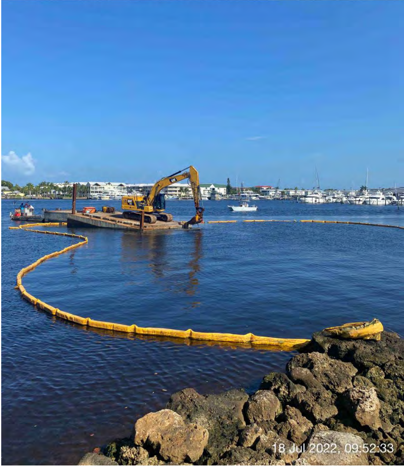
323 excavator removing material from station 0+00
