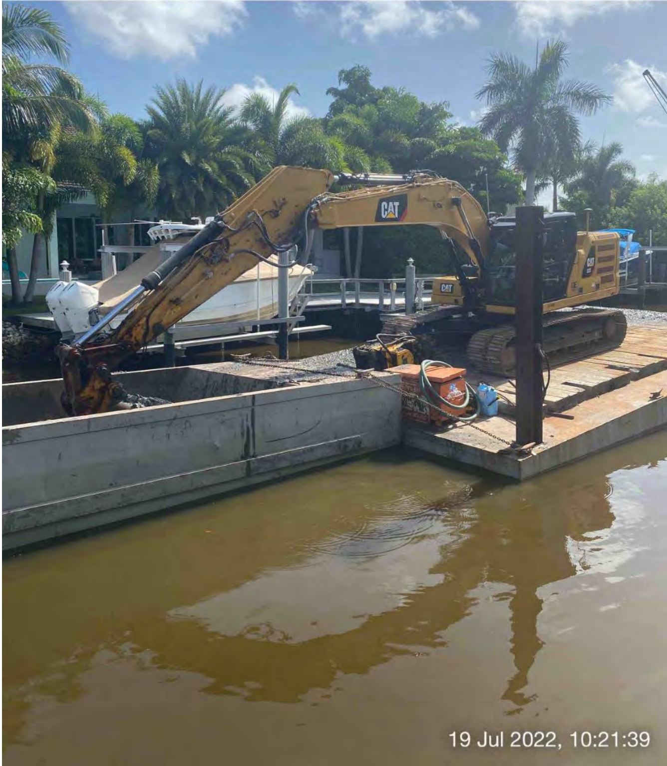
323 excavator removing material from station 11+25 and transferring to hopper
