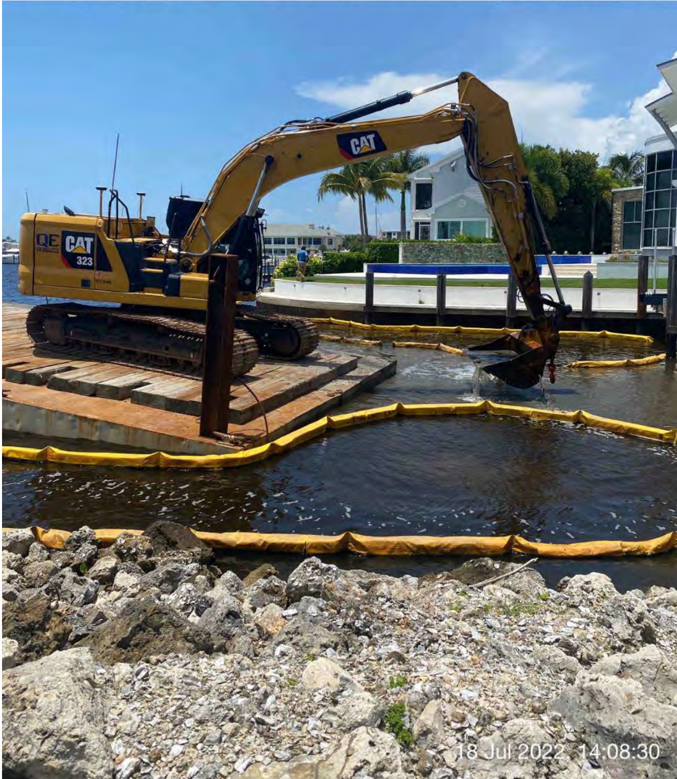
323 excavator removing material from station 1+50
