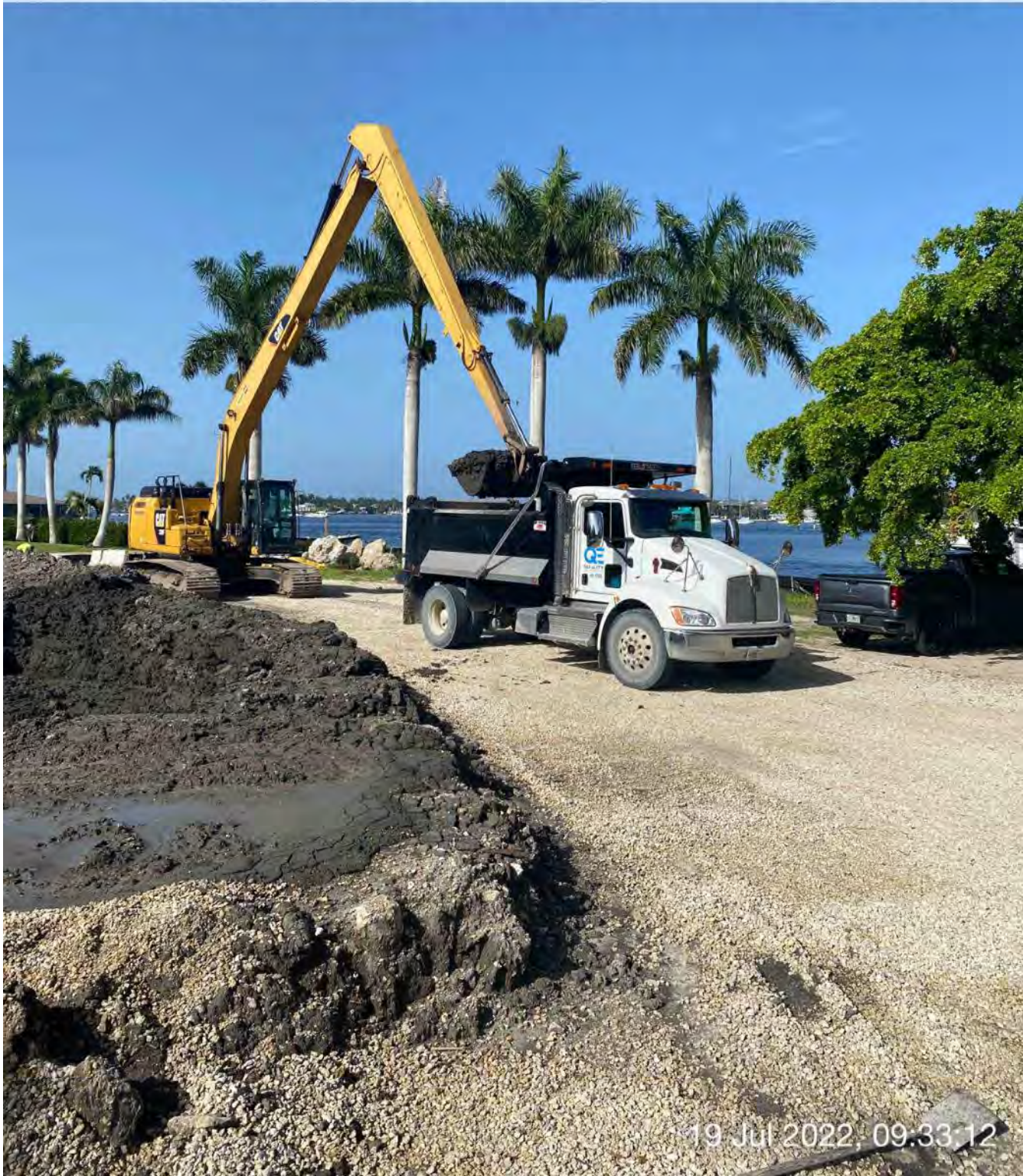
326 excavator transporting removed material from dewatering site to dump truck bed
