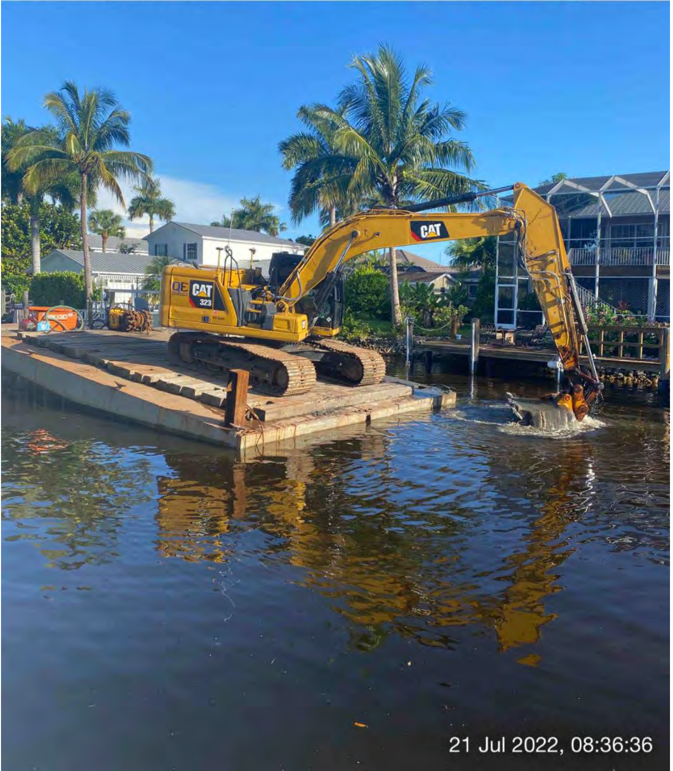
323 excavator removing material from station 9+00
