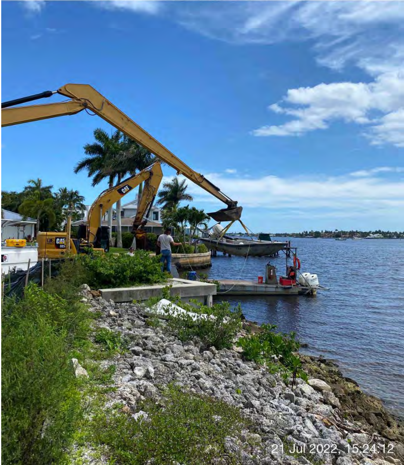
326 excavator transporting support boat from 1300 Curlew Avenue to water
