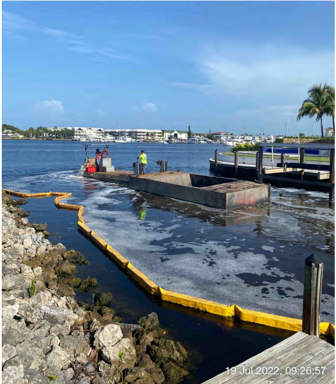
Push boat transporting full hopper of removed material from Canal BB-BB to Canal CC-CC
