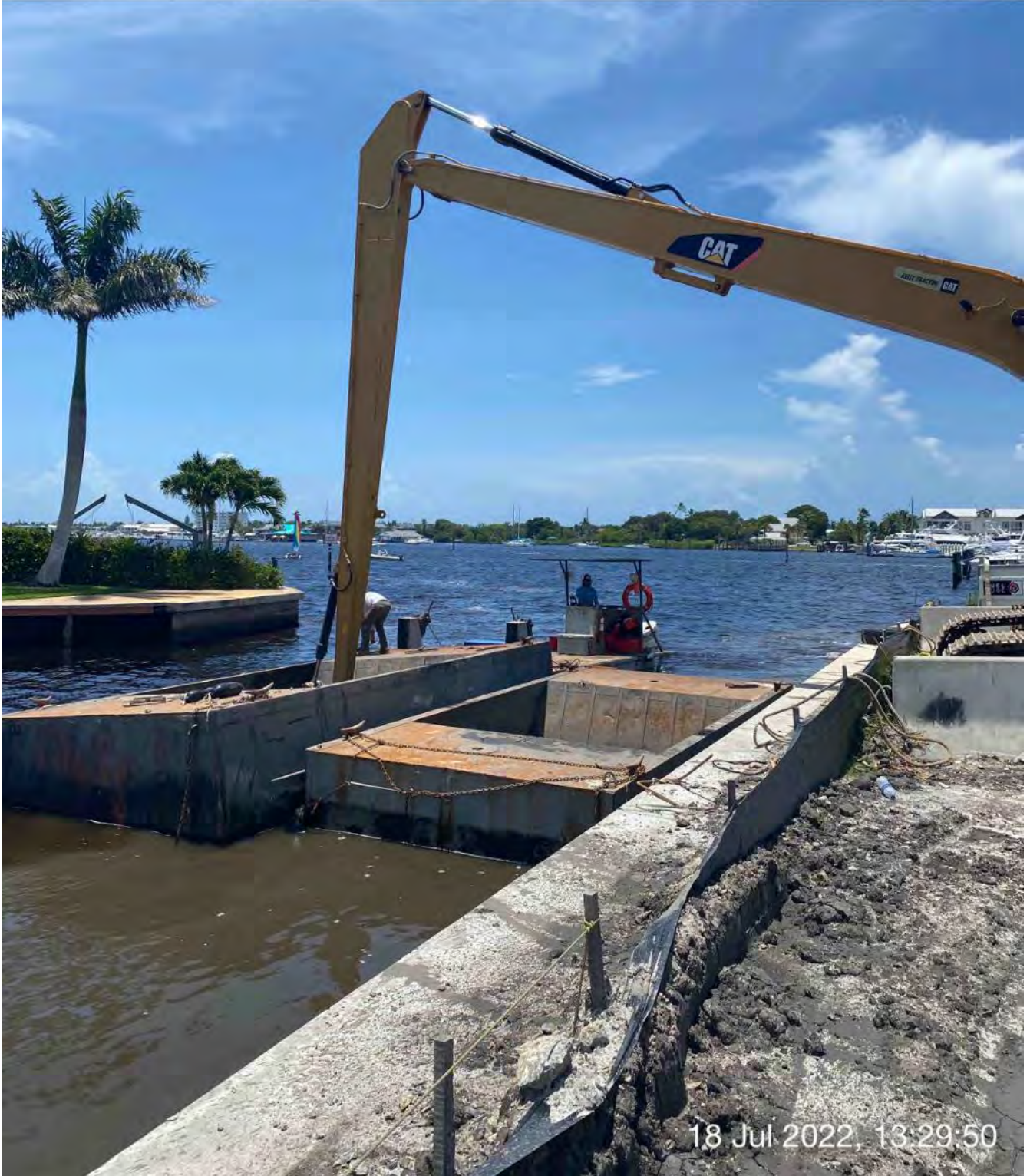
Push boat dropping off full hopper of removed material in Canal CC-CC and picking up empty hopper
