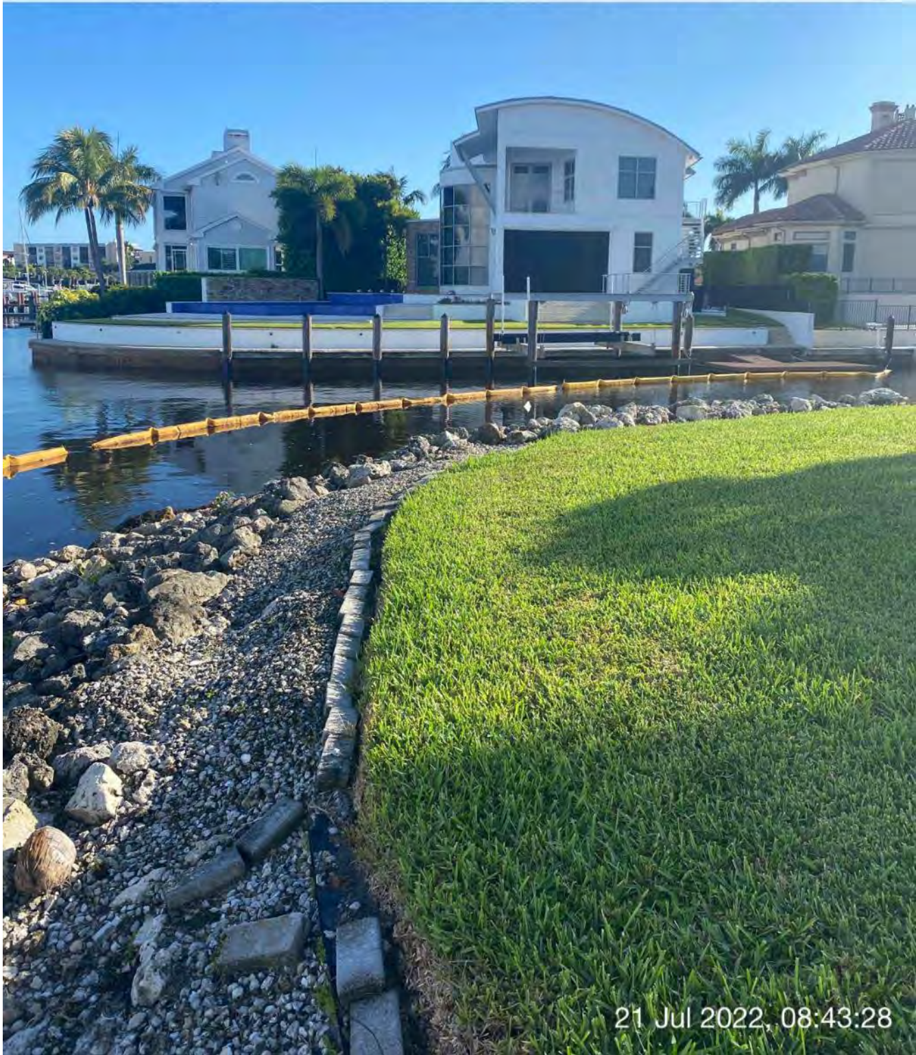
Turbidity curtain installed across the mouth of Canal BB-BB
