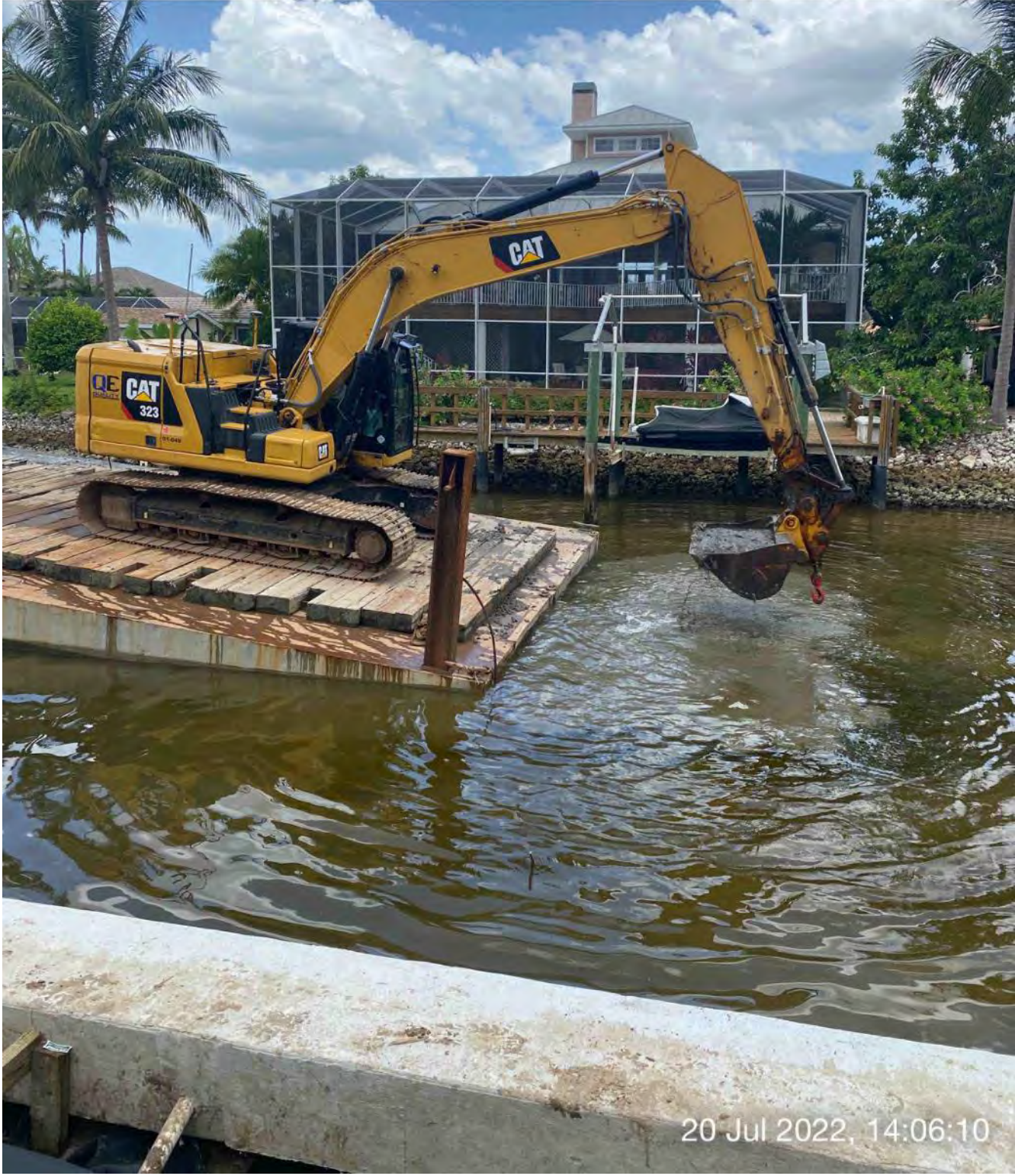
323 excavator removing material from station 9+00
