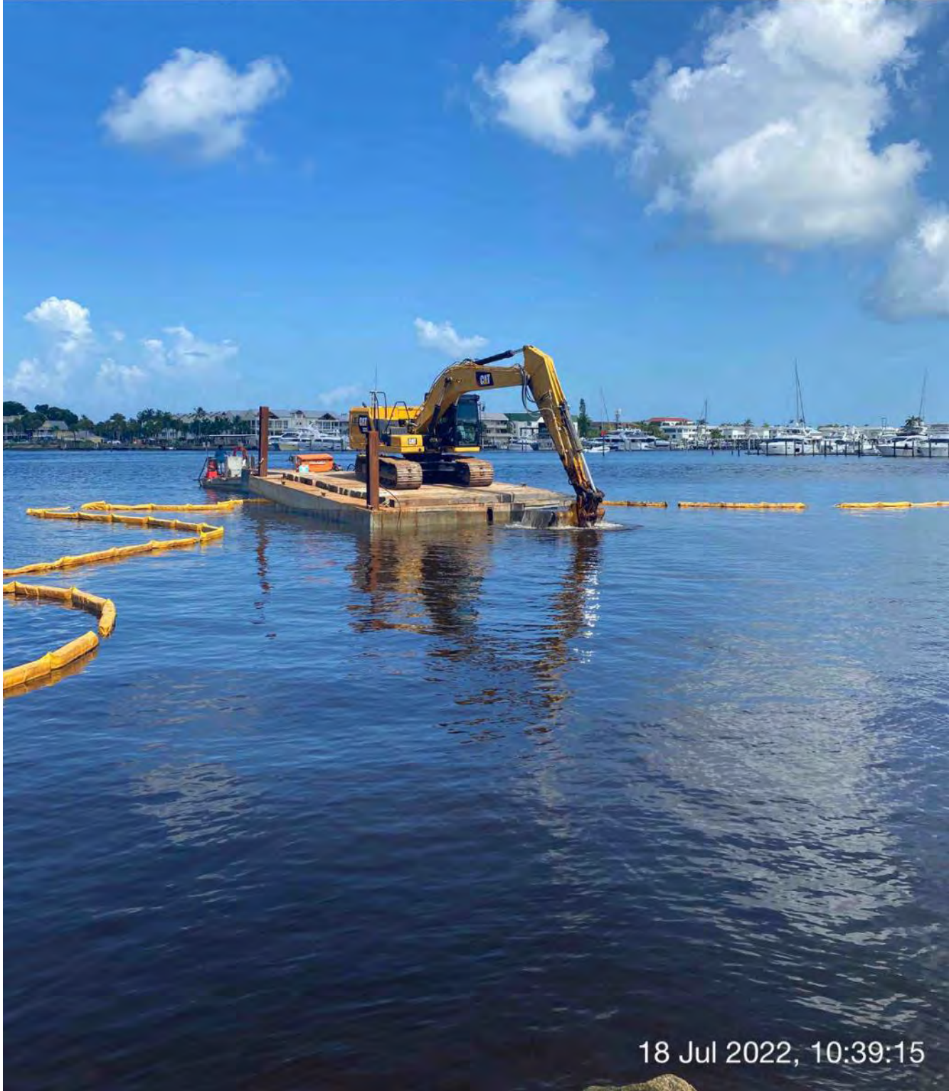
323 excavator removing material from station 0+50
