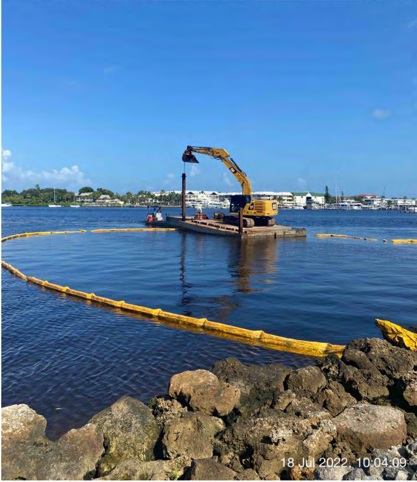
323 excavator lifting spud to allow push boat to mobilize barge at station 0+00
