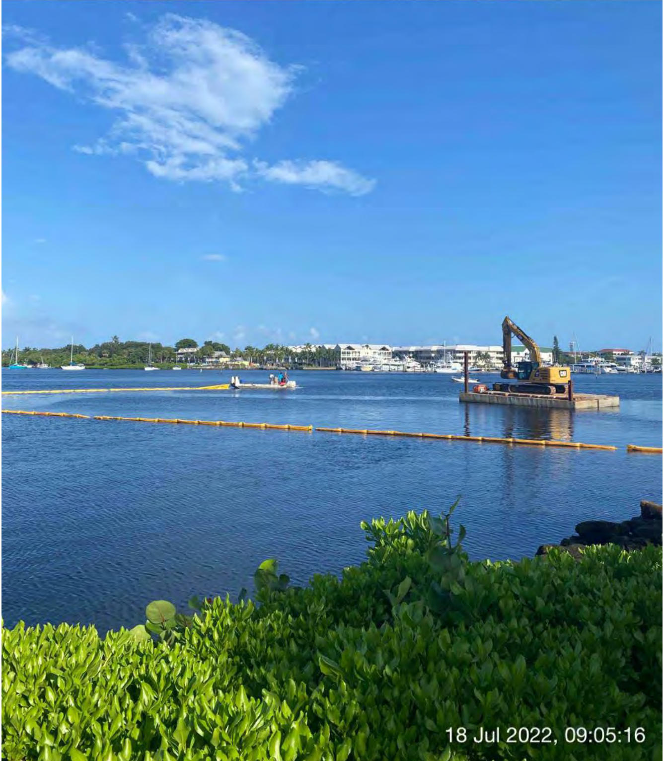
Push boat installing turbidity curtain across the mouth of Canal BB-BB
