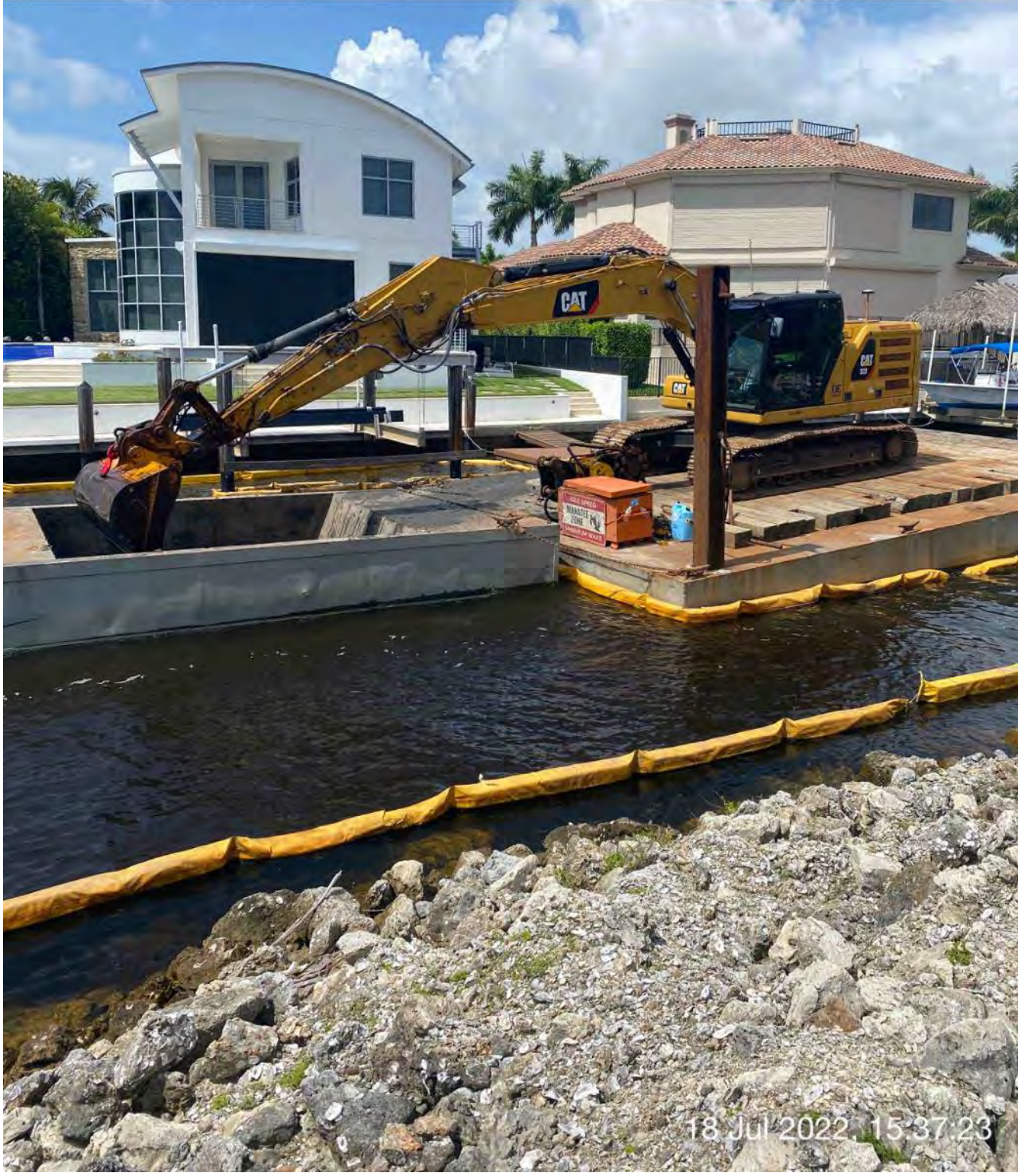
323 excavator removing material from station 2+00 and transferring to hopper
