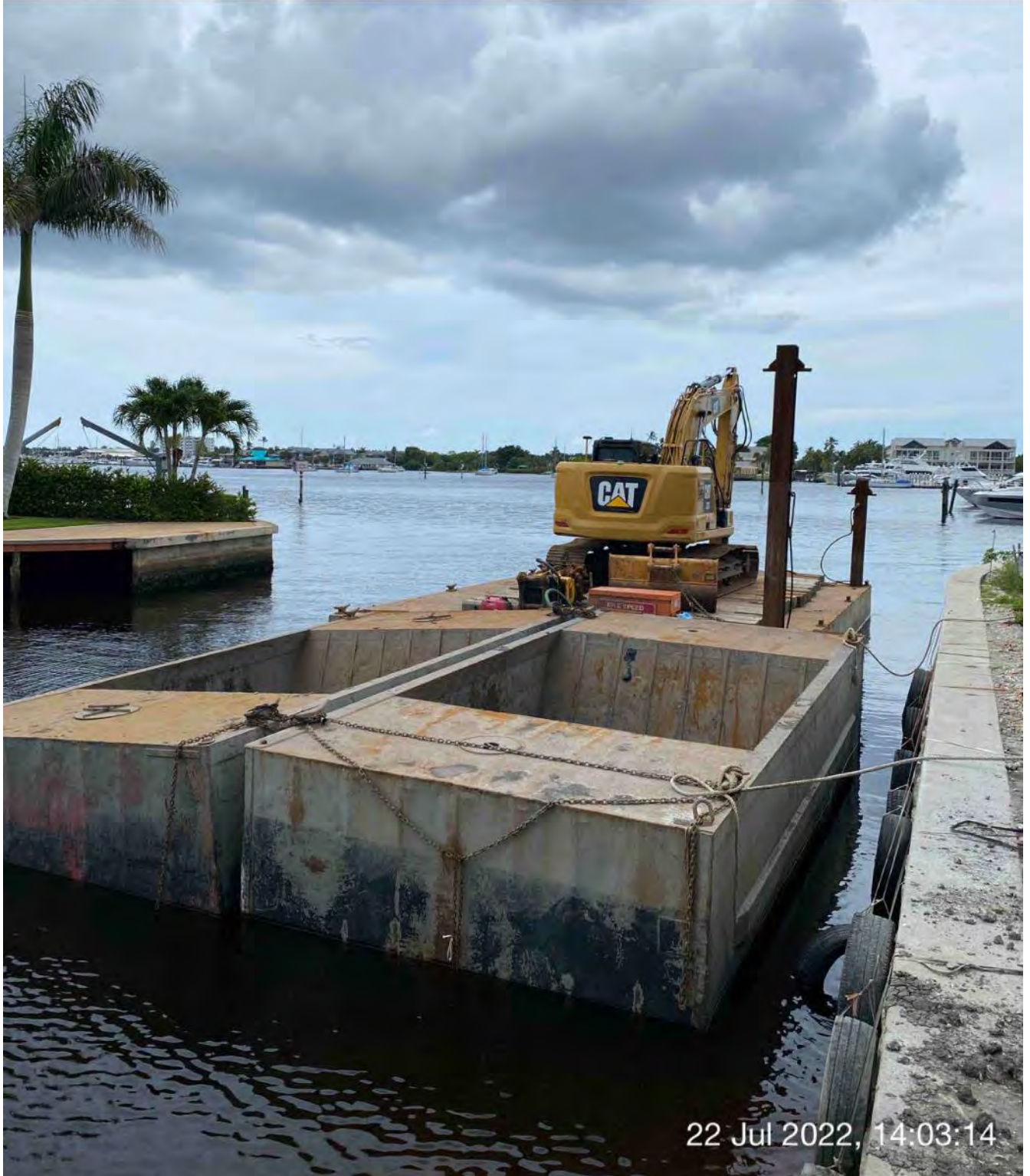
2 hoppers, barge, and 323 excavator staged in canal CC-CC between stations 1+00 and 2+00
