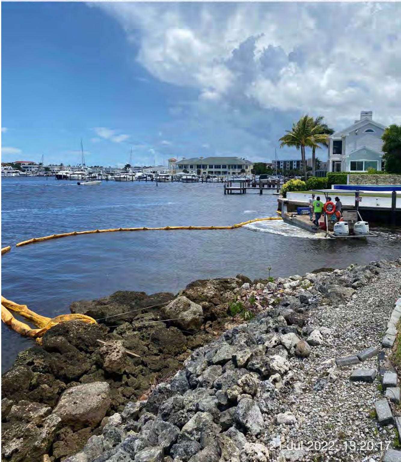
Push boat opening turbidity curtain
