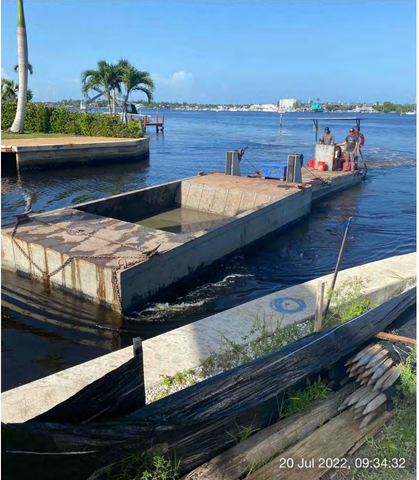
Push boat dropping off full hopper of material in Canal CC-CC
