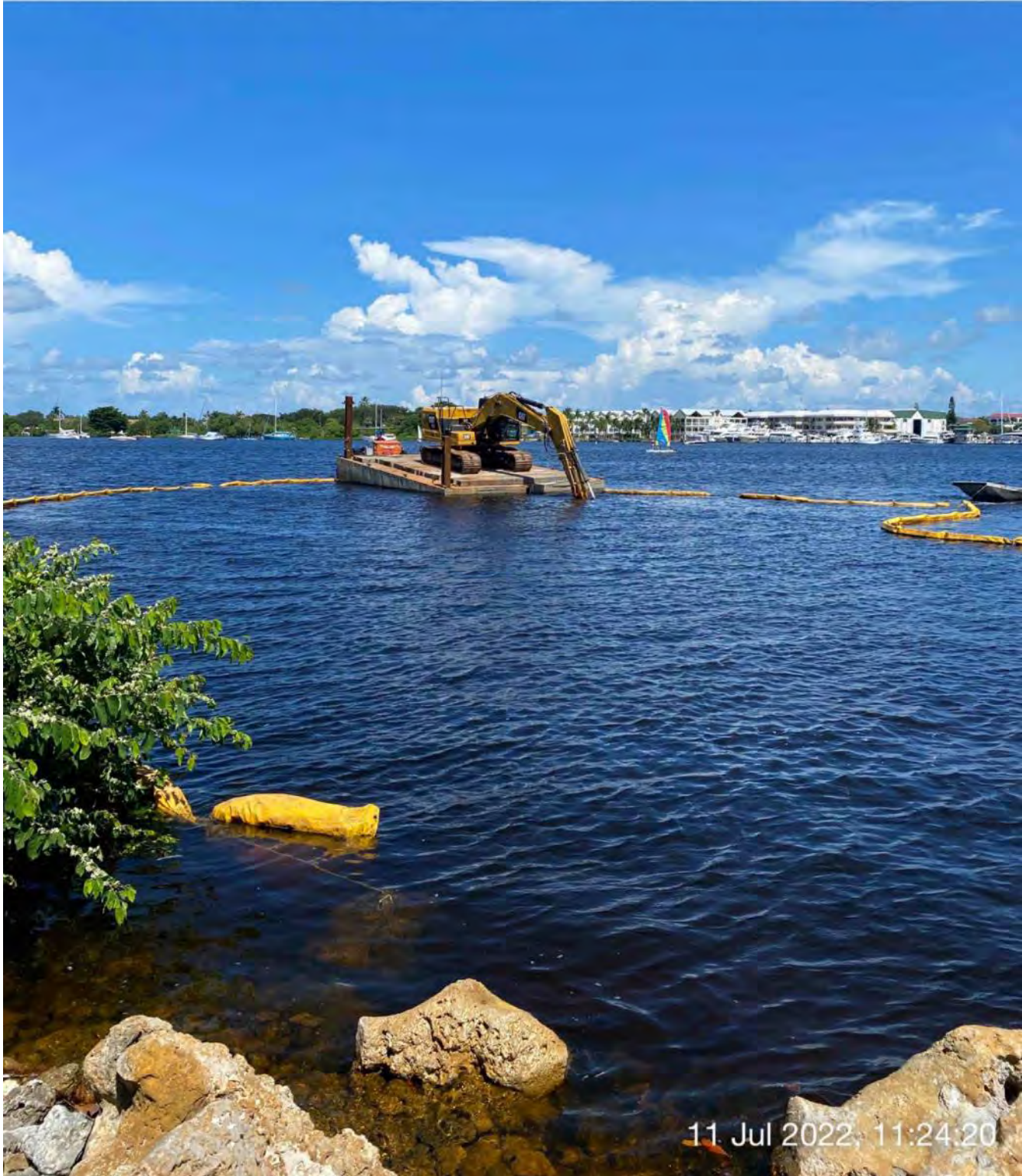
323 excavator grinding rock at station 0+25
