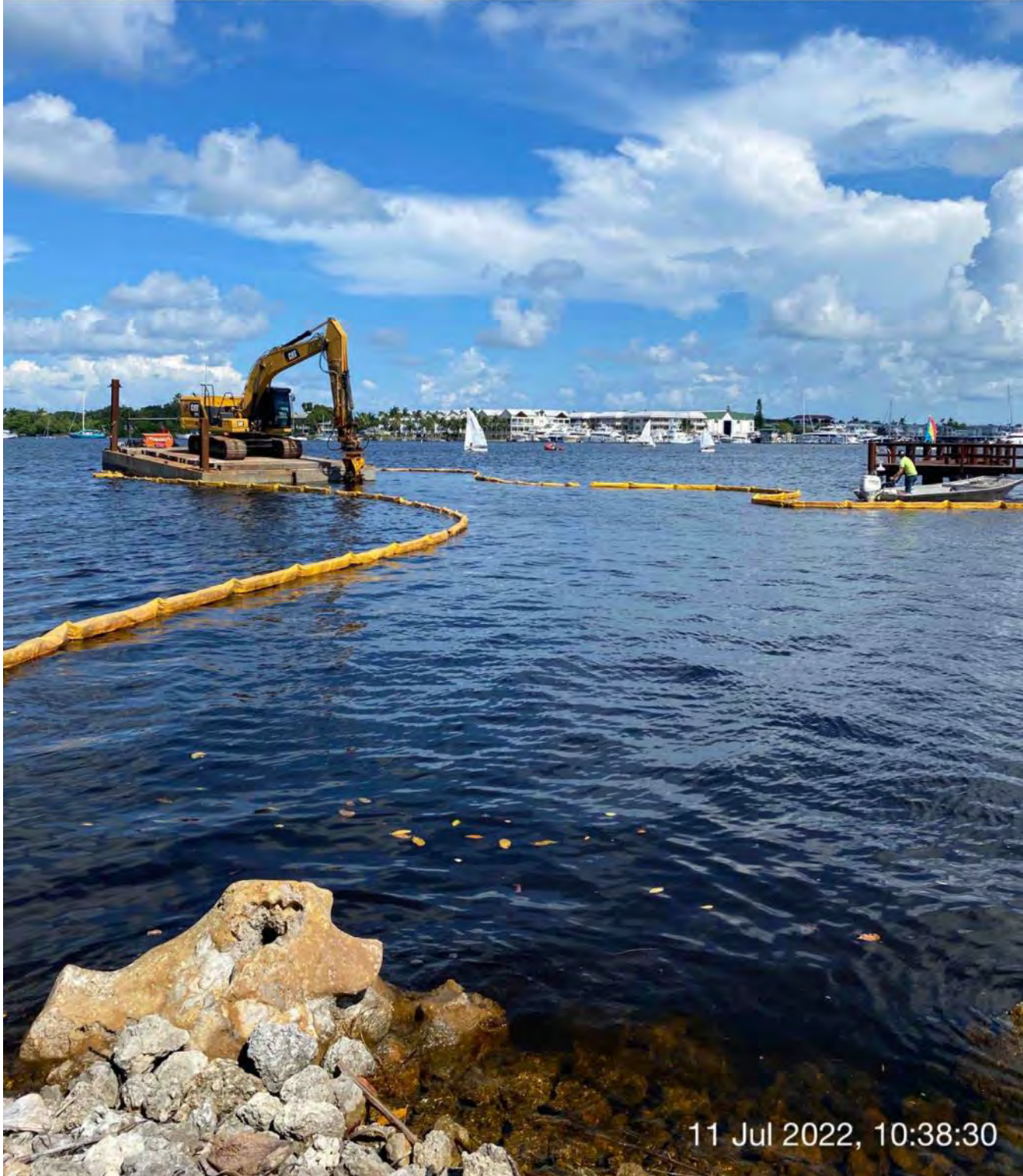
323 excavator grinding rock at station 0+00
