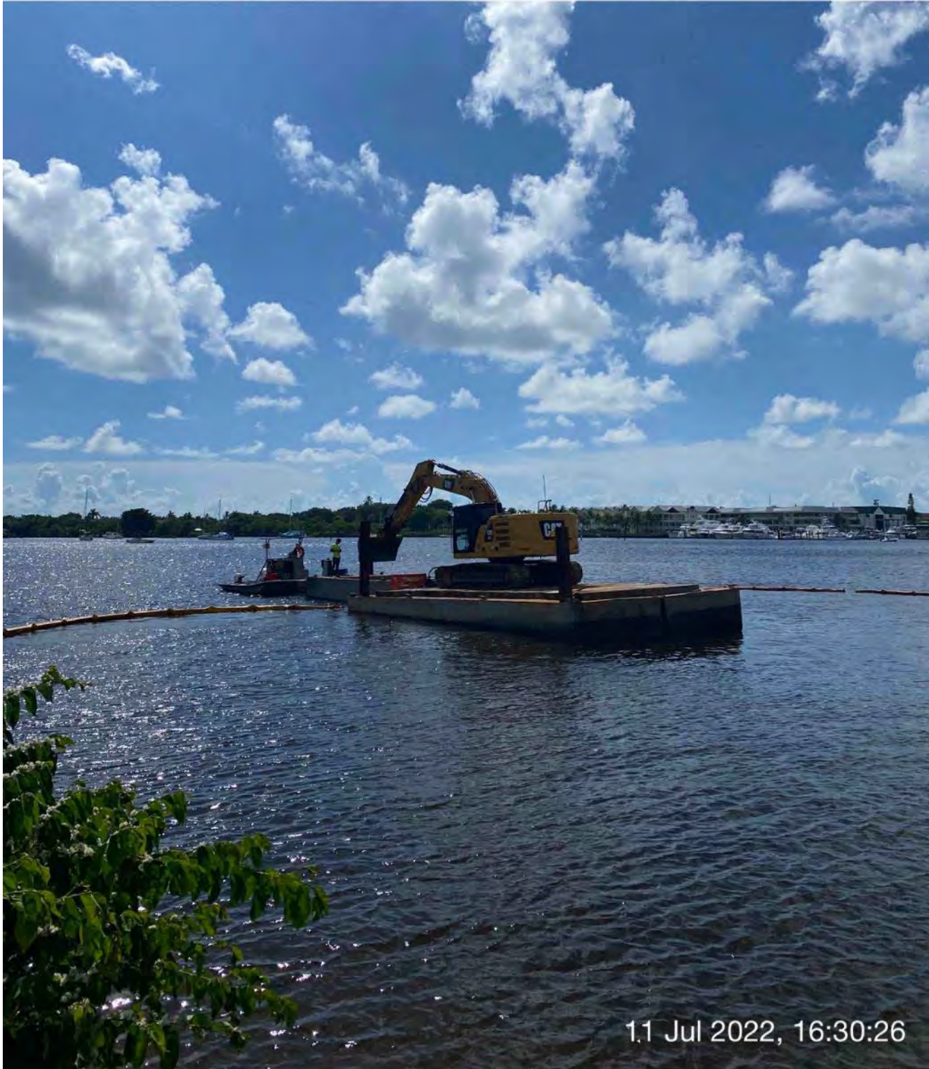
323 excavator removing material from station 0+25 and transferring to hopper
