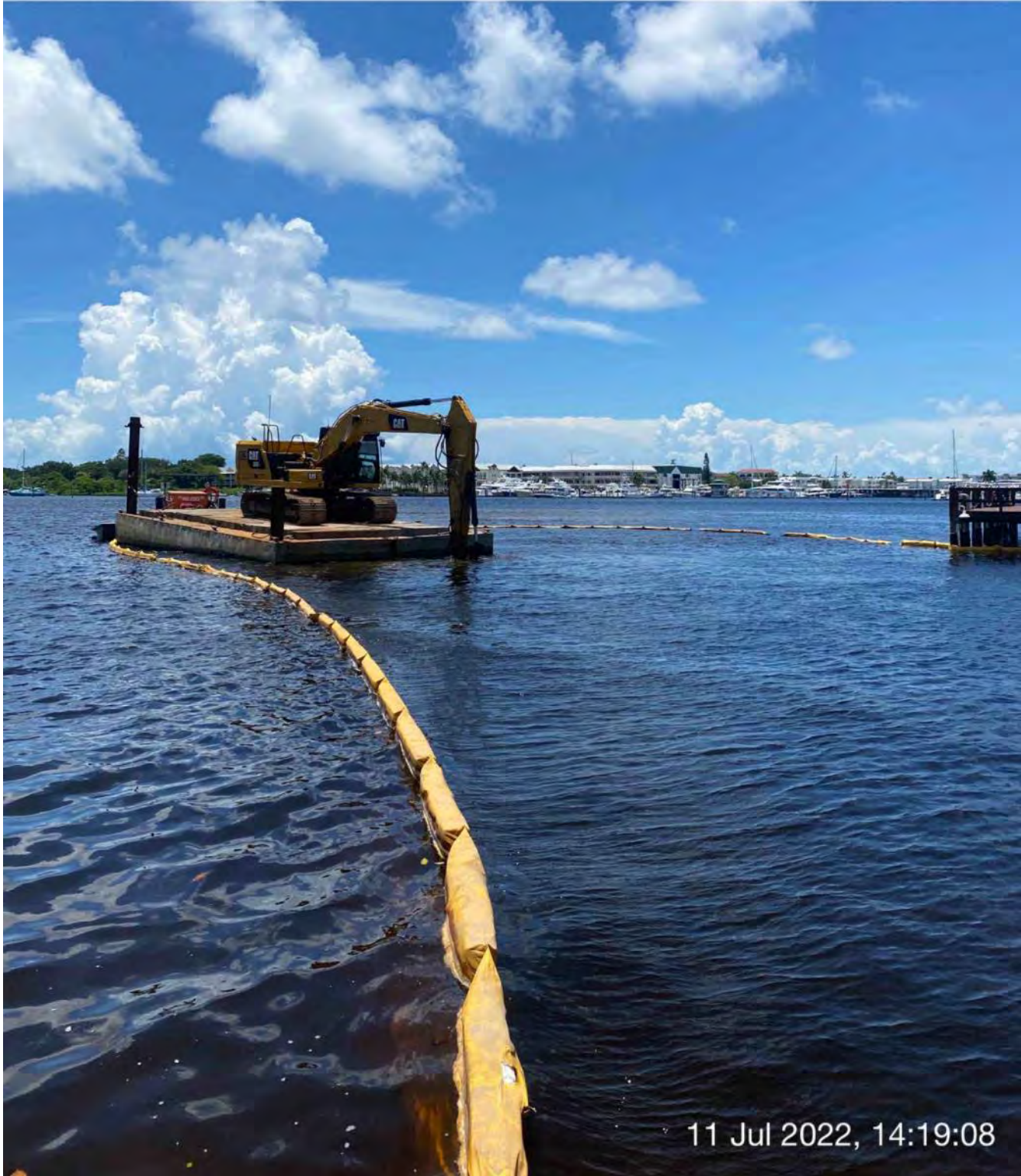
323 excavator grinding rock at station 0+50
