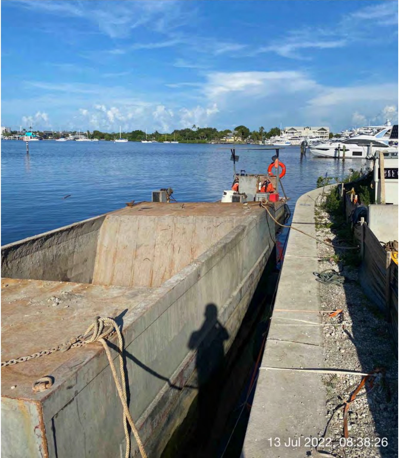
Hopper and push boat staged in Canal CC-CC between stations 1+00 and 1+50
