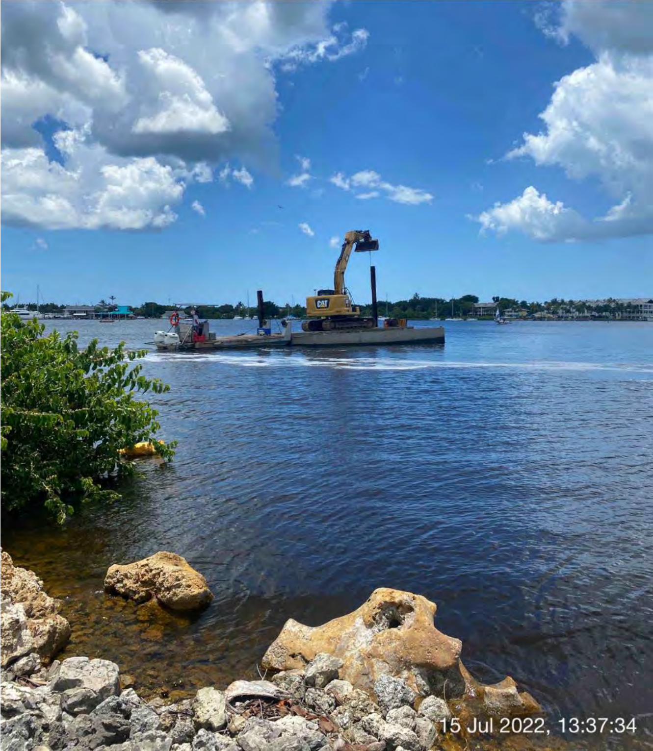
323 excavator lifting spud to allow push boat to transport barge and 323 excavator from Canal X-X to Canal CC-CC
