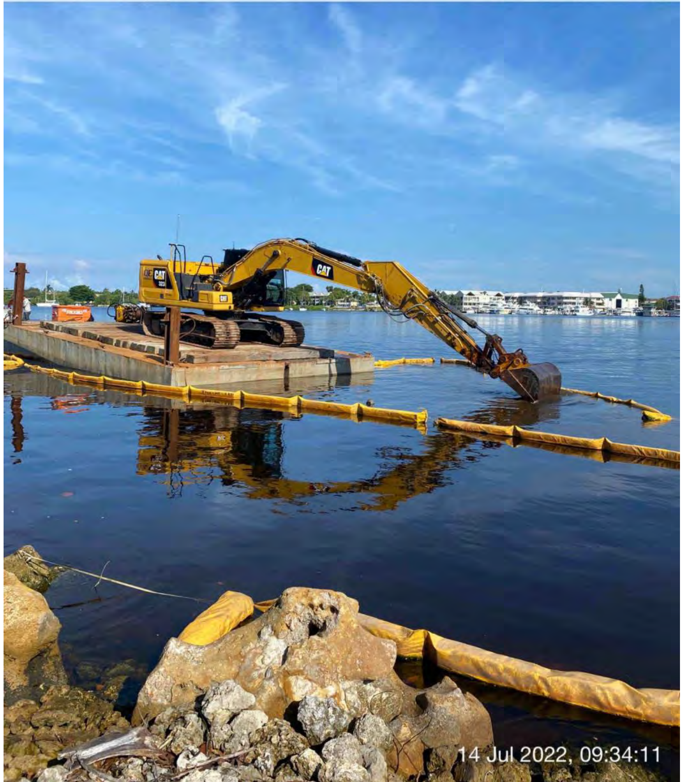
323 excavator removing material from station 0+75 and transferring to hopper
