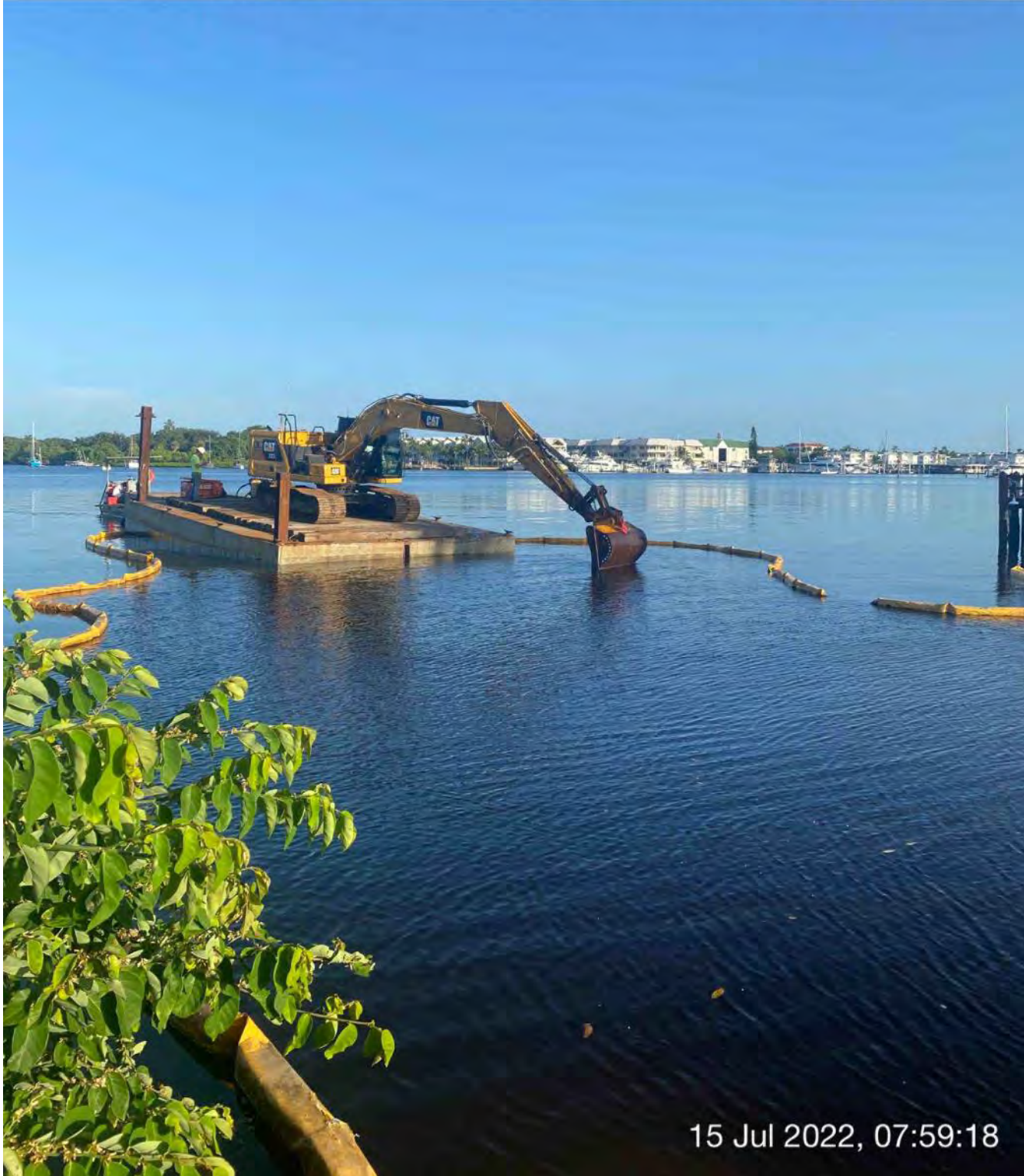
323 excavator removing material from station 0+25
