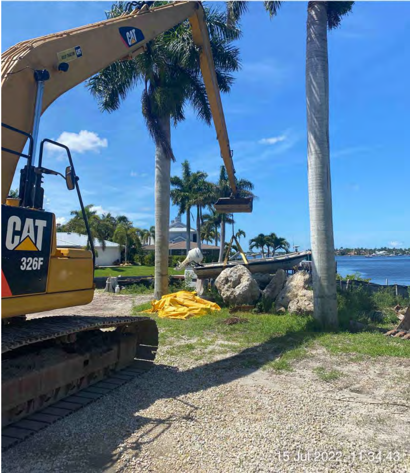
326 excavator moving support boat to southwest corner of 1300 Curlew Avenue
