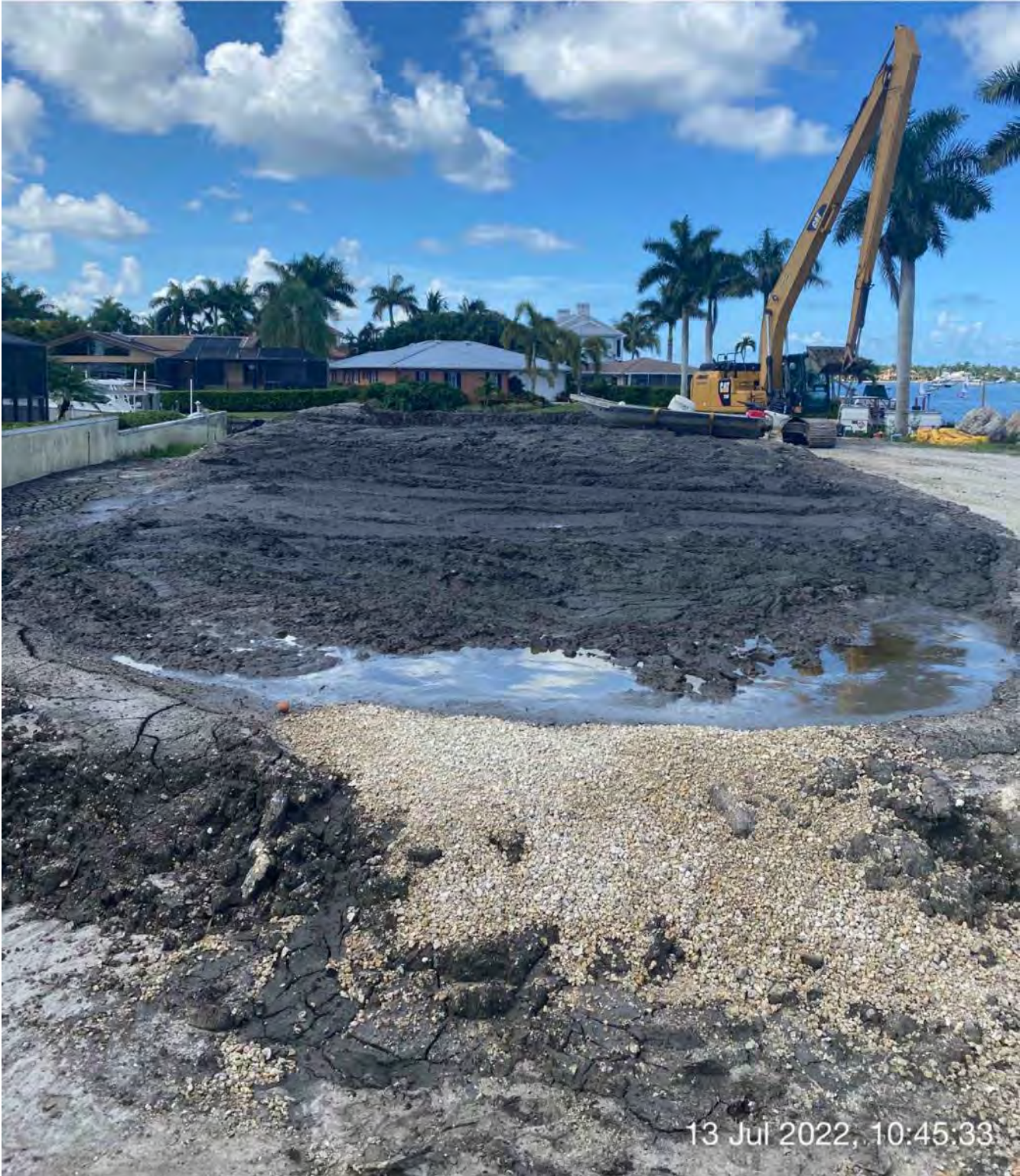
Removed material at dewatering site at 1300 Curlew Avenue
