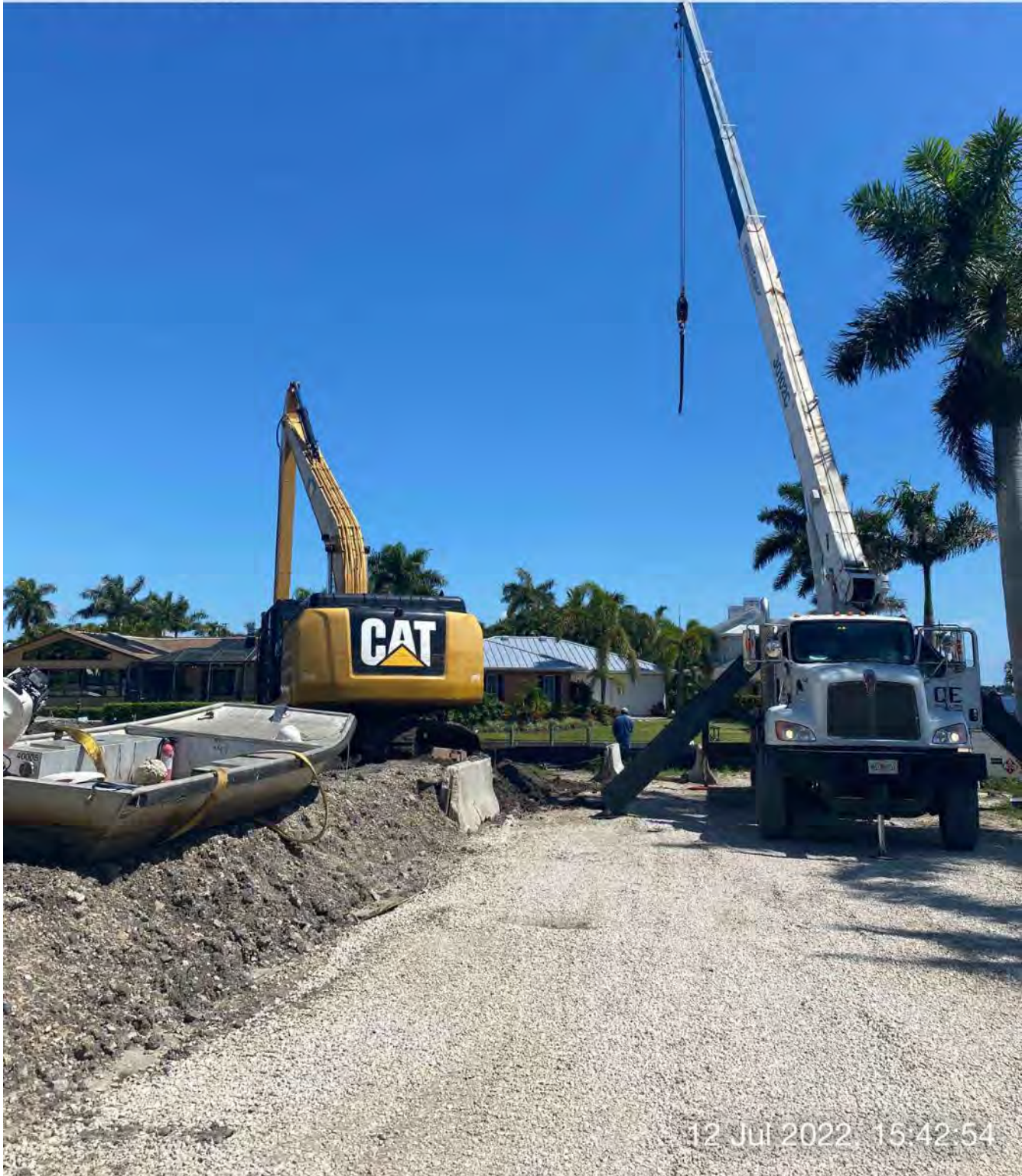
326 excavator, crane truck, and support boat on site at 1300 Curlew Avenue
