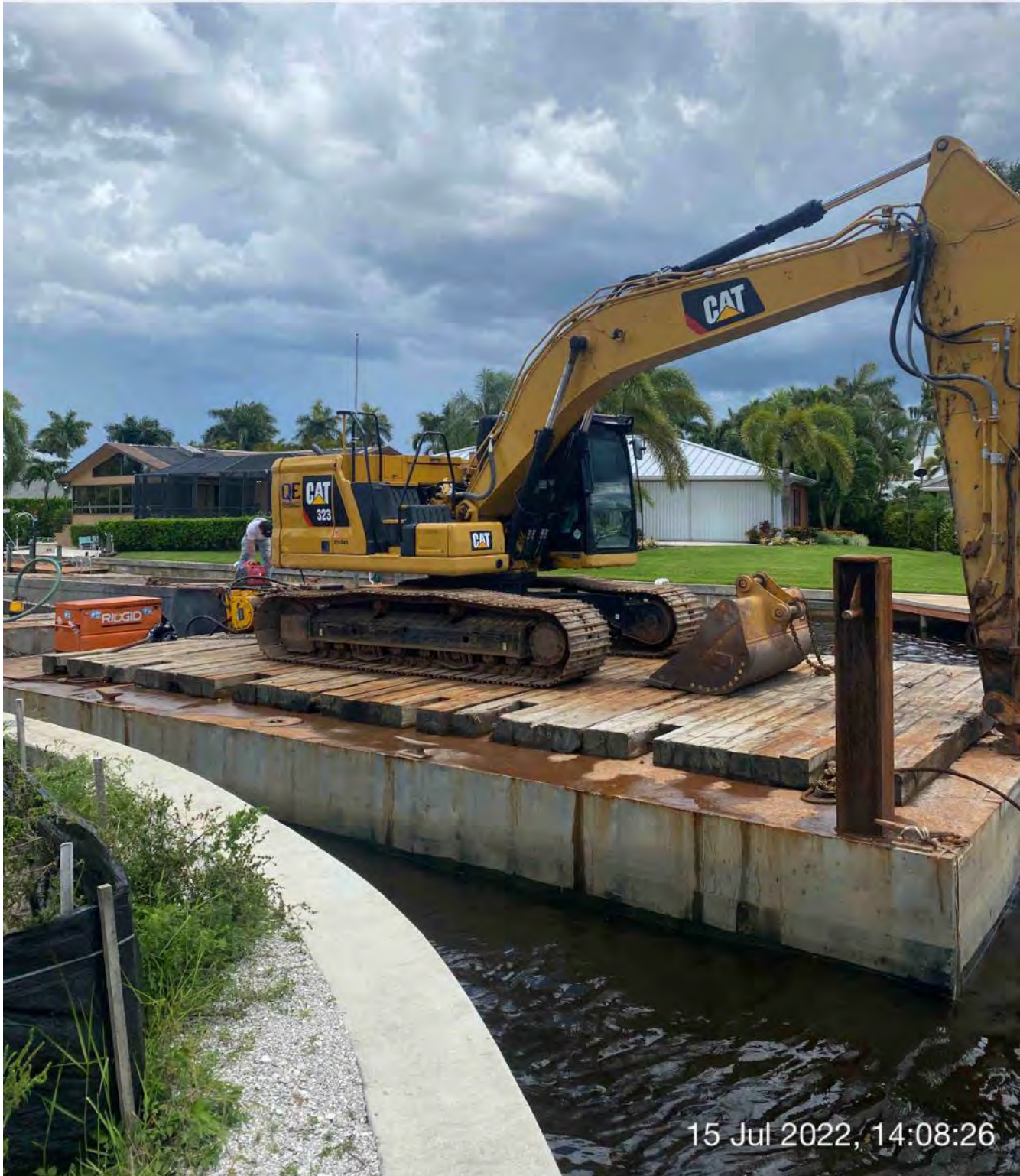
Barge, 323 excavator, and 2 hoppers staged in Canal CC-CC between stations 1+00 and 1+50
