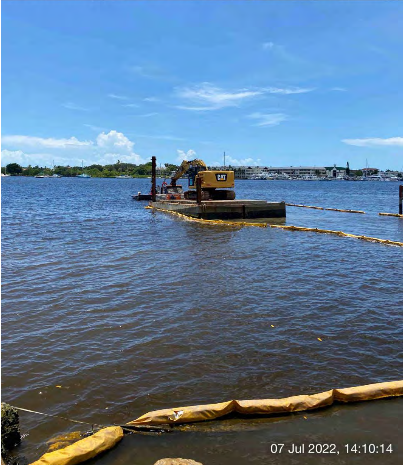
323 excavator removing material and transferring it to hopper at station 0+50
