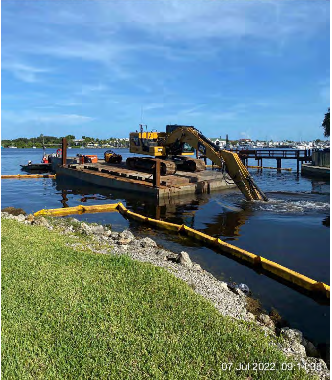
323 excavator removing material from station 1+50
