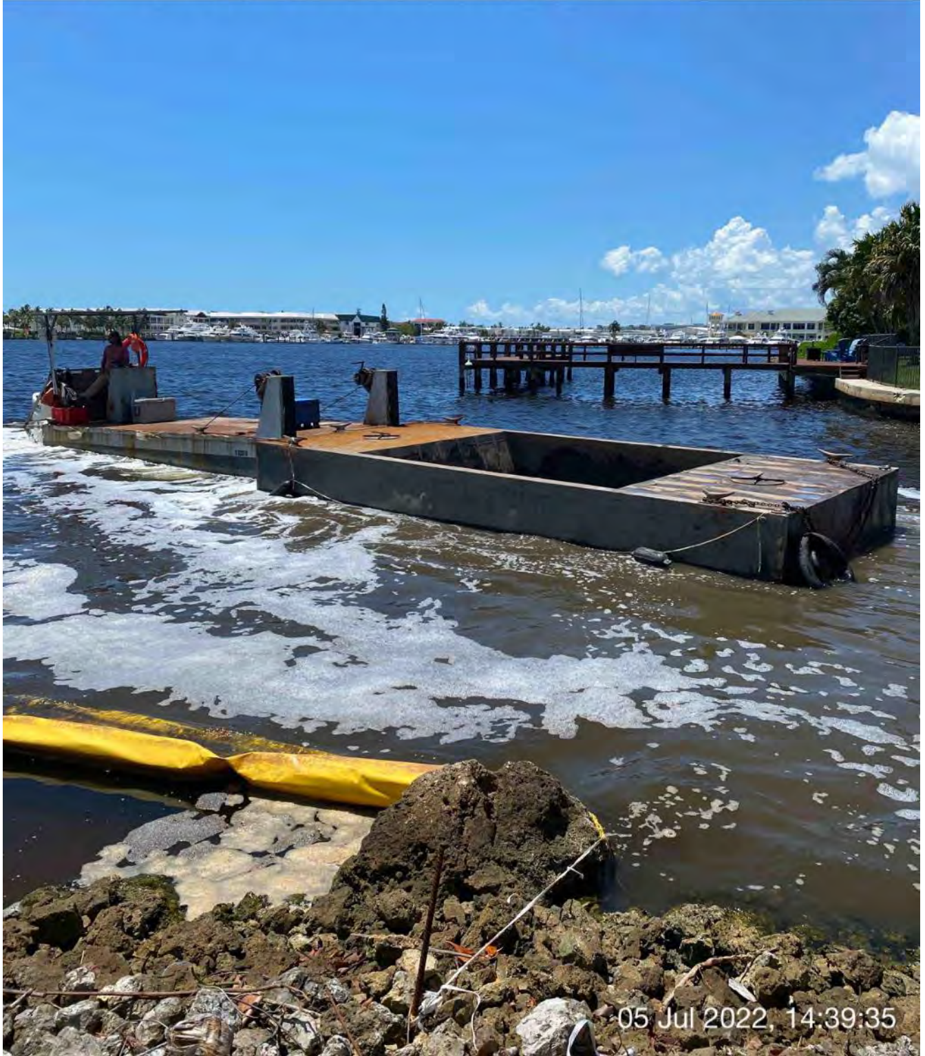
Push boat transporting full hopper of material from Canal X-X to Canal CC-CC
