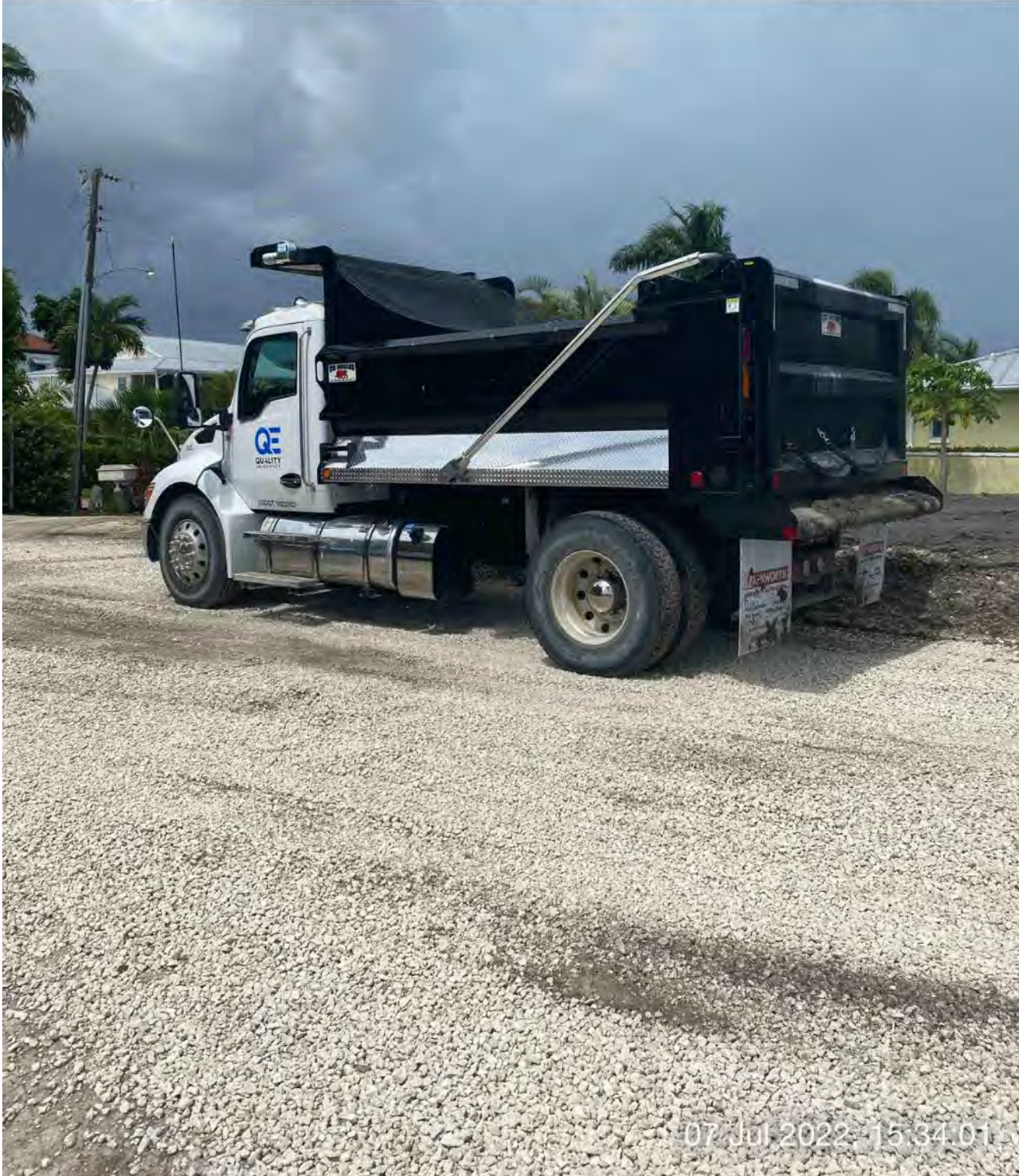
Dump truck on site at 1300 Curlew Avenue
