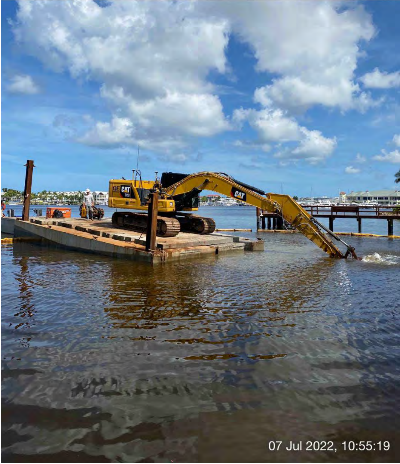
323 excavator removing material from station 1+00
