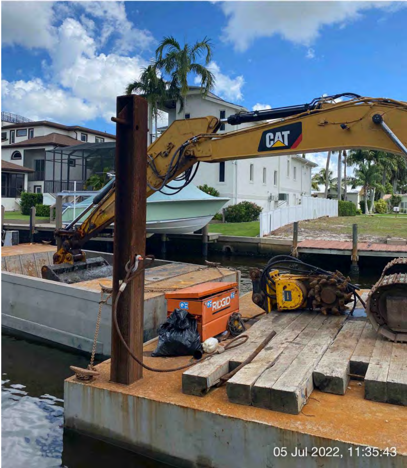
323 excavator removing material and transferring it to hopper at station 3+00
