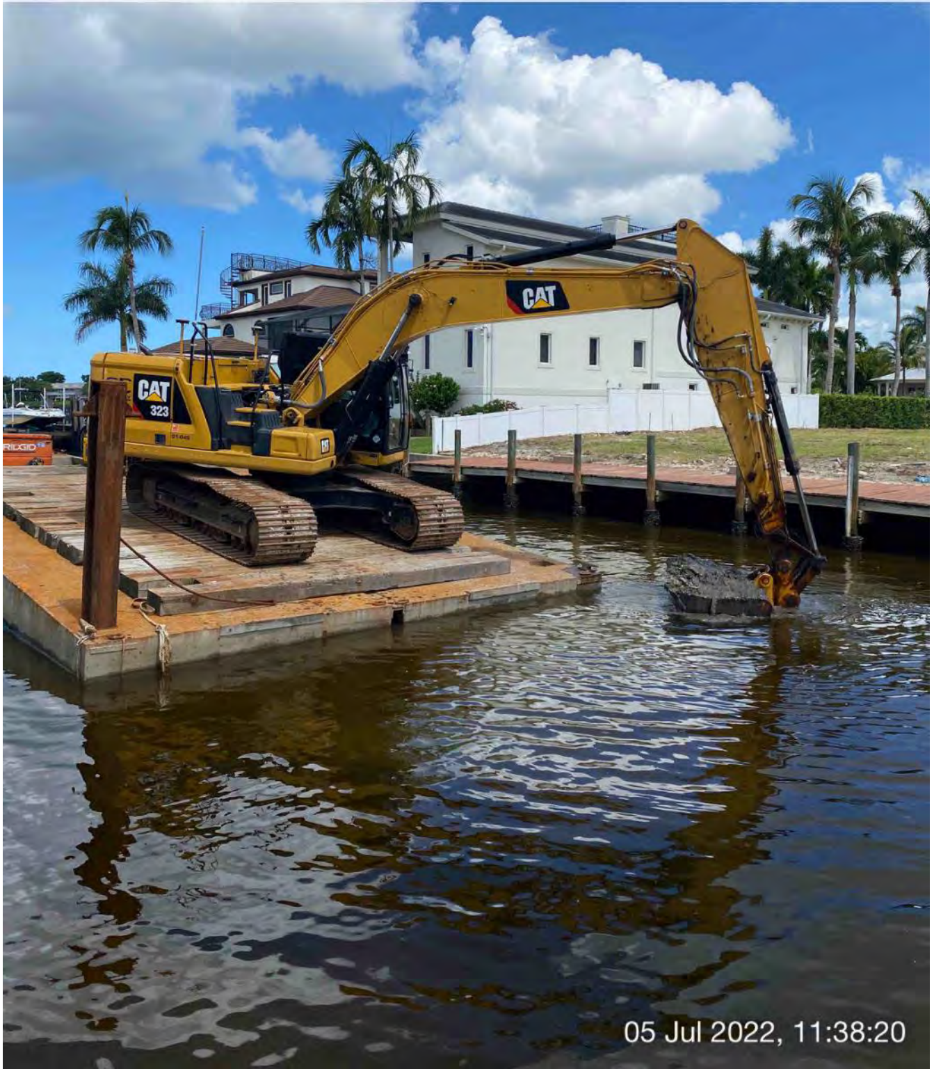
323 excavator removing material from station 3+00
