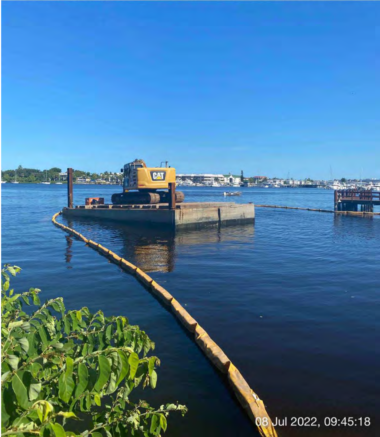
323 excavator grinding rock at station 0+00
