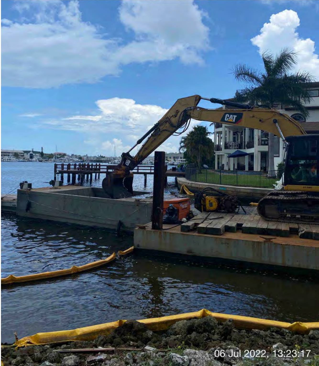
323 excavator removing material and transferring it to hopper at station 1+50
