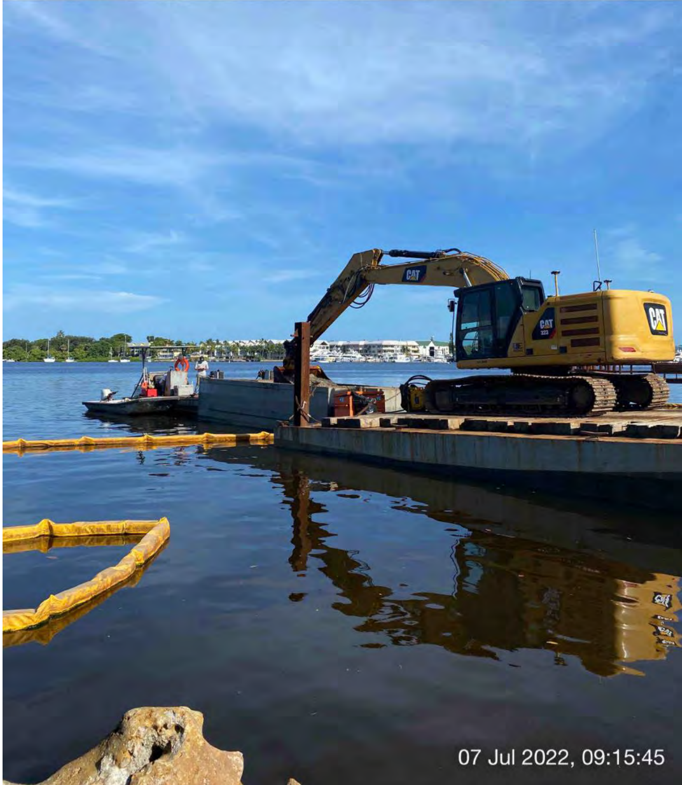
323 excavator transferring removed material to hopper at station 1+00
