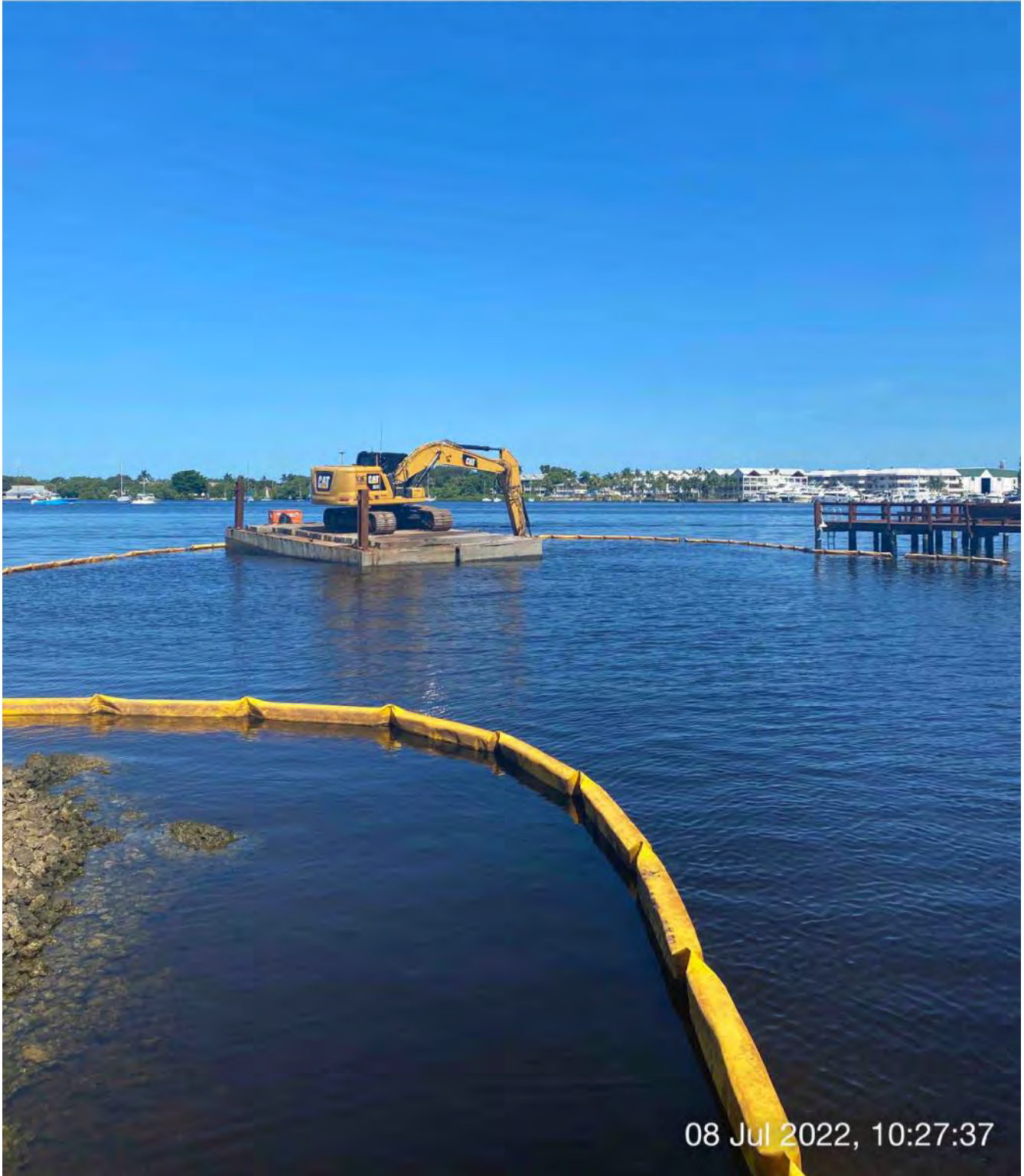
323 excavator grinding rock at station 0+25
