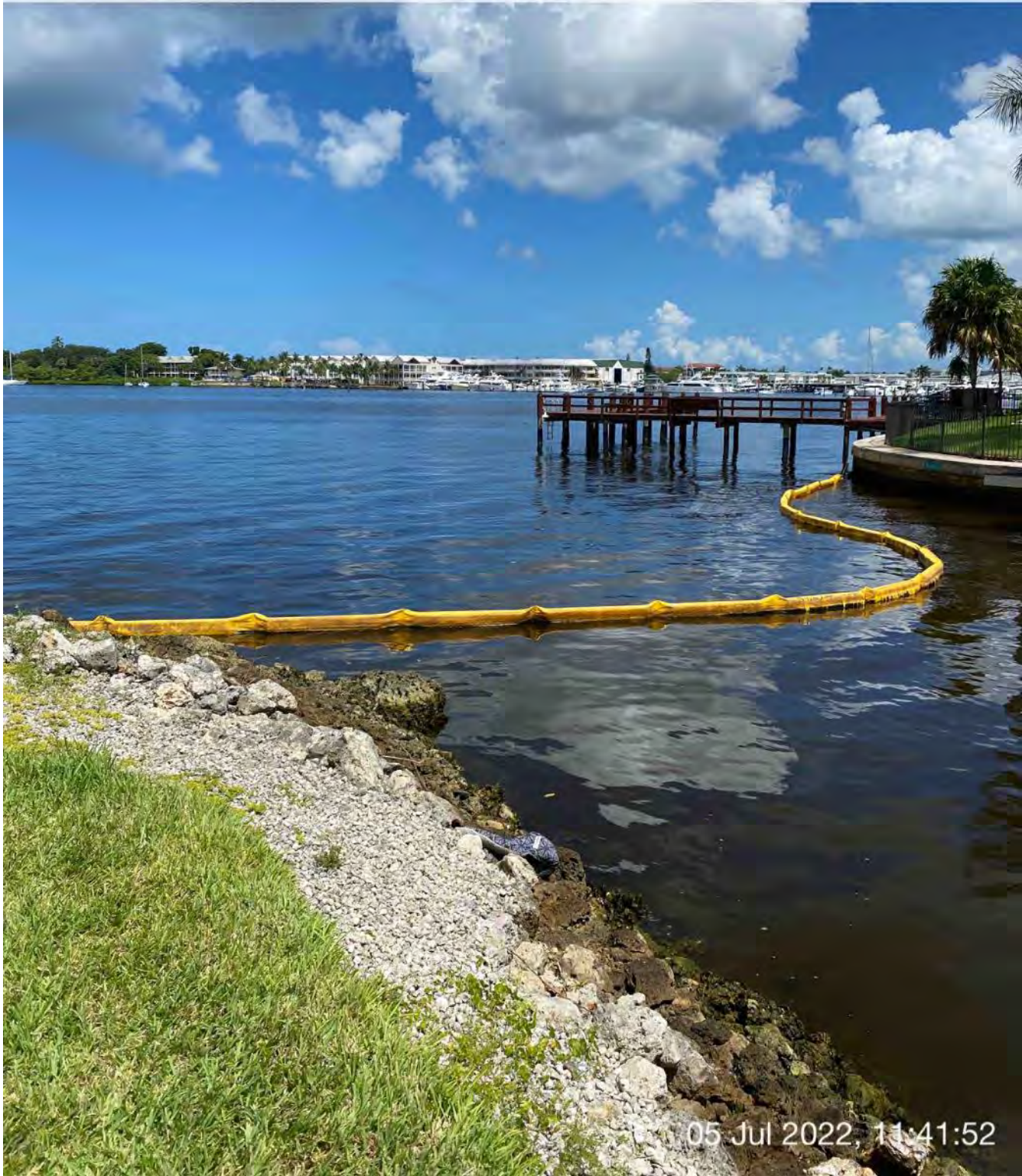
Turbidity curtain installed across the mouth of Canal X-X
