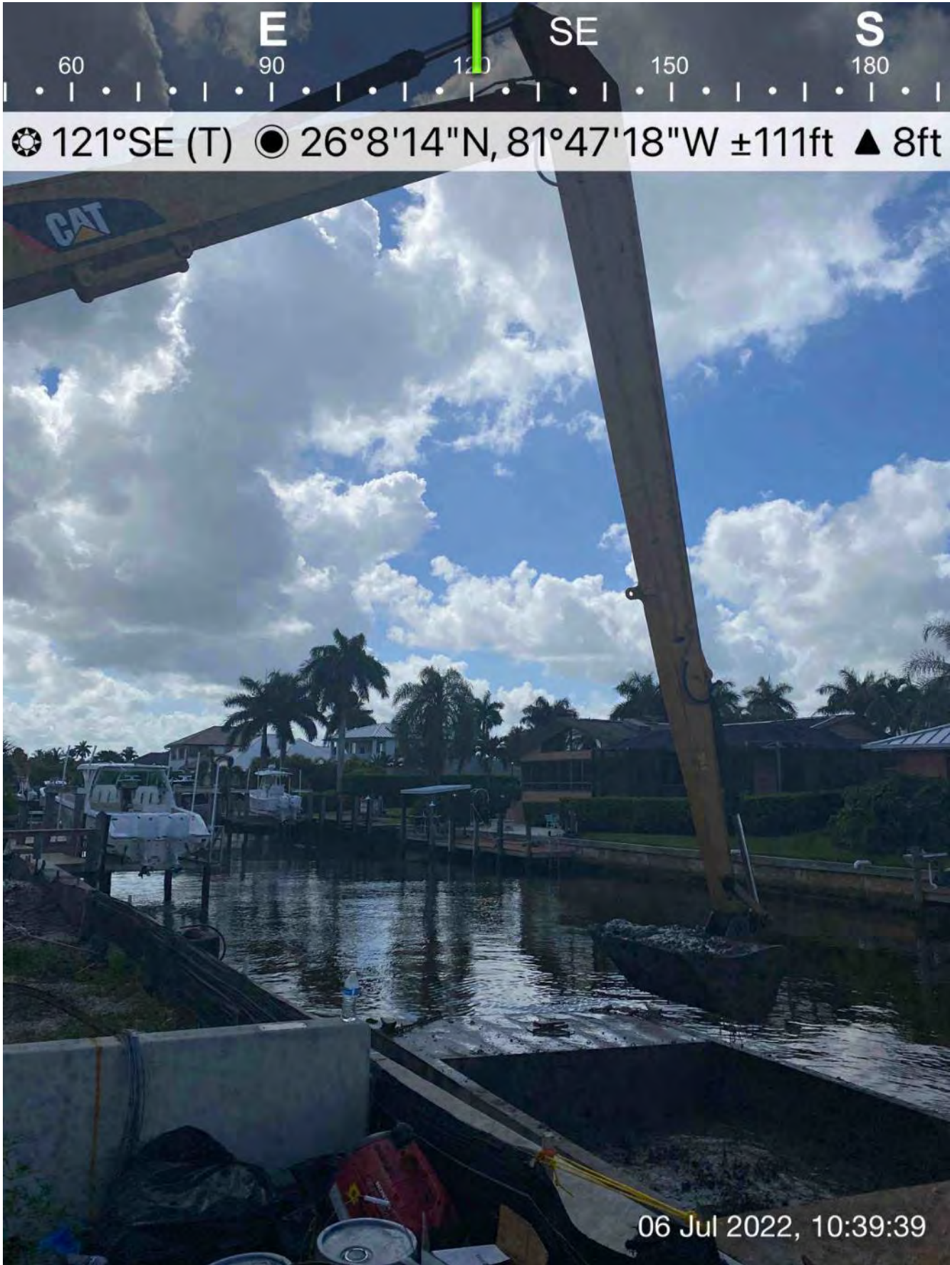
326 excavator transferring removed material from hopper to dewatering site at 1300 Curlew Avenue
