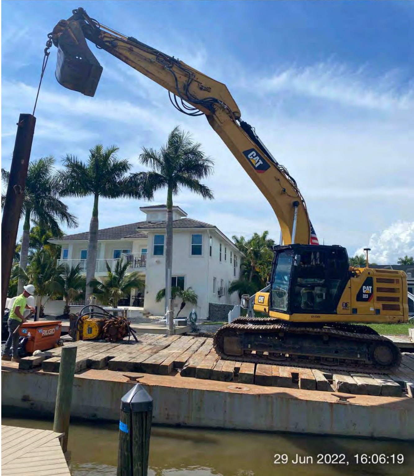
326 excavator lifting spud to allow push boat to mobilize barge at station 5+00 in Canal X-X
