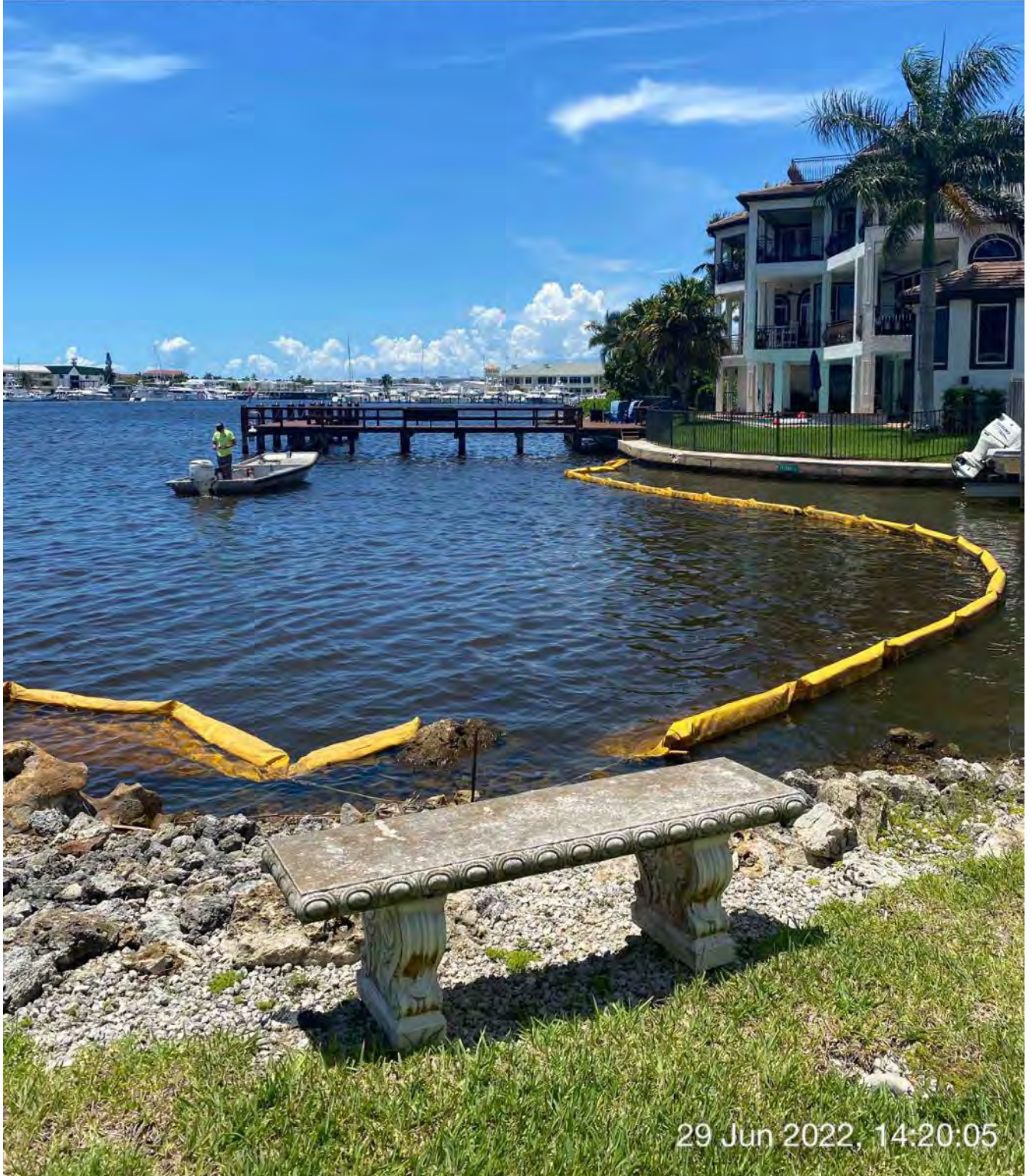
Contractor using support boat to test turbidity levels in the mouth of Canal X-X
