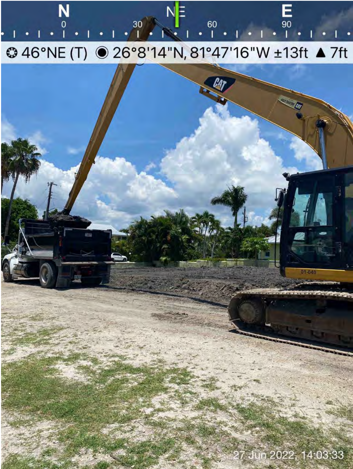
326 excavator transferring removed material from dewatering site to dump truck bed at 1300 Curlew Avenue
