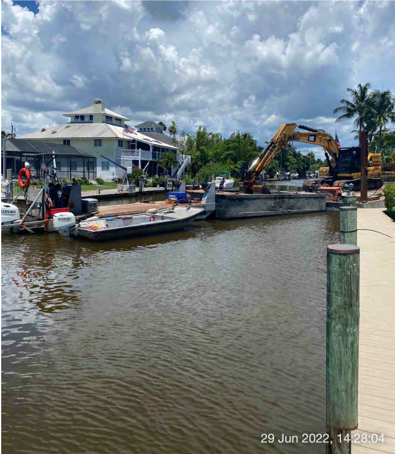
Hopper, barge, and 323 excavator staged in Canal X-X between stations 4+00 and 5+00
