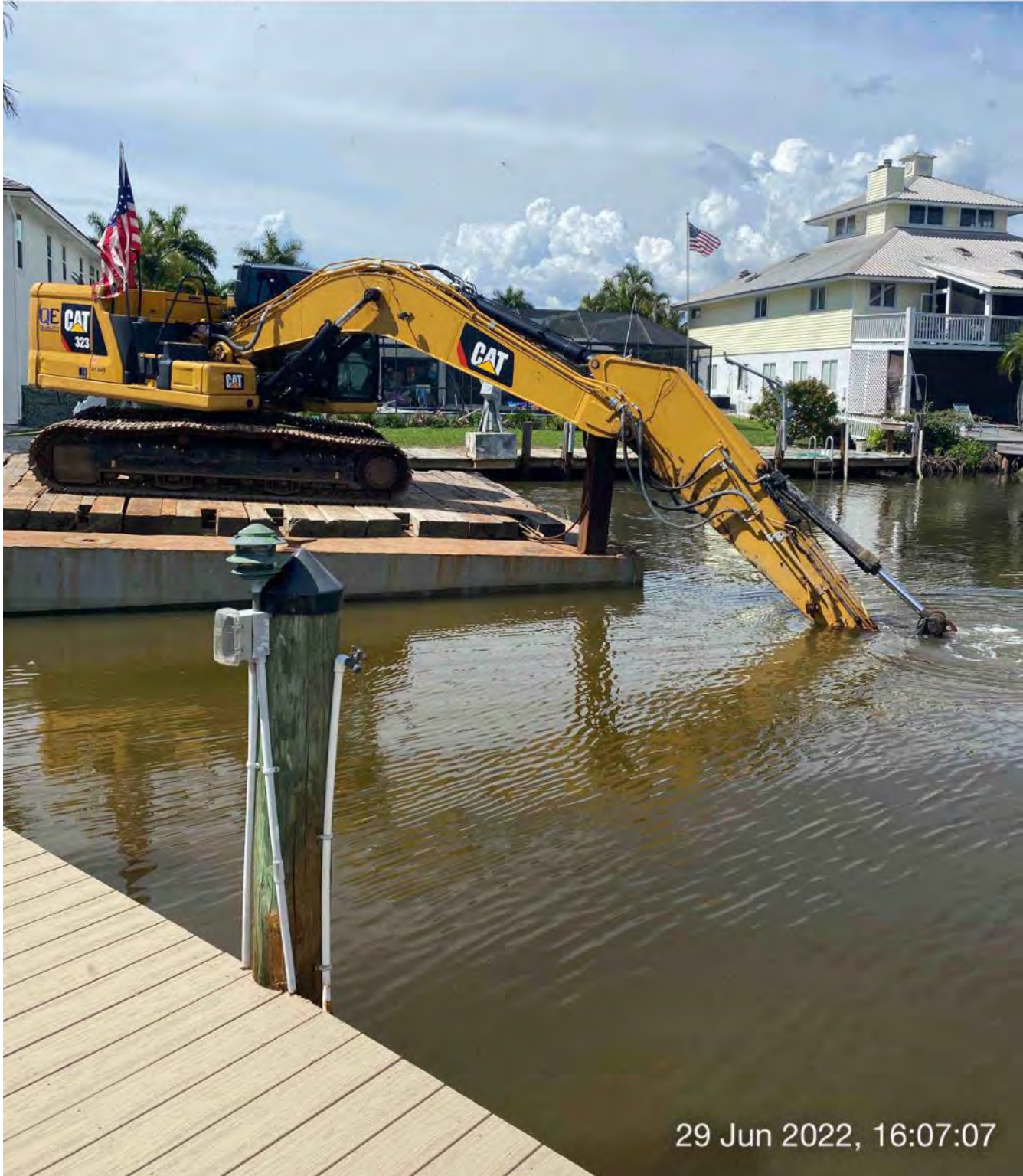
323 excavator removing material from station 0+50
