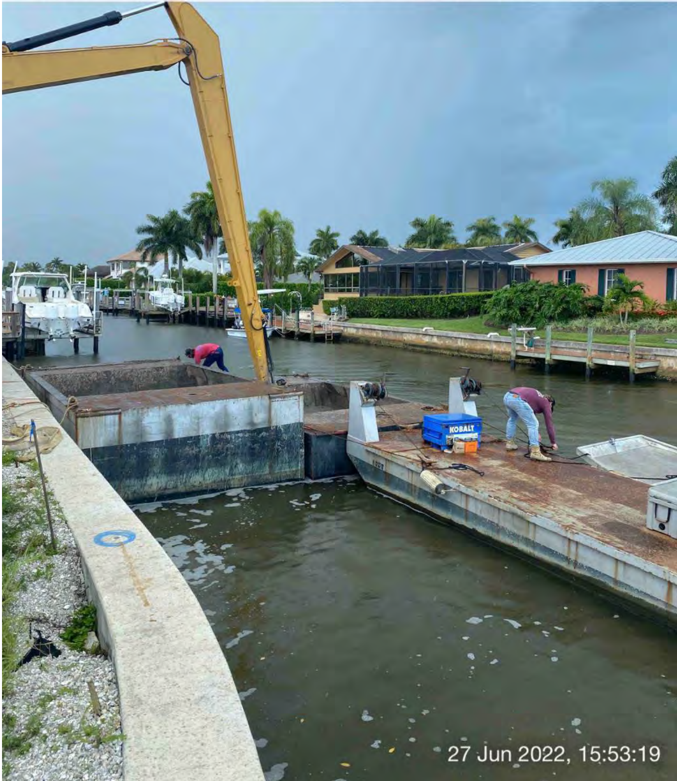
Push boat dropping off full hopper of material in Canal CC-CC station 1+50
