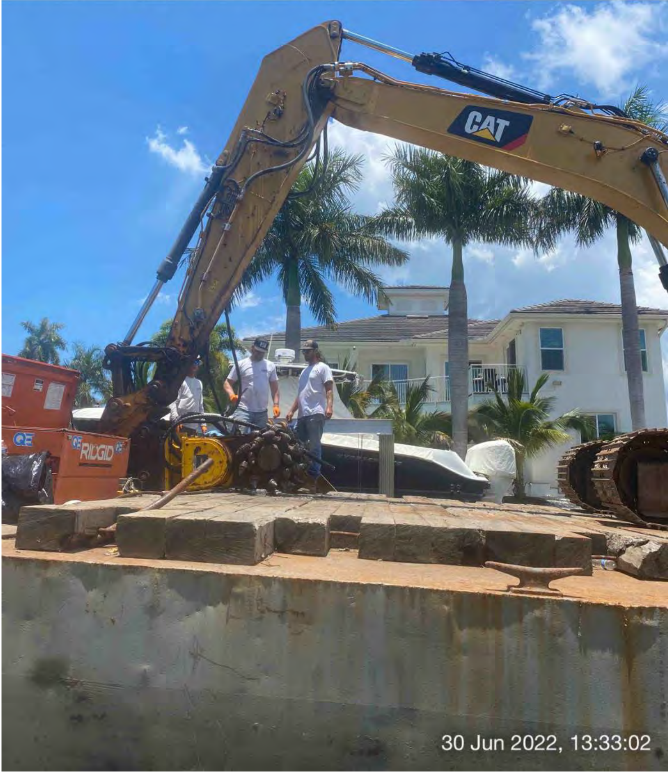
Contractor switching from Epiroc grinder to bucket attachment on 323 excavator
