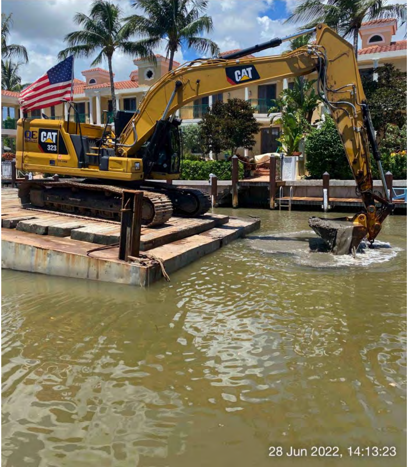
323 excavator removing material from station 2+00
