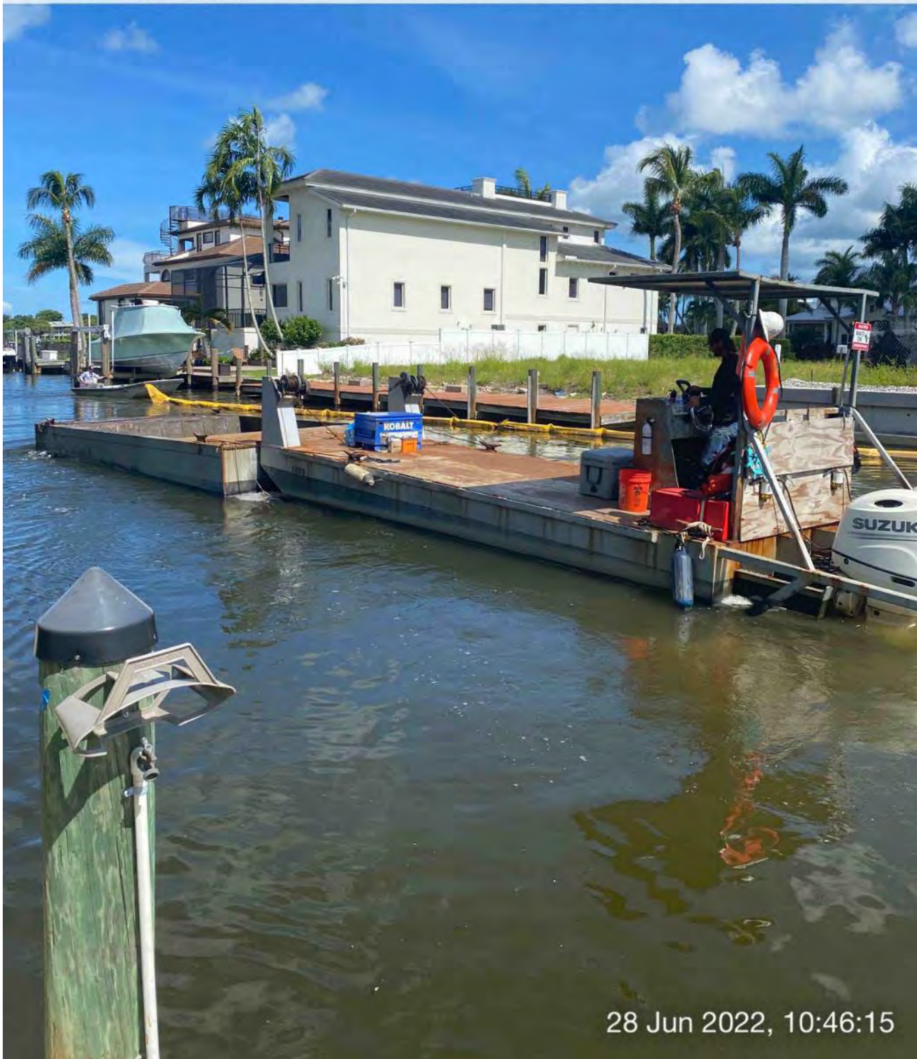
Support boat opening turbidity curtain to allow push boat to transport full hopper of material to Canal CC-CC
