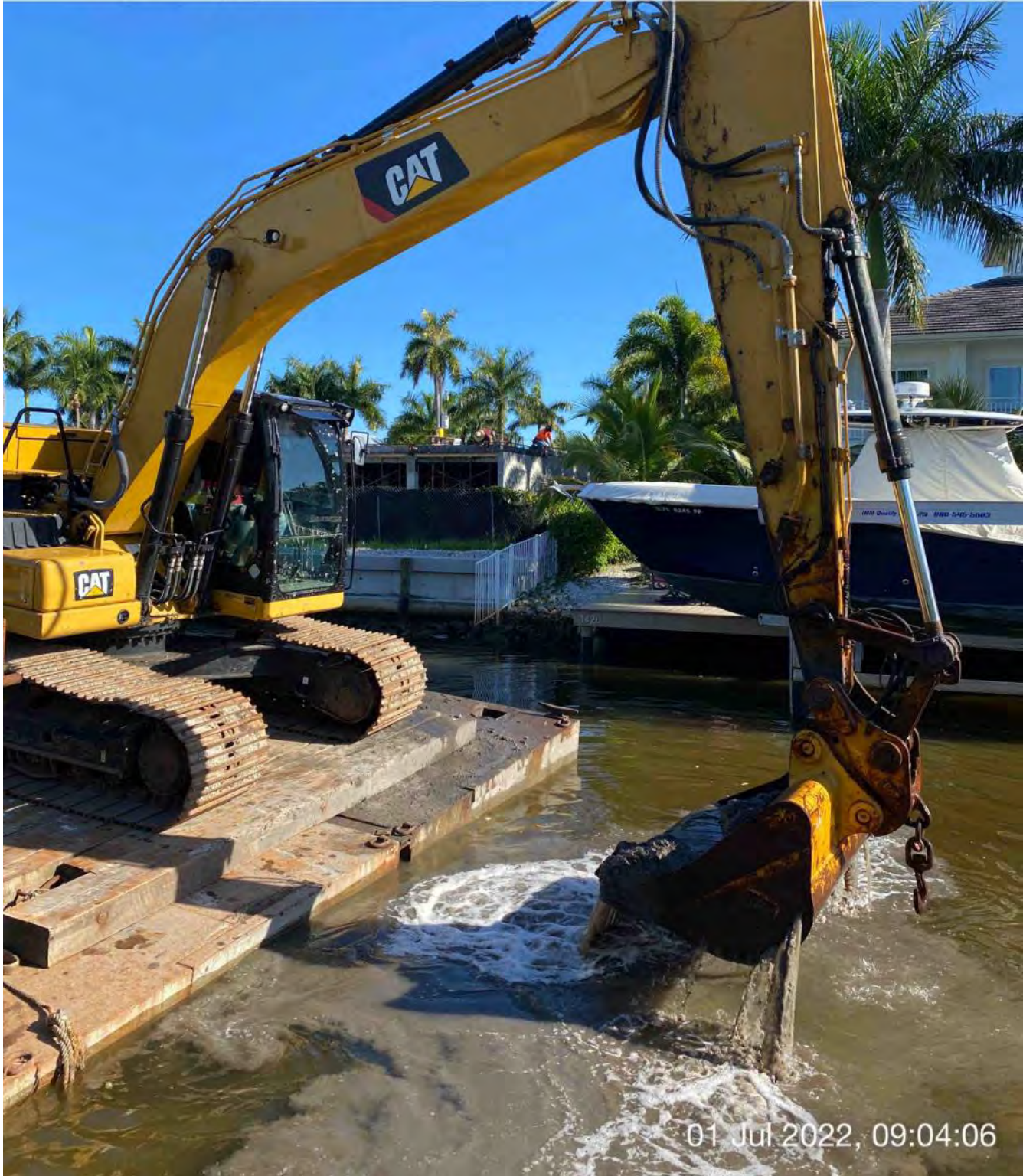
323 excavator removing material from station 4+00
