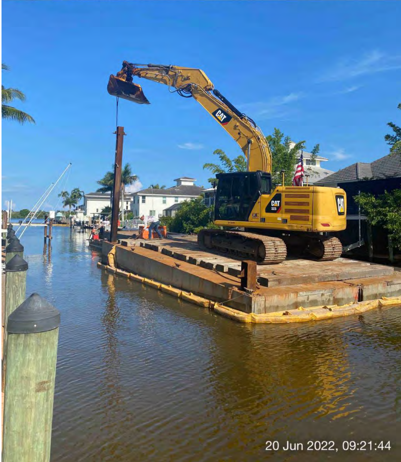
323 excavator lifting spud to allow push boat to mobilize barge at station 7+00
