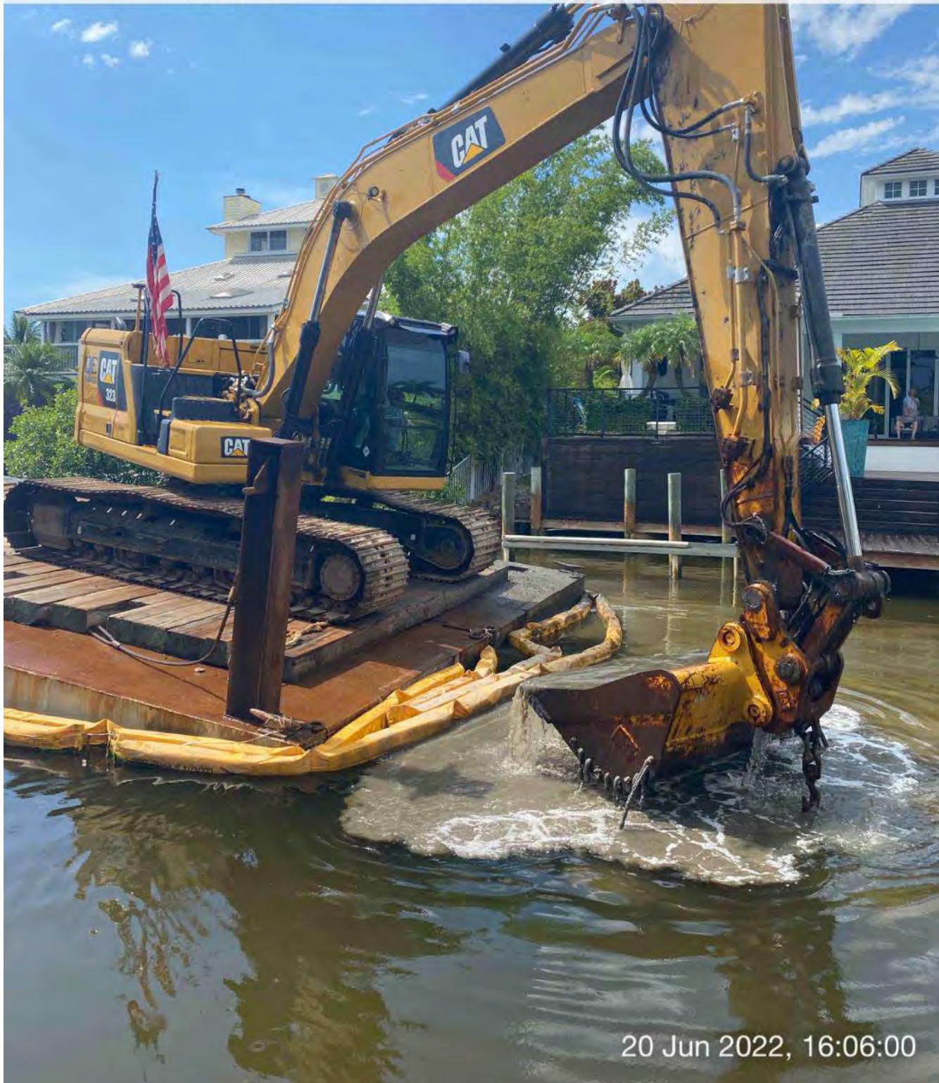
323 excavator removing material from station 6+50
