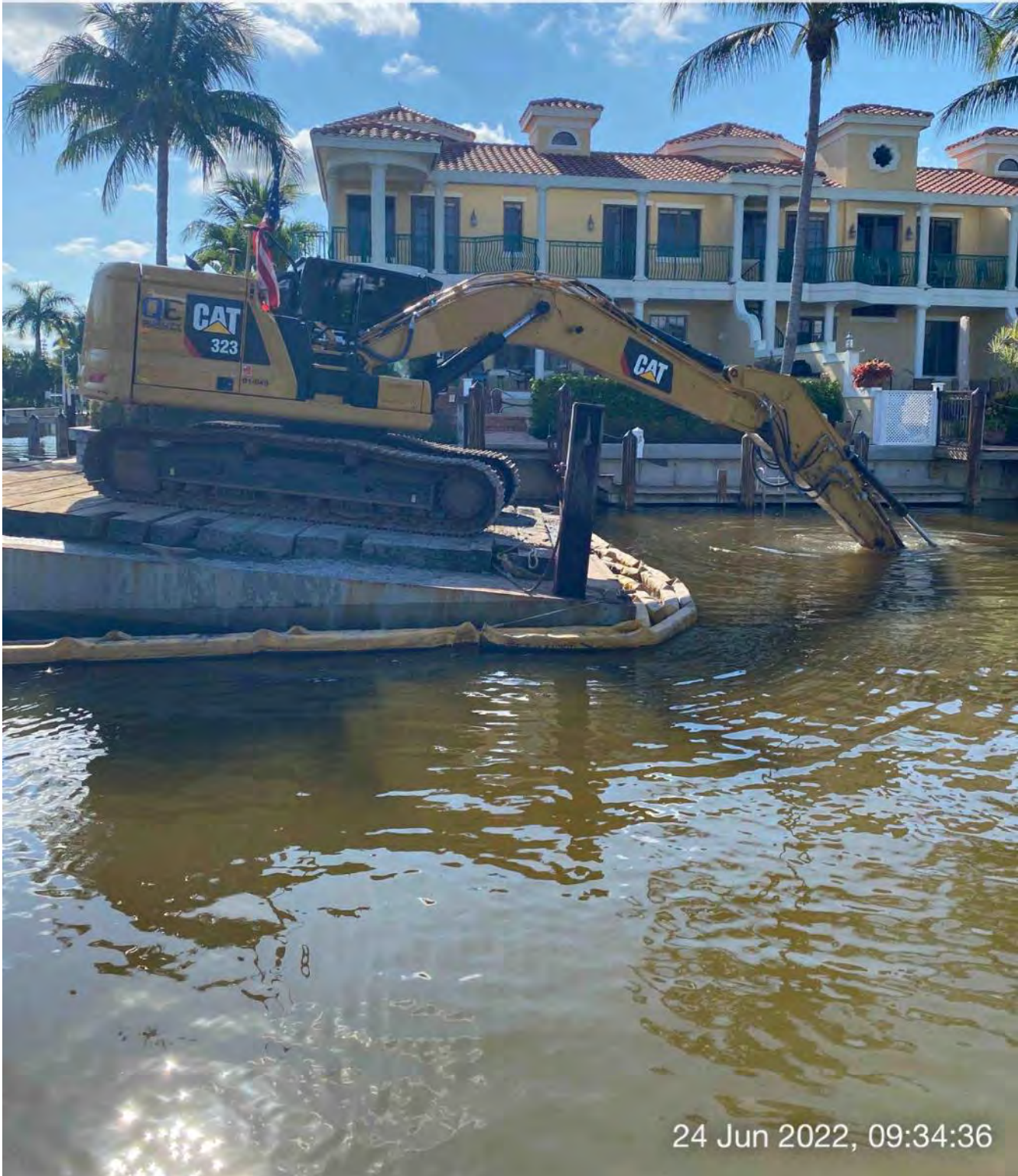
323 excavator grinding rock at station 1+50 in Canal Y-Y
