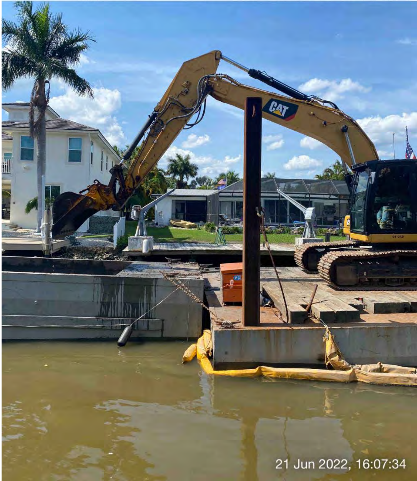
323 excavator transferring removed material to hopper
