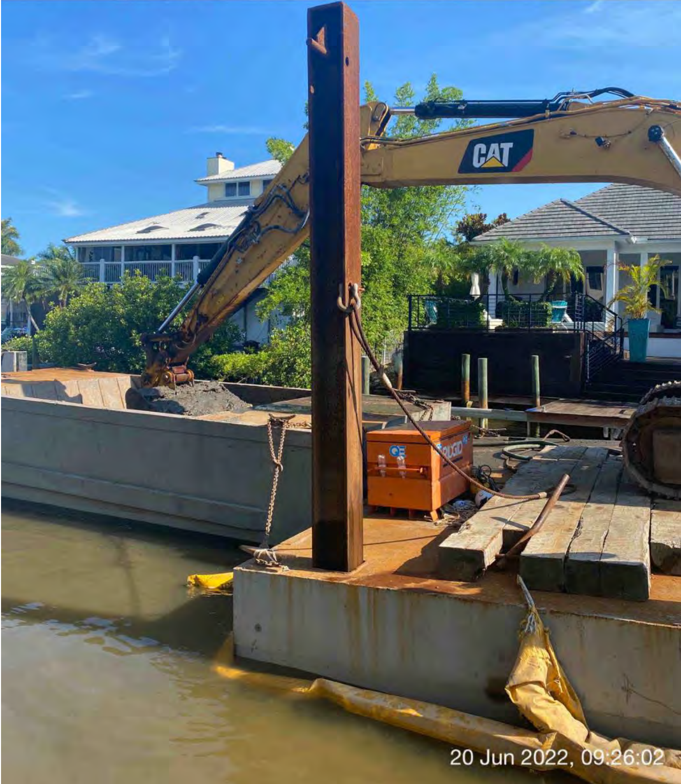
323 excavator transferring removed material to hopper at station 7+00
