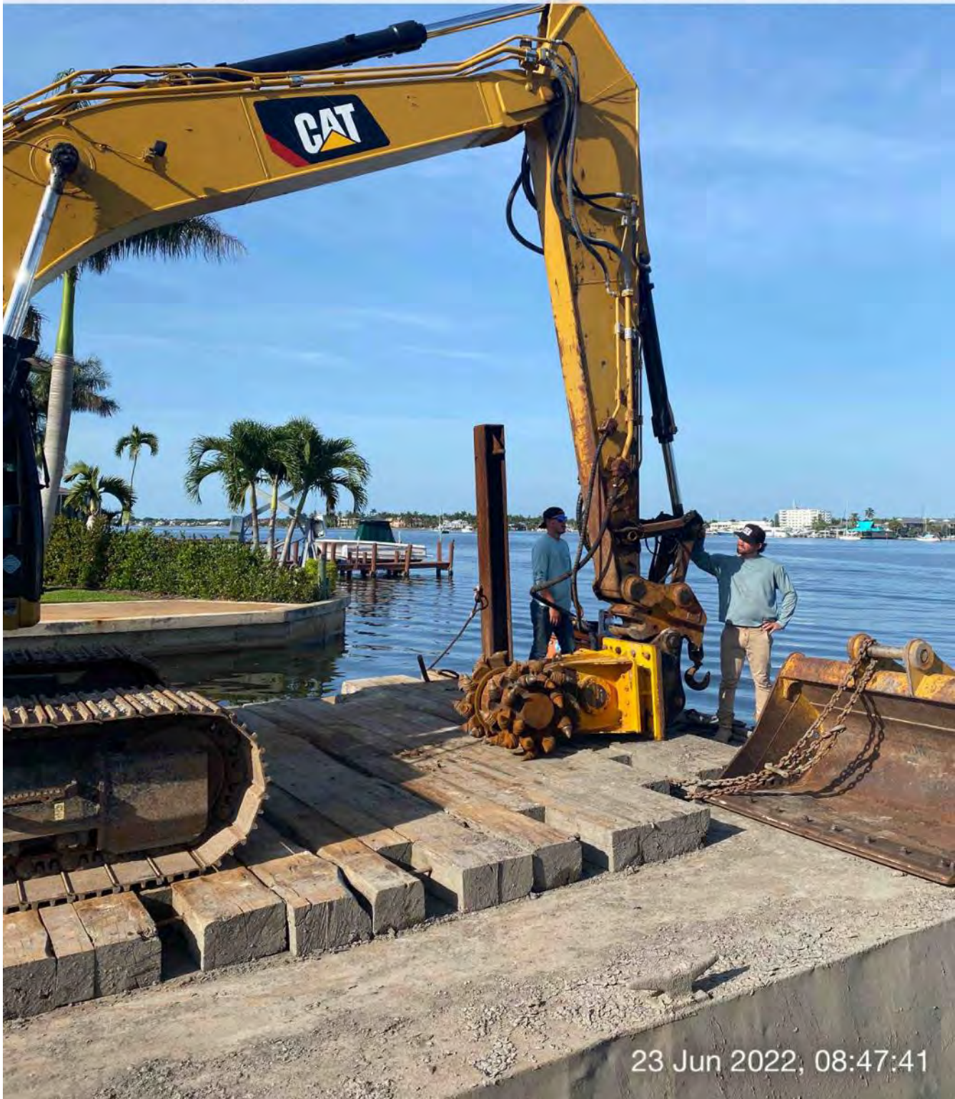
323 excavator on barge with Epiroc grinder in Canal CC-CC at station 1+00
