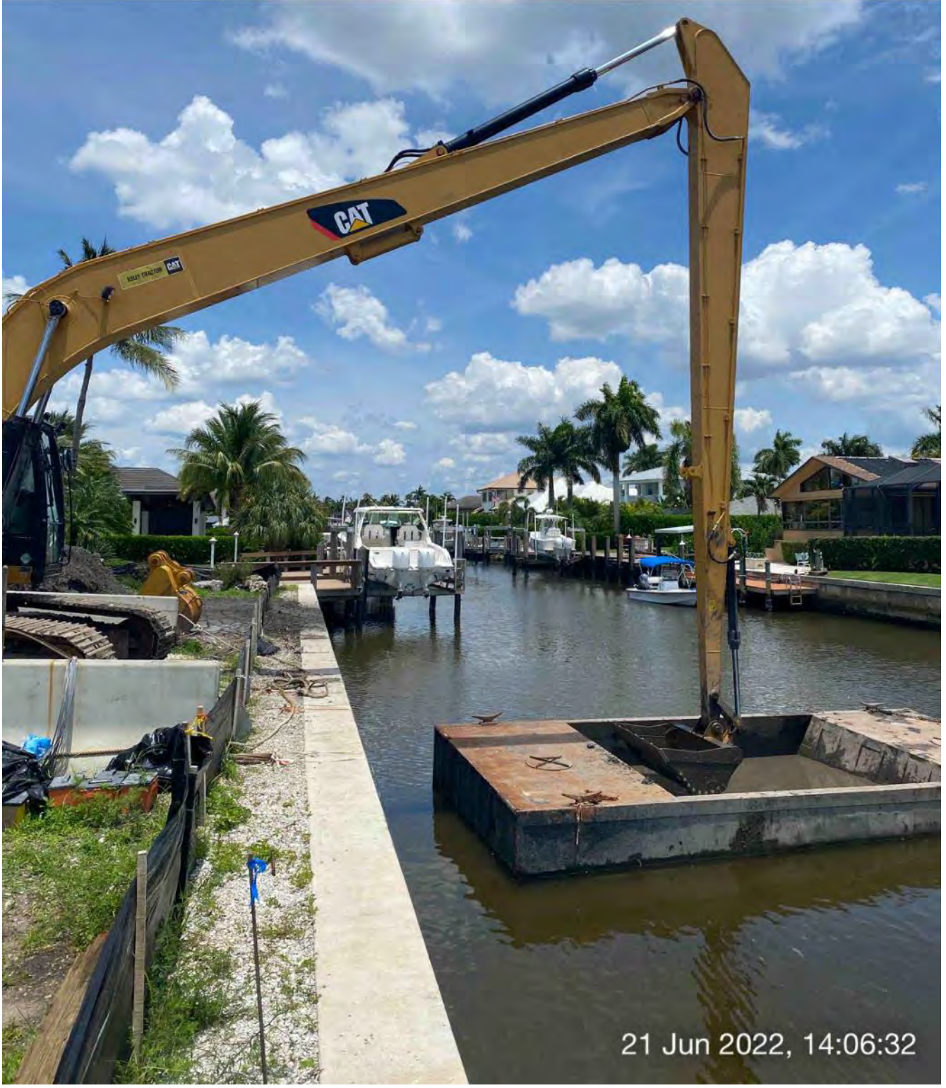
326 excavator removing material from hopper
