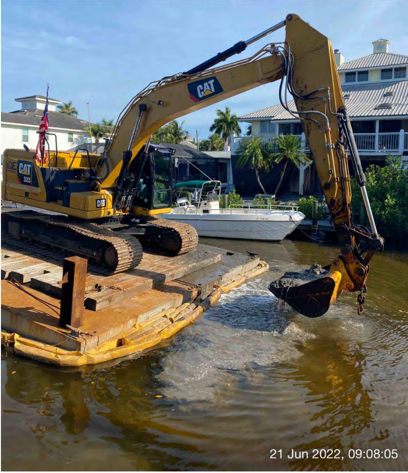
323 excavator removing material from station 6+75
