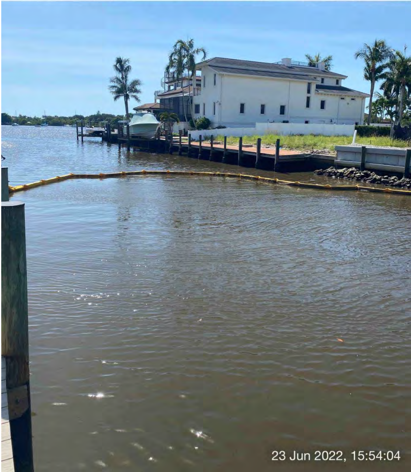
Turbidity curtain installed across the mouth of Canal X-X at station 3+75
