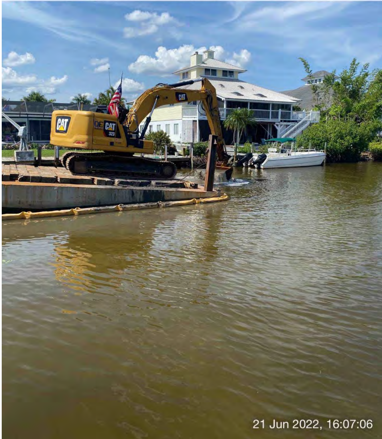
323 excavator removing material from station 5+50
