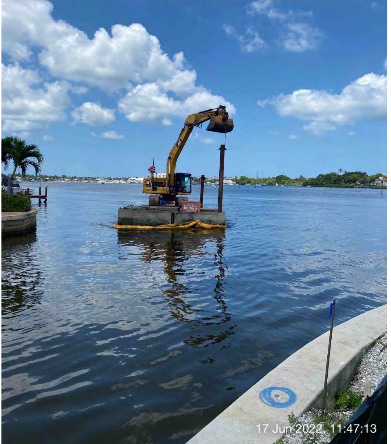
Push boat transporting barge and 323 excavator back to Canal CC-CC
