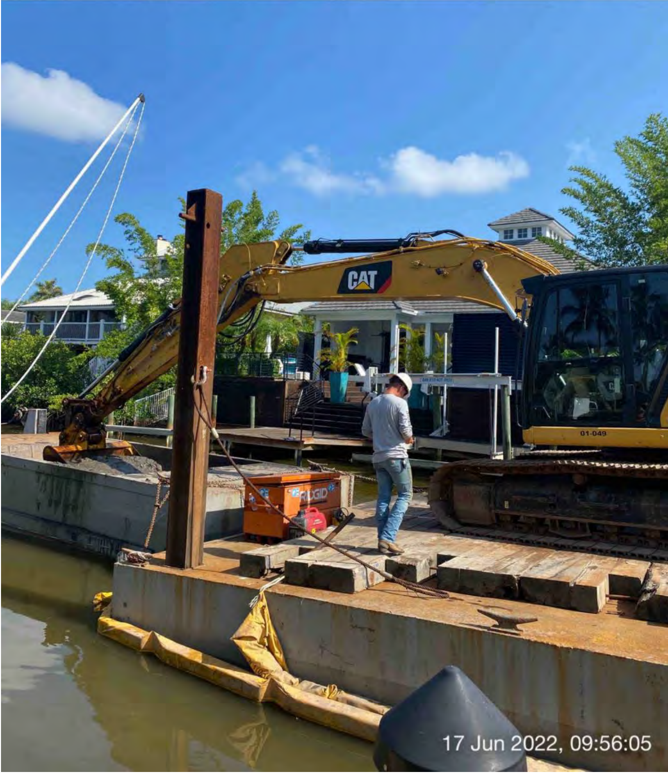
323 excavator removing material from station 7+50 and transferring it to hopper
