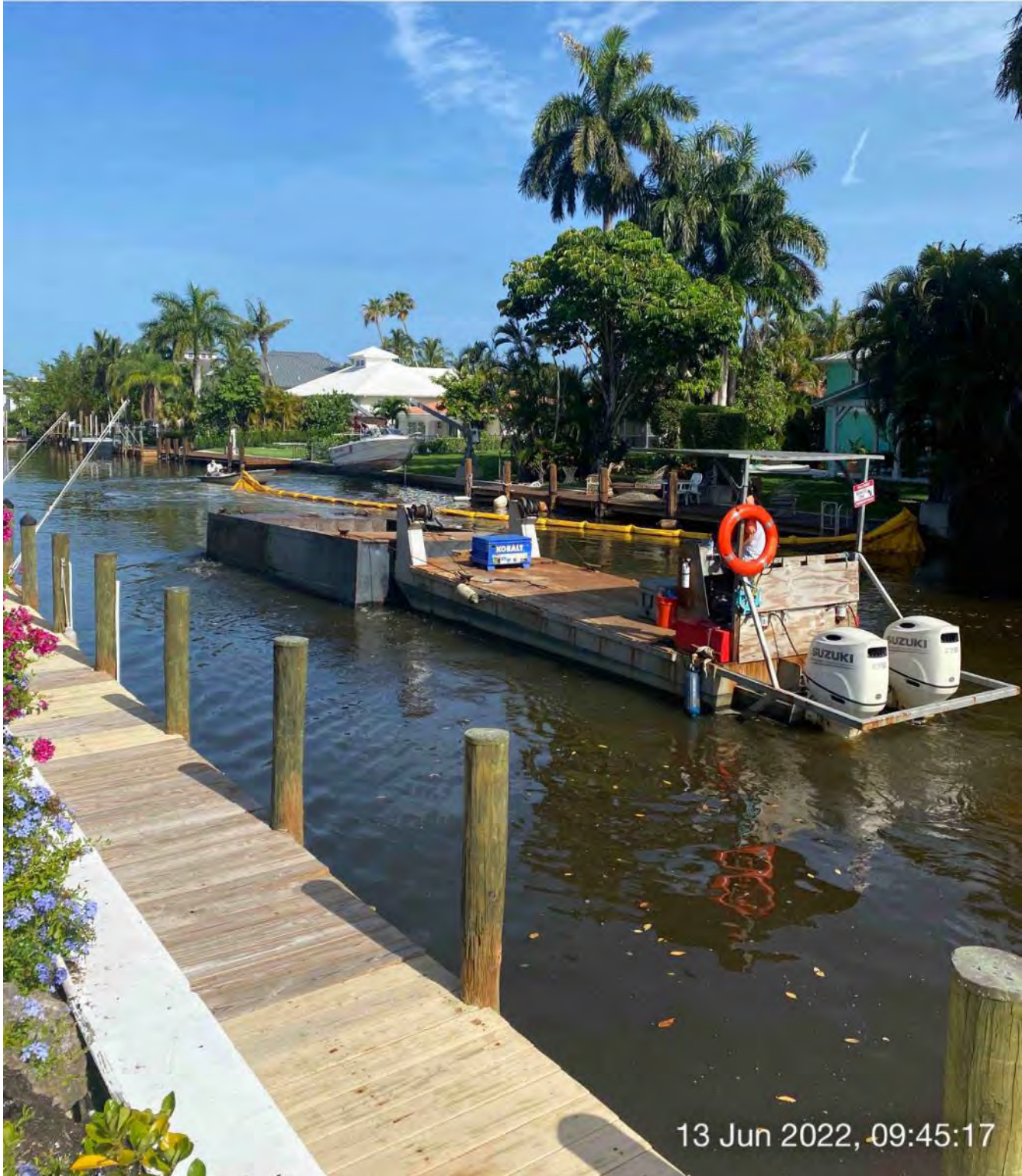
Support boat being used to open turbidity curtain to allow push boat to transport full hopper back to Canal CC-CC
