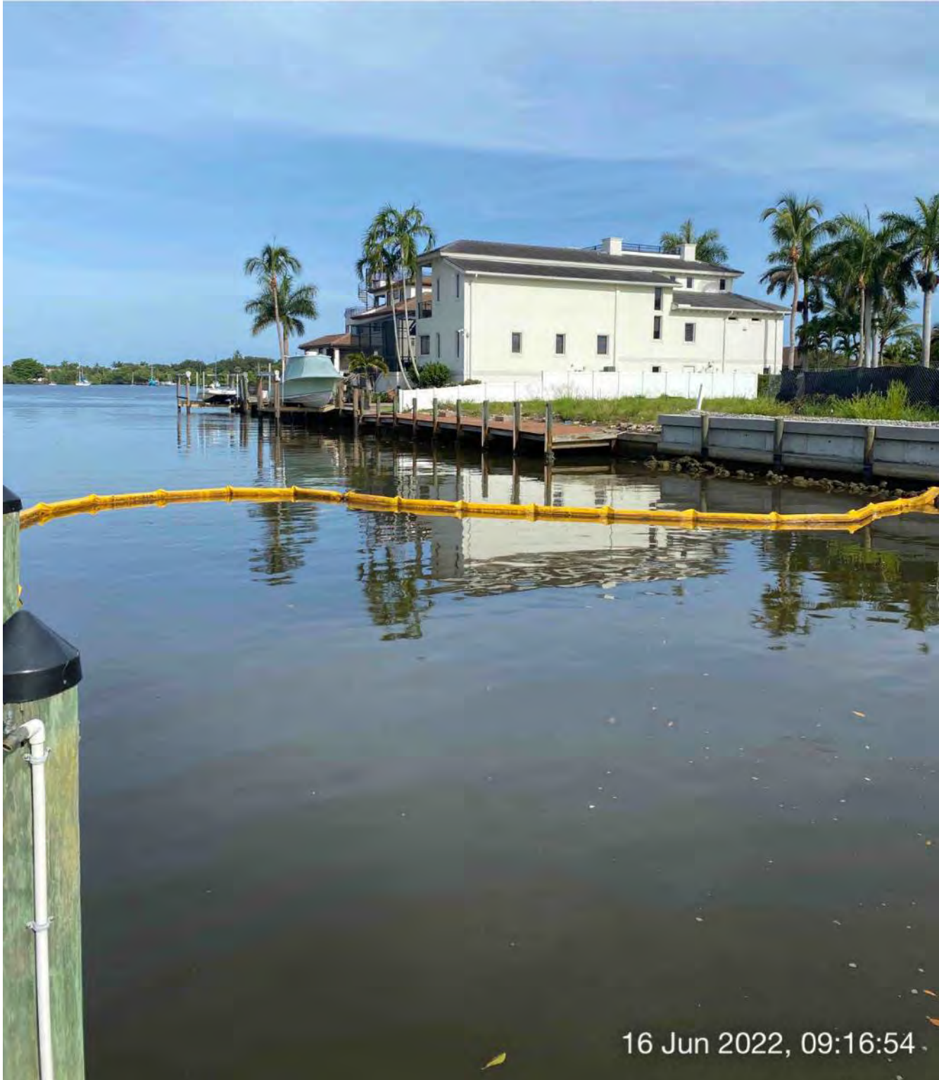
Turbidity curtain installed across Canal X-X at station 3+50
