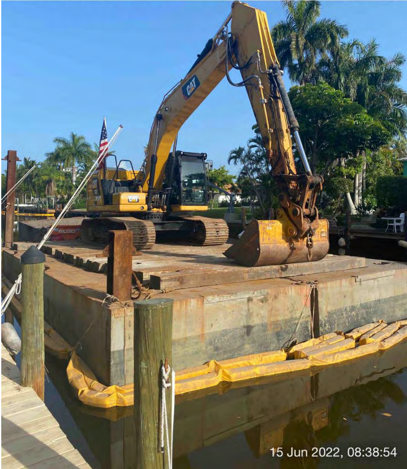
323 excavator on barge at station 10+50
