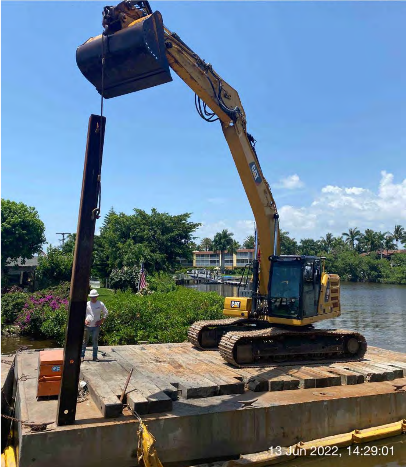
323 excavator lifting spud to allow push boat to mobilize barge at station 12+00
