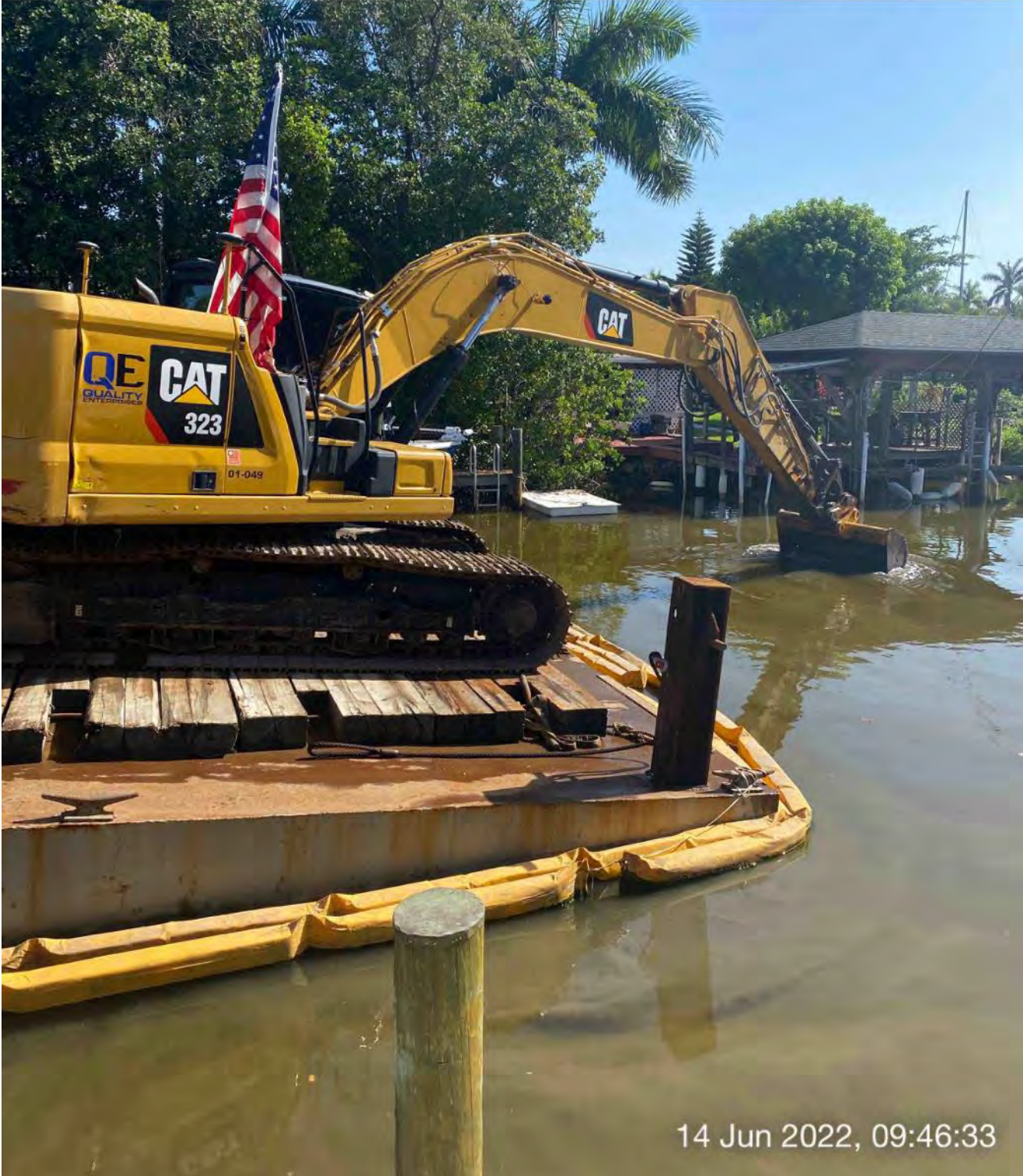
323 excavator removing material from station 11+50
