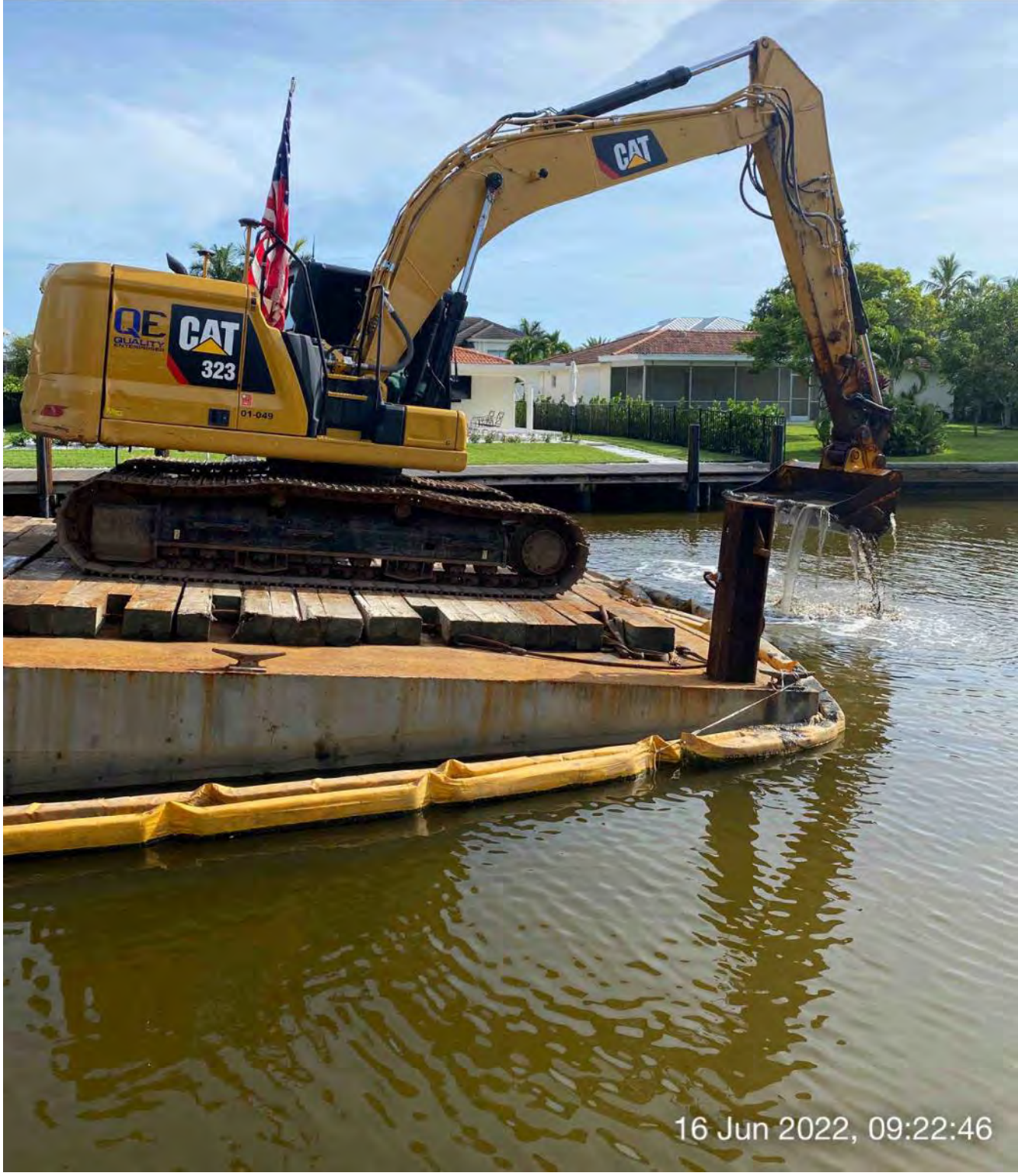
323 excavator removing material from station 9+25
