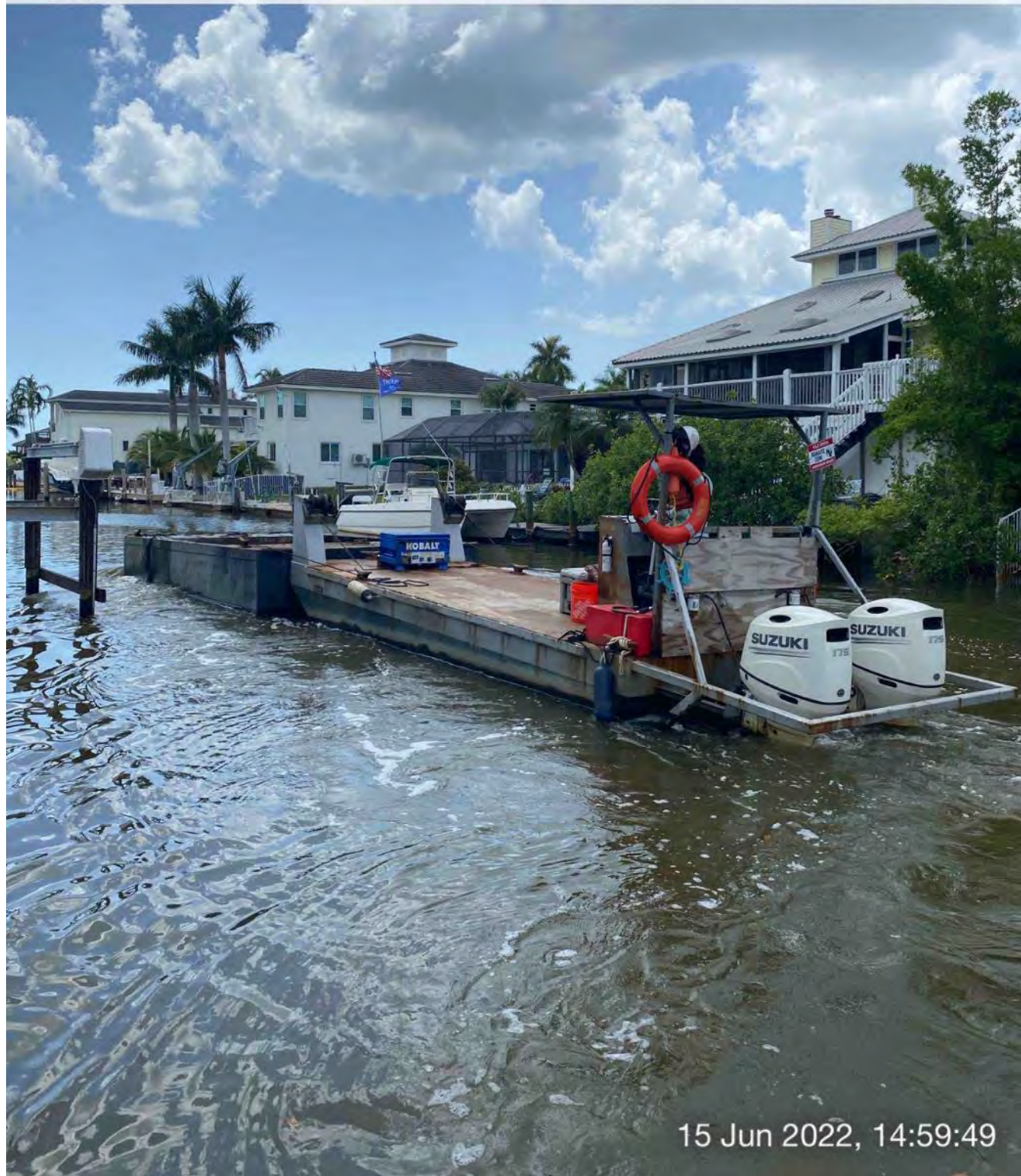
Support boat opening turbidity curtain to allow push boat to transport full hopper from Canal X-X to Canal CC-CC
