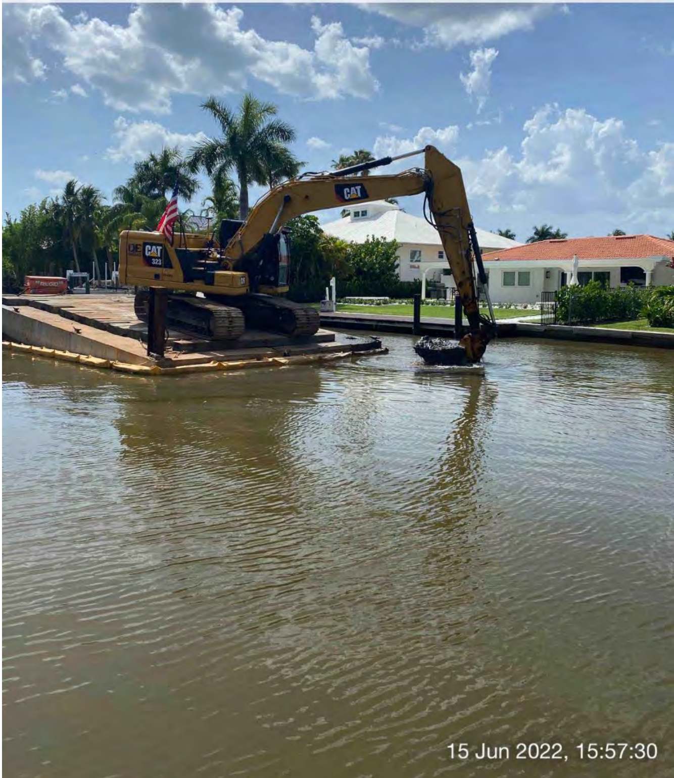
323 excavator removing material from station 9+75
