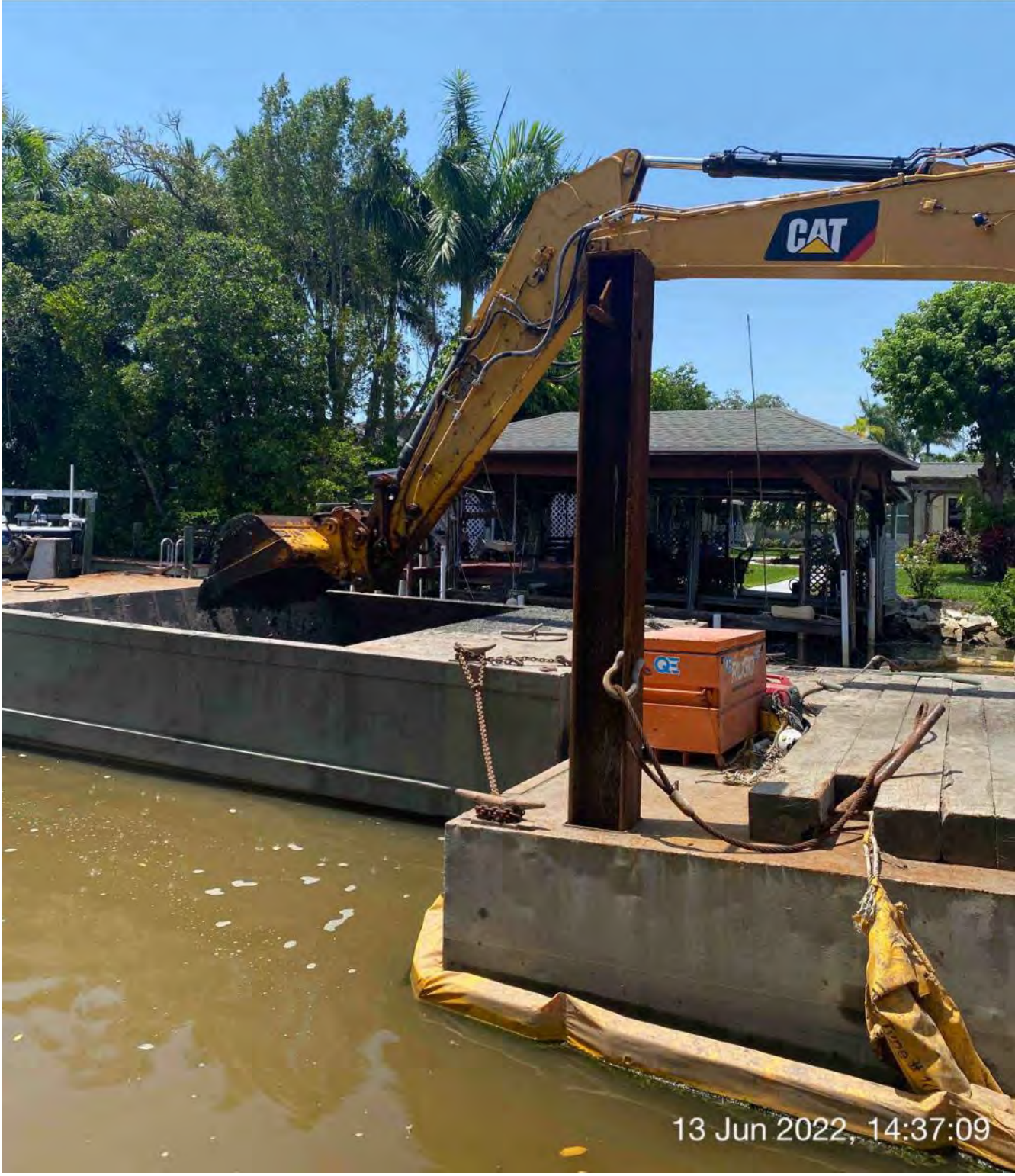
323 excavator transferring removed material to hopper at station 11+75
