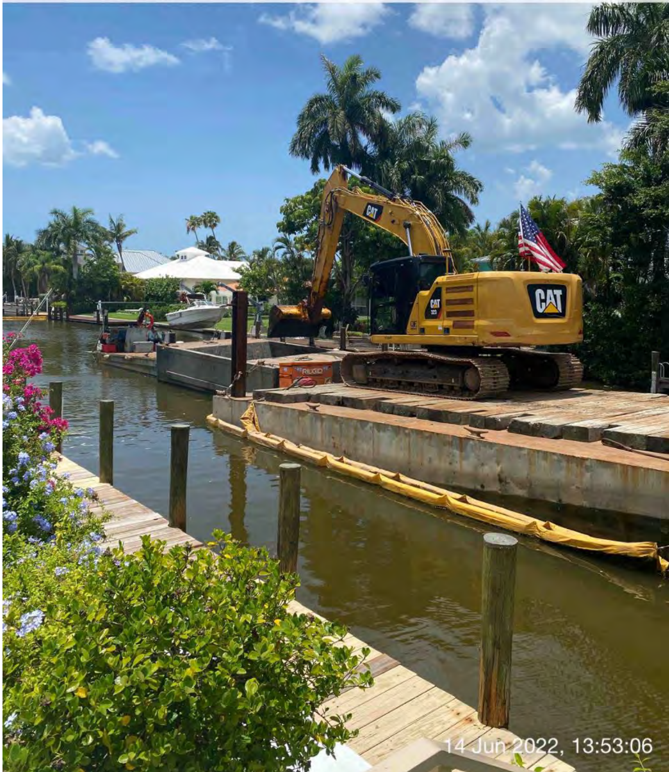
323 excavator transferring removed material to hopper at station 11+00
