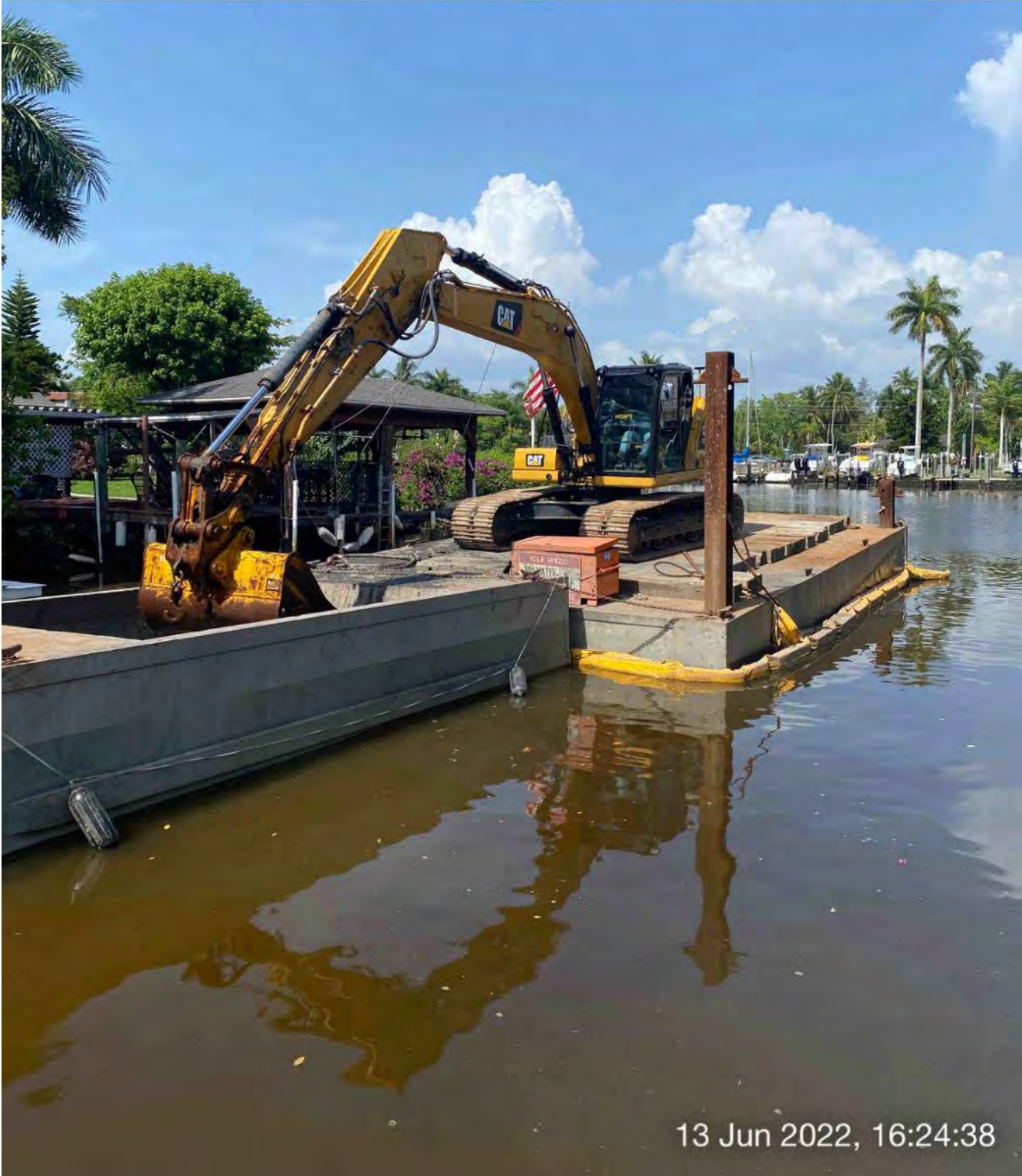
323 excavator transferring removed material to hopper at station 11+50
