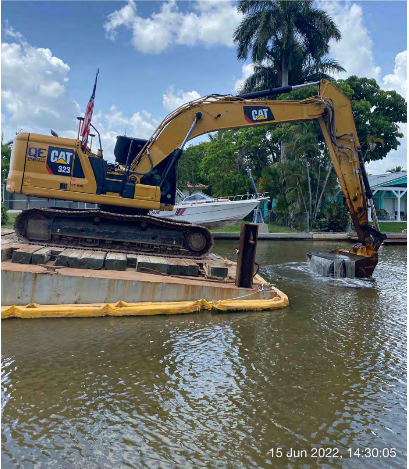
323 excavator removing material from station 10+00
