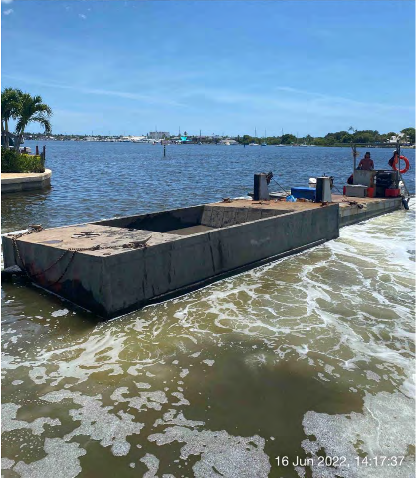
Push boat dropping off a full hopper of removed material in Canal CC-CC
