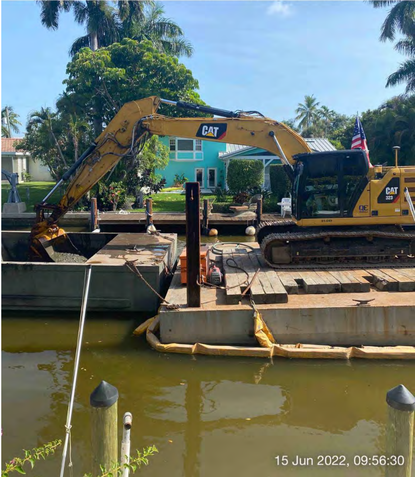
323 excavator removing material from station 10+75 and transferring to hopper
