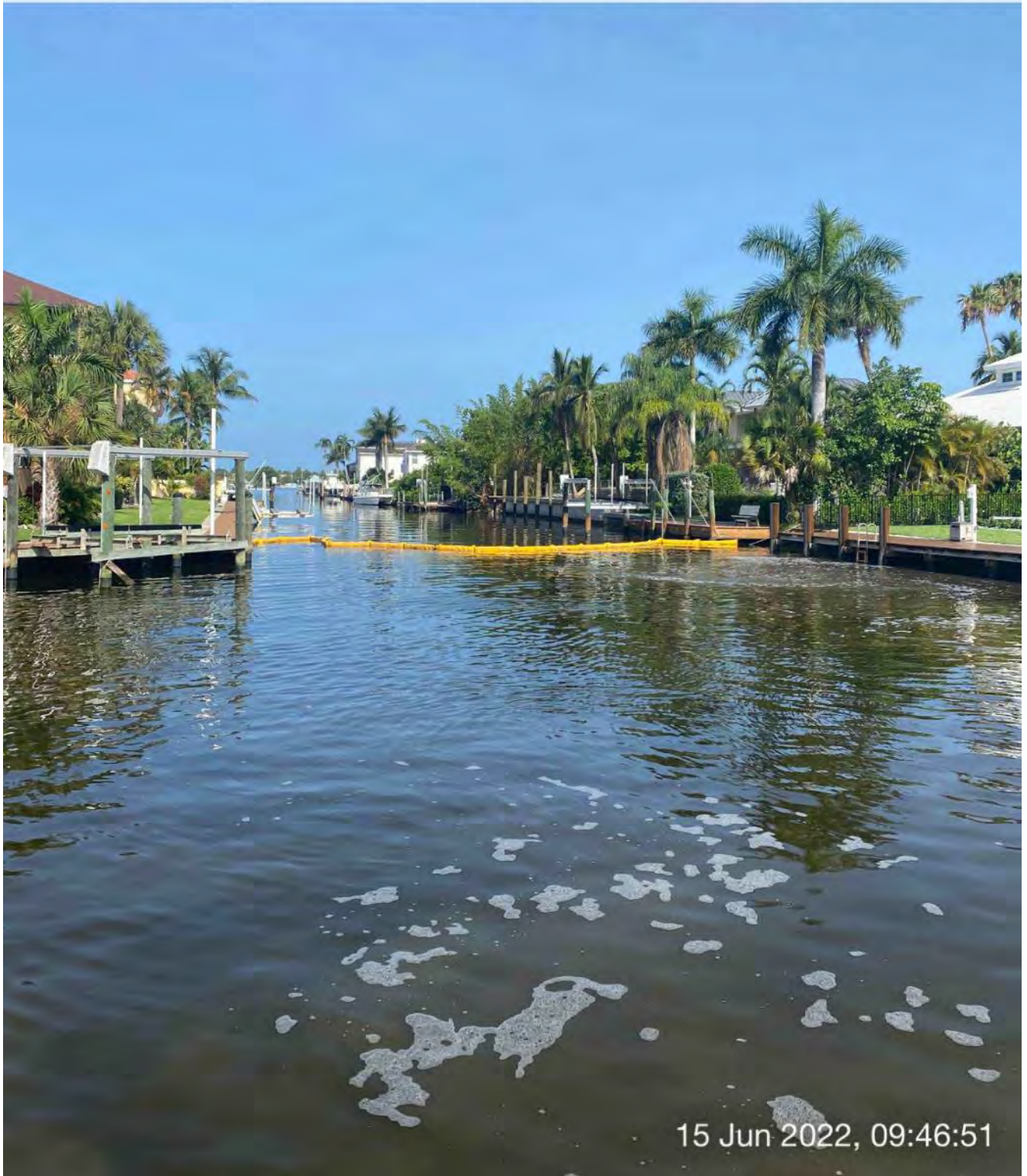
Turbidity curtain installed across Canal X-X at station 8+75
