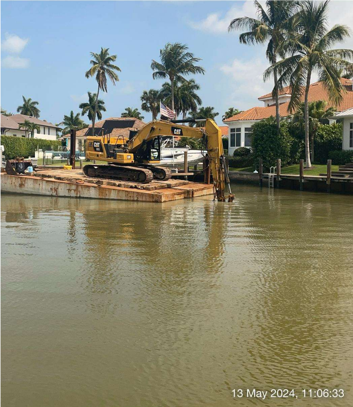
323 excavator grinding rock at station 13+70 in Canal A-A.
