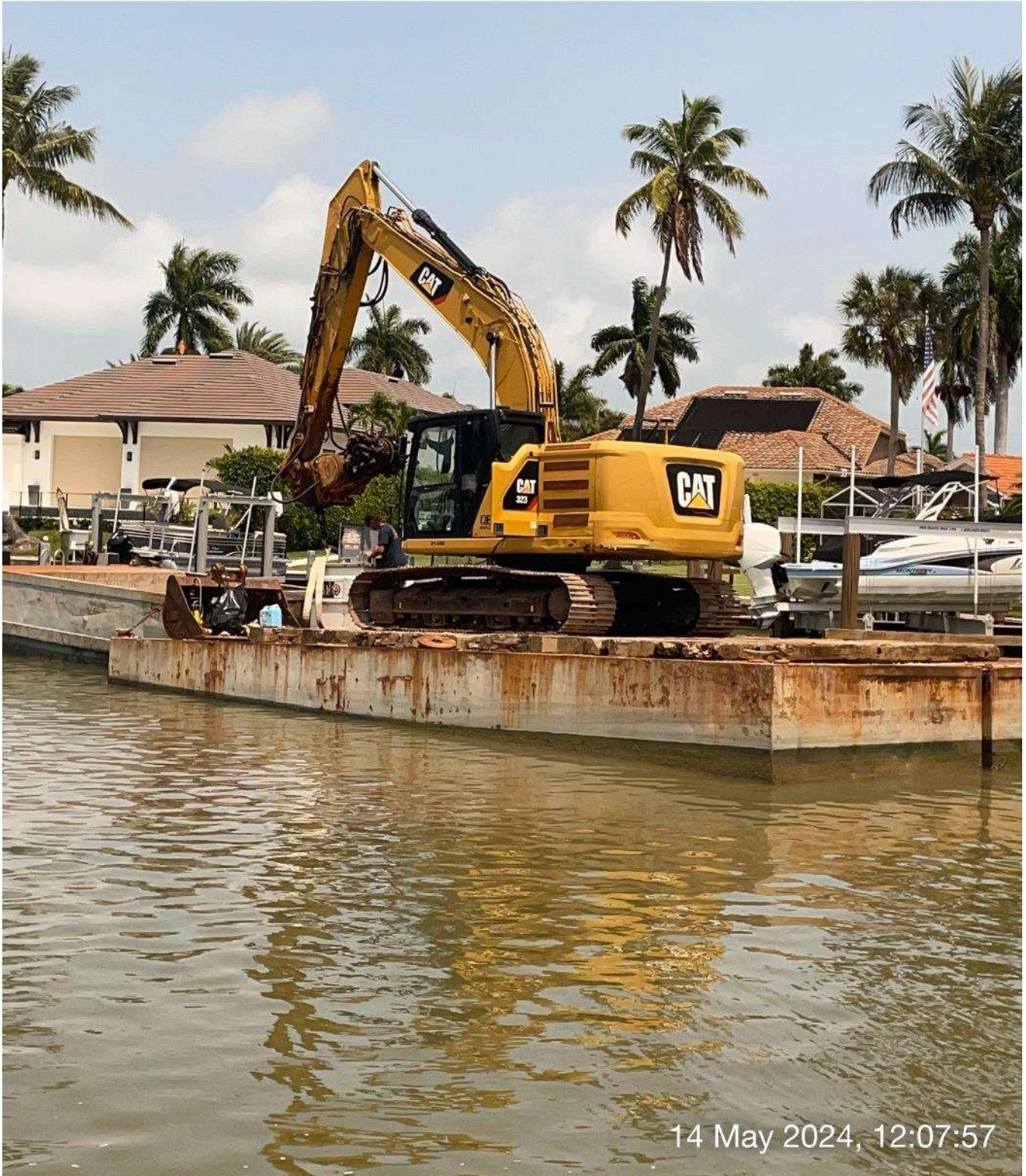
Contractor refueling 323 excavator.
