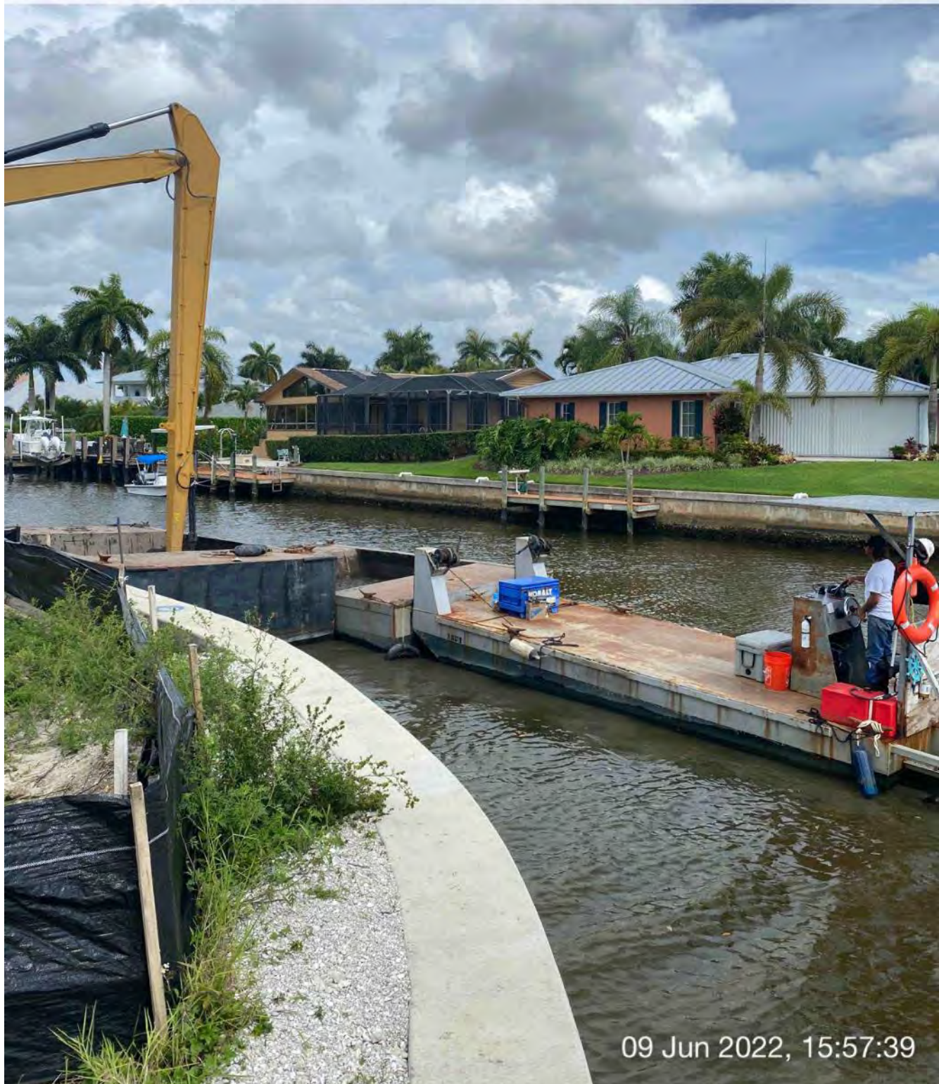
Push boat dropping off full hopper of material and picking up empty hopper of material in Canal CC-CC
