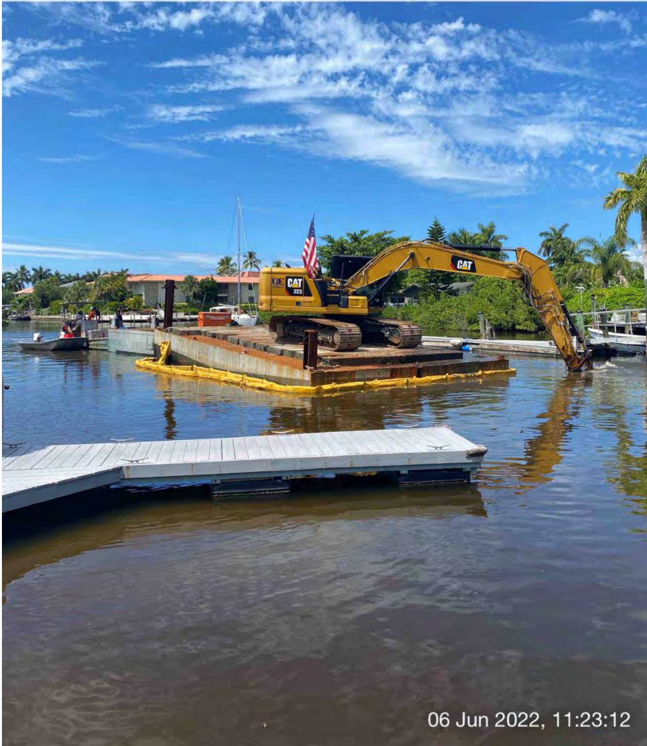
323 excavator removing material from station 16+00
