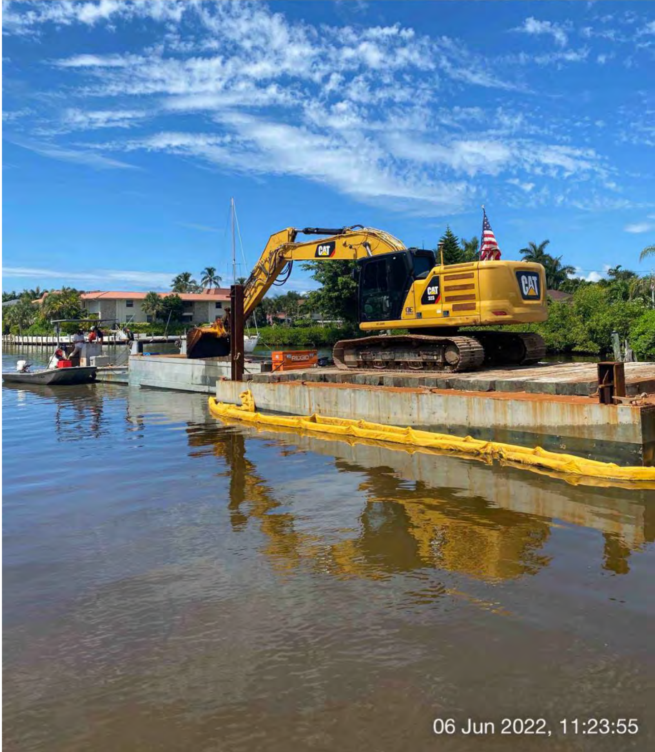
323 excavator transferring removed material to hopper
