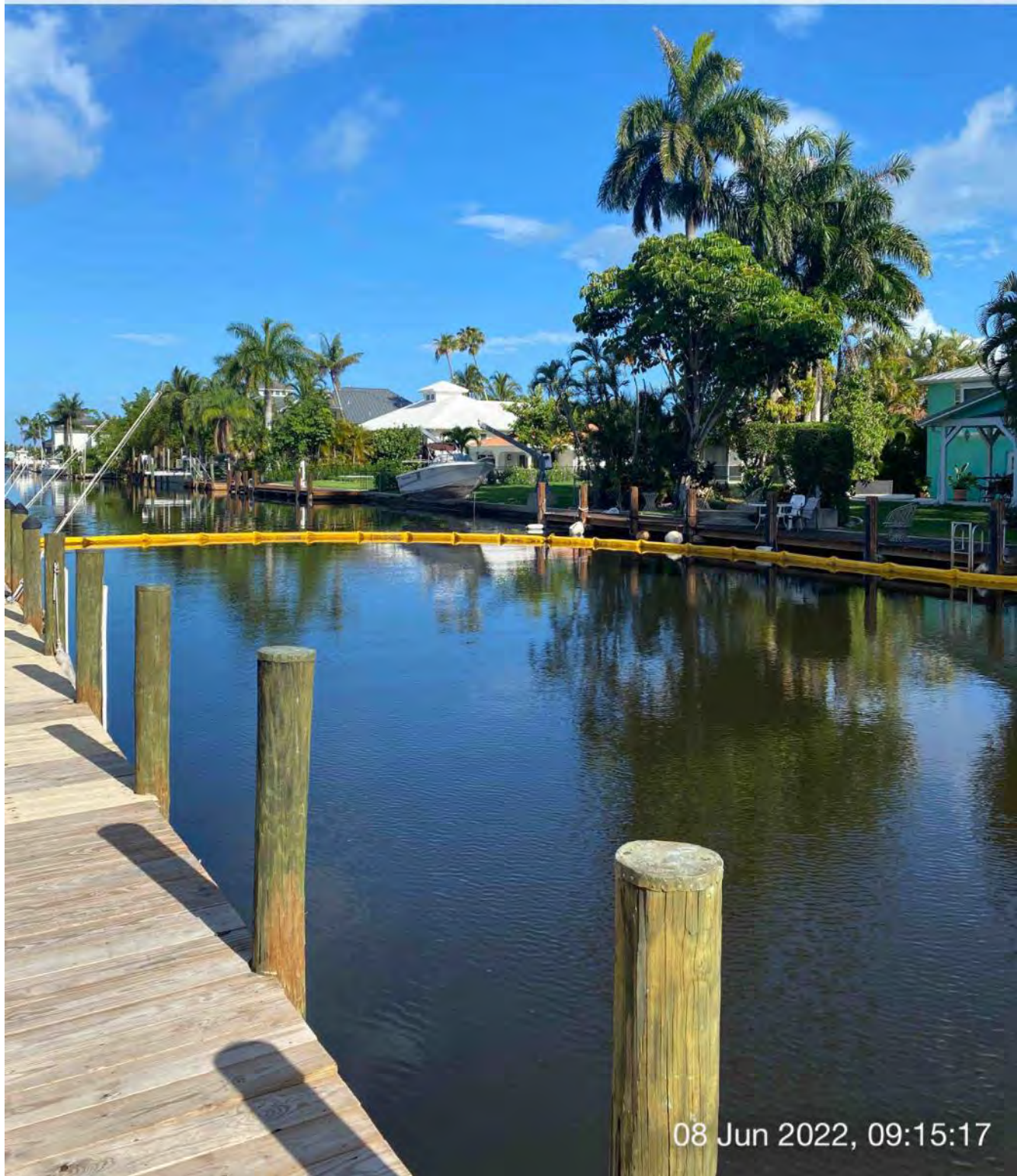
Turbidity curtain installed across Canal X-X at station 10+50
