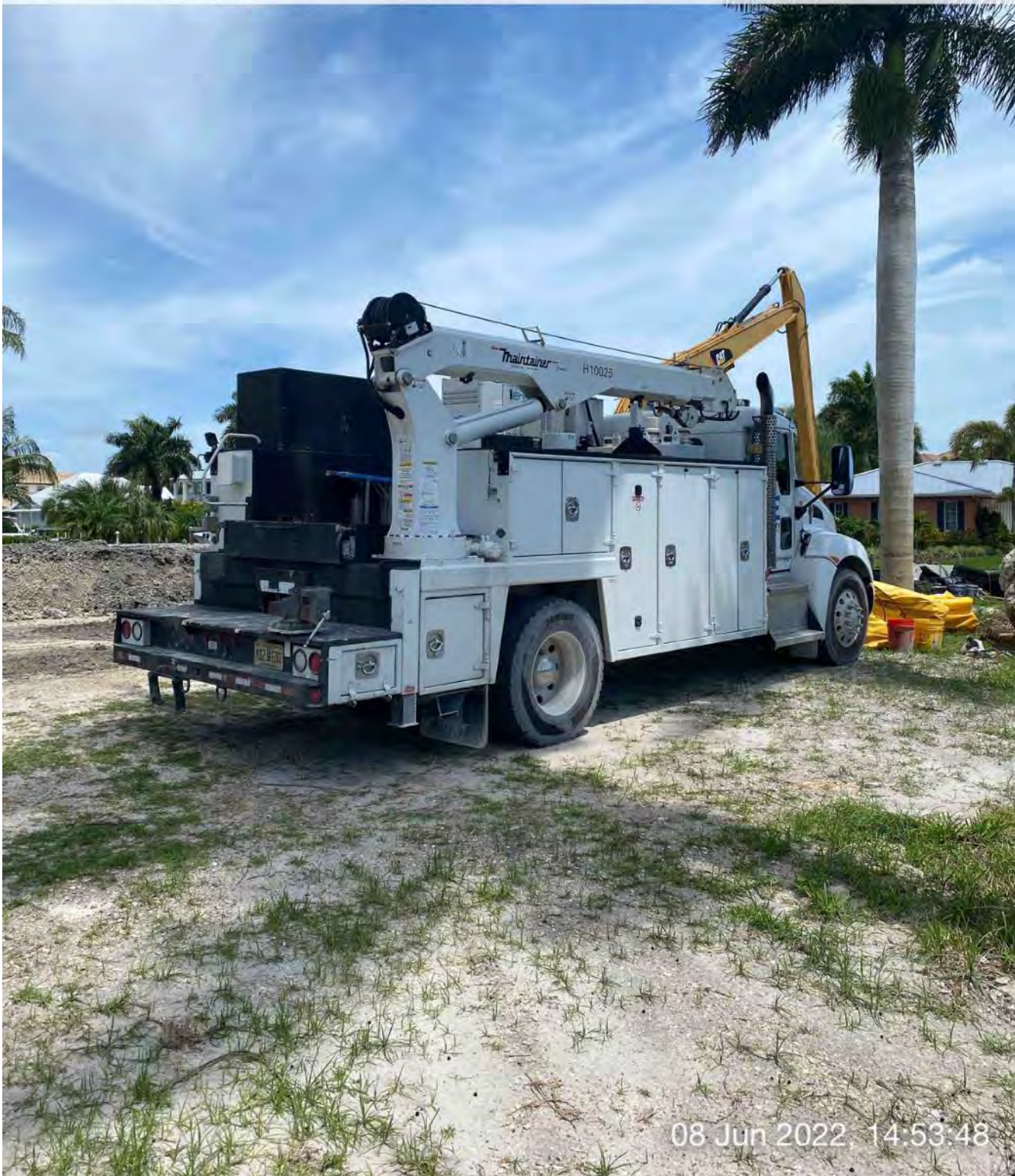
Utility truck on site at 1300 Curlew Avenue
