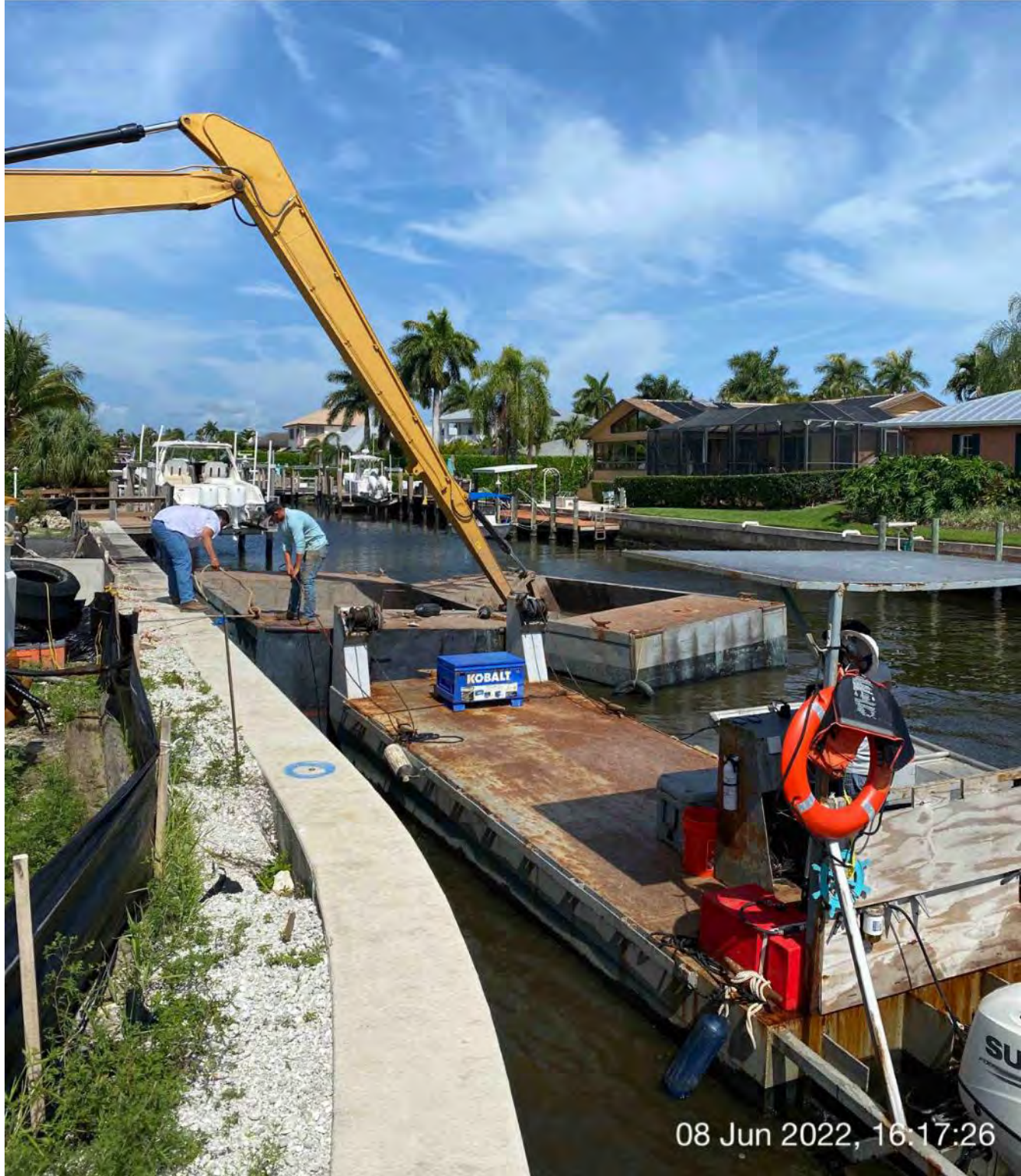
Push boat dropping off full hopper of material and picking up empty hopper of material in Canal CC-CC
