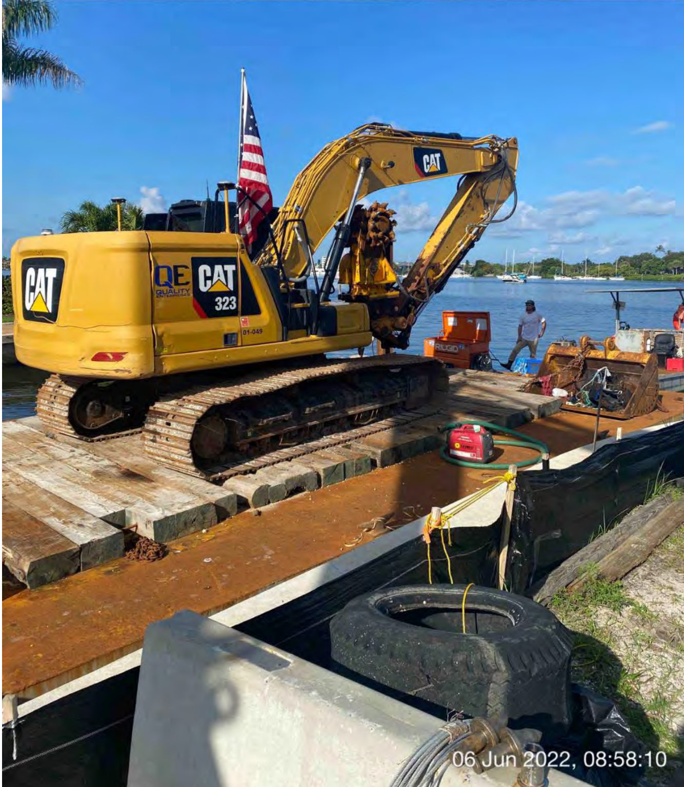
Contractor removing Epiroc grinder from 323 excavator
