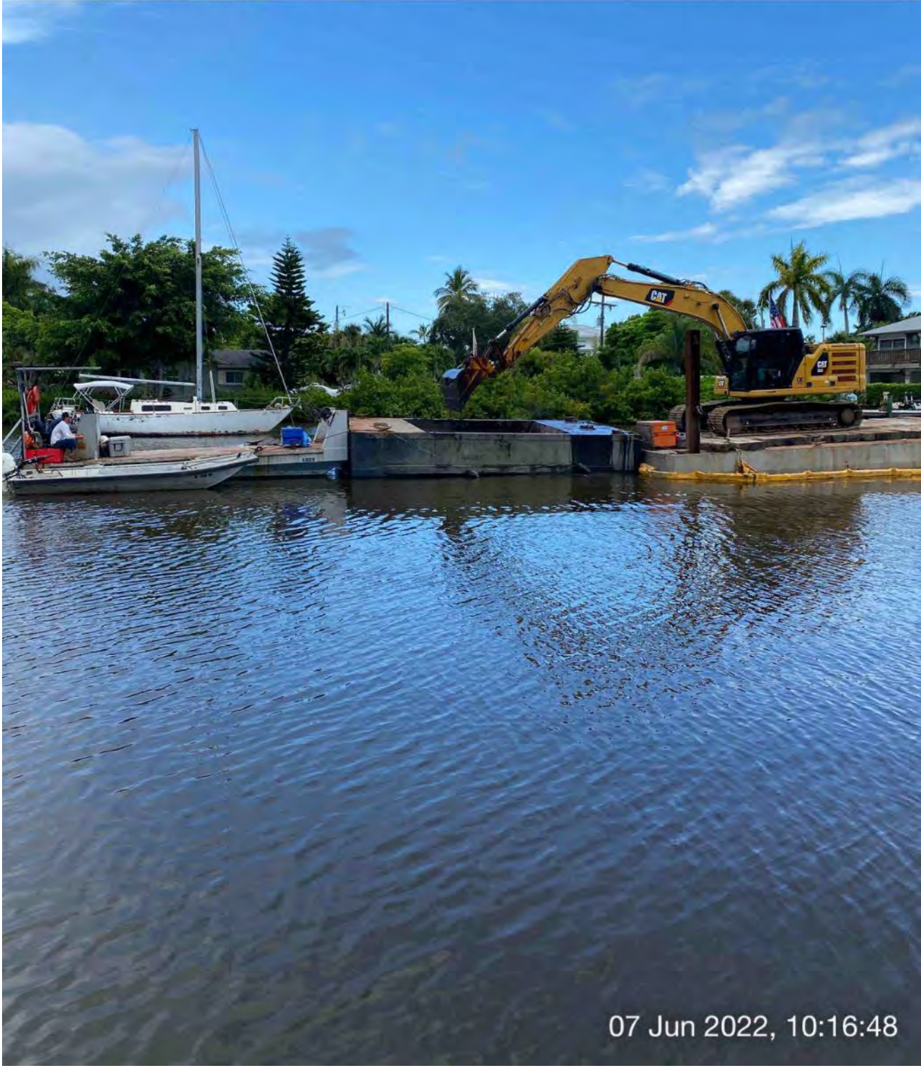
323 excavator transferring removed material to hopper
