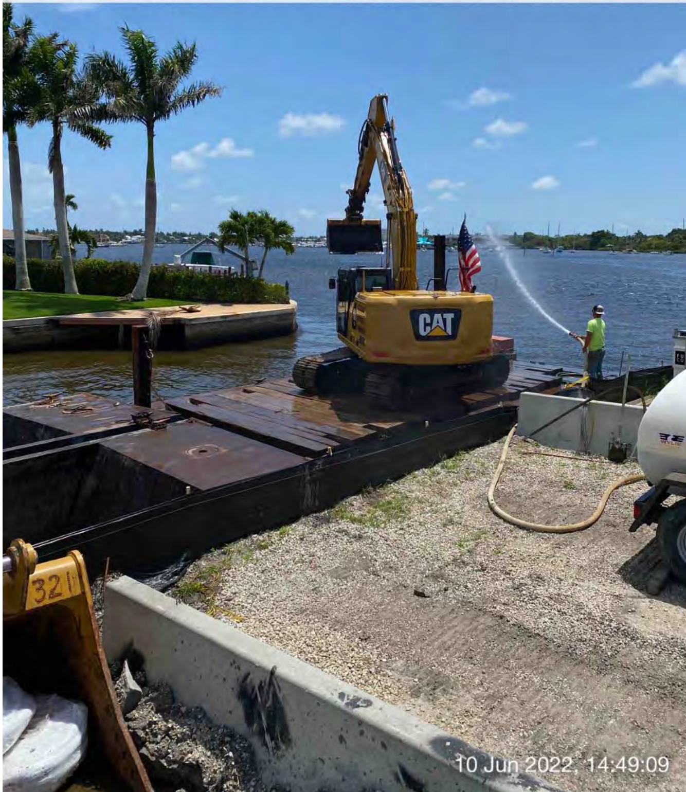
Contractor using water tank and hose to clean equipment
