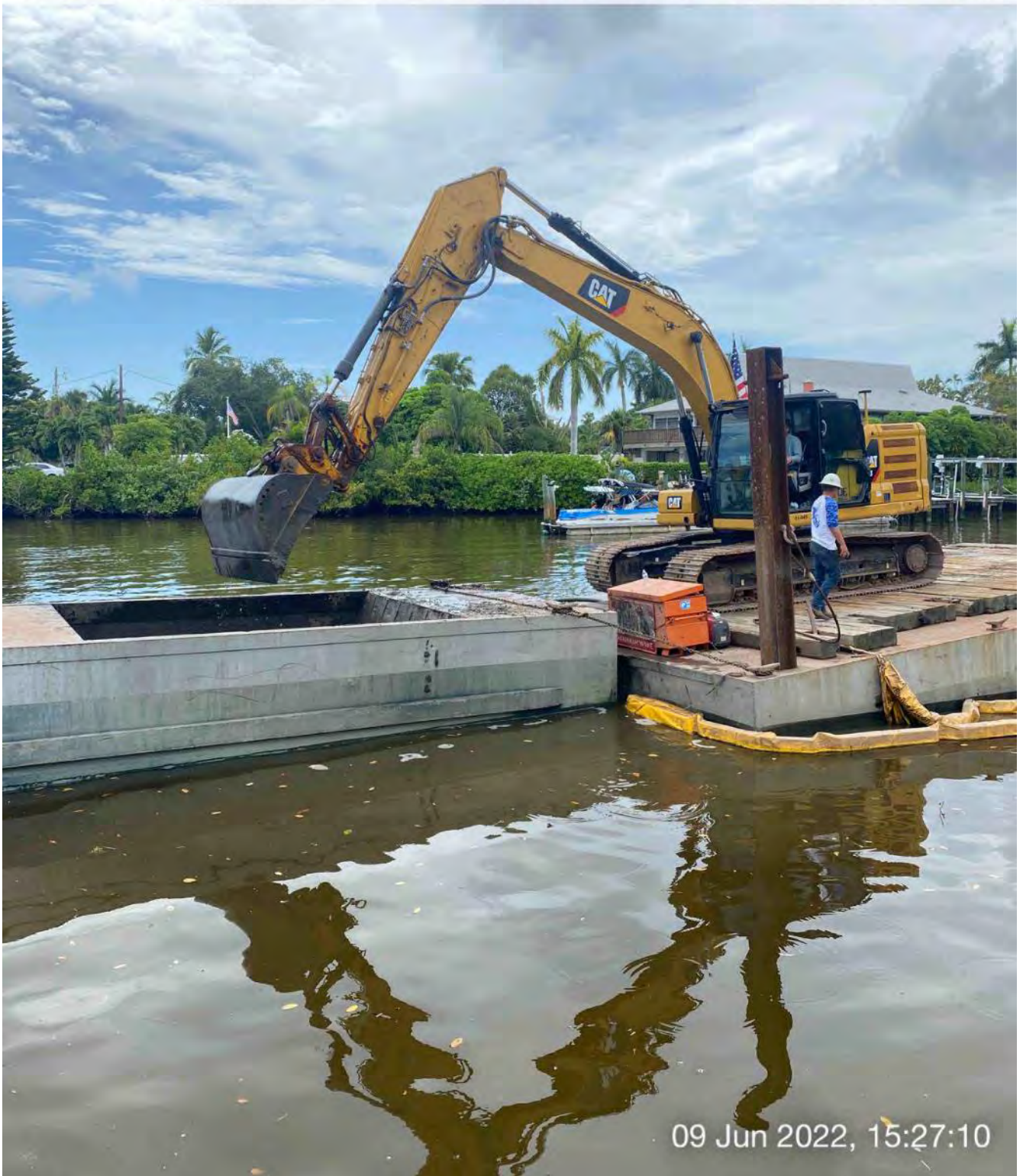
323 excavator removing material from station 15+50 and transferring to hopper
