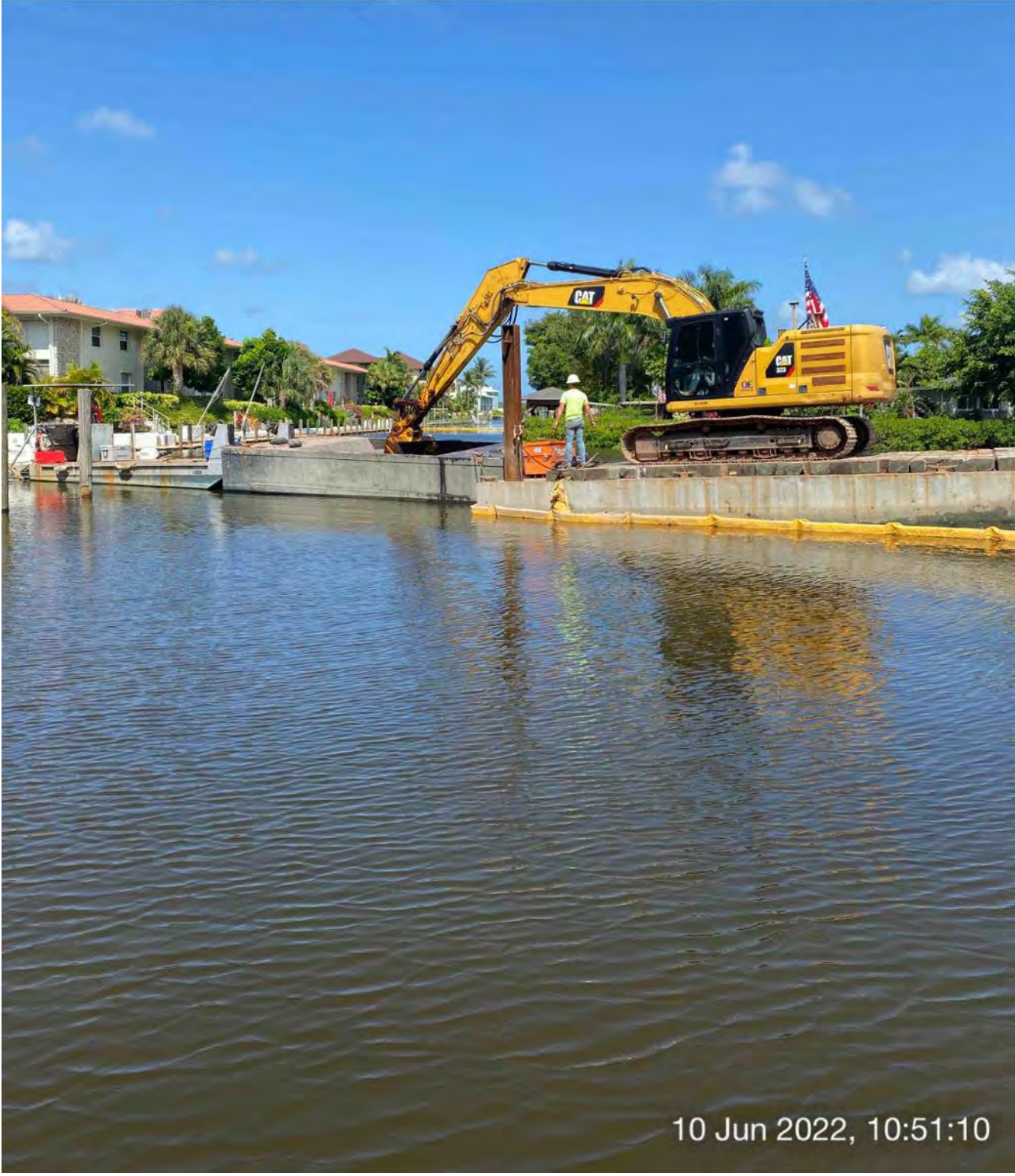
323 excavator removing material from station 14+00 and transferring to hopper
