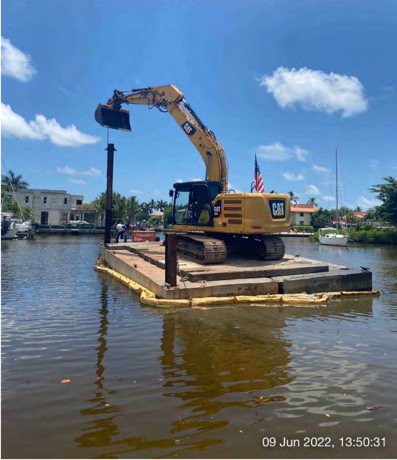
323 excavator lifting spud to allow push boat to mobilize barge at station 15+50
