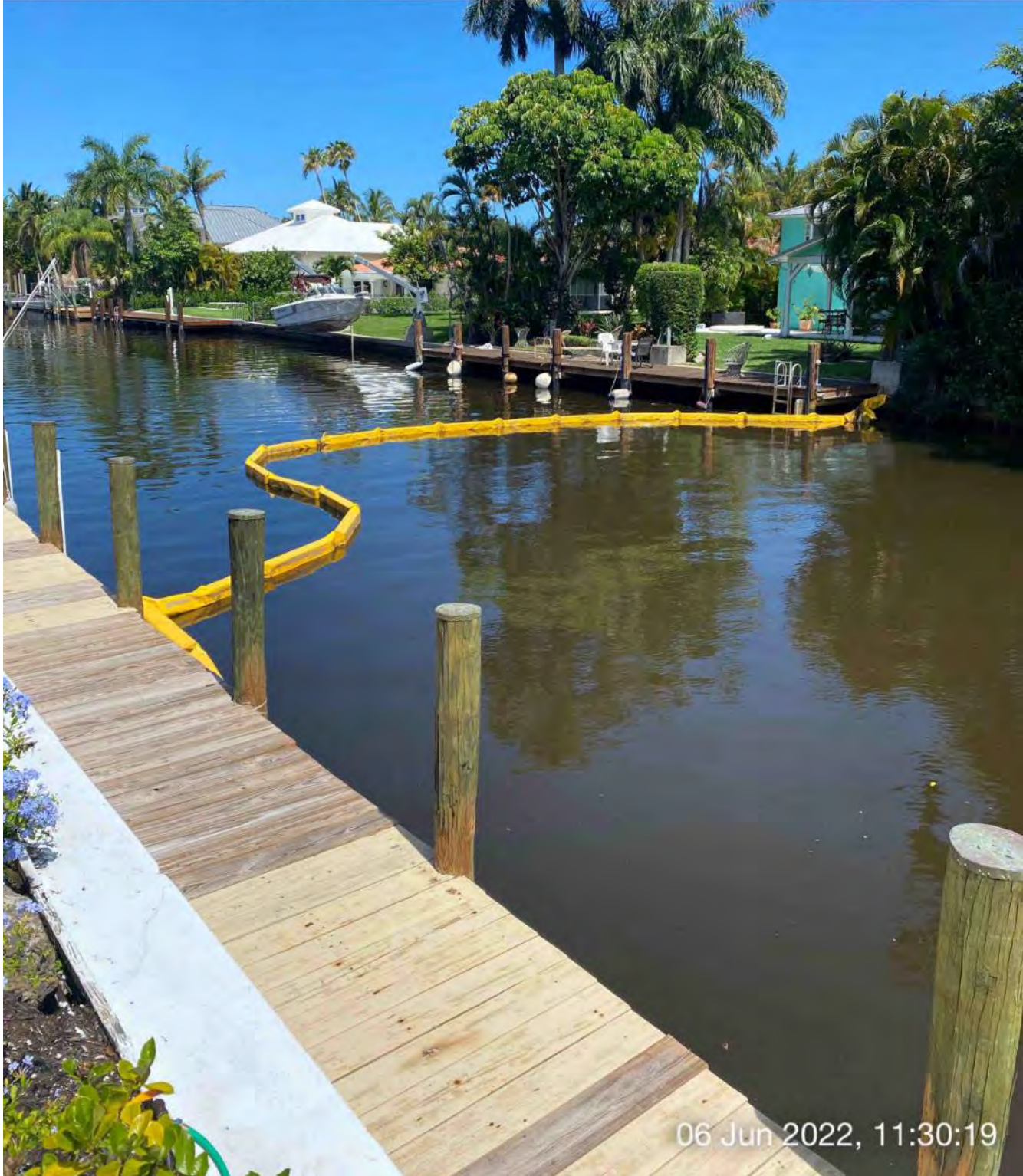
Turbidity curtain installed across Canal X-X at station 10+75
