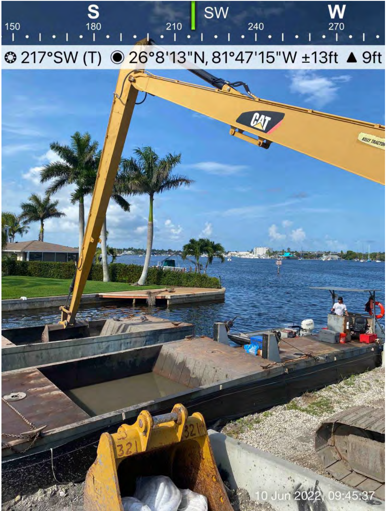
326 excavator transferring material rom hopper to dewatering site at 1300 Curlew Avenue
