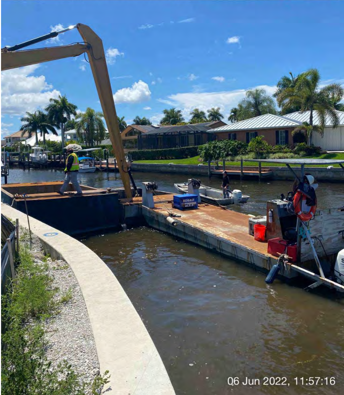
Push boat dropping full hopper off in Canal CC-CC at station 1+50
