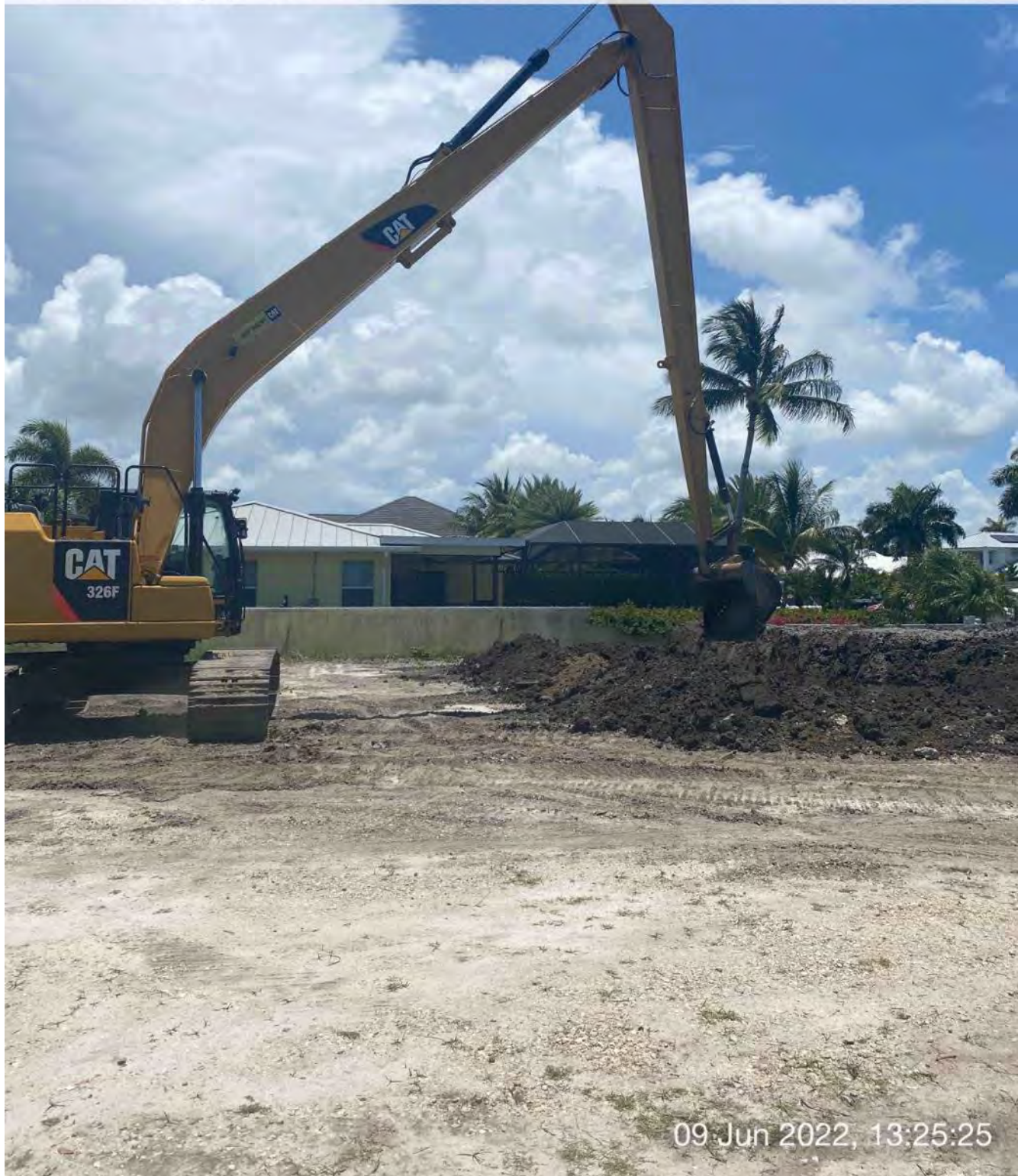
326 excavator redistributing removed material at dewatering site at 1300 Curlew Avenue
