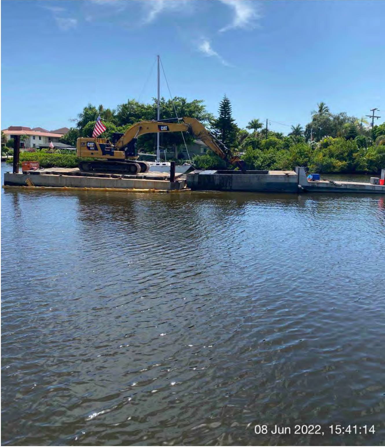
323 excavator removing material from station 14+25 and transferring to hopper
