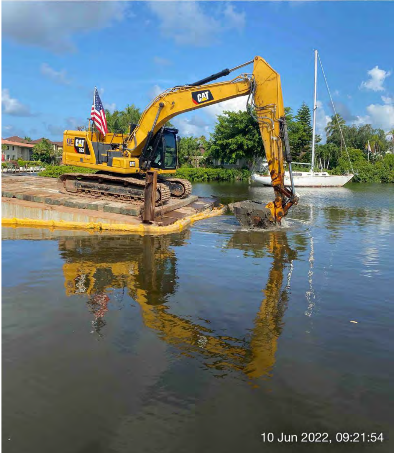
323 excavator removing material from station 14+50
