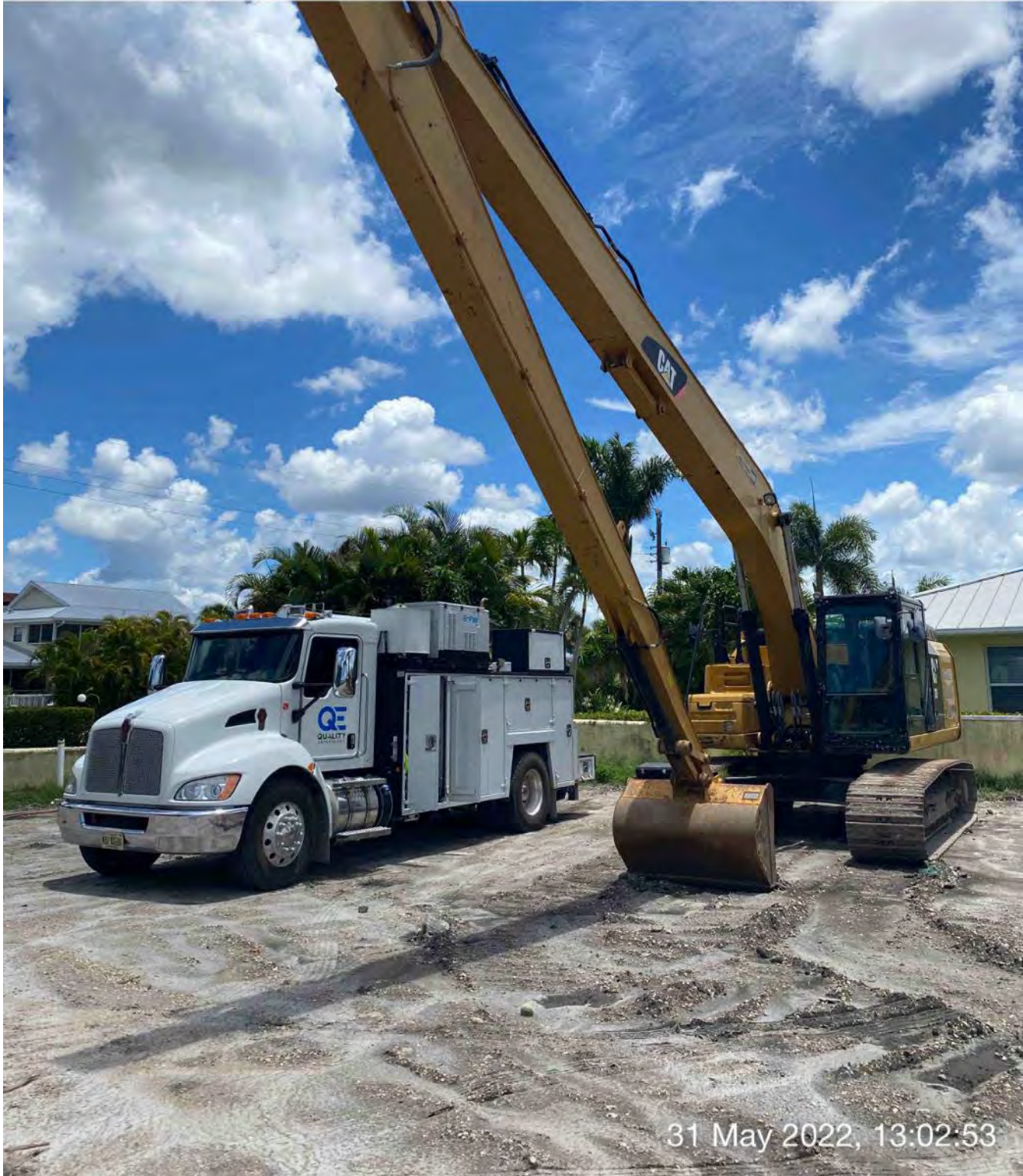
Utility truck and 326 excavator at 1300 Curlew Avenue
