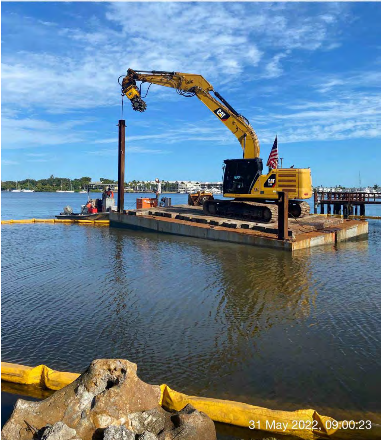
323 excavator lifting spud to allow push boat to mobilize barge at station 0+75
