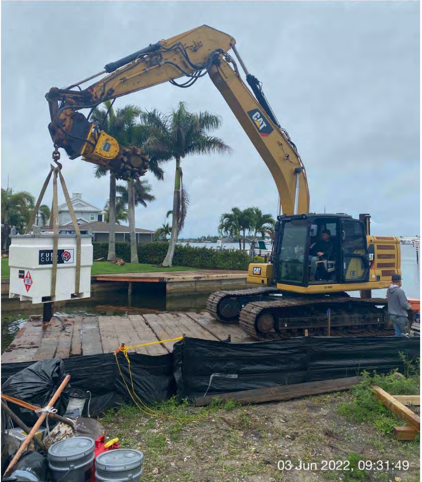
323 excavator transporting fuel cube from barge to site at 1300 Curlew Avenue
