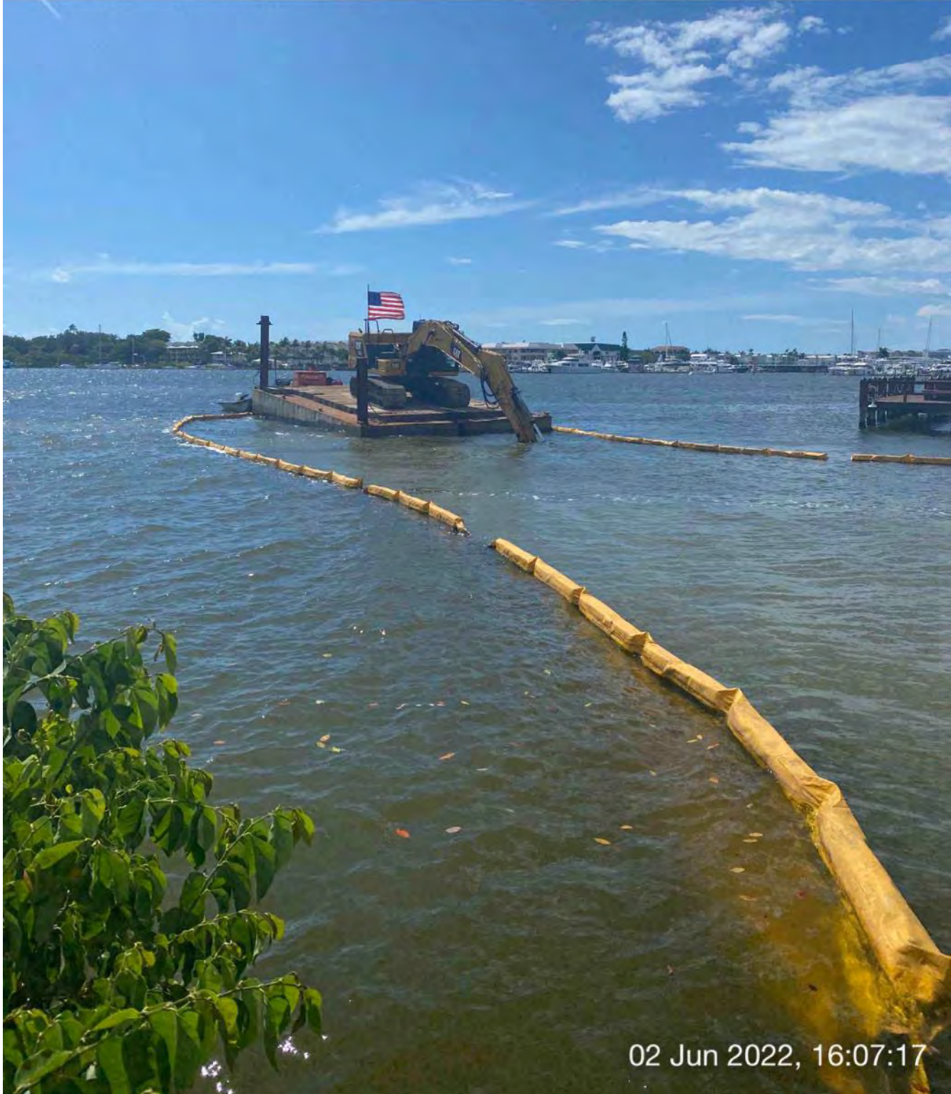
323 excavator grinding rock at station 0+00
