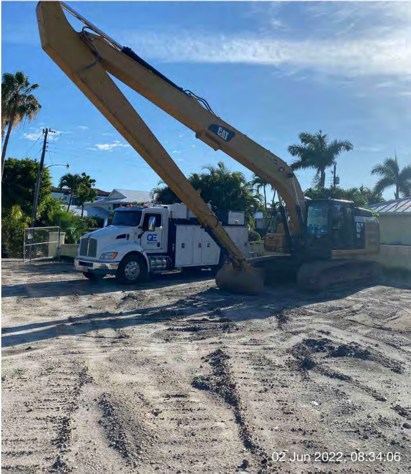
Utility truck and 326 excavator on site at 1300 Curlew Avenue
