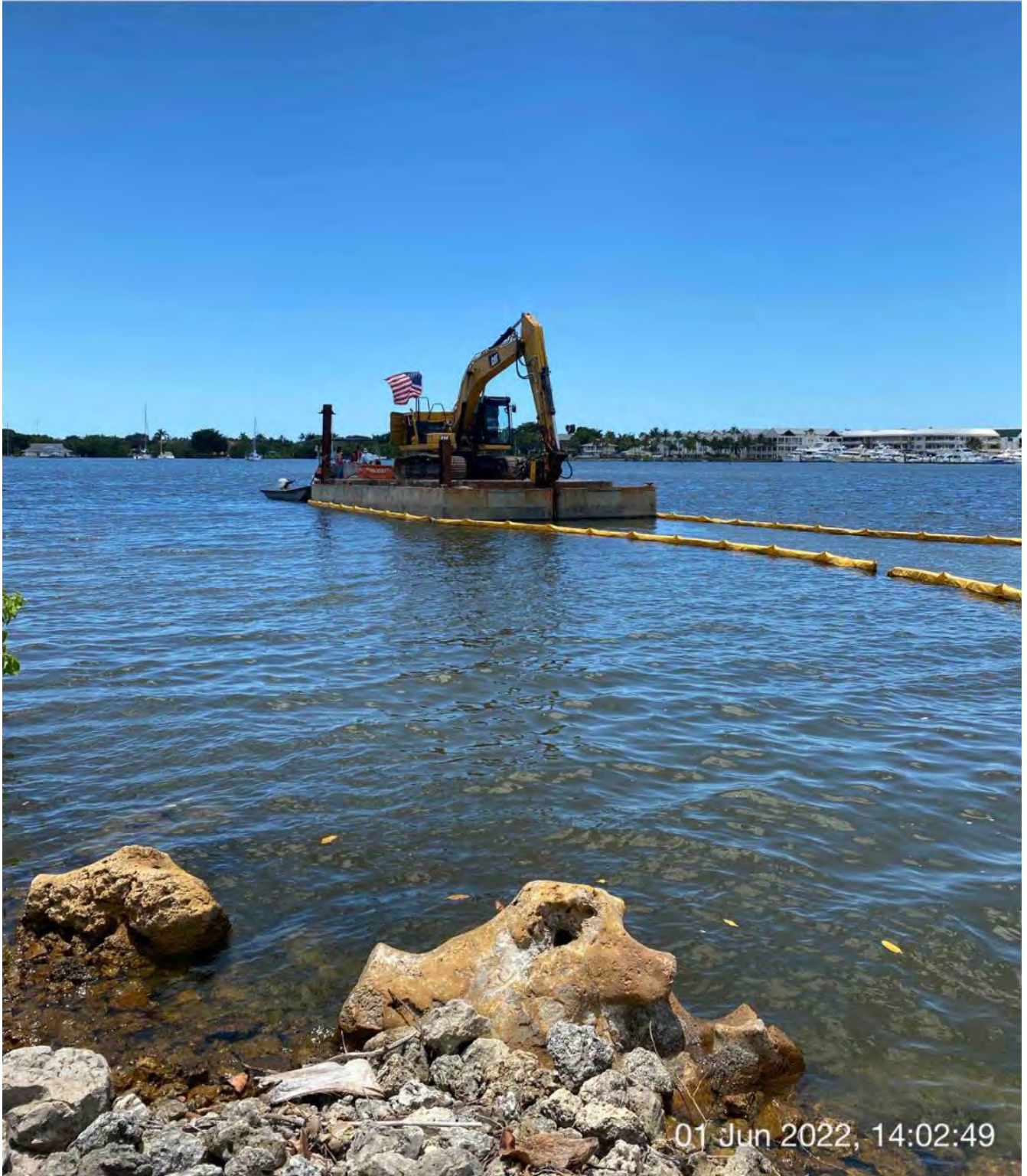
323 excavator on barge at station 0+25
