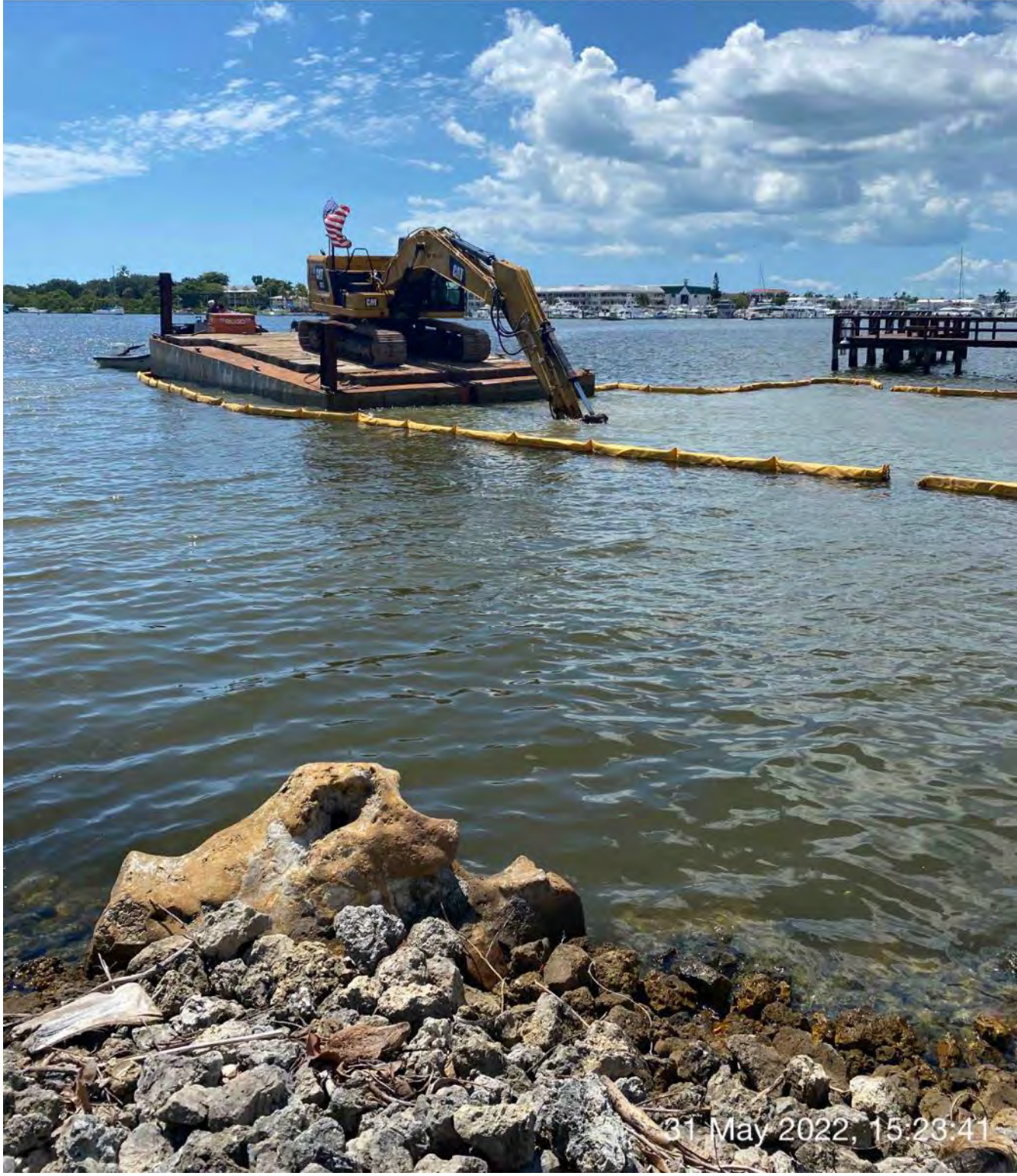
323 excavator grinding rock at station 0+50
