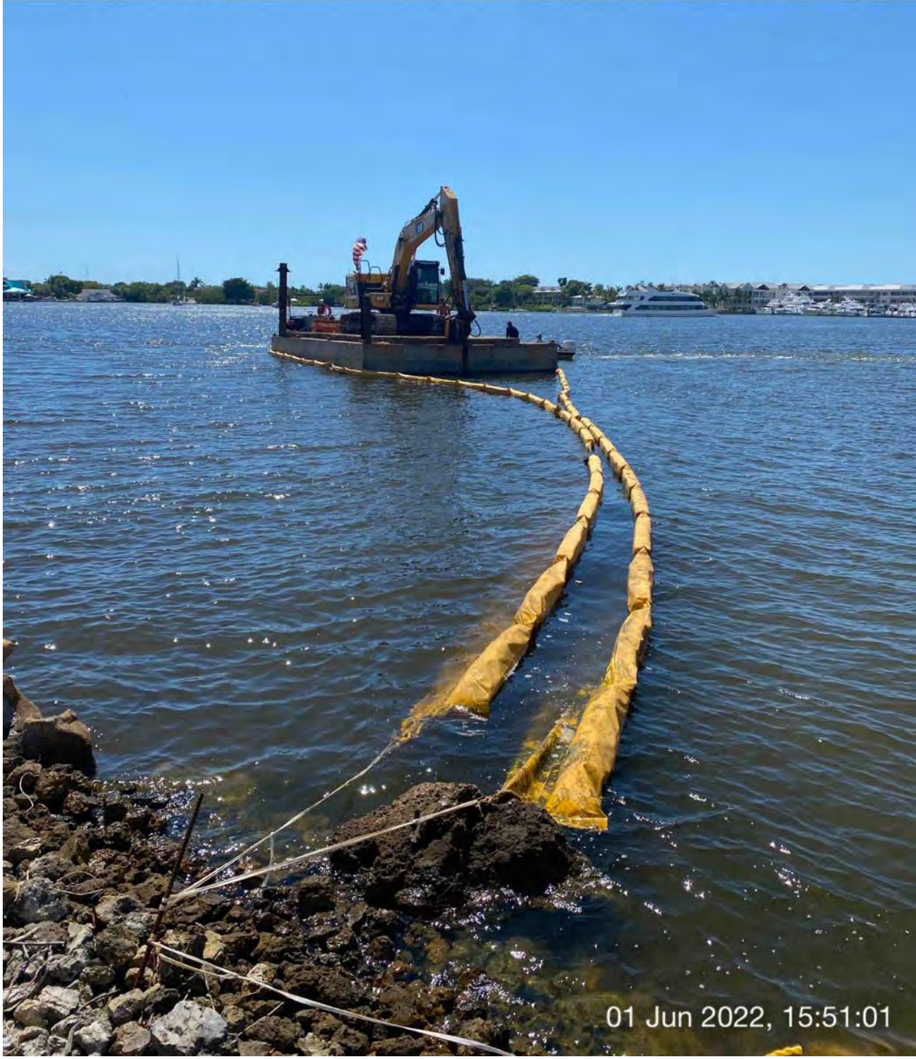
323 excavator on barge at station 0+25 and turbidity curtain tied up
