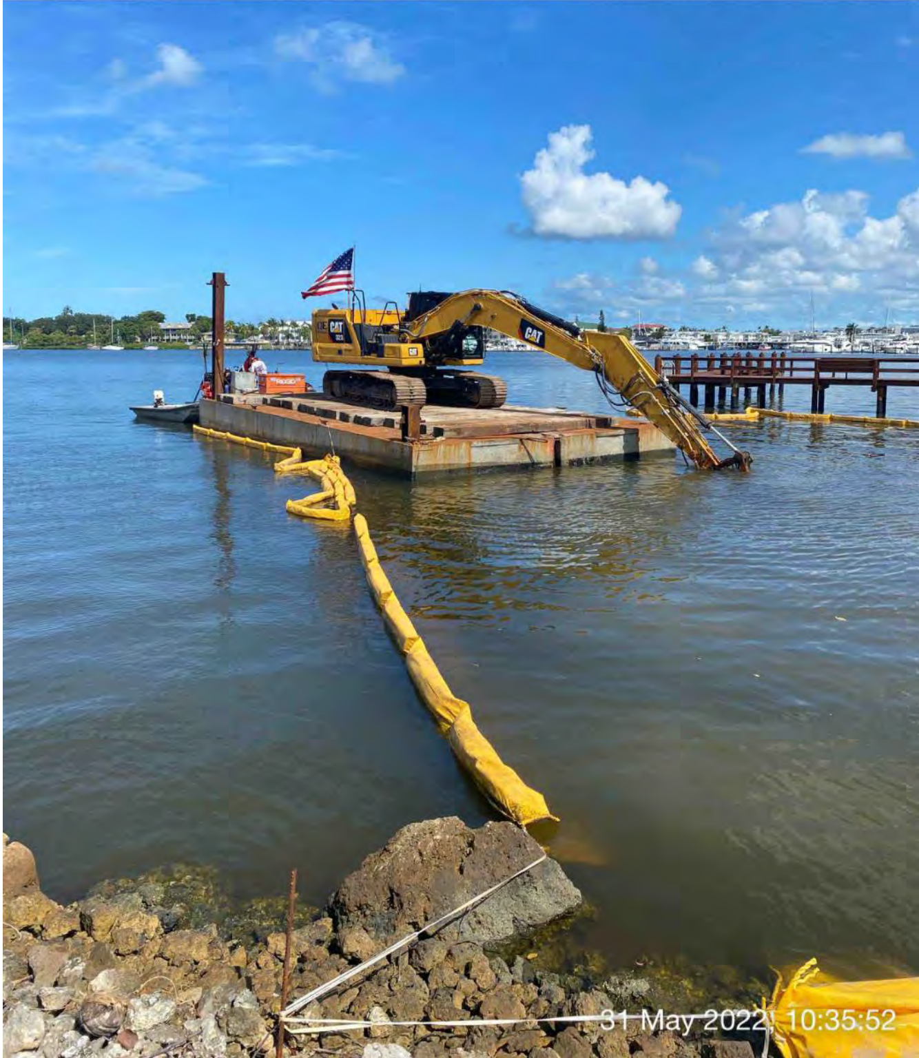
323 excavator grinding rock at station 0+75
