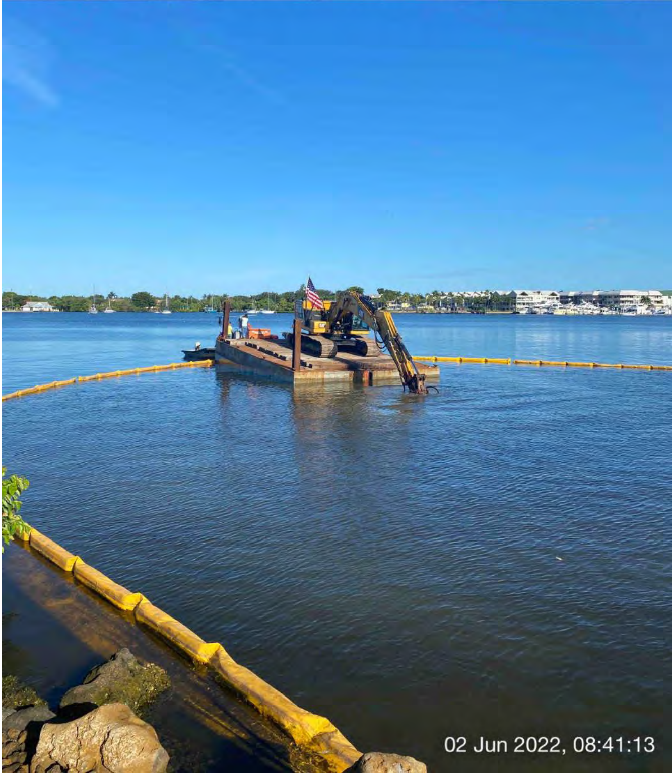
323 excavator grinding rock at station 0+25
