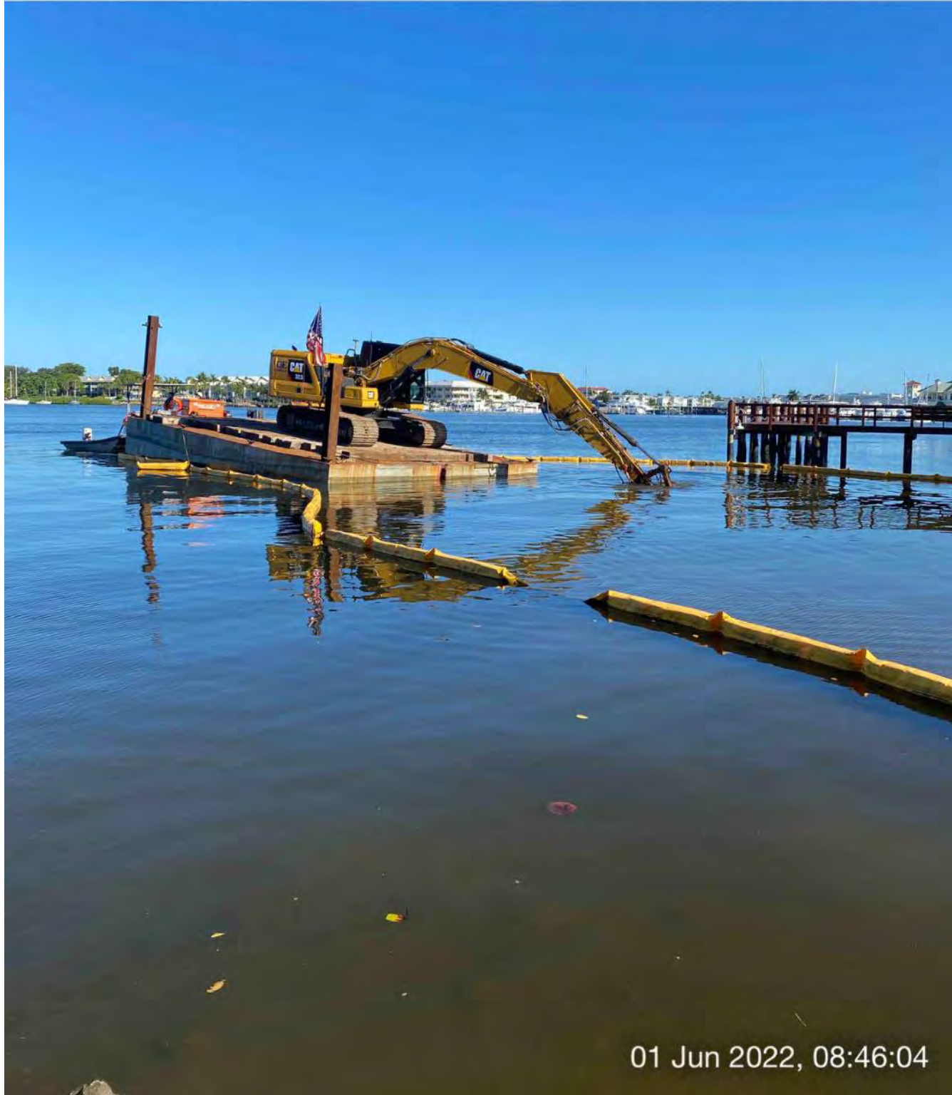
323 excavator grinding rock at station 0+50
