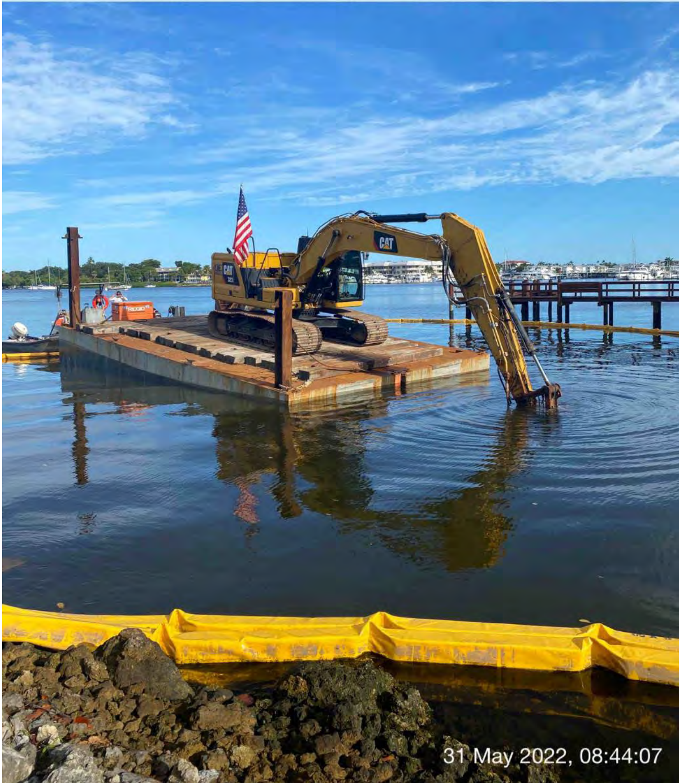
323 excavator grinding rock at station 1+00
