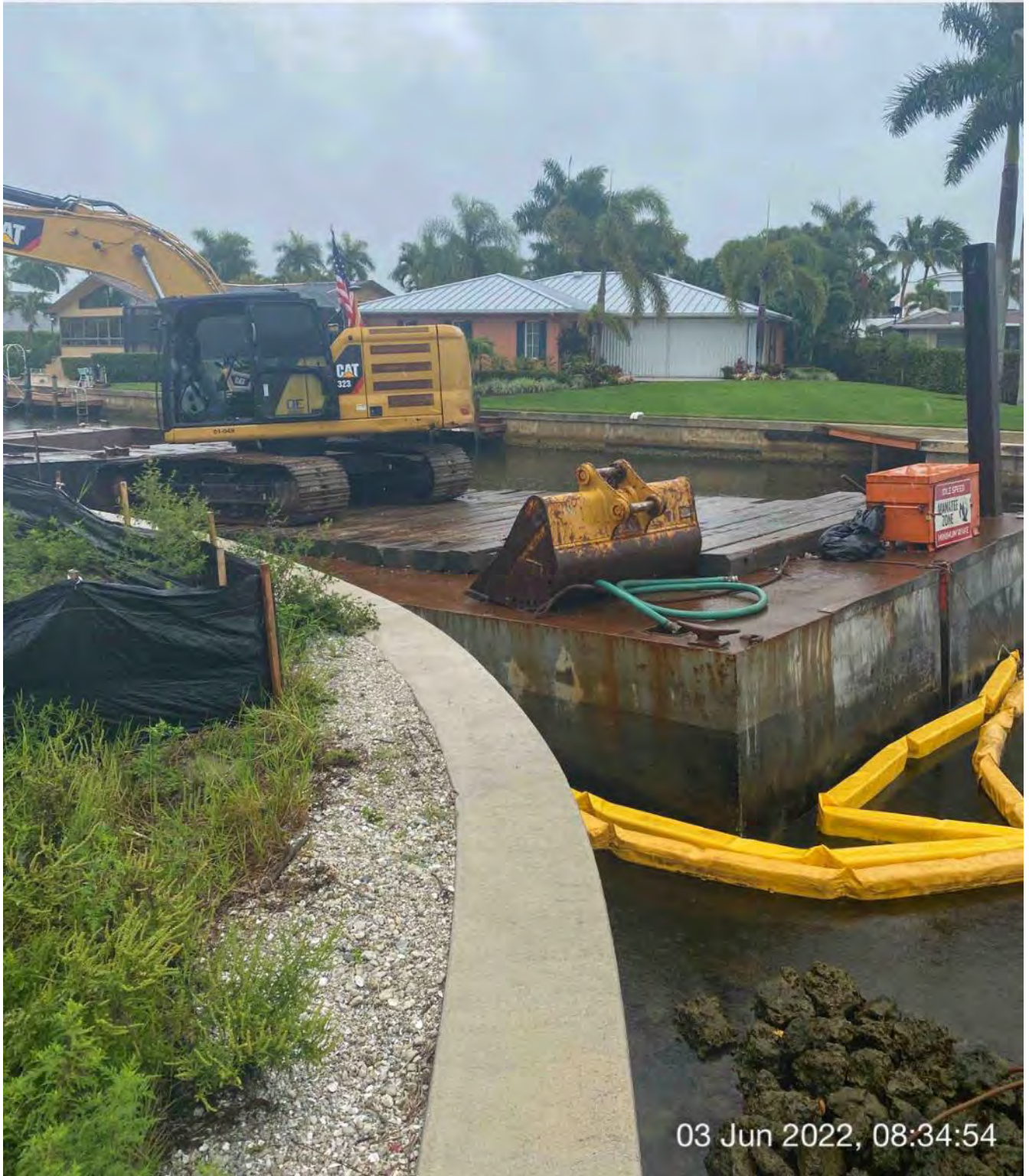
Barge, 323 excavator, and turbidity curtain stationed in Canal CC-CC at station 1+00
