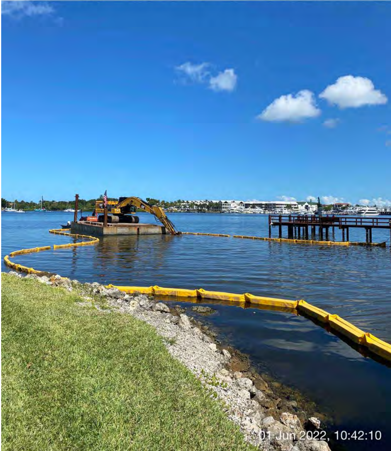
323 excavator grinding rock at station 0+50
