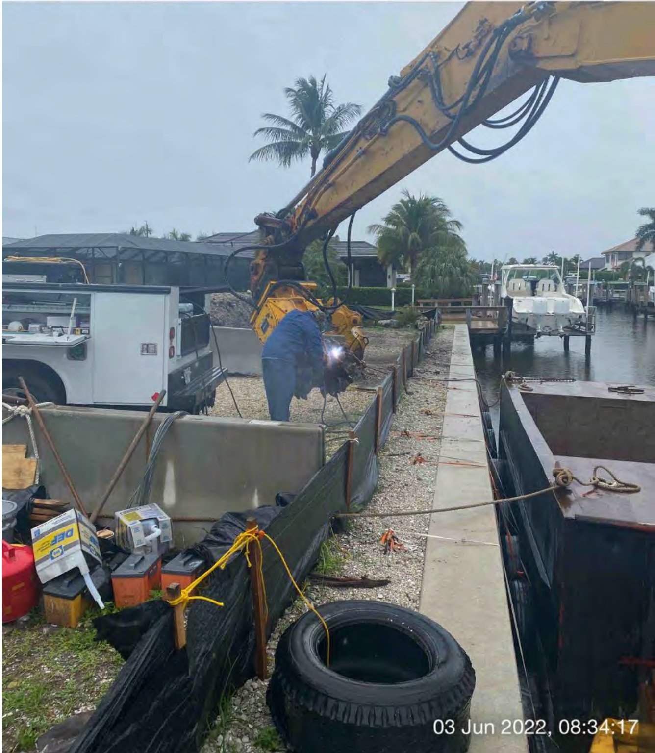
Contractor welding sleeves on Epiroc grinder attachment
