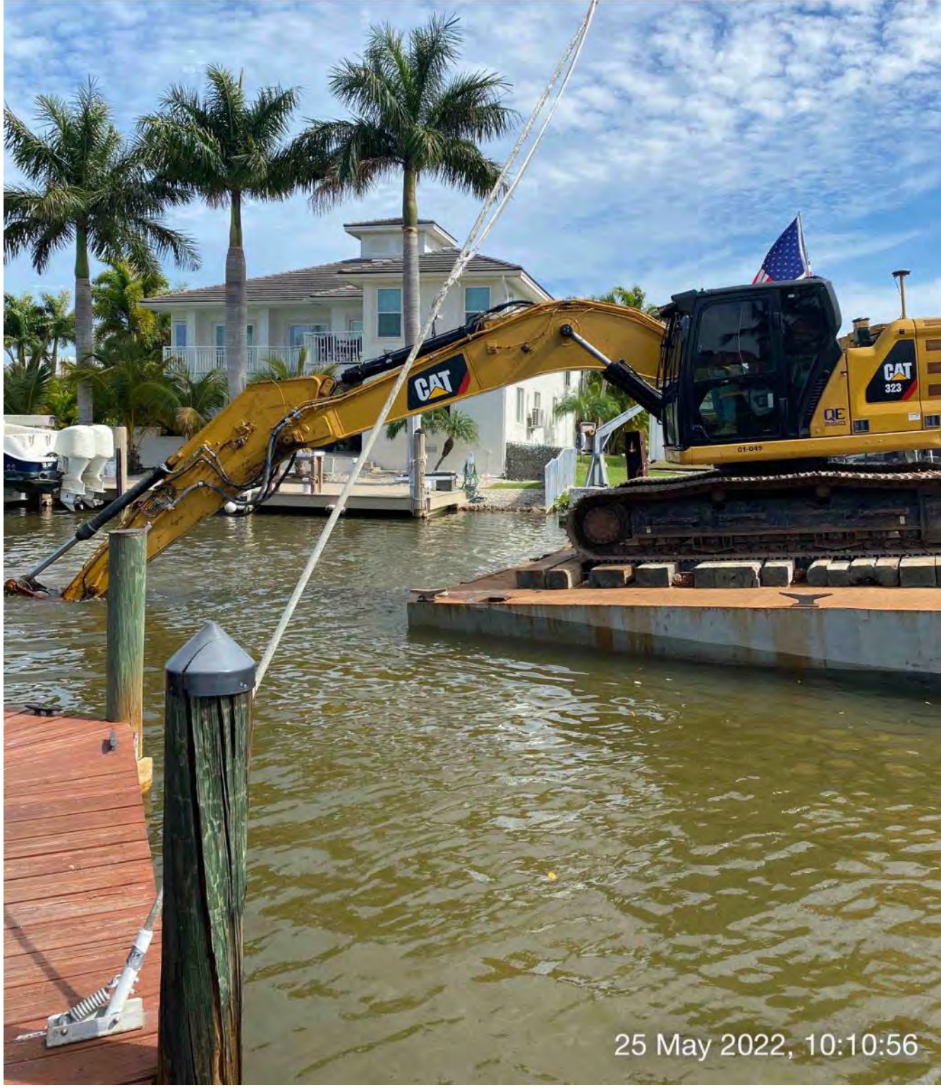
323 excavator grinding rock at station 4+50
