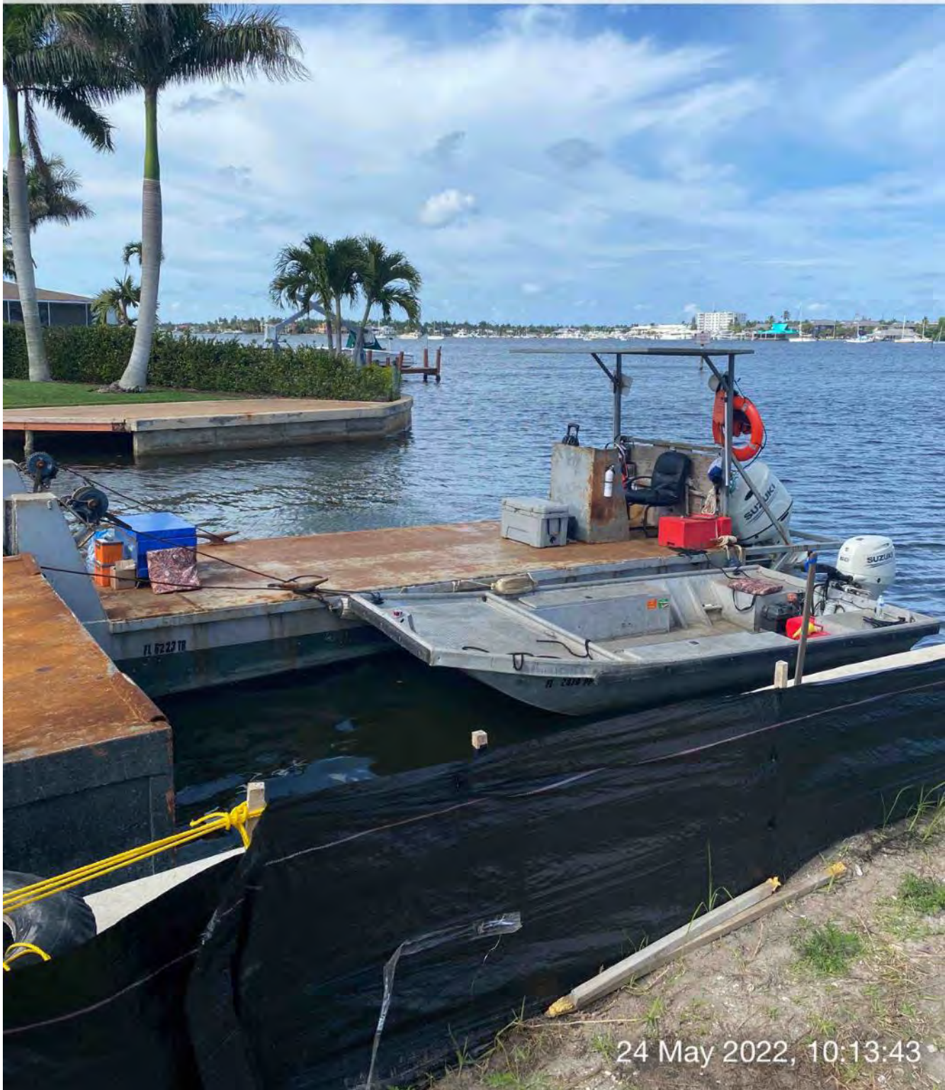
Push boat and support boat staged in Canal CC-CC at station 1+00.
