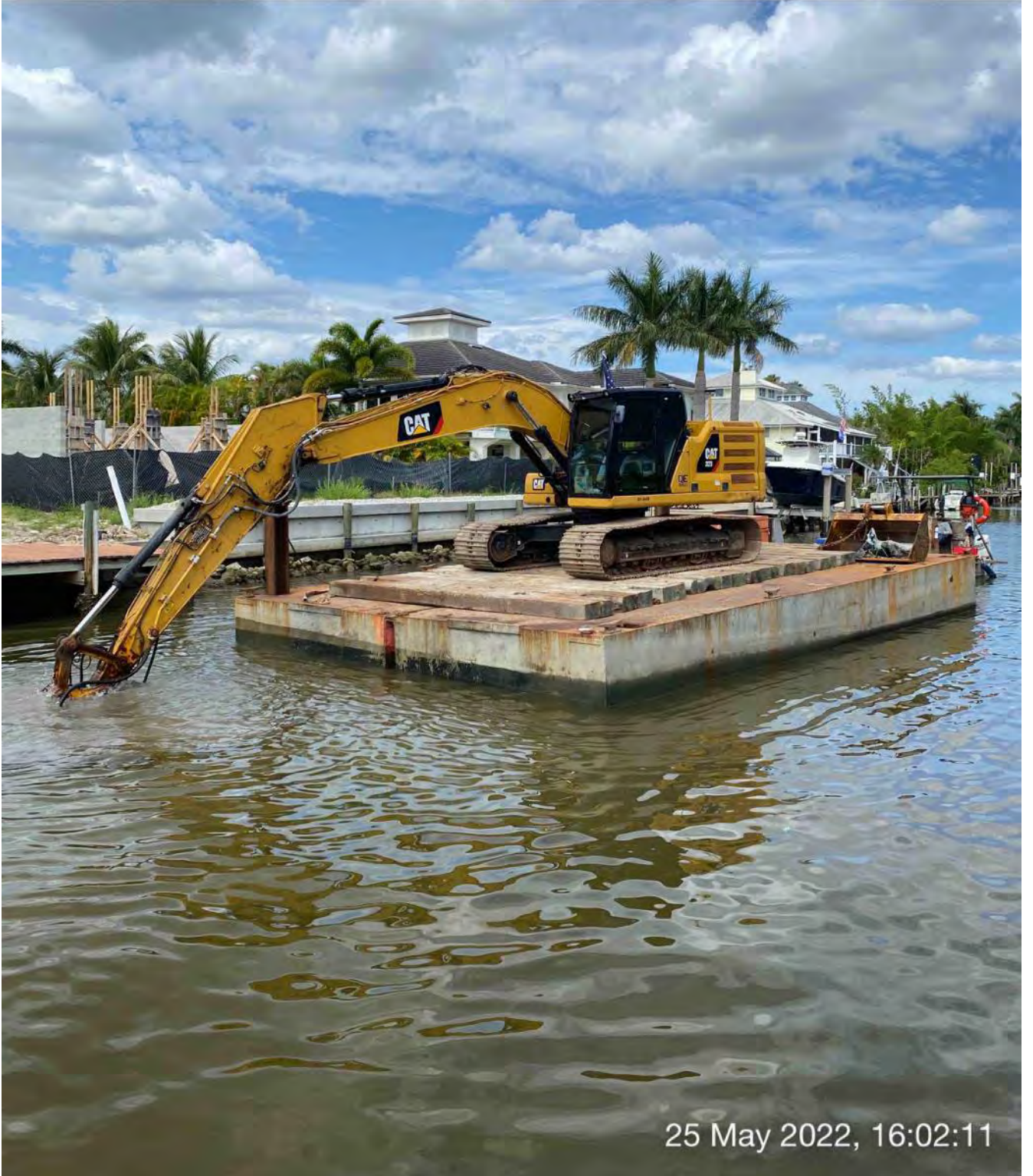
323 excavator grinding rock at station 3+00
