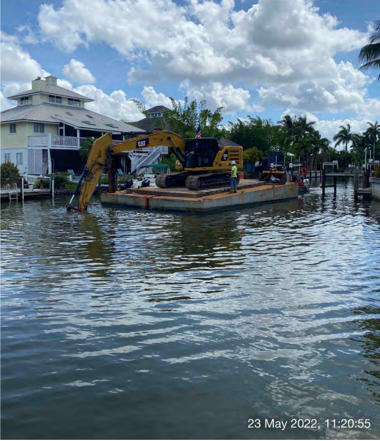
323 excavator checking elevations and grinding rock at station 5+75
