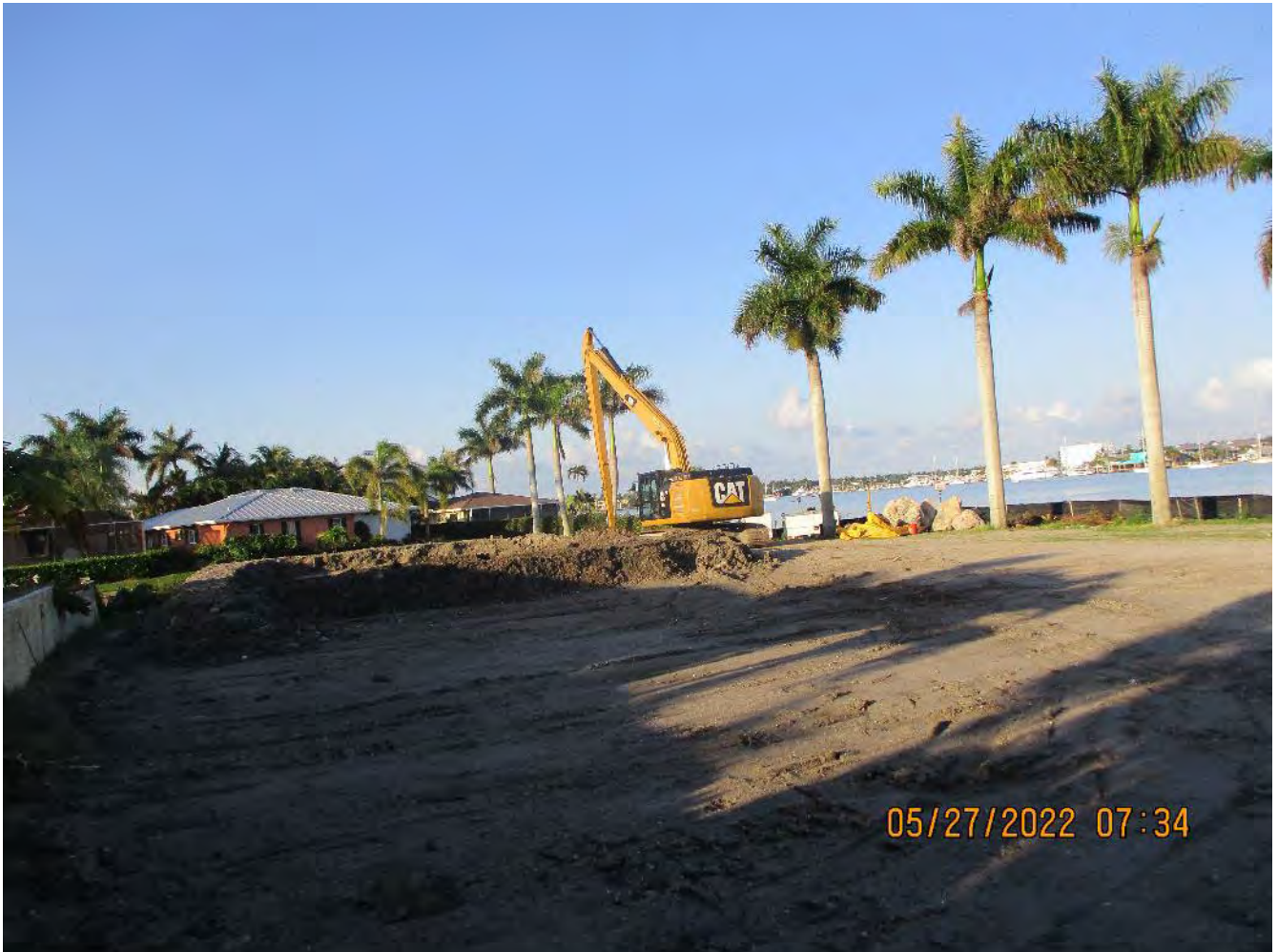
Current status of staging area/stockpile at 1300 Curlew Ave
