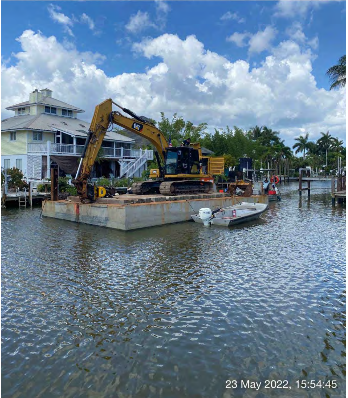
Mechanic on barge fixing coolant hose on 323 excavator
