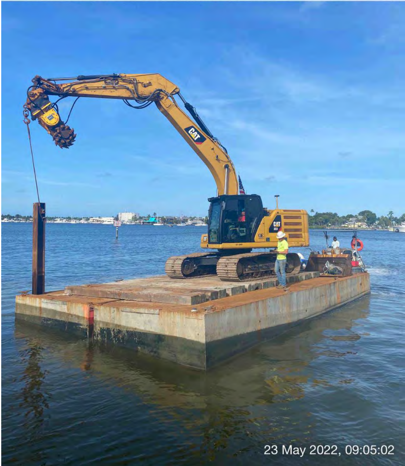
323 excavator lifting spud to allow push boat to transport barge from Canal CC-CC to Canal X-X
