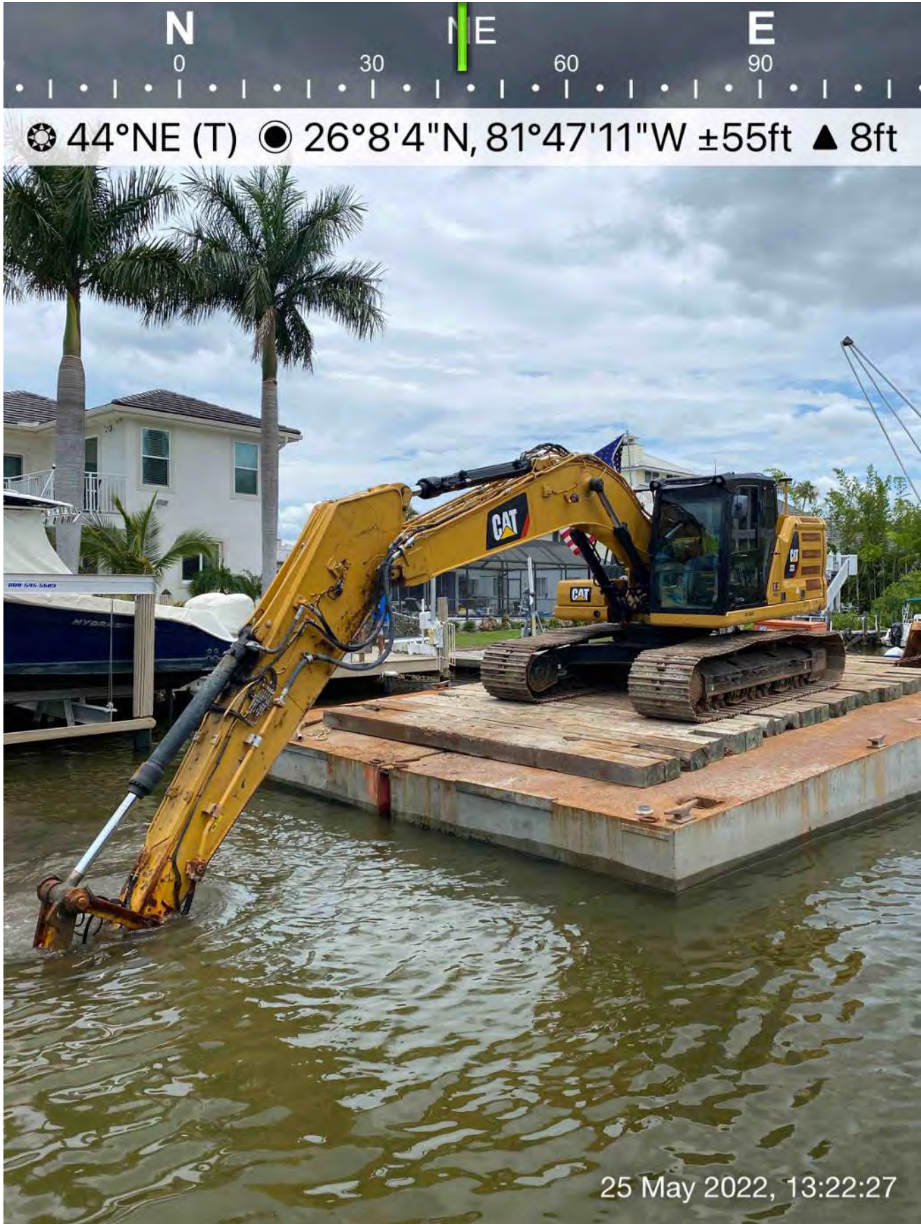
323 excavator grinding rock at station 3+50
