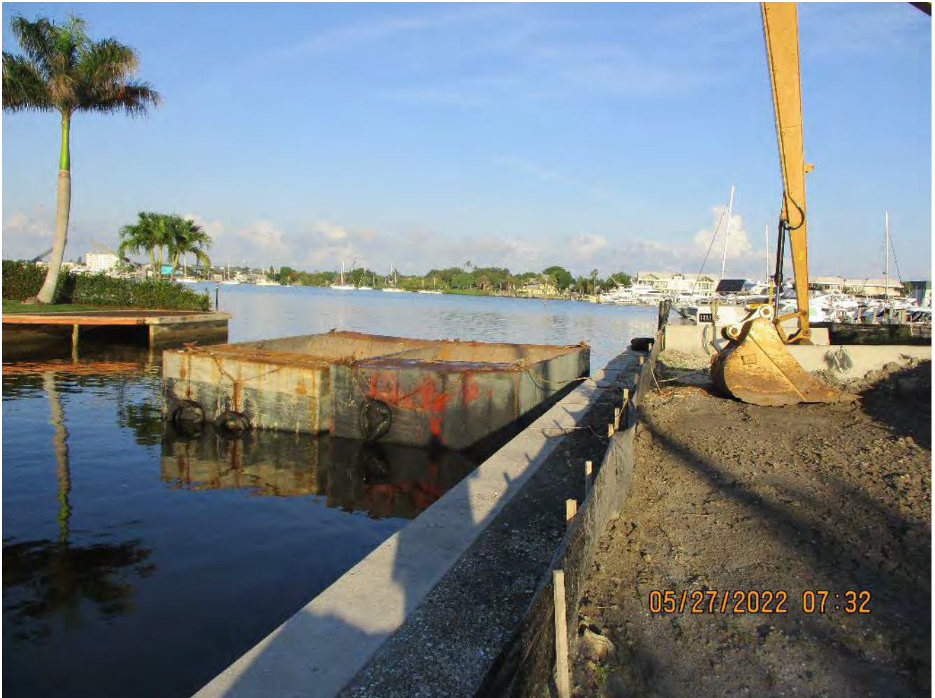
Staged hoppers at 1300 Curlew Ave. canal location
