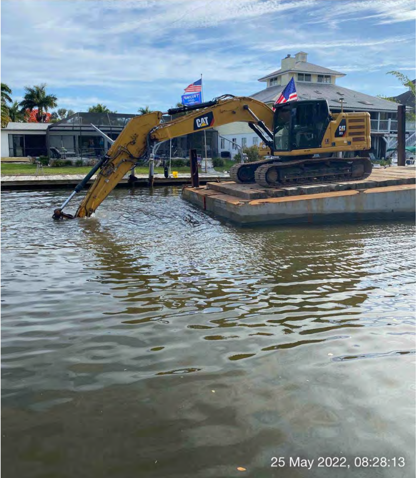
323 excavator grinding rock at station 5+25
