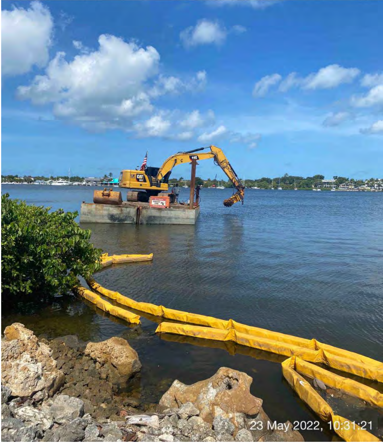
Pumping water out from the bottom of the barge
