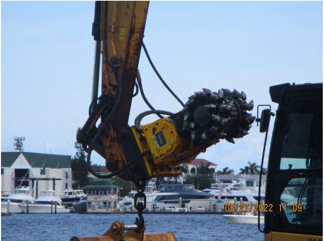
Epiroc attachment being used for today's canal bottom grinding
