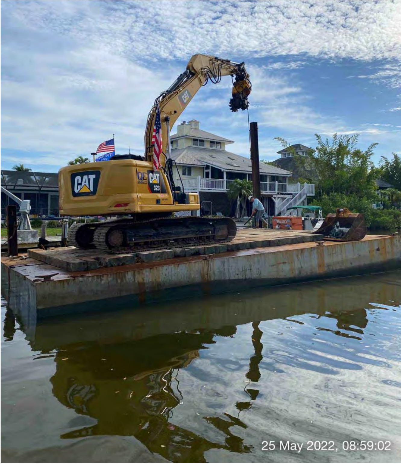
323 excavator lifting spud to allow push boat to mobilize barge at station 5+25
