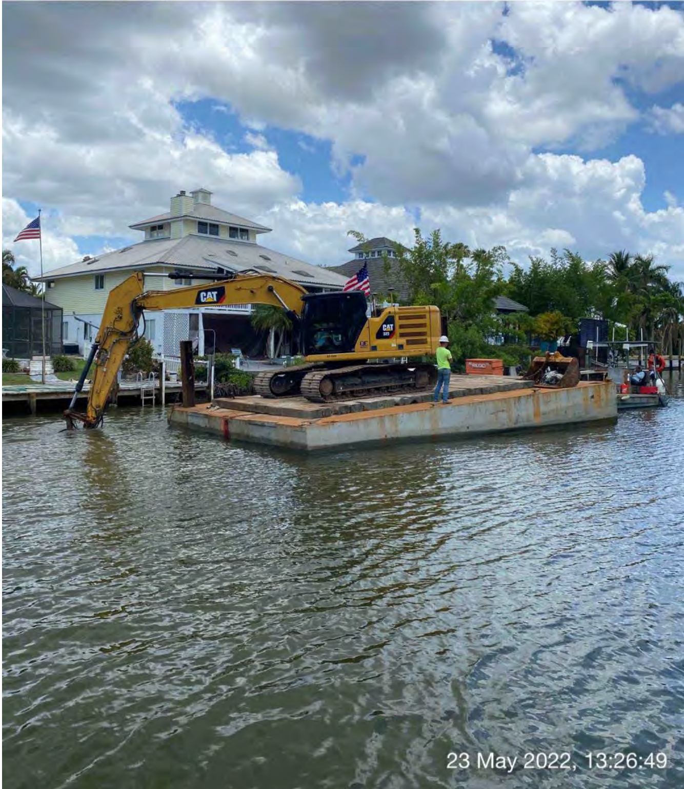
323 excavator checking elevations and grinding rock at station 5+50
