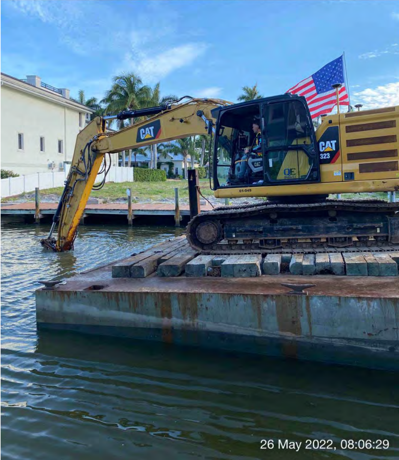
323 excavator grinding rock at station 3+00
