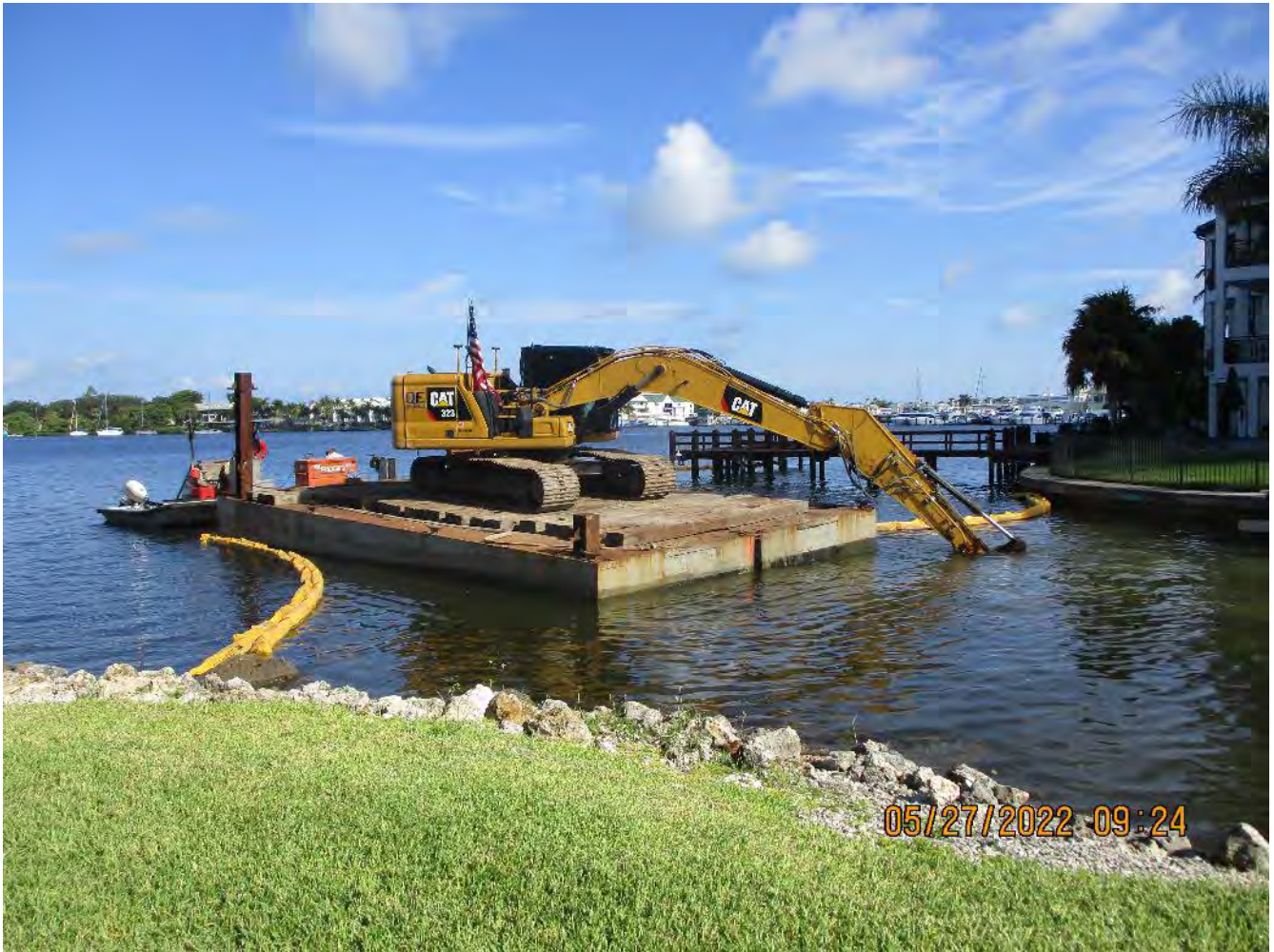
Canal bottom grinding at approx. station 1+00 (Canal X-X)
