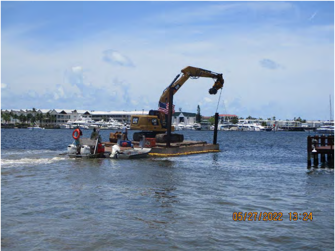
Barge being pushed back to 1300 Curlew Ave. location
