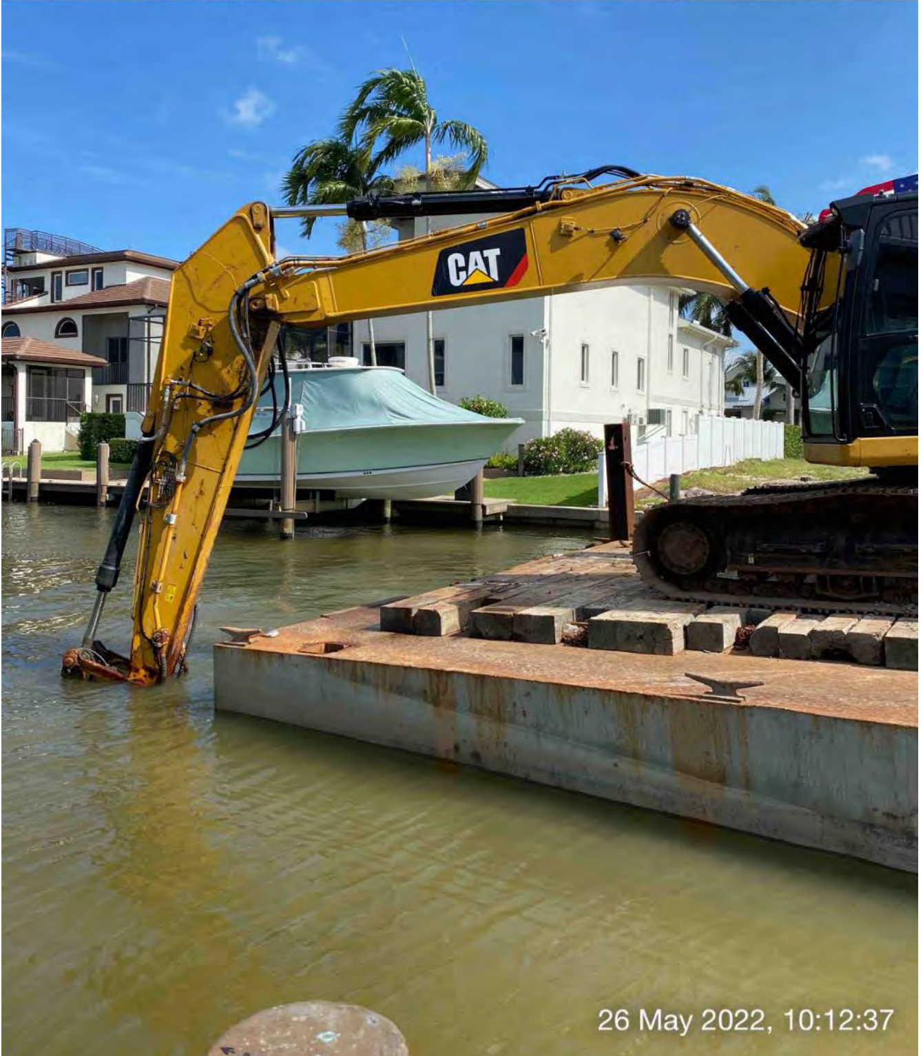
323 excavator grinding rock at station 2+50
