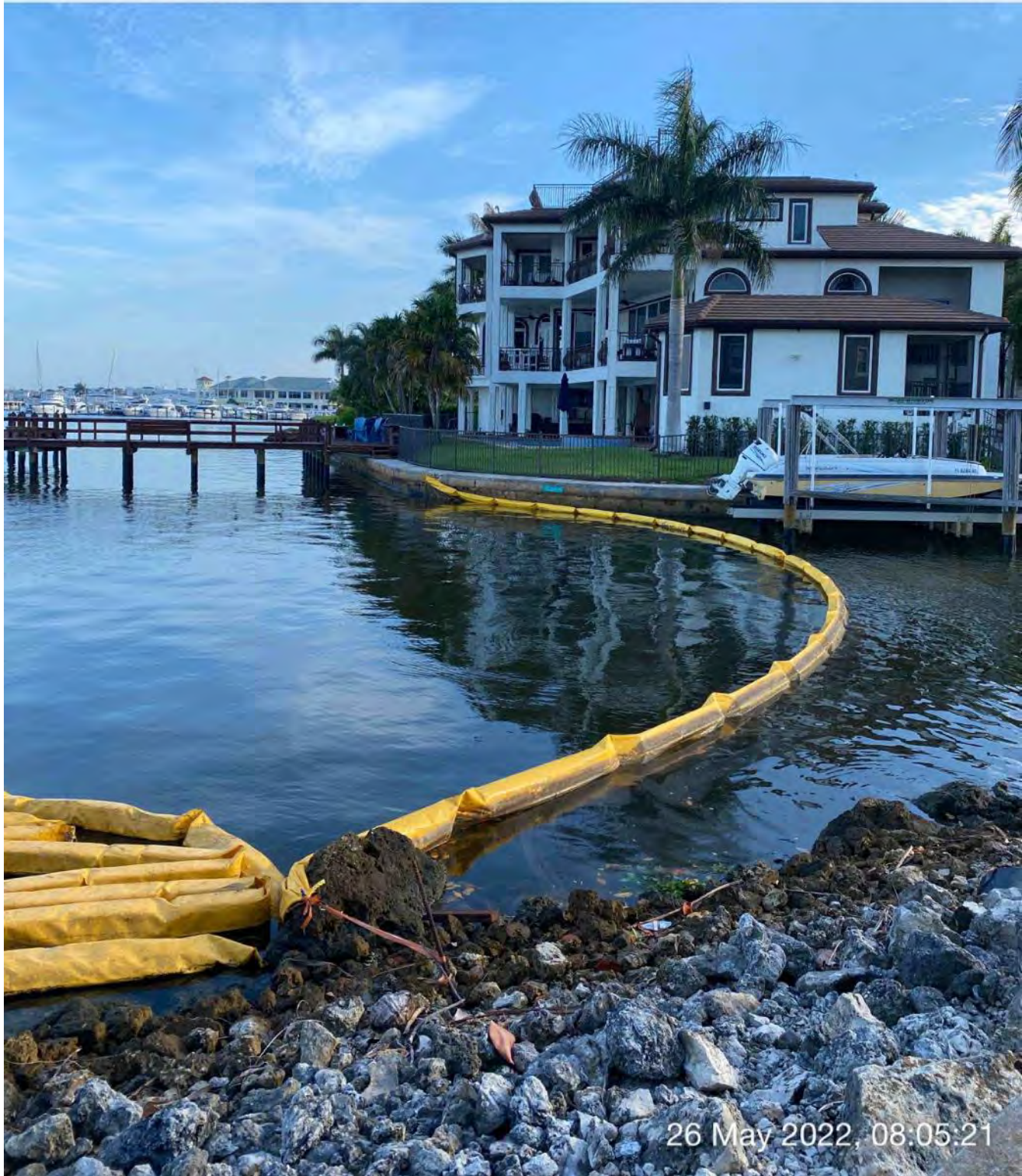
Turbidity curtain installed across mouth of Canal X-X
