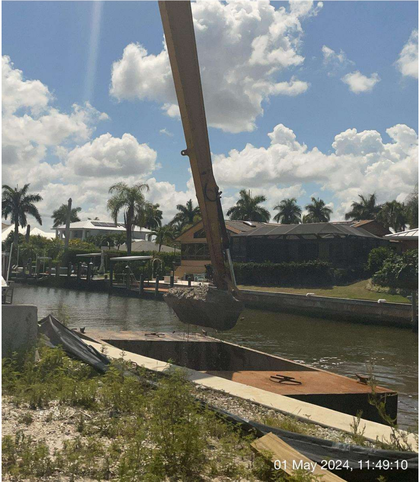
Long reach excavator removing sediment from hopper.
