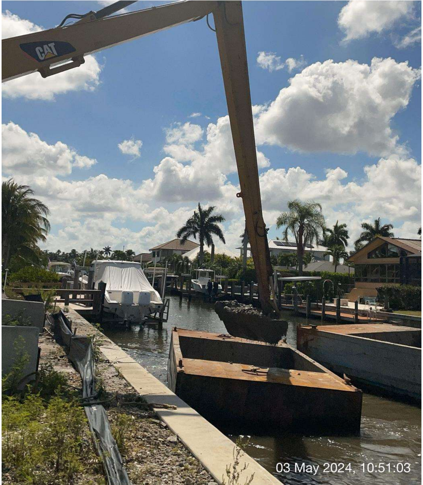
Long reach excavator removing sediment from hopper.
