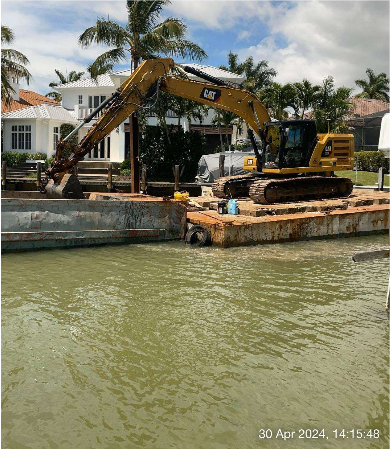
323 excavator removing sediment at station 14+50 in Canal A-A.
