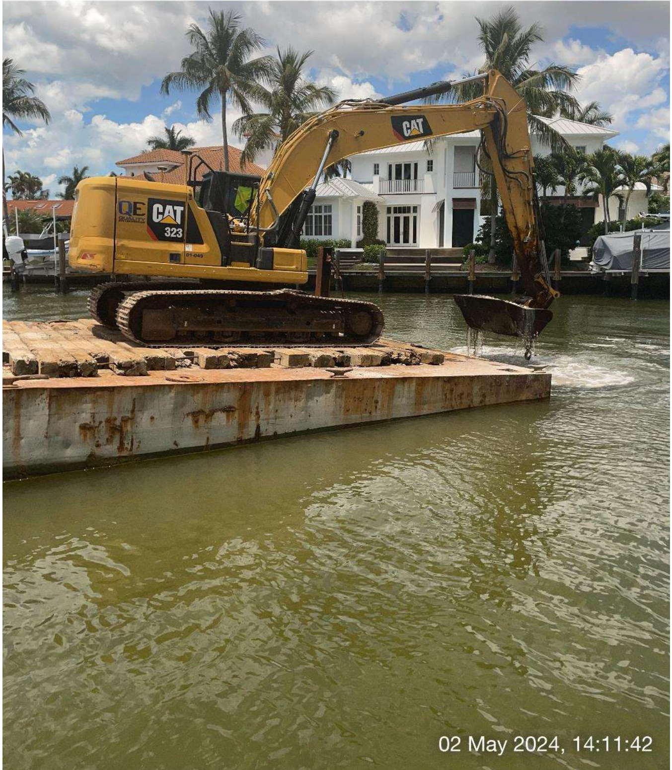
323 excavator removing sediment at station 13+50 in Canal A-A.
