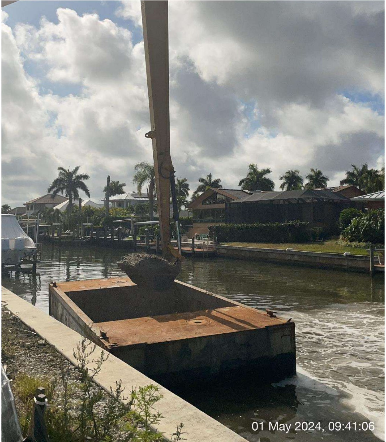
Long reach excavator removing sediment from hopper.
