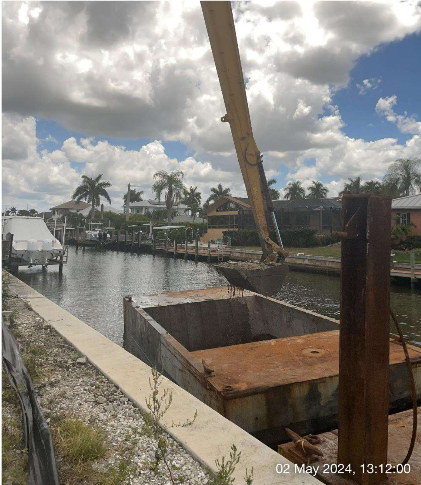
Long reach excavator removing sediment from hopper.
