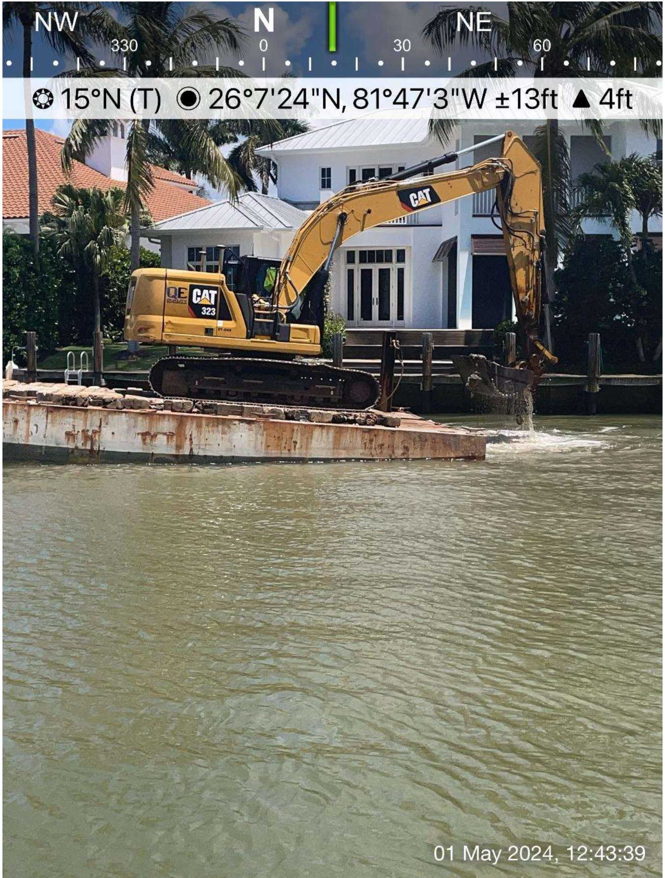
323 excavator removing sediment at station 13+80 in Canal A-A.
