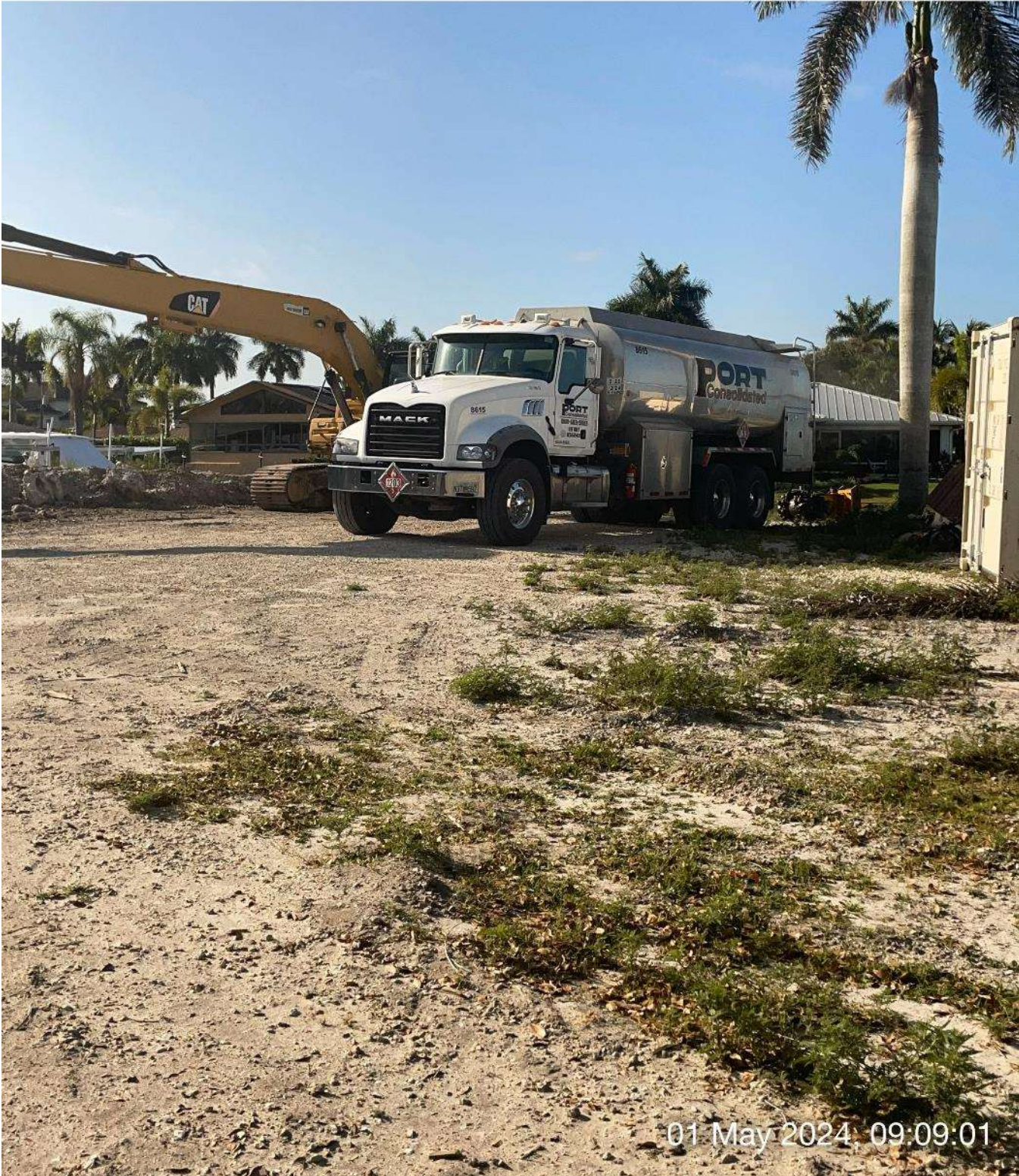
Port Consolidated delivering fuel to staging area.
