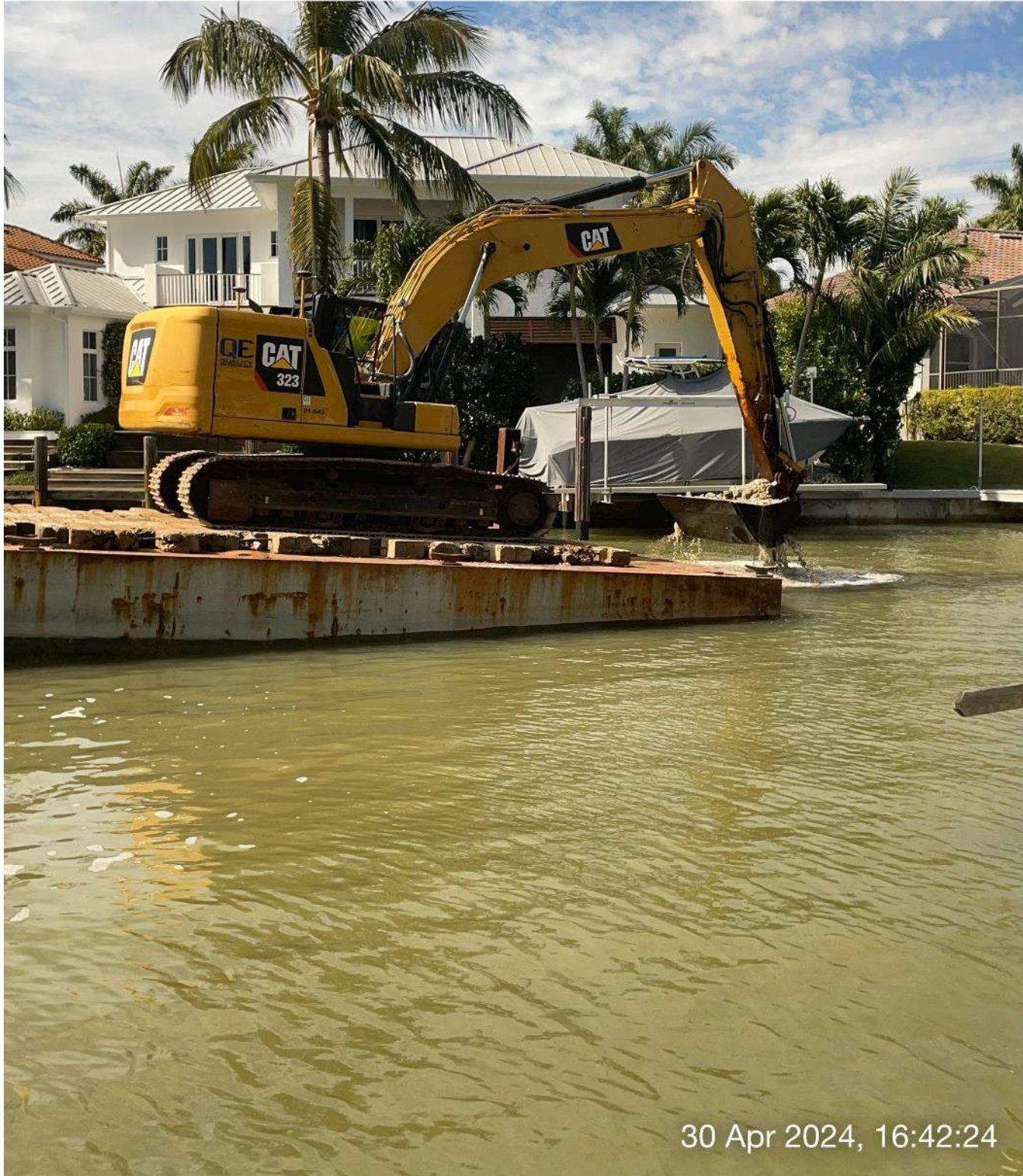
323 excavator removing sediment at station 14+00 in Canal A-A.
