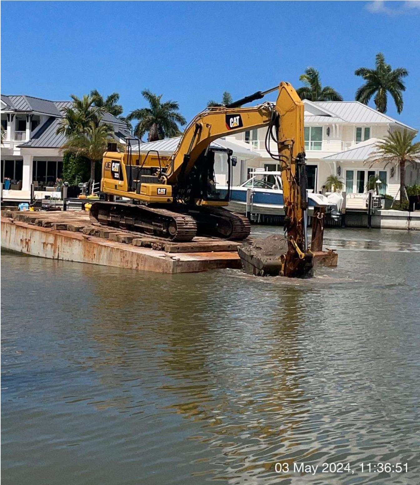
323 excavator removing sediment at station 12+50 in Canal A-A.
