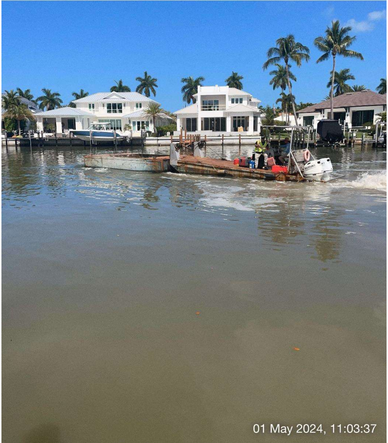
Push boat taking hopper to staging area.
