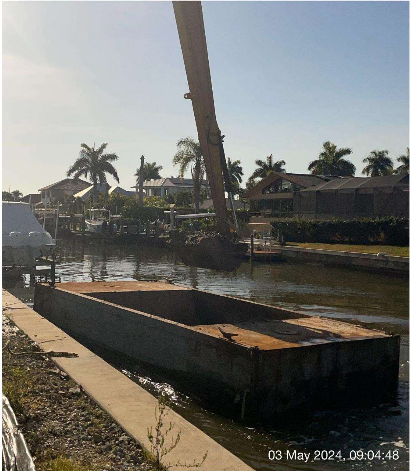
Long reach excavator removing sediment from hopper.
