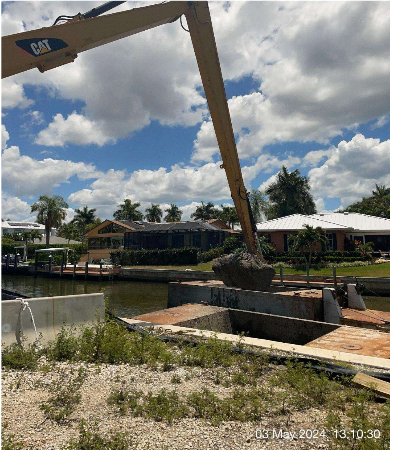
Long reach excavator removing sediment from hopper.
