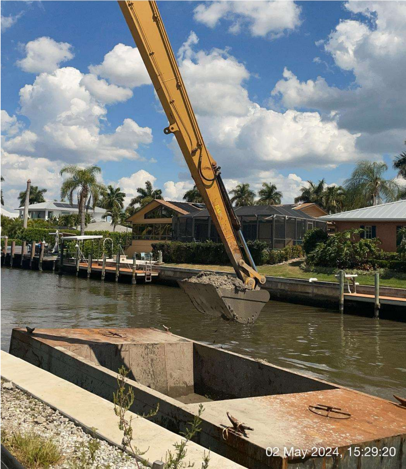
Long reach excavator removing sediment from hopper.
