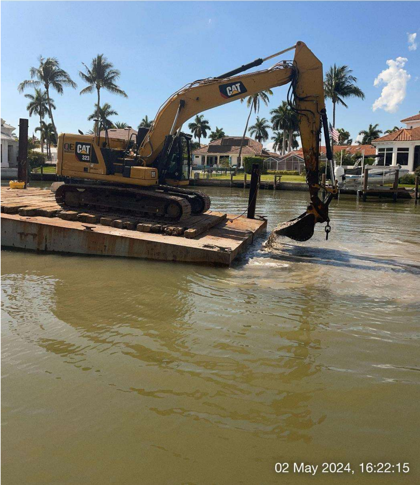
323 excavator removing sediment at station 13+00 in Canal A-A.
