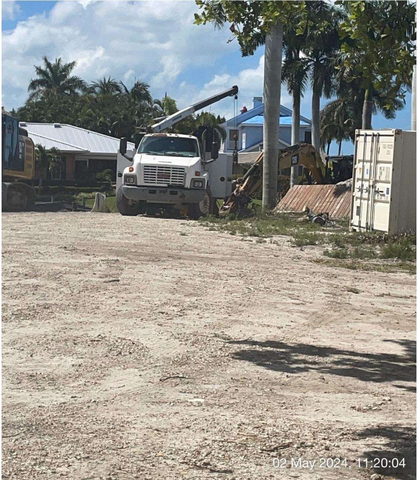
Mechanic working on 323 excavator.
