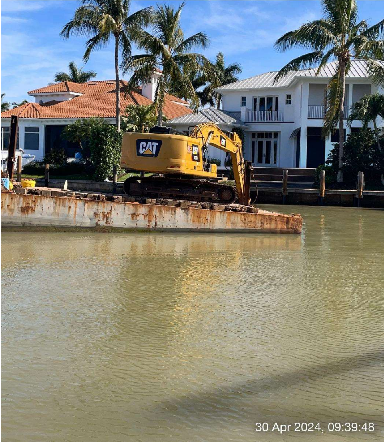
323 excavator grinding rock at station 13+80 in Canal A-A.
