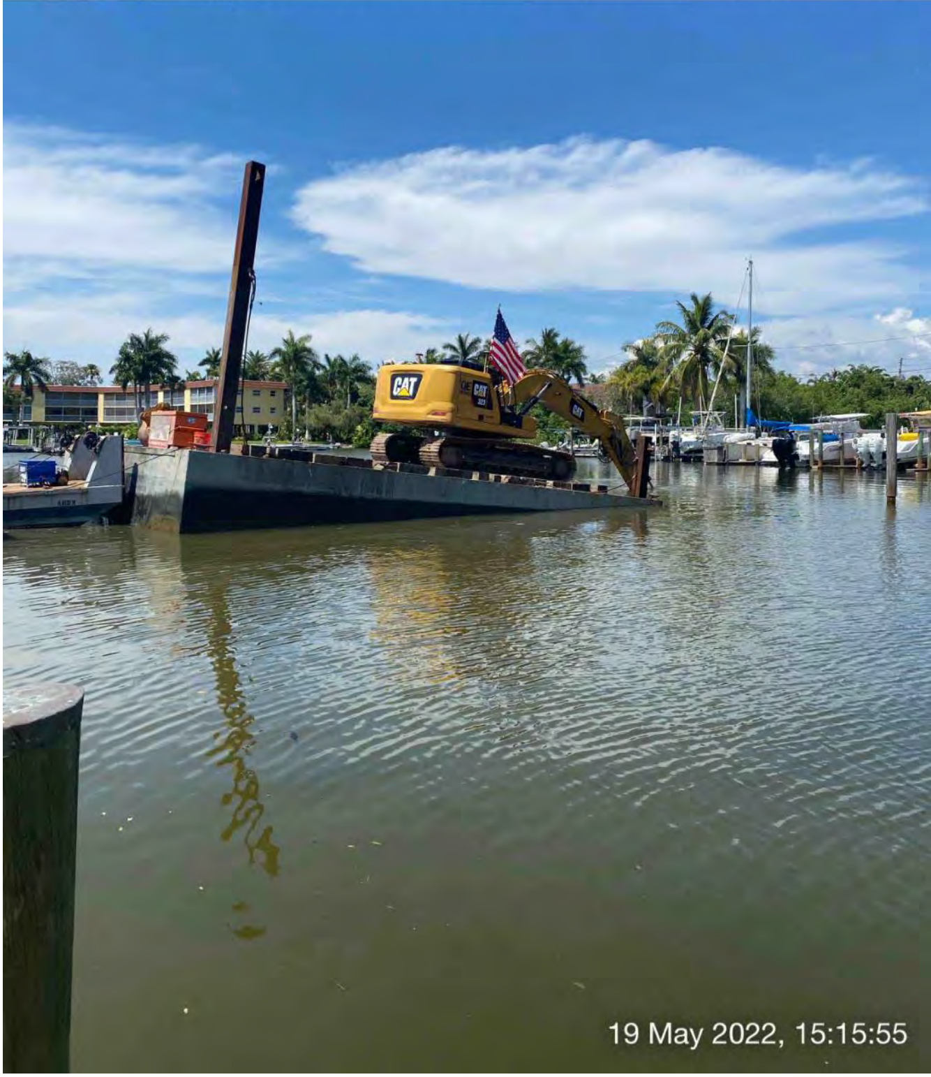
323 excavator checking elevations at station 13+50
