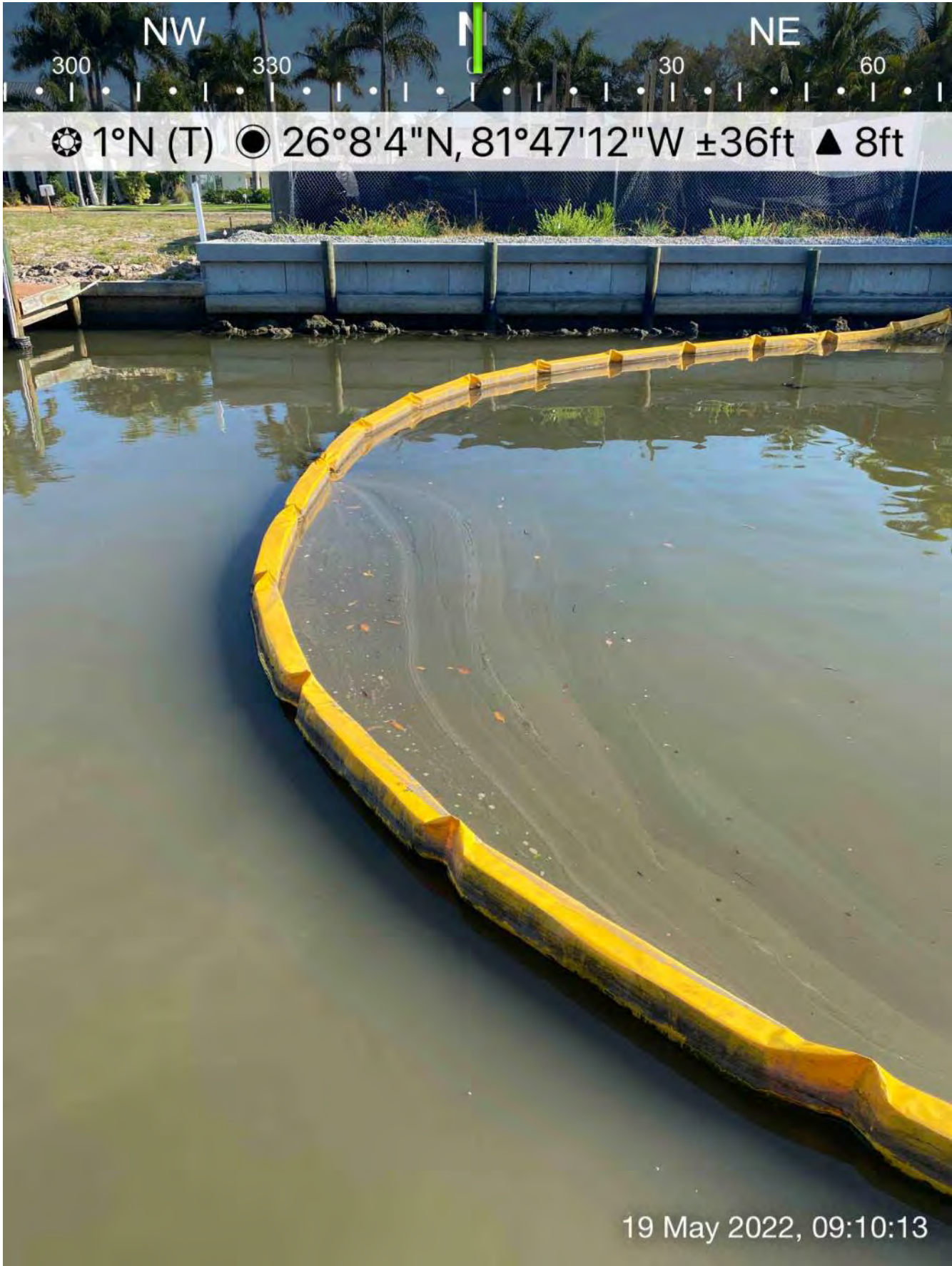
Turbidity curtain installed across Canal X-X at station 3+75
