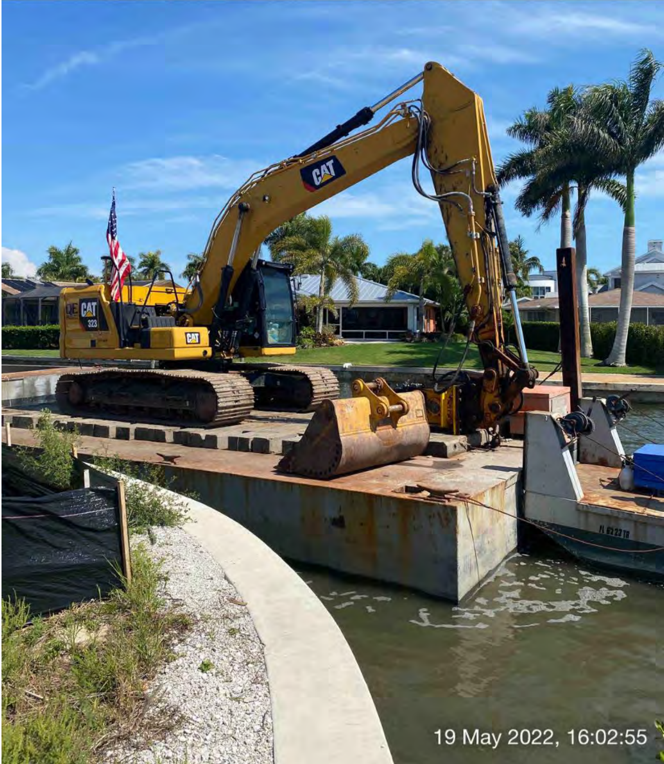
Barge and 323 excavator in Canal CC-CC at station 1+00.
