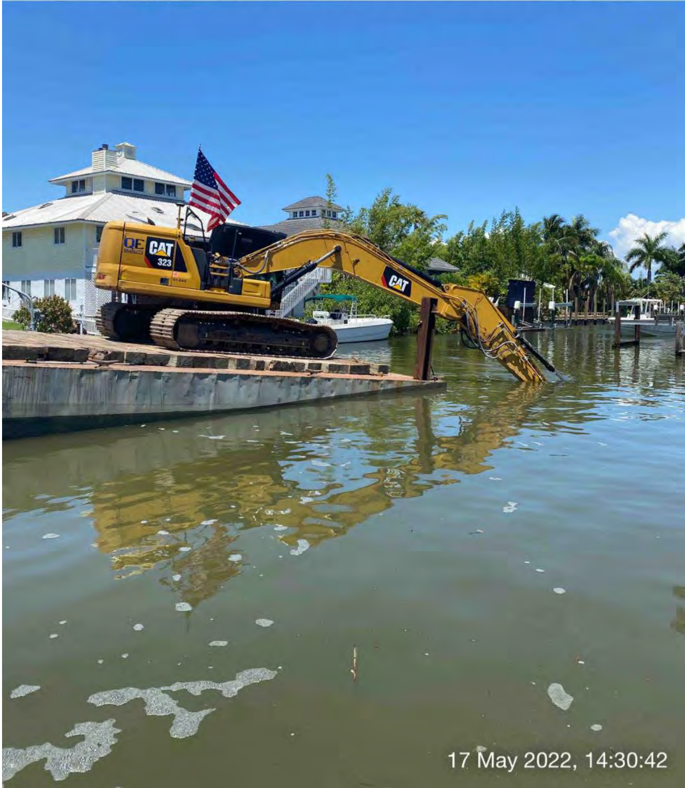
323 excavator grinding rock at station 5+50 in Canal X-X
