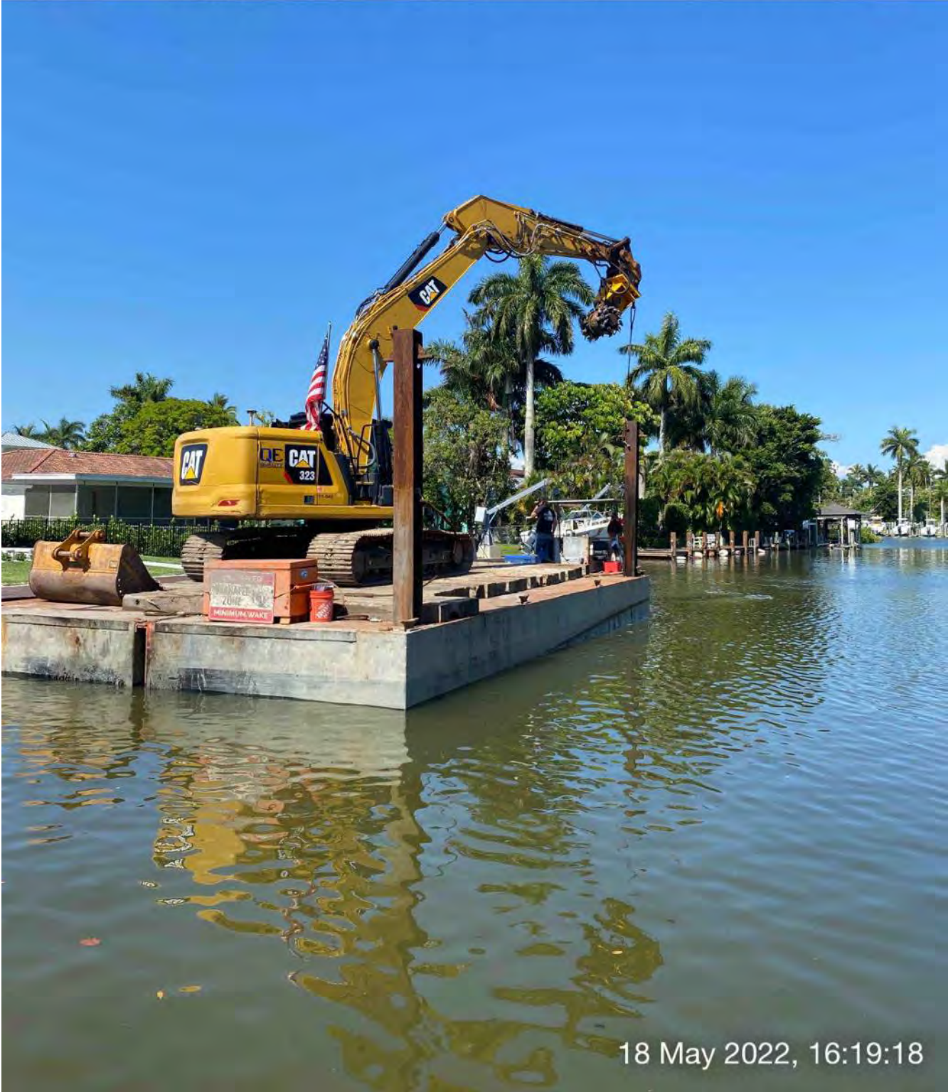
323 excavator lifting spud to allow push boat to transport barge from Canal X-X to Canal CC-CC
