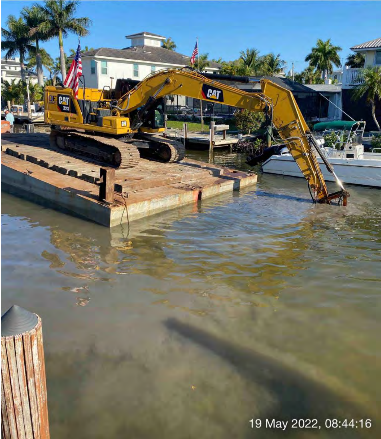
323 excavator grinding rock at station 6+00
