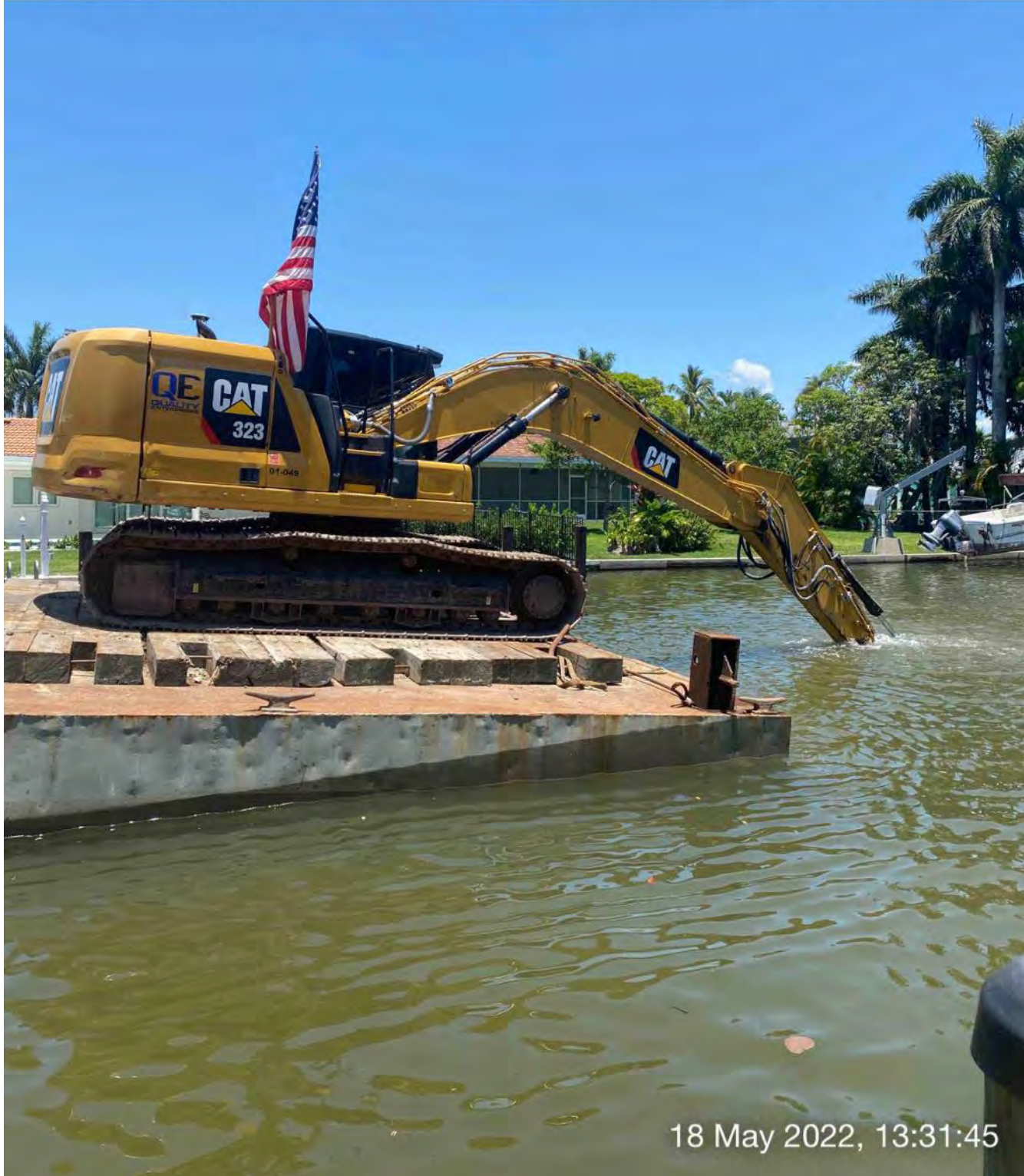
323 excavator grinding rock at station 9+00
