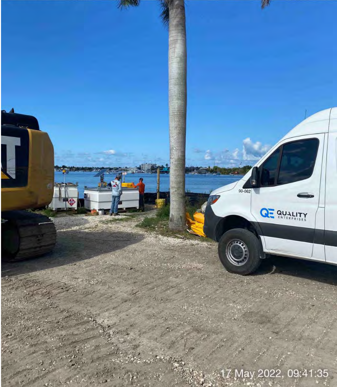
Technicians inspecting Trimble base station GPS connection at 1300 Curlew Avenue
