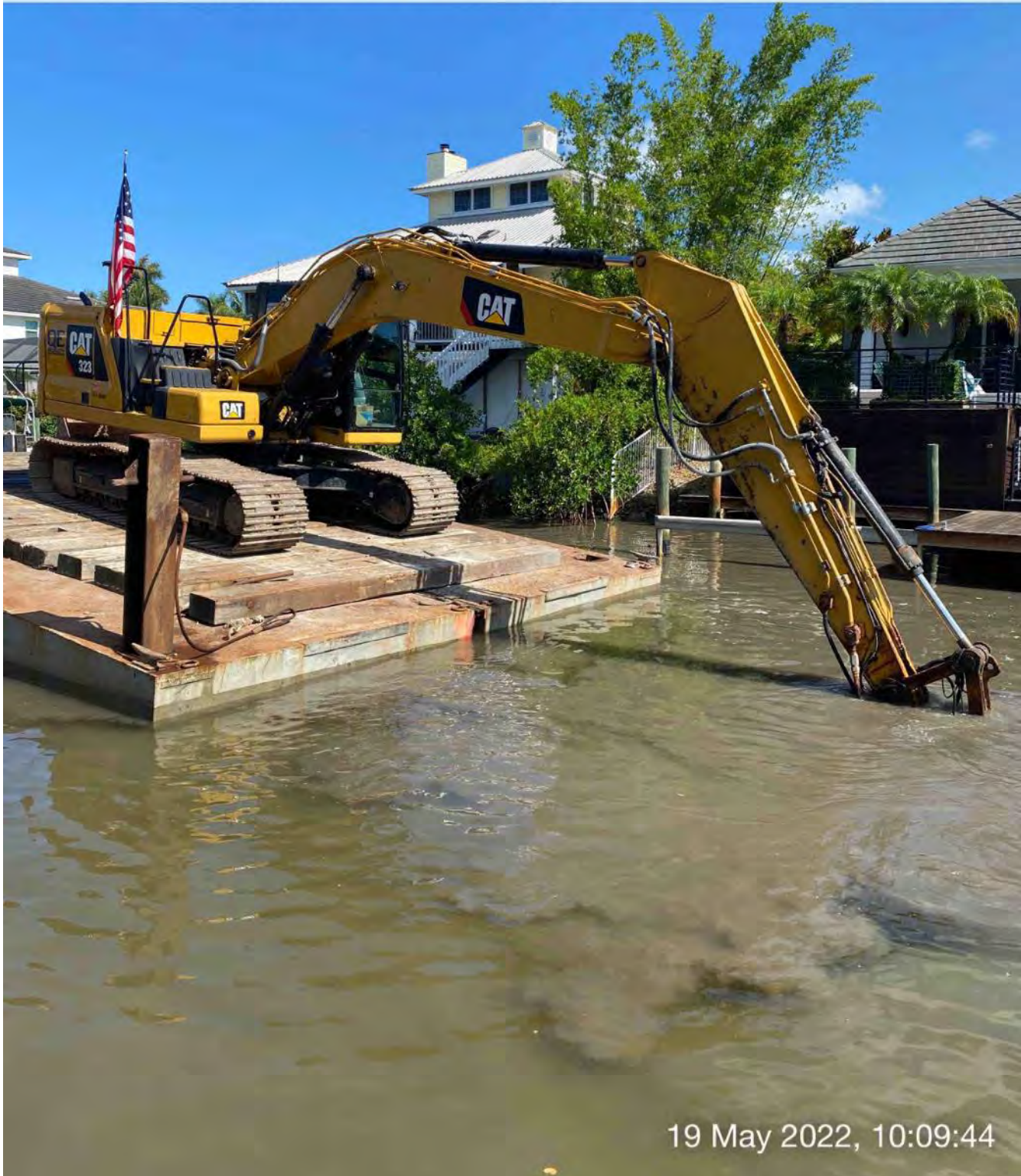
323 excavator grinding rock at station 7+00
