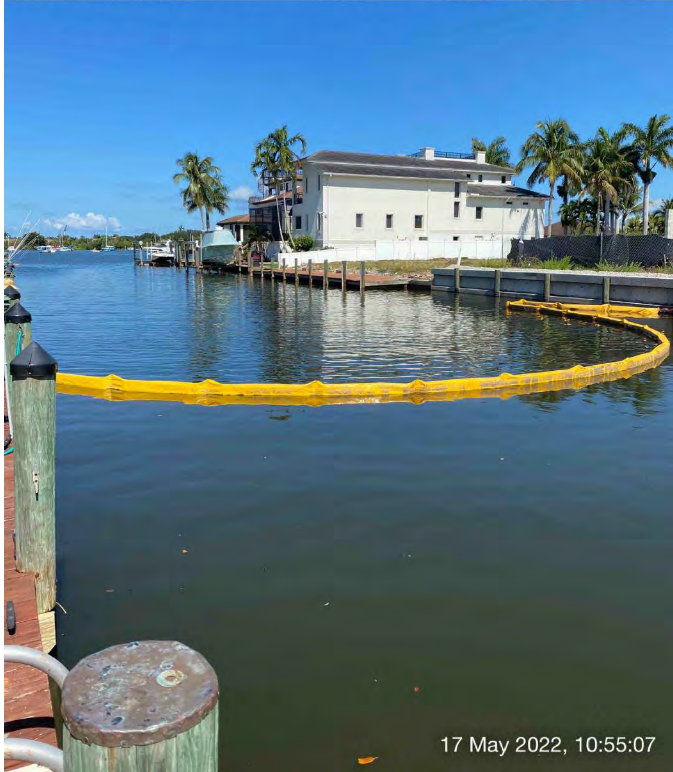
Turbidity curtain install across Canal X-X at station 3+75
