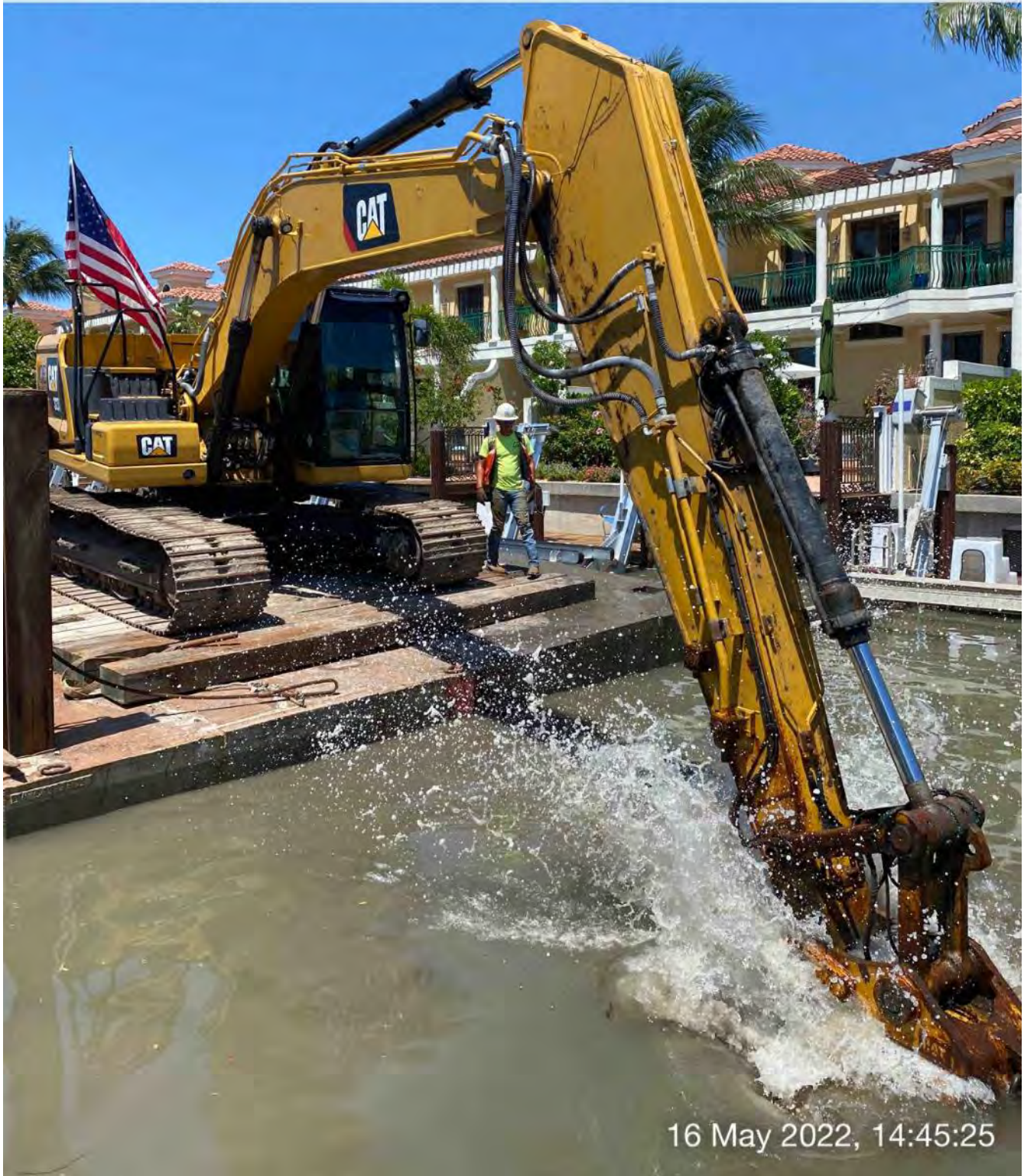
323 excavator removing material at station 3+50 and transferring to hopper
