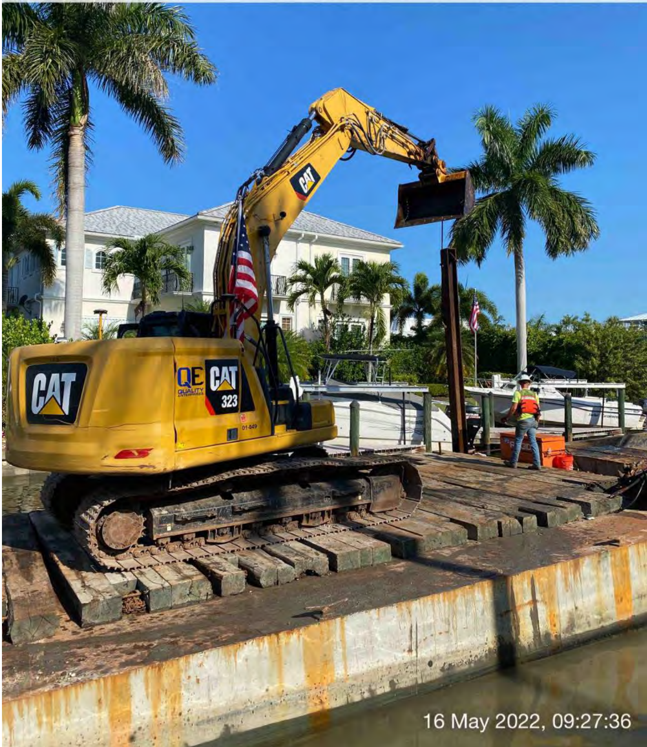
323 excavator lifting spud to allow push boat to mobilizer barge at station 4+00
