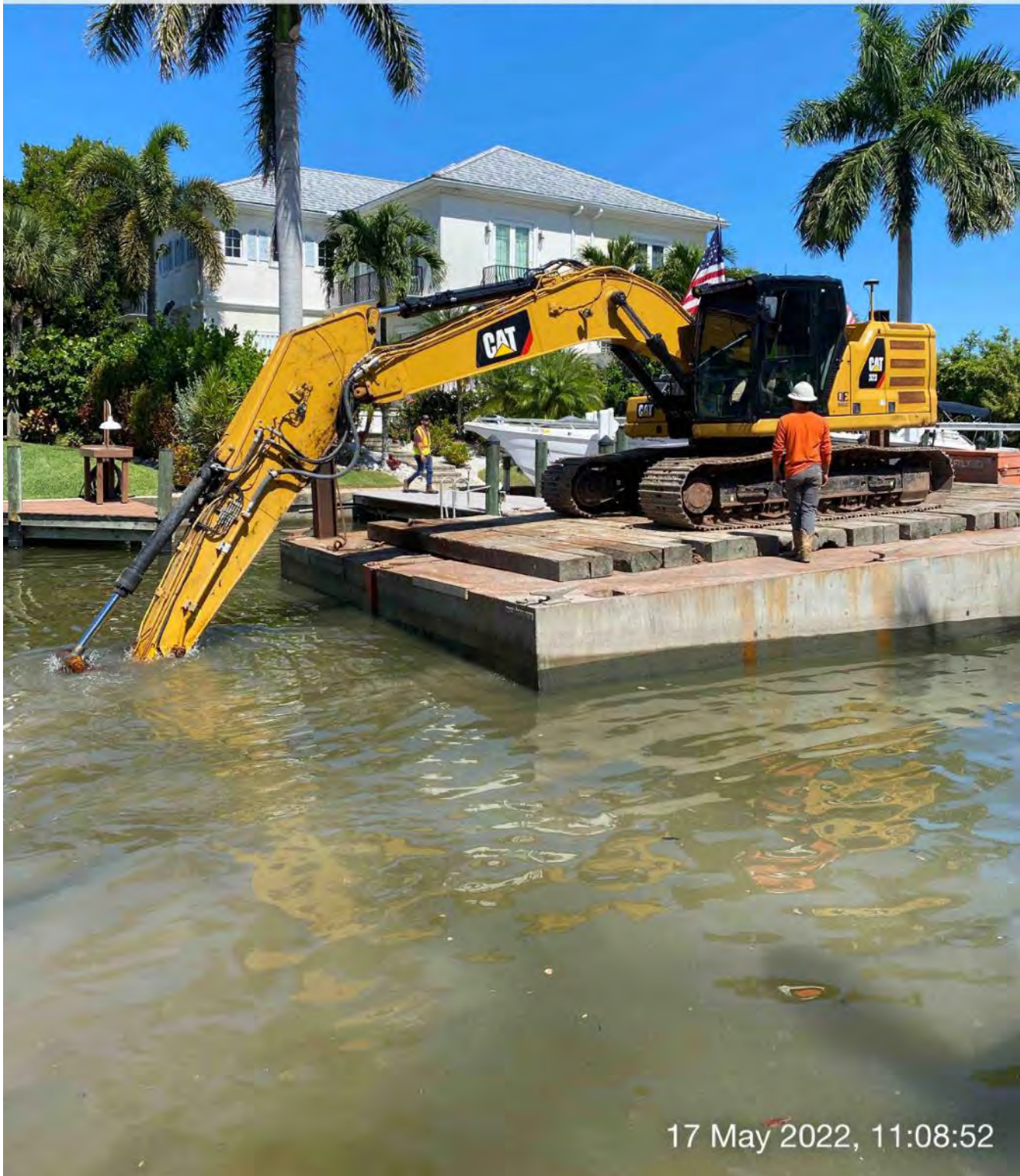
323 excavator grinding rock at station 4+00
