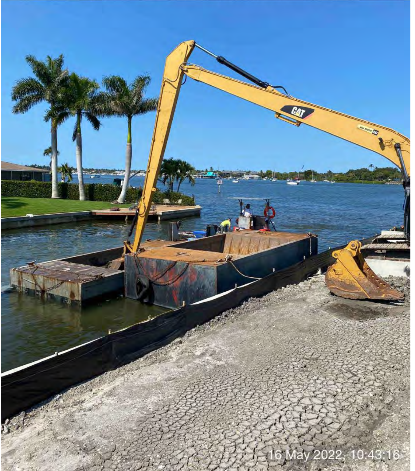
Push boat dropping off a full hopper of removed material in Canal CC-CC station 1+50
