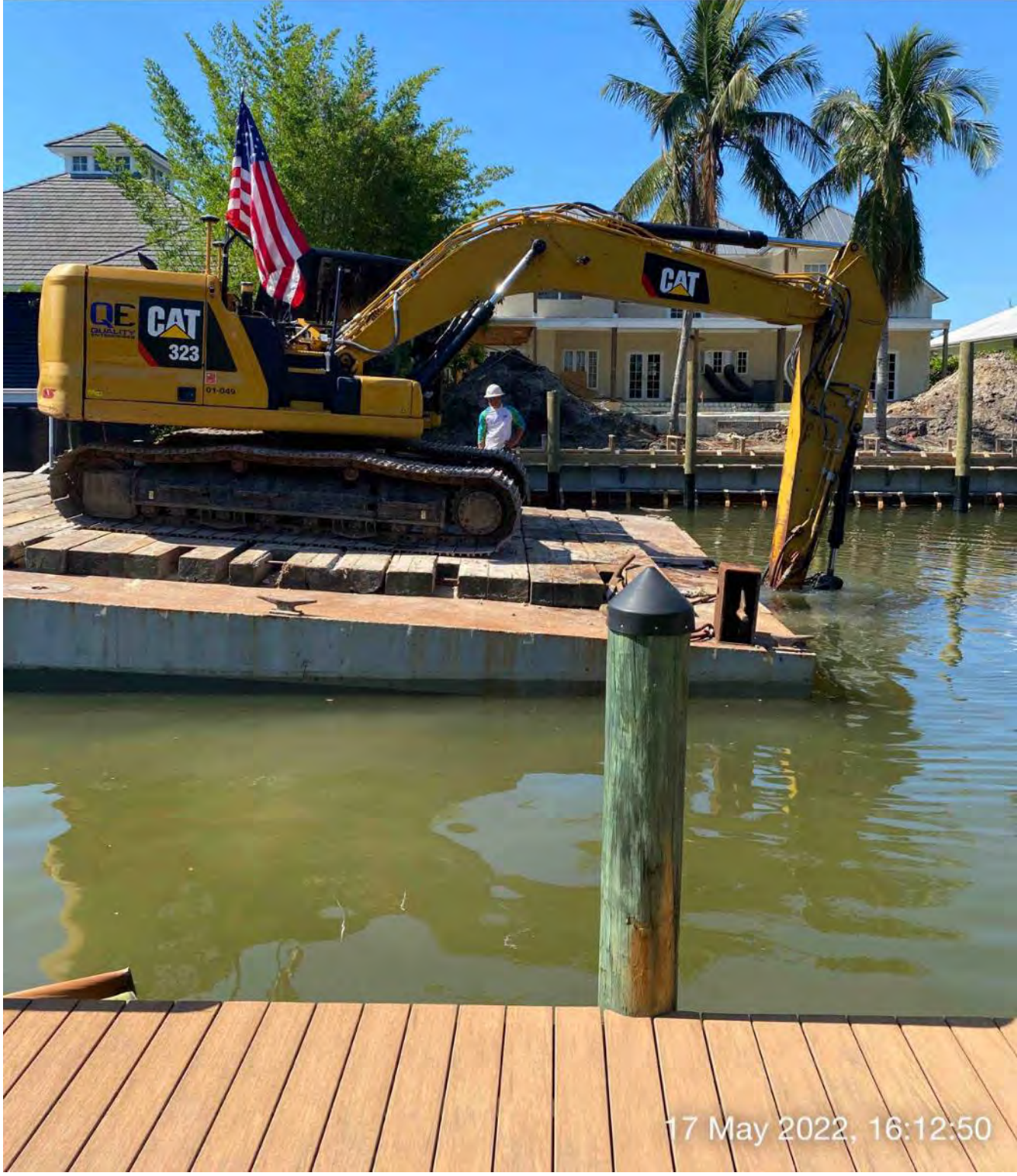
323 excavator grinding rock at station 7+50 in Canal X-X
