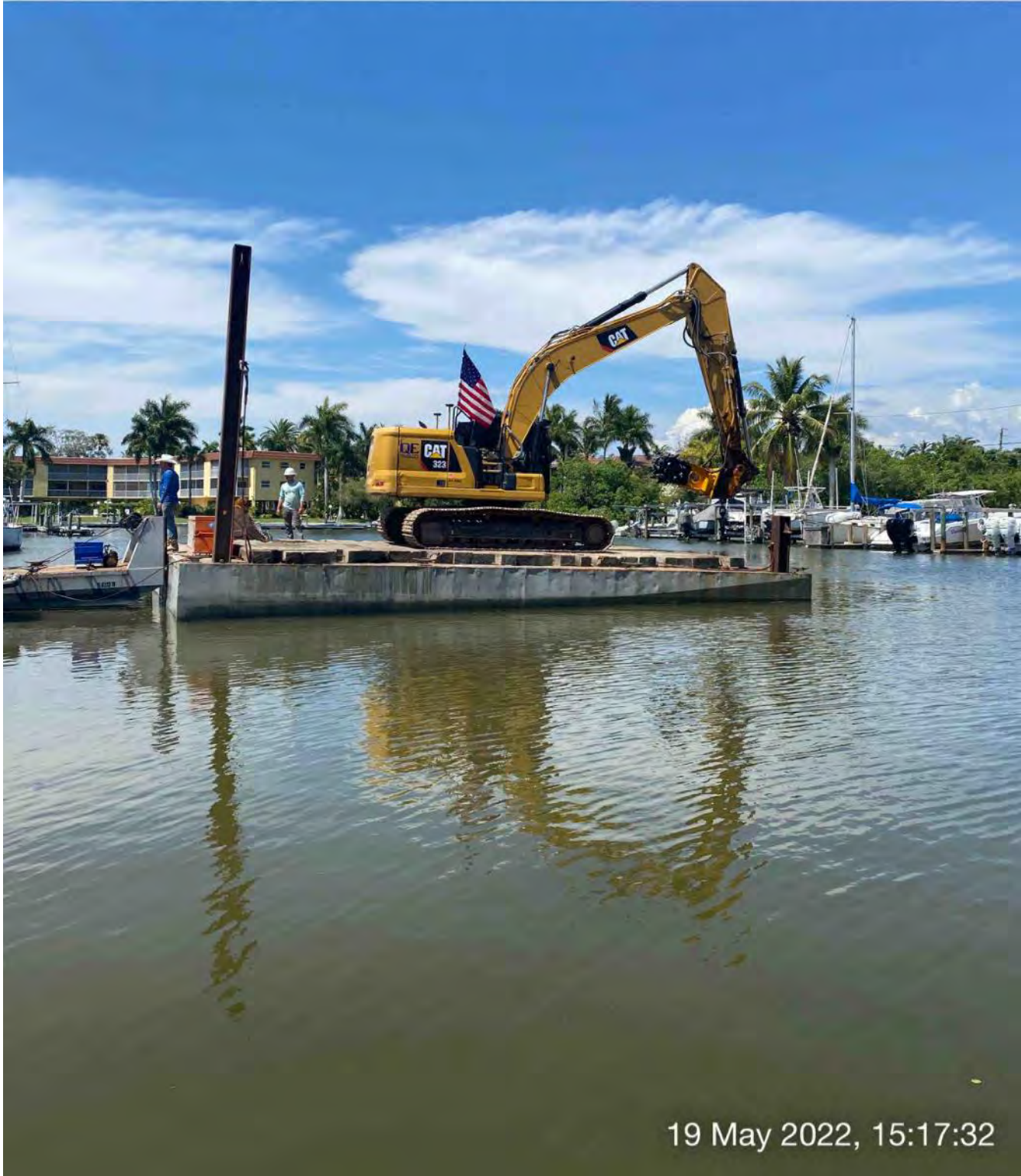
323 excavator lifting spud to allow push boat to mobilize barge at station 14+00
