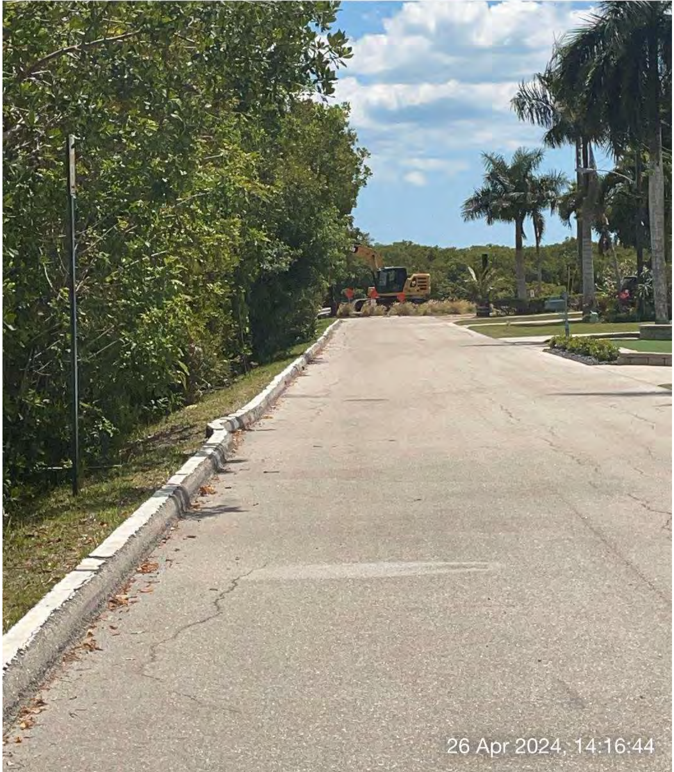
Equipment staged at station 4+00 in Canal Main B1.
