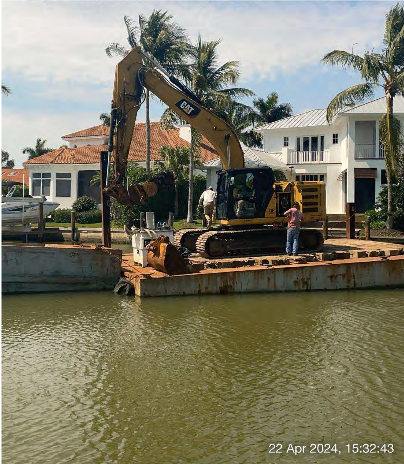
Contractor refueling 323 excavator.
