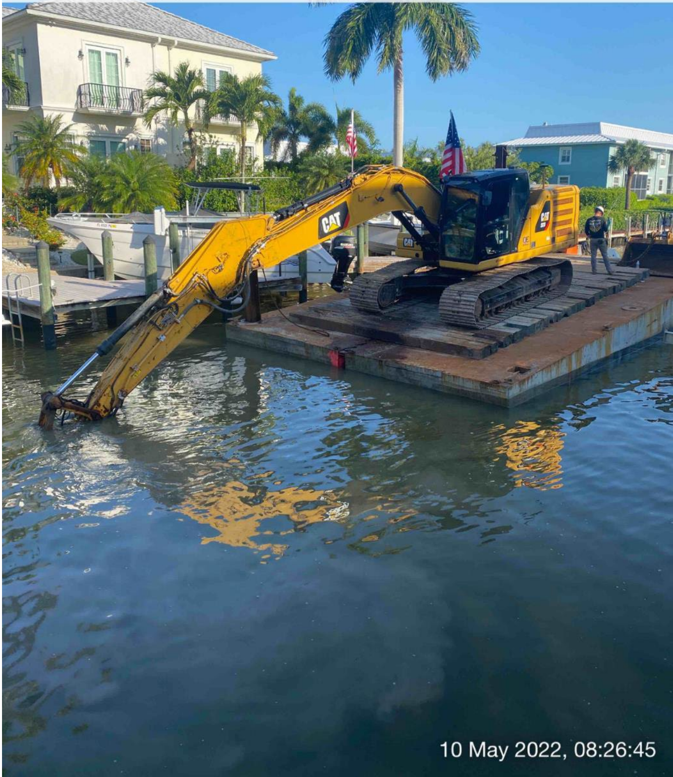
323 excavator grinding rock at station 3+75
