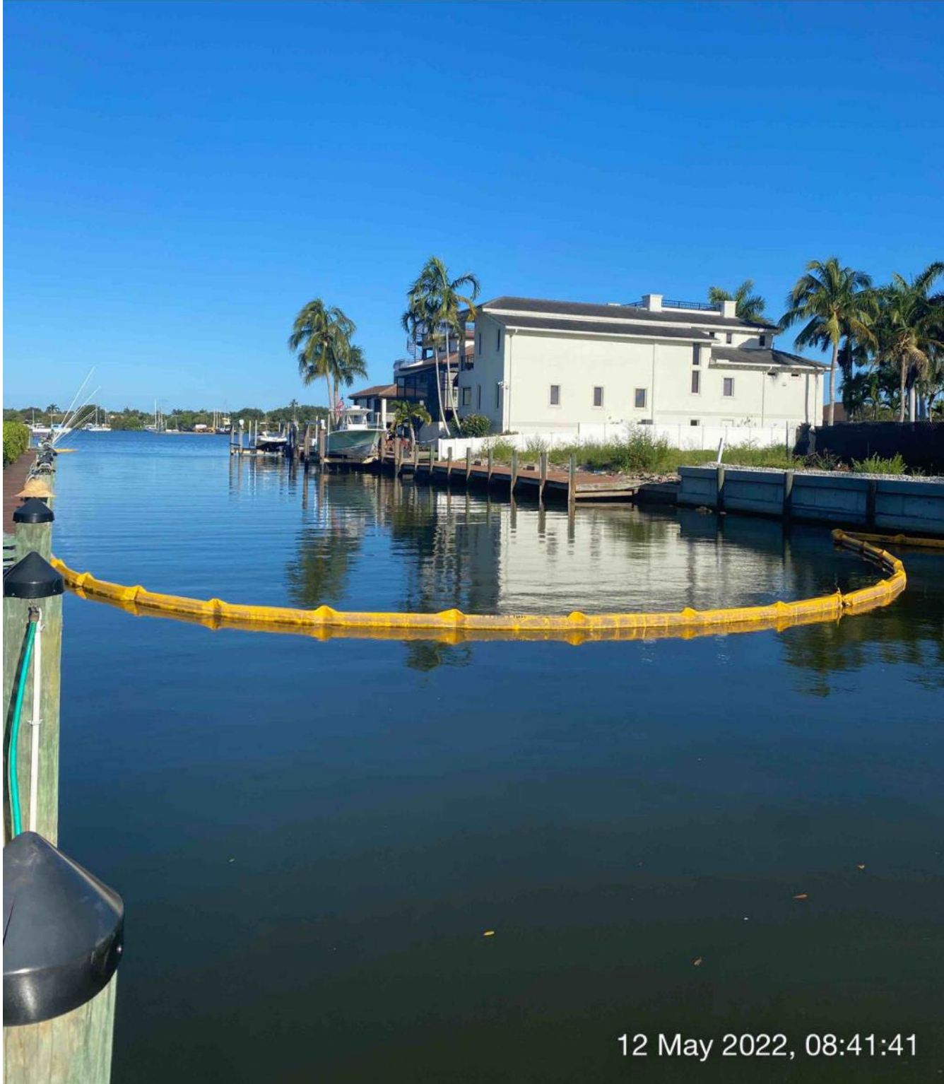
Turbidity curtain installed across Canal X-X at station 3+75
