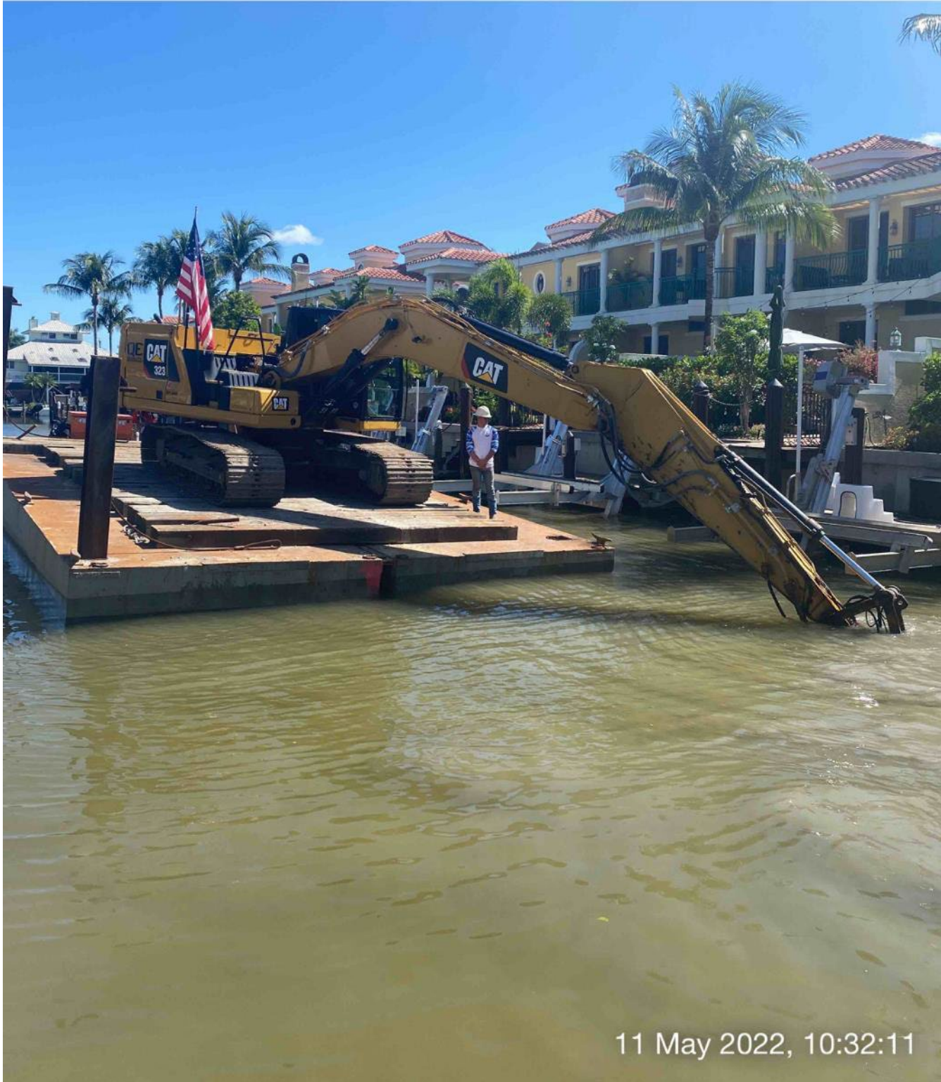
323 excavator grinding rock at station 3+50
