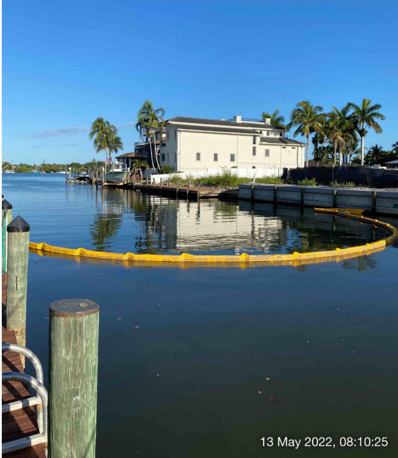
Turbidity curtain installed across Canal X-X a station 3+75
