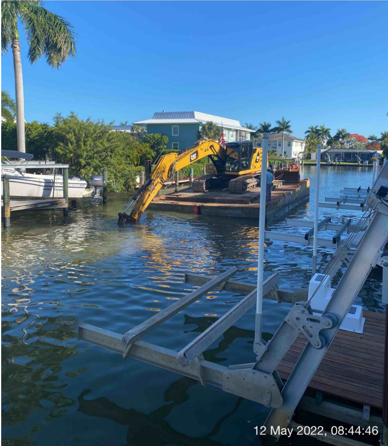
323 excavator grinding rock at station 3+00
