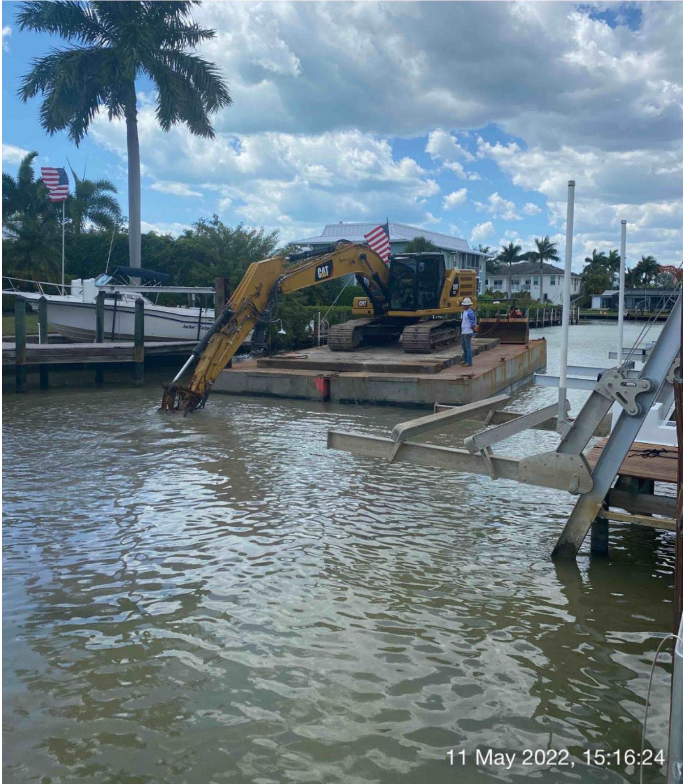
323 excavator grinding rock at station 3+25
