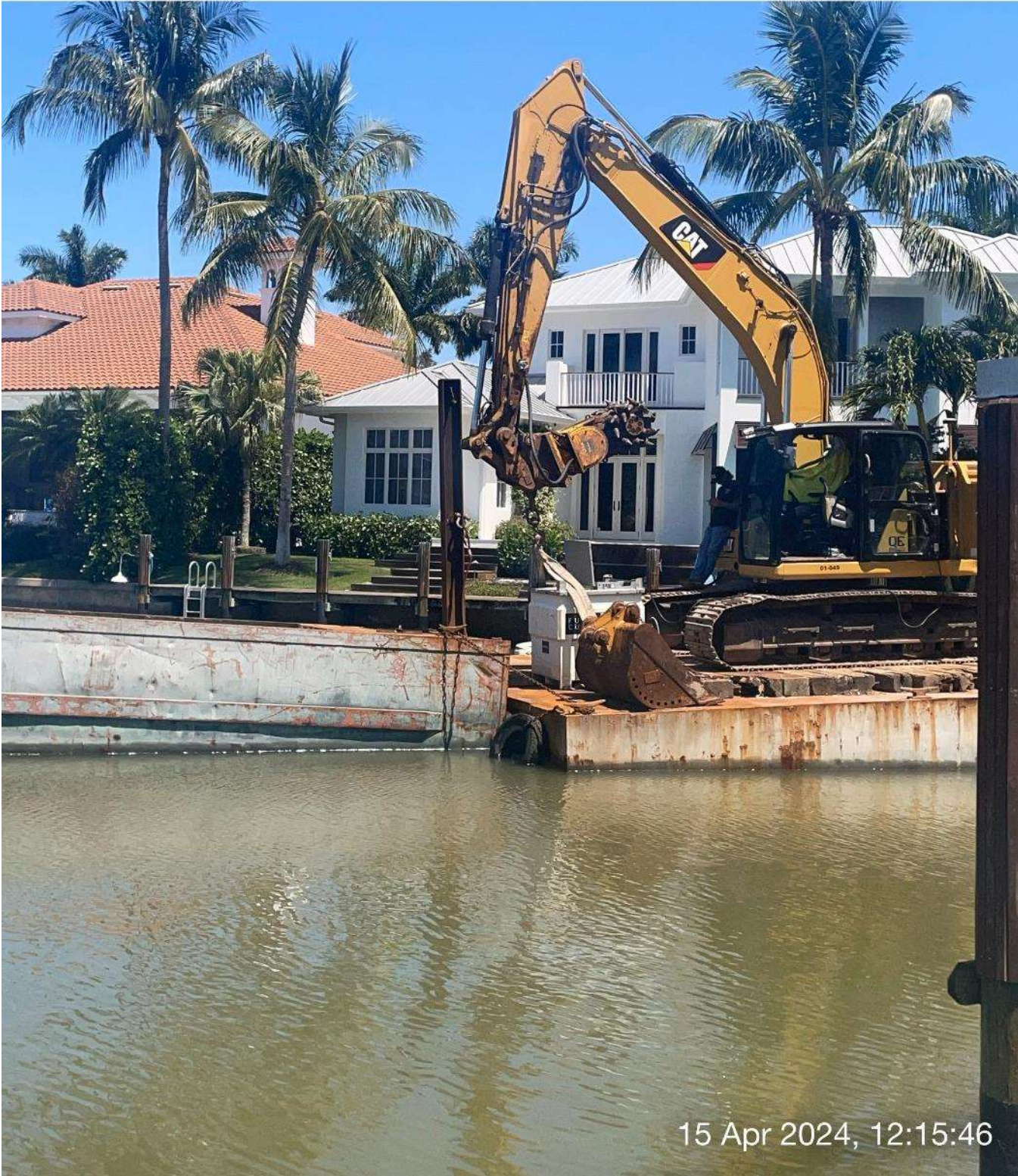
Contractor refueling 323 excavator.
