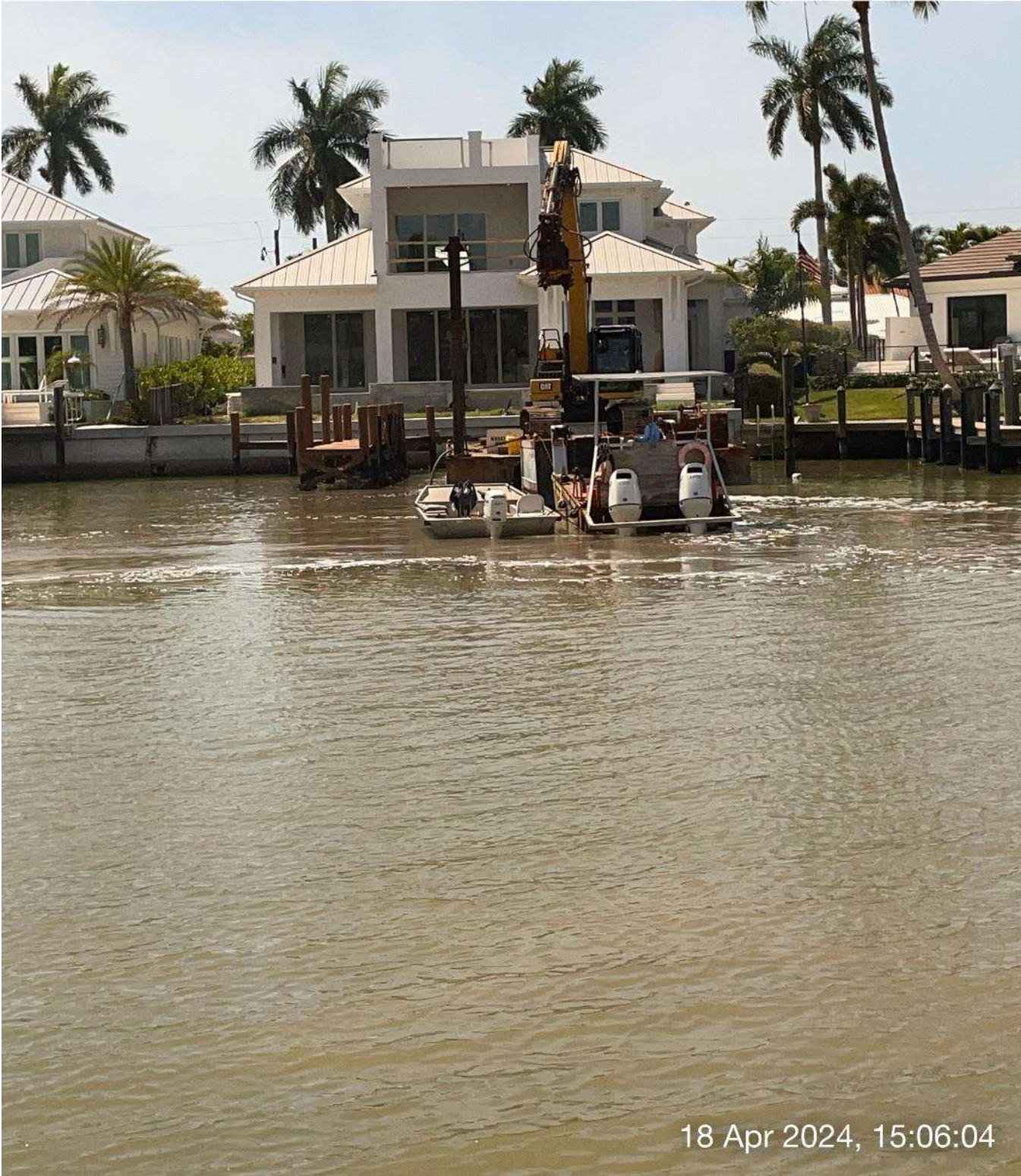
Equipment staged at station 12+00 in Canal A-A.
