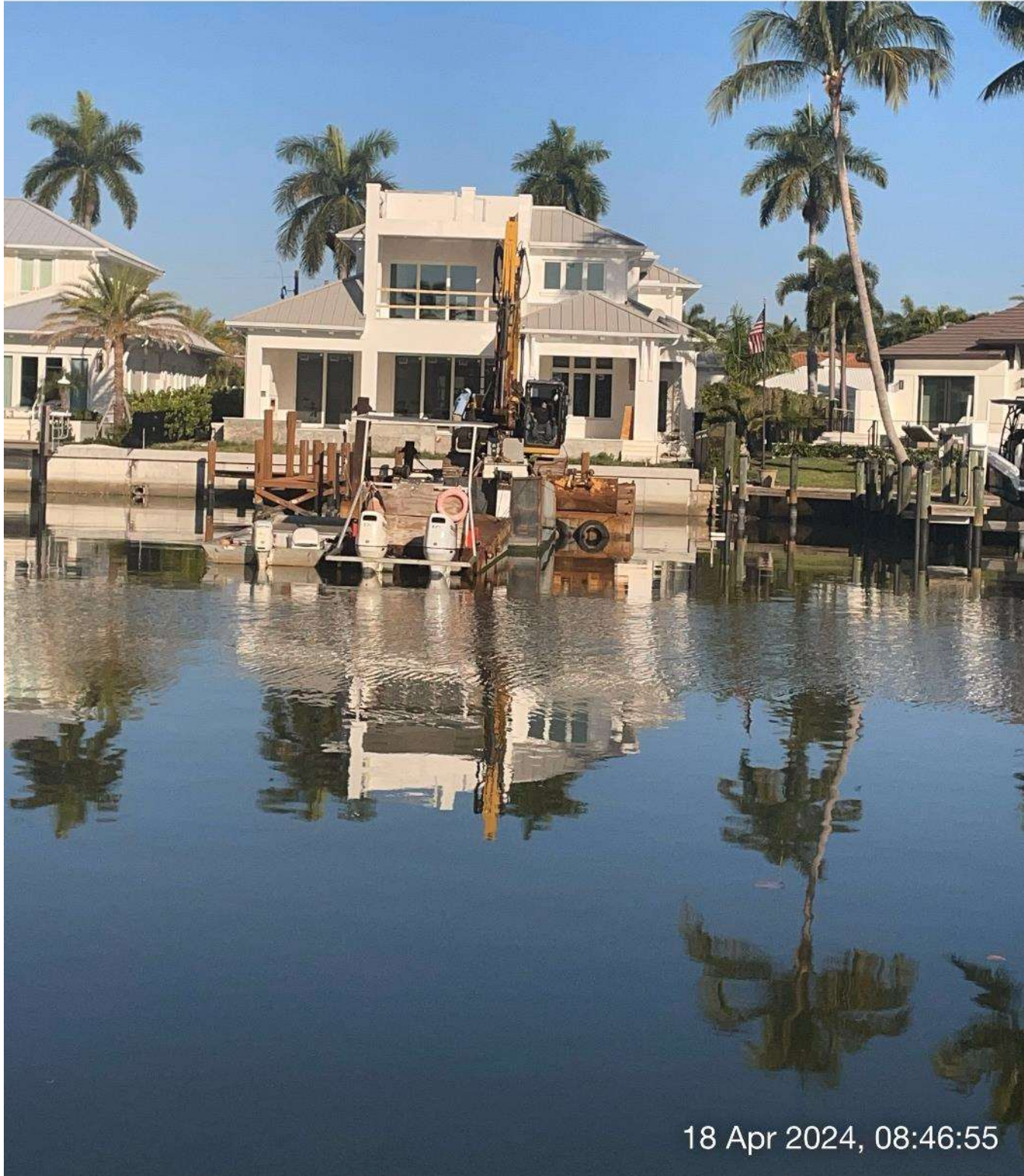
Contractor refueling 323 excavator.
