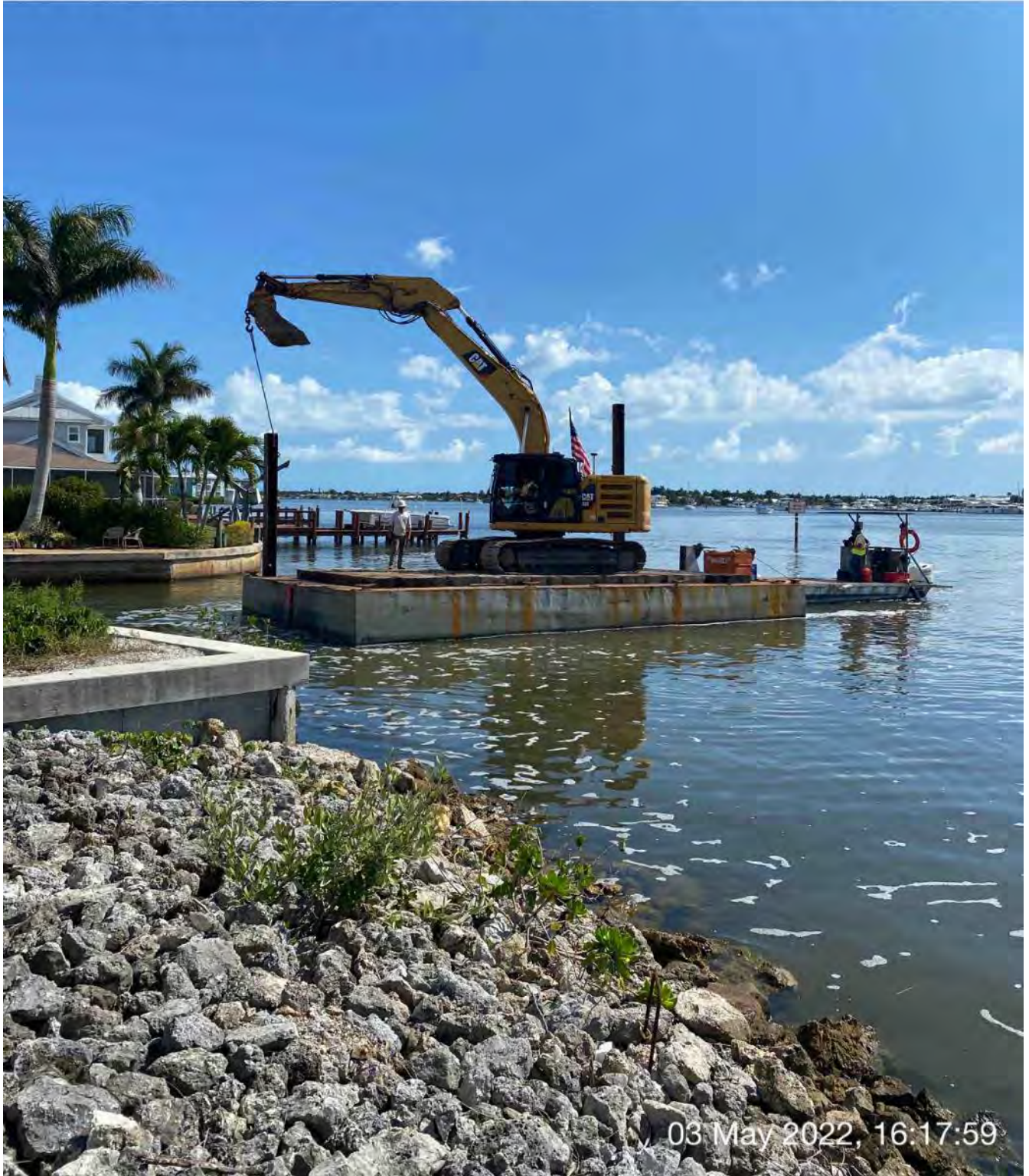
323 excavator lifting spud to allow push boat to mobilize barge at station 0+50 in Canal CC-CC.
