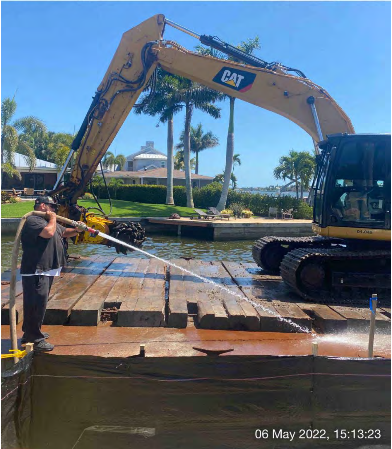
Contractor using water hose to clean barge and 323 excavator
