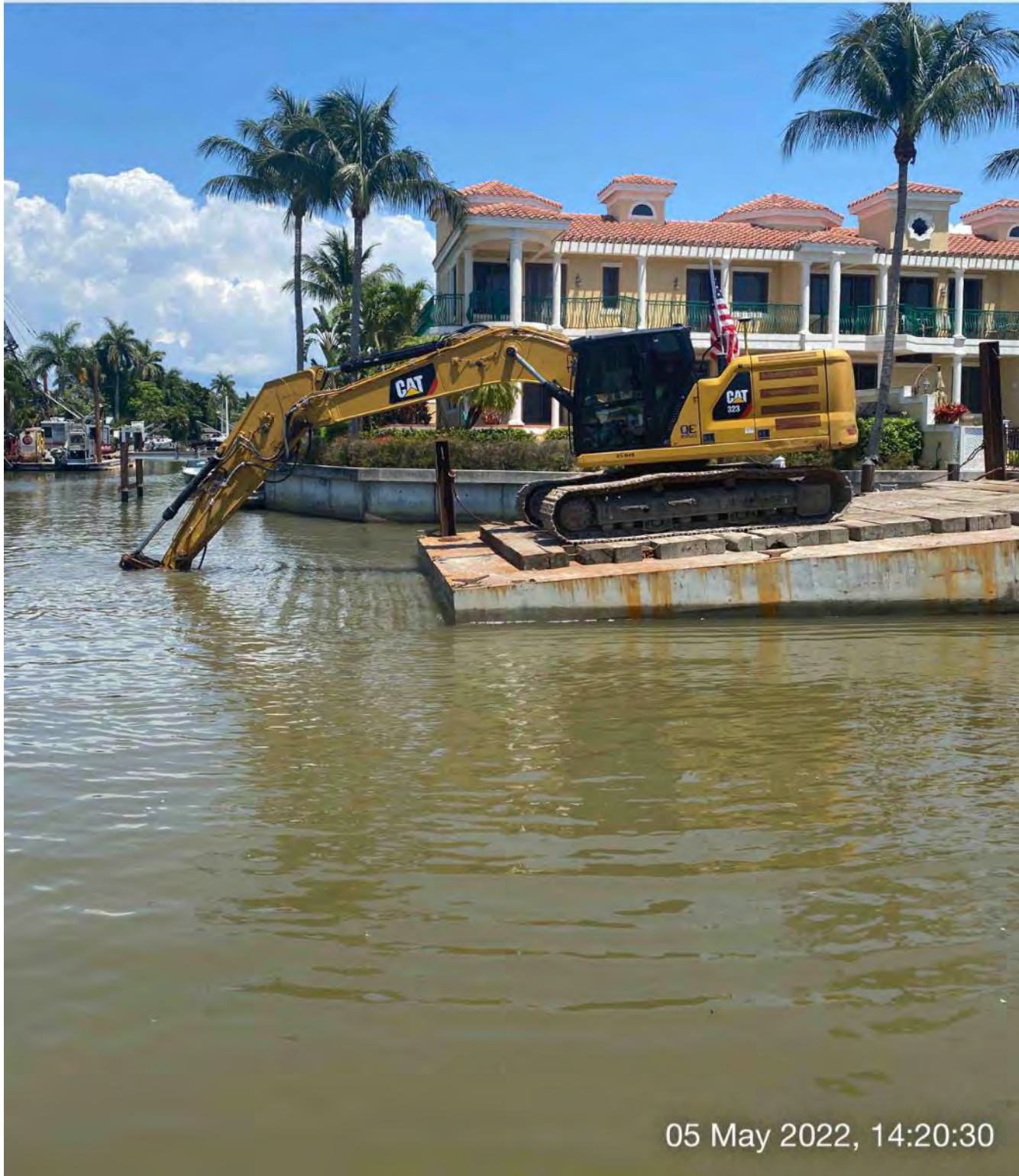
323 excavator grinding rock at station 0+25
