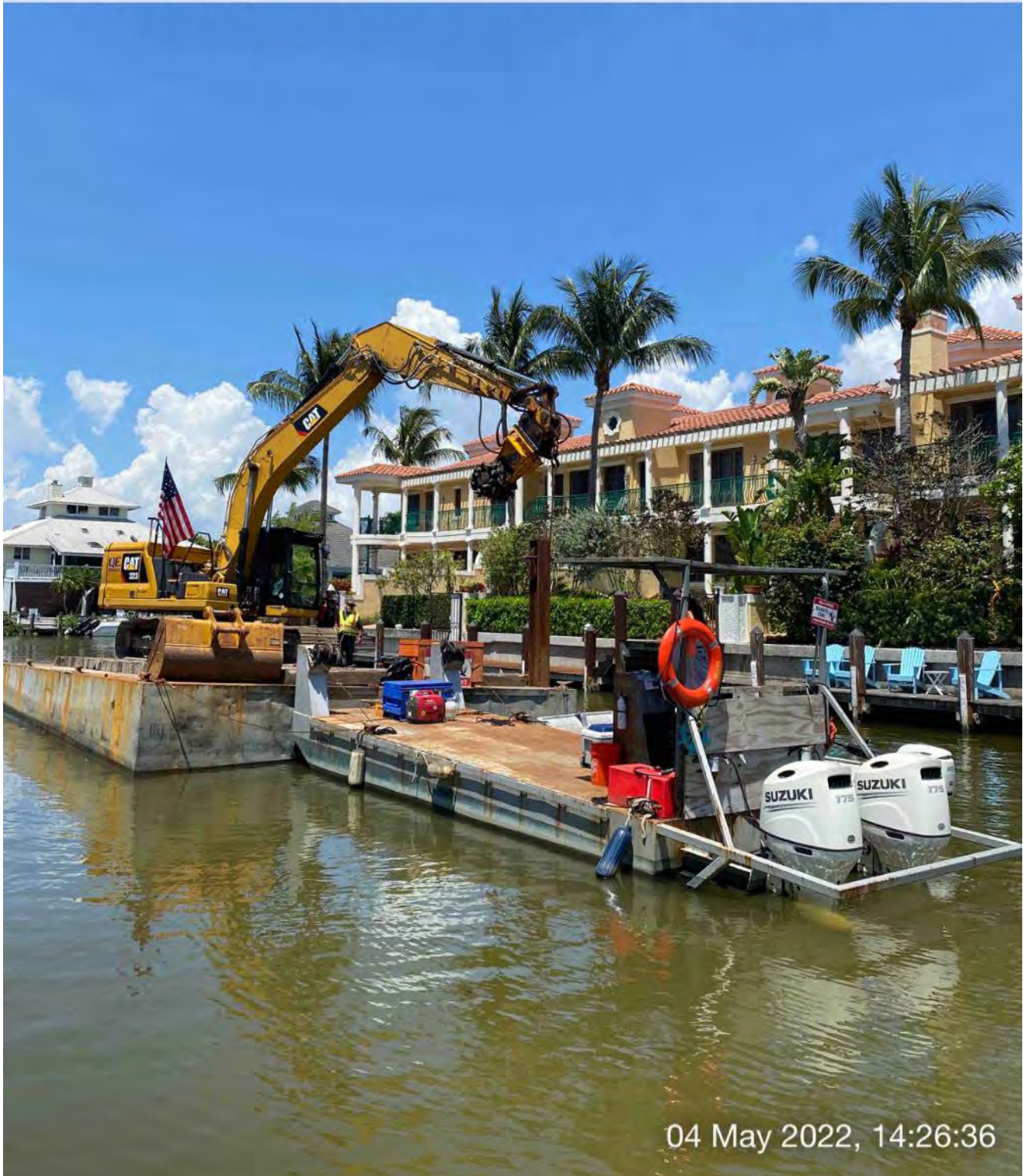
323 excavator lifting spud to allow push boat to mobilize barge at station 1+25 in Canal Y-Y
