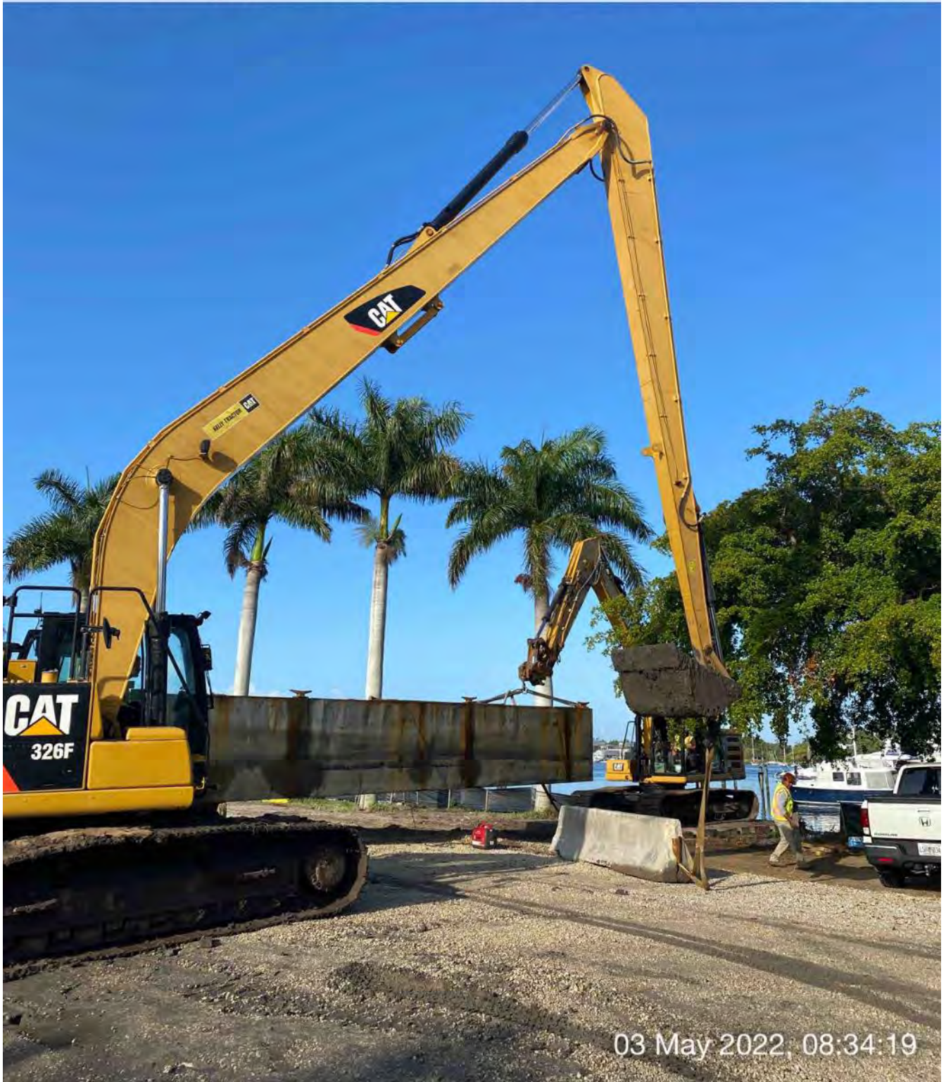
323 excavator lifting barge section to allow 326 excavator to remove jersey barrier from underneath barge
