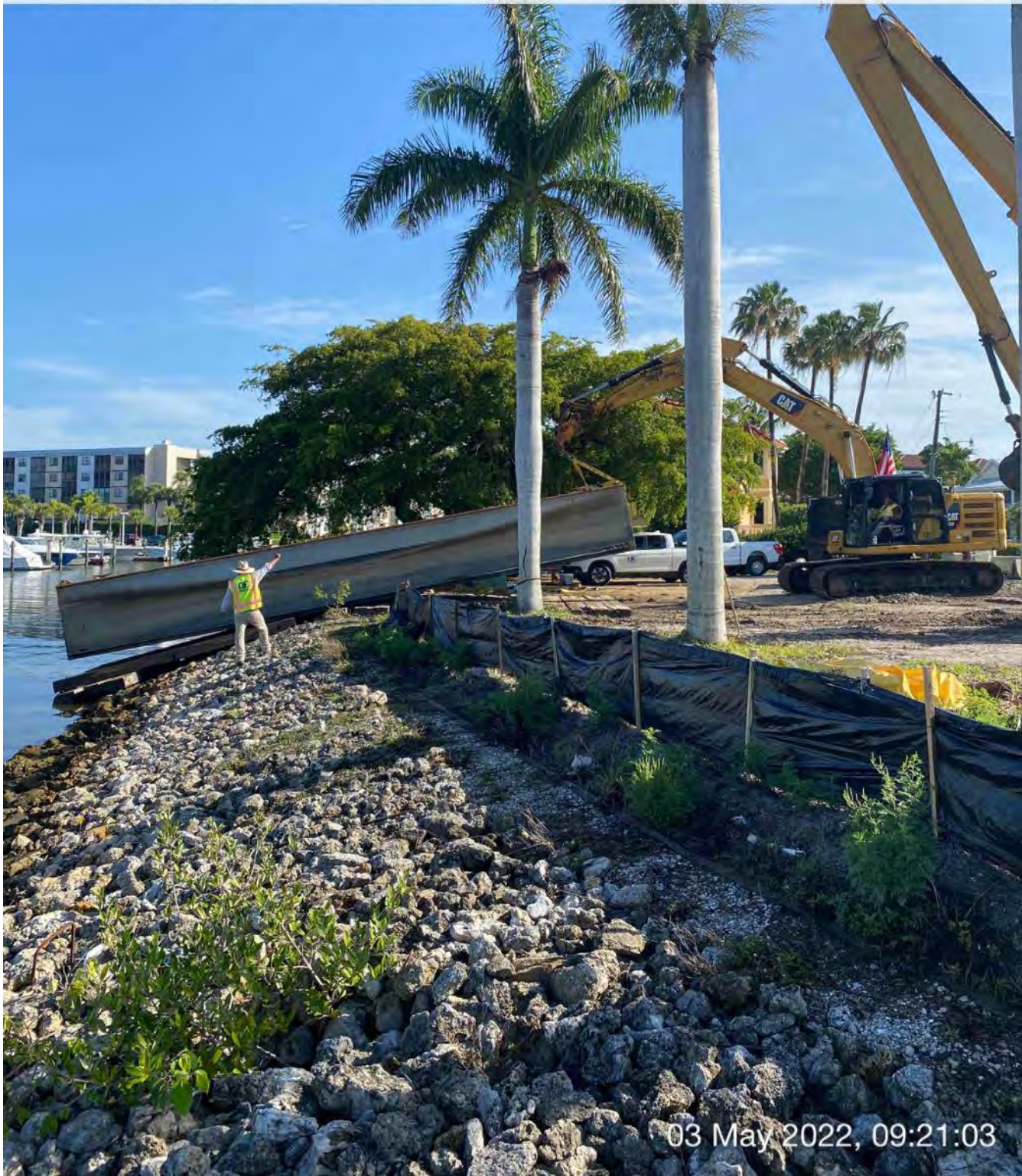
323 excavator lifting barge section at the west side of the property at 1300 Curlew Avenue
