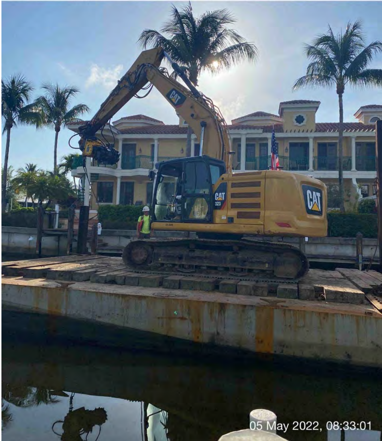
323 excavator lifting spud at station 1+00
