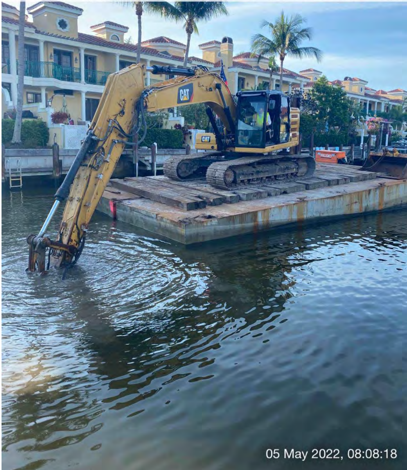
323 excavator grinding rock at station 0+75
