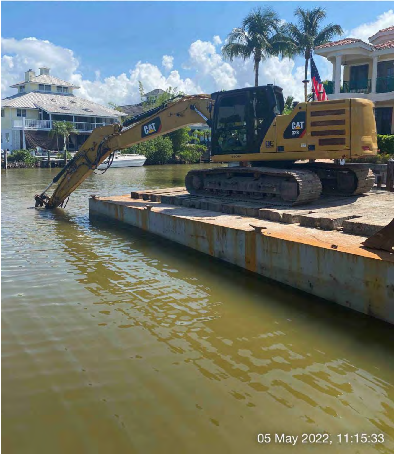
323 excavator grinding rock at station 0+50
