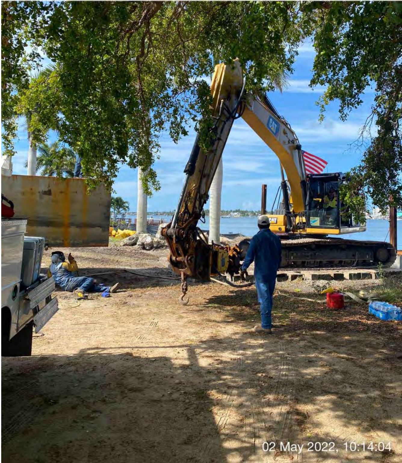
323 excavator and barge on site at 1300 Curlew Avenue
