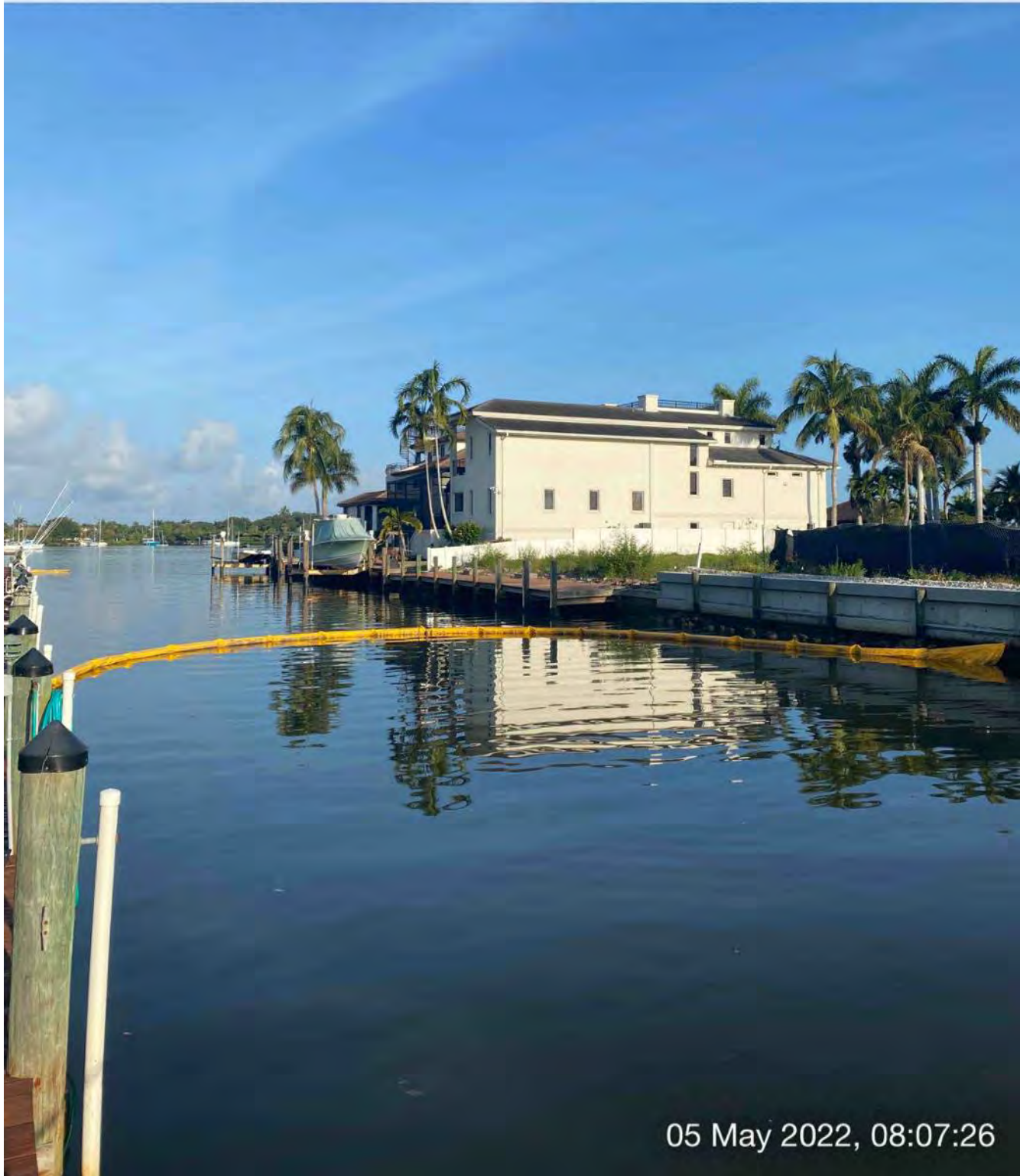
Turbidity curtain installed across Canal X-X at station 4+00
