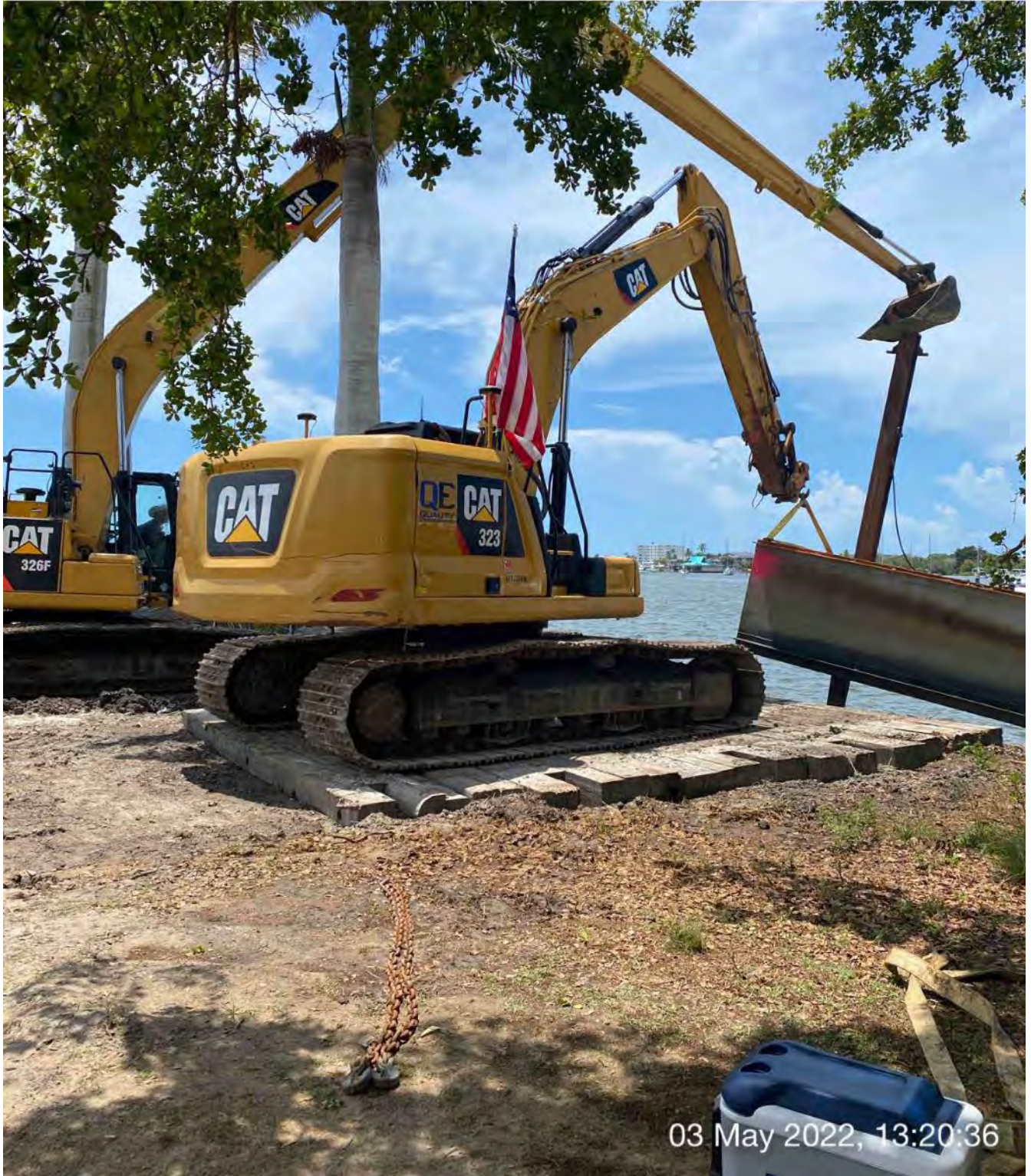
323 excavator lifting barge section and 326 excavator pushing spud
