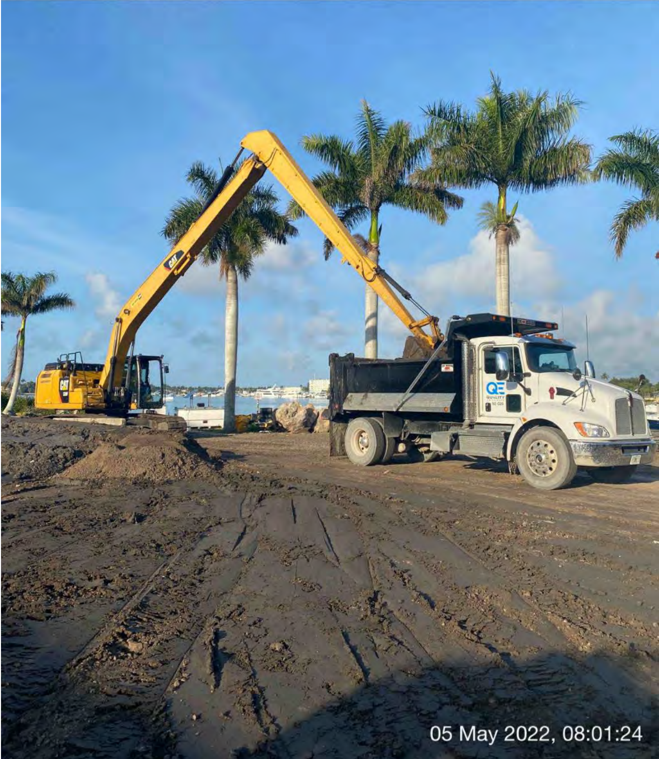
326 excavator transferring removed material from the dewatering site to dump truck bed at 1300 Curlew Avenue
