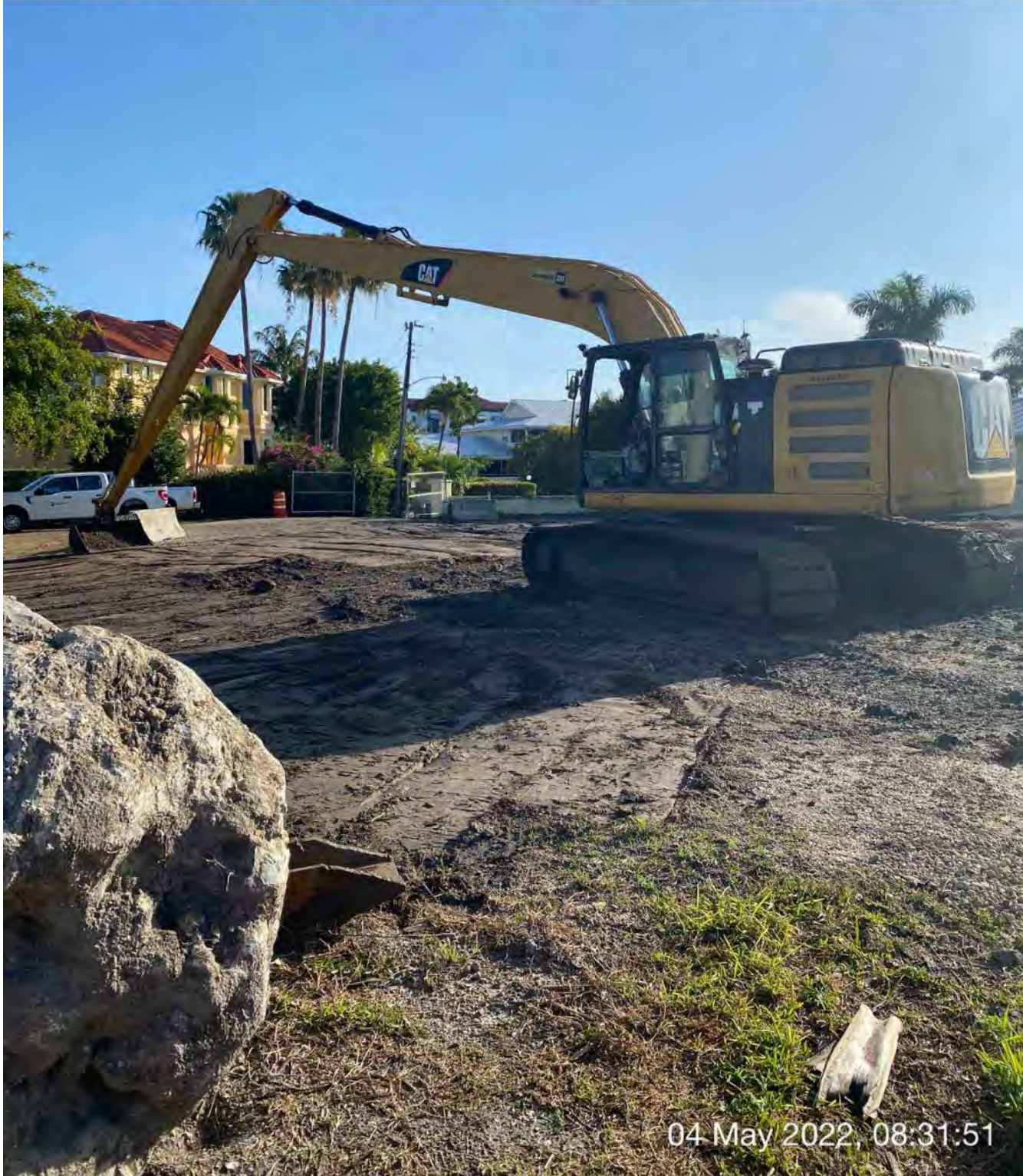
326 excavator grading the lot at 1300 Curlew Avenue.
