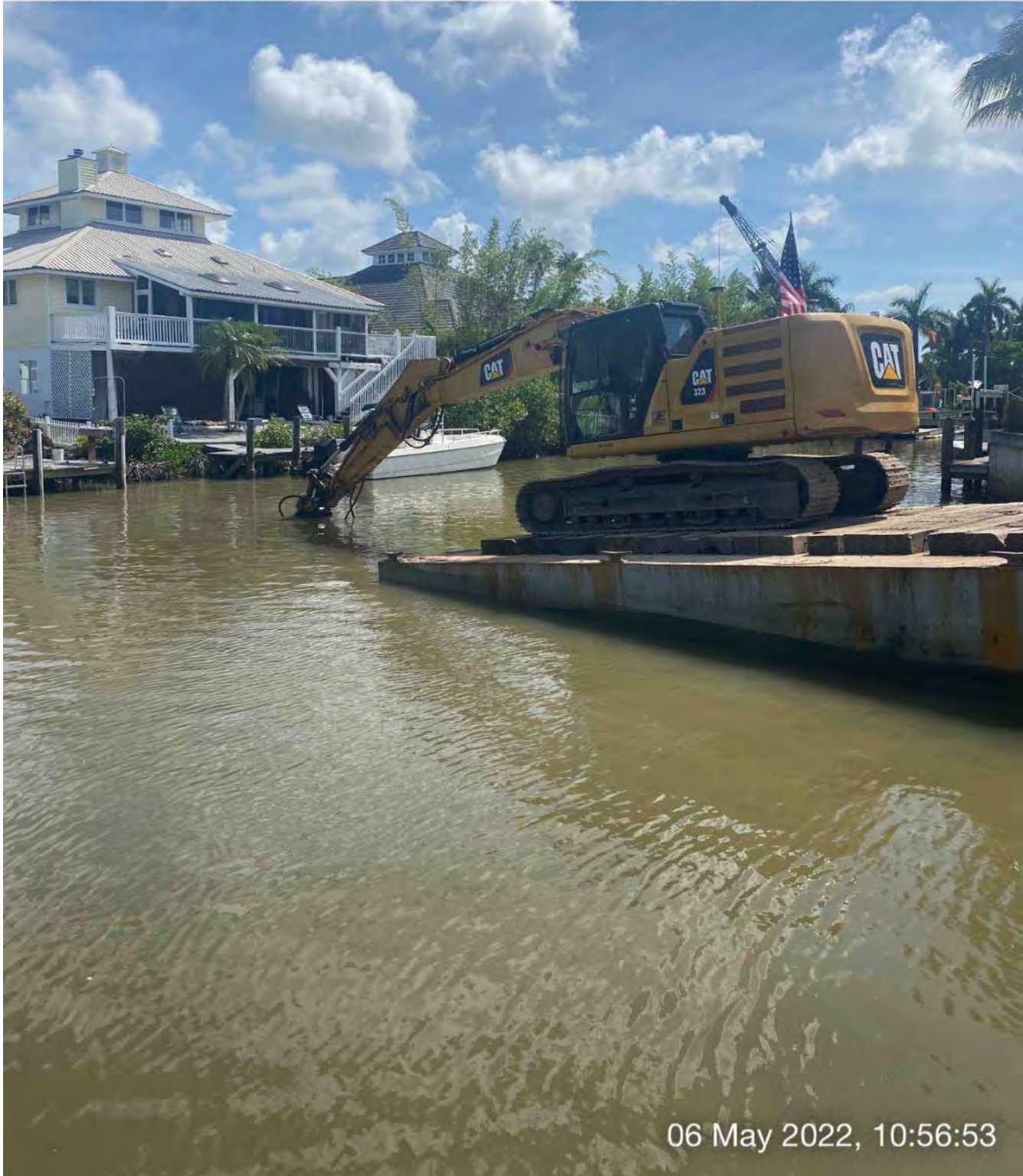
323 excavator lifting spud at station 0+00
