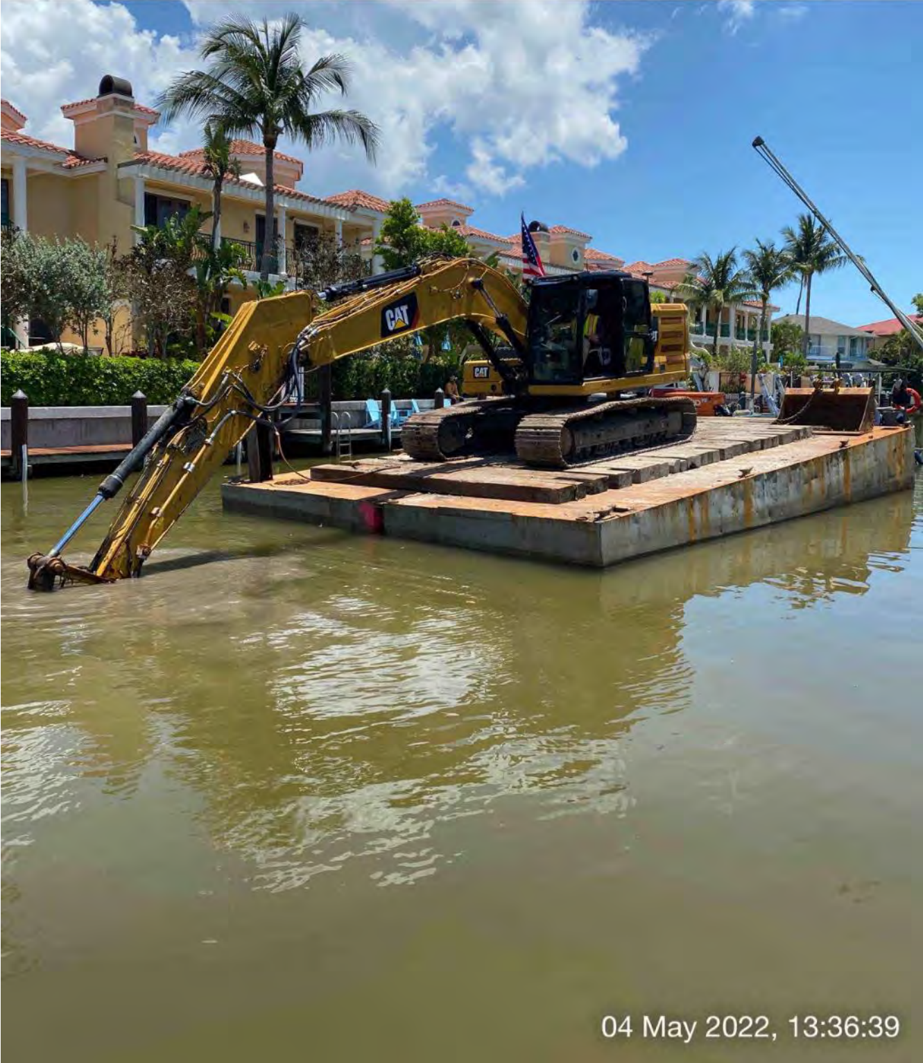
323 excavator grinding rock at station 1+25 in Canal Y-Y
