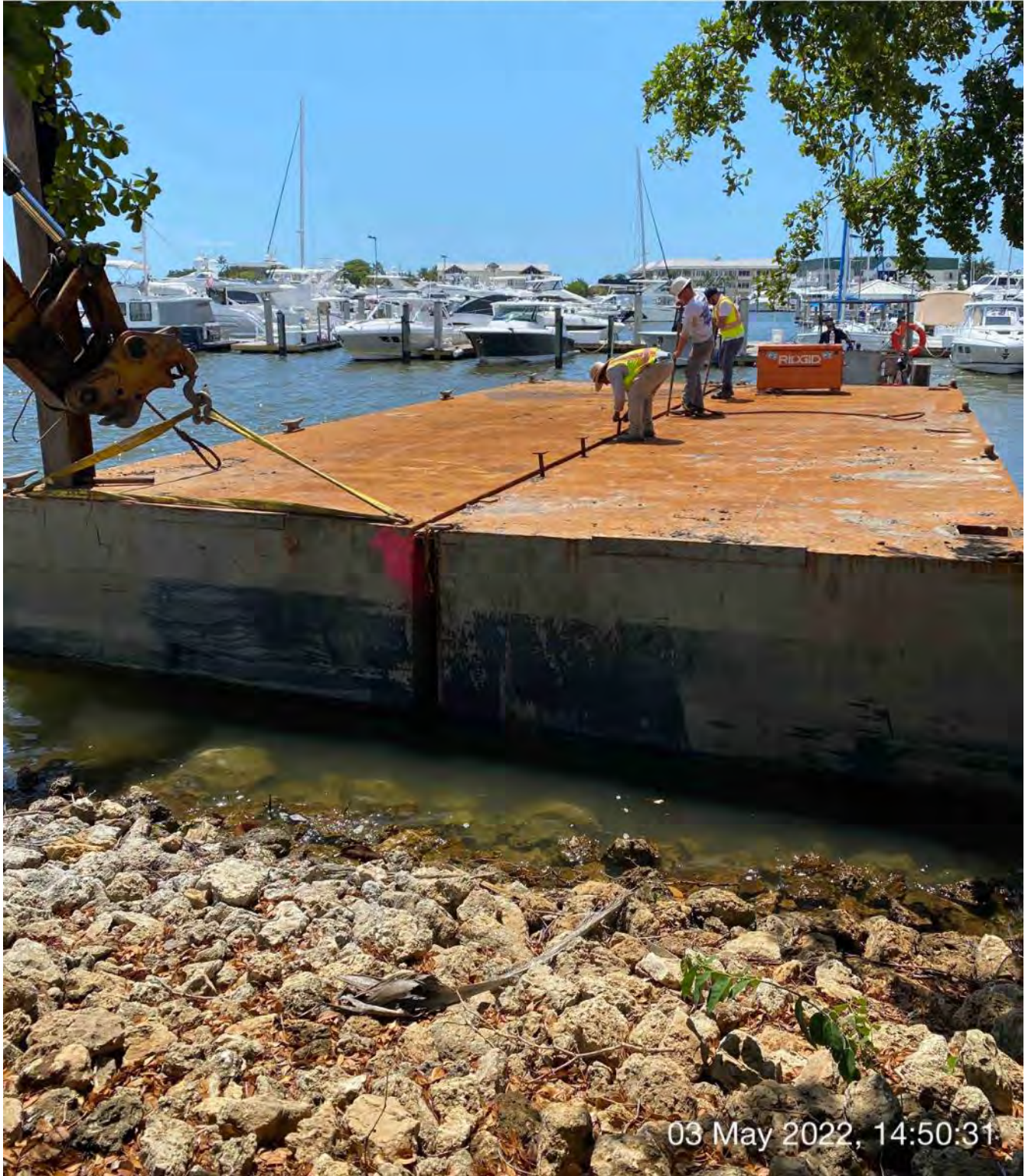
Contractor connecting two barge sections back together
