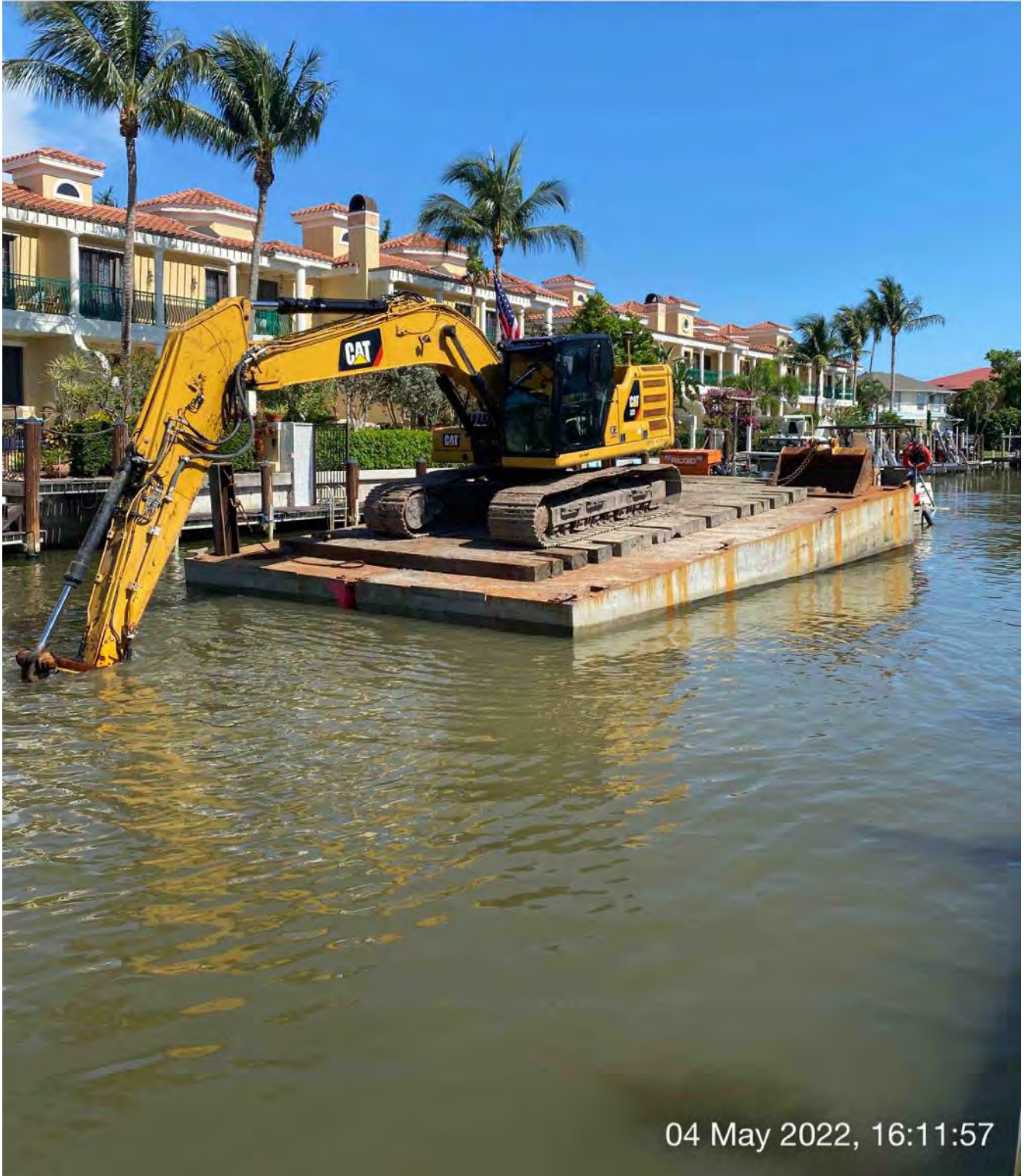
323 excavator grinding rock at station 1+00 in Canal Y-Y
