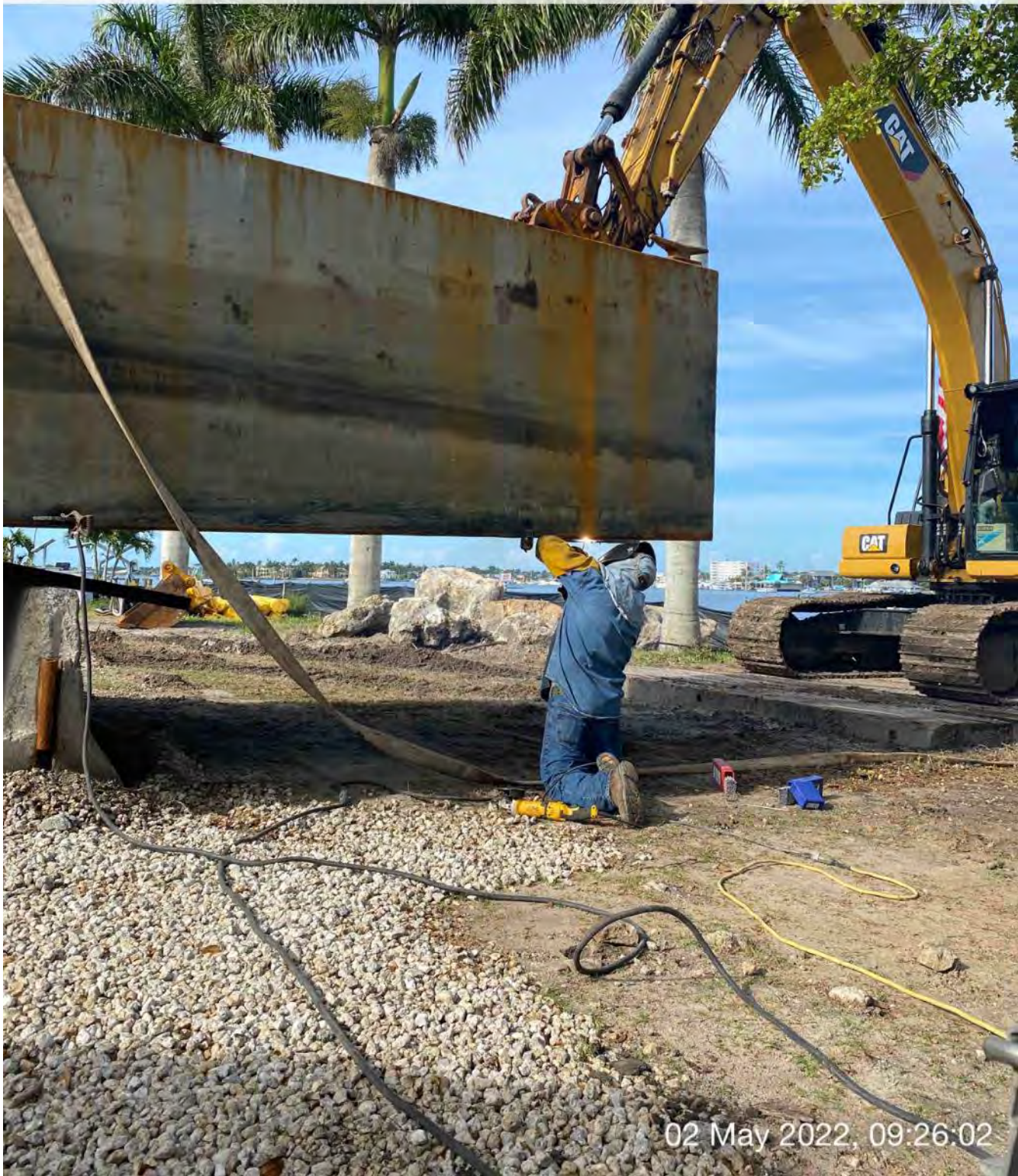
Welding the leaky area around the spud sleeve
