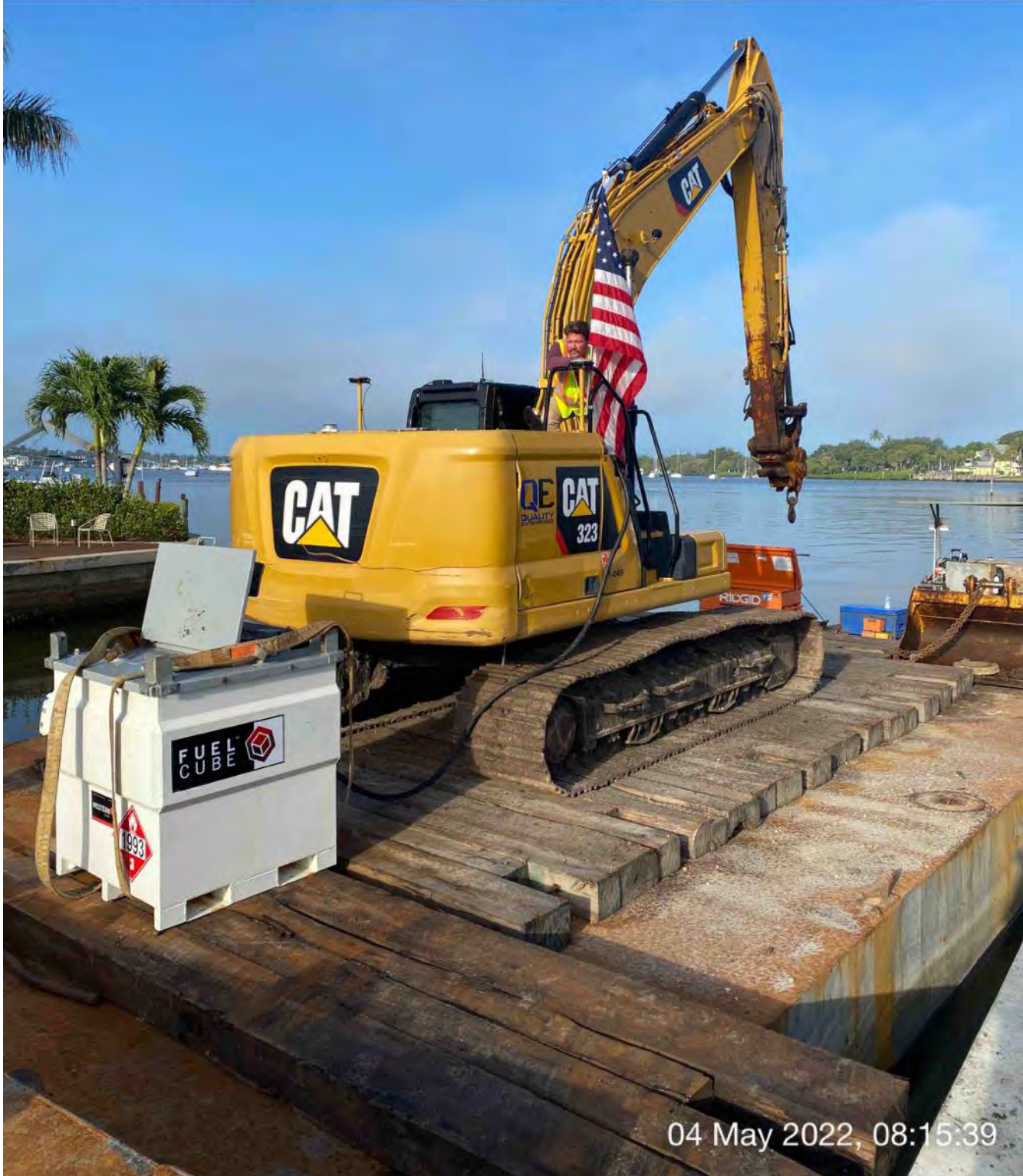
Refueling 323 excavator with small fuel cube in Canal CC-CC at station 1+25
