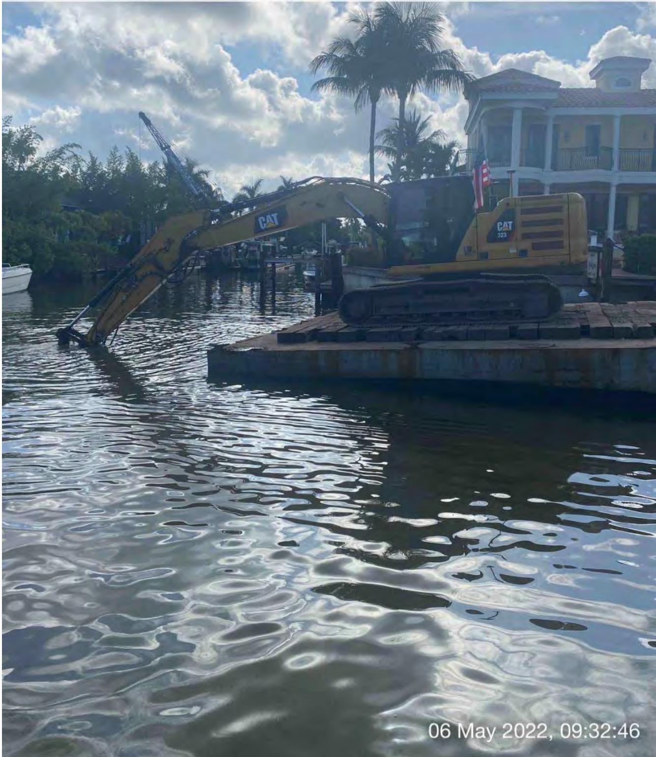
323 excavator grinding rock at station 0+25
