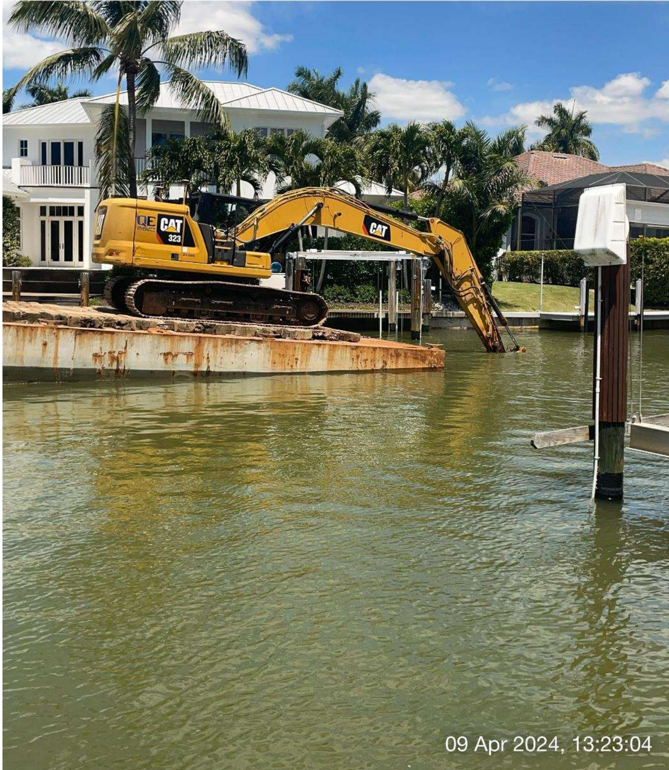
323 excavator grinding rock at station 14+00 in Canal A-A.
