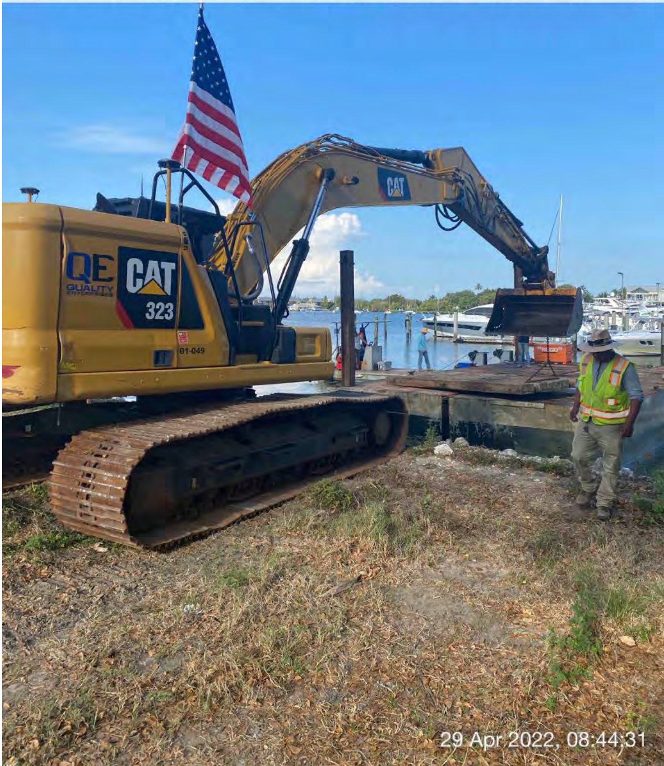
323 excavator lifting crane tracks from barge to 1300 Curlew Avenue
