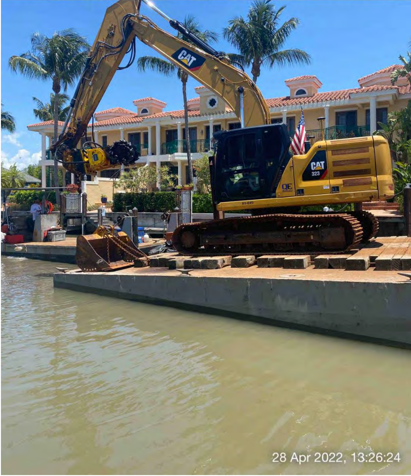
323 excavator on barge with Epiroc grinder at station 1+25
