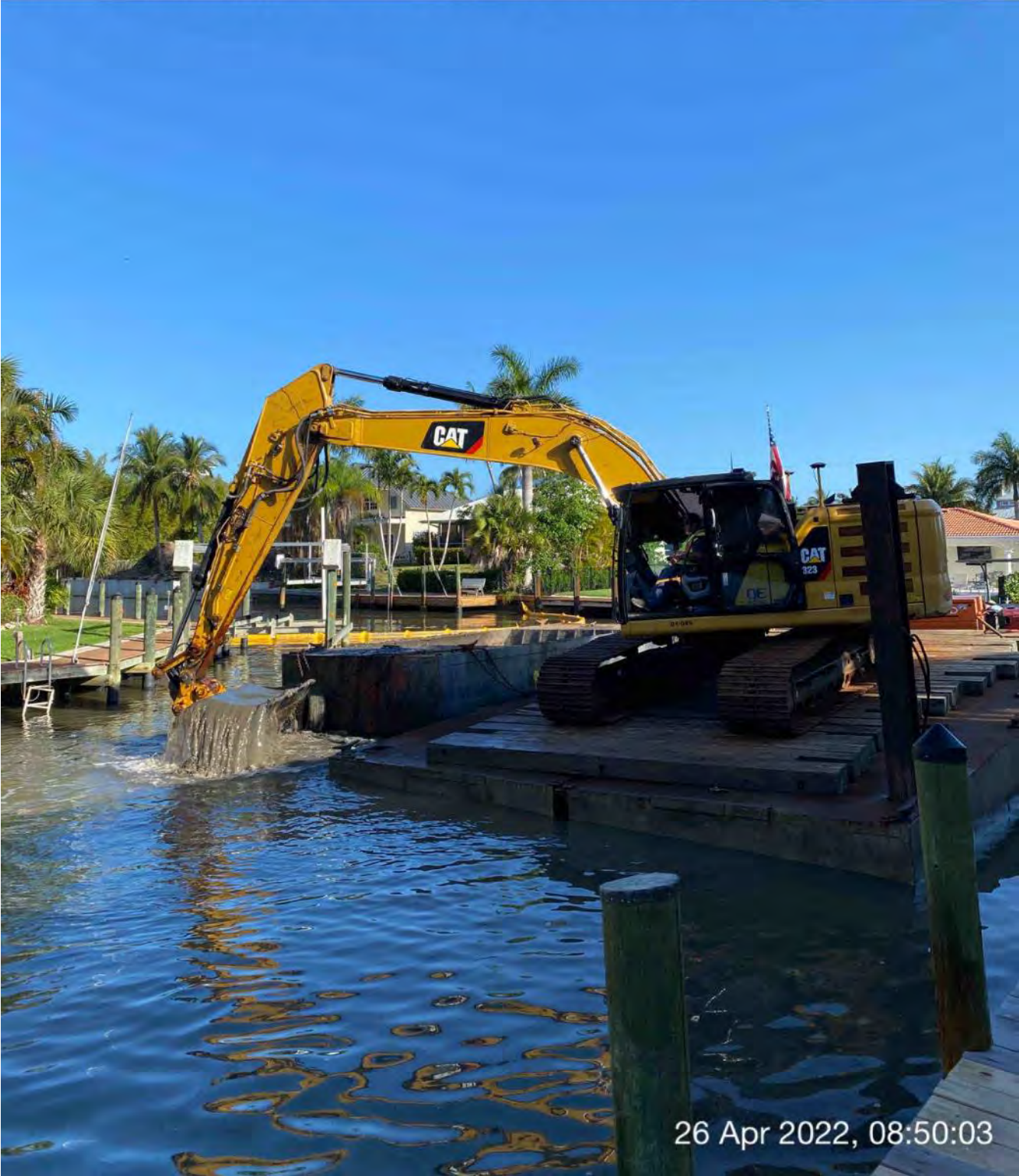
323 excavator removing material from station 1+50
