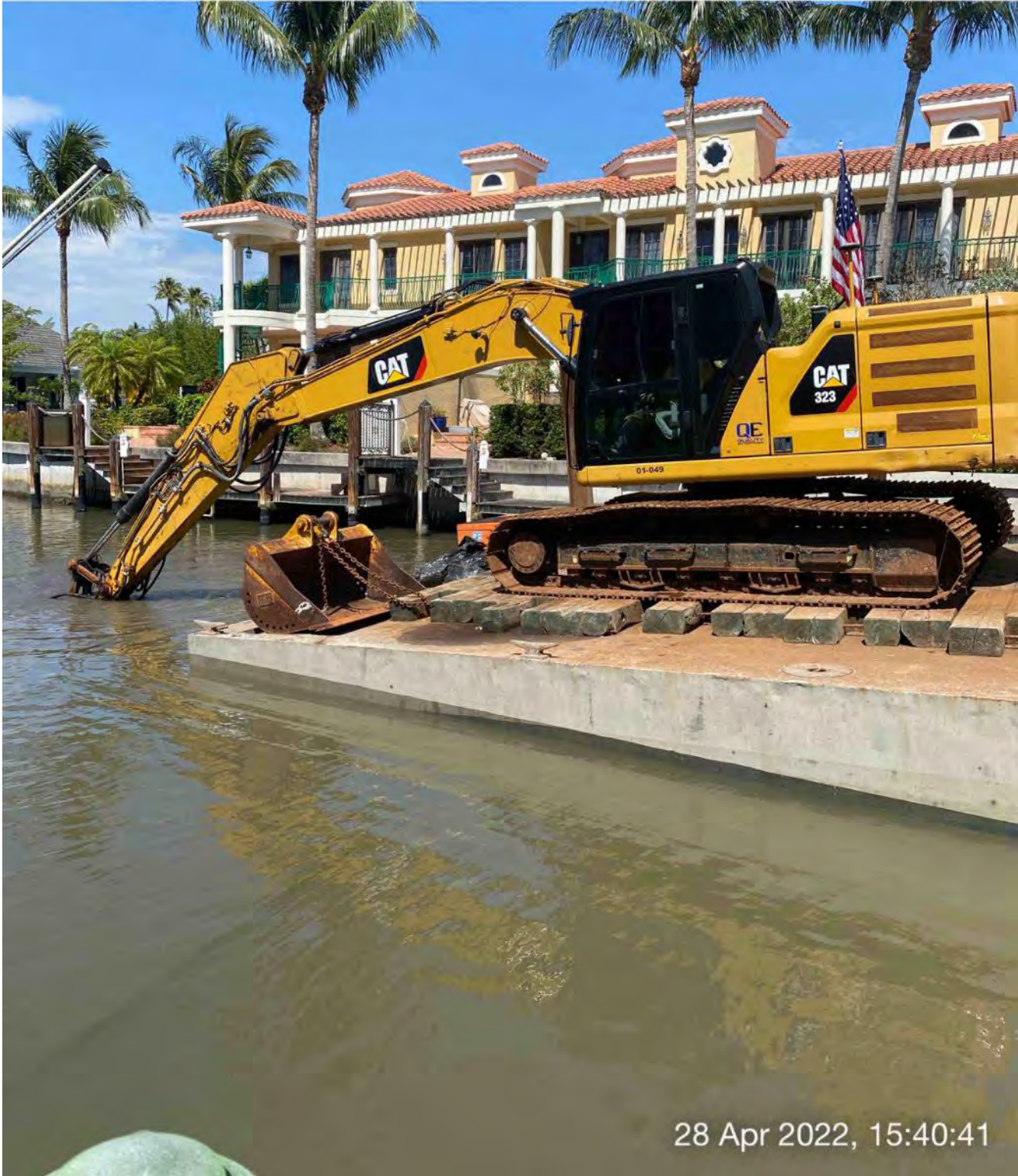
323 excavator grinding rock at station 1+00
