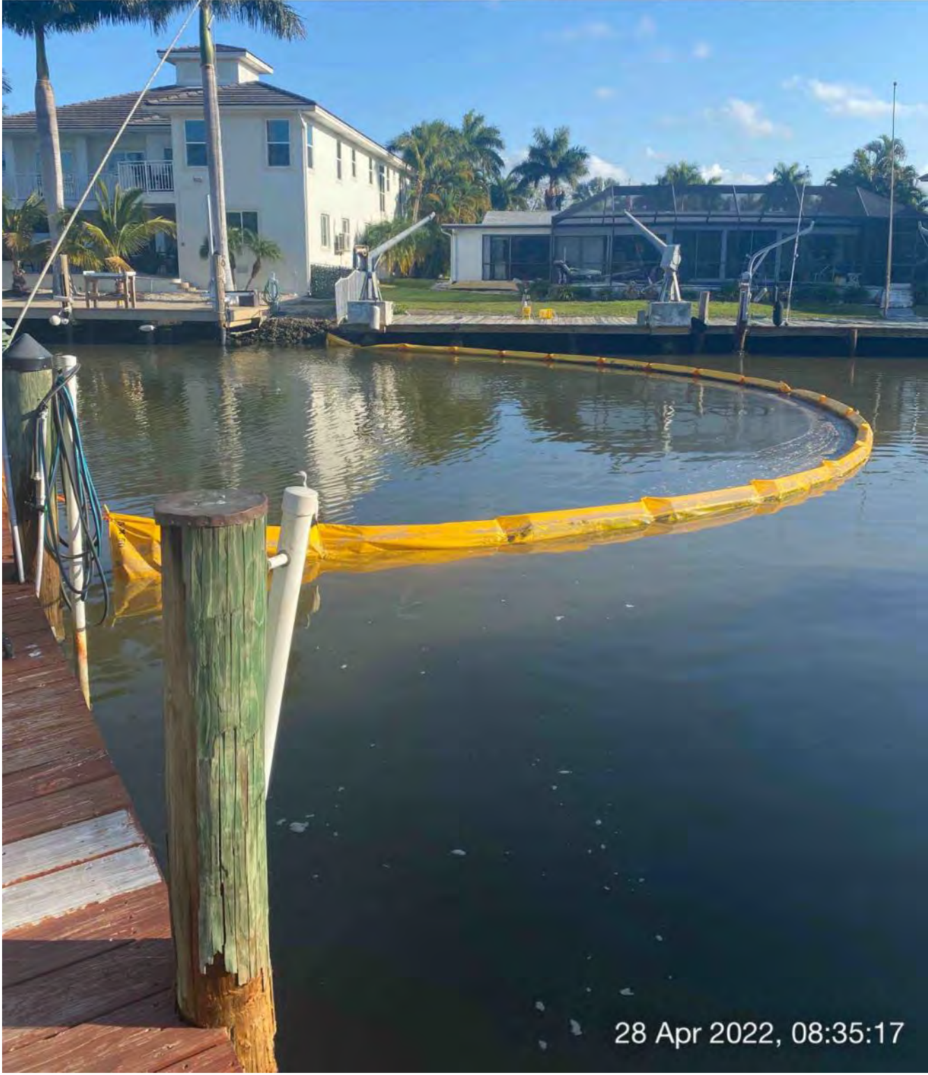
Turbidity curtain installed across Canal X-X at station 4+75
