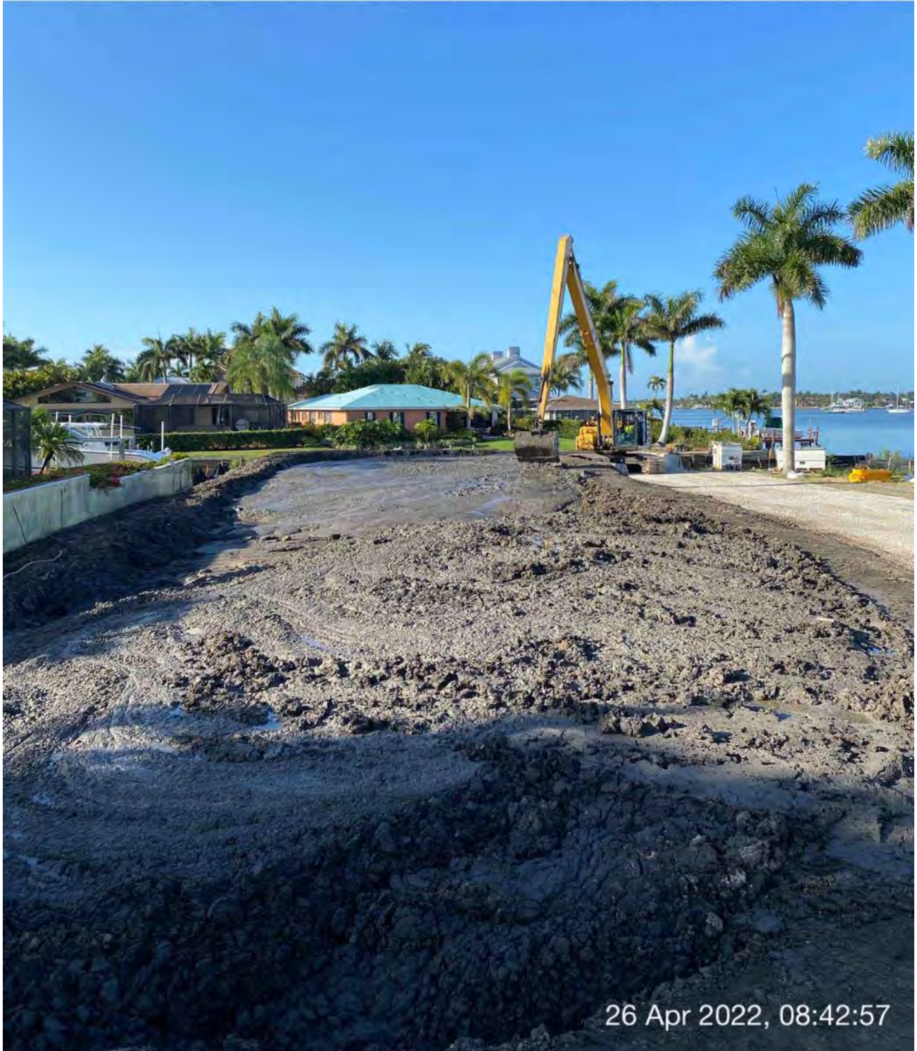
326 excavator transferring one hopper of removed material from hopper to dewatering site at 1300 Curlew Avenue
