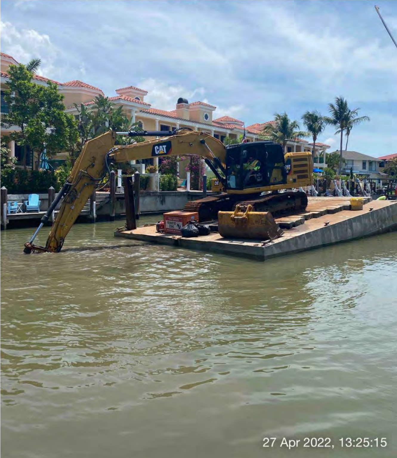
323 excavator grinding material at station 1+50 in Canal Y-Y
