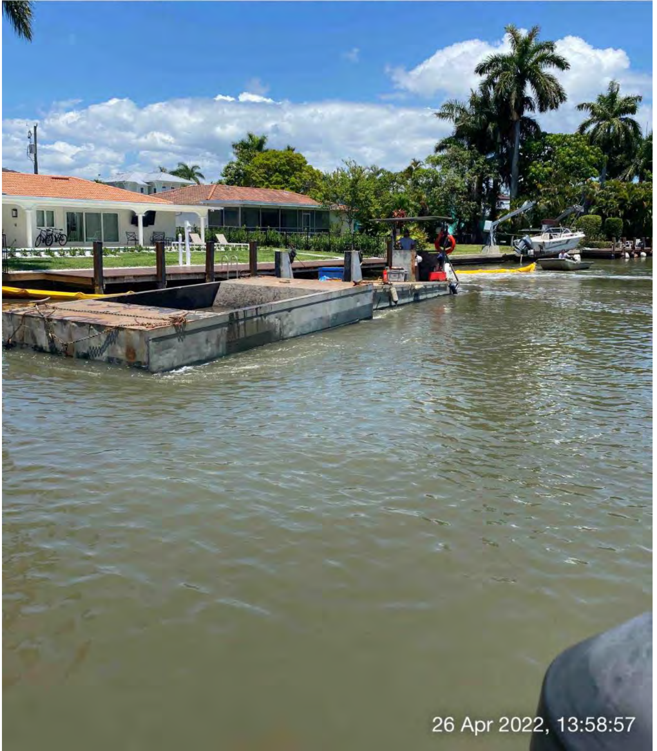
Support boat opening turbidity curtain to allow push boat to transport hopper out of Canal X-X
