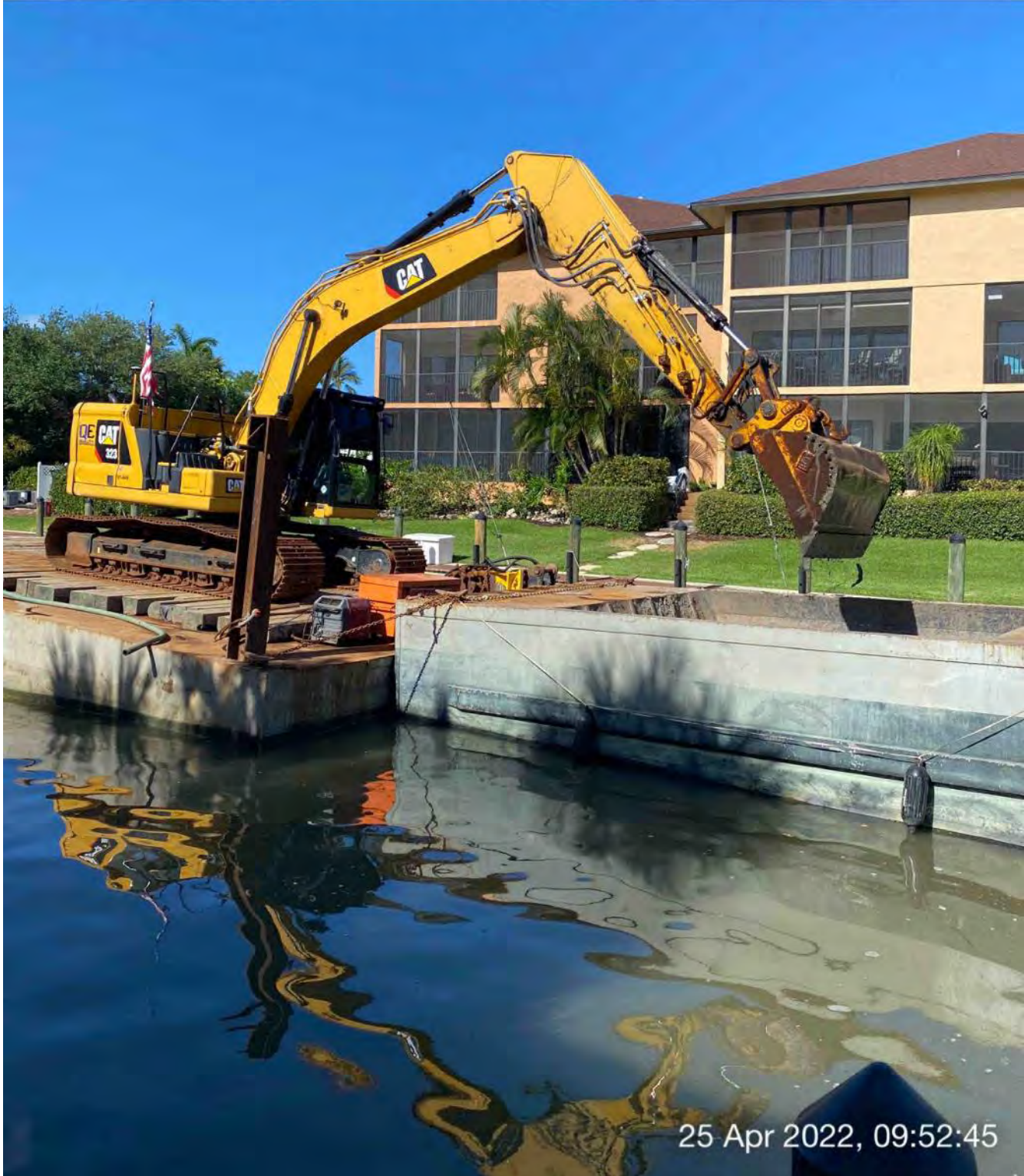
323 excavator removing material from station 2+50 and transferring it to hopper
