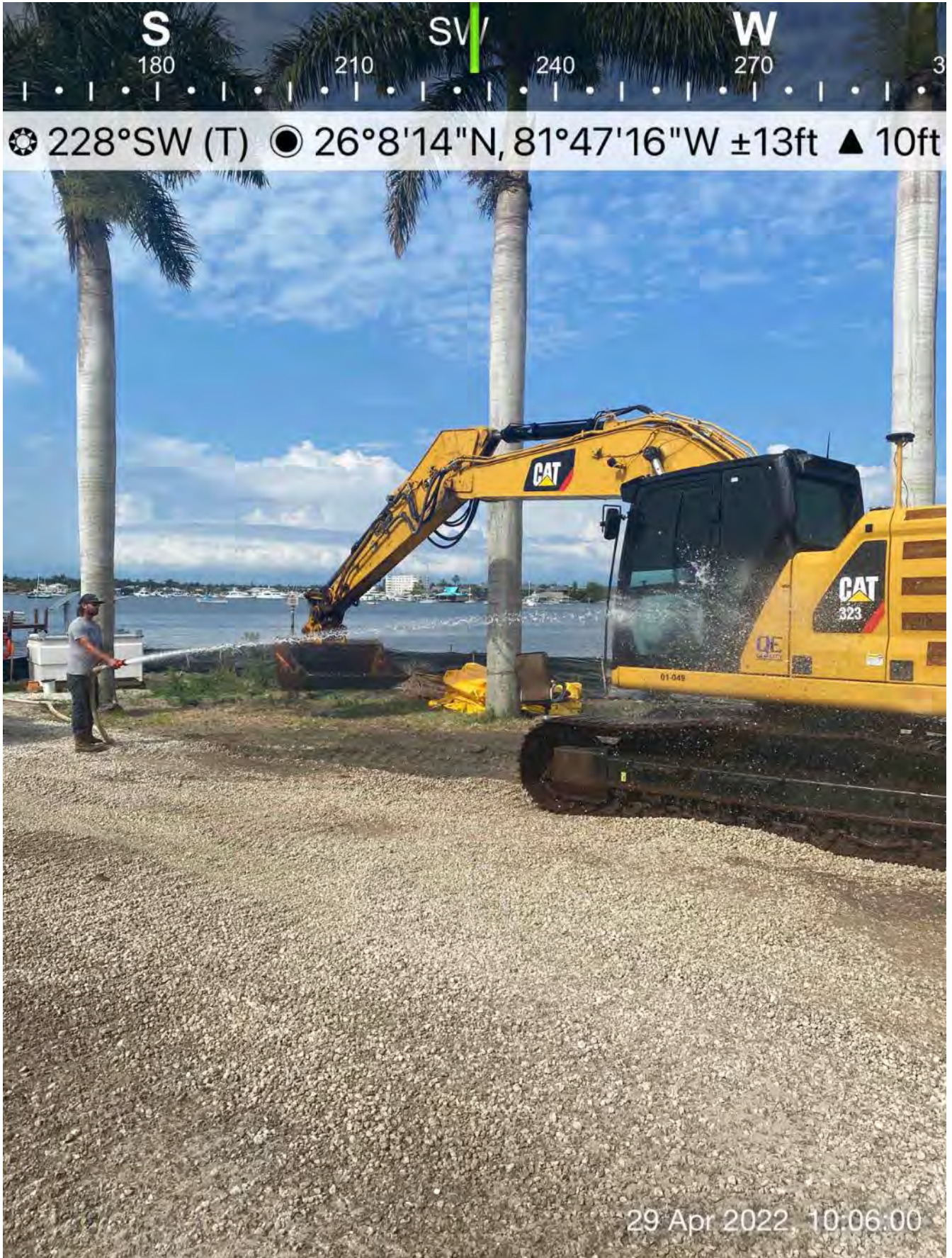
Contractor using water tank and hose to clean 323 excavator
