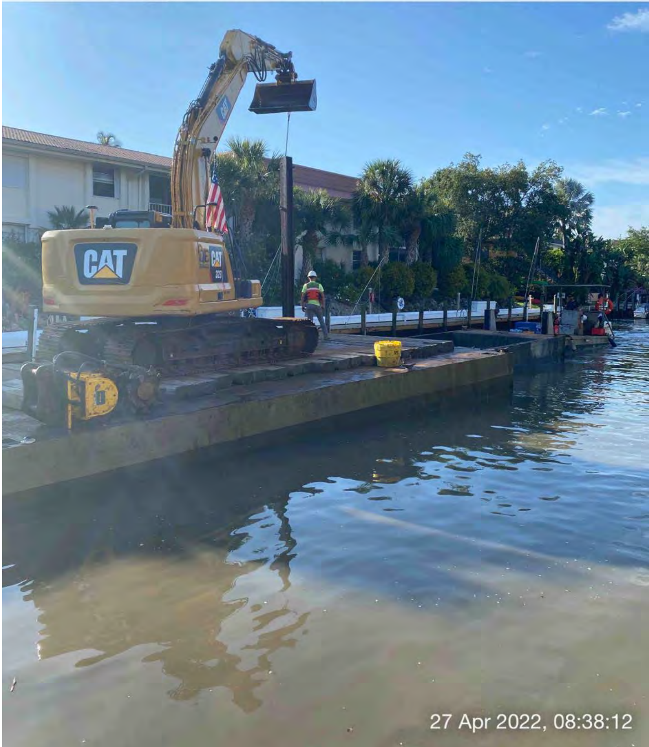
323 excavator lifting spud to allow push boat to mobilize barge at station 2+50 in Canal Z-Z
