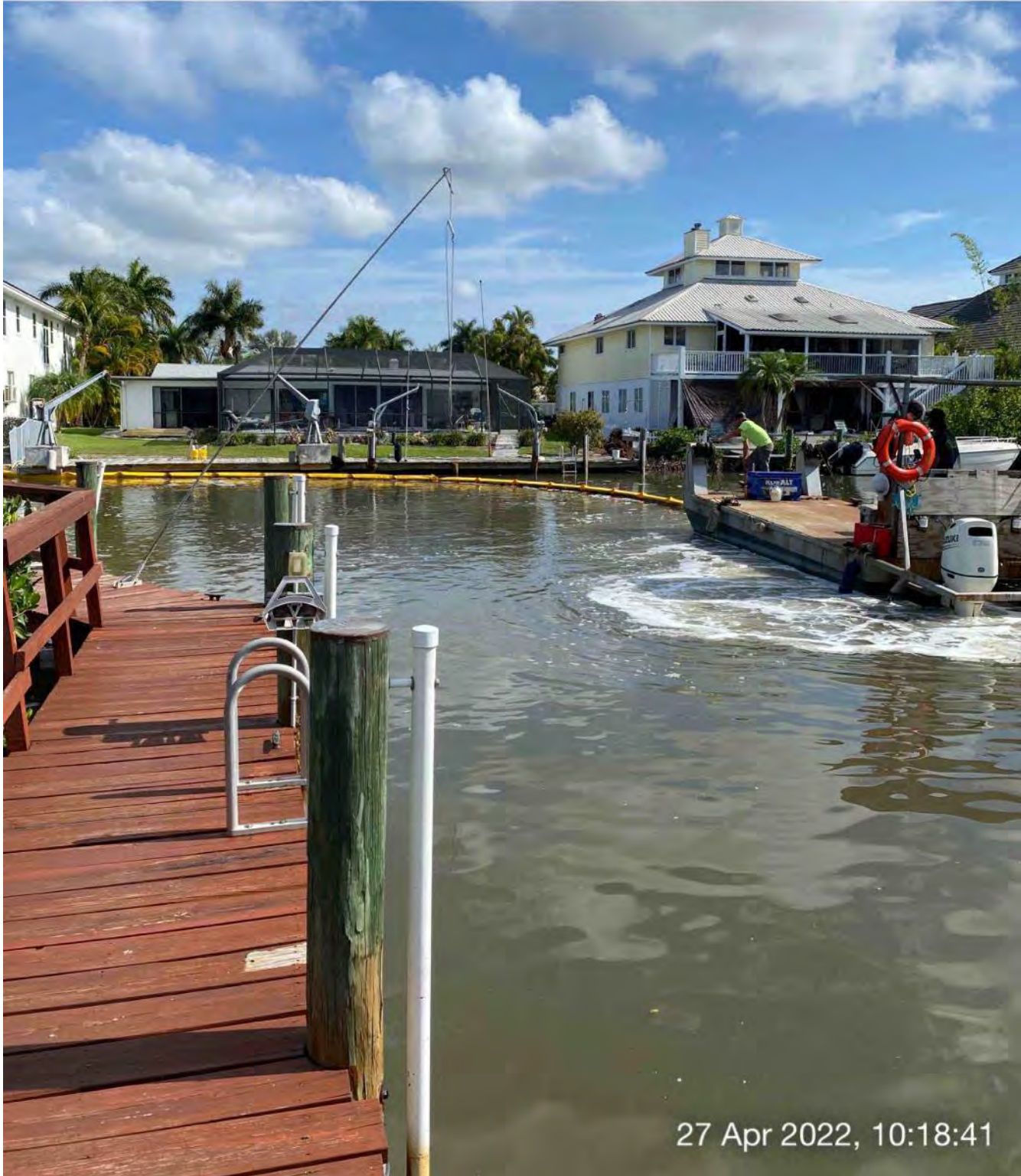
Push boat being used to installing turbidity curtain across Canal X-X at station 4+75
