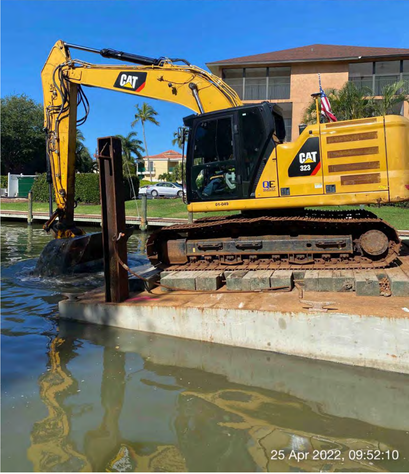
323 excavator removing material from station 2+50
