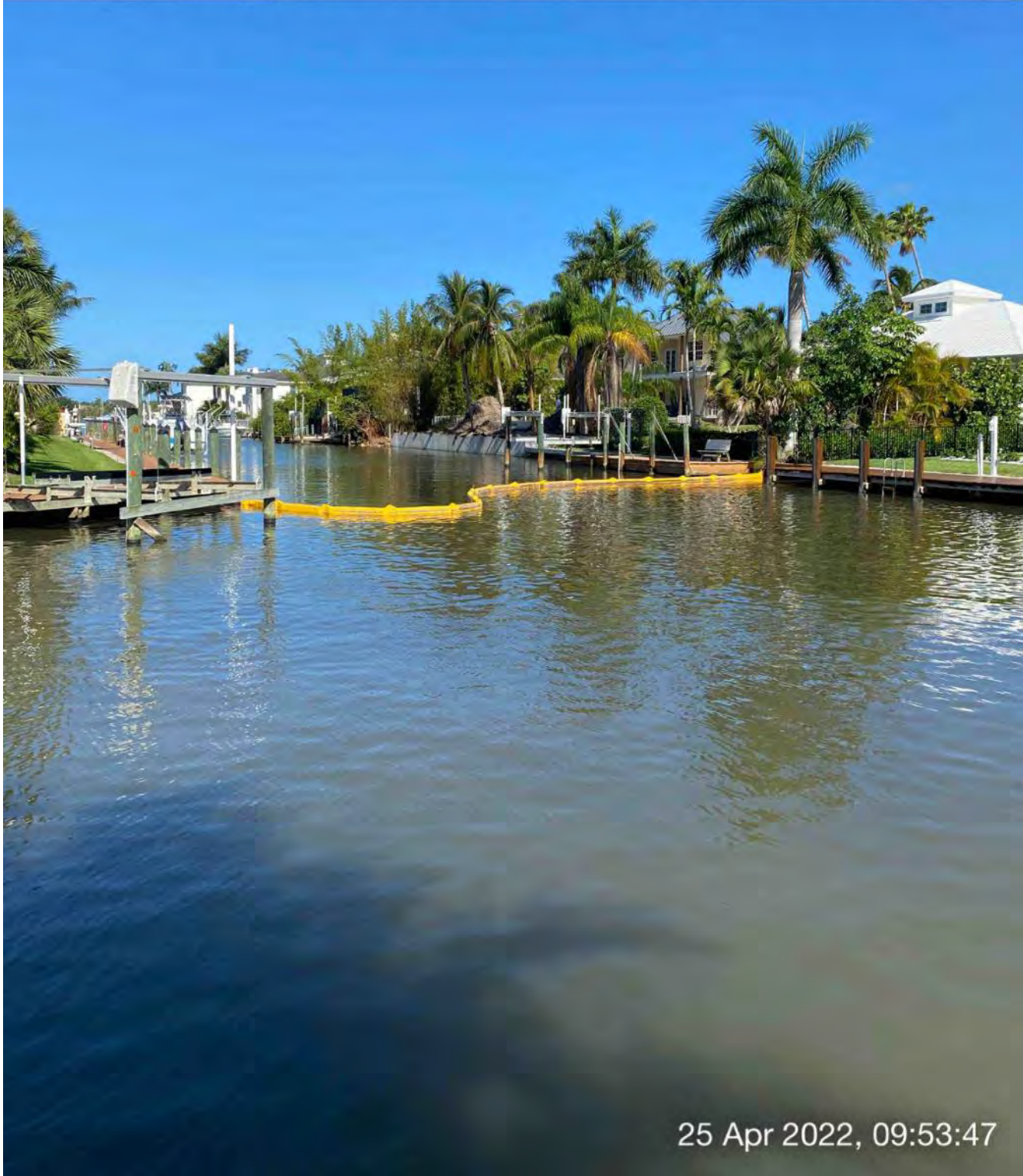
Turbidity curtain installed across Canal X-X at station 8+50
