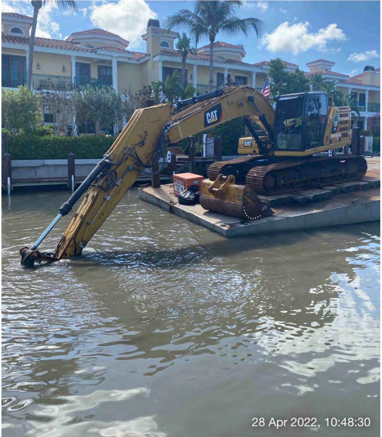
323 excavator grinding rock at station 1+50
