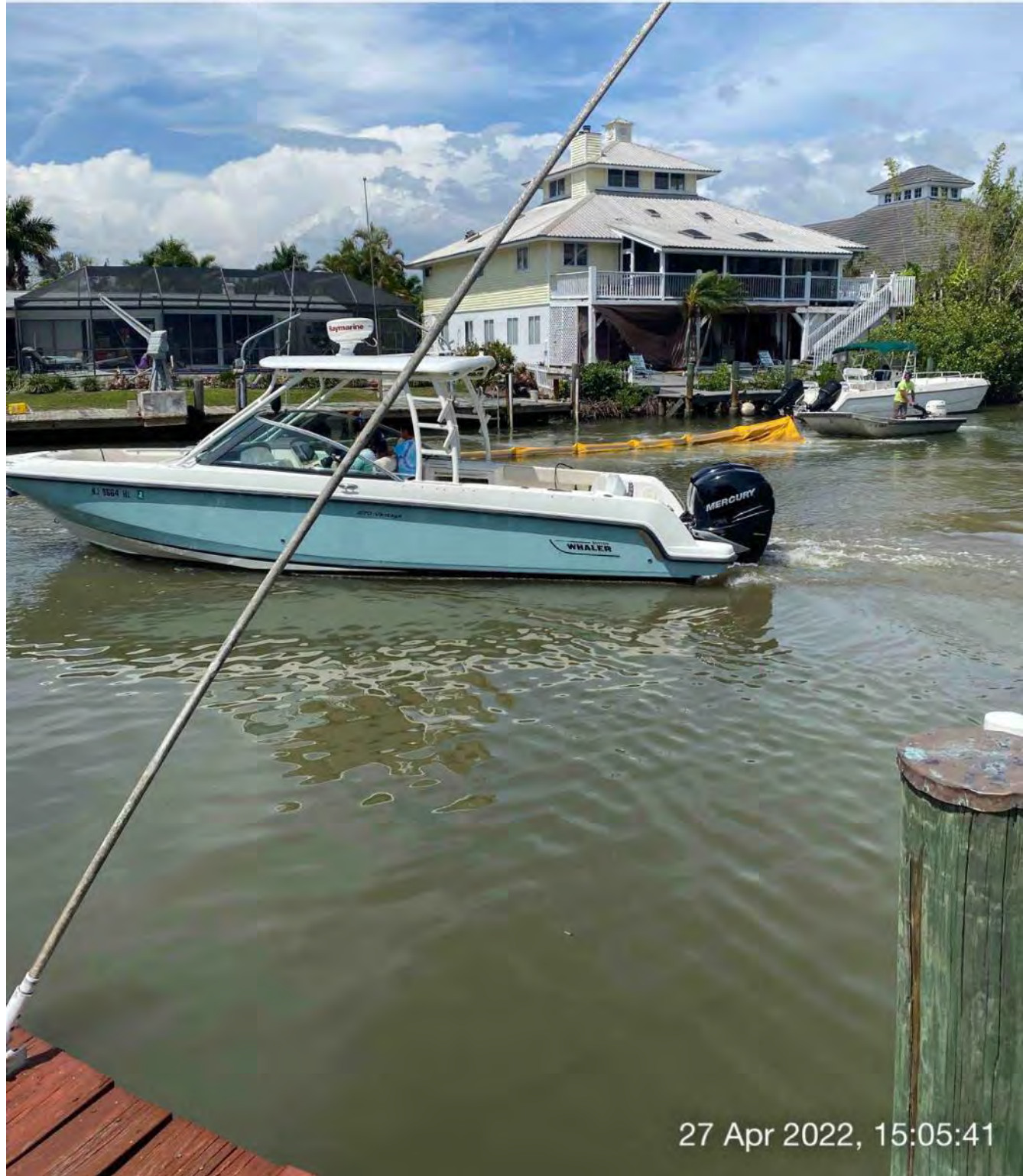
Support boat opening turbidity curtain to allow resident to exit Canal X-X
