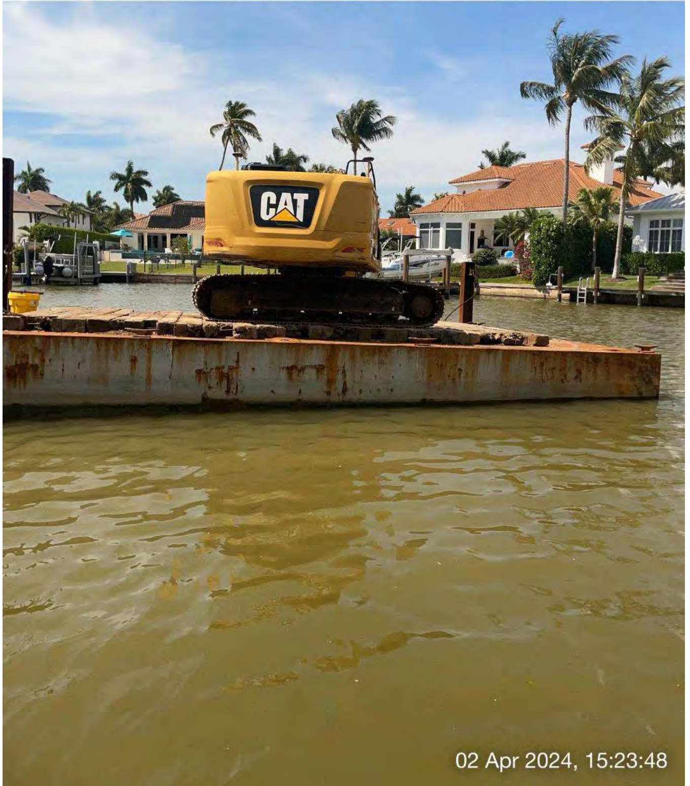
323 excavator grinding rock at station 13+40 in Canal A-A.
