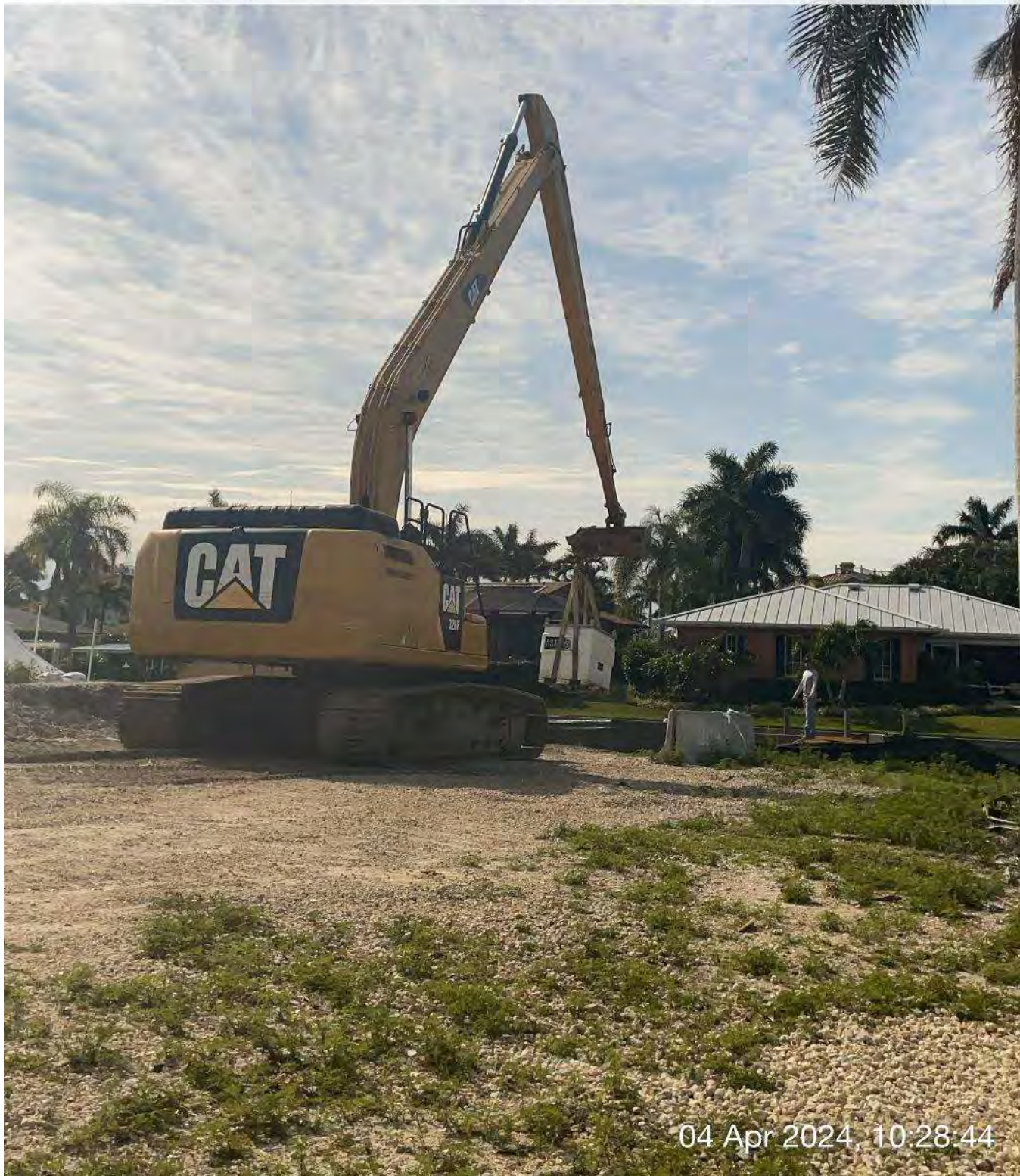
Long reach excavator loading fuel cube into hopper.
