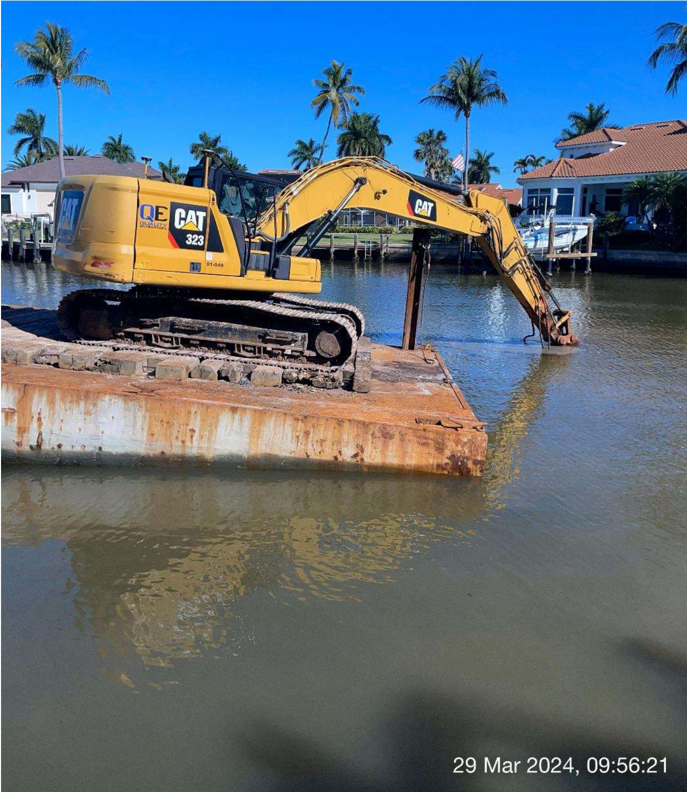
323 excavator grinding rock at station 13+25 in Canal A-A.
