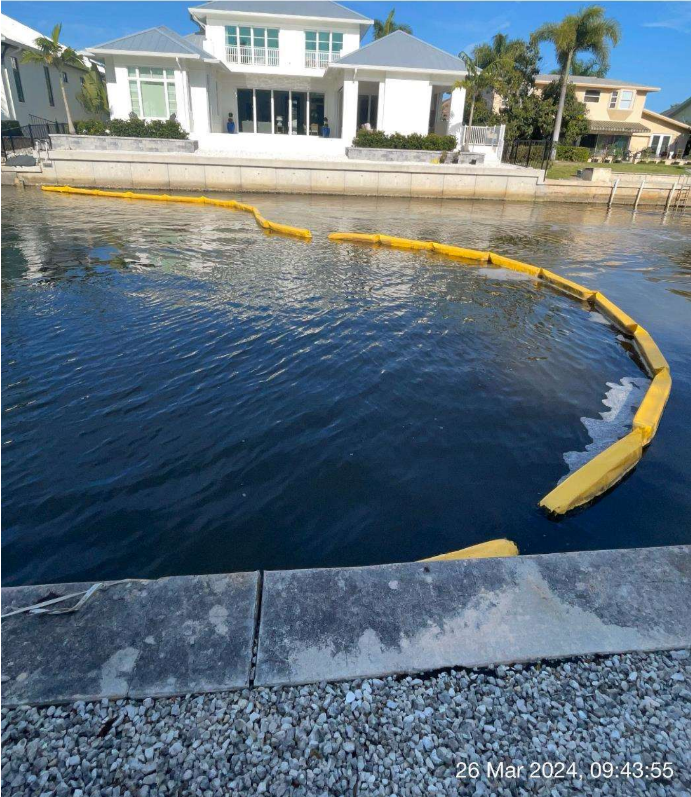
Turbidity curtain in place at station 6+00 in Canal A-A.
