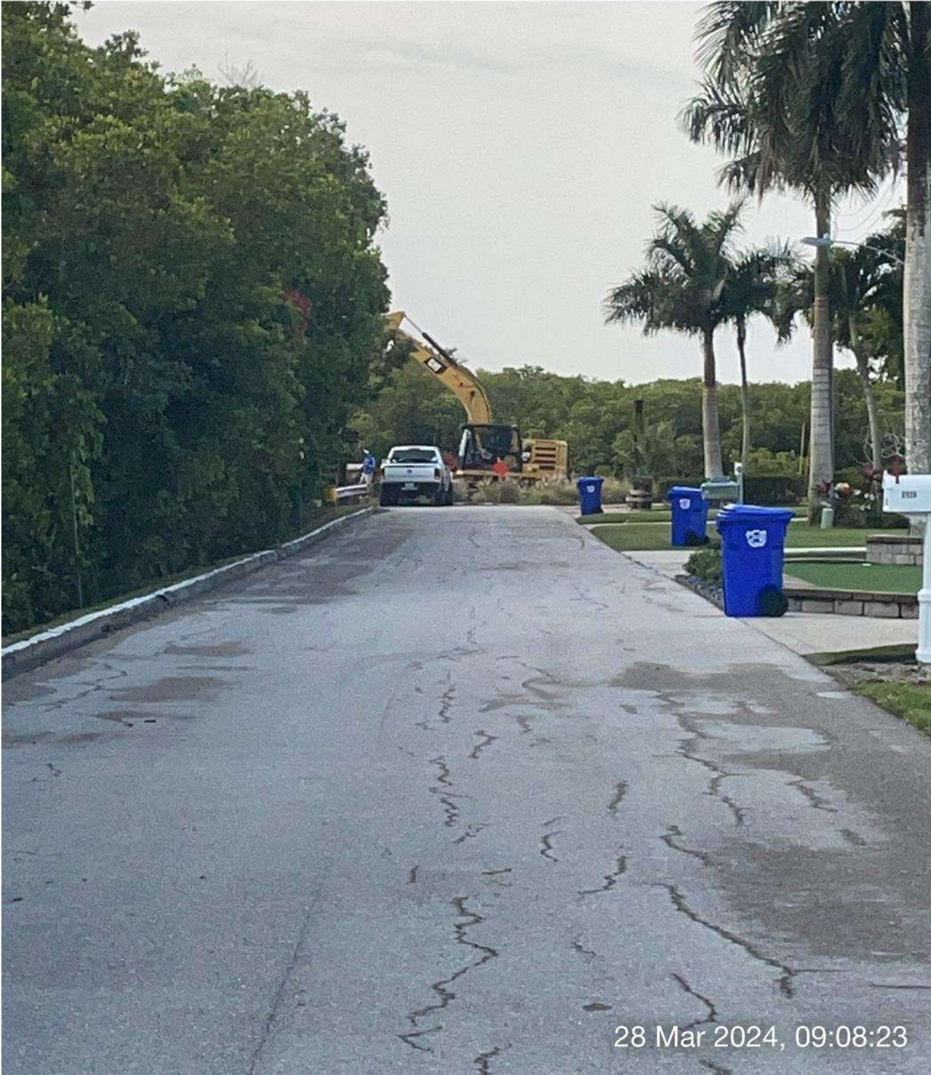
323 excavator lifting support boat out of water for maintenance work.
