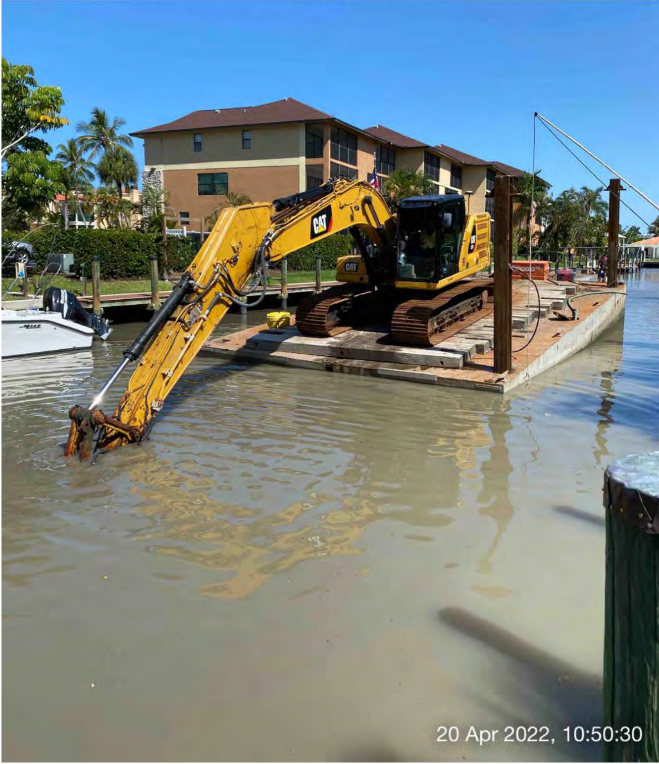
323 excavator grinding rock at station 3+50
