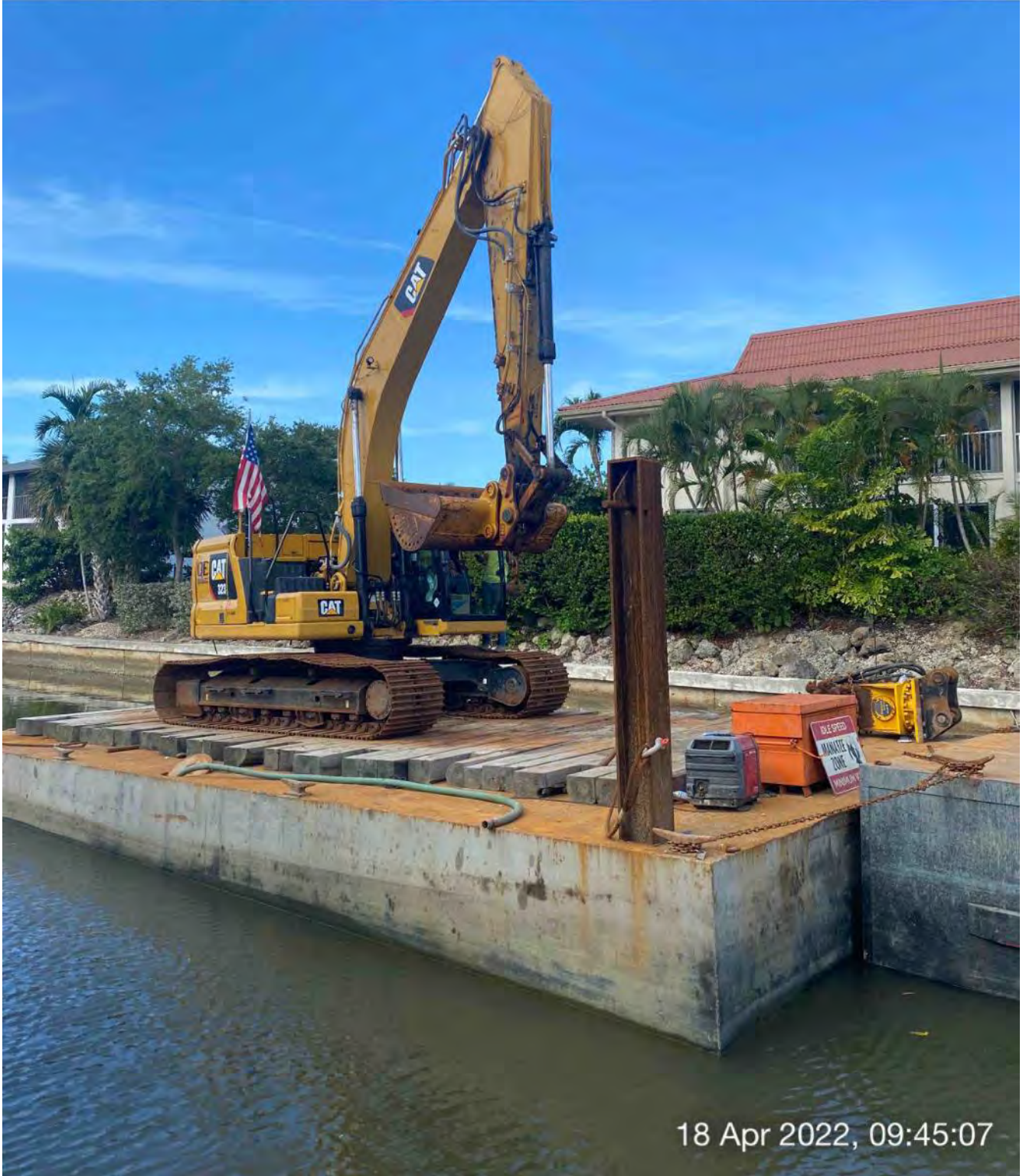
323 excavator on barge at station 1+75
