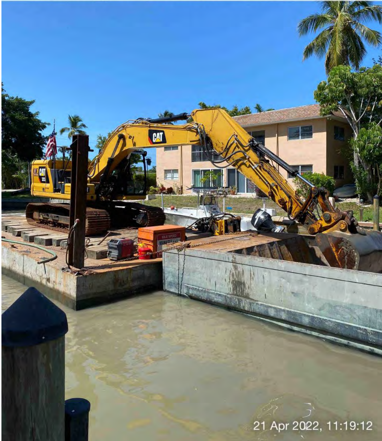
323 excavator removing material from station 3+50 and transferring it to hopper
