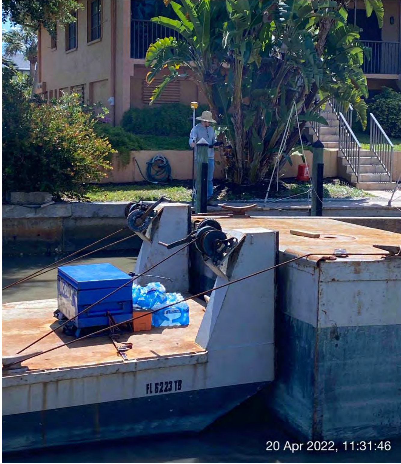
Contractor using Trimble RTK to survey dock locations in Canal Z-Z
