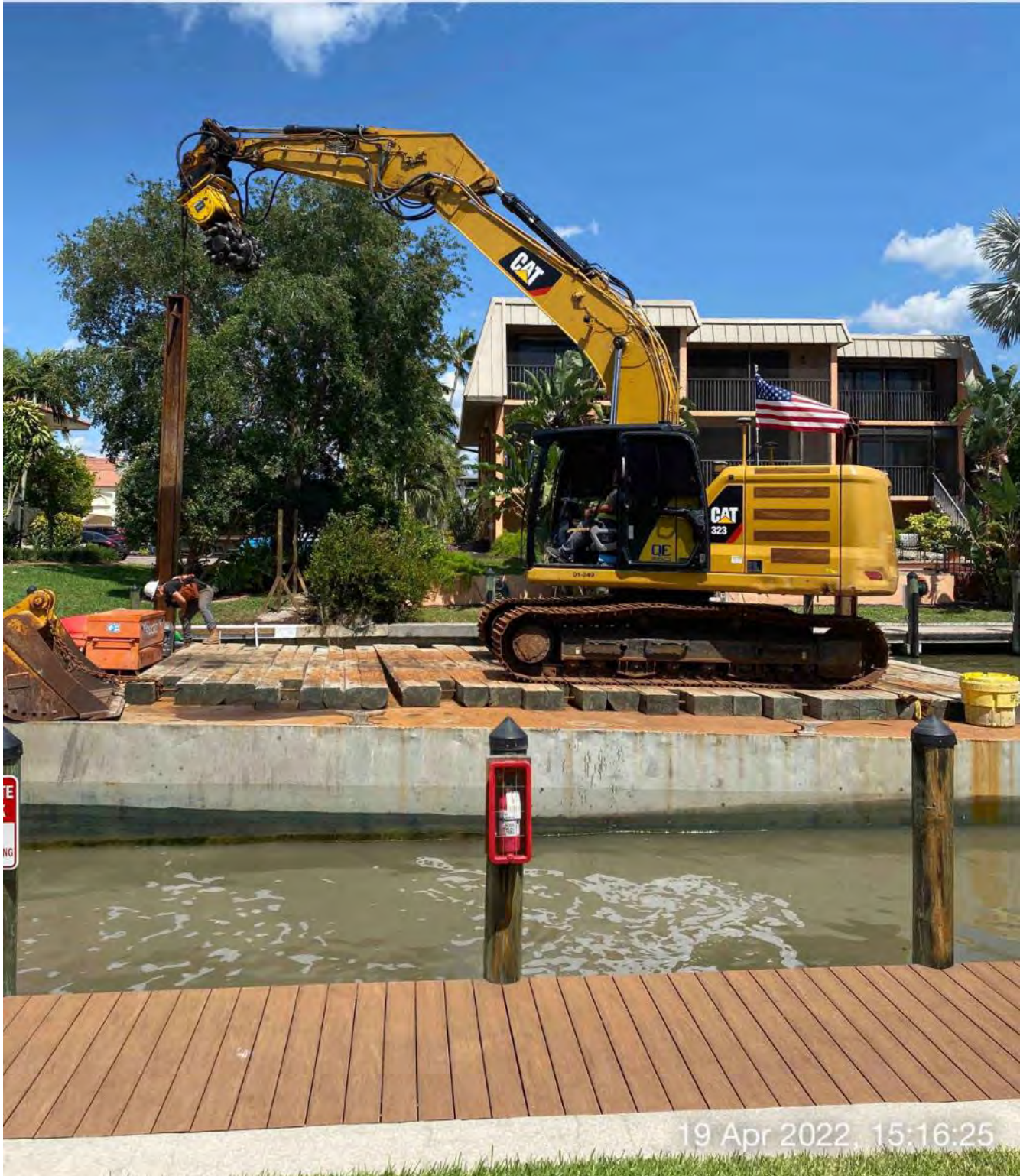
323 excavator lifting spud to allow push boat to mobilize barge in Canal Z-Z at station 3+50
