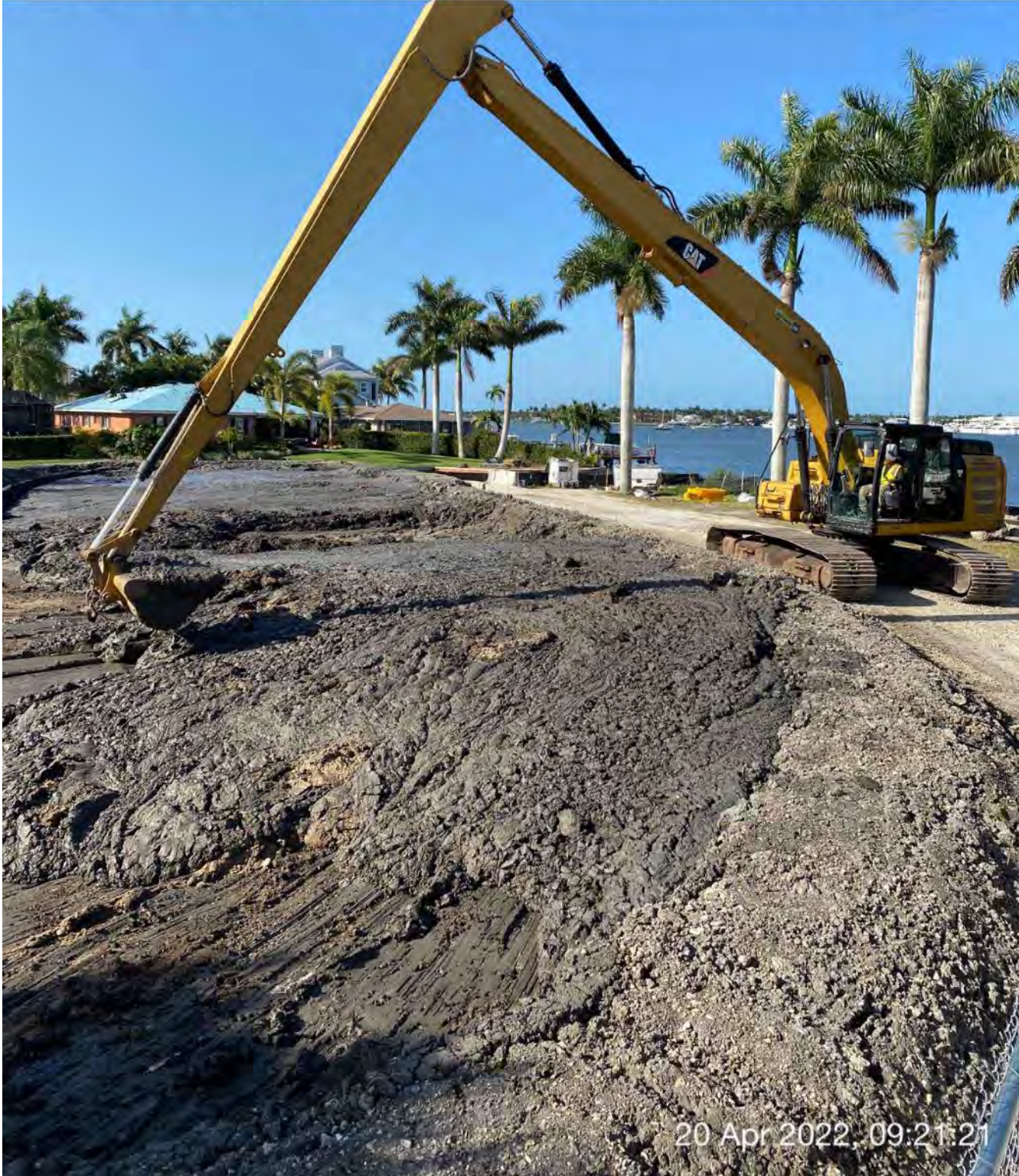
326 excavator removing material from dewatering site at 1300 Curlew Avenue
