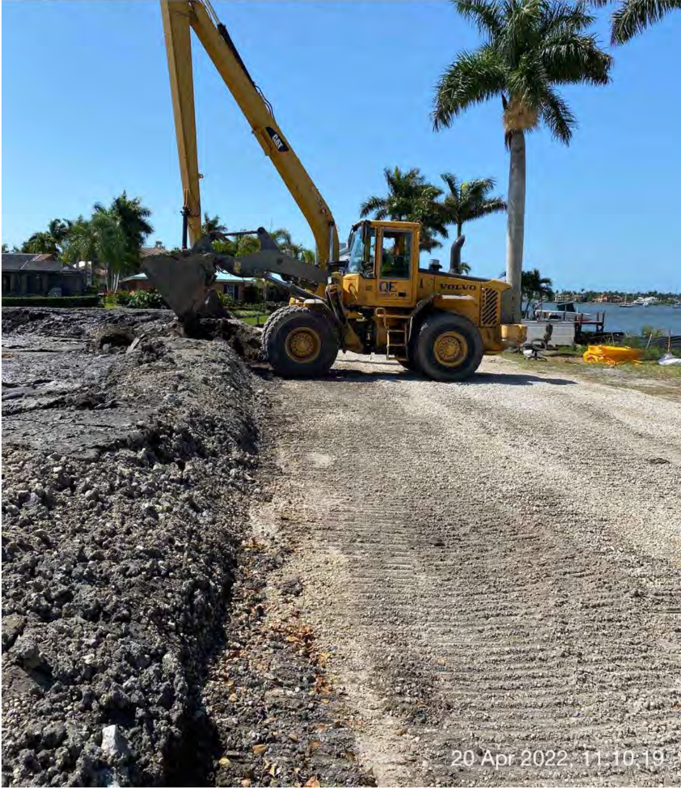
Front end loader redistributing removed material at 1300 Curlew Avenue
