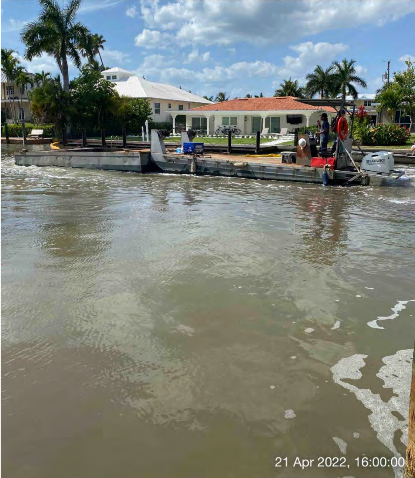
Support boat opening turbidity curtain to allow push boat to transport full hopper to Canal CC-CC
