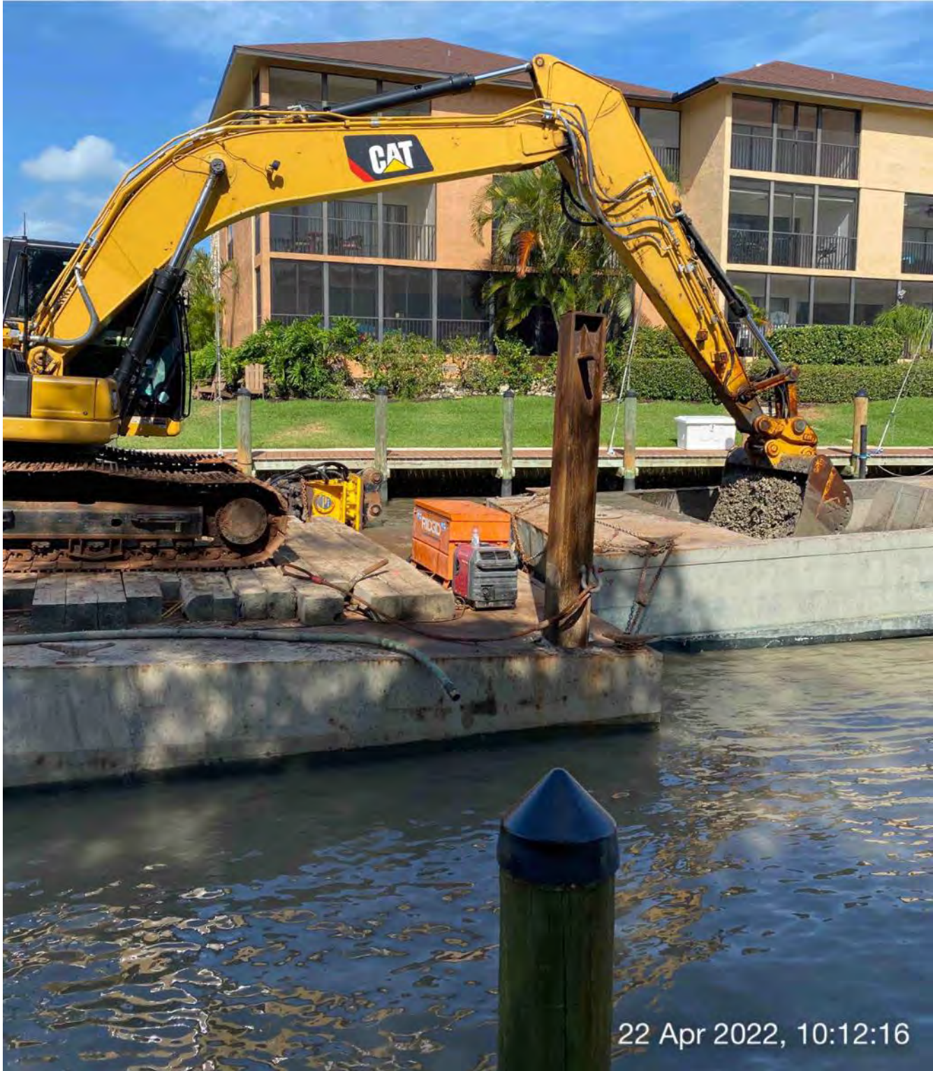
323 excavator removing material from station 2+75 and transferring it to hopper
