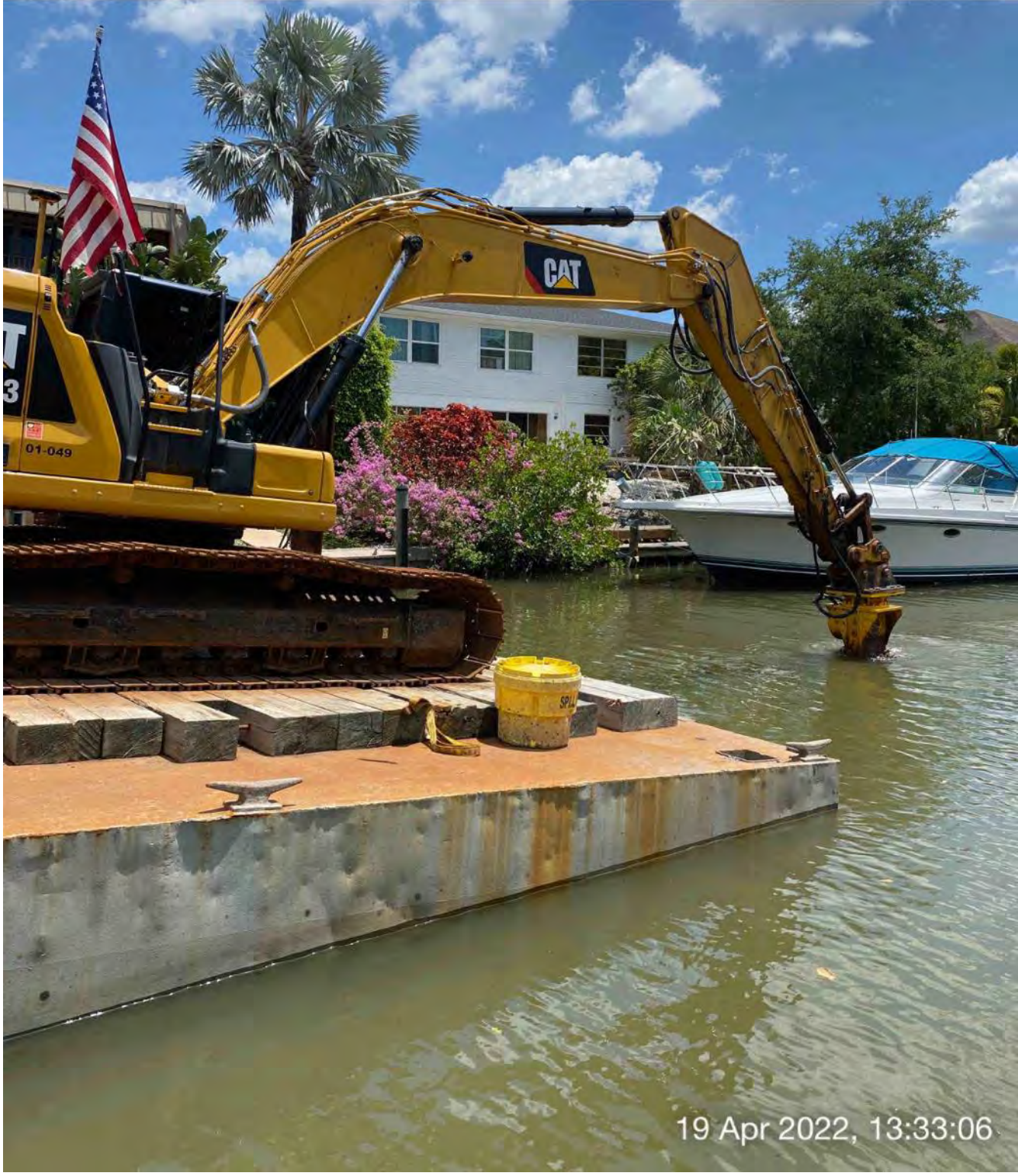
323 excavator grinding rock in Canal Z-Z at station 3+75
