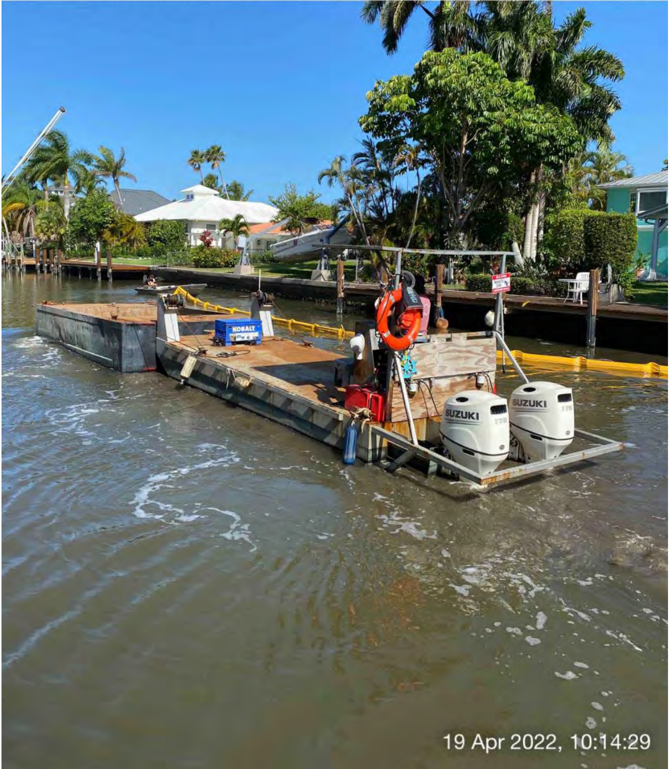
Support boat opening turbidity curtain to allow push boat to transport hopper to Canal CC-CC
