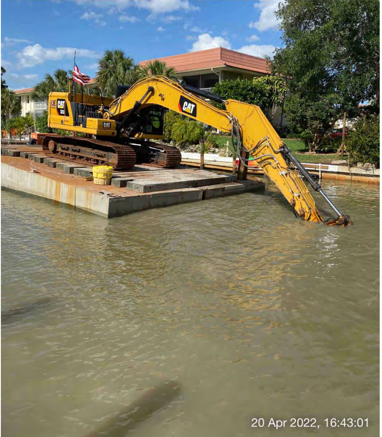
323 excavator grinding material at station 2+50
