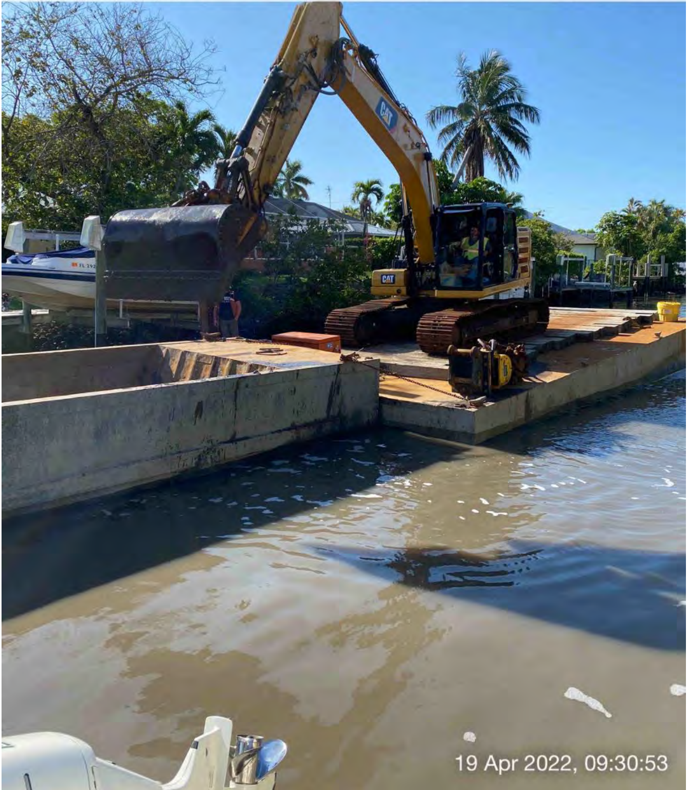
323 excavator removing material and transferring it to hopper in Canal AA-AA at station 3+00
