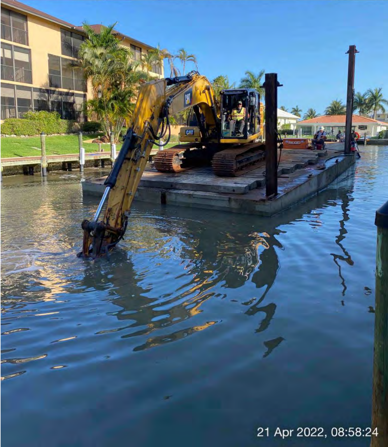
323 excavator grinding material at station 2+00
