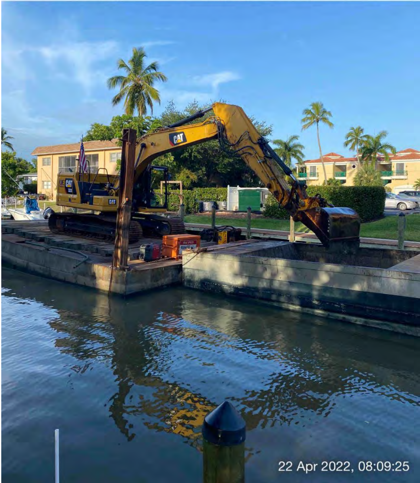
323 excavator removing material from station 3+25 and transferring it to hopper
