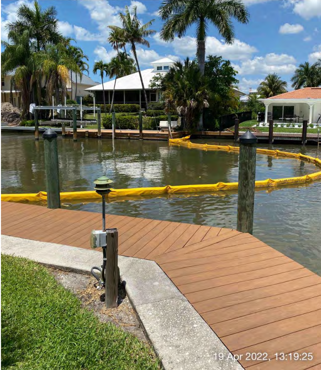
Turbidity curtain installed in Canal X-X at station 8+50
