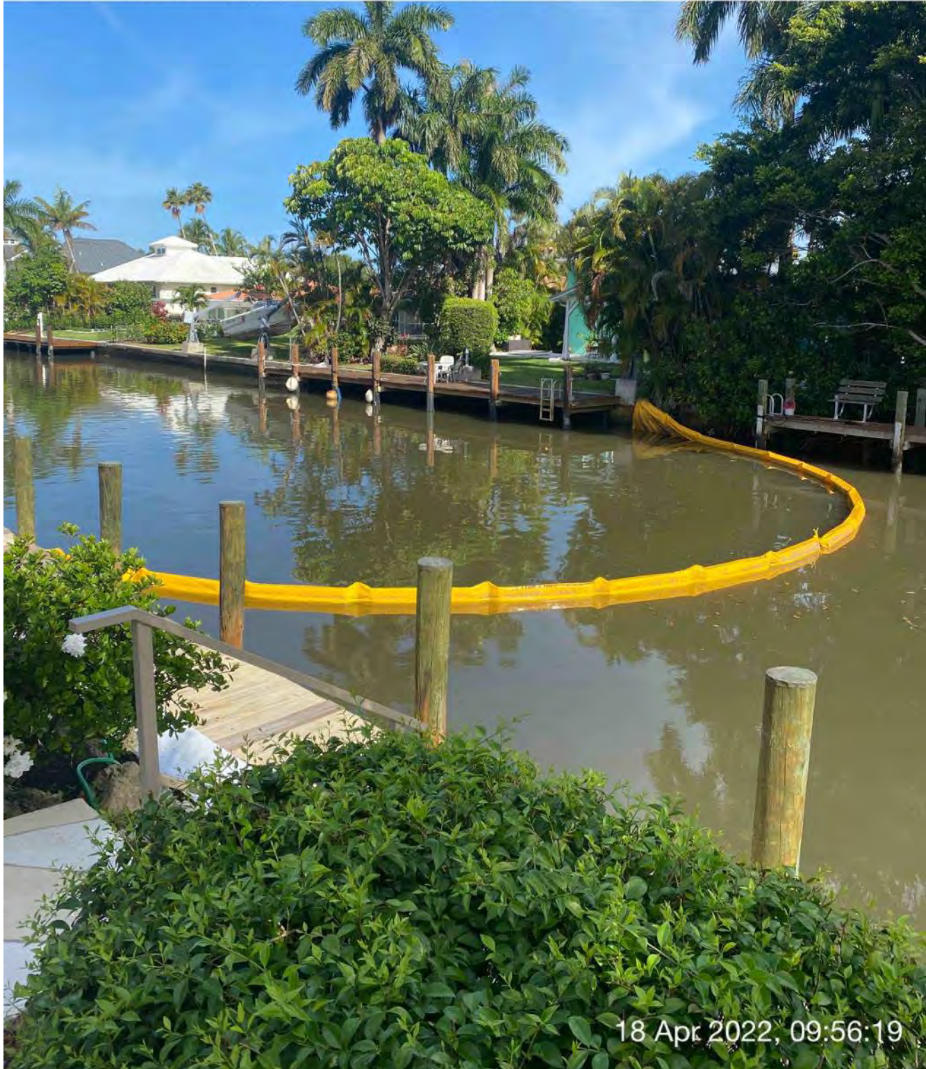
Turbidity curtain installed in Canal X-X at station 11+00
