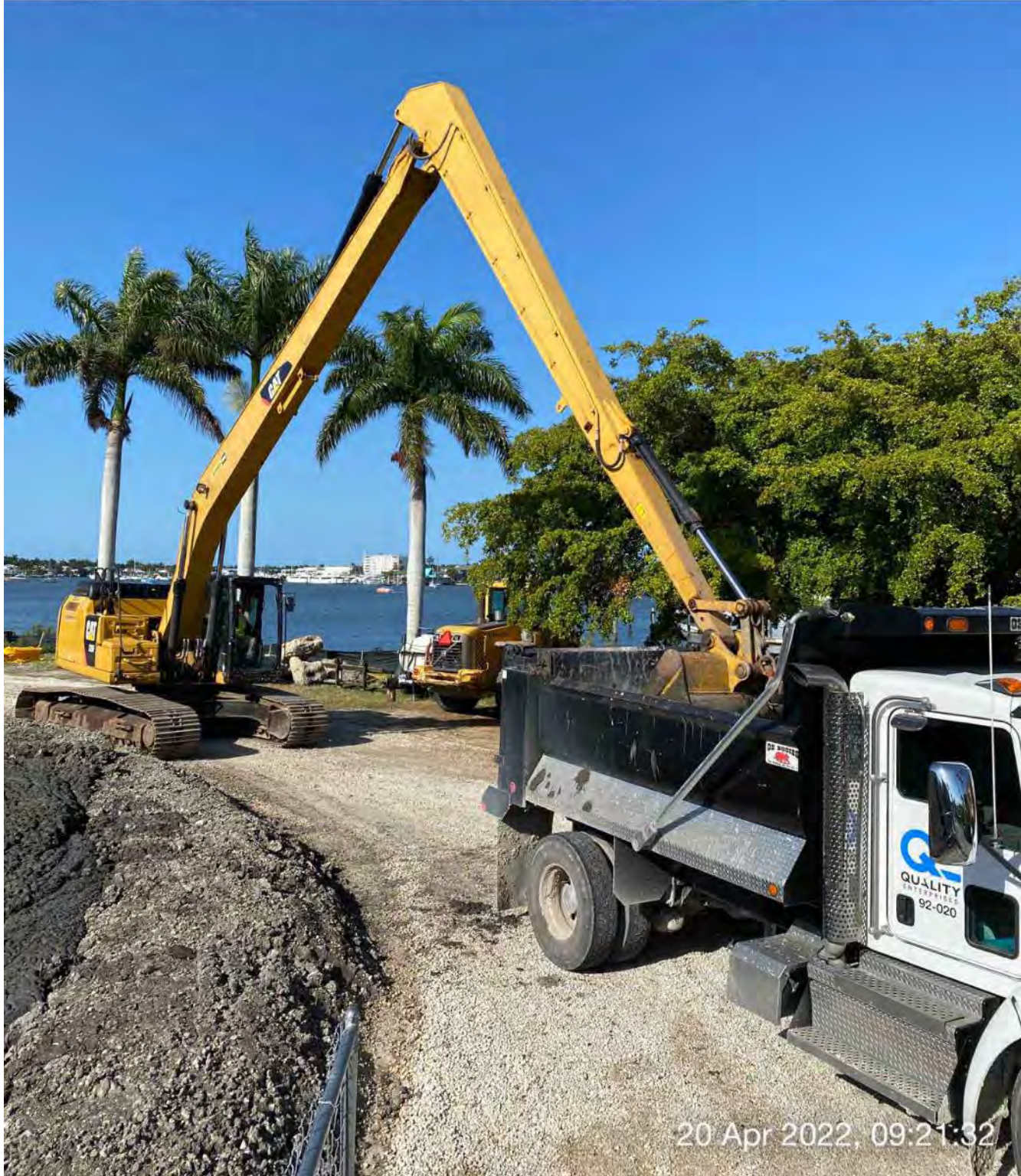
326 excavator transferring removed material to dump truck bed at 1300 Curlew Avenue
