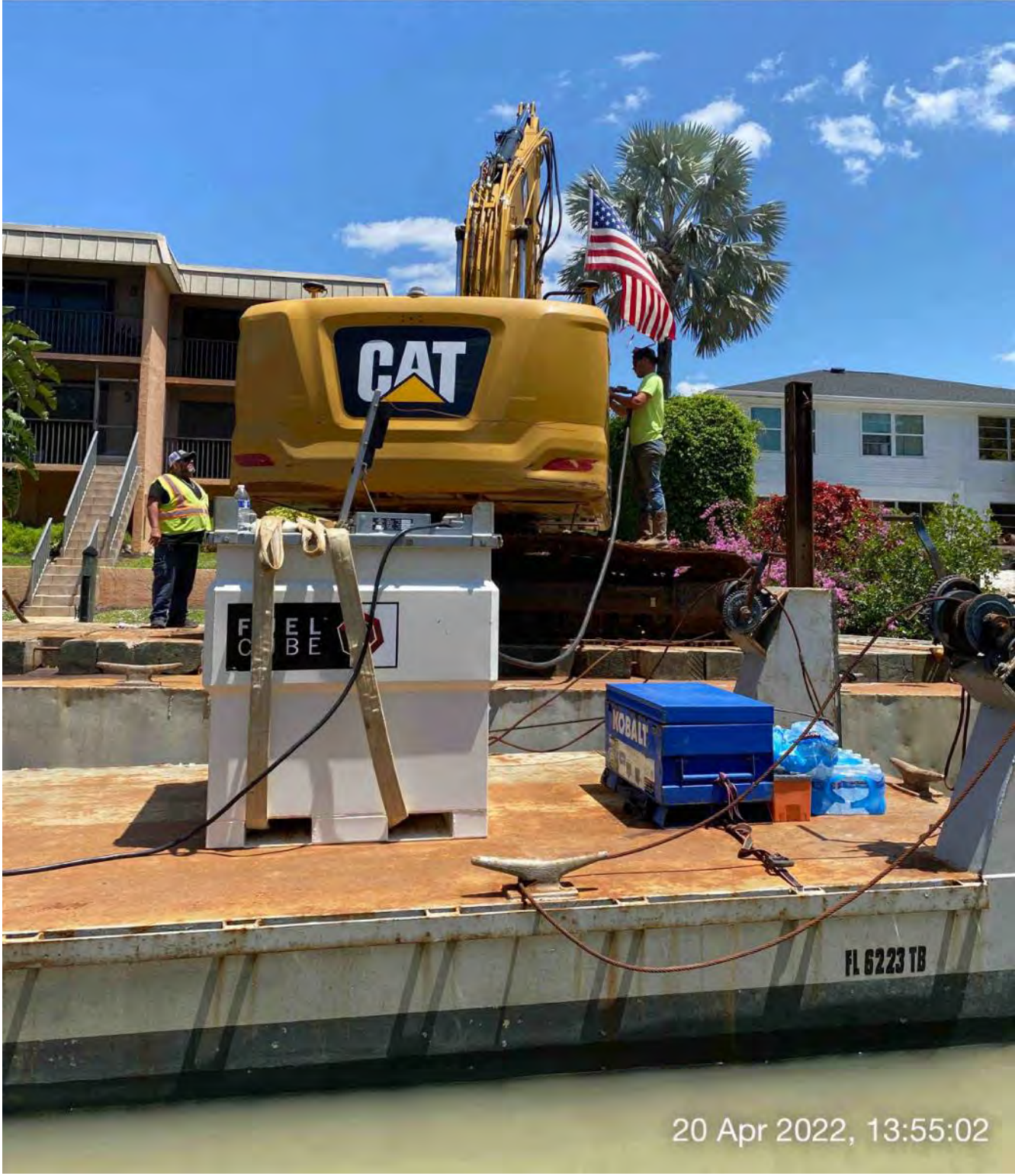
Contractor using fuel cube to refuel 323 excavator at station 3+00
