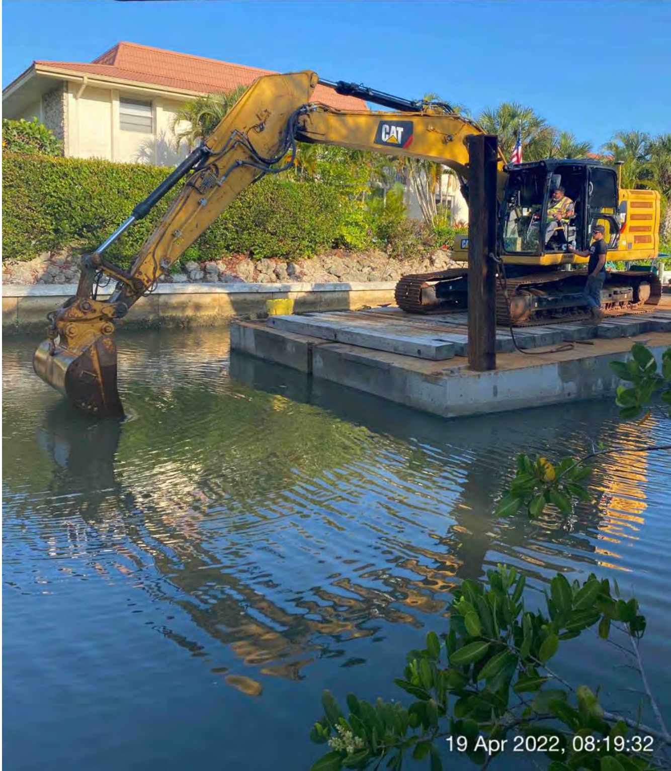
323 excavator removing material from Canal AA-AA at station 2+00
