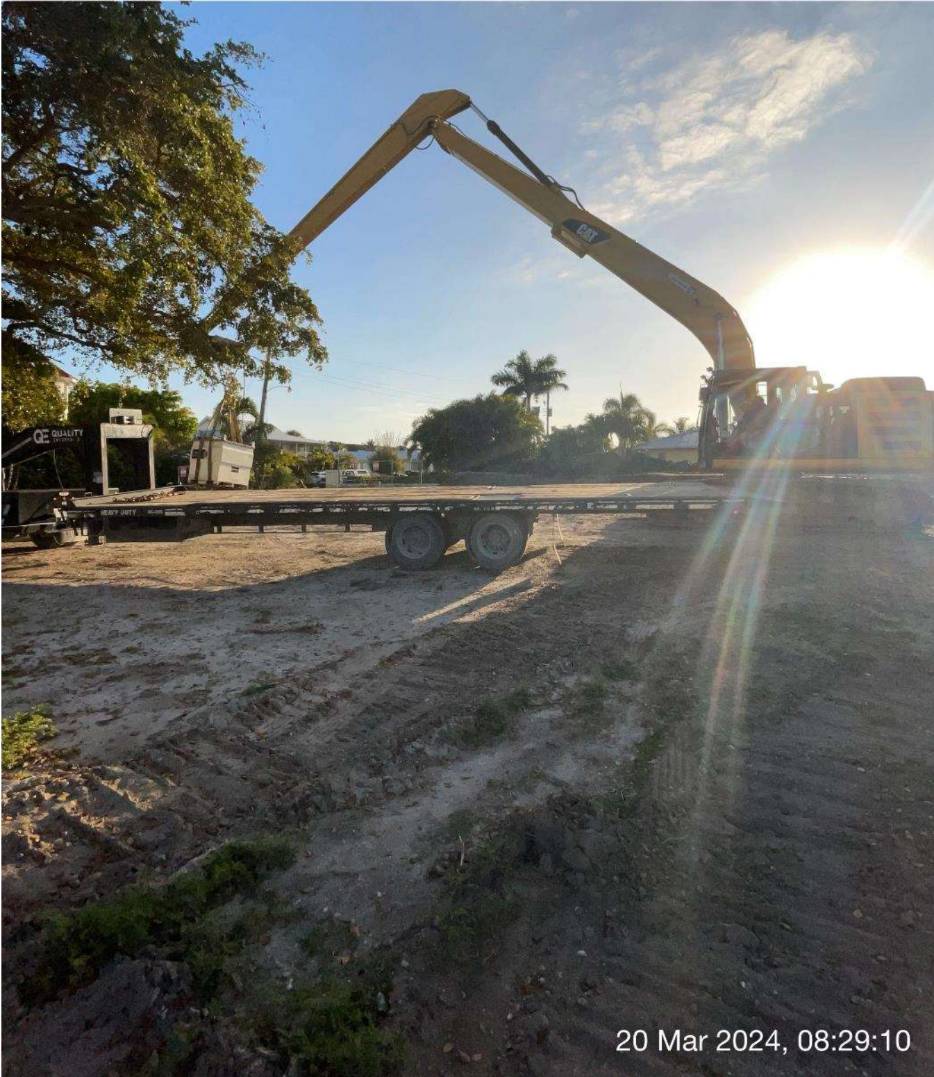
Long reach excavator moving fuel cube to be filled.
