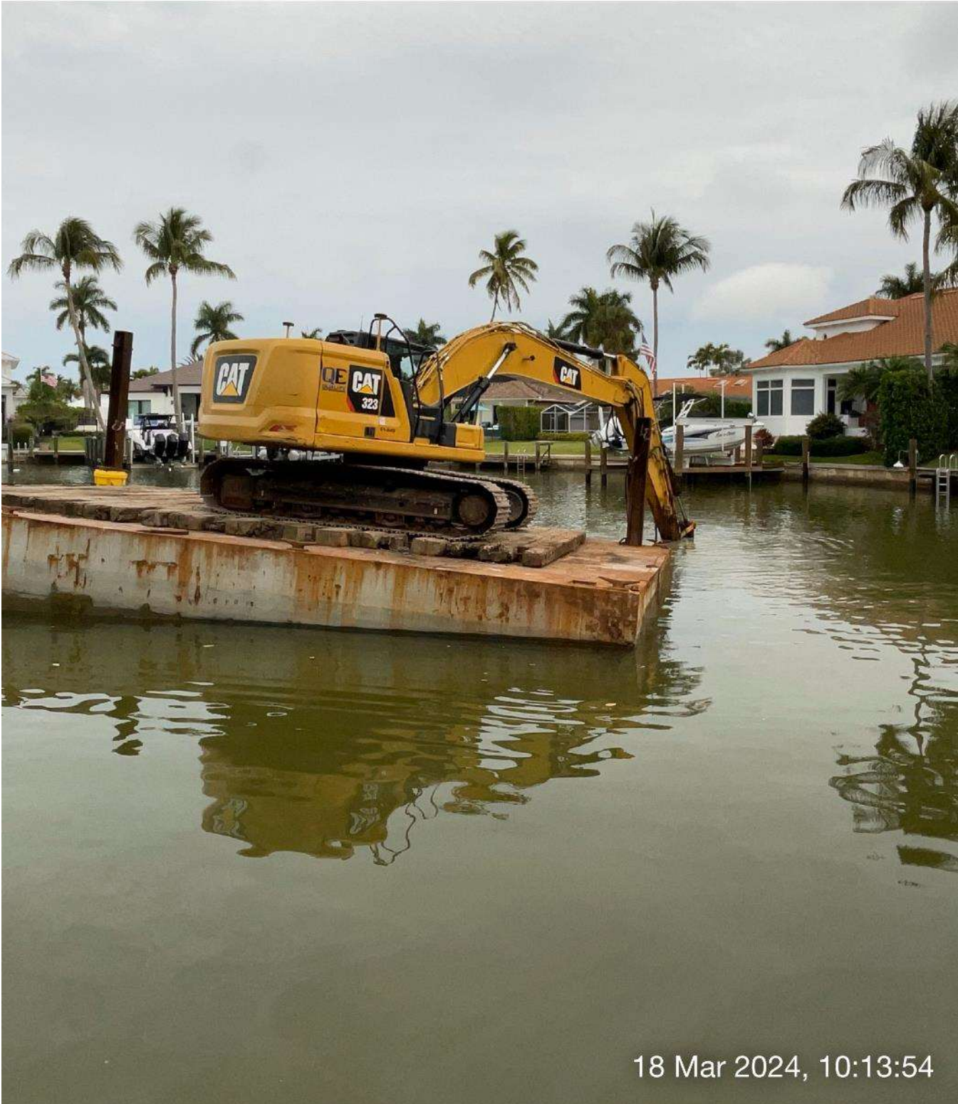
323 excavator grinding rock at station 13+50 in Canal A-A.
