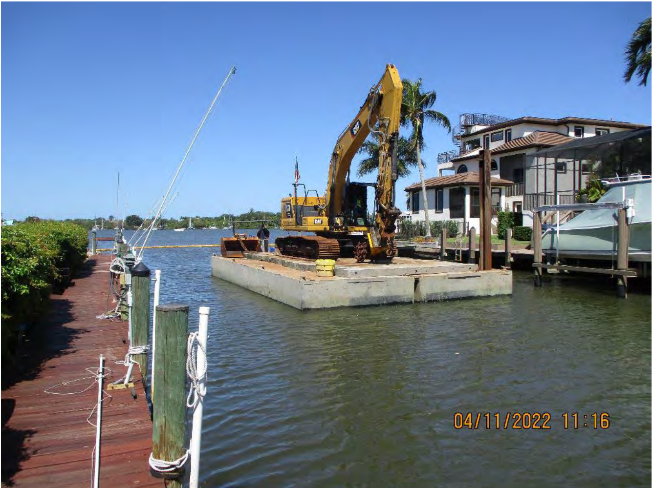
Dredging/grinding equipment at approx. station 2+50 (canal X-X)
