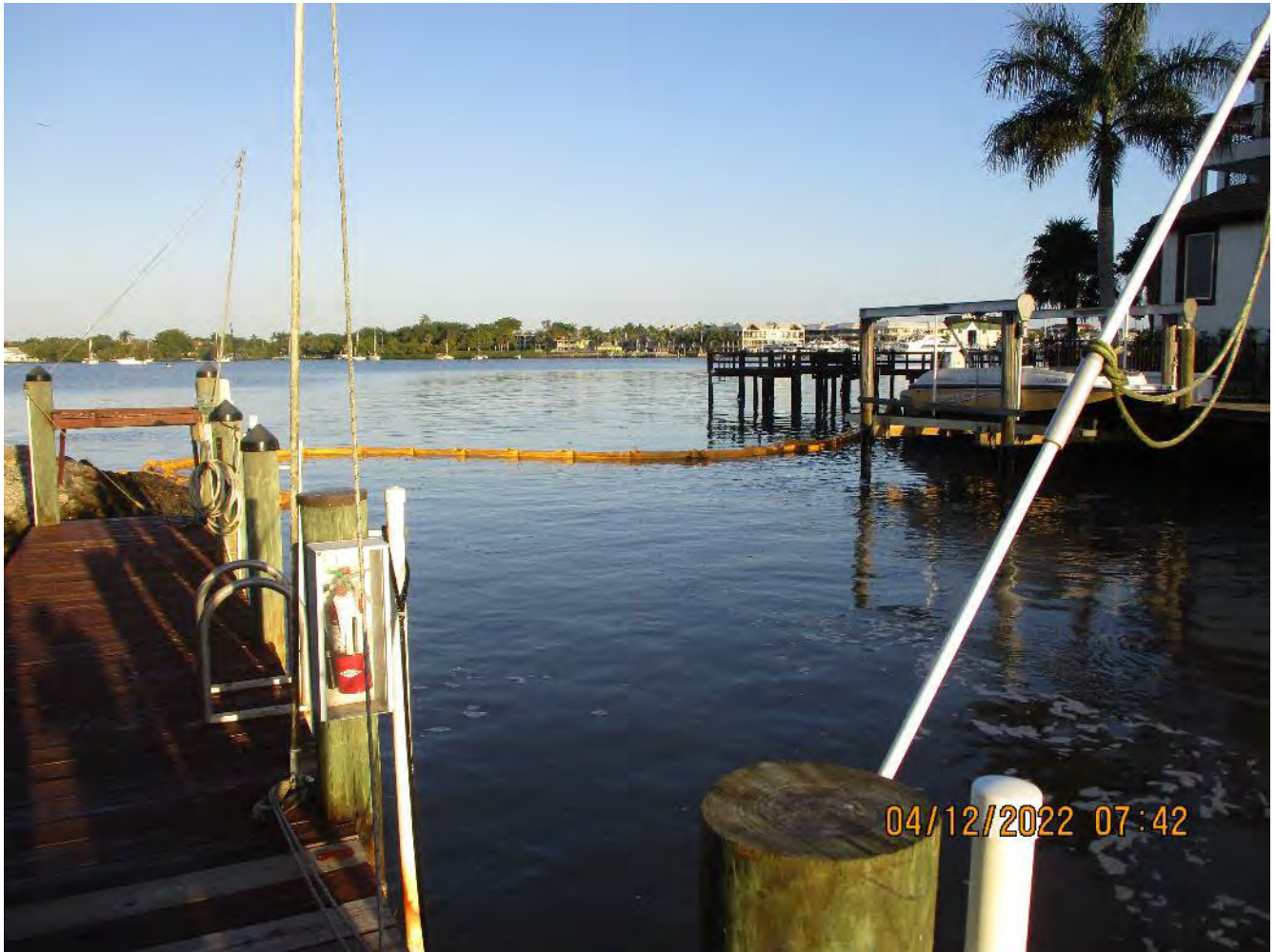
Turbidity curtain across mouth of Canal X-X
