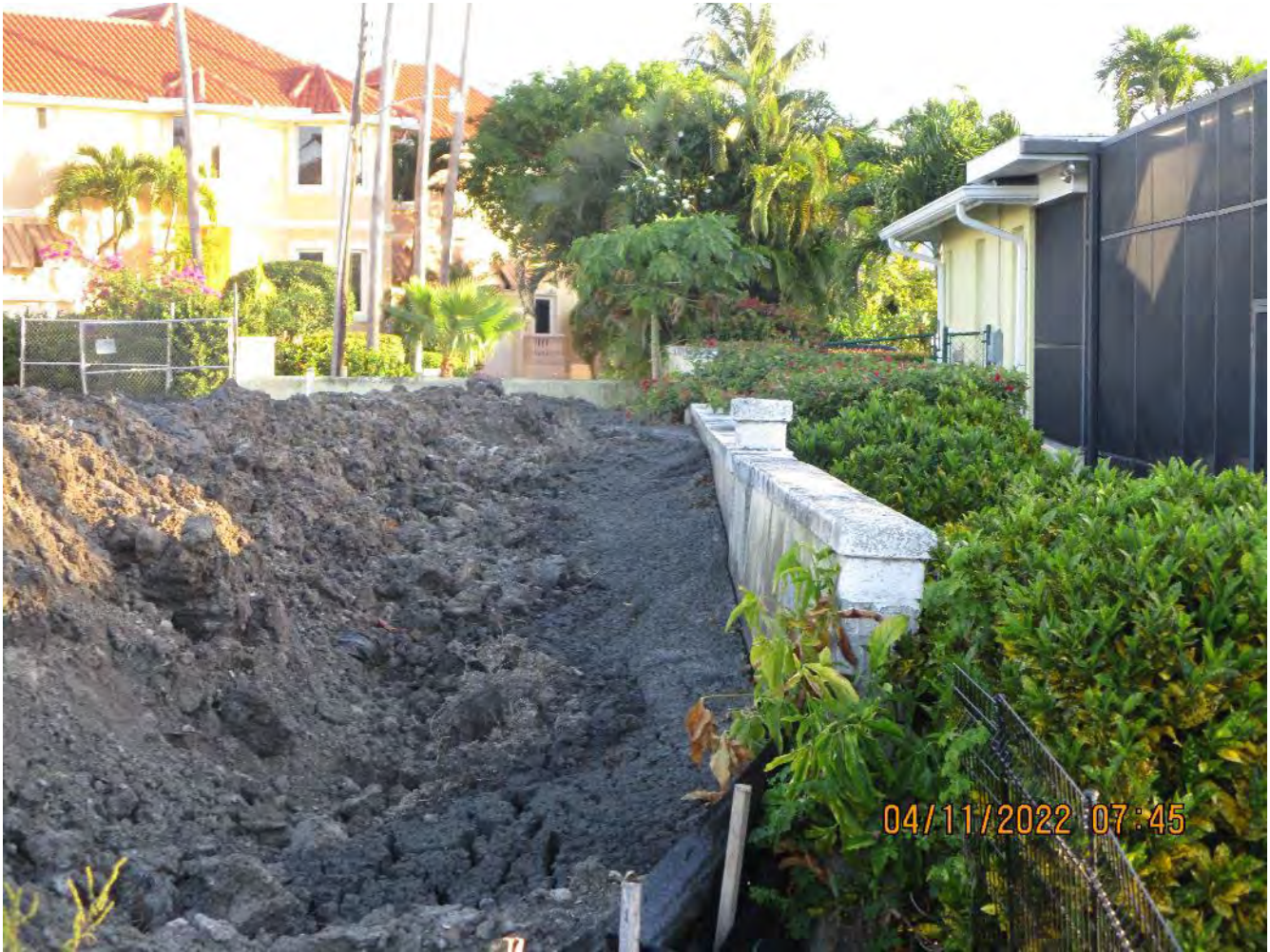
Retaining wall between 1300/1350 Curlew Ave.
