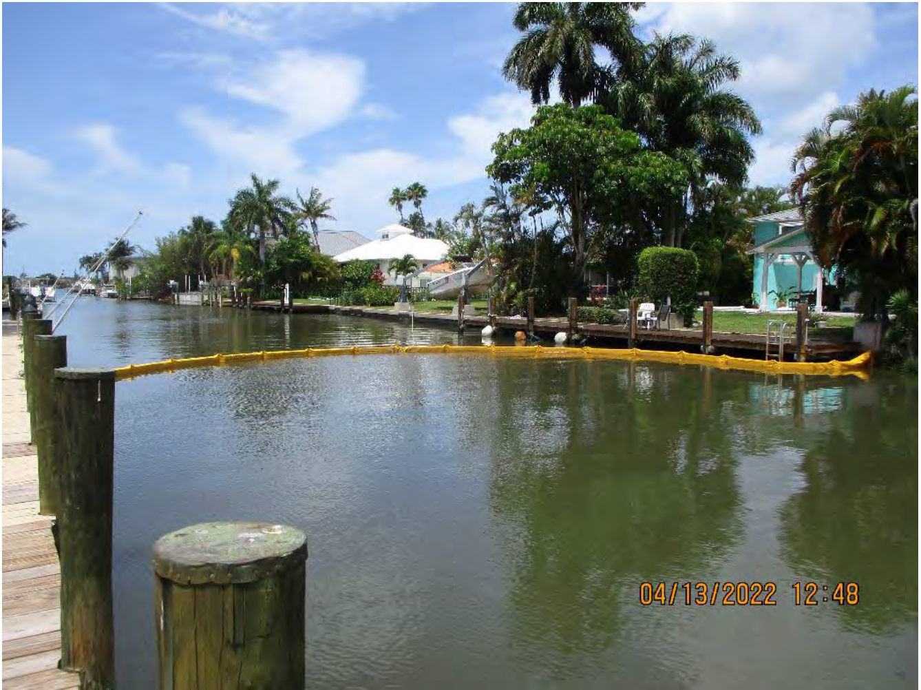
Turbidity curtain in place at approx. station 11+00 (canal X-X)
