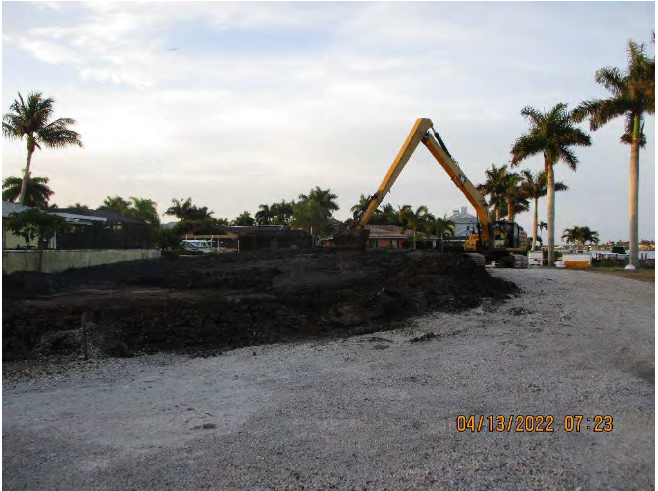
Current status of project dredging material stockpile (1300 Curlew Ave.)
