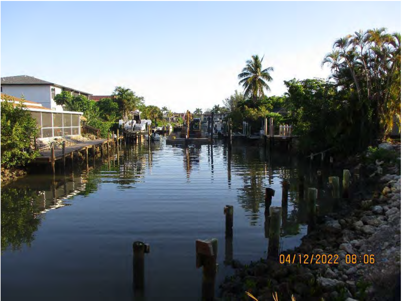
Start location for todays bottom grinding (approx. sta. 3+00, canal AA-AA)
