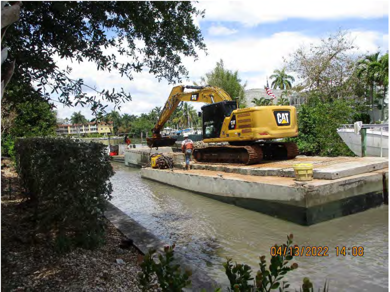
Dredged material from canal AA-AA being emptied into hopper
