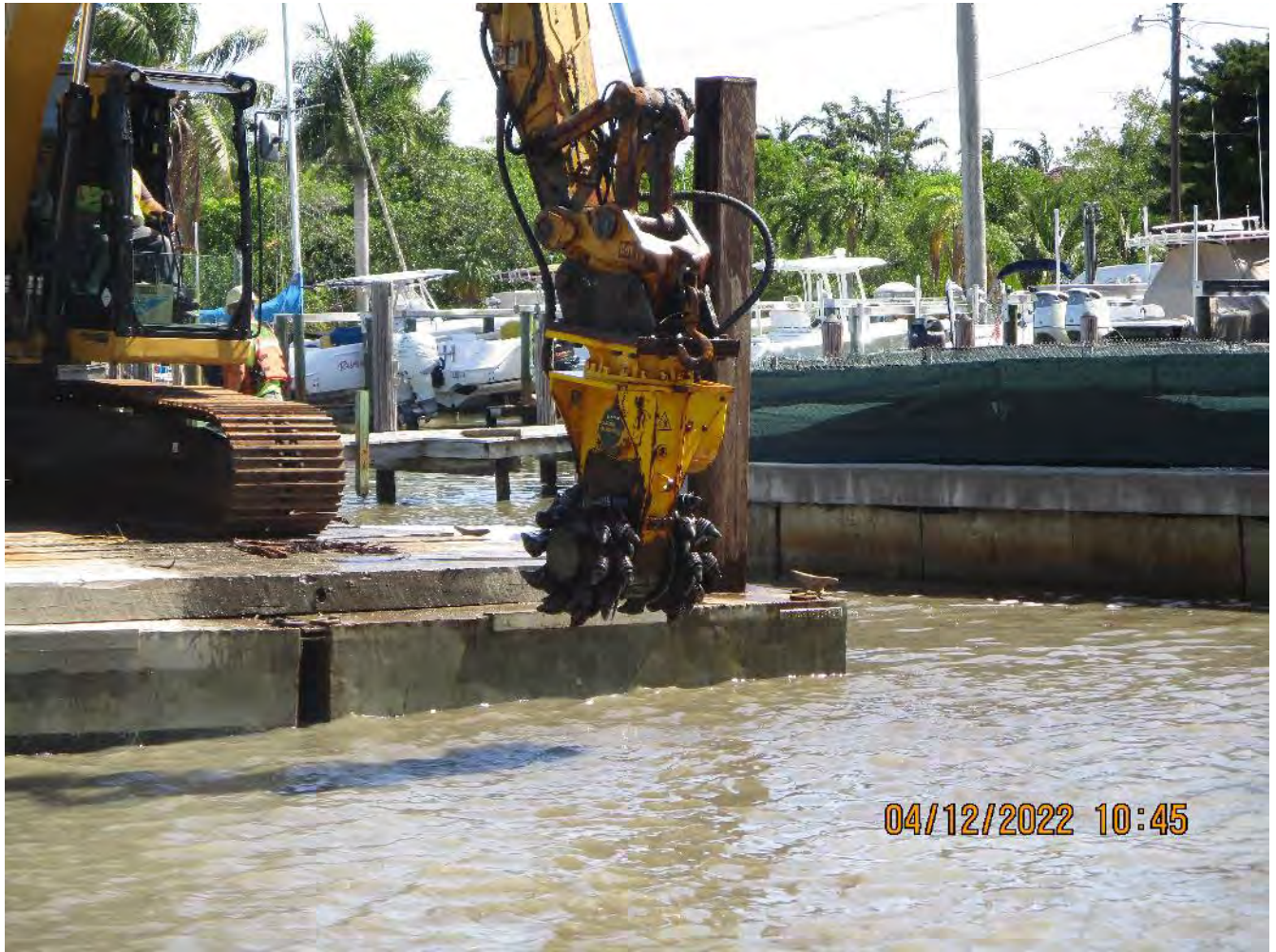
Epiroc grinder head being utilized today
