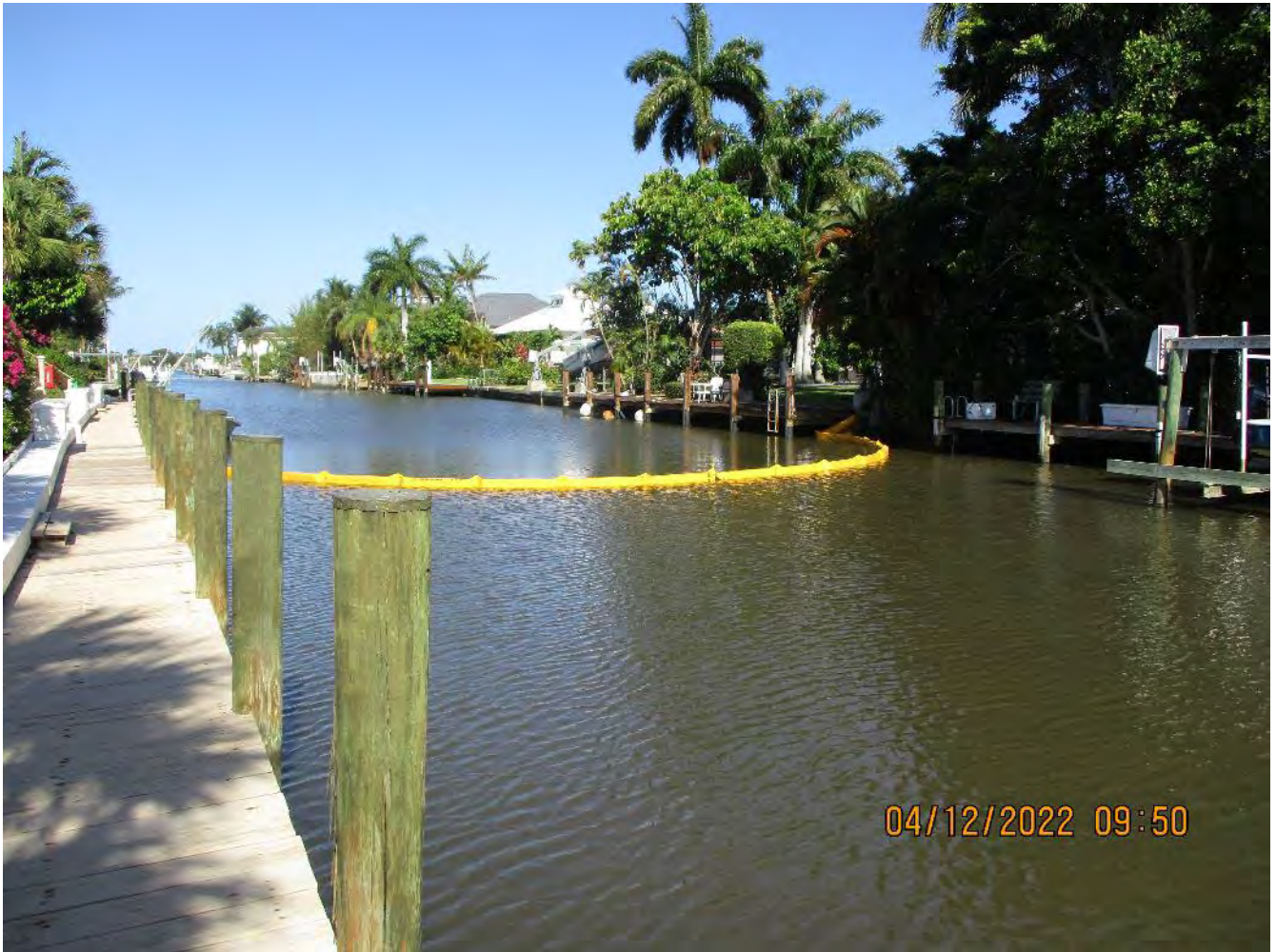
Relocated turbidity curtain location (approx. sta. 11+00, canal X-X)
