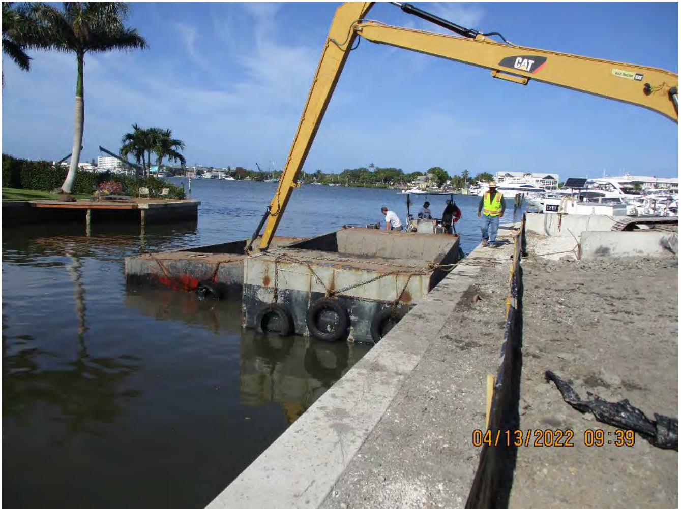
Dropping off full hopper and picking up empty hopper
