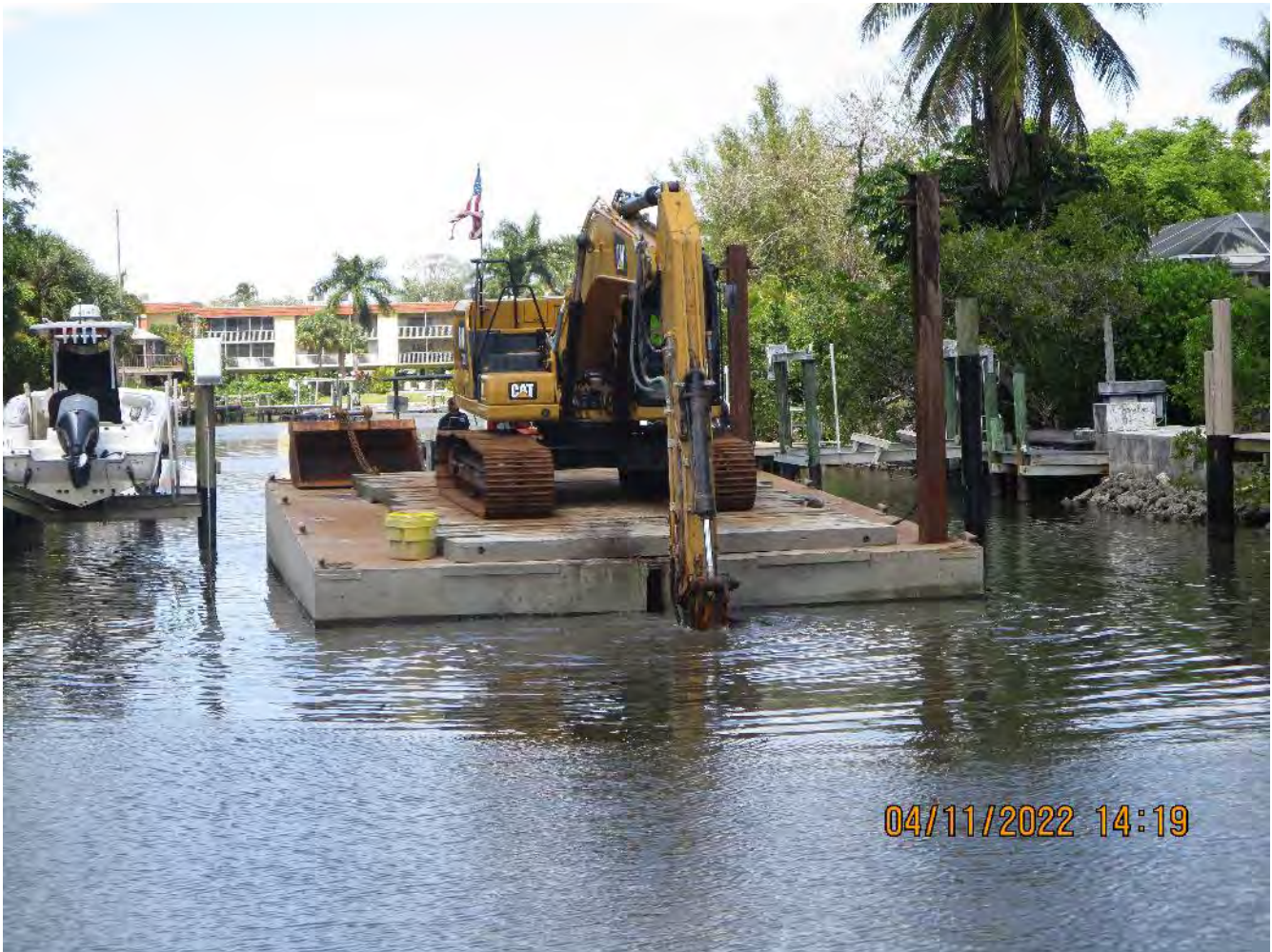
Canal bottom grinding in progress at approx. station 4+00 (canal AA-AA)
