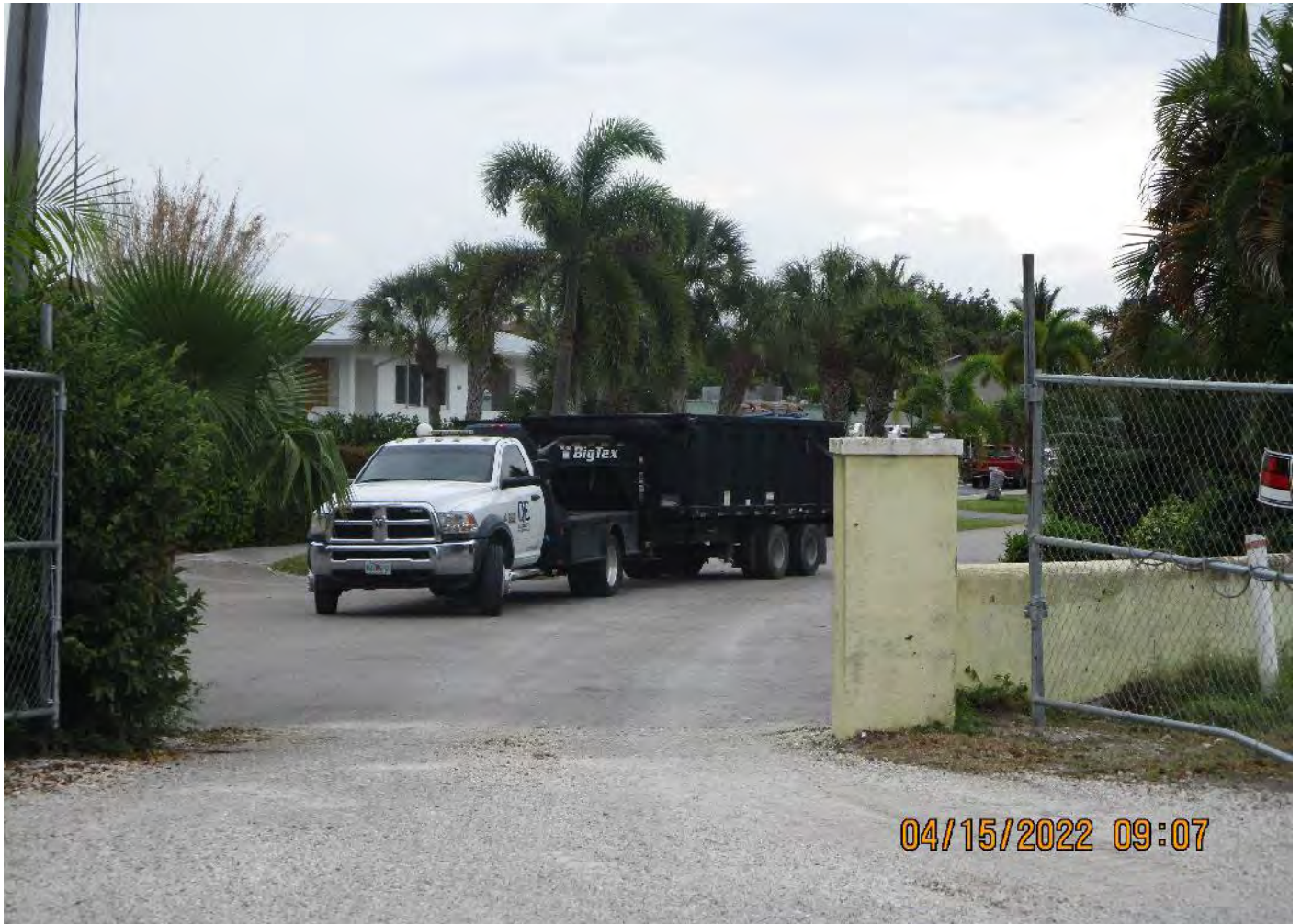
Dump truck entering the site at 1300 Curlew Avenue
