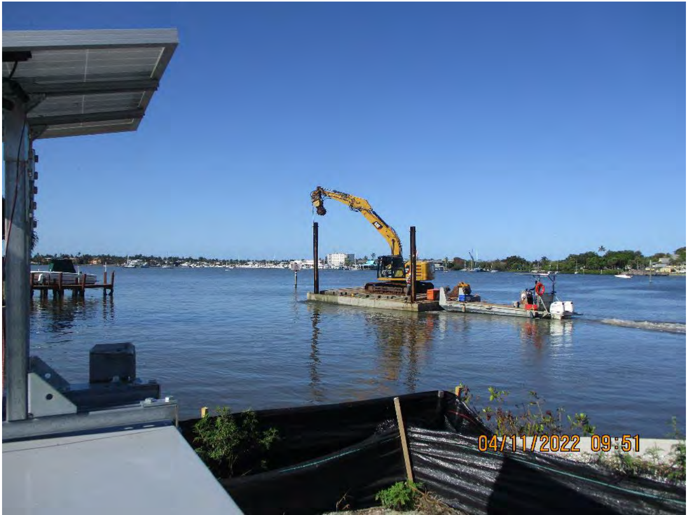
Dredging/grinding equipment heading towards canal X-X
