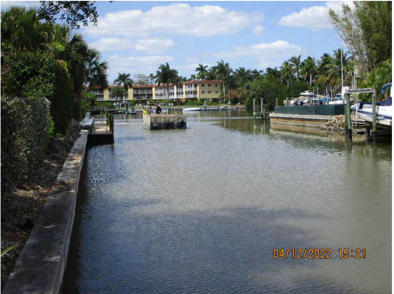
Push boat bringing back recently emptied hopper to canal AA-AA
