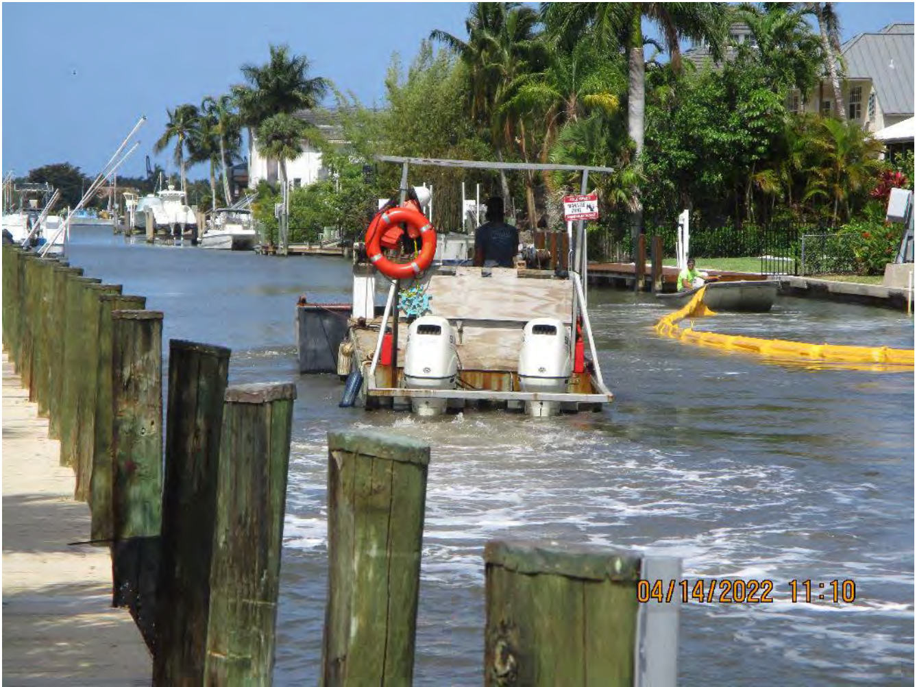
Pushing hopper containing dredged material to 1300 Curlew Ave. location
