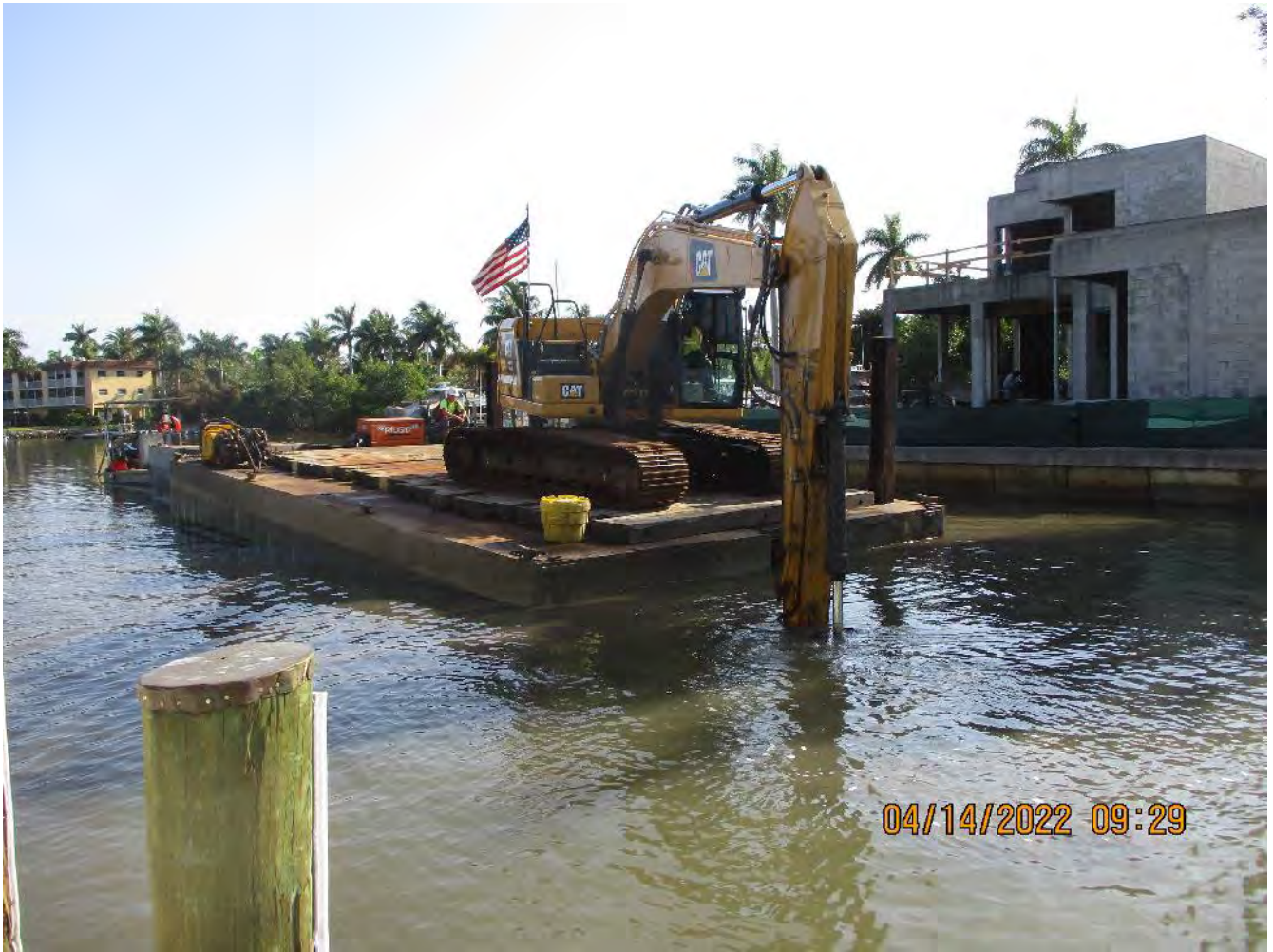
Dredging in progress at approx. station 1+00, canal AA-AA
