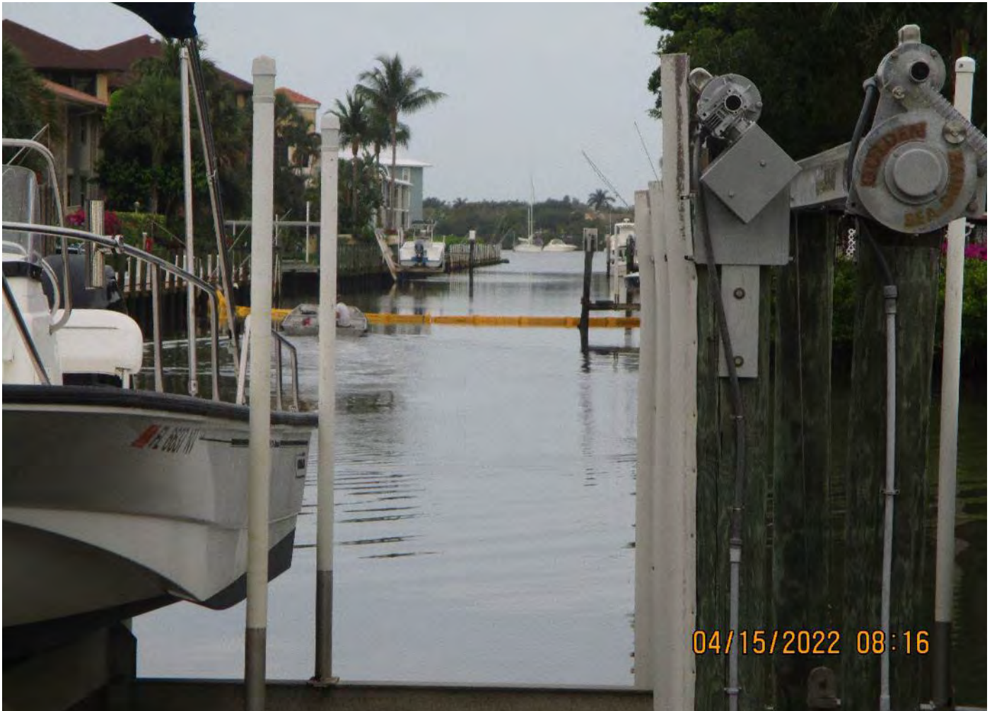
Turbidity curtain installed across Canal X-X at station 13+00
