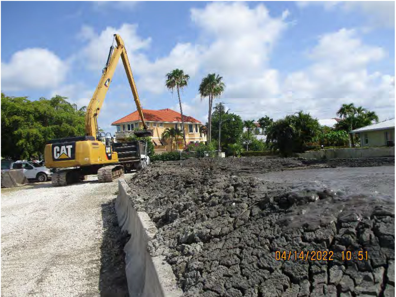
Loading stockpile dredged material into dump truck
