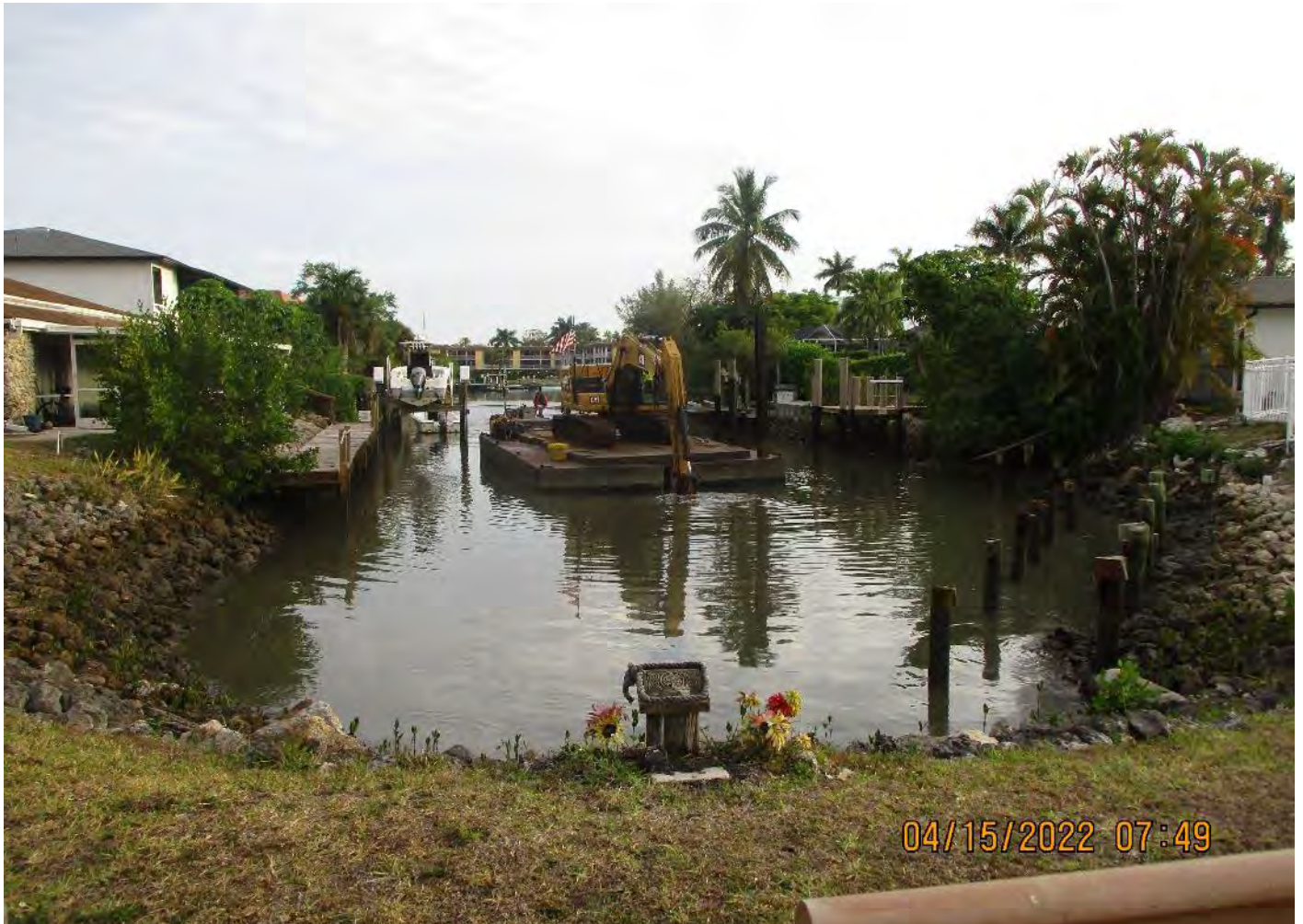
323 excavator removing material and transferring to hopper at station 4+00
