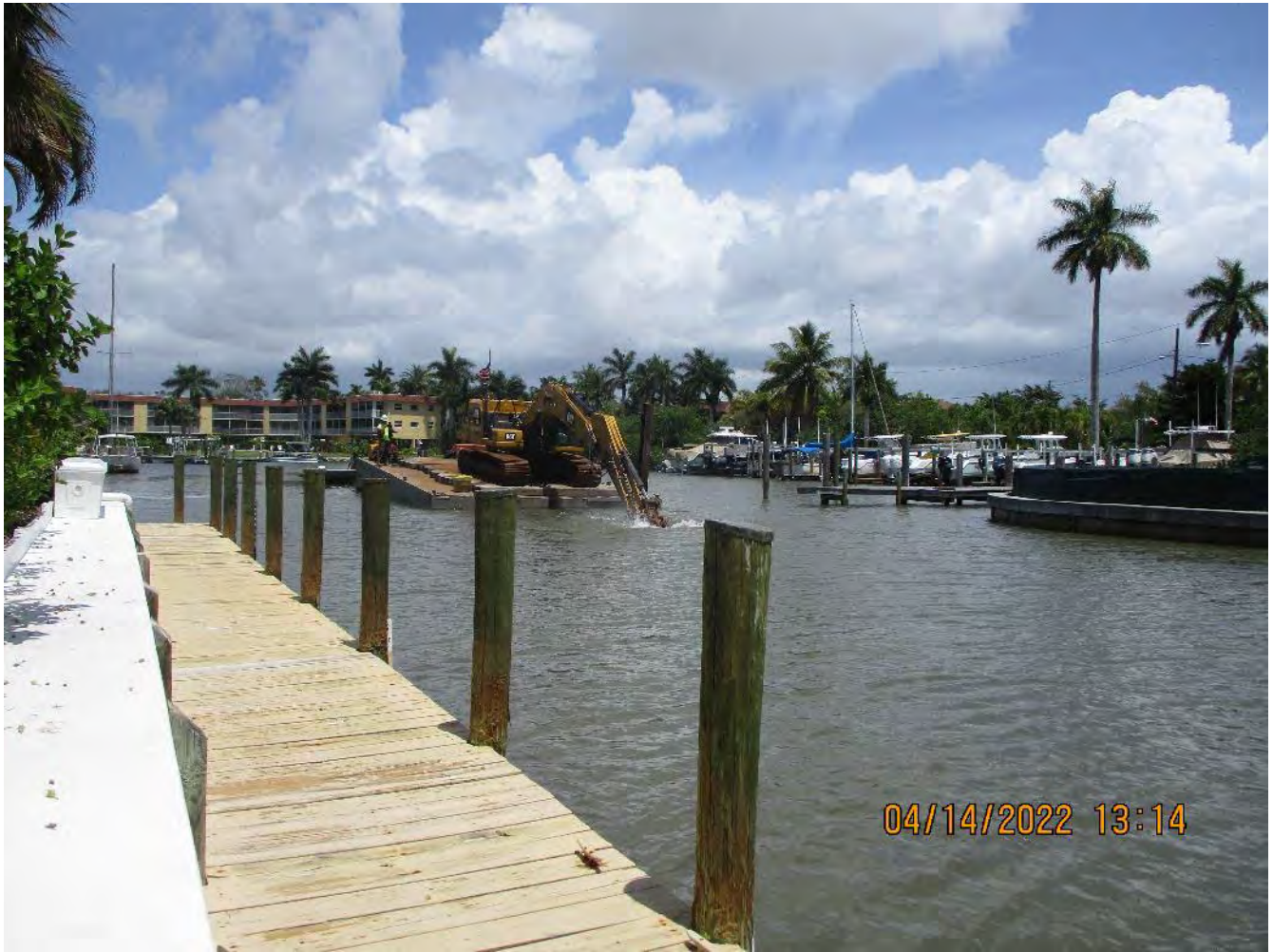
Dredging in progress at north mouth of Canal AA-AA
