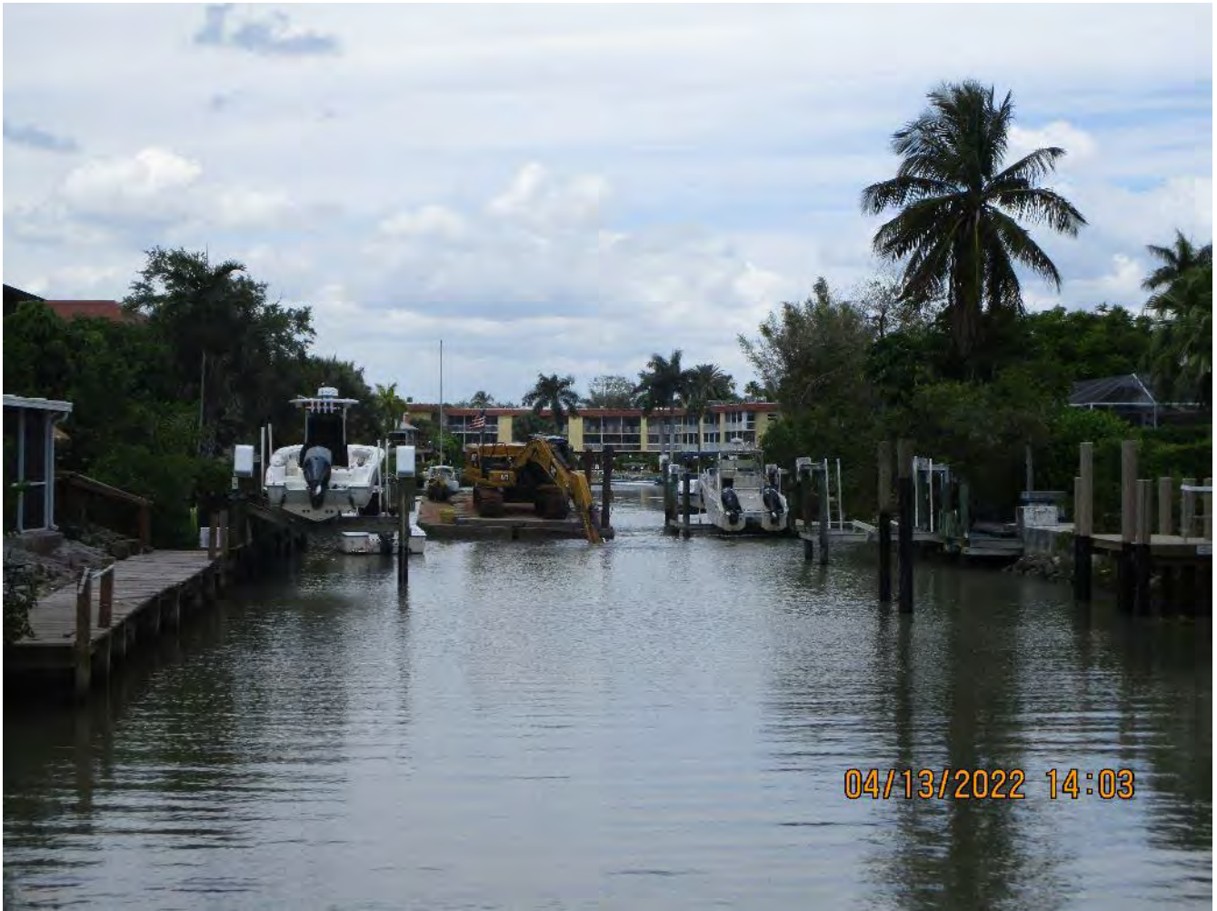
Dredging in progress (approx. station 2+50, canal AA-AA)
