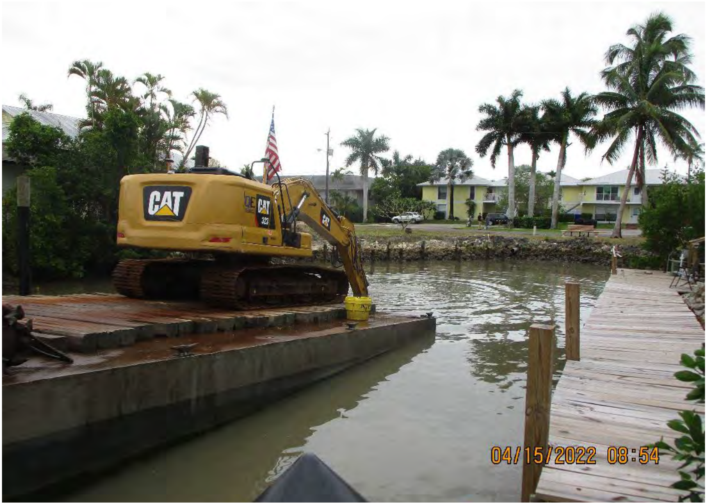
323 excavator removing material from station 4+00
