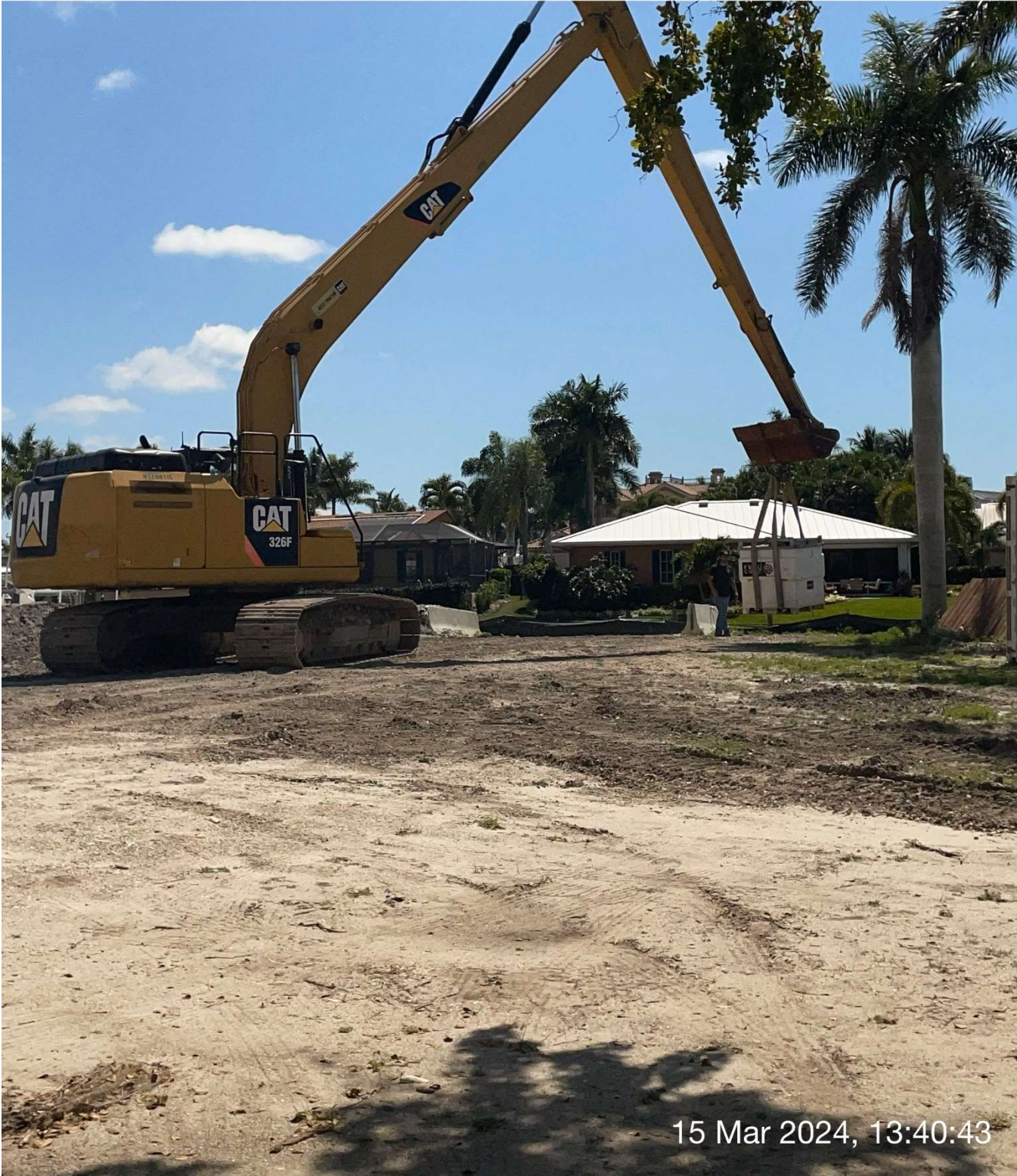
Contractor loading fuel cube into hopper.
