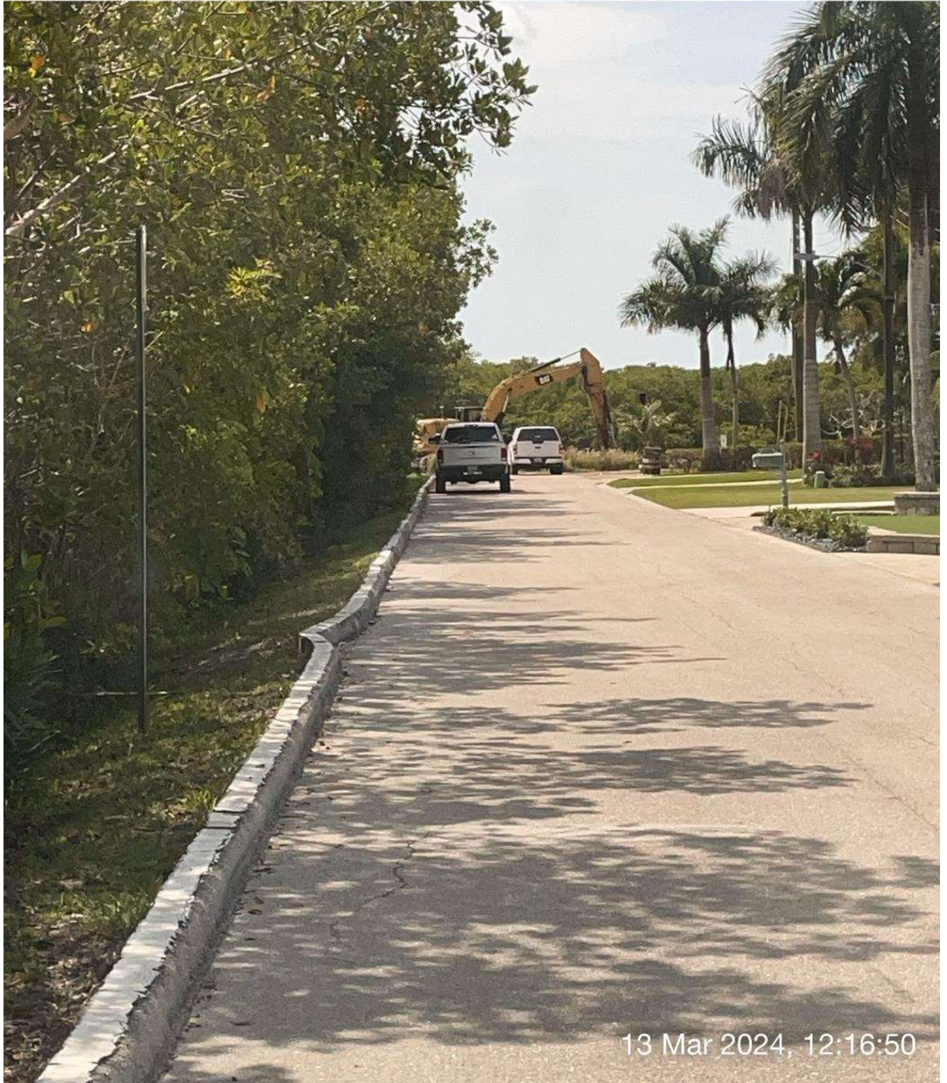
Site Tech working on GPS computer system in 323 excavator.
