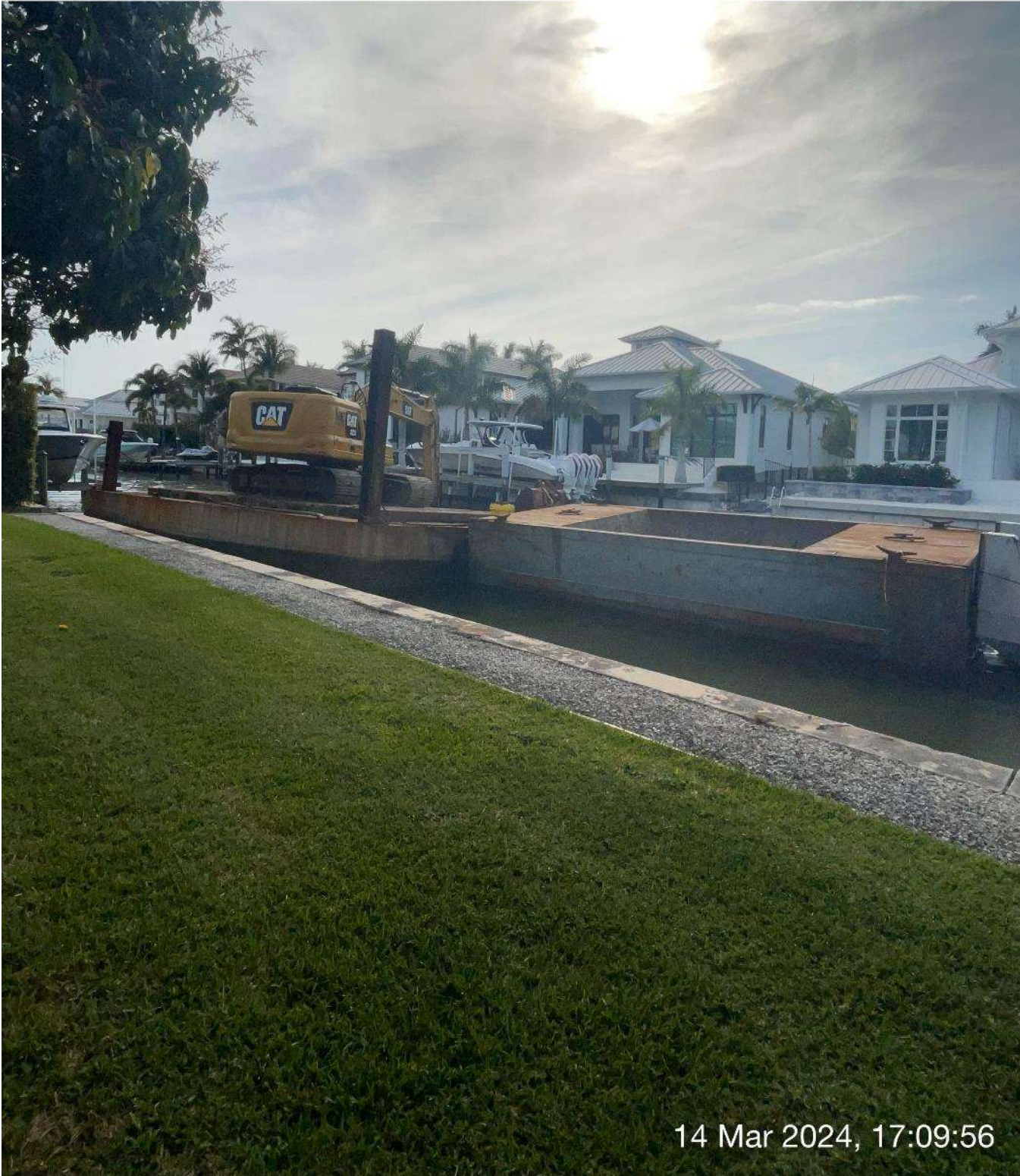
Equipment staged at station 6+00 in Canal A-A.
