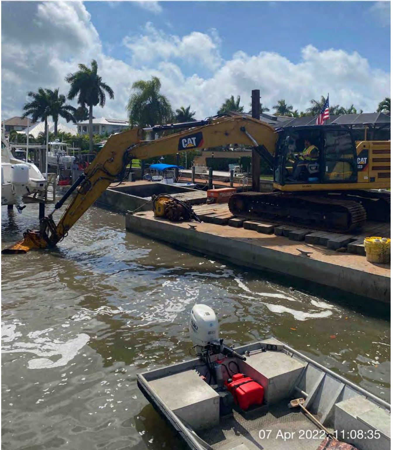
323 excavator removing material from station 2+25 and transferring to hopper
