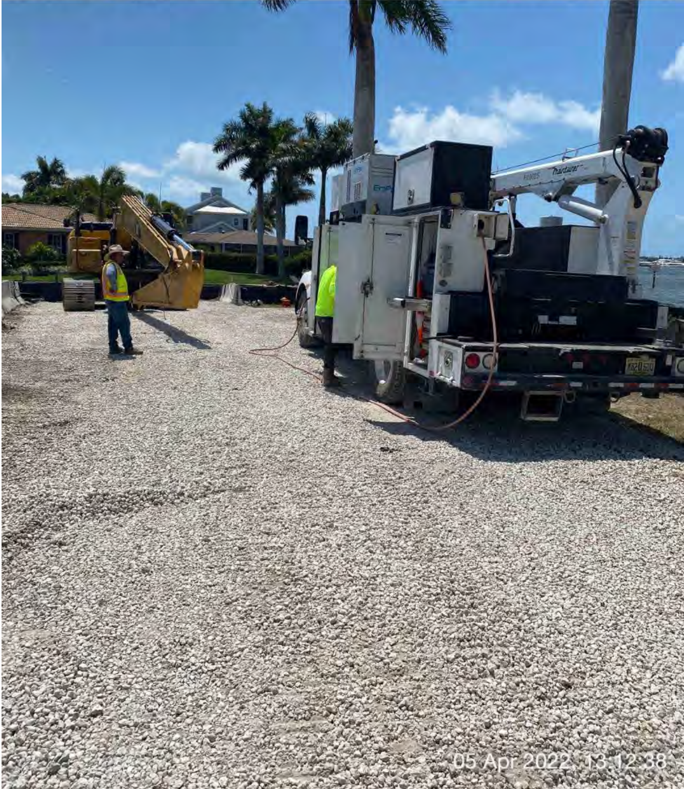
Mechanic on site at 1300 Curlew Avenue to fix 326 excavator
