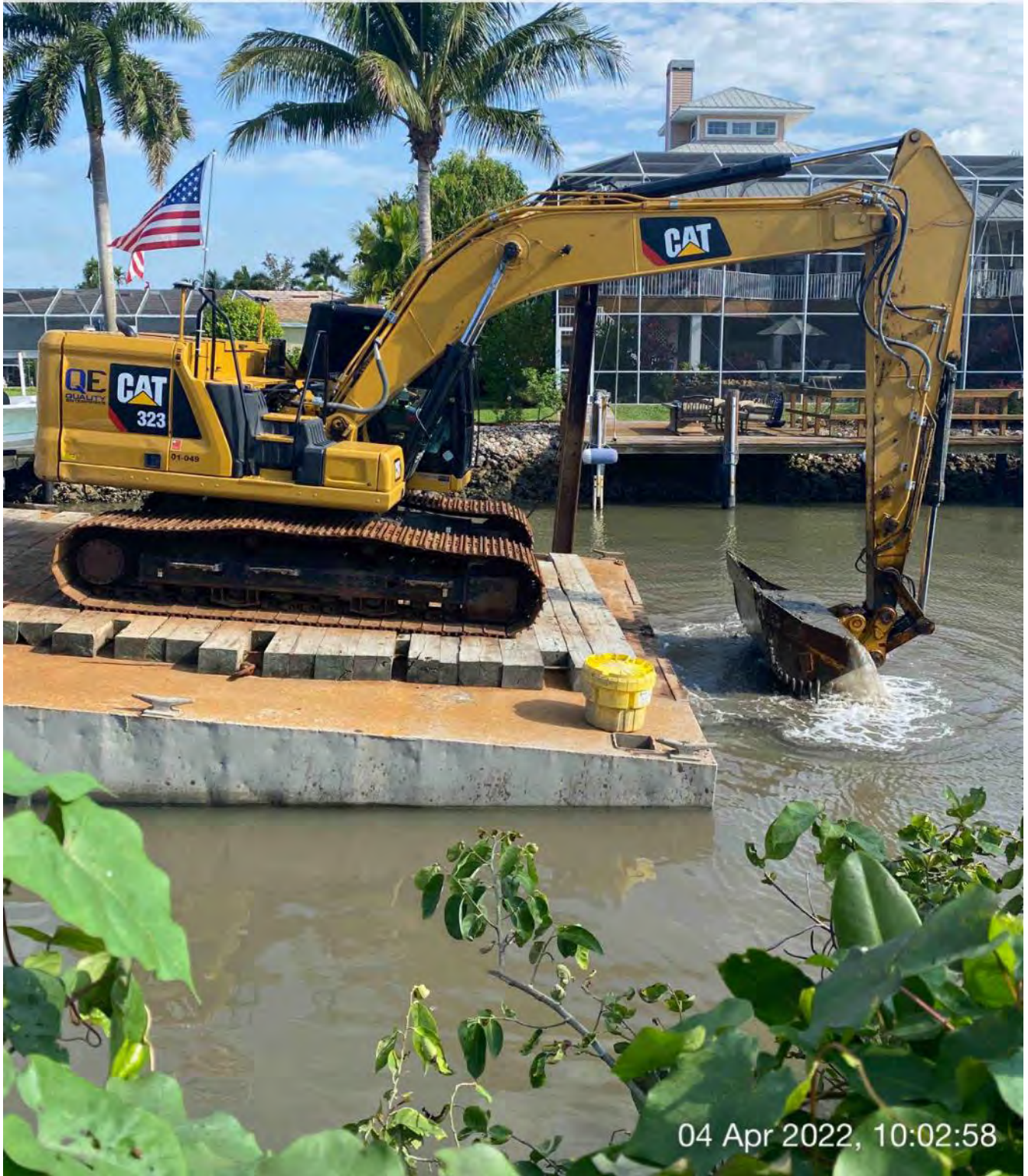
323 excavator removing material from station 9+00
