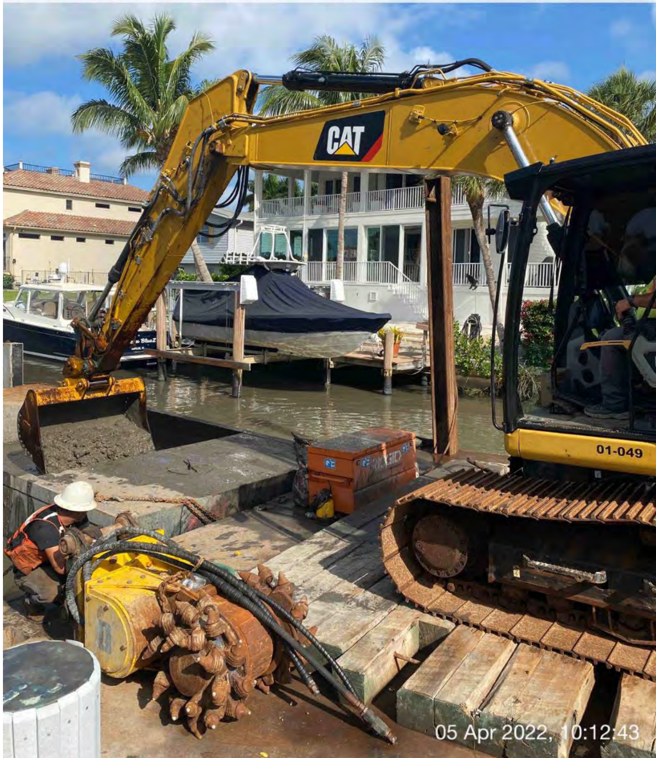
323 excavator removing material and transferring to hopper at station 4+50
