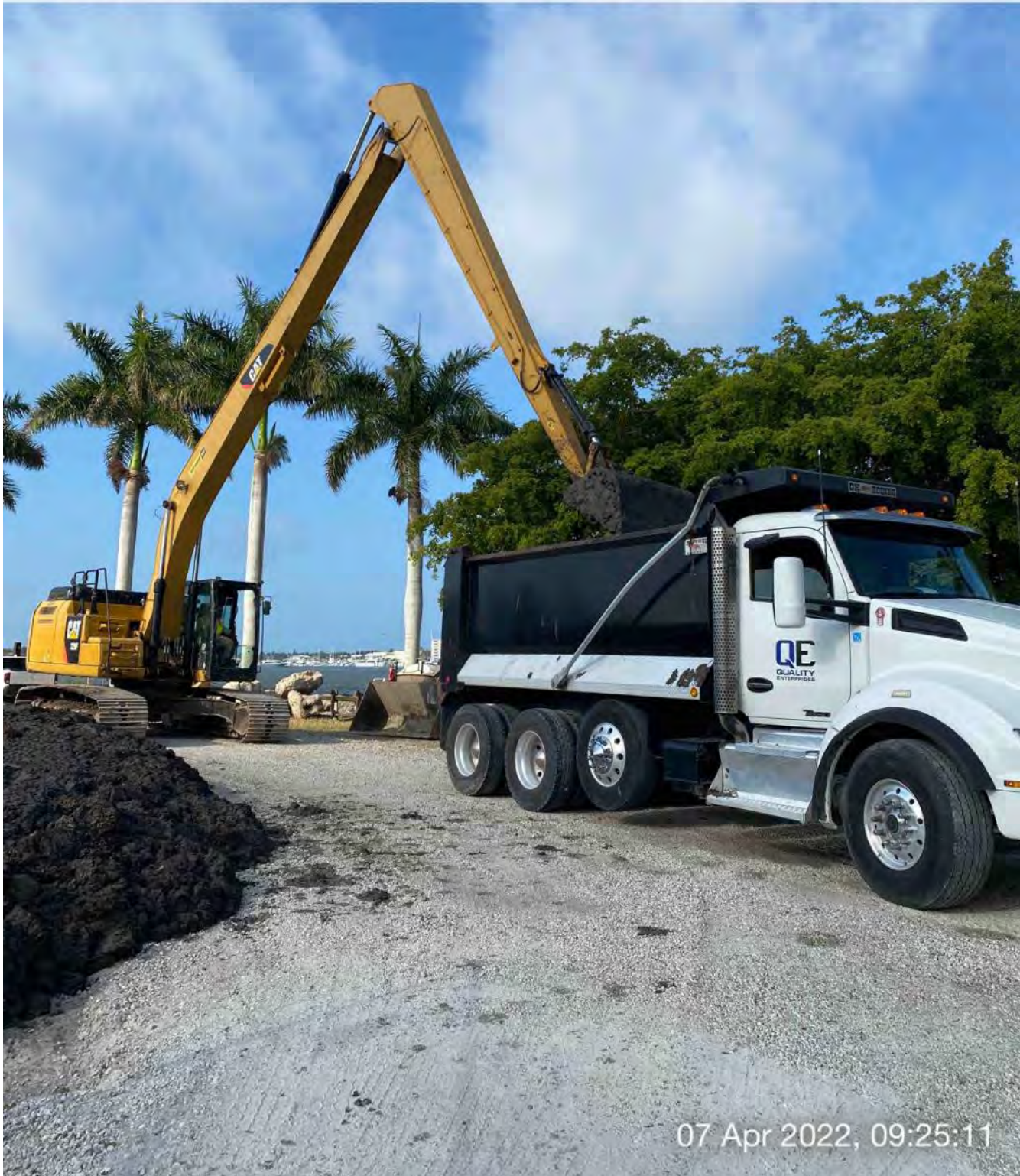
326 excavator transferring removed material from dewatering site to dump truck at 1300 Curlew Avenue
