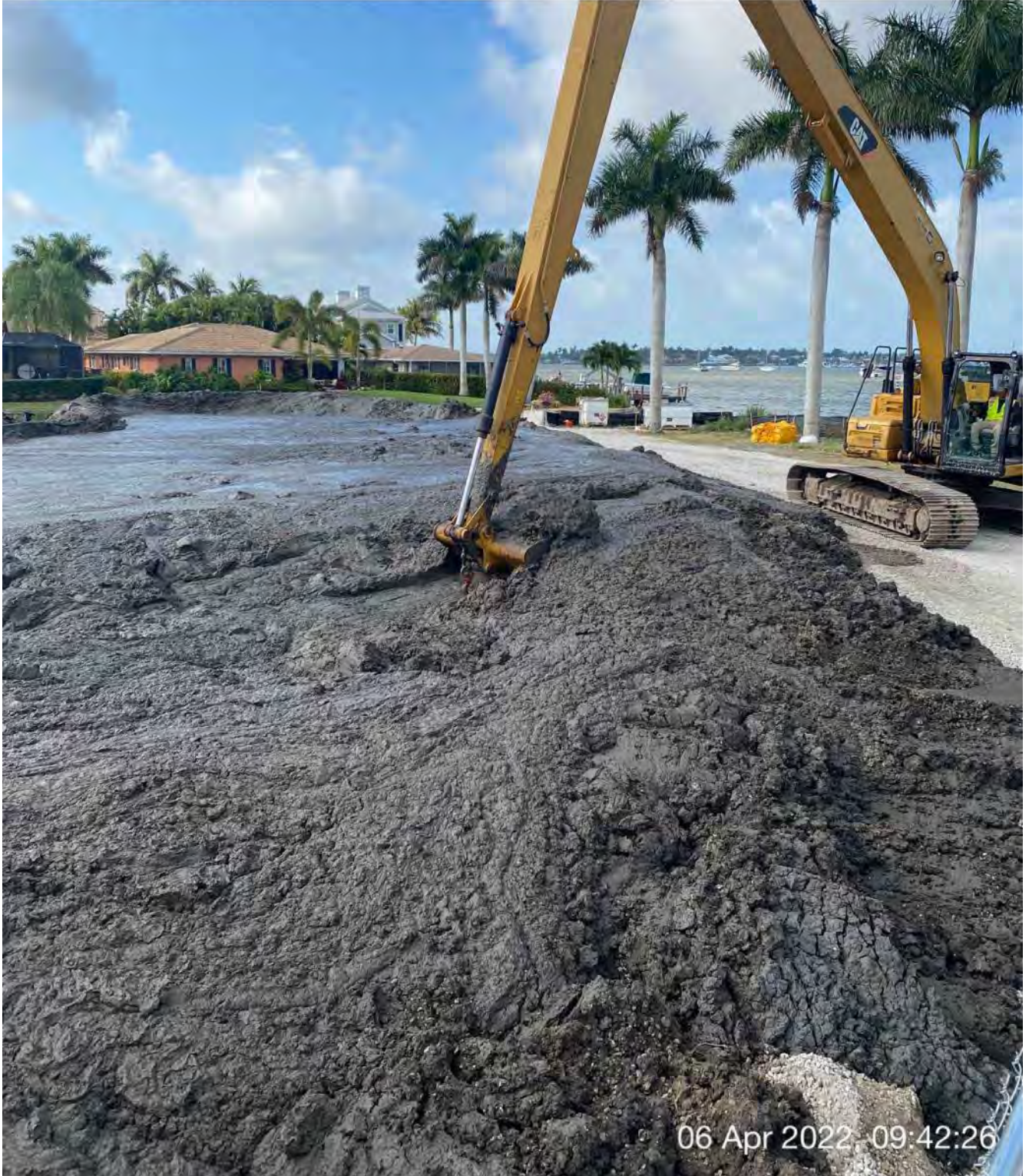
326 excavator transferring removed material from dewatering site at 1300 Curlew Avenue to dump truck
