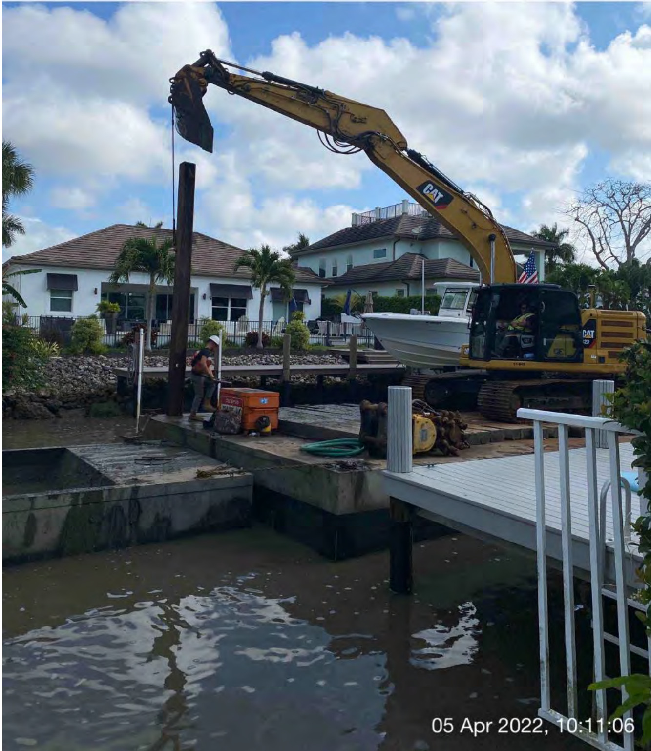
323 excavator lifting spud to allow push boat to mobilize barge at station 4+50
