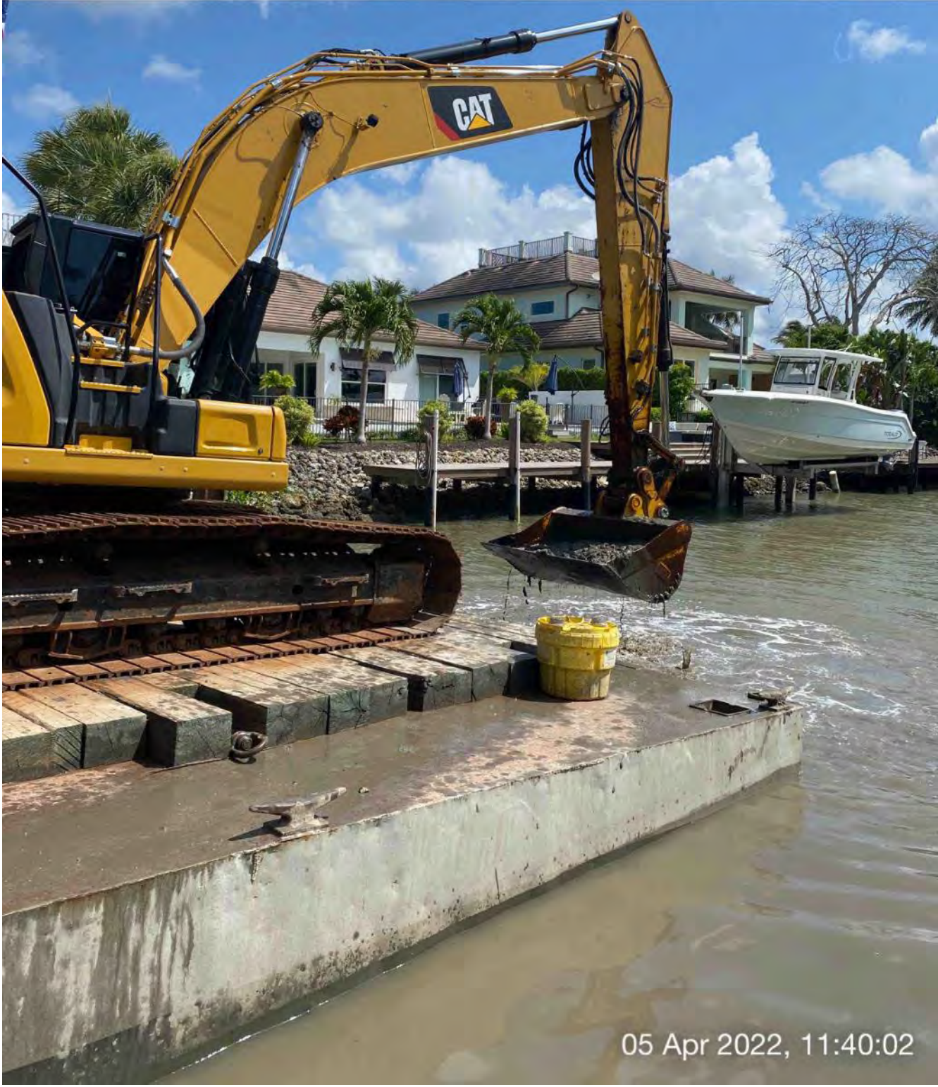
323 excavator removing material from station 4+00
