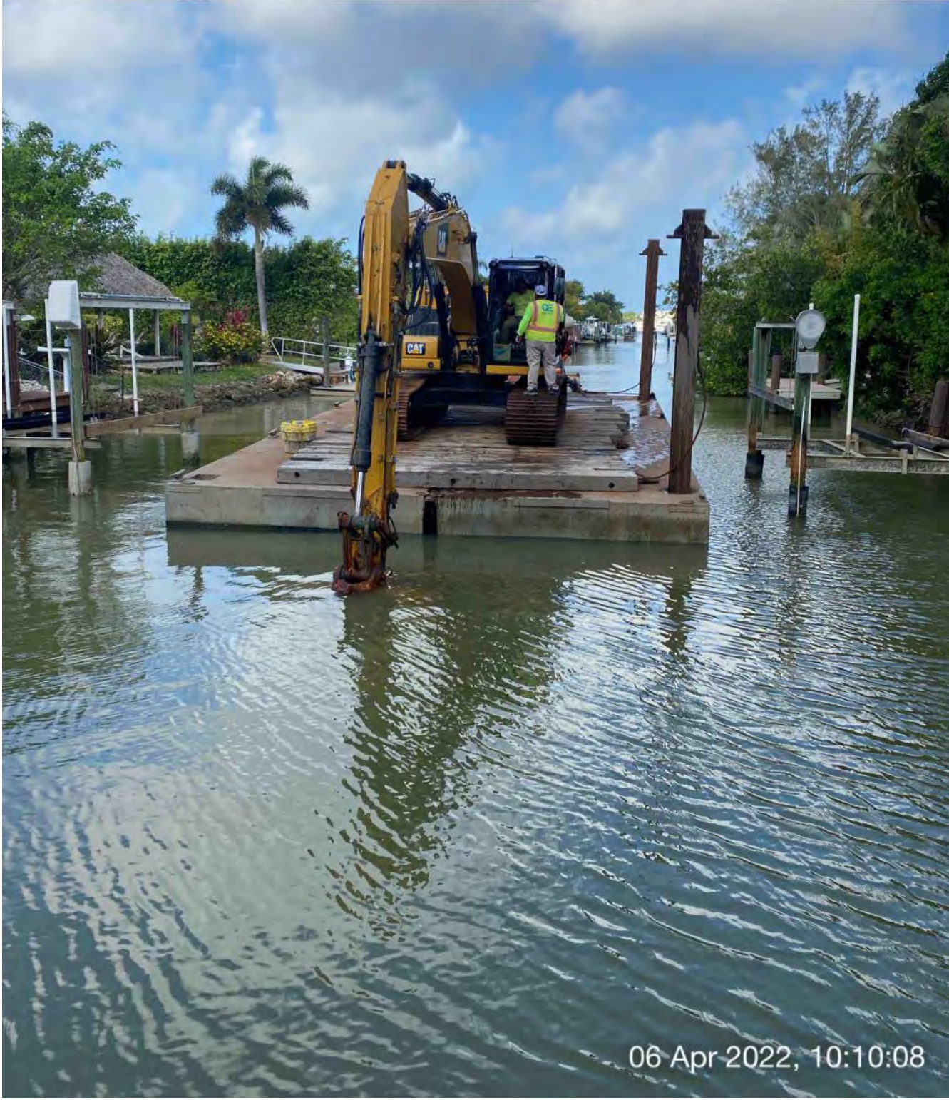
323 excavator removing checking depths and removing material from Station 14+50
