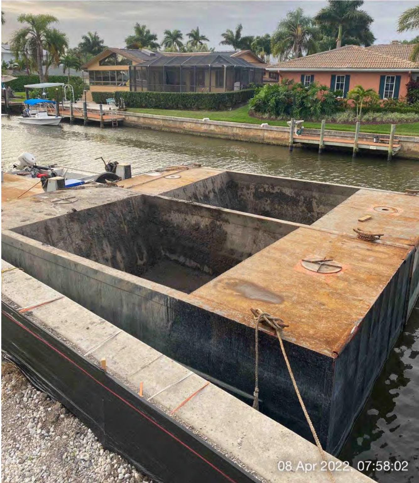
2 empty hoppers staged at station 1+50
