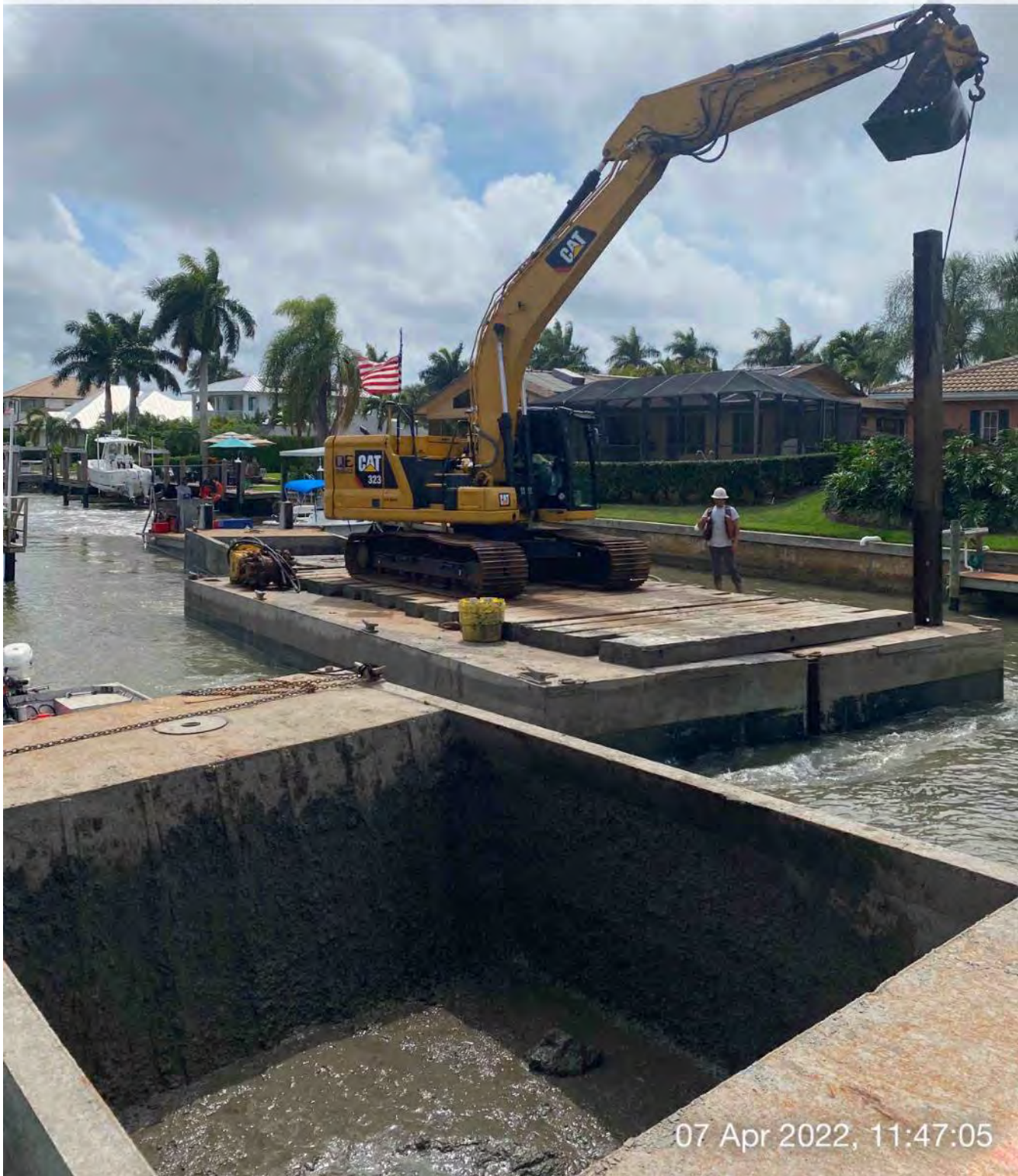
323 excavator lifting spud to allow push boat to mobilize barge at station 1+75
