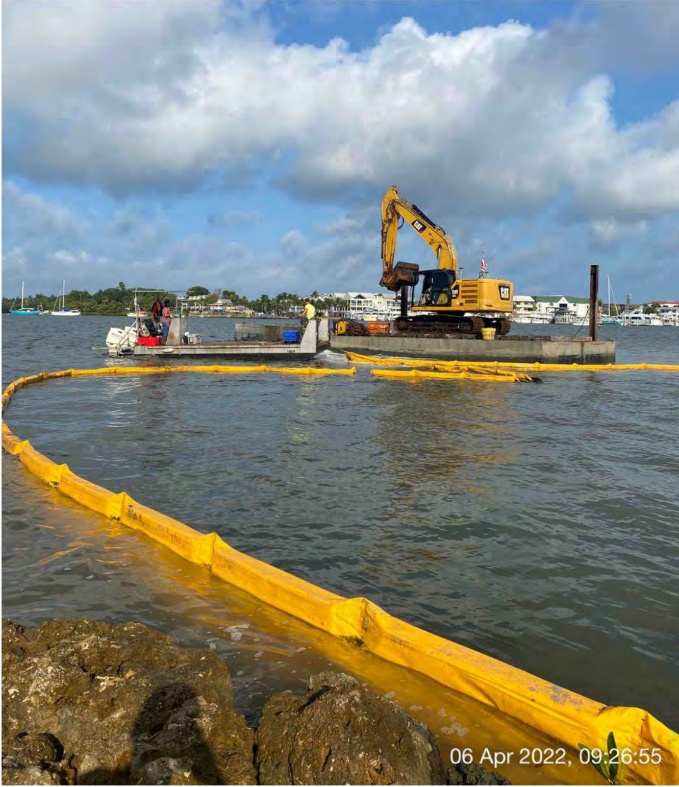
Push boat adjusting turbidity curtain across the mouth of Canal BB-BB
