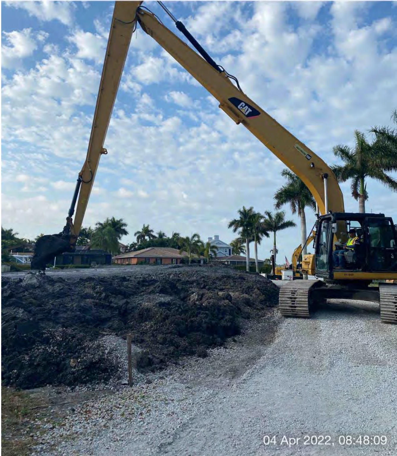
326 excavator redistributing removed material at the dewatering site at 1300 Curlew Avenue
