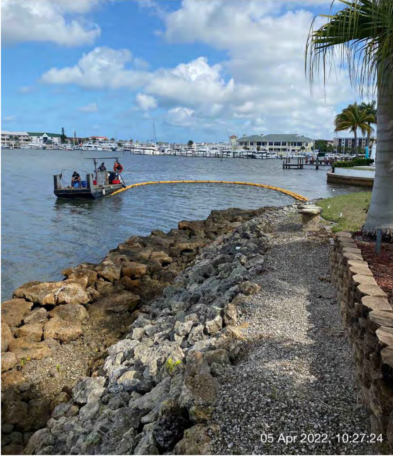
Push boat opening turbidity curtain from across the mouth of Canal BB-BB
