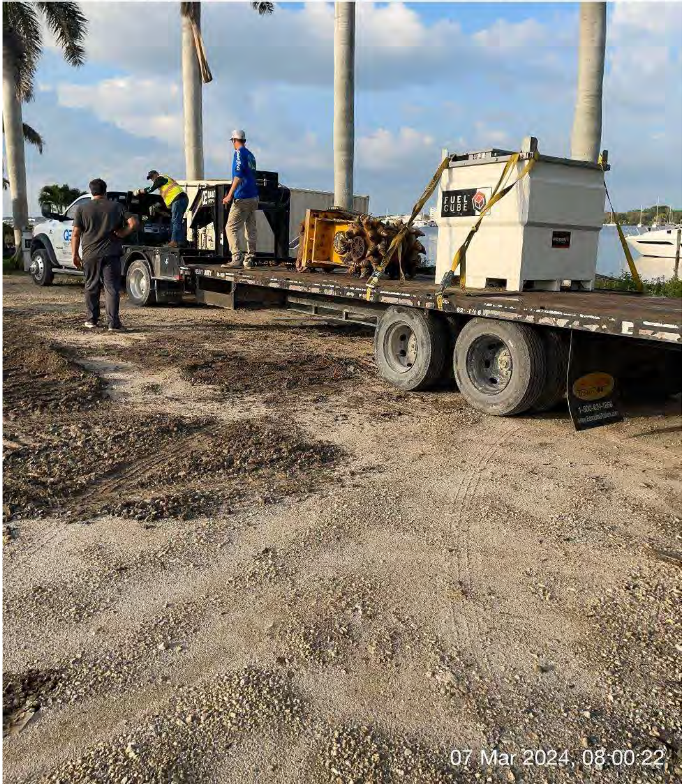
Contractor delivering Epiroc grinder and small fuel cube to site.
