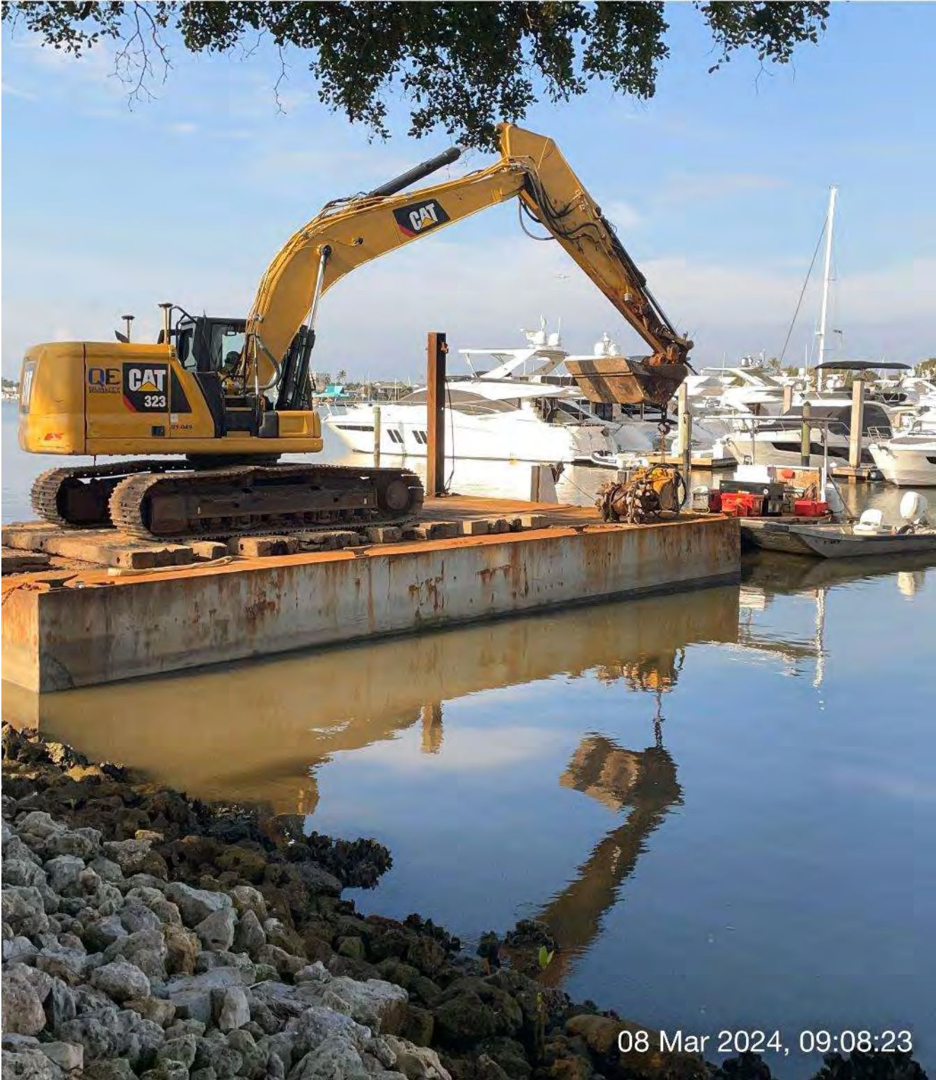
323 excavator loading Epiroc grinder onto barge.
