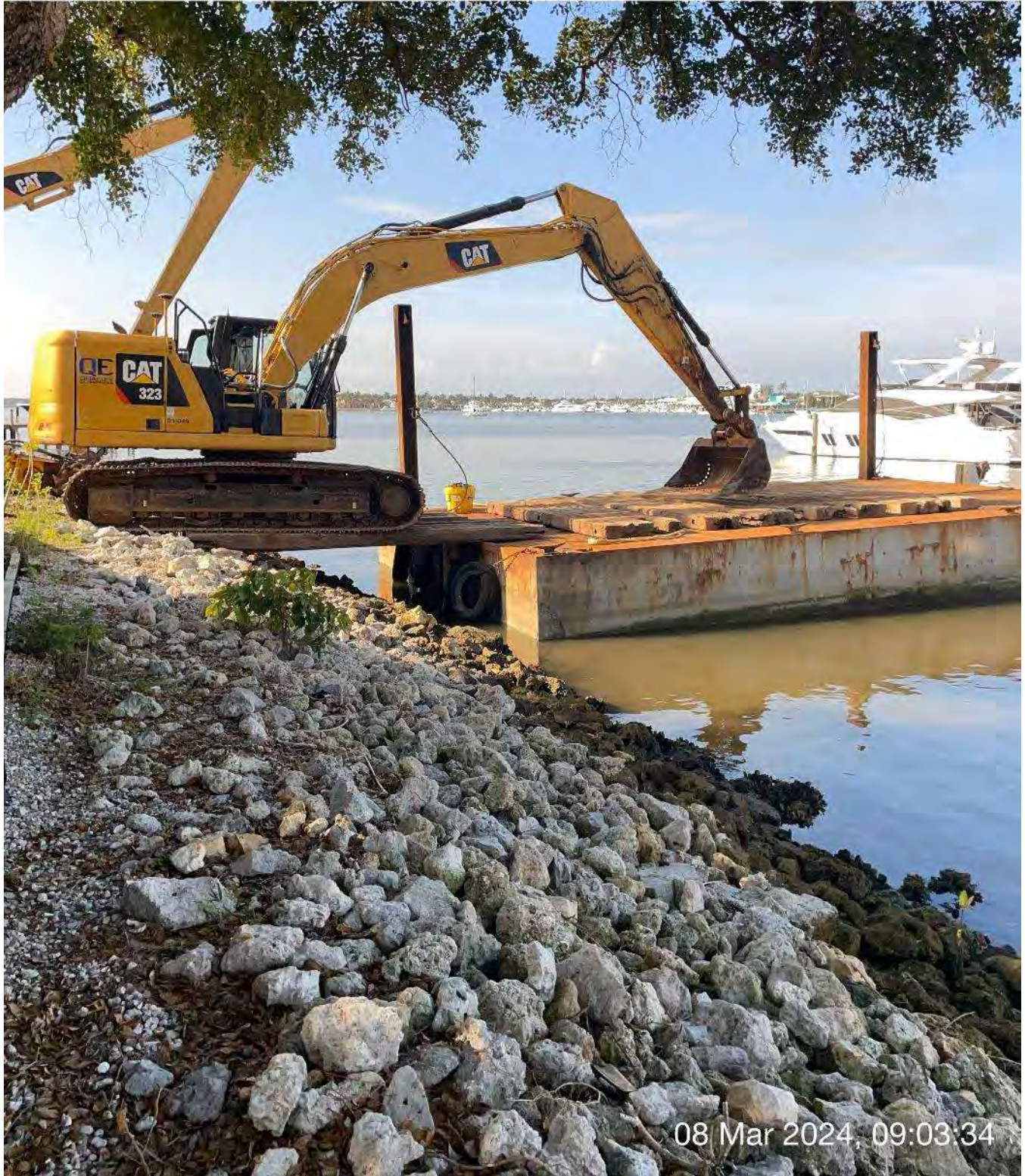
Contractor loading 323 excavator onto barge.
