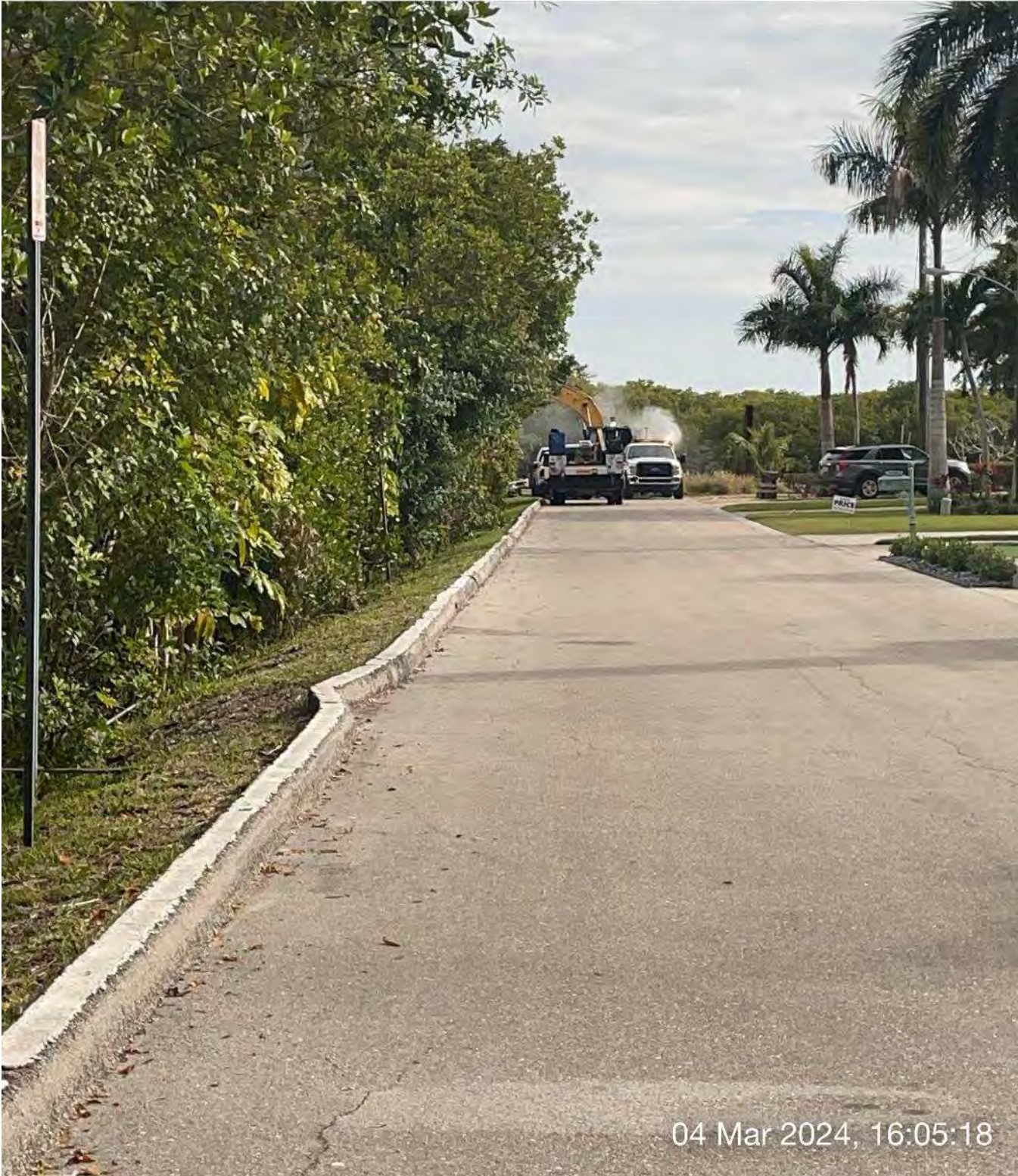
Contractor using water tank on trailer to wash down equipment.
