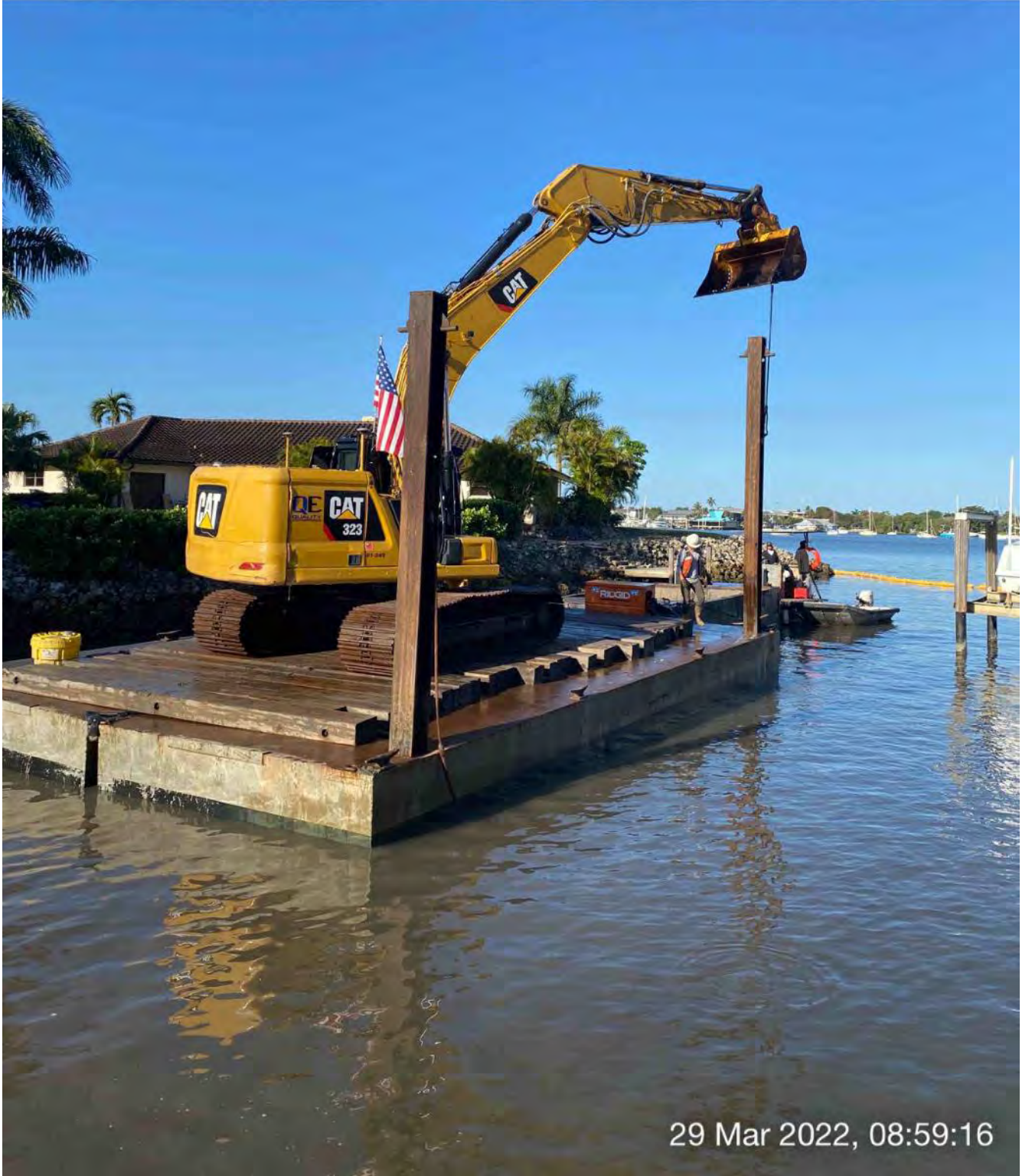
323 excavator lifting spud to allow push boat to mobilize barge at station 3+00
