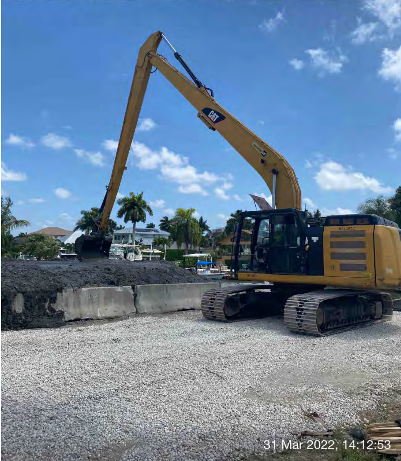
326 excavator transferring material from hopper to dewatering site at 1300 Curlew Avenue
