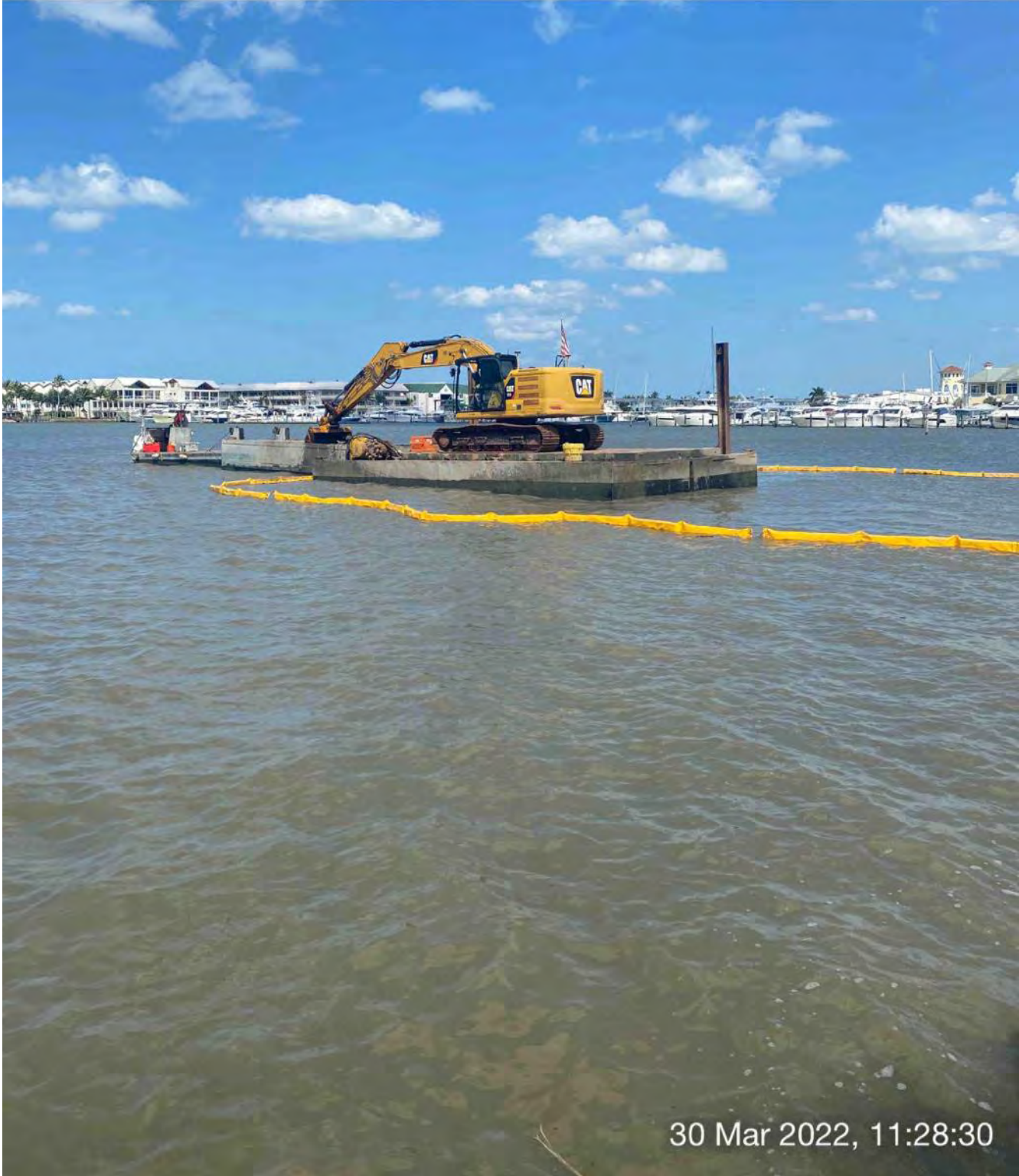
323 excavator removing material from station 0+00 and transferring to hopper
