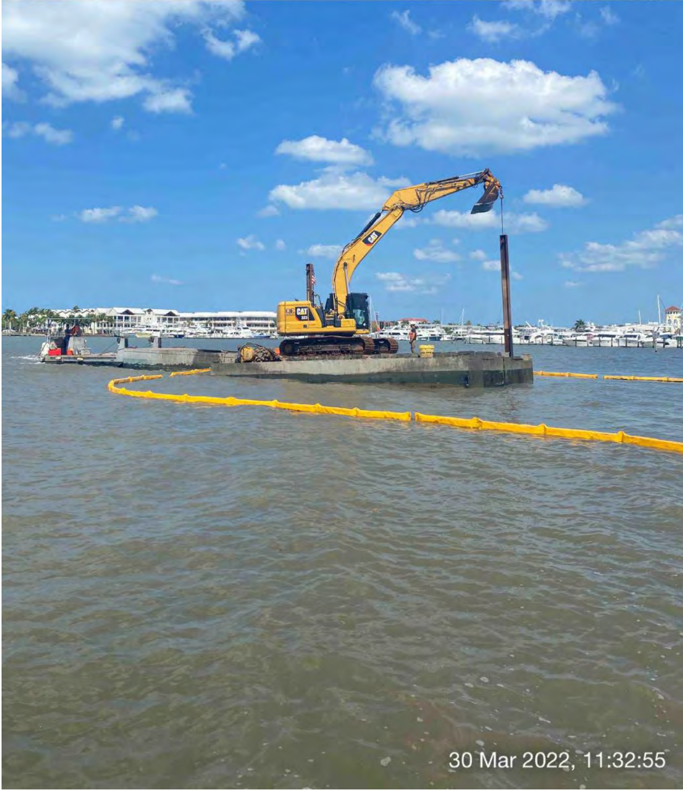
323 excavator lifting spud to allow push boat to mobilize barge at station 0+50
