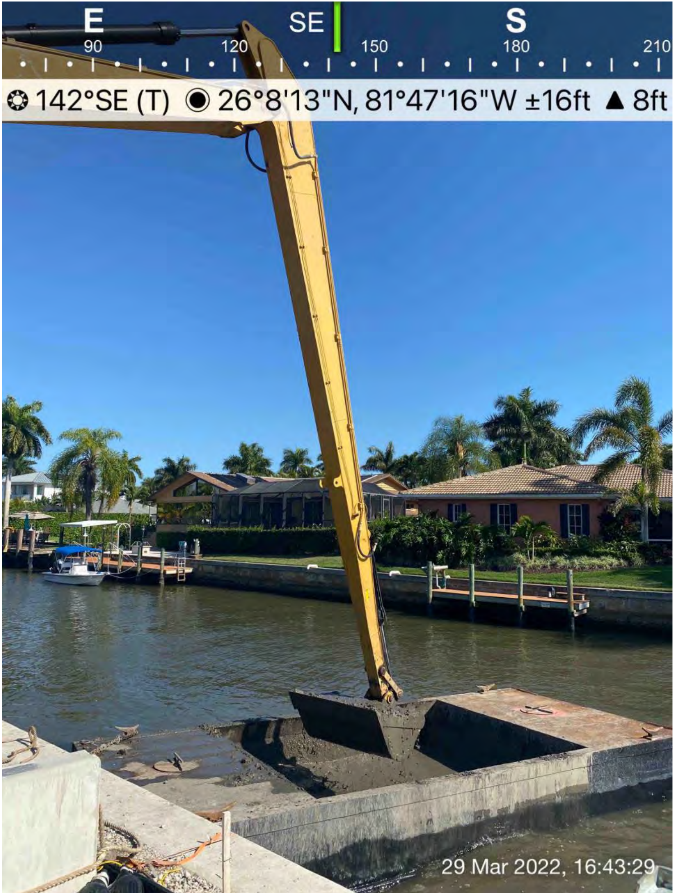
326 excavator transferring material from hopper to dewatering site at 1300 Curlew Avenue
