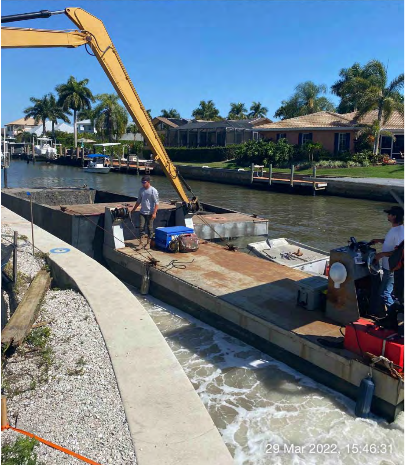
Push boat dropping off full hopper of removed material and taking empty hopper back to barge in Canal BB-BB
