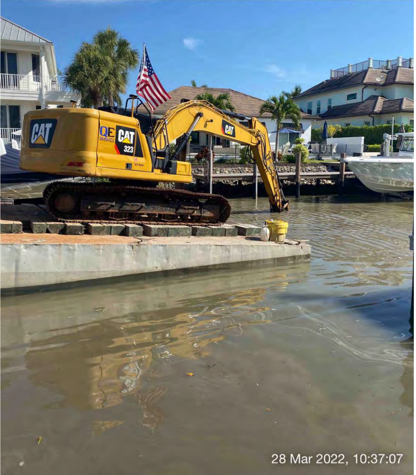
323 excavator grinding rock at station 4+50
