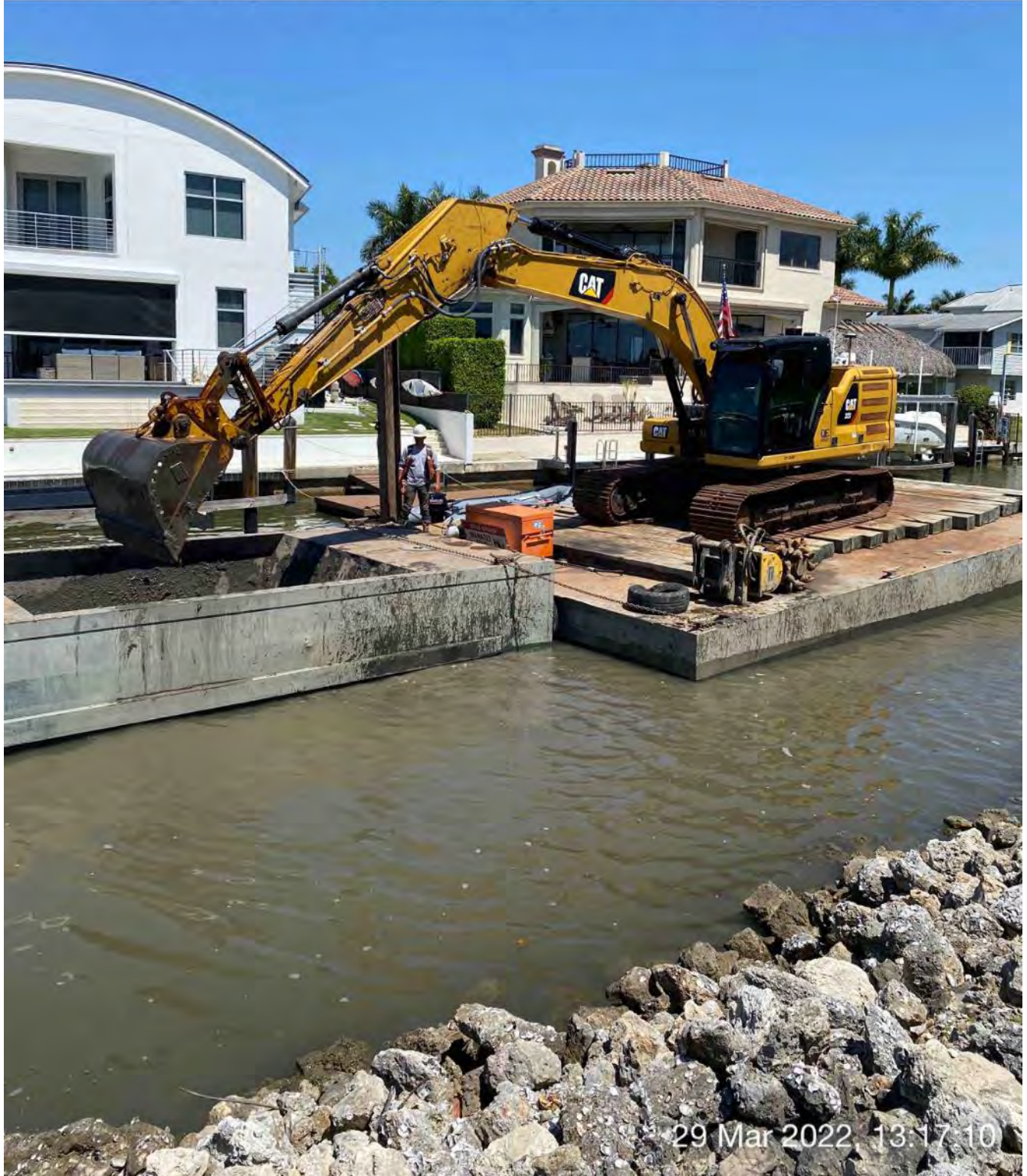
323 excavator removing material from station 3+50 and transferring to hopper
