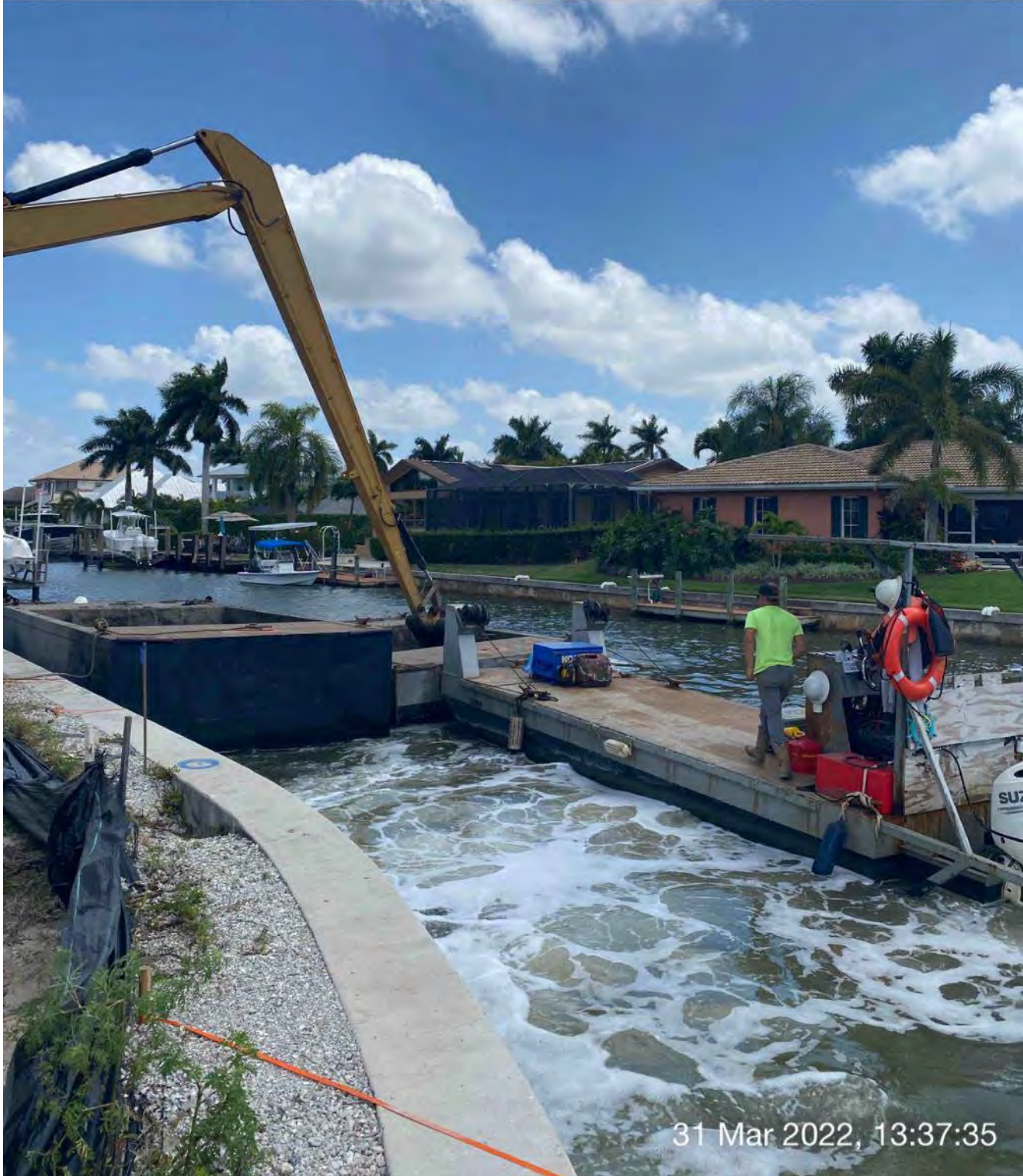
Push boat dropping off full hopper of material and picking up empty hopper to transport back to barge
