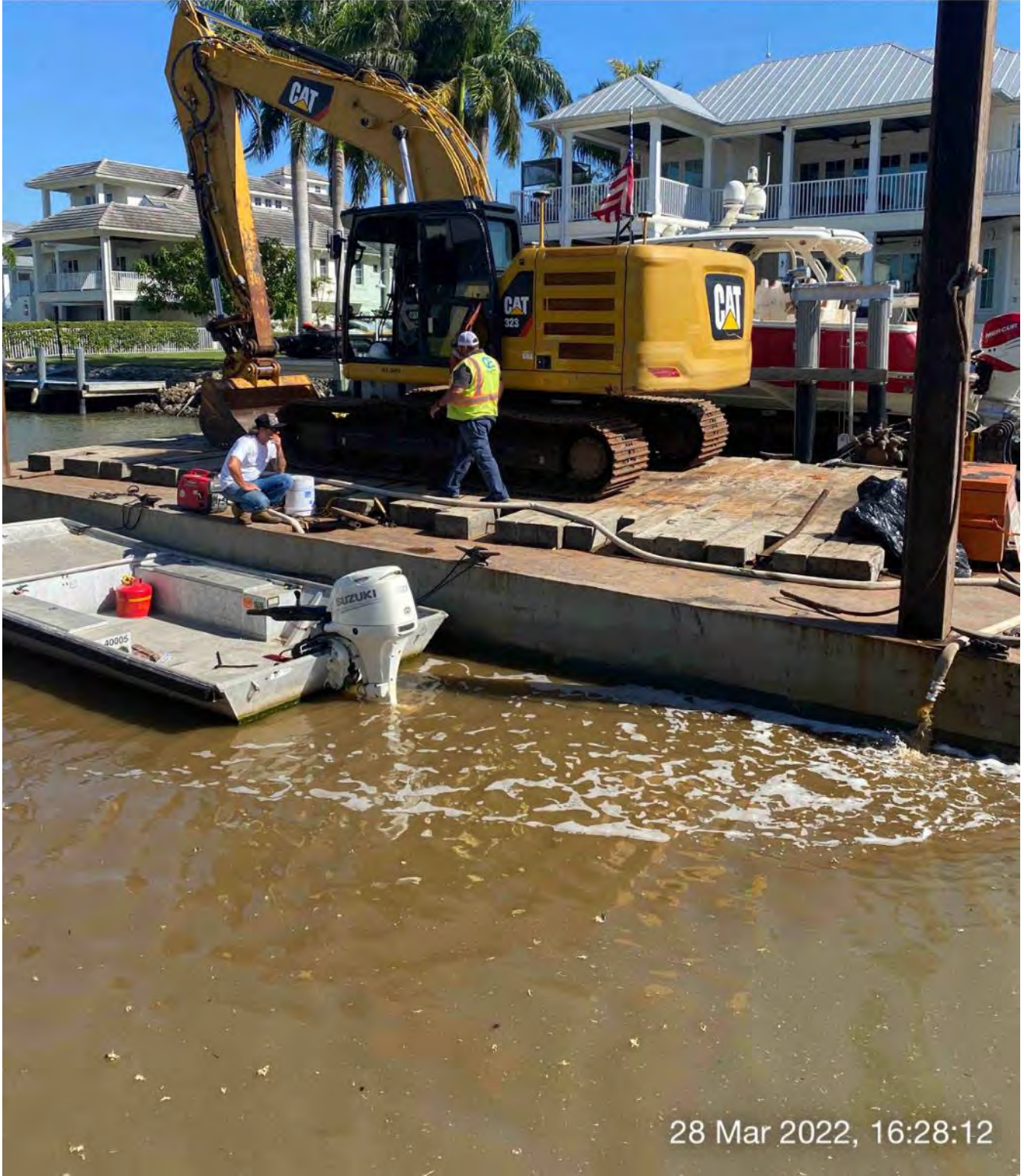
Pumping water out of the bottom of the barge at station 3+00
