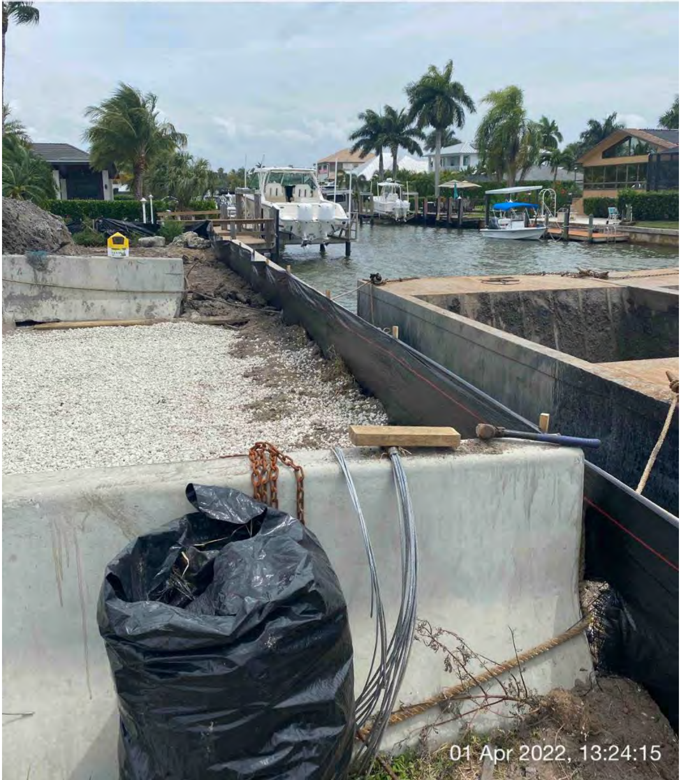
New silt fence installed around perimeter of property at 1300 Curlew Avenue
