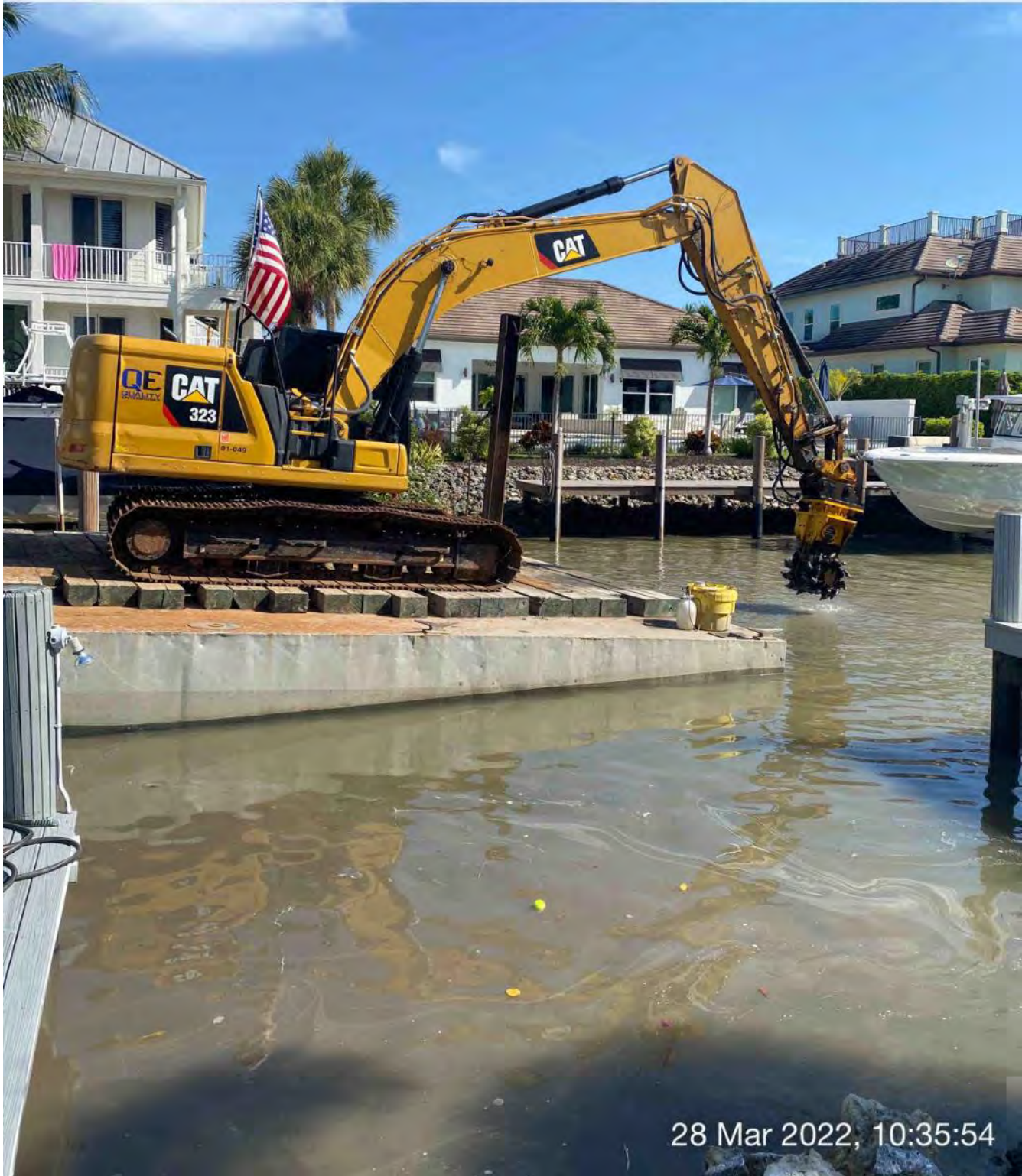
323 excavator grinding rock at station 4+50
