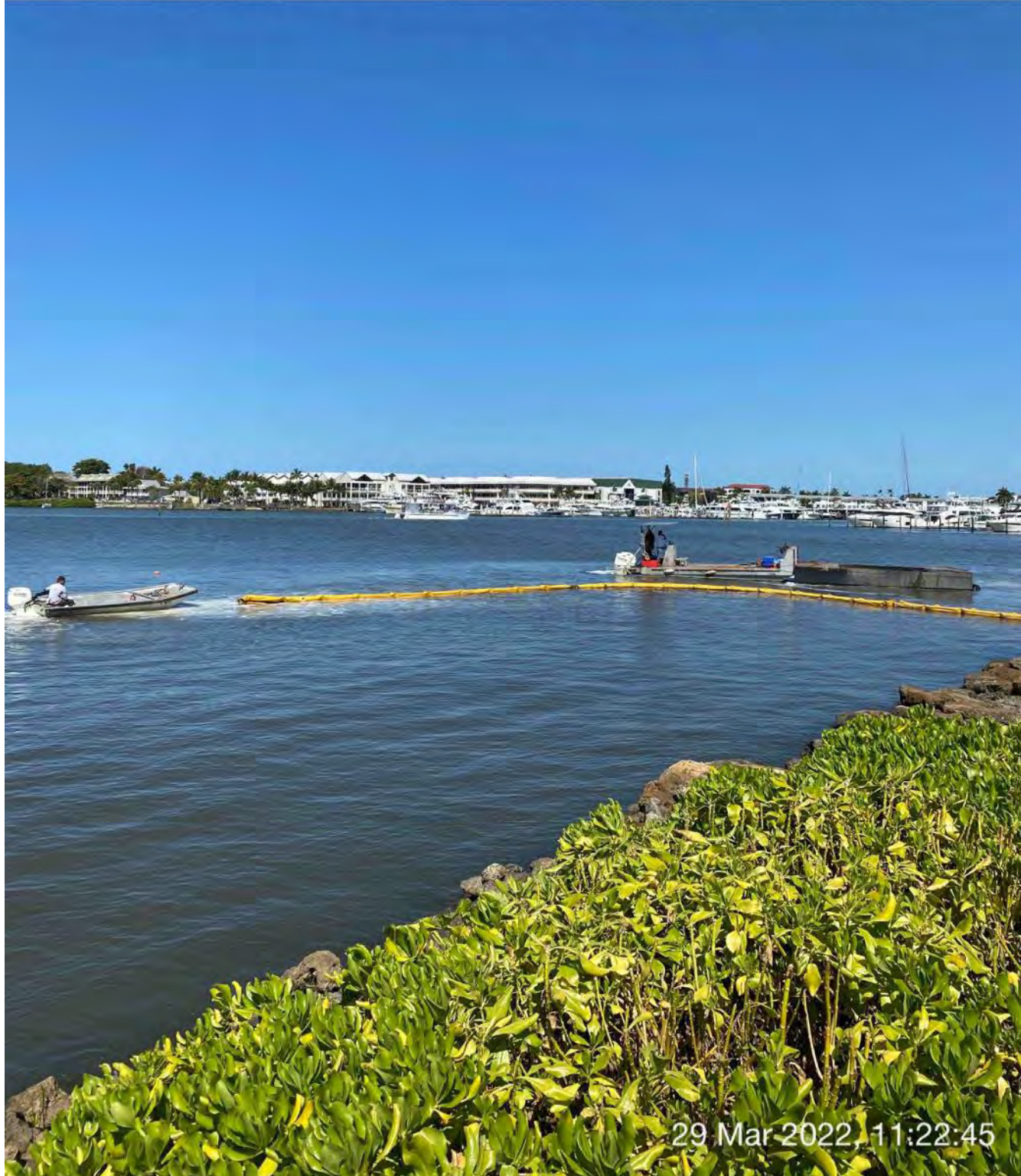
Support boat holding open turbidity curtain so that push boat can exit Canal BB-BB with hopper
