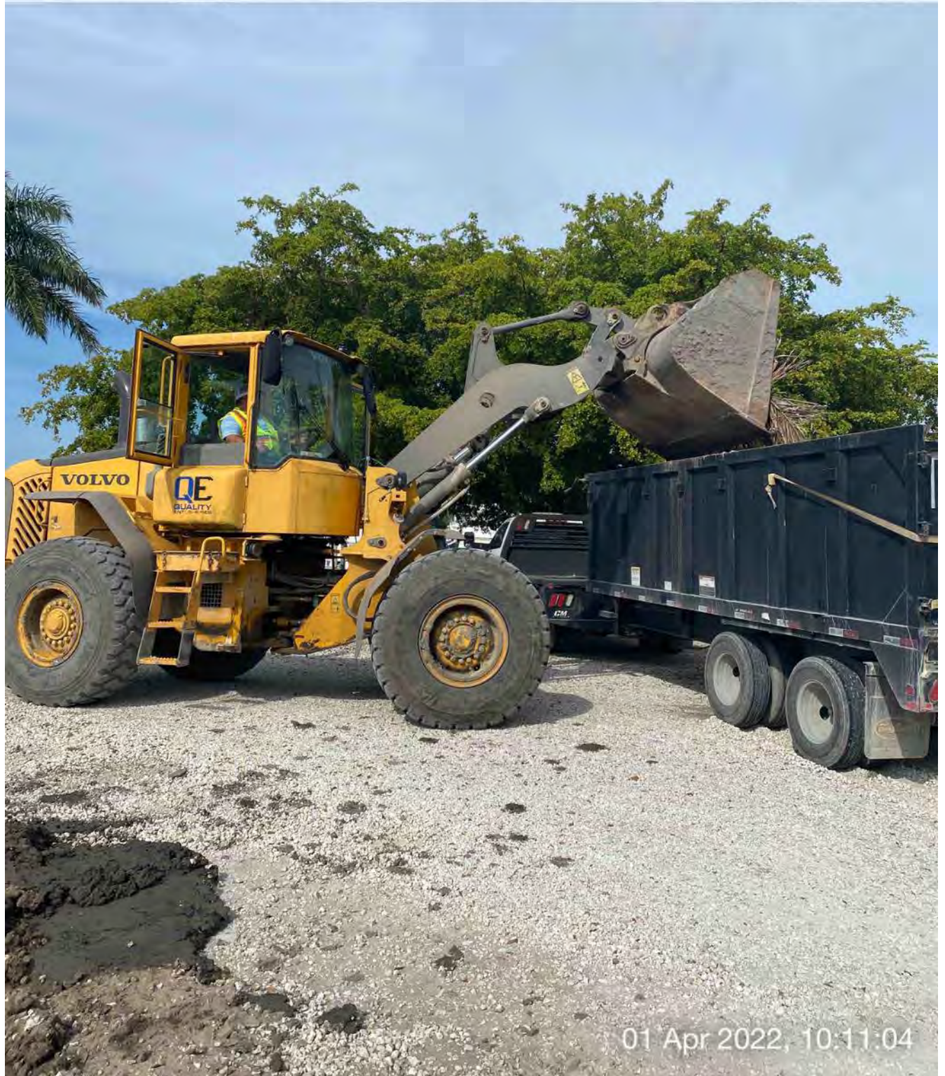
Front end loader transporting debris from 1300 Curlew Avenue to truck bed
