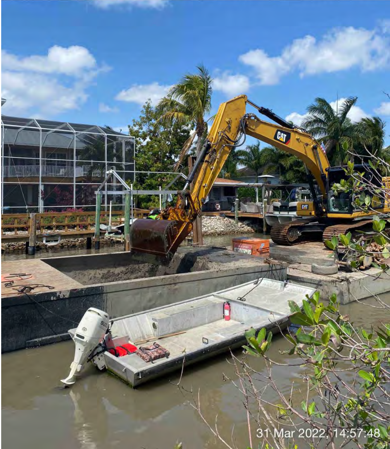
323 excavator removing material from station 10+00 and transferring to hopper
