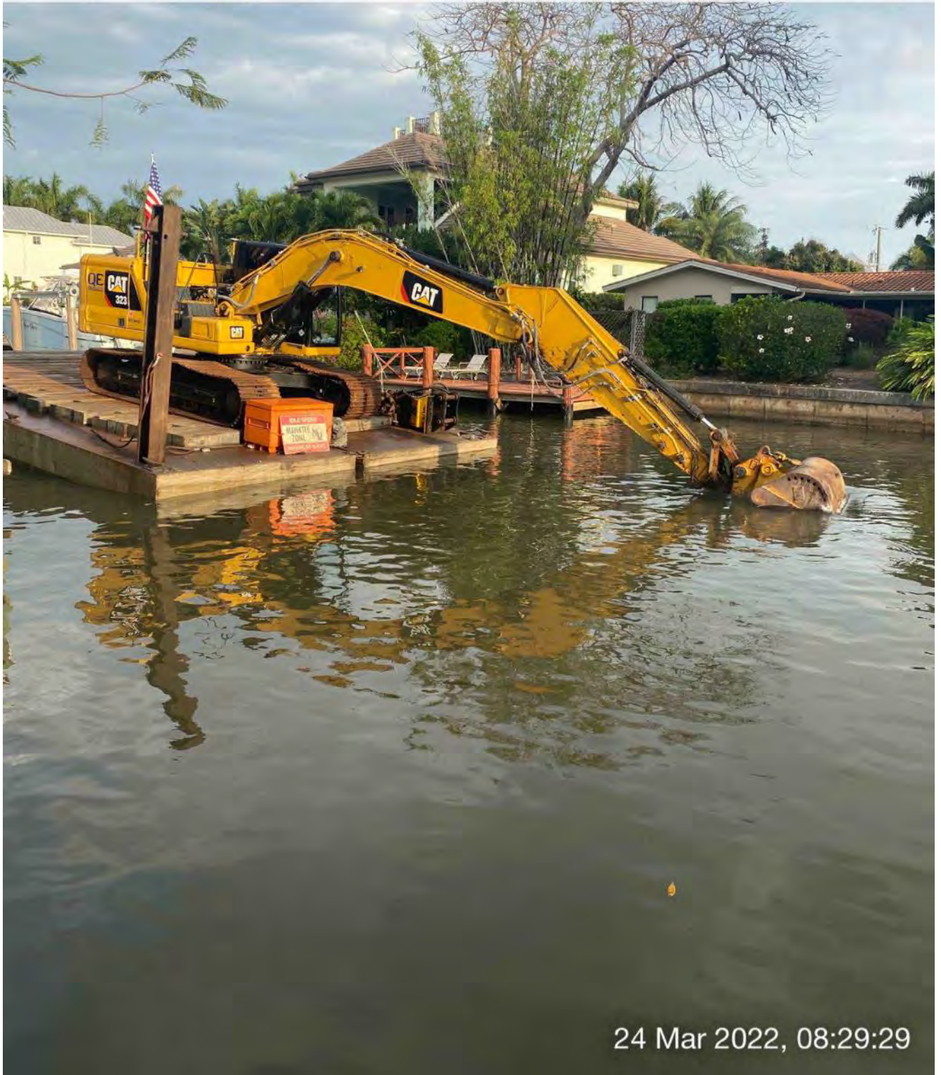
323 excavator removing material from station 6+50 and transferring to hopper
