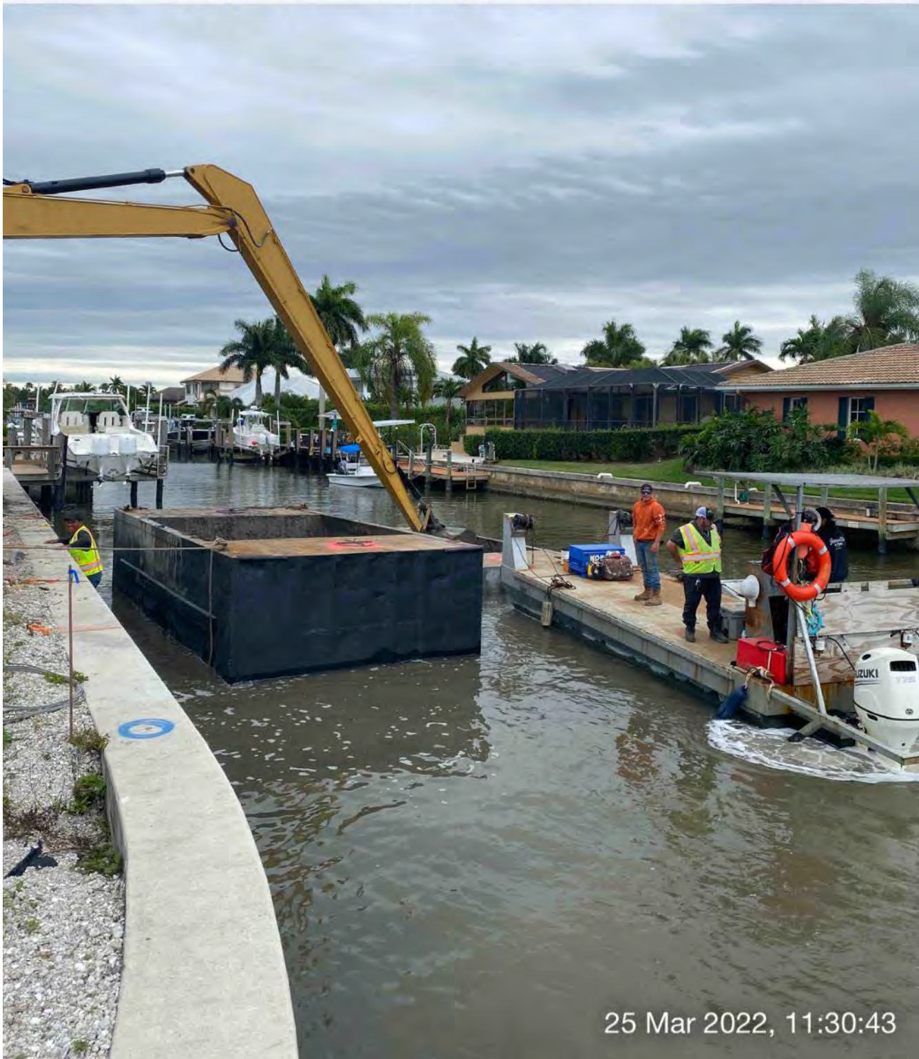
Push boat dropping off hopper full of material and picking up empty hopper at station 1+50 in Canal CC-CC
