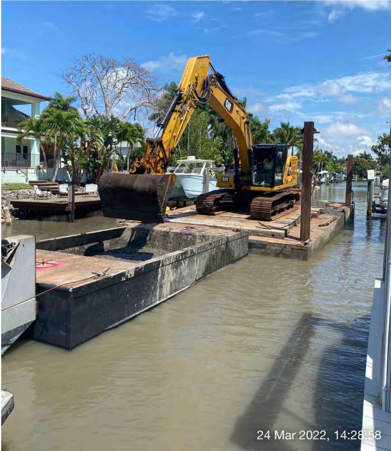
323 excavator removing material from station 6+00 and transferring to hopper
