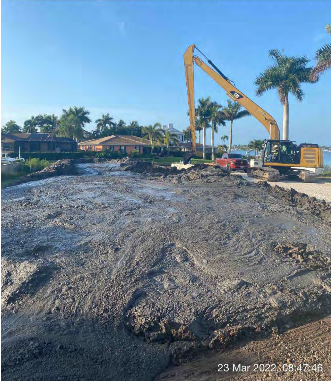
Removed material at the dewatering site at 1300 Curlew Avenue
