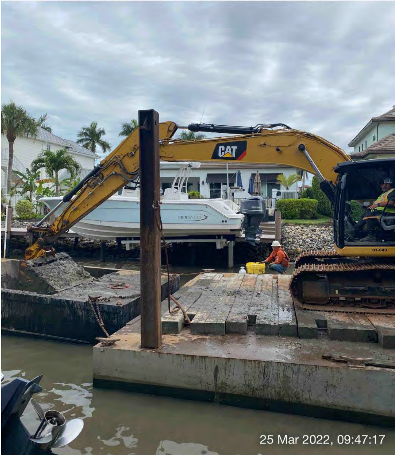
323 excavator removing material from station 5+50 and transferring to hopper
