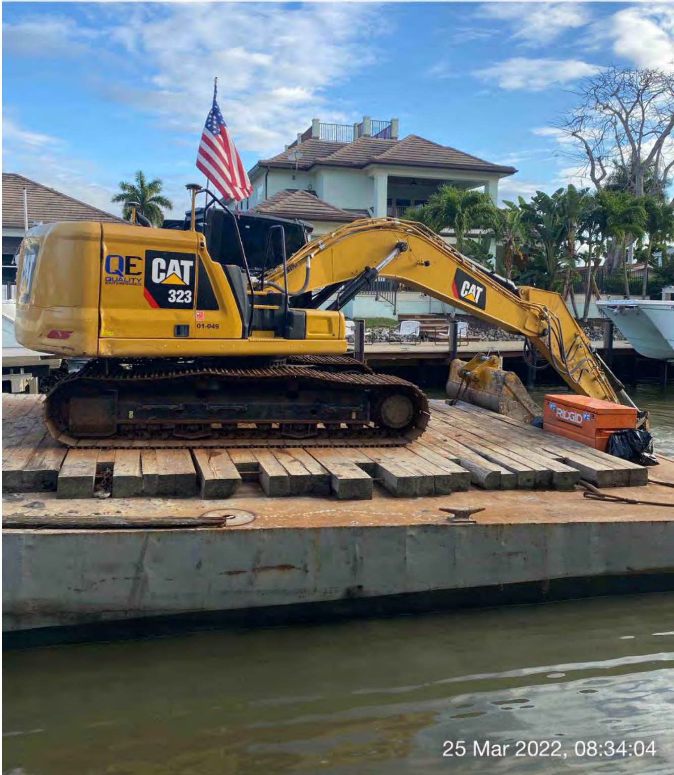
323 excavator grinding rock at station 5+50
