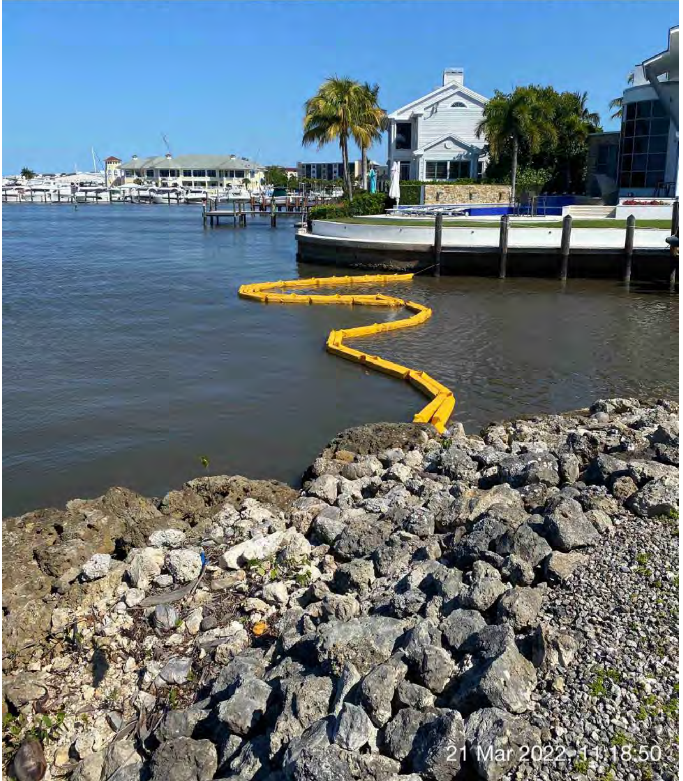
Turbidity curtain installed across the mouth of Canal CC-CC
