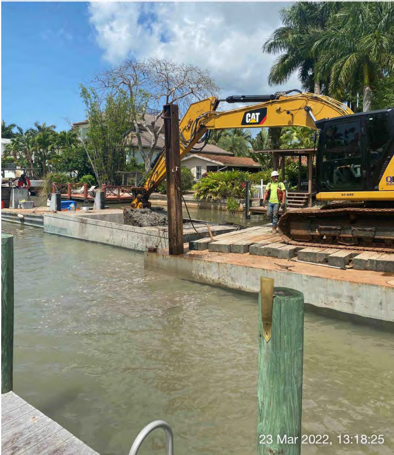
323 excavator removing material from station 7+50 and transferring to hopper
