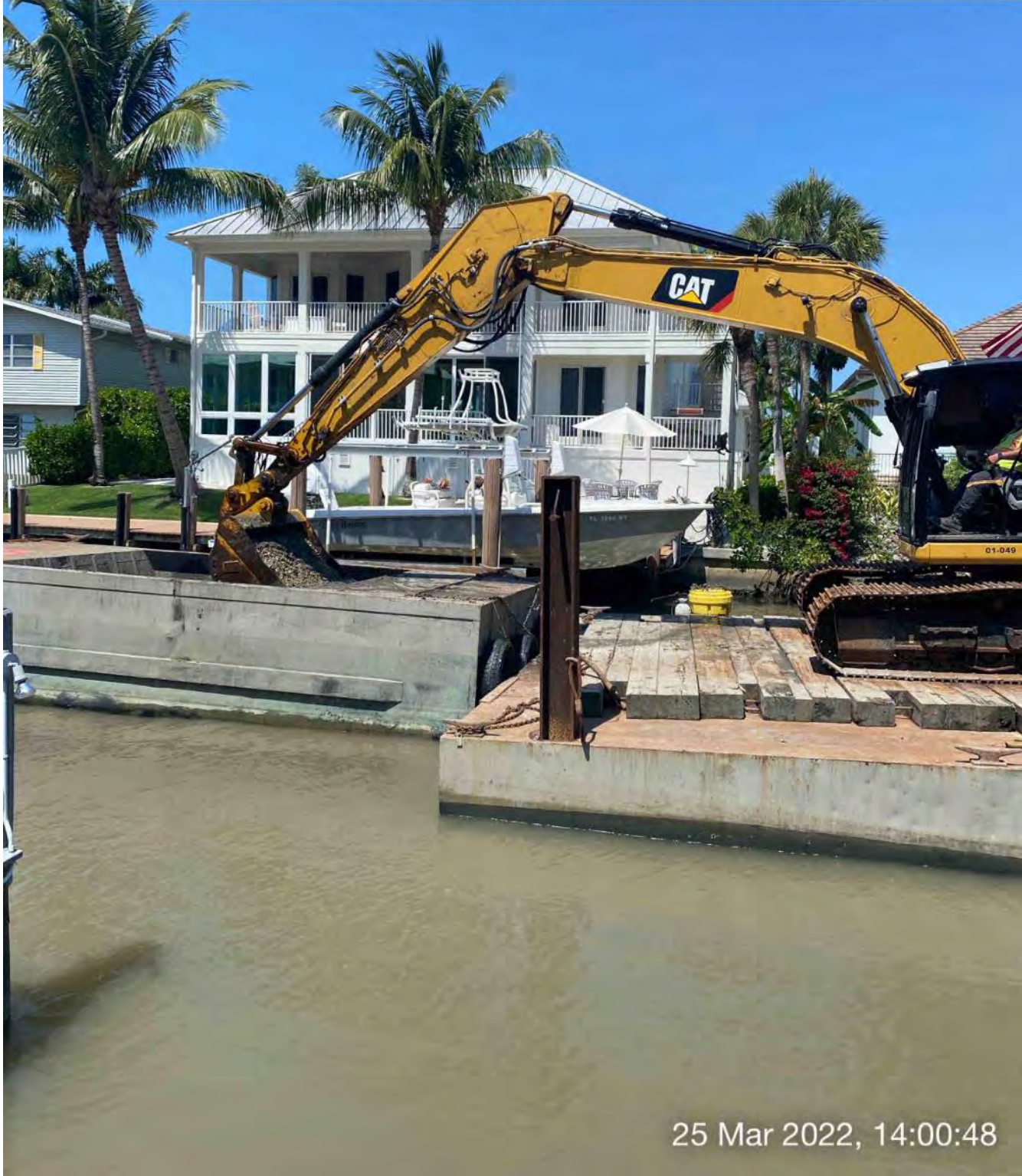
323 excavator removing material from station 4+50 and transferring to hopper
