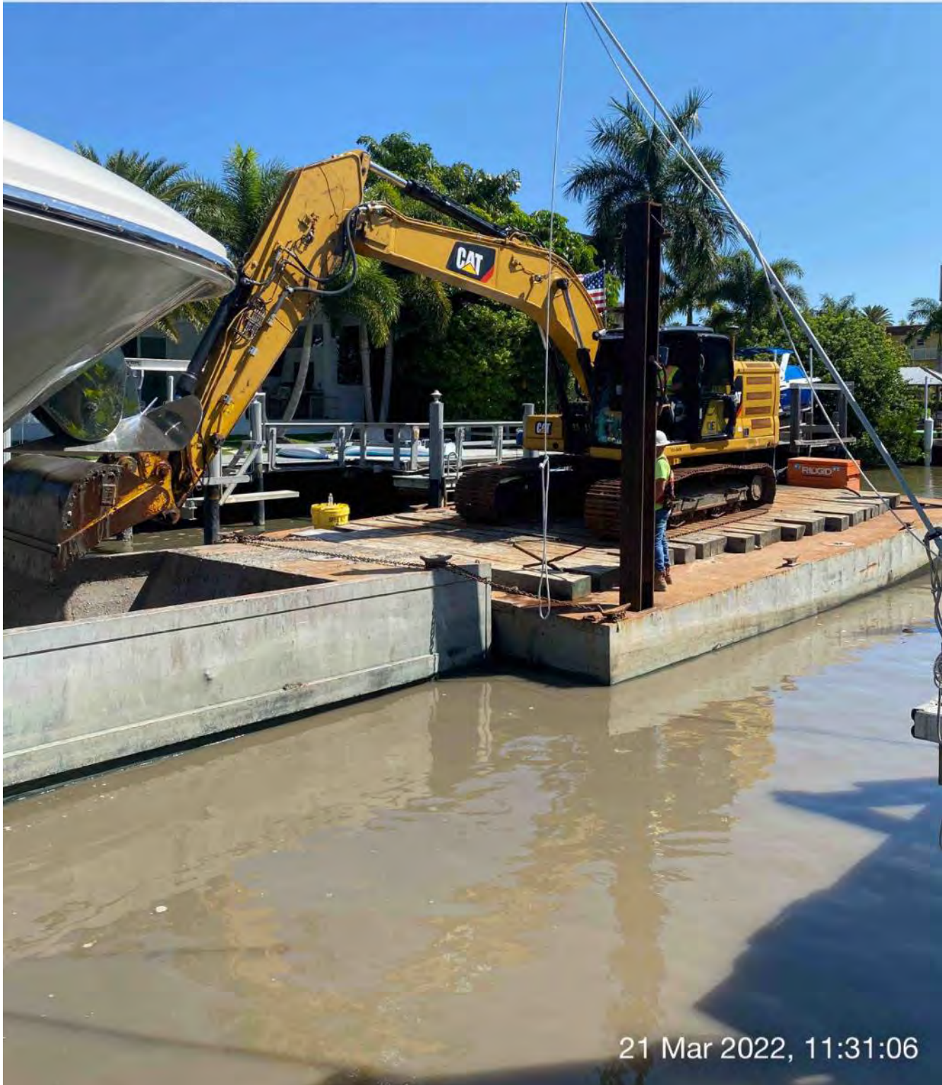
323 excavator removing material from station 11+00 and transferring to hopper
