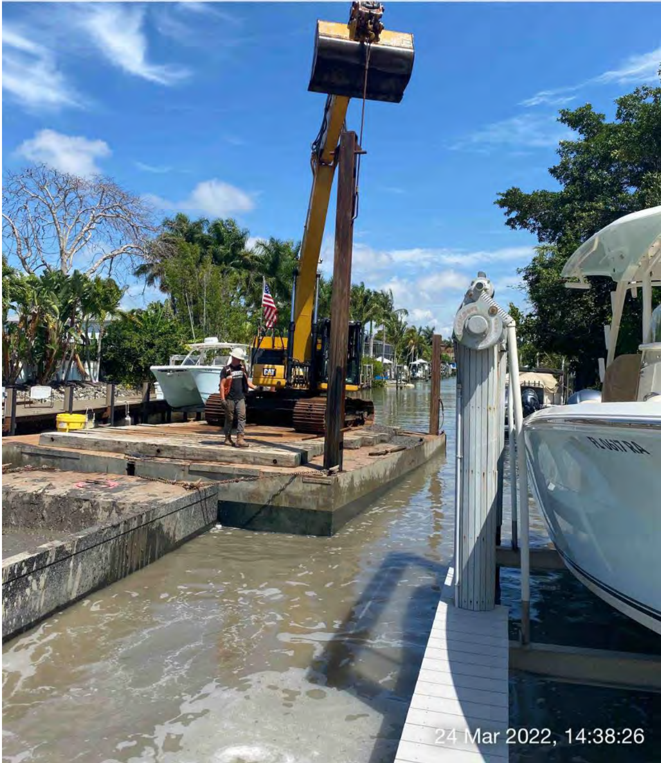
323 excavator lifting spud to allow push boat to mobilize barge at station 5+50 in Canal CC-CC
