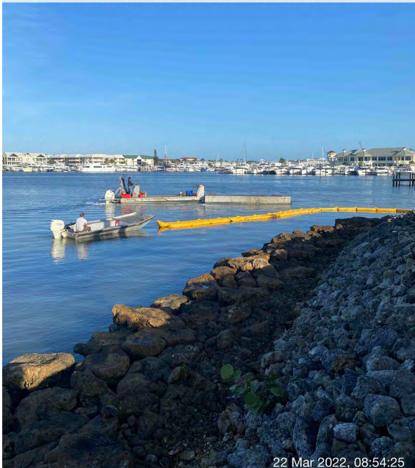
Support boat holding open curtain to allow push boat to exit Canal BB-BB and transport hopper to Canal CC-CC
