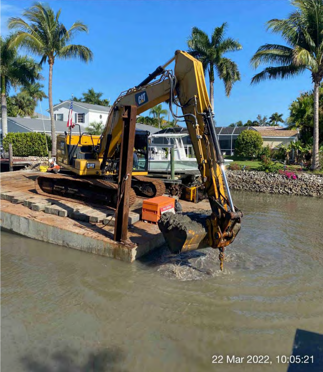
323 excavator removing material from station 9+50 and transferring to hopper
