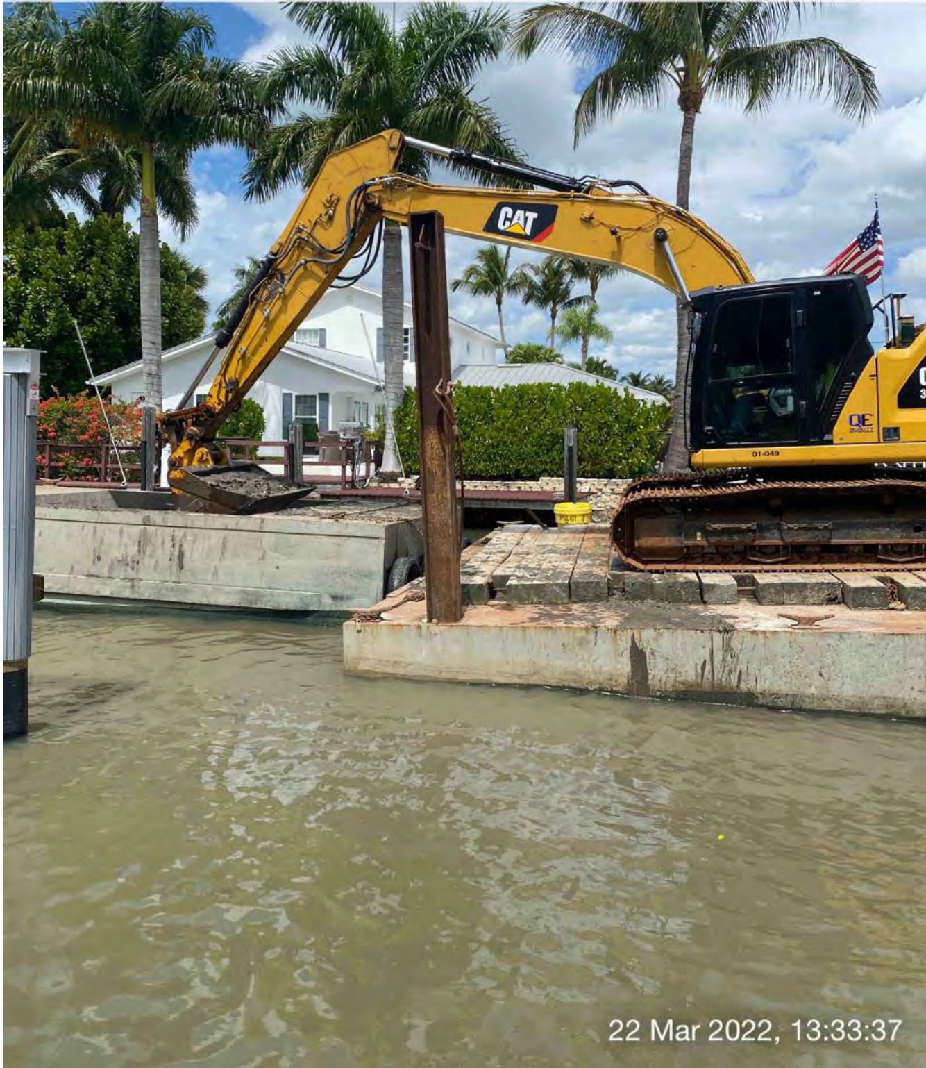
323 excavator removing material from station 8+50 and transferring to hopper
