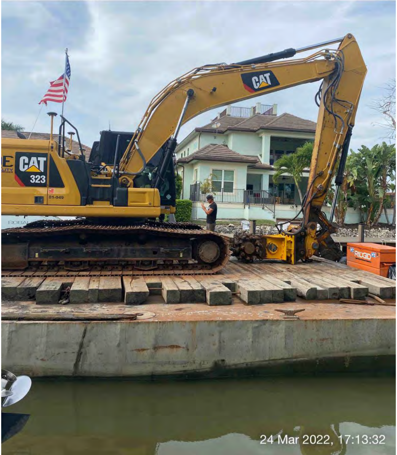
323 excavator on barge with Epiroc grinder at station 5+50
