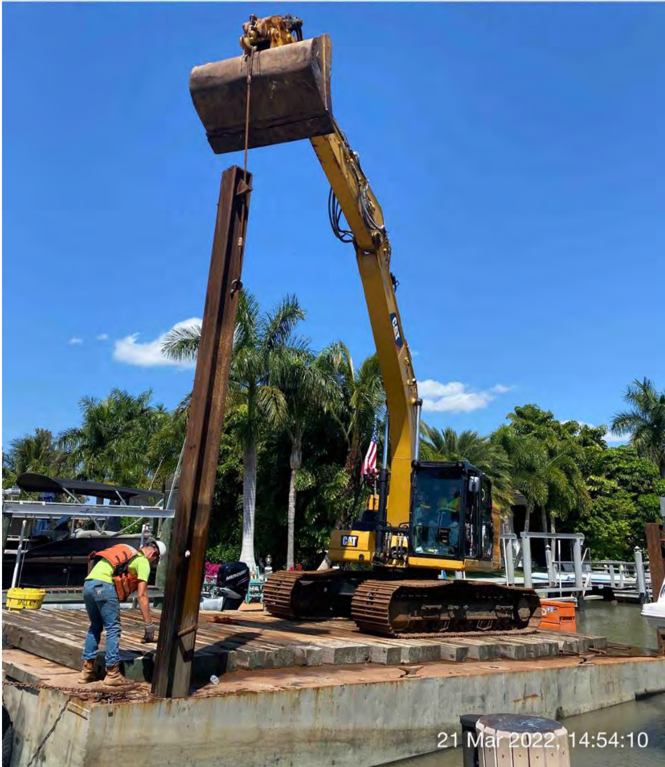
323 excavator lifting spud to allow push boat to mobilize barge at station 10+00
