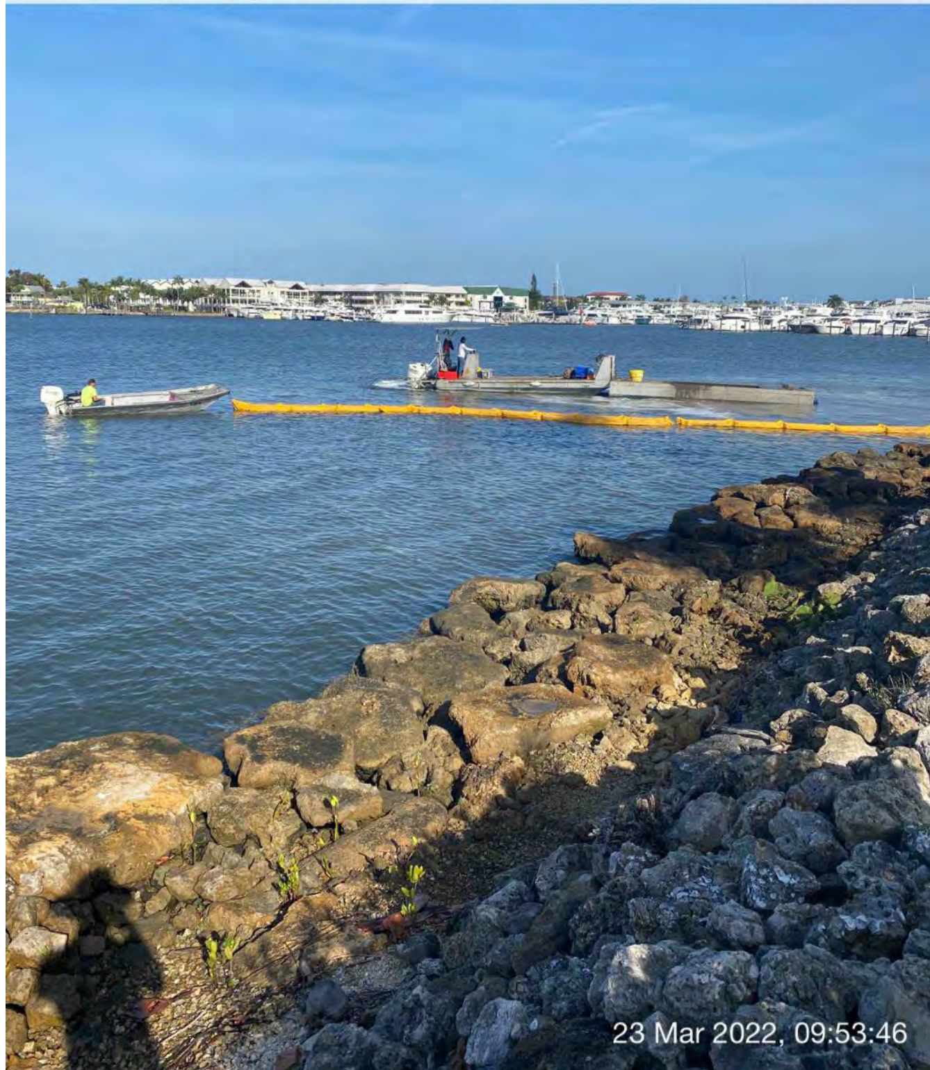
Support boat holding open curtain to allow push boat to exit Canal BB-BB and transport hopper to Canal CC-CC
