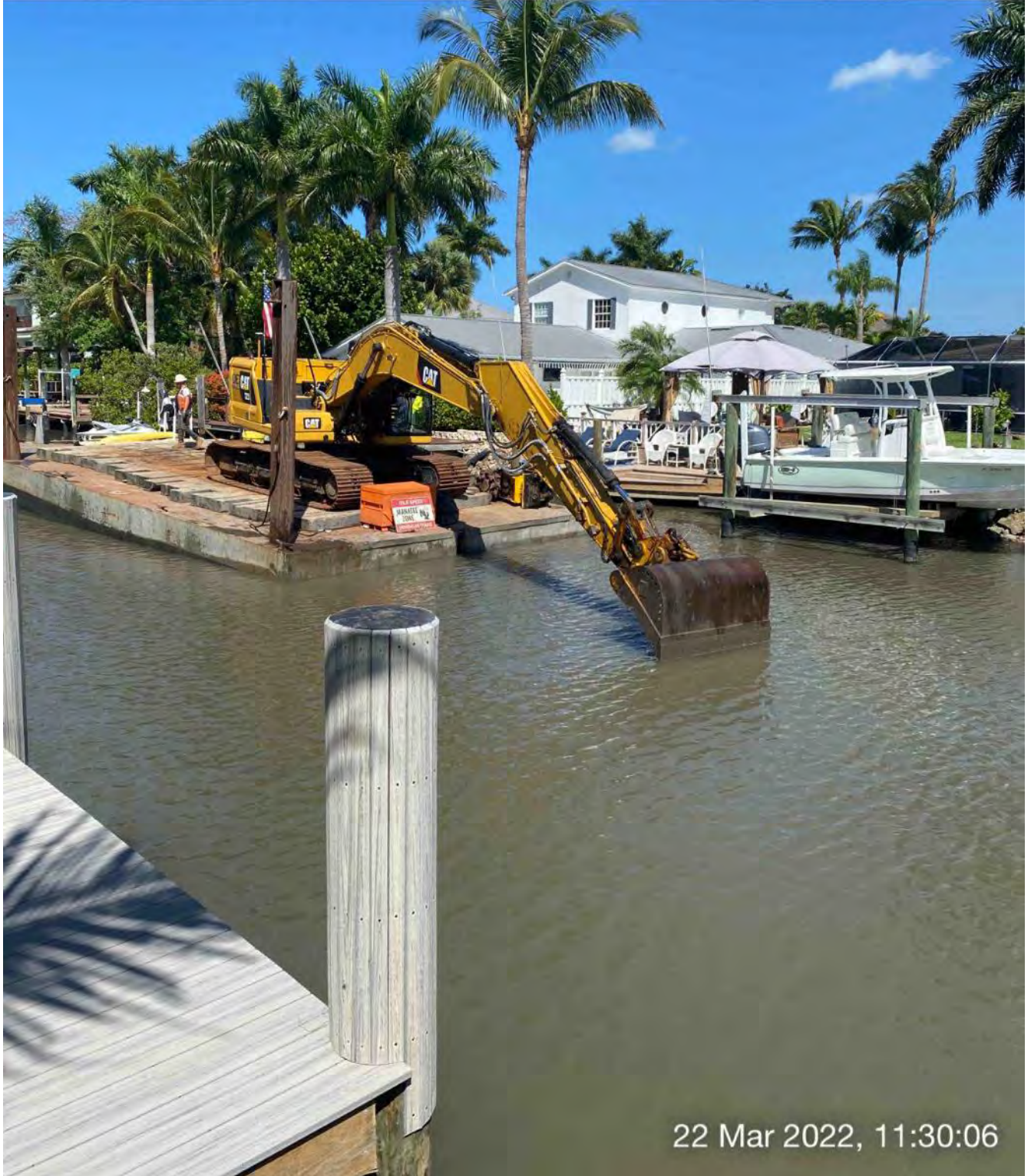
323 excavator removing material from station 9+00 and transferring to hopper
