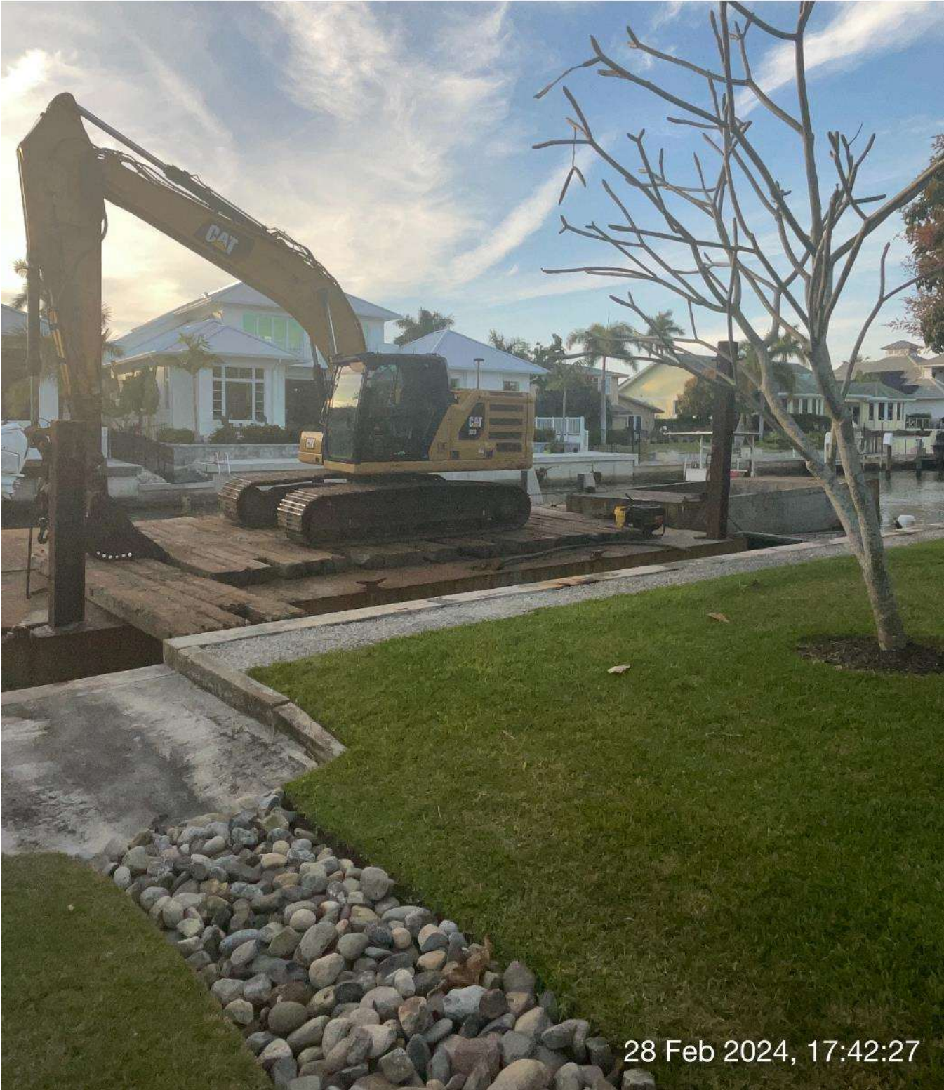
Equipment staged at station 6+00 in Canal A-A.
