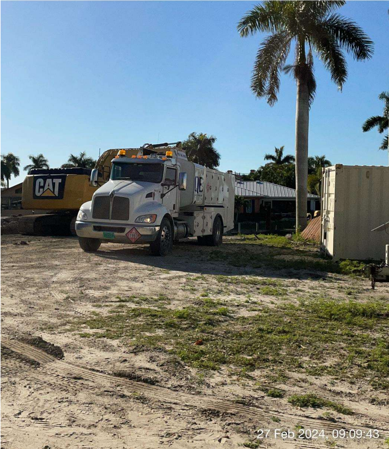
Mechanic arriving on site to service the 323 excavator.
