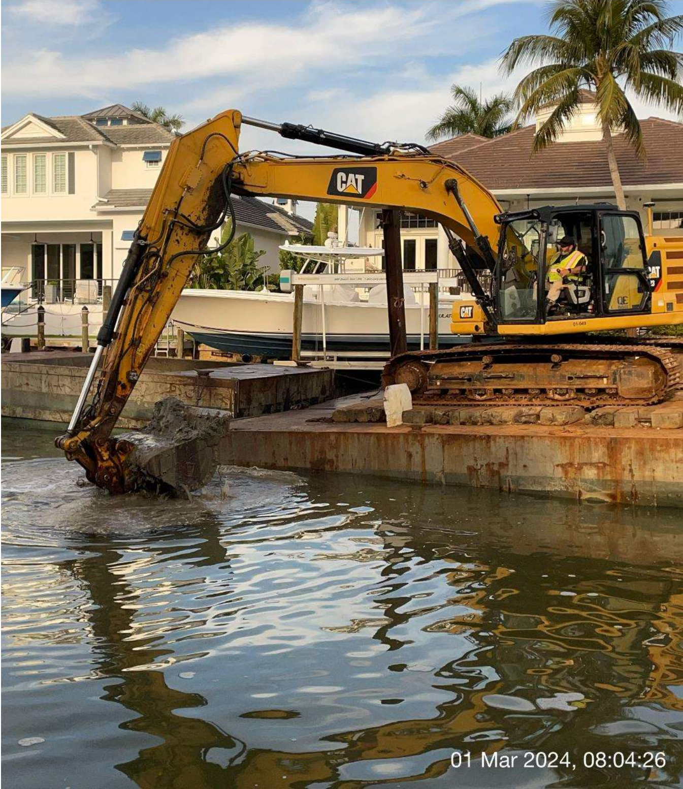
323 excavator removing sediment at station 10+00 in Canal A-A.
