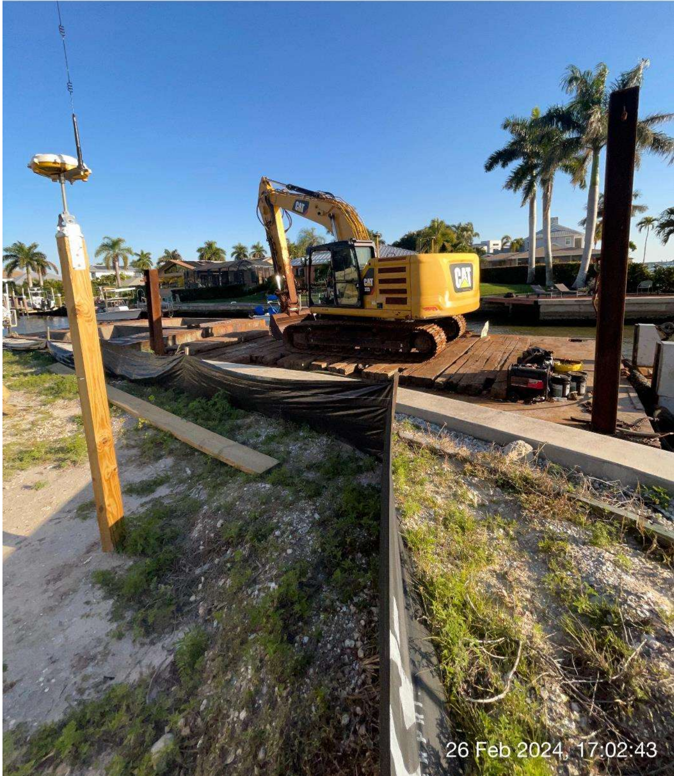
Equipment staged at station 1+00 in Canal CC-CC.
