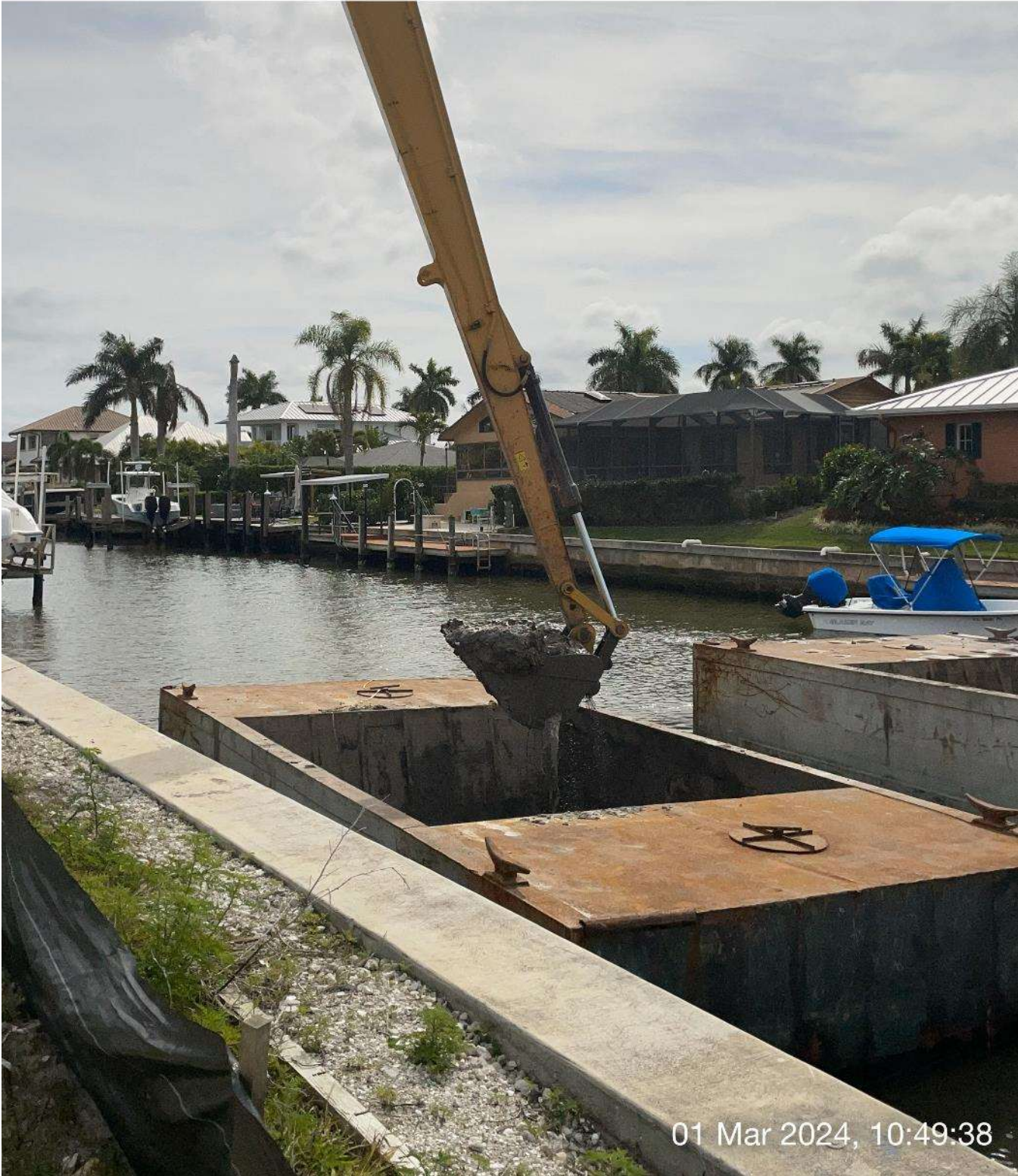
Long reach excavator removing sediment from hopper.
