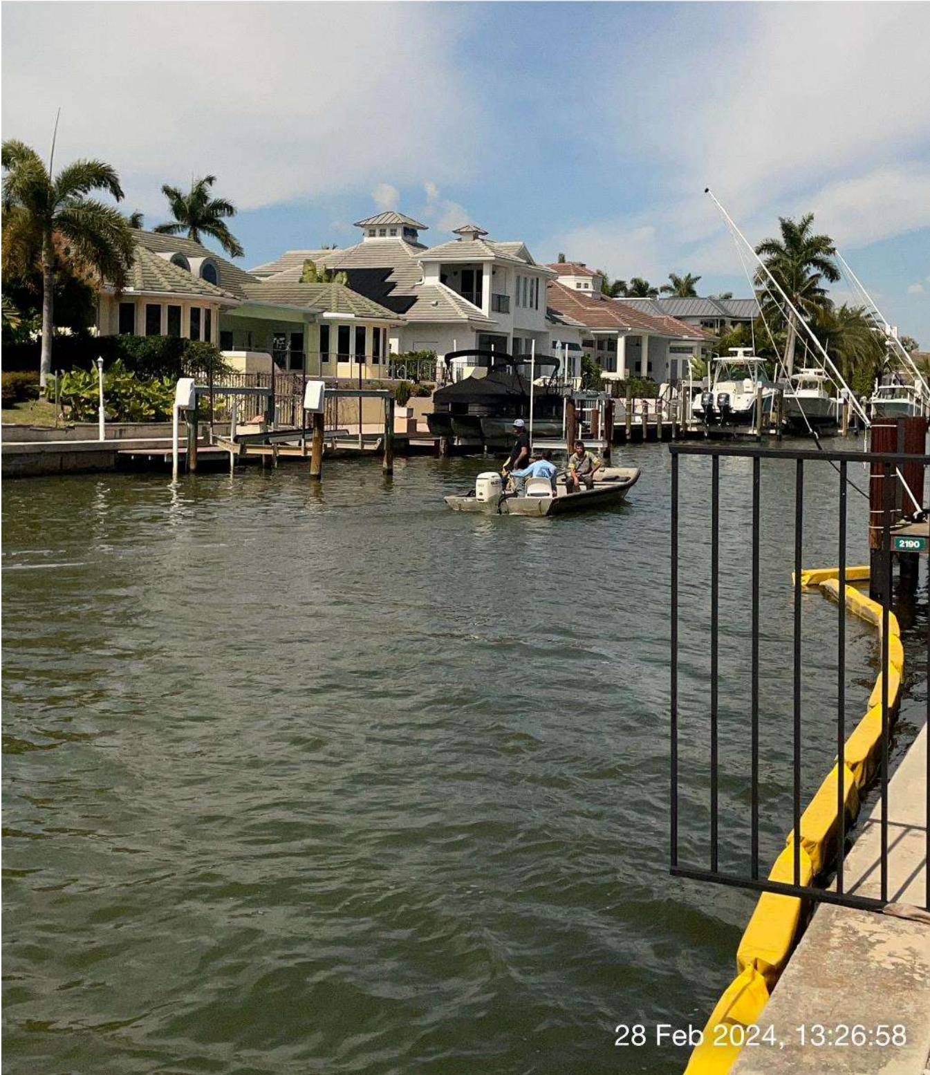
Contractor taking mechanic to the 323 excavator.
