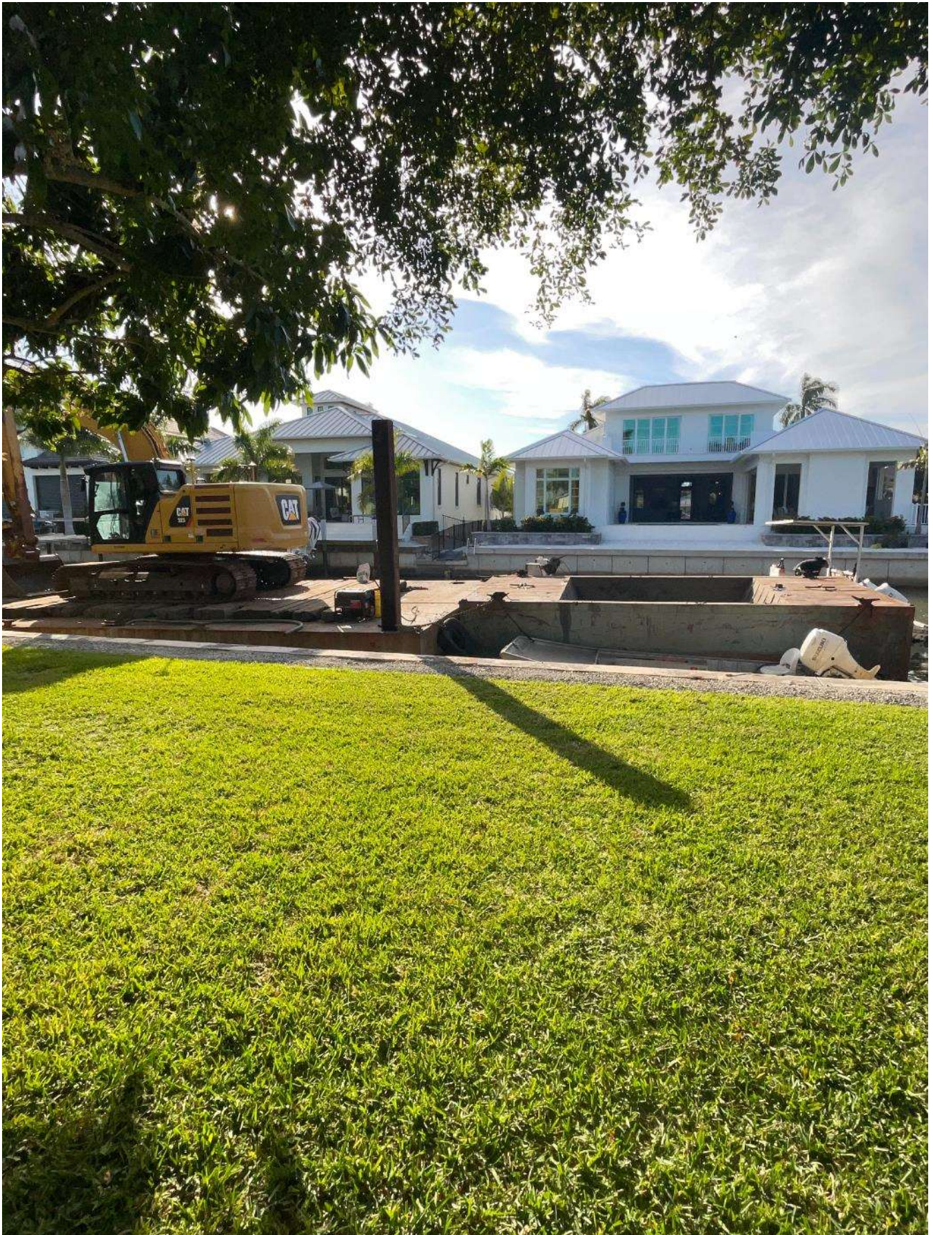
Equipment staged at station 6+00 in Canal A-A.
