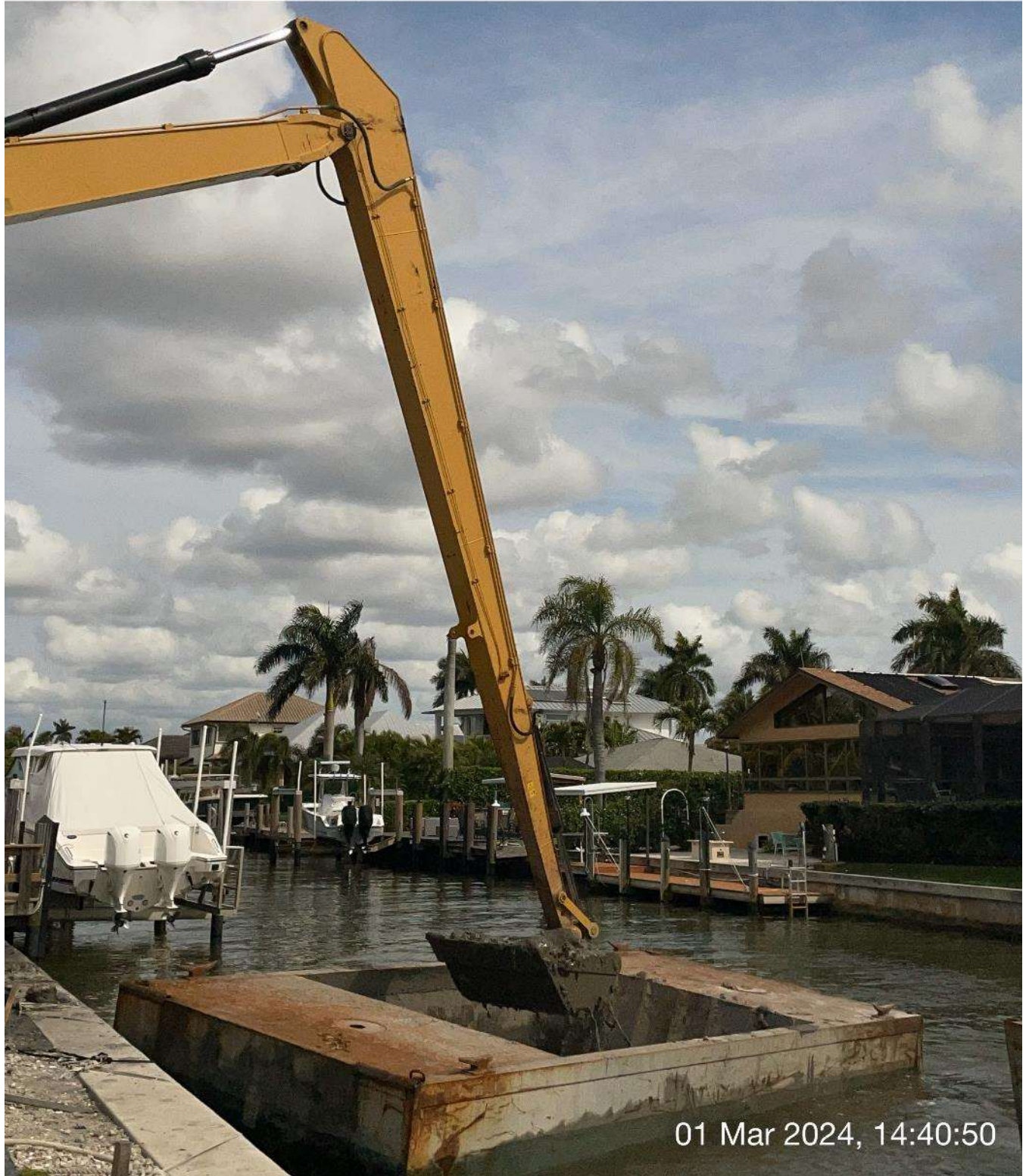
Long reach excavator removing sediment from hopper.
