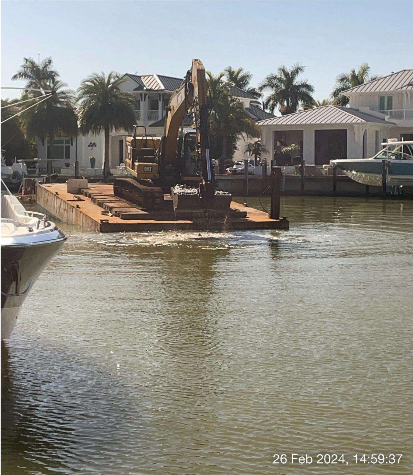
323 excavator removing sediment at station 11+25 in Canal A-A
