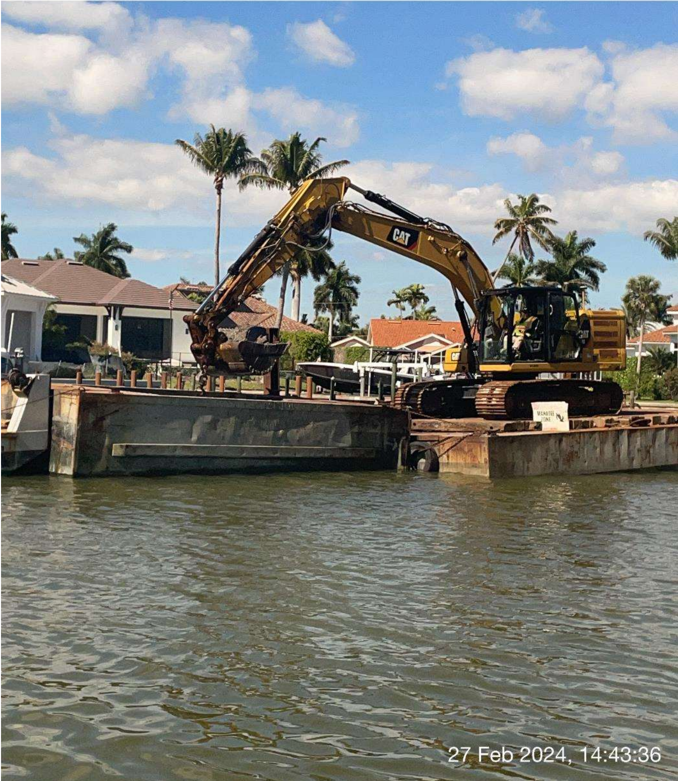
323 excavator removing sediment at station 11+00 in Canal A-A.
