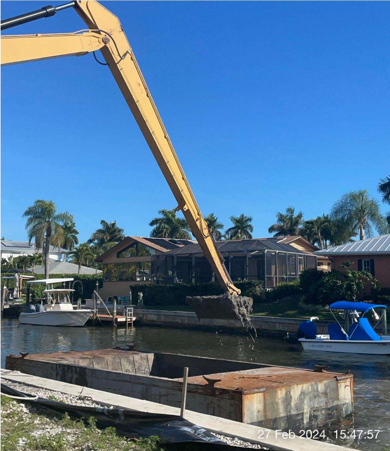
Long reach excavator removing sediment from hopper.
