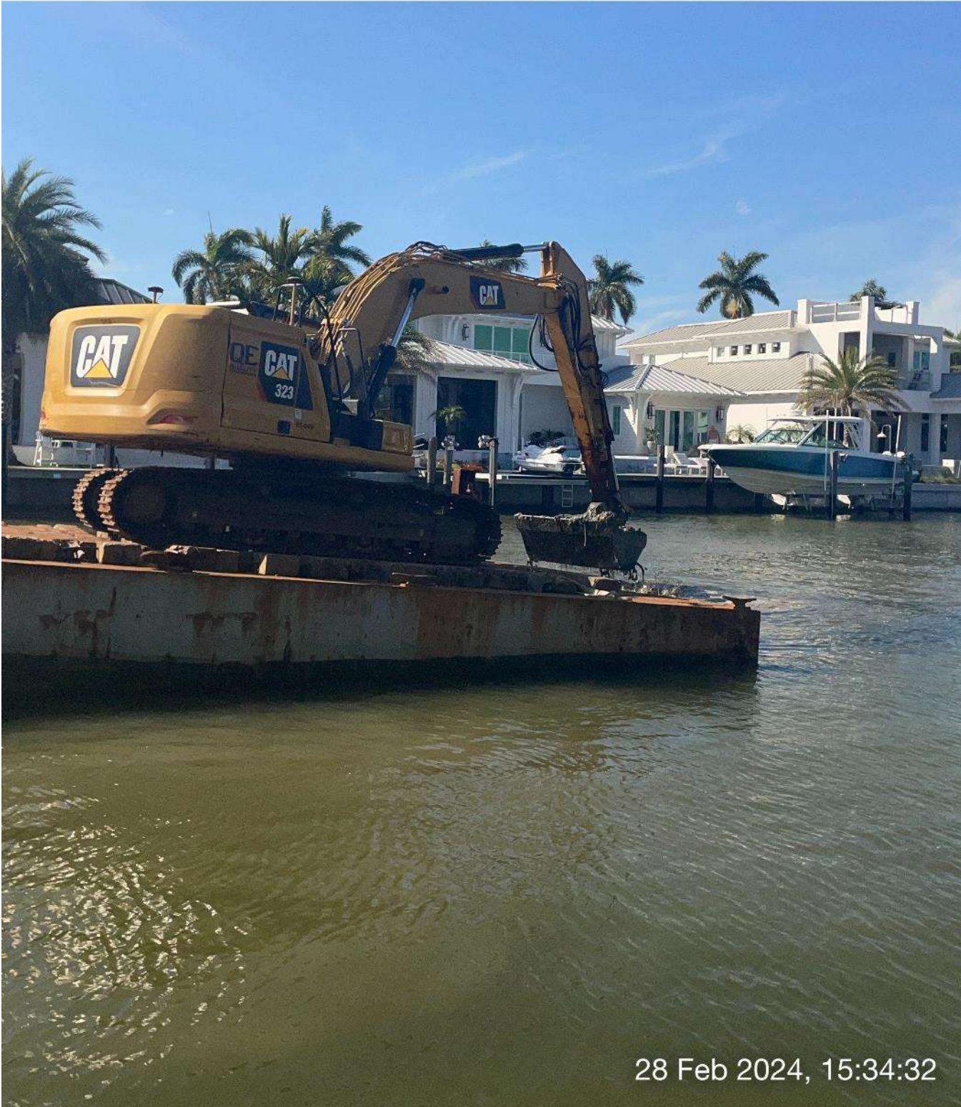
323 excavator removing sediment at station 10+50 in Canal A-A.
