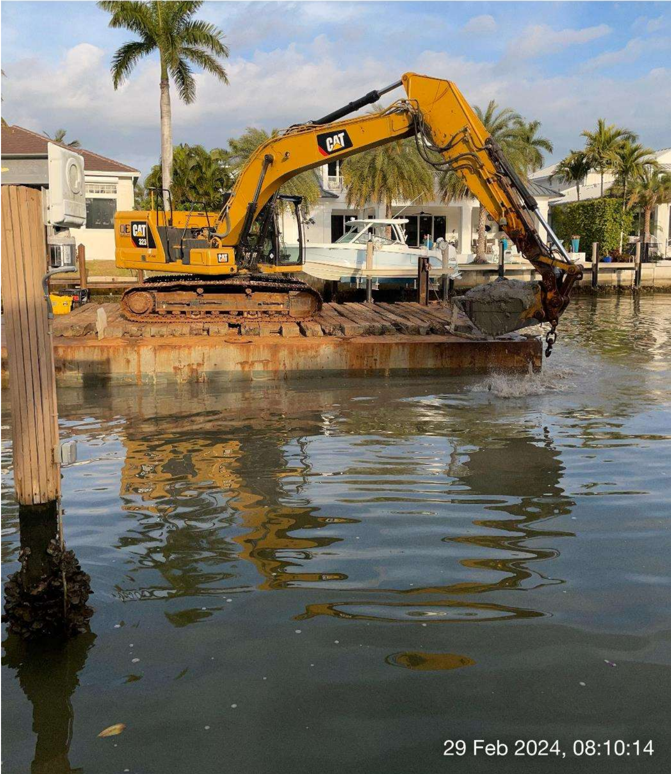
323 excavator removing sediment at station 10+25 in Canal A-A.
