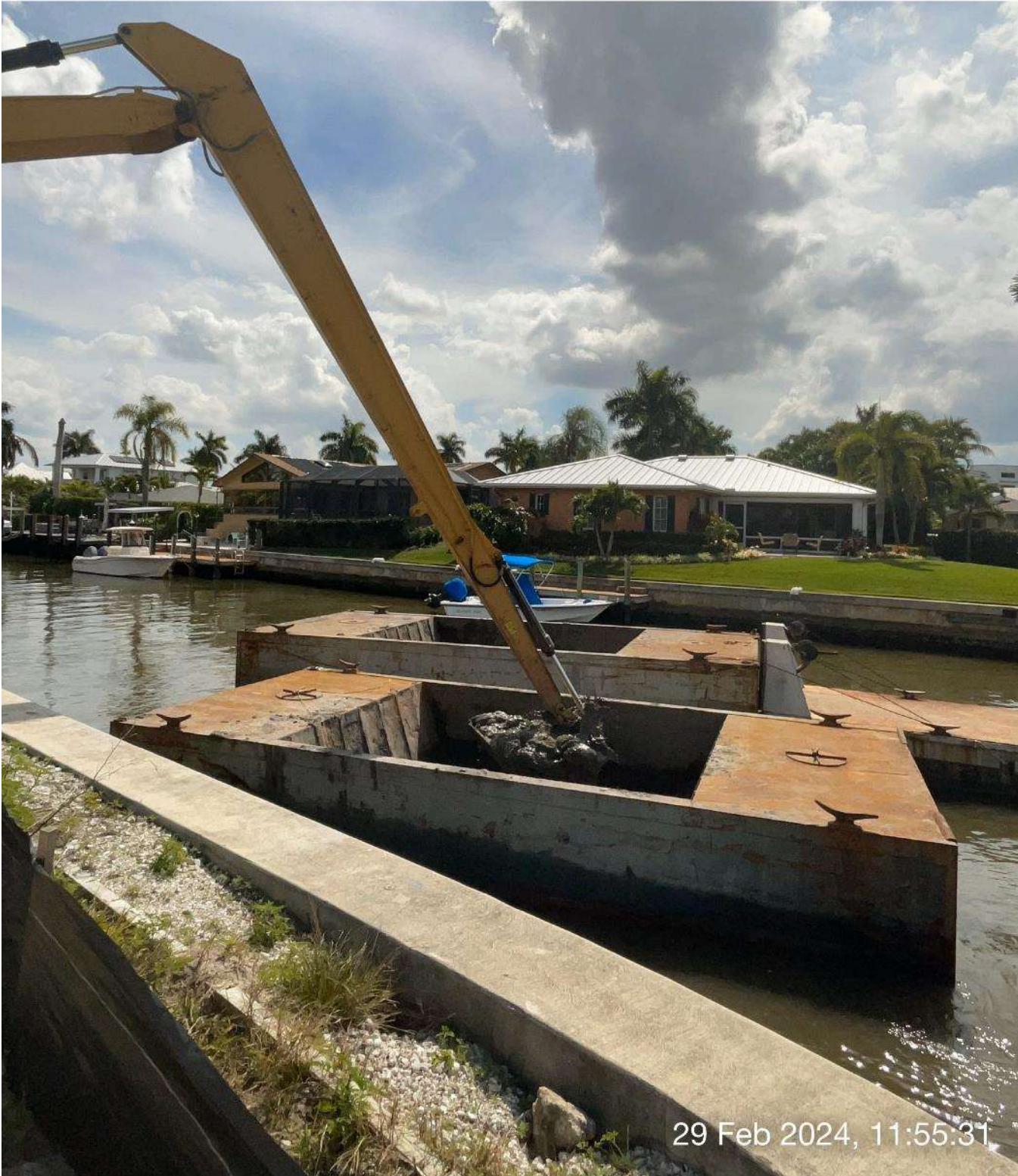
Long reach excavator removing sediment from hopper.
