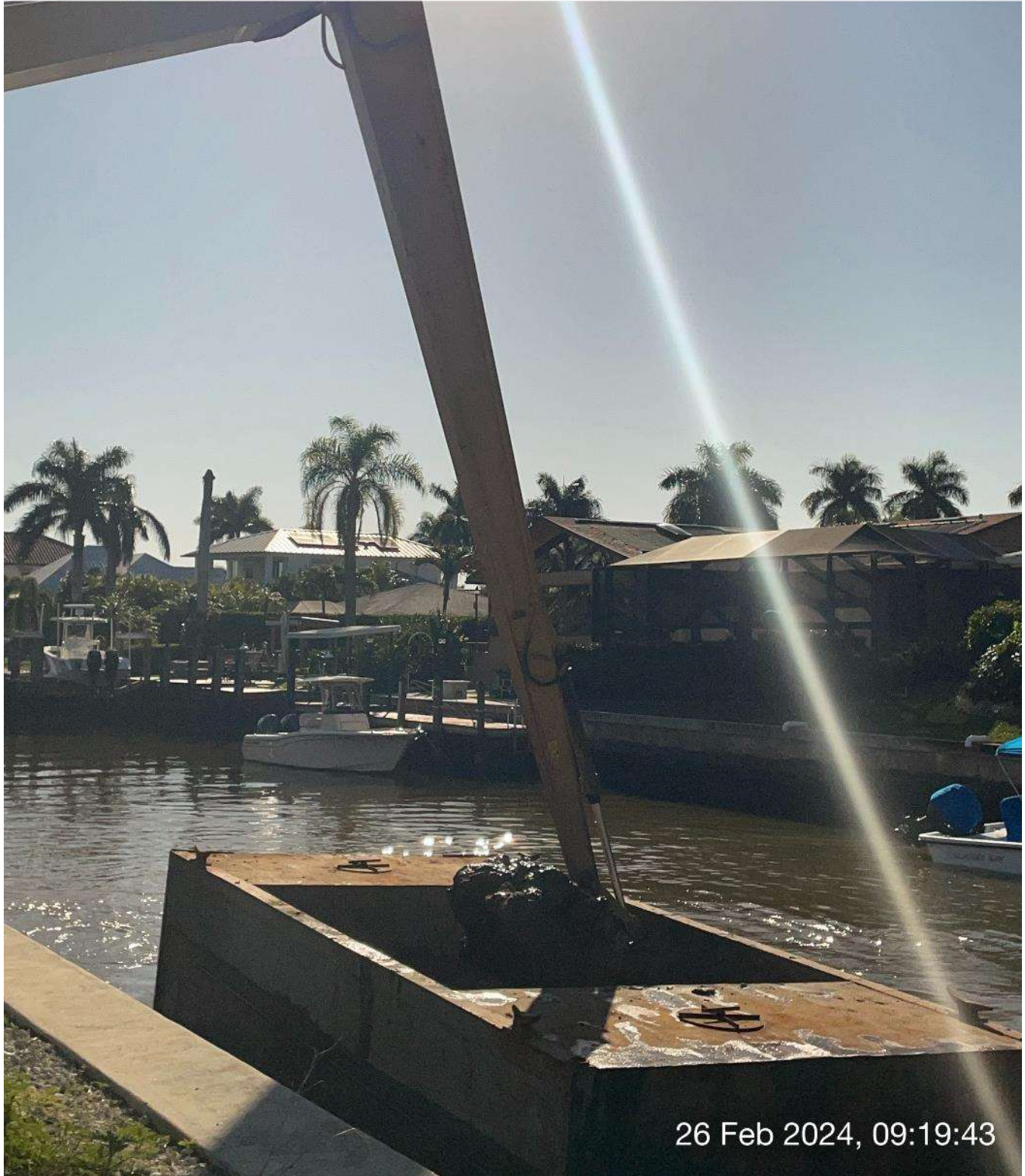
Long reach excavator removing sediment from hopper.
