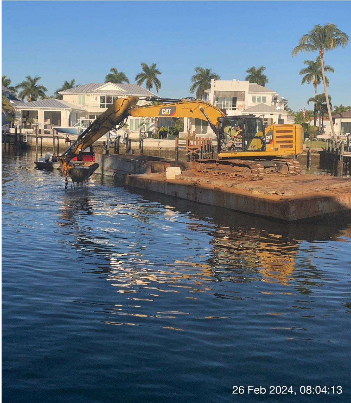
323 excavator removing sediment at station 12+75 in Canal A-A.
