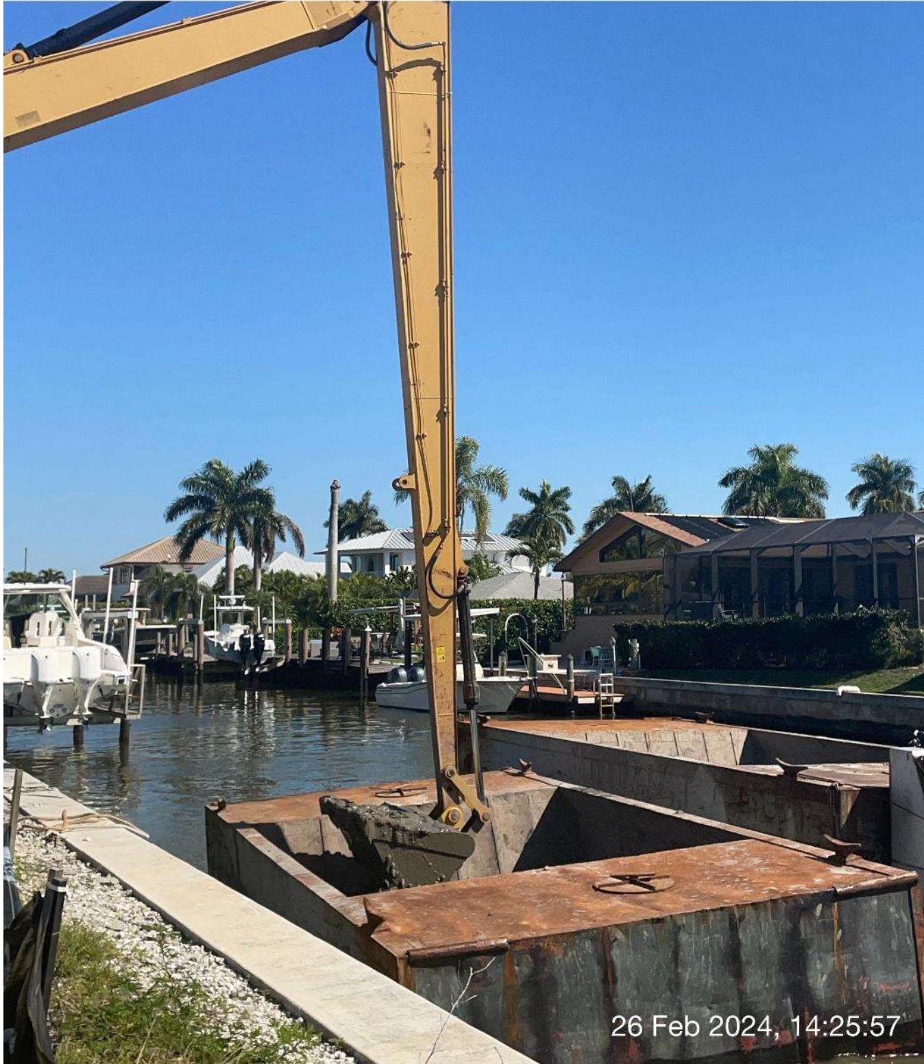
Long reach excavator removing sediment from hopper.
