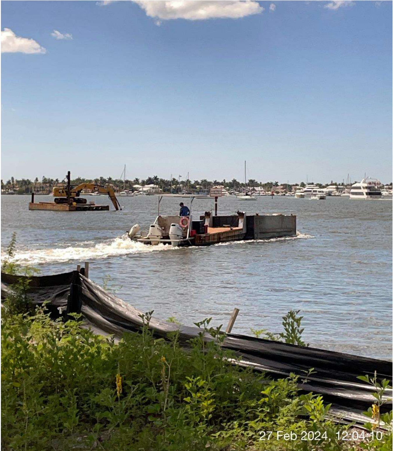
Push boat moving hopper out of Canal CC-CC to transport to Canal A-A.
