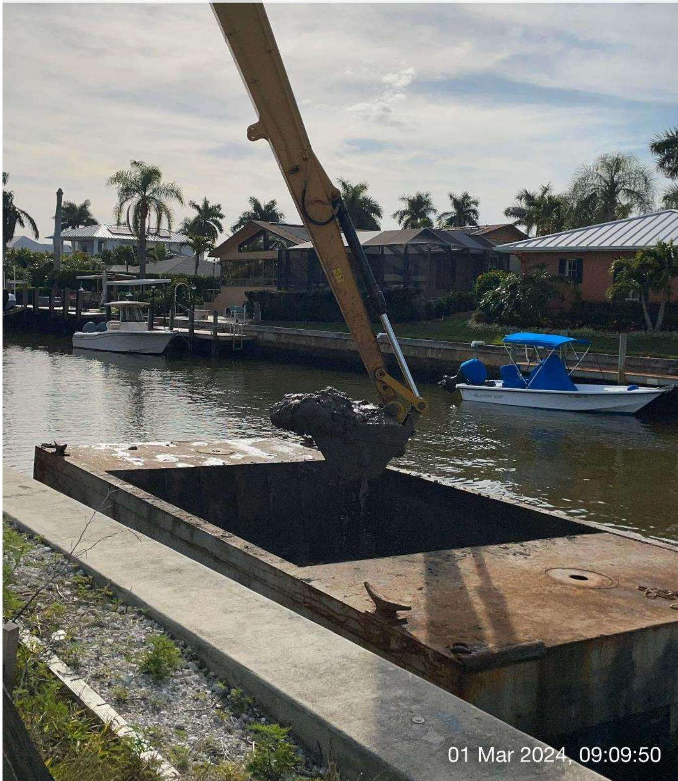
Long reach excavator removing sediment from hopper.
