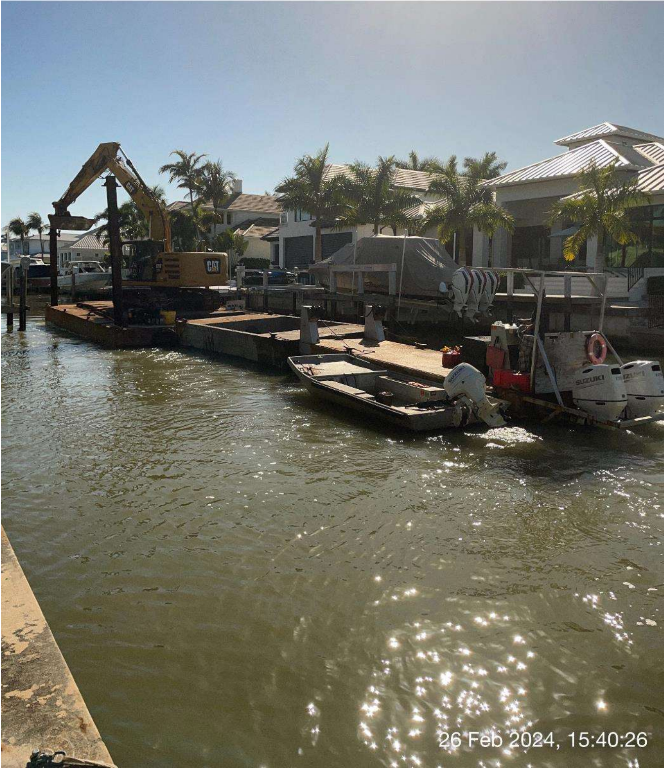
Push boat taking hopper and barge to staging area.
