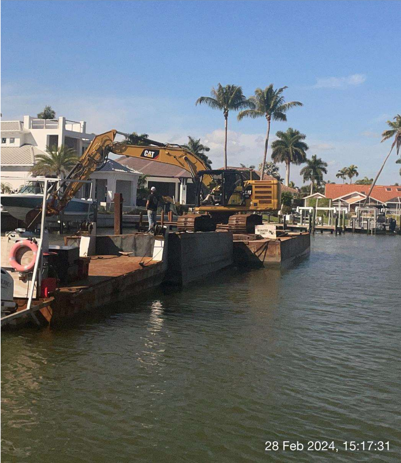
Contractor testing the GPS system in the 323 excavator.
