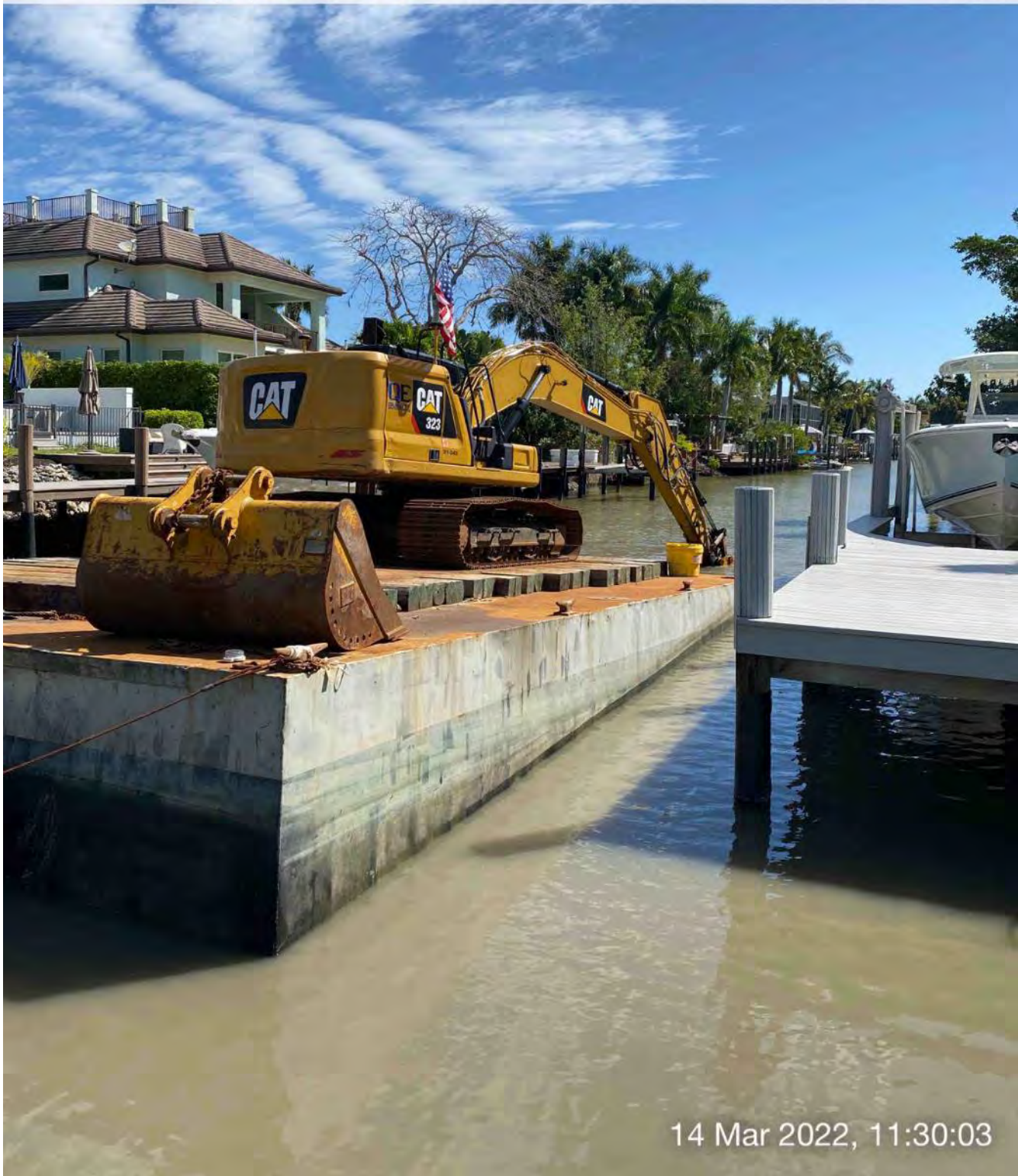
323 excavator grinding rock at station 5+00
