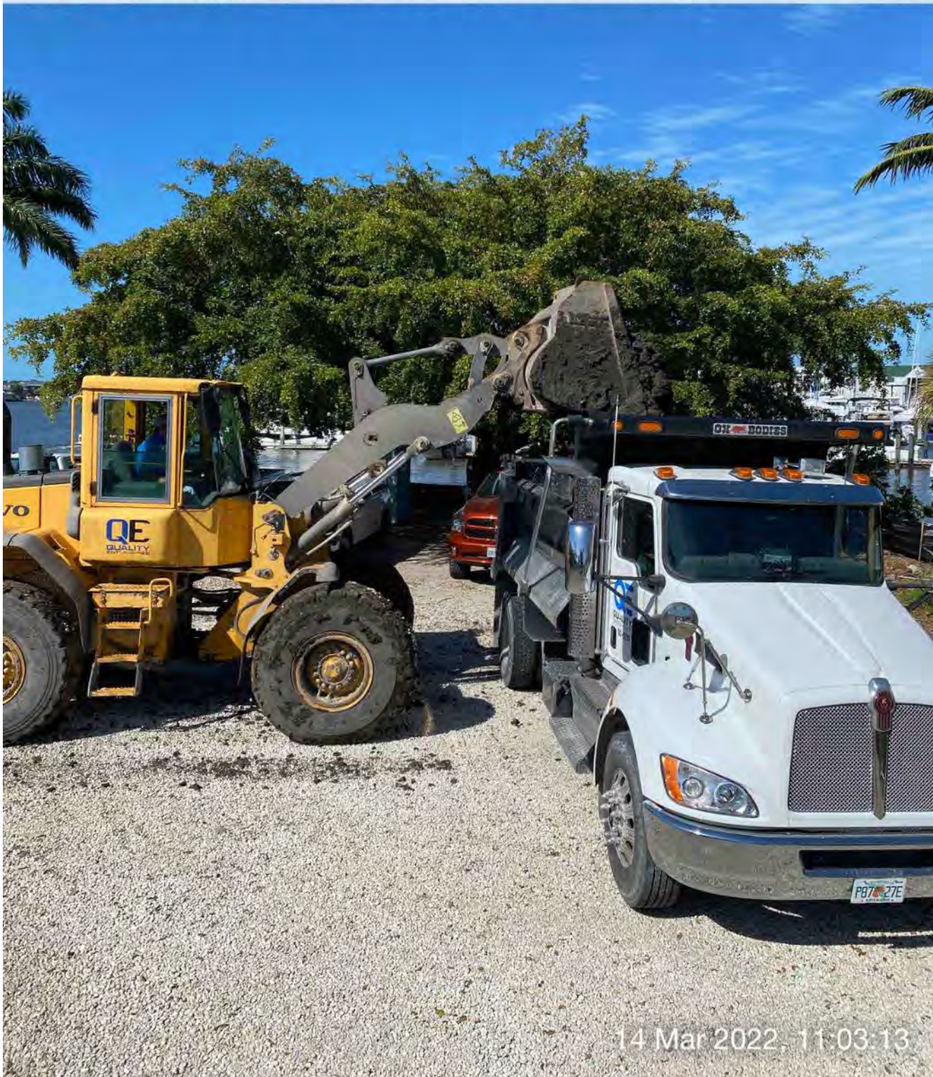
Using front end loader to transfer removed material from dewatering site to dump truck bed
