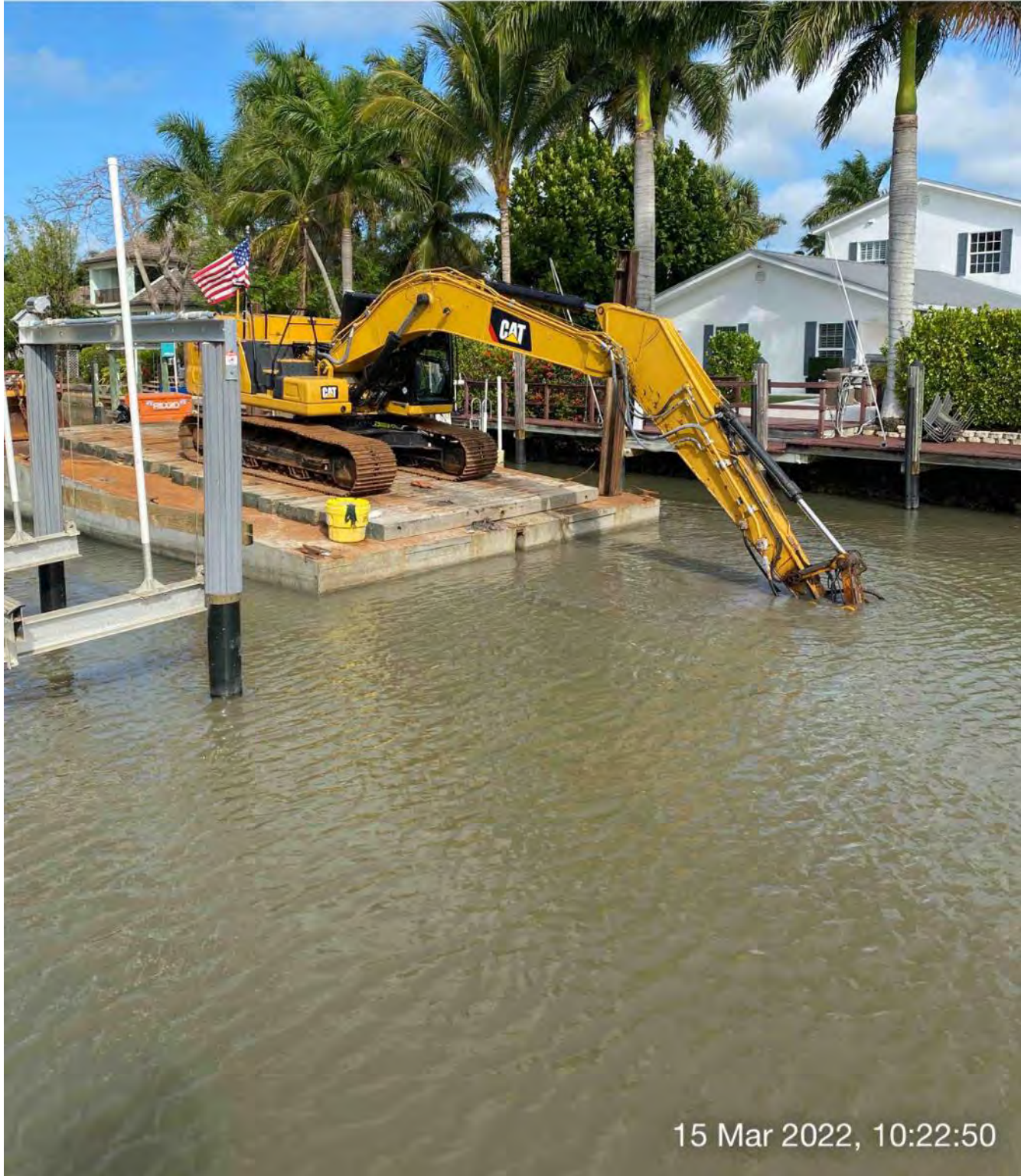
323 excavator grinding rock at station 8+25
