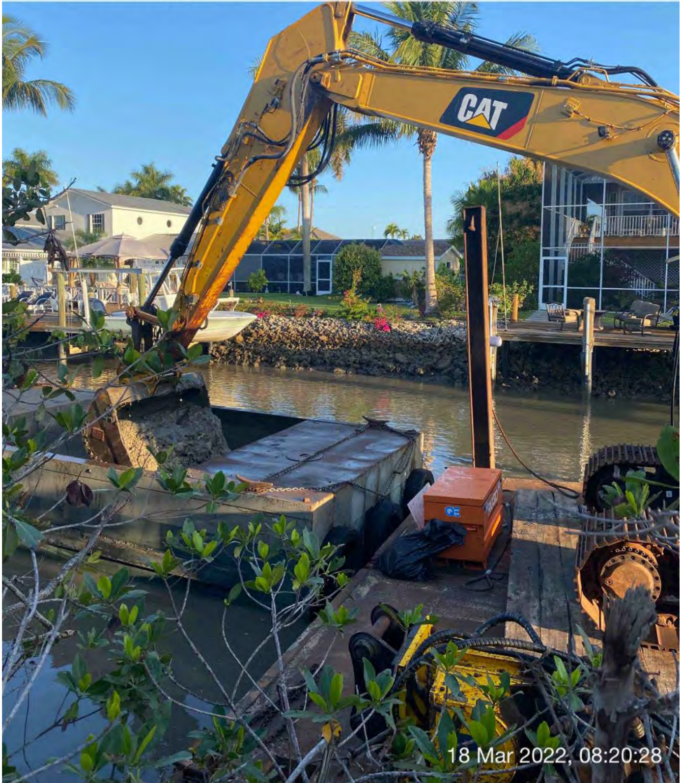
323 excavator removing material and transferring to hopper at station 10+50
