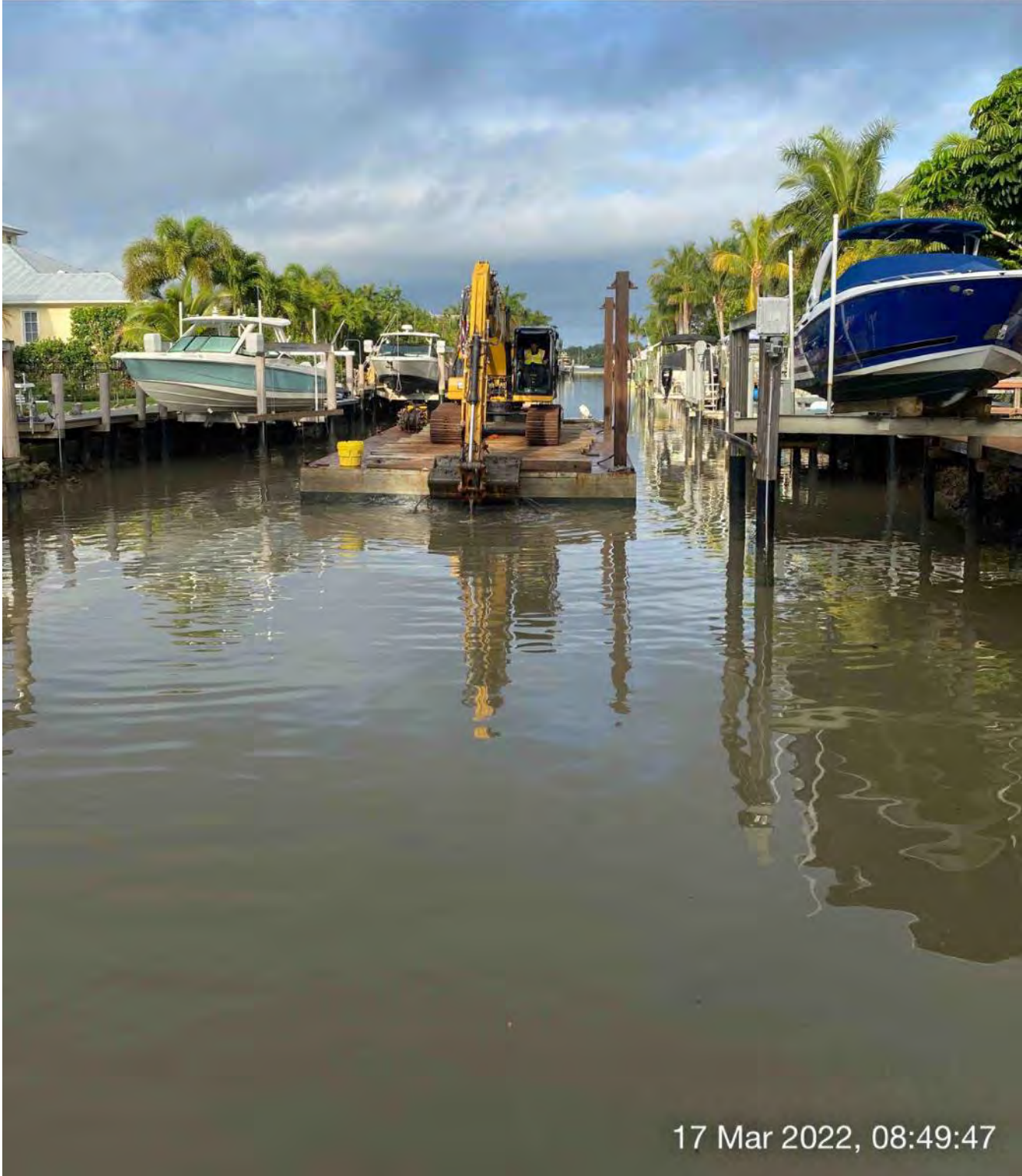
323 excavator removing material at station 11+50
