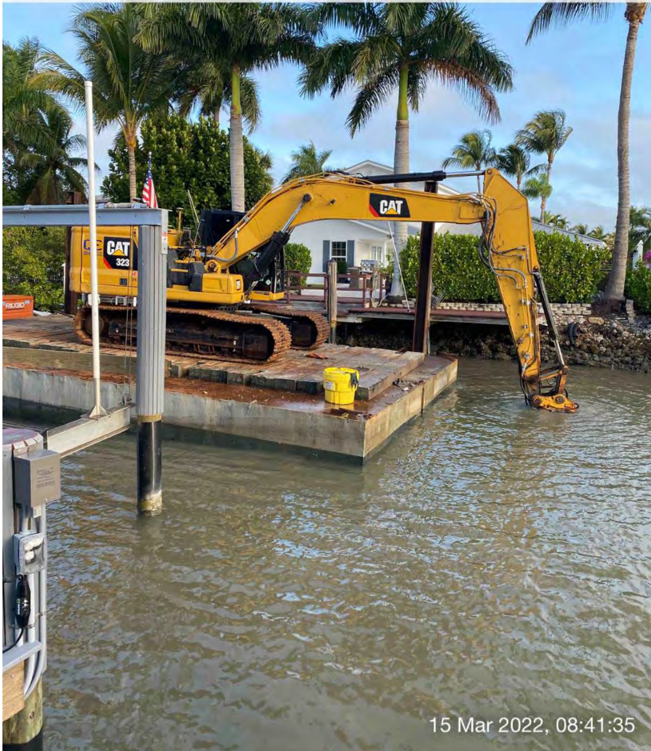
323 excavator grinding rock at station 8+00
