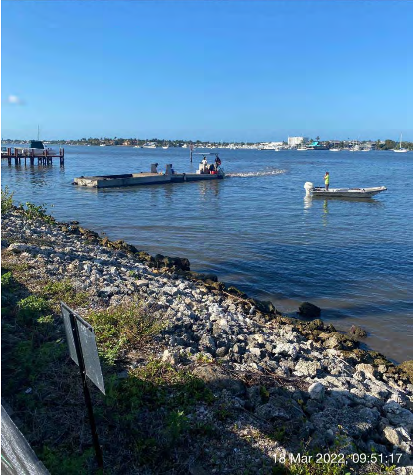
Push boat transporting full hopper of removed material from Canal BB-BB to Canal CC-CC
