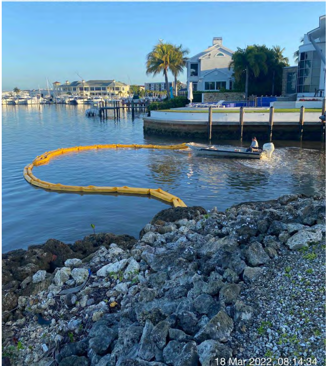
Installing turbidity curtain across the mouth of Canal BB-BB with support boat
