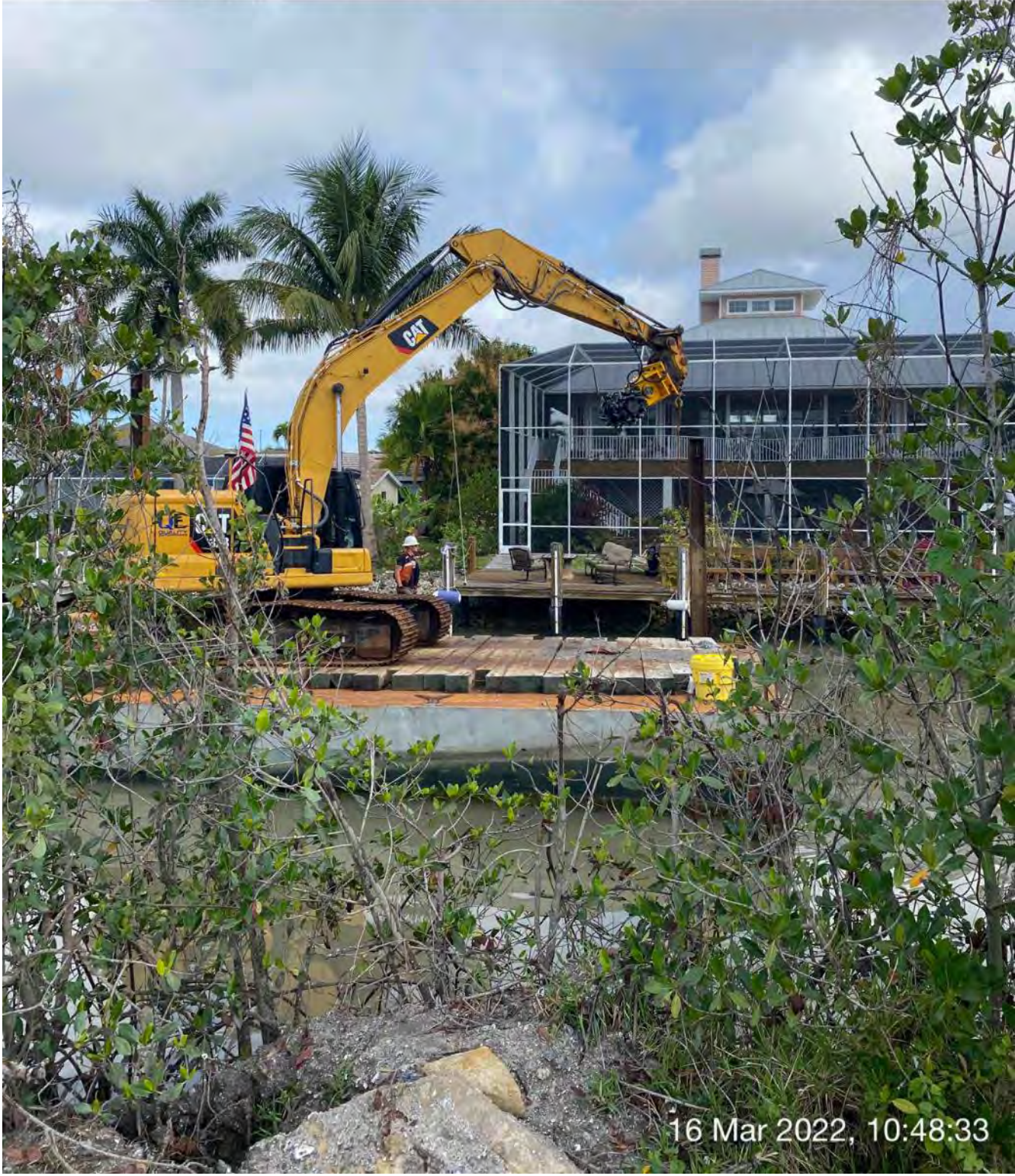
323 excavator lifting spud to allow push boat to mobilize barge at station 9+00
