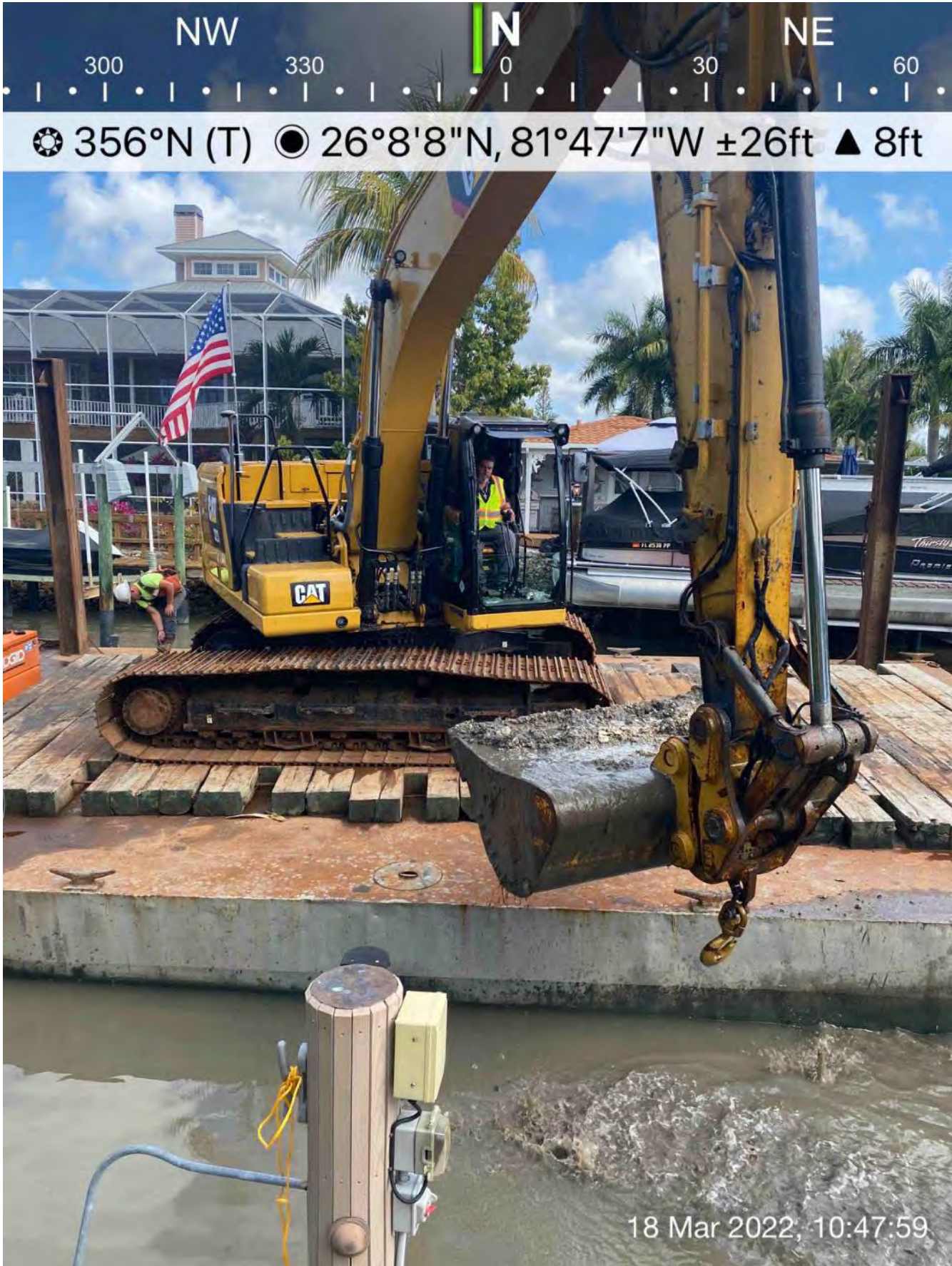
323 excavator removing material from station 10+00
