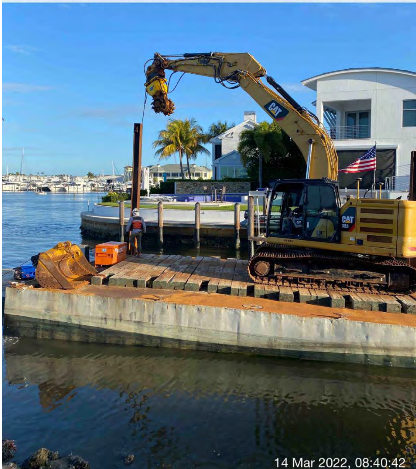
323 excavator lifting spud to allow push boat to mobilize barge at station 1+50
