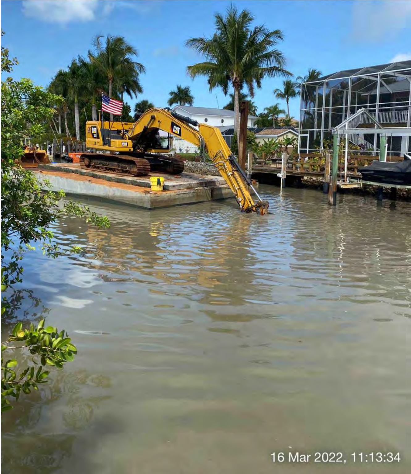
323 excavator grinding rock at station 9+50
