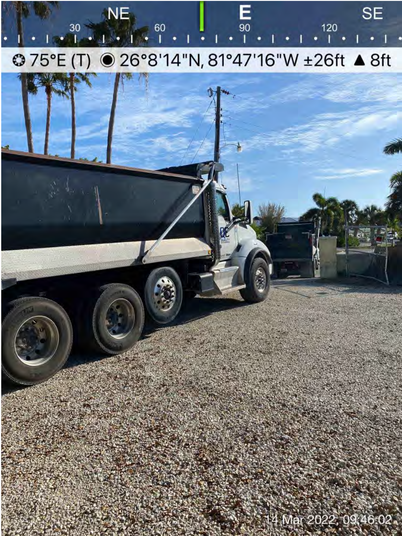
Two dump trucks entering site at 1300 Curlew Avenue
