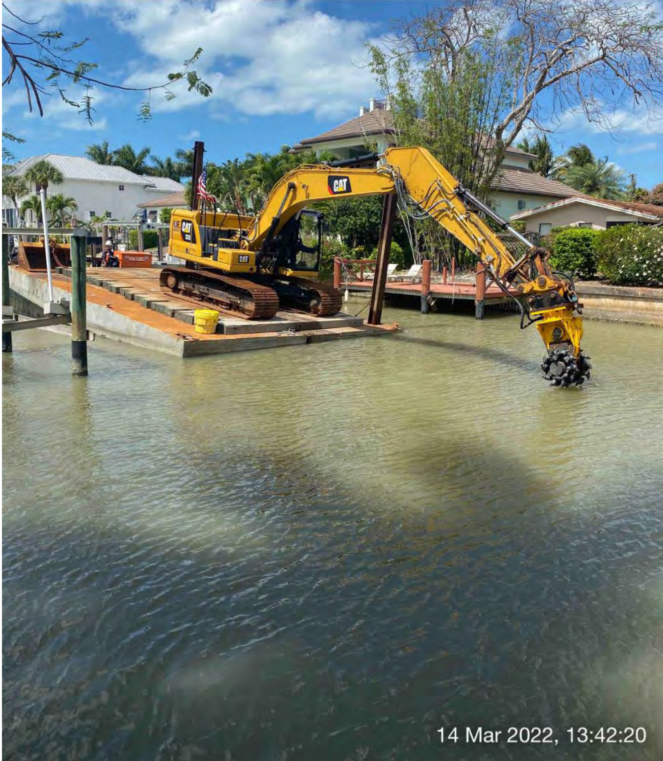
323 excavator grinding rock at station 6+50
