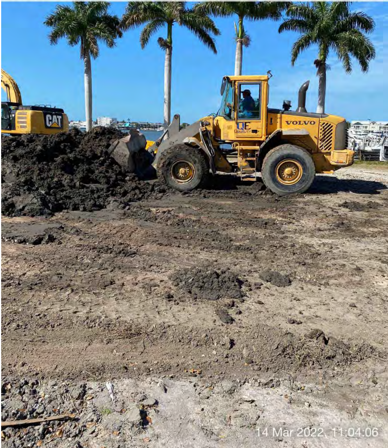
Front end loader removing material from the dewatering site
