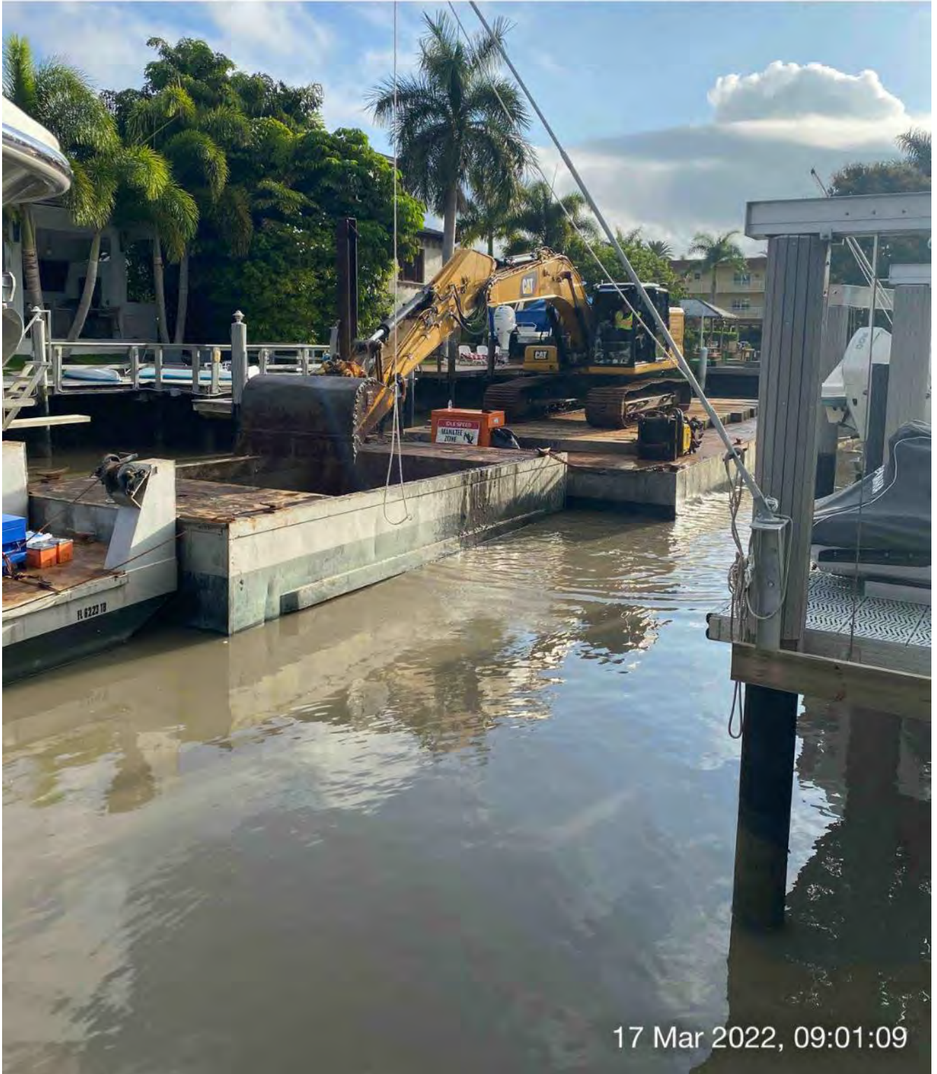
323 excavator transferring material to hopper at station 11+00
