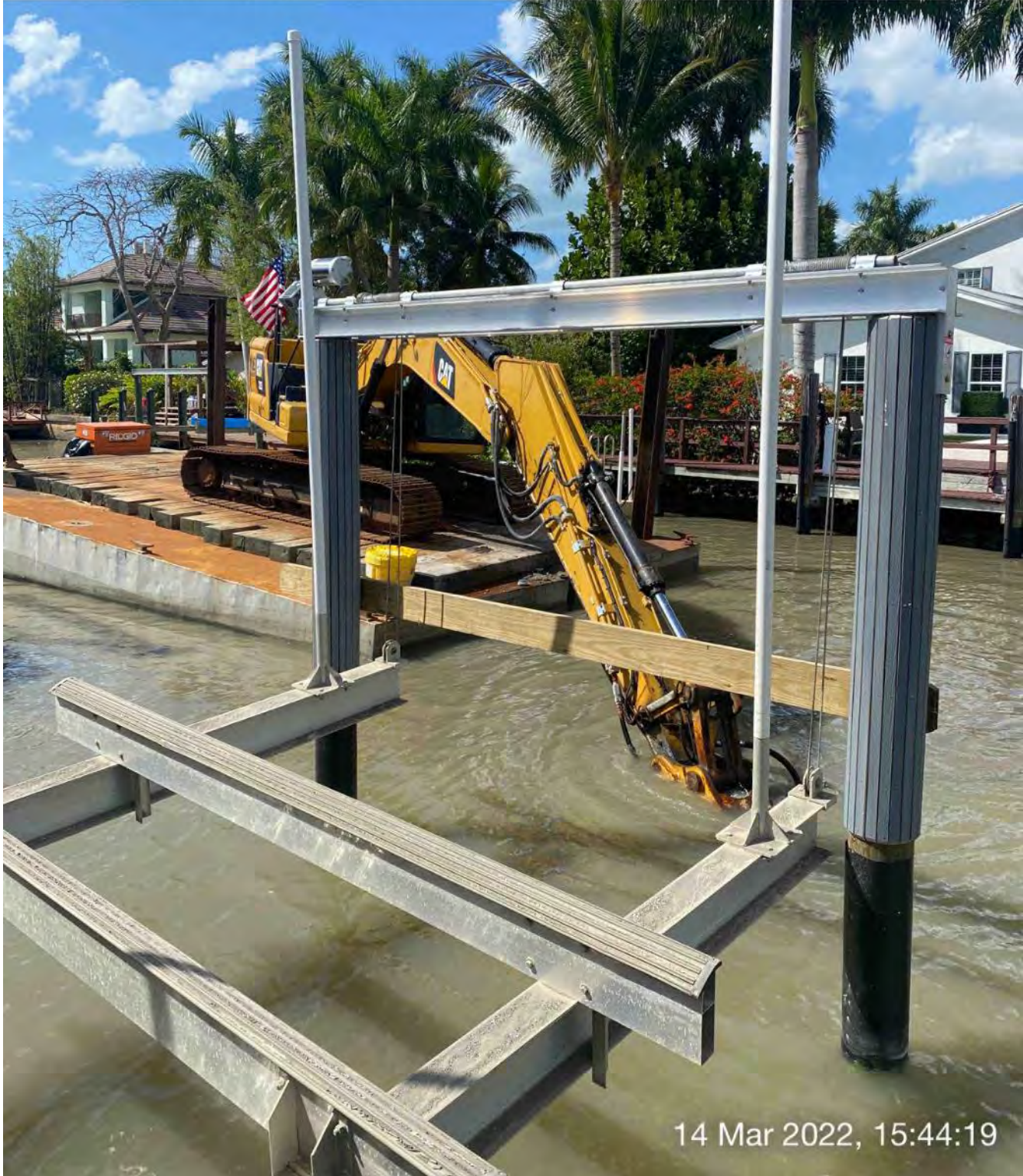
323 excavator grinding rock at station 8+00
