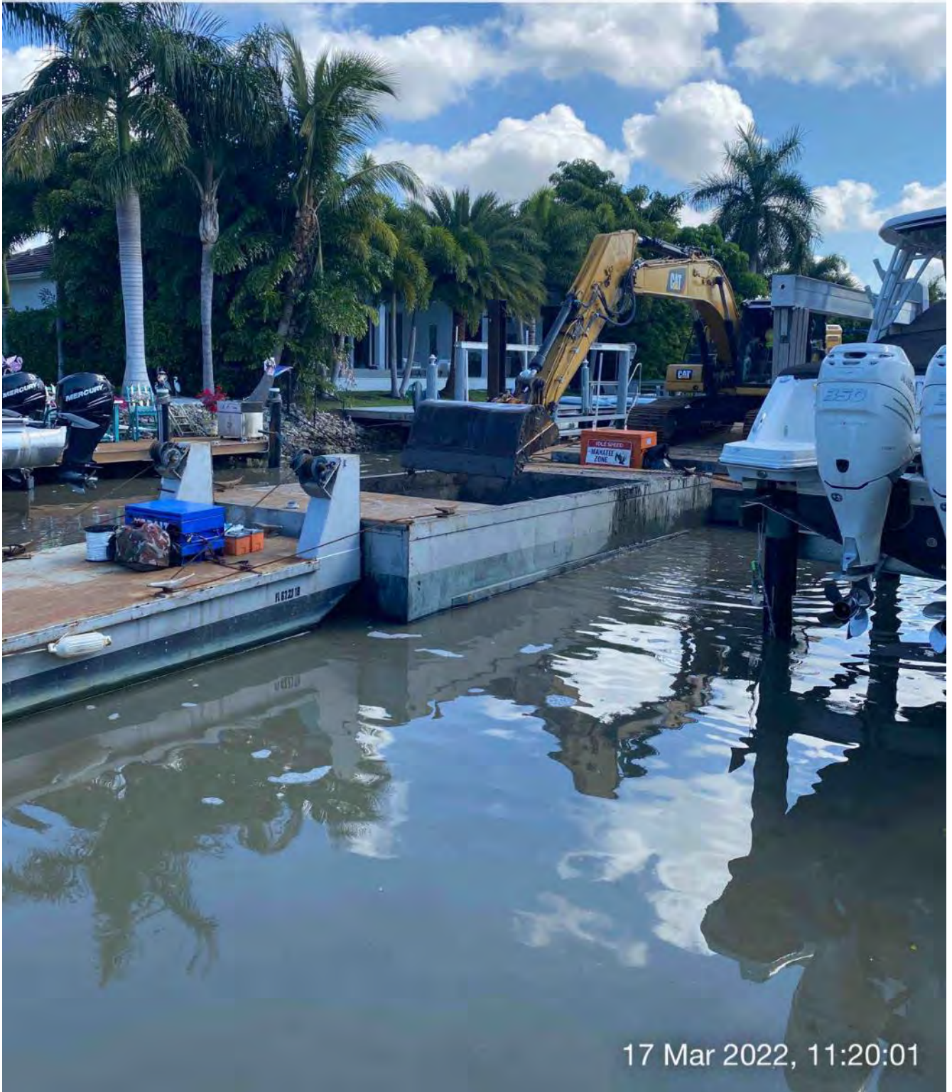
323 excavator transferring material to hopper at station 10+50
