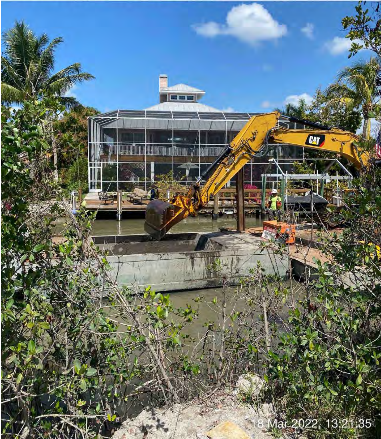
323 excavator removing material and transferring to hopper at station 9+50
