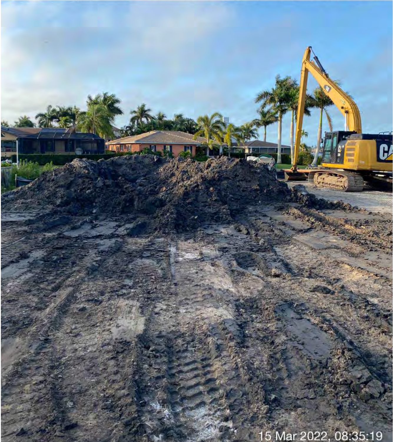
Removed material at dewatering site at 1300 Curlew Avenue
