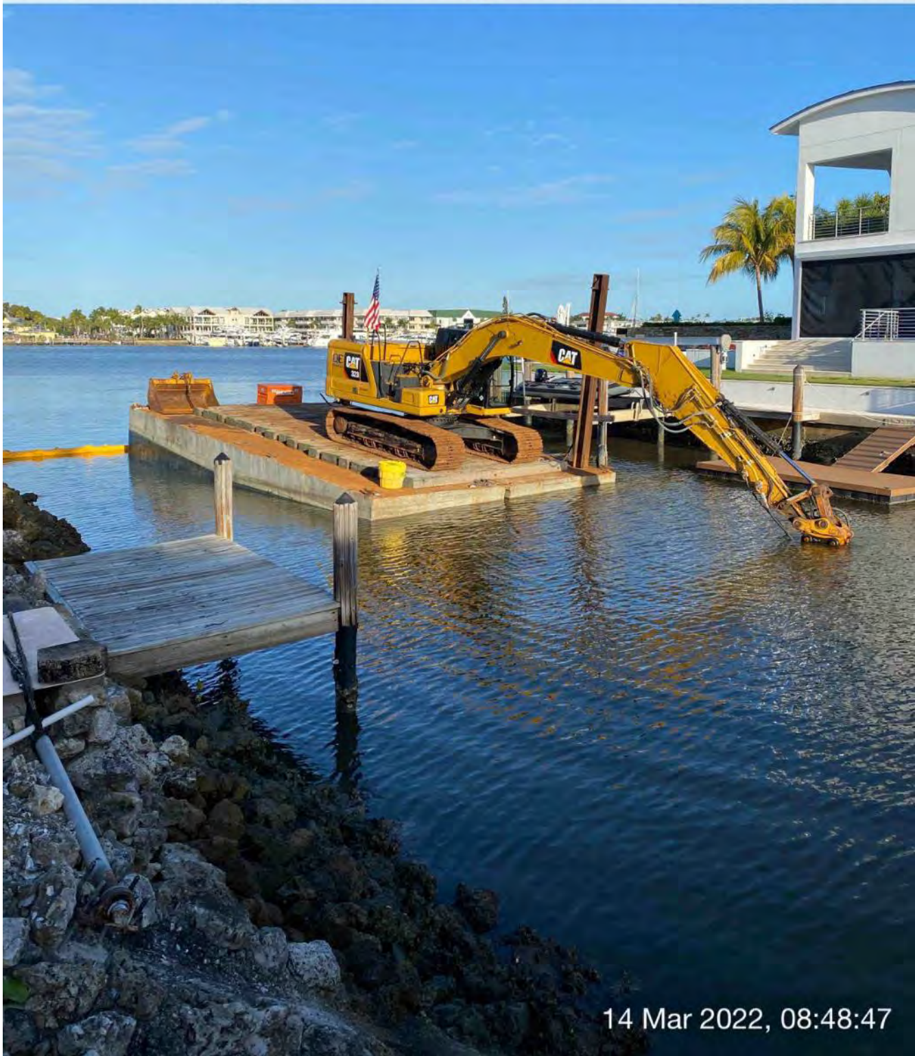
323 excavator grinding rock at station 1+75
