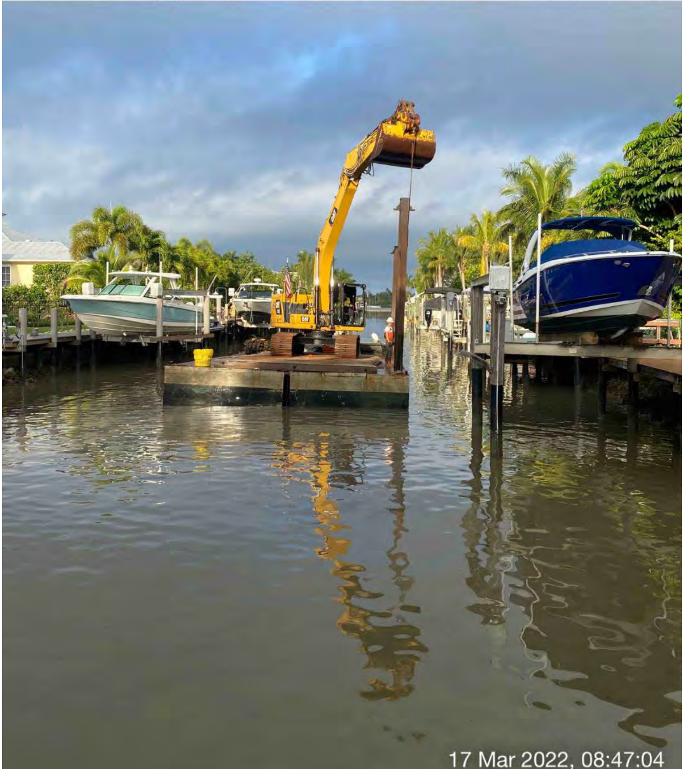
323 excavator lifting spud to allow push boat to mobilize barge at station 11+00
