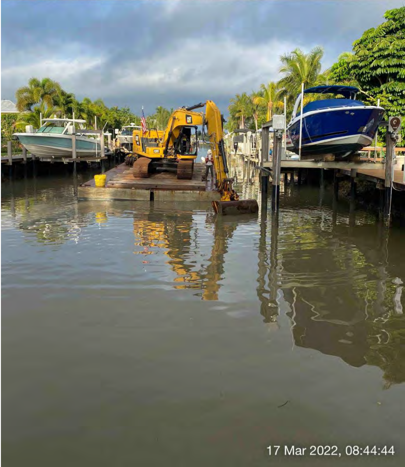
323 excavator removing material at station 11+50
