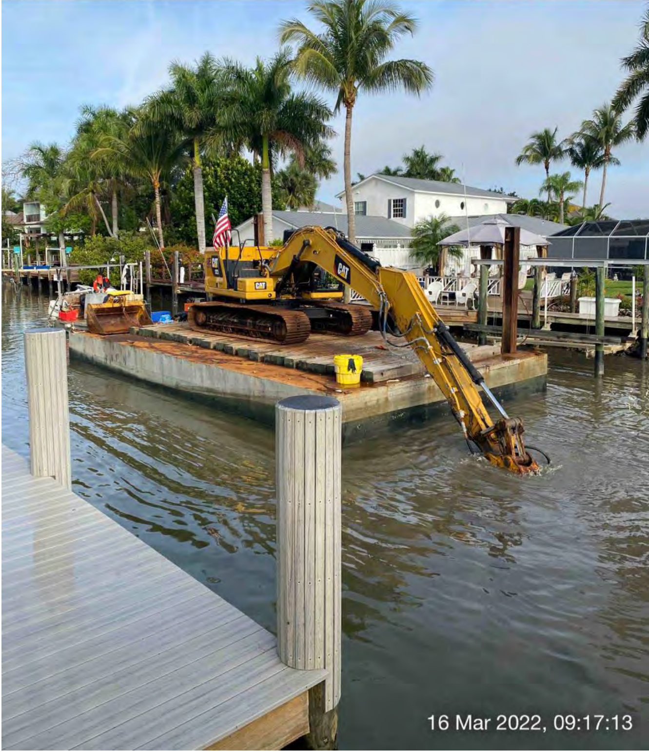
323 excavator grinding rock at station 8+00
