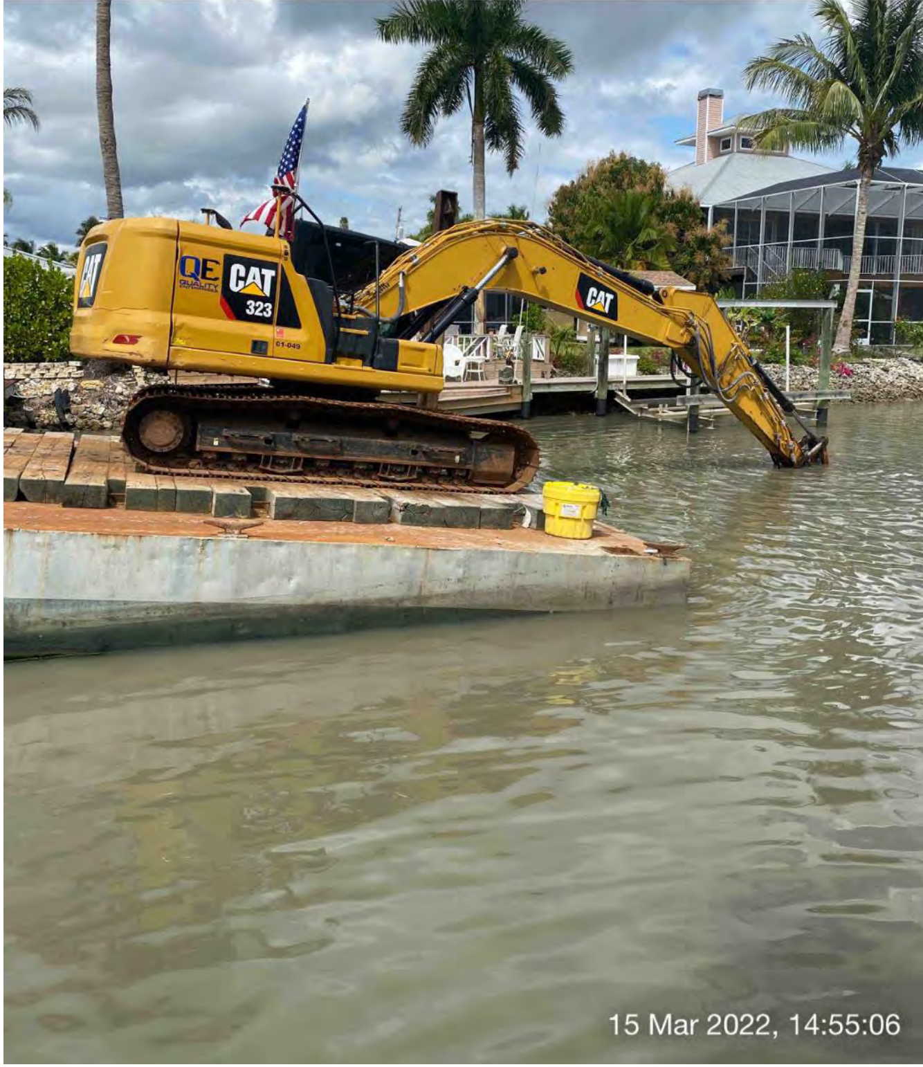
323 excavator grinding rock at station 8+50
