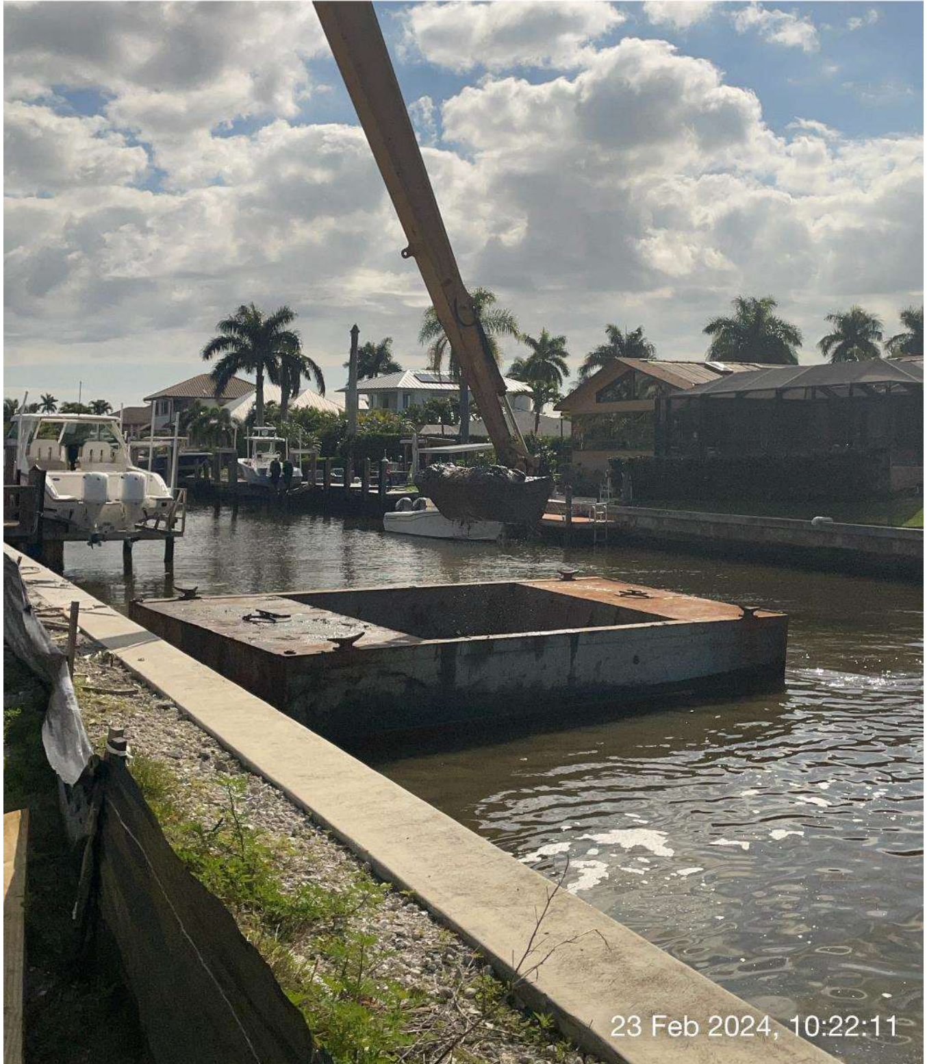
Long reach excavator removing sediment from hopper.
