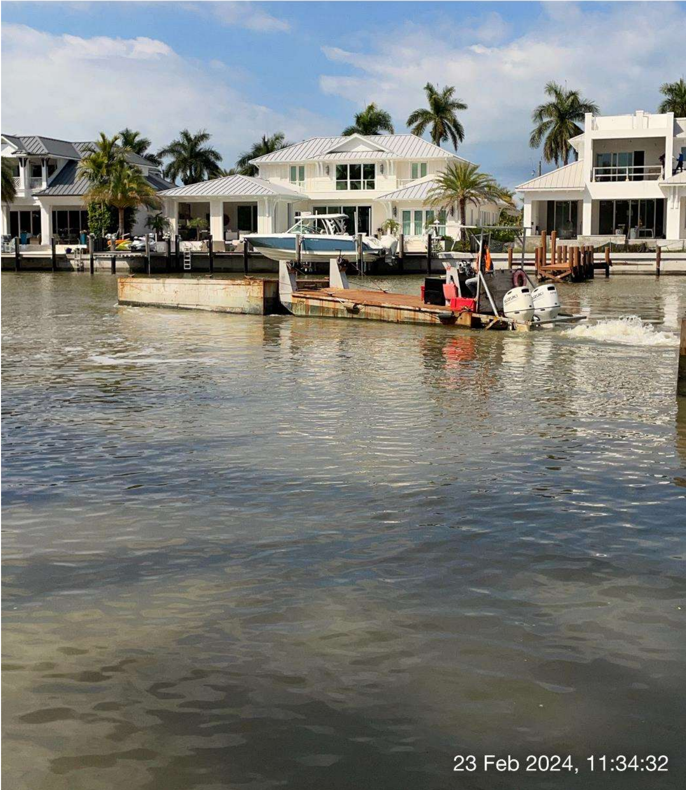
Push boat taking hopper to staging area.
