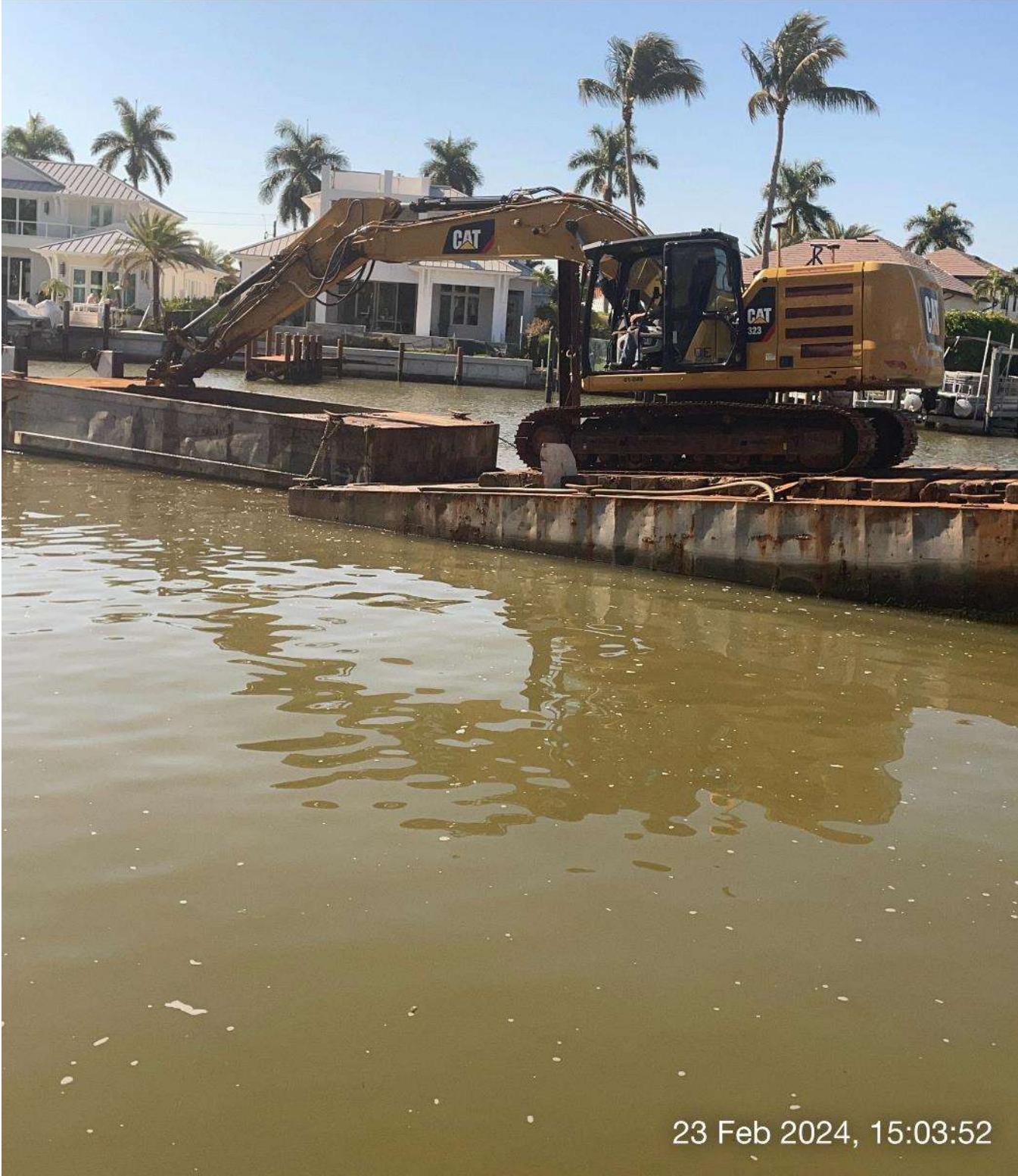
323 excavator removing sediment at station 13+25 in Canal A-A.
