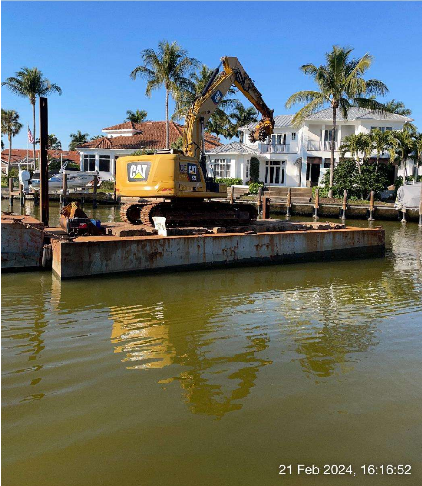
323 excavator lifting spuds to move barge out of Canal A-A.
