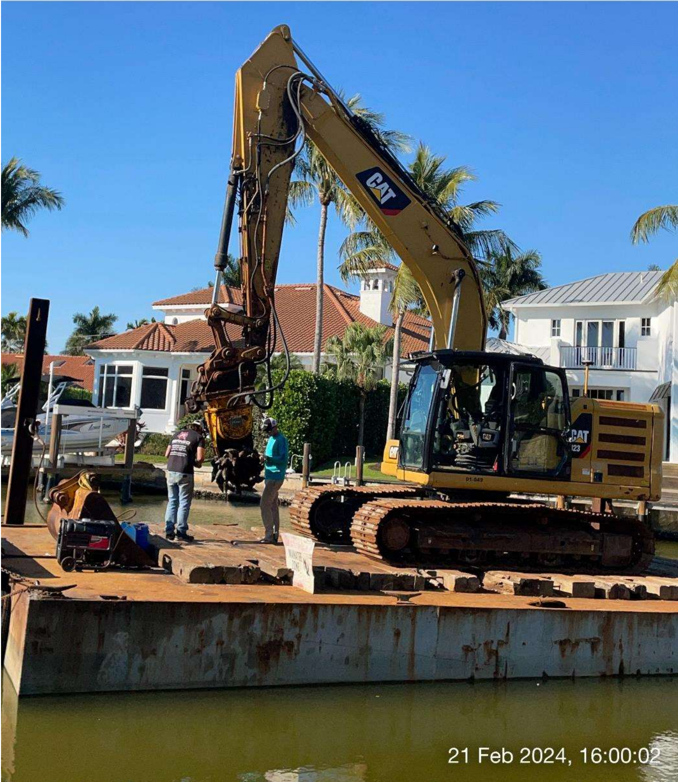
Contractor removing teeth from Epiroc grinder.
