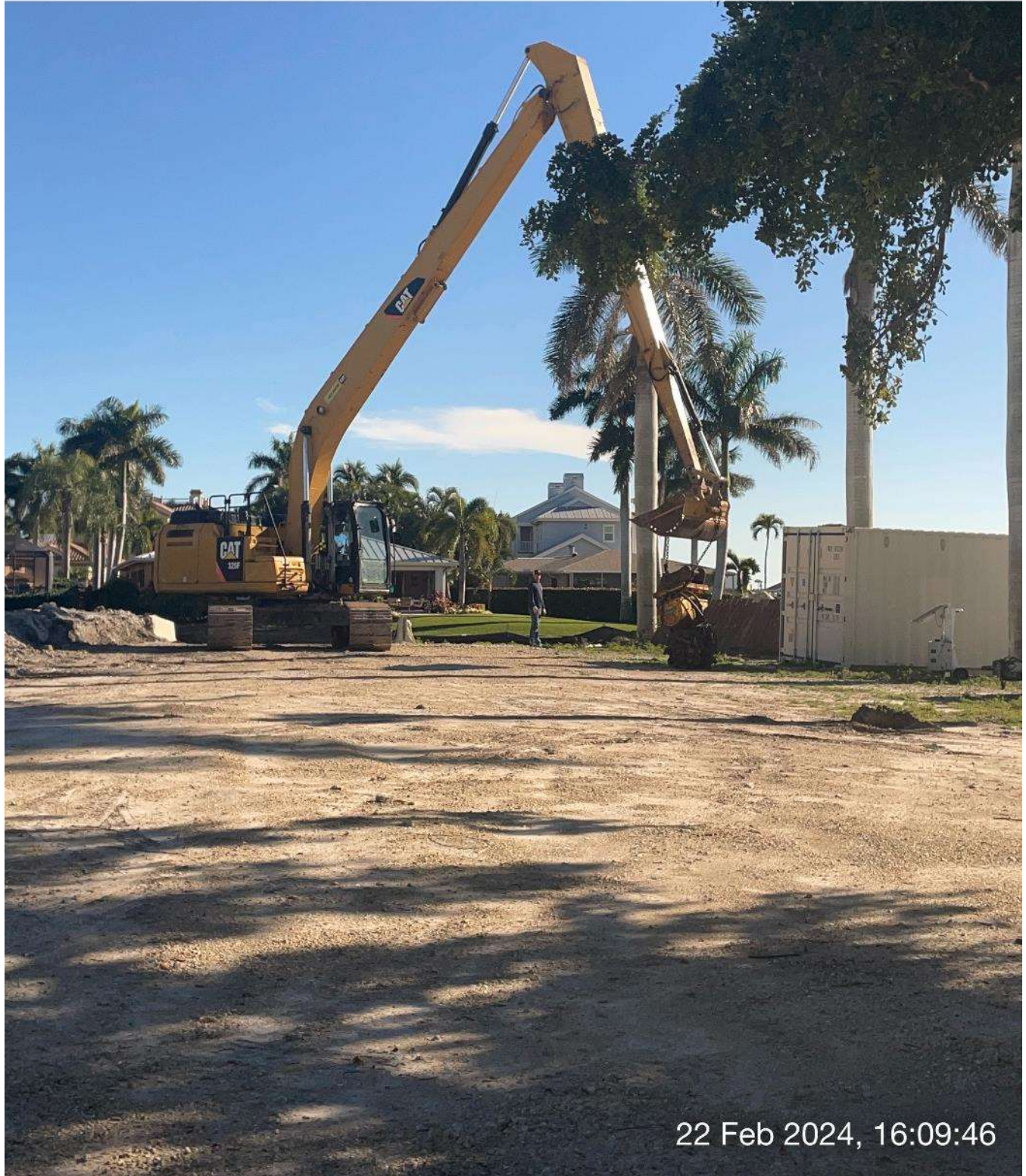
Long reach excavator lifting Epiroc grinder onto staging area.
