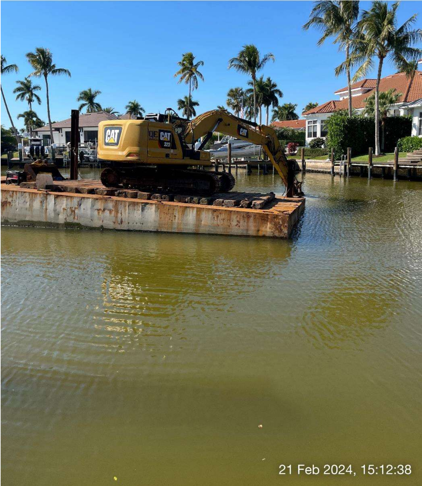
323 excavator grinding rock at station 13+75 in Canal A-A.
