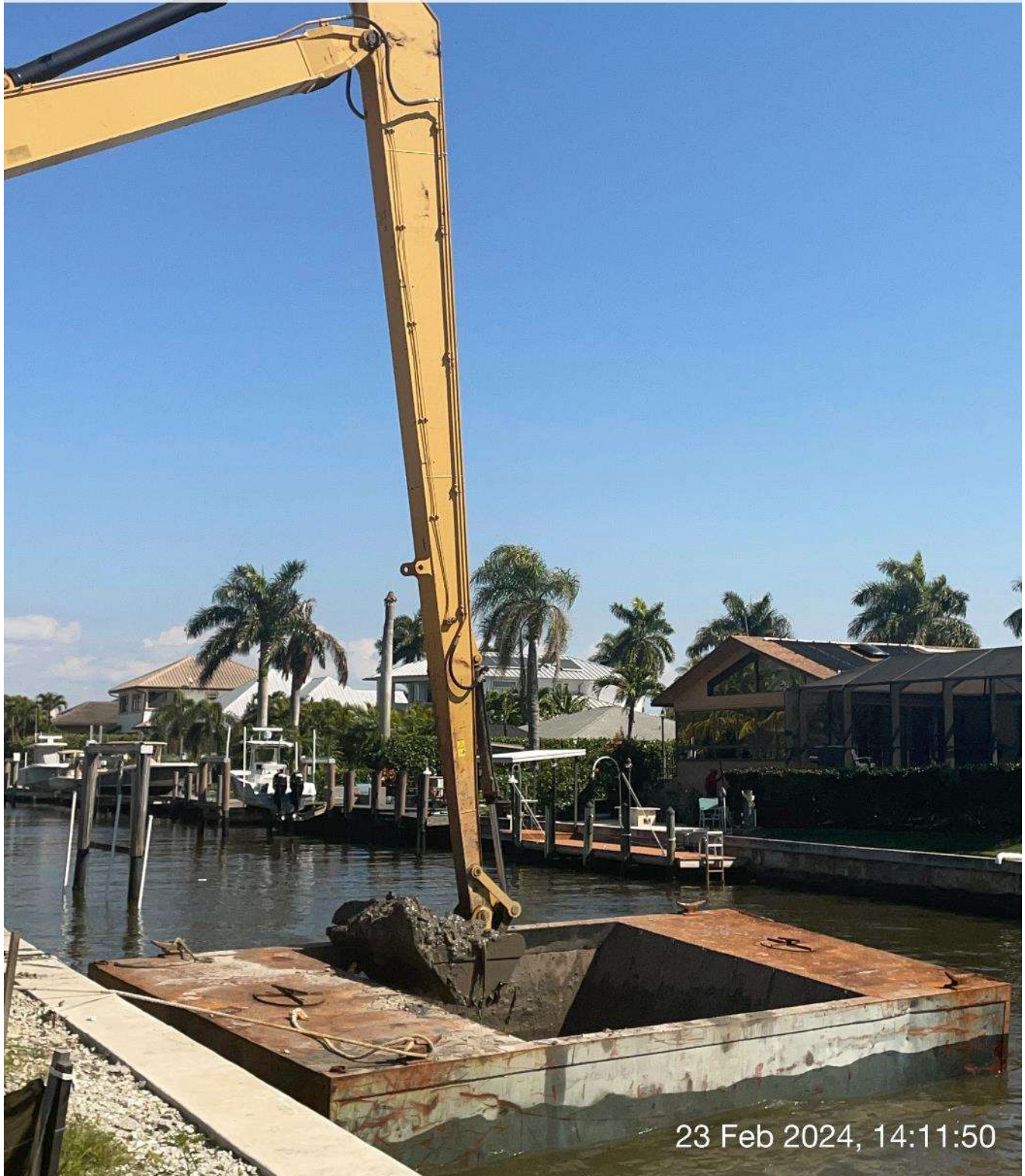
Long reach excavator removing sediment from hopper.
