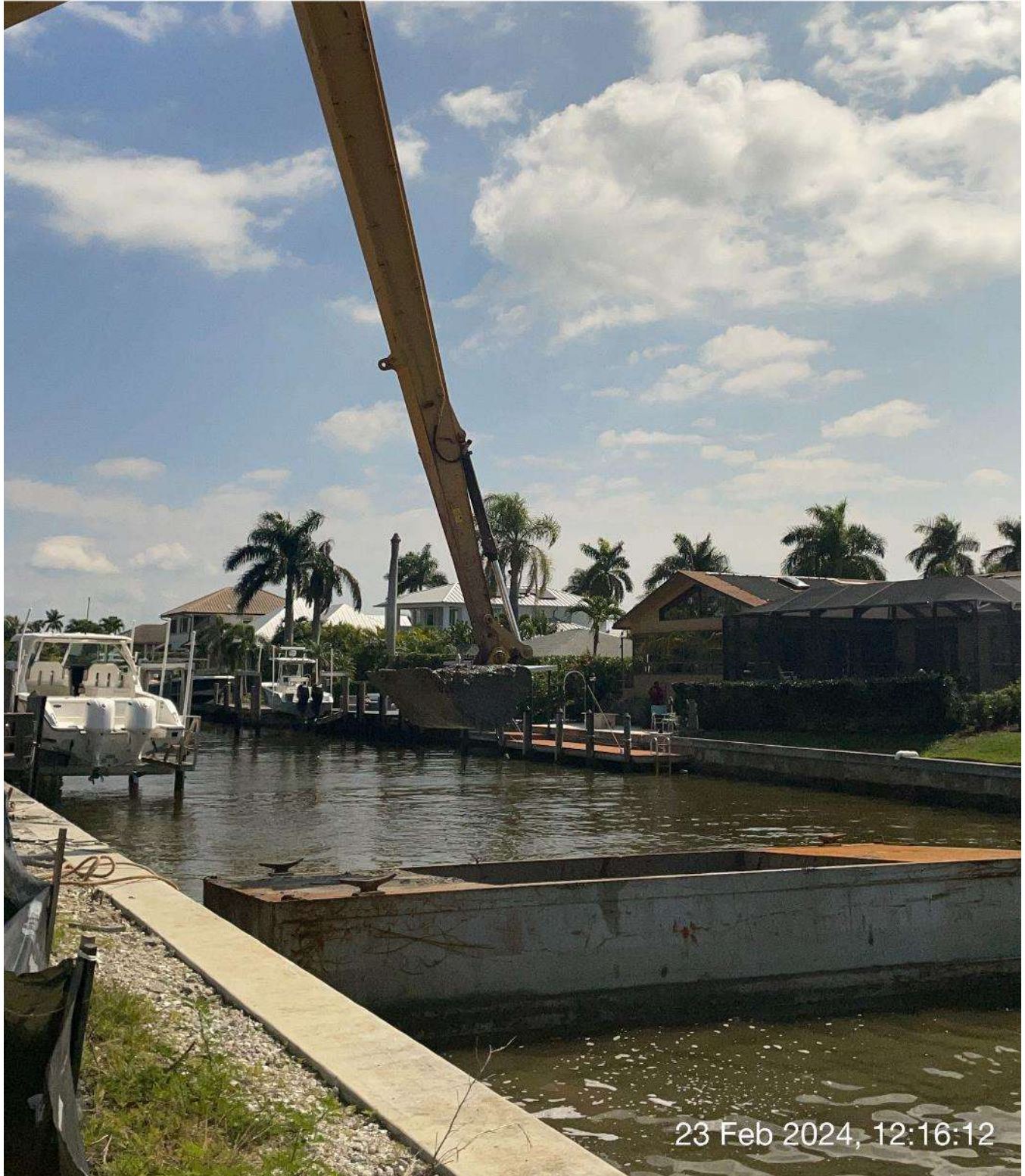
Long reach excavator removing sediment from hopper.
