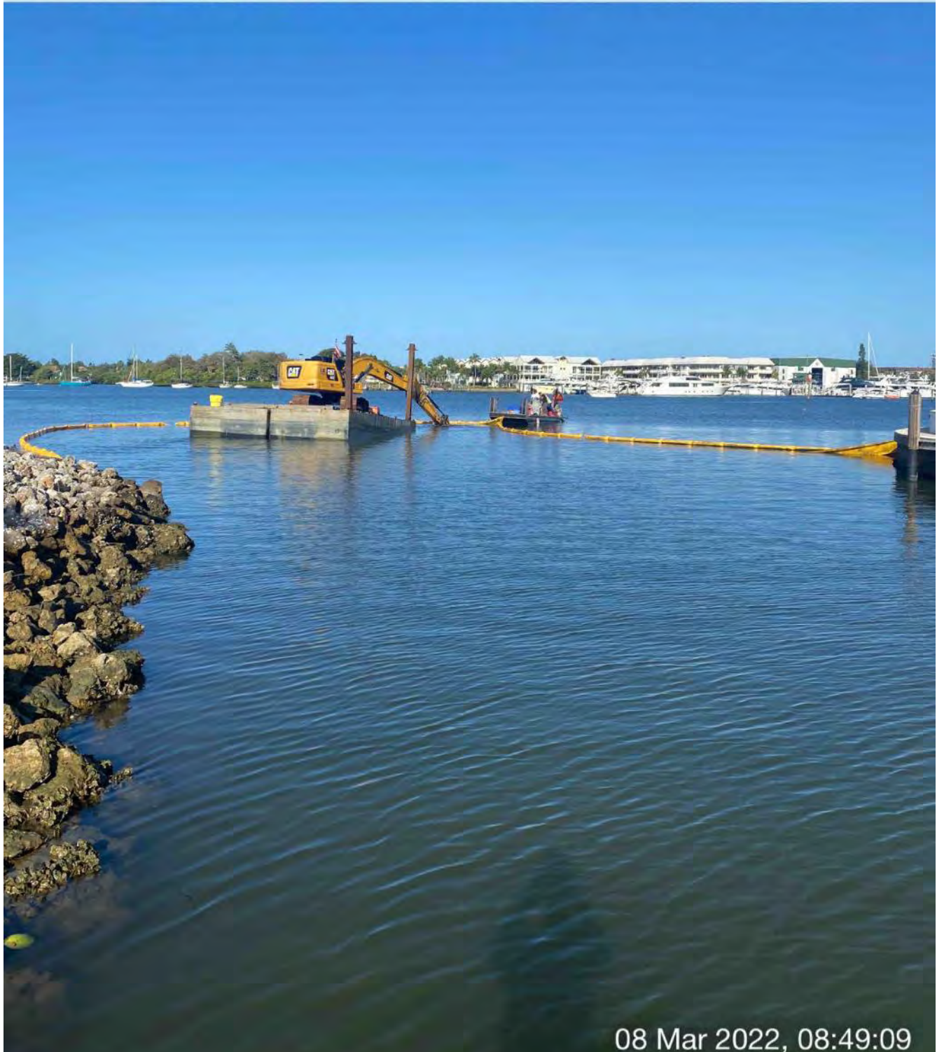
323 excavator grinding rock at station 0+00. Push boat pulling turbidity curtain out of the way.
