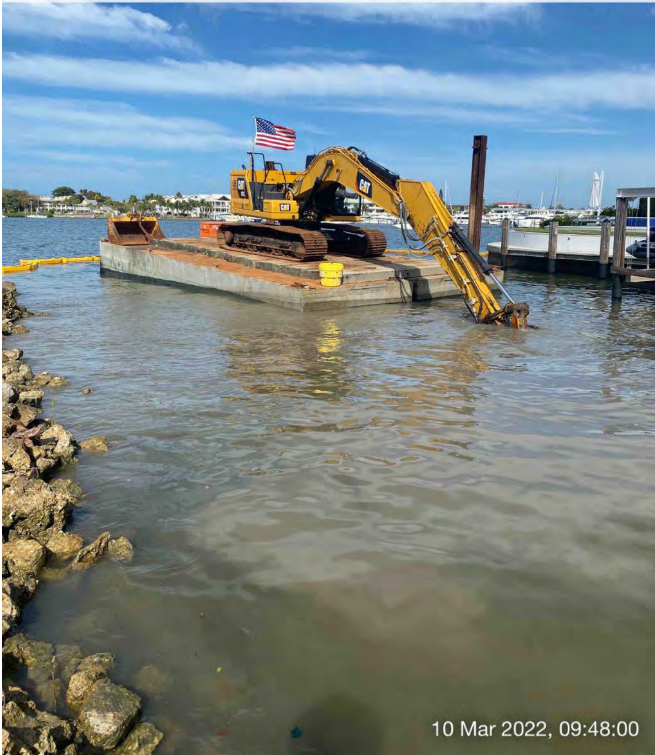
323 excavator grinding rock at station 1+50
