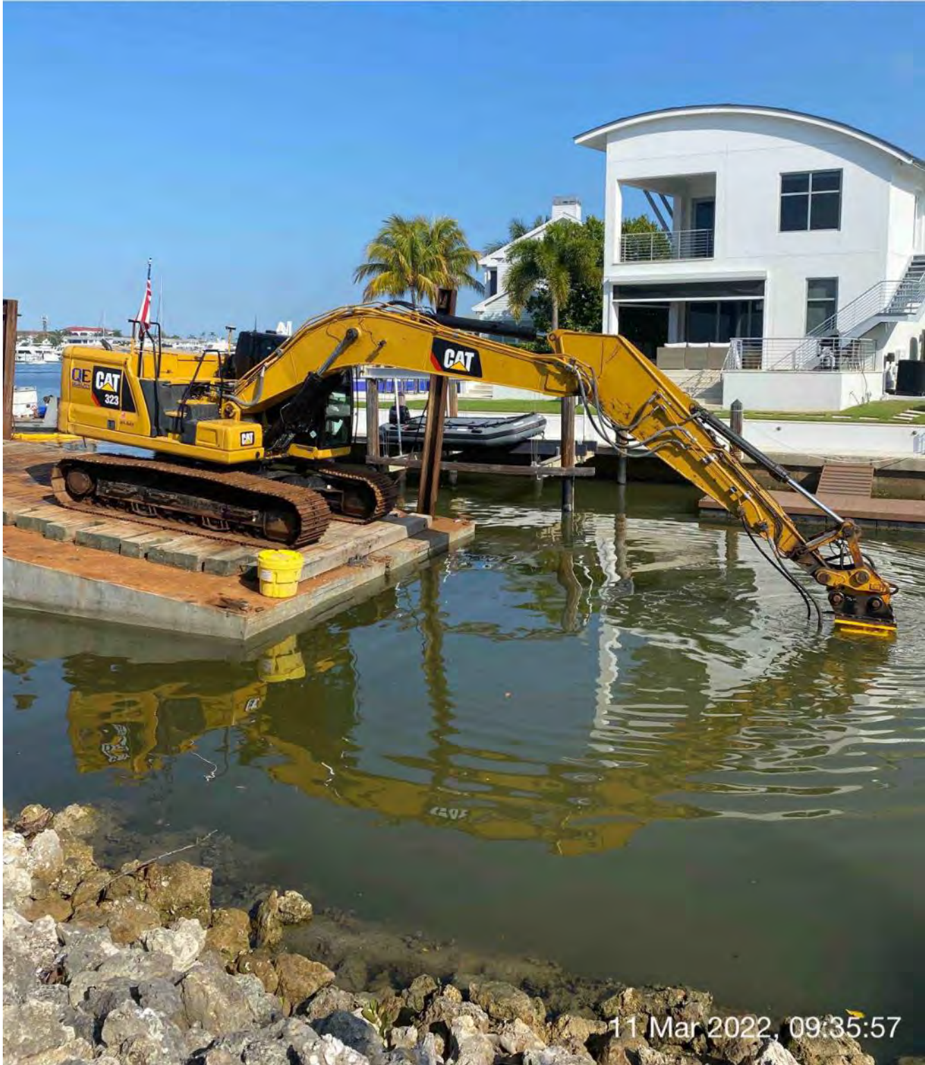
323 excavator grinding rock at station 1+75
