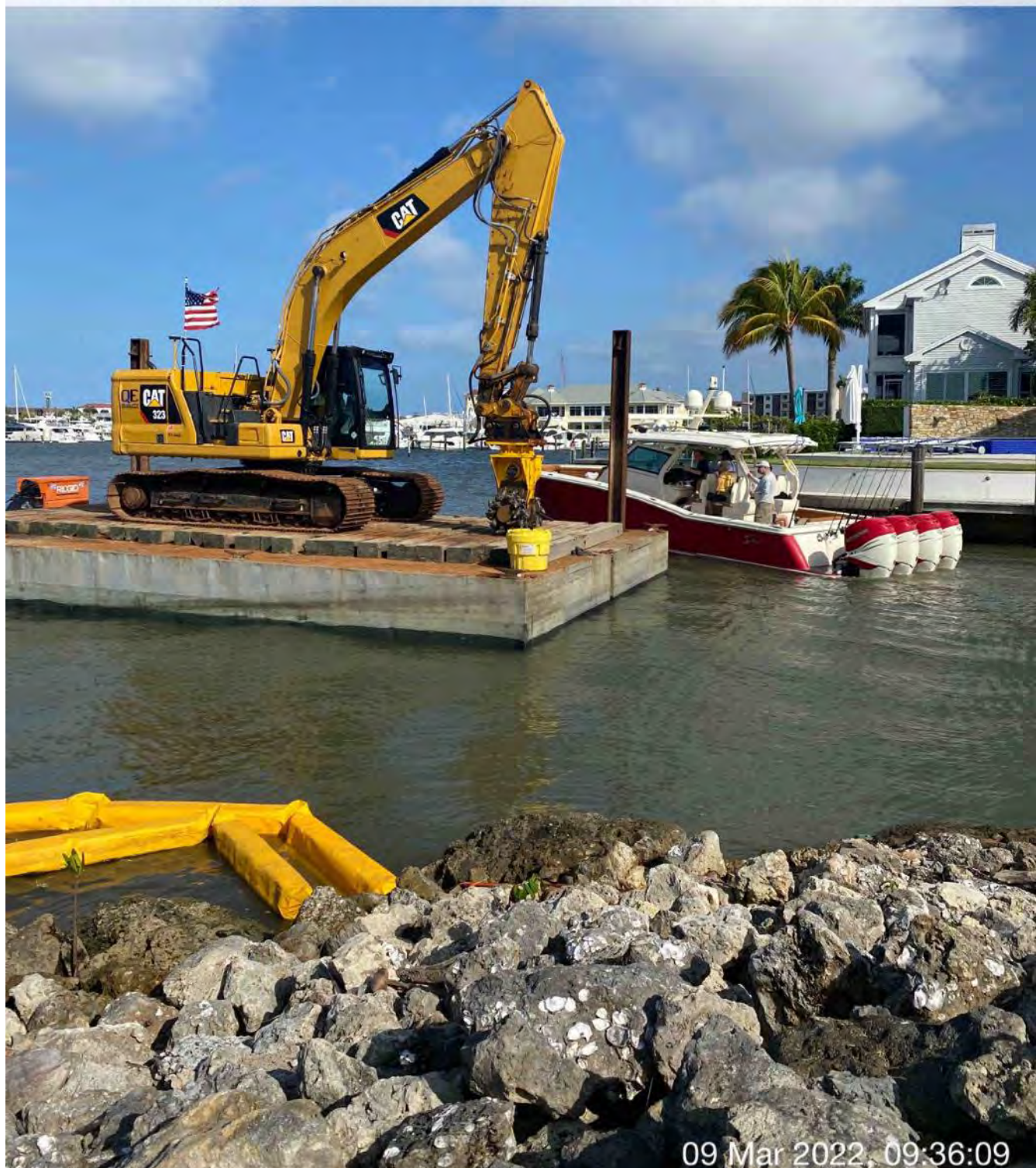
323 excavator on barge with Epiroc grinder at station 1+00 as Canal BB-BB resident exits canal
