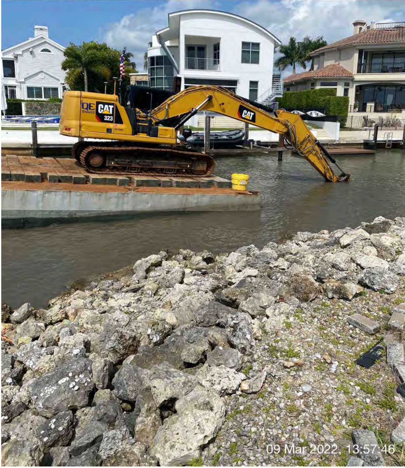
323 excavator grinding rock at station 1+50
