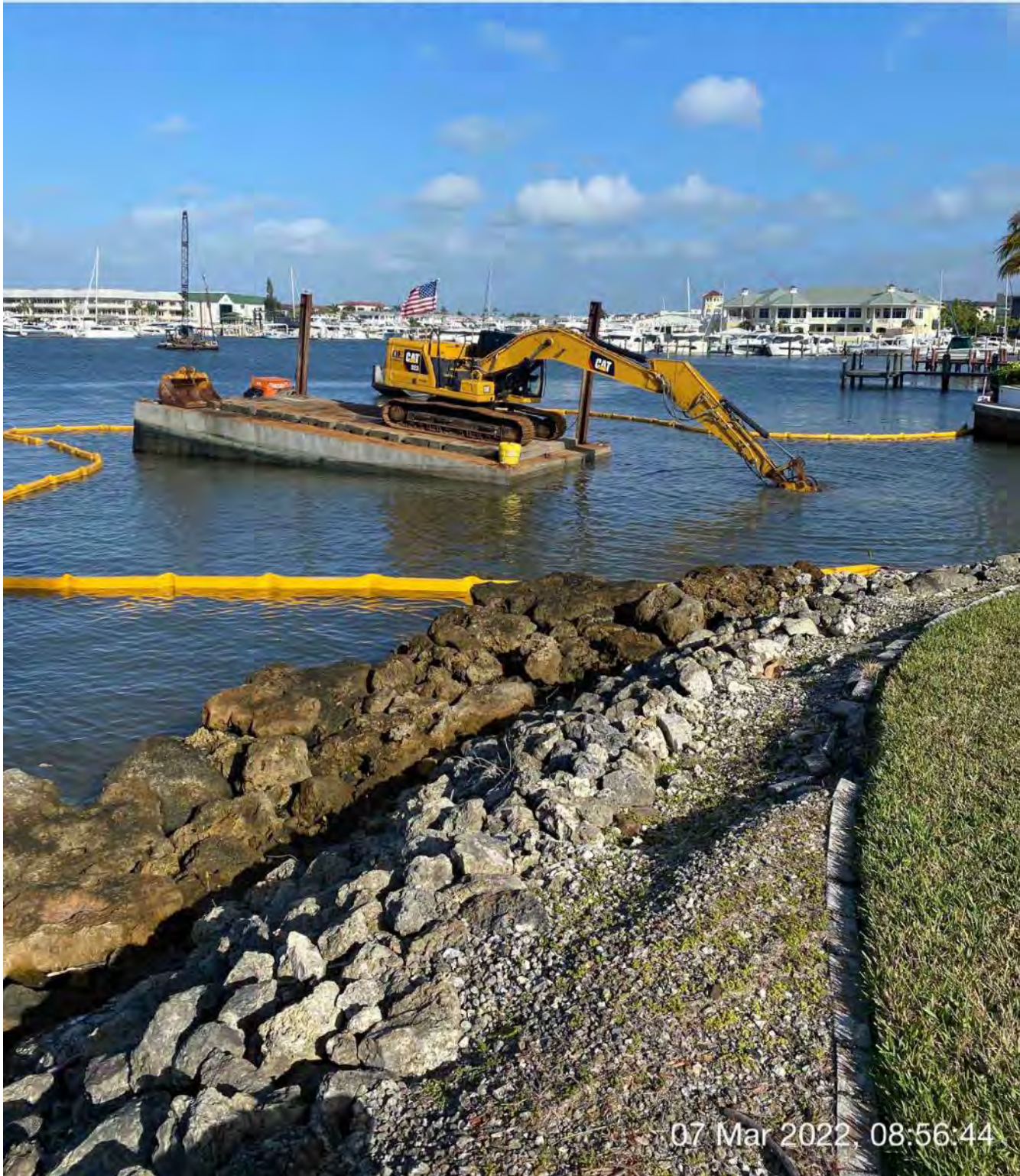
323 excavator grinding rock at station 1+00
