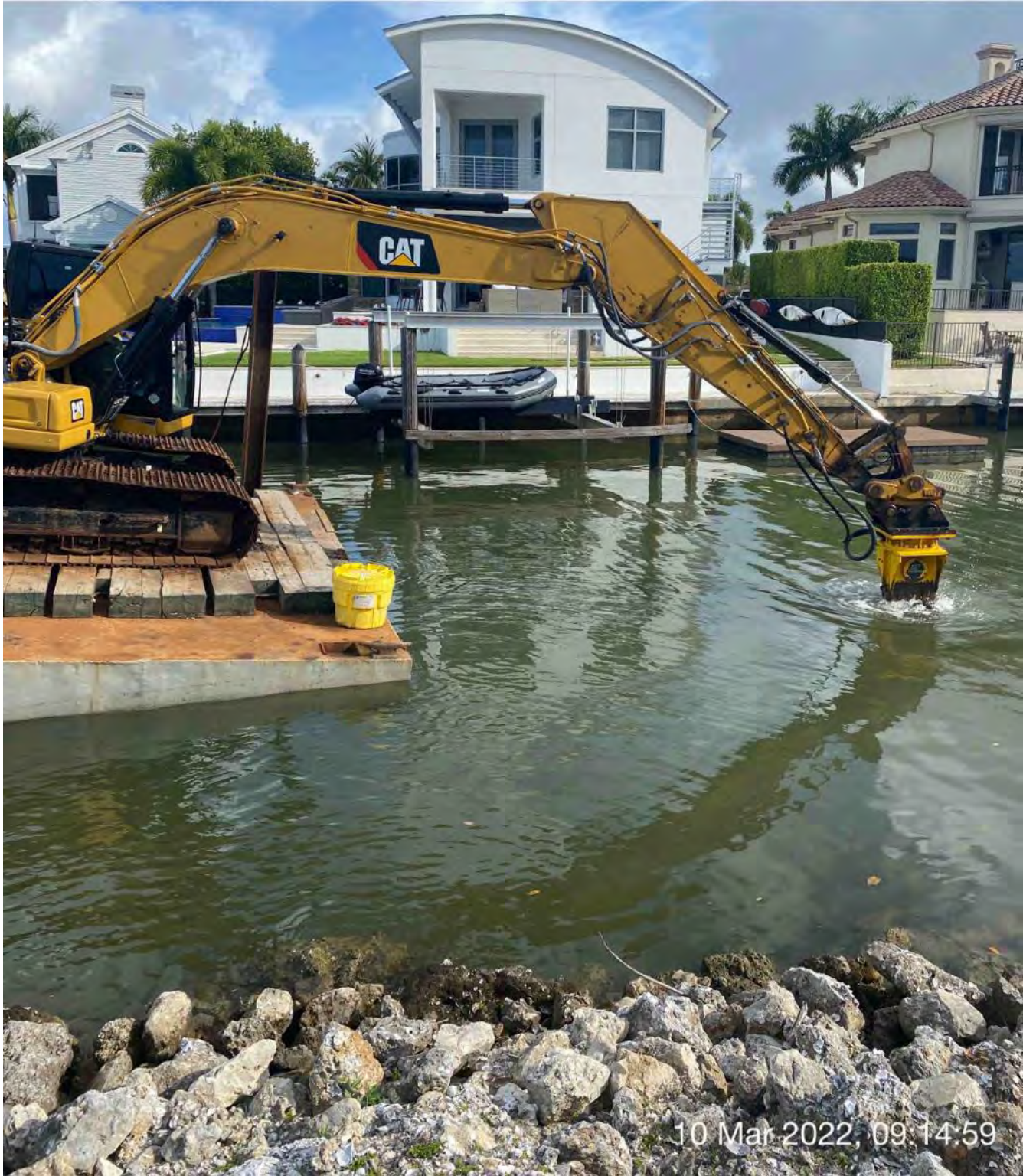
323 excavator grinding rock at station 1+50
