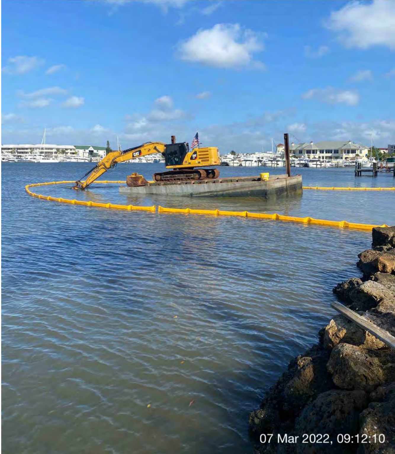
323 excavator grinding rock at station 0+00
