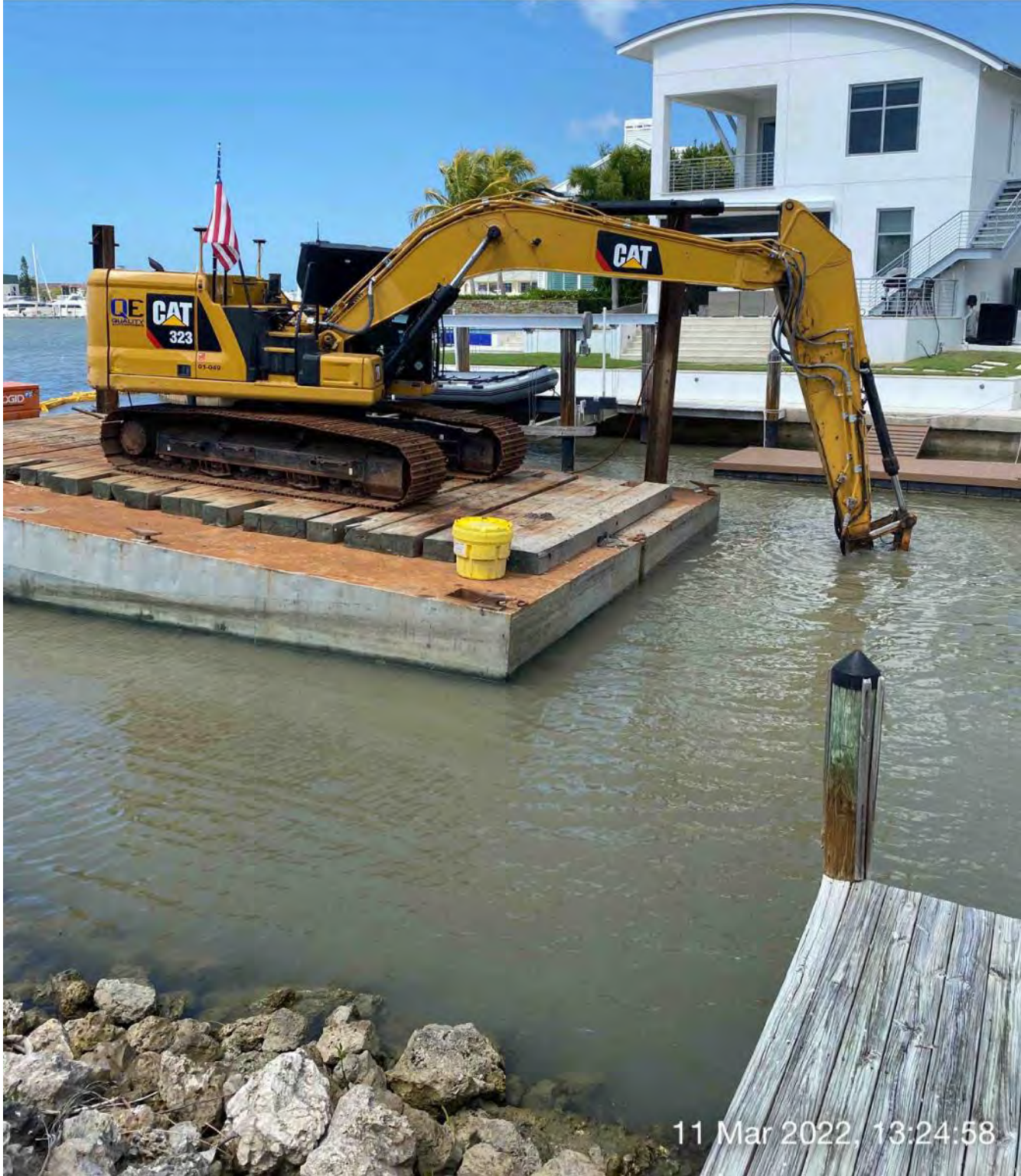
323 excavator grinding rock at station 1+75
