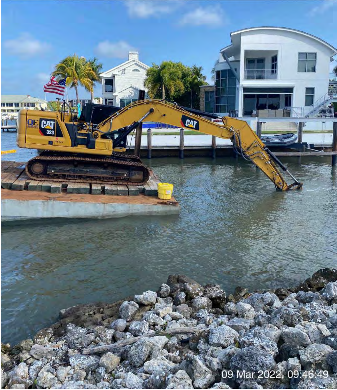
323 excavator grinding rock at station 1+50
