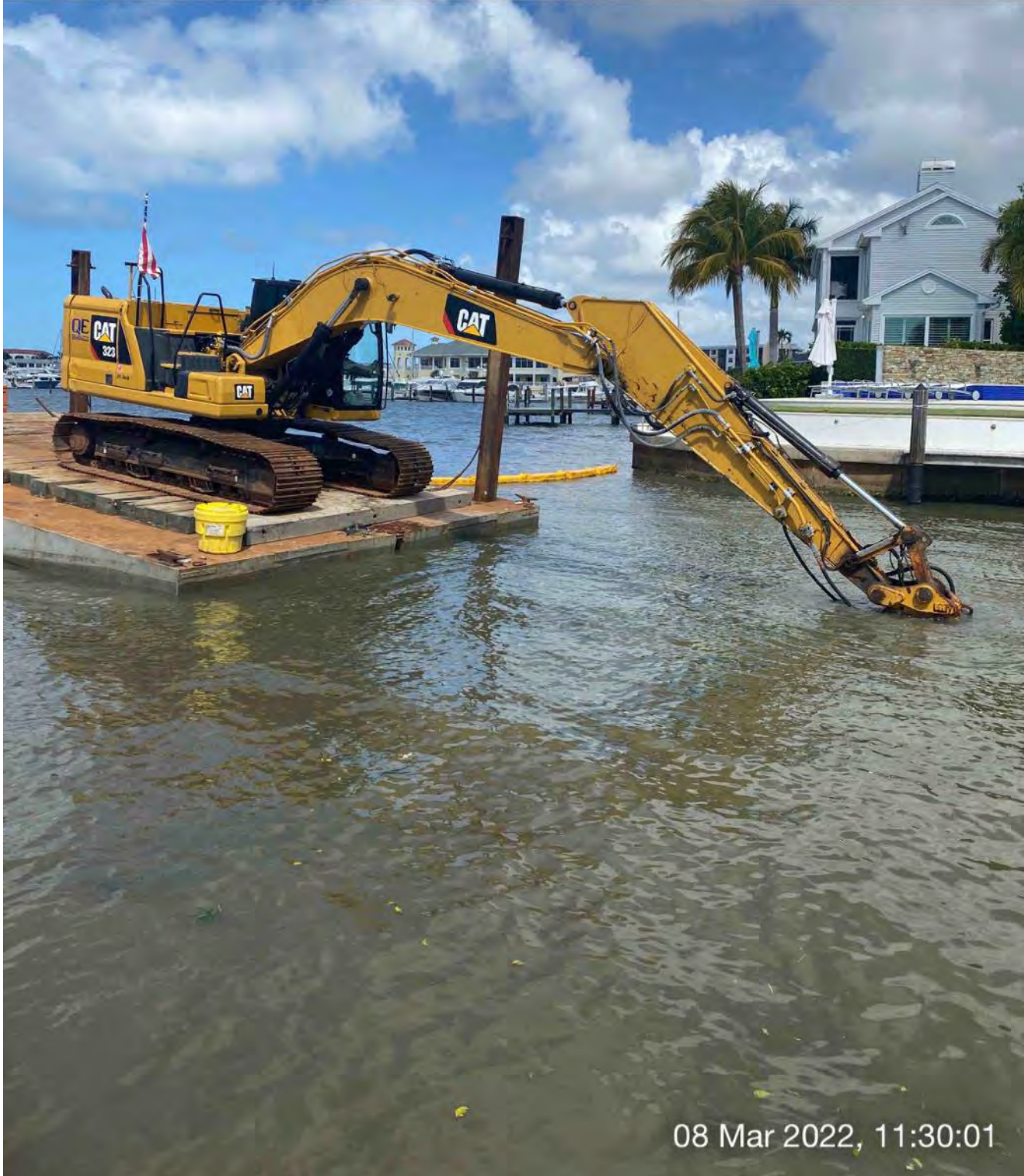
323 excavator grinding rock at station 1+25
