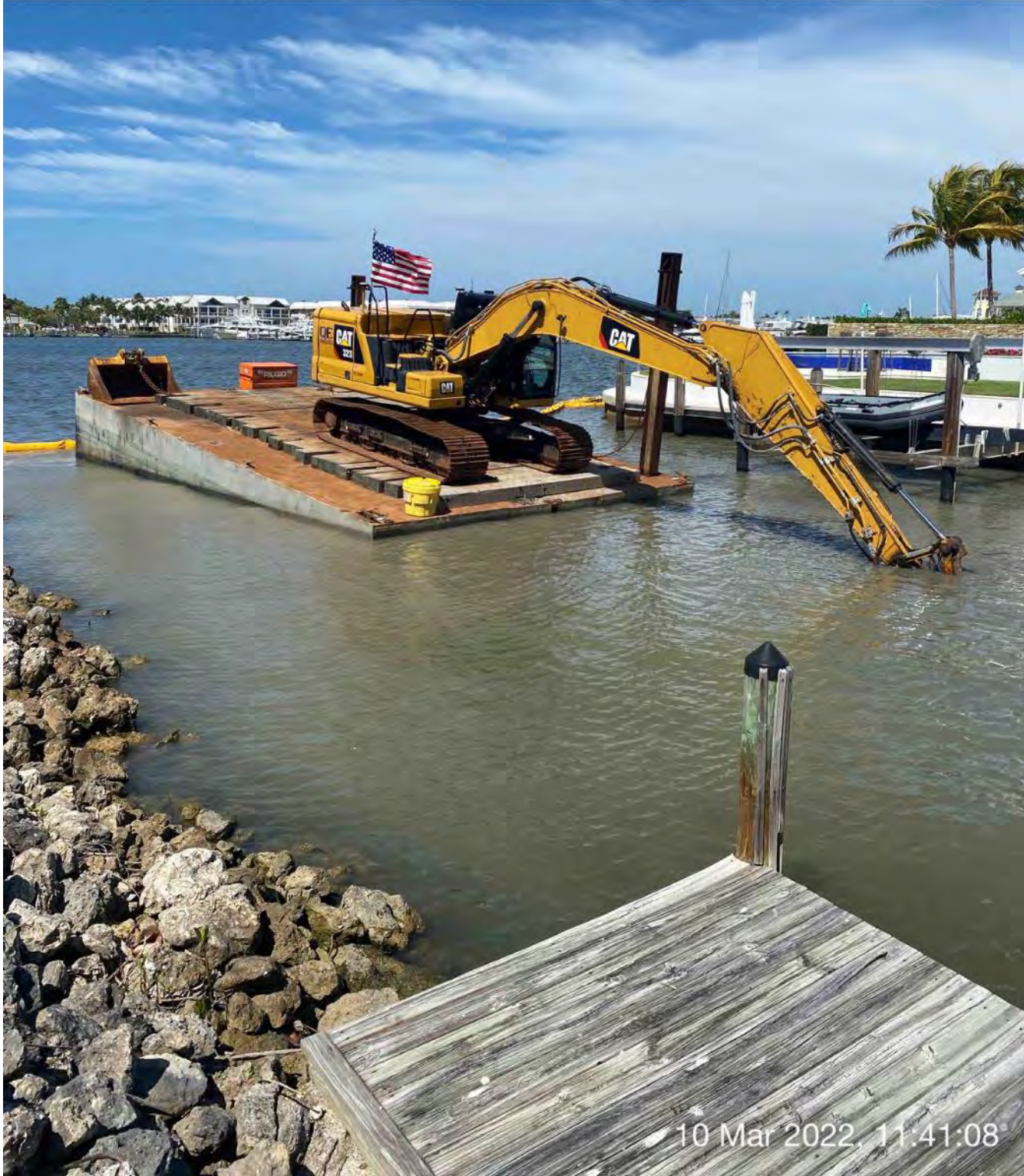
323 excavator grinding rock at station 1+75
