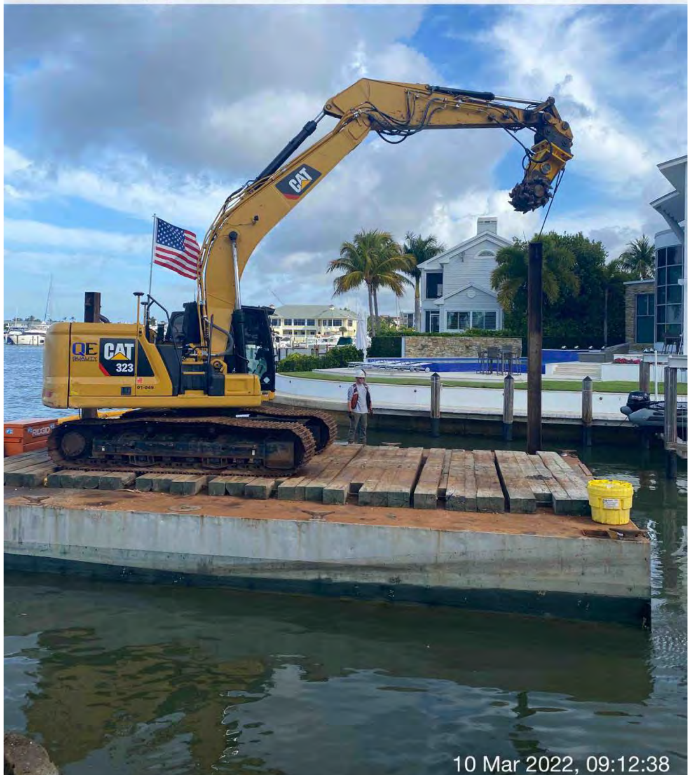
323 excavator lifting spud to allow push boat to mobilize barge at station 1+25
