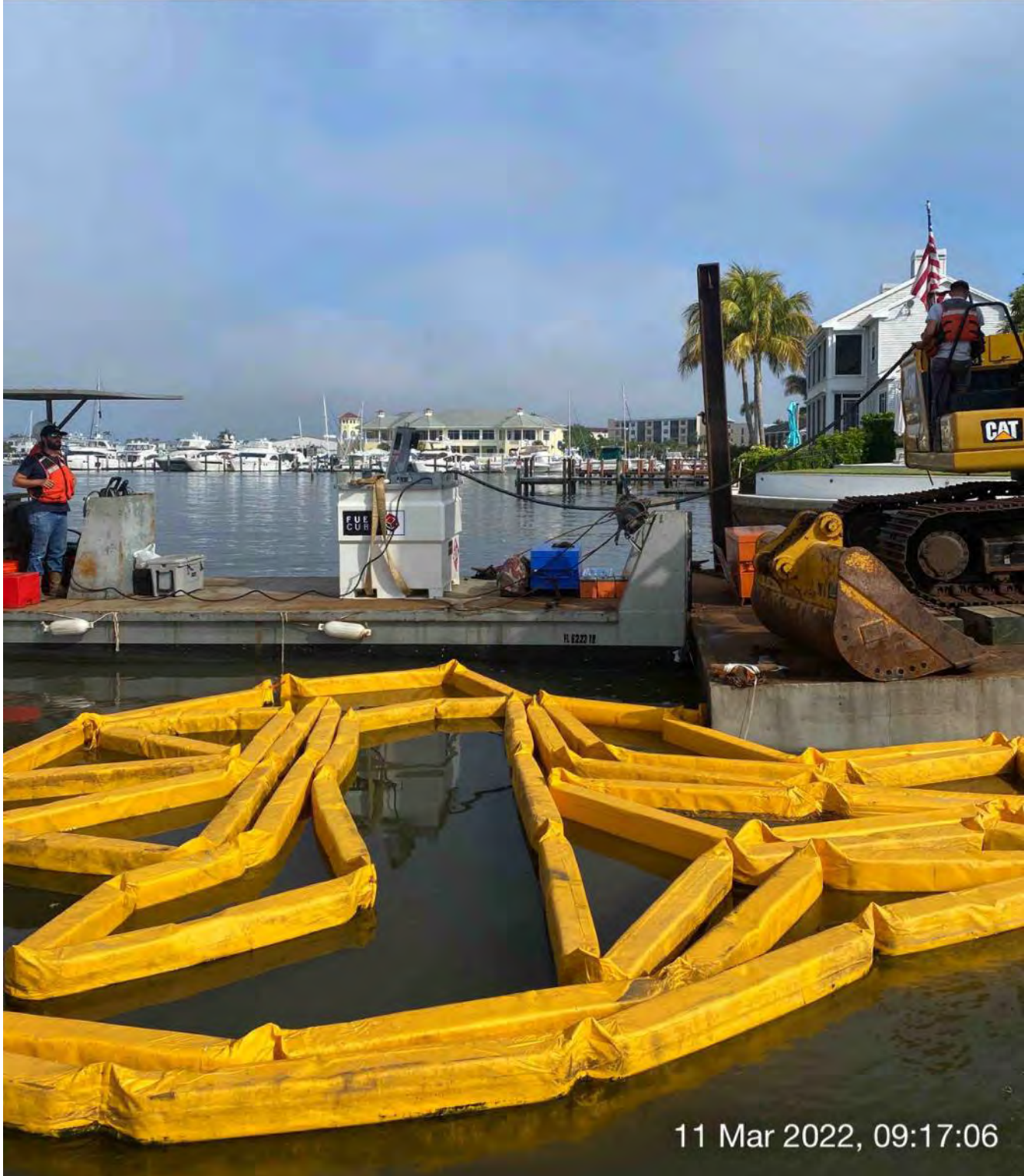
Contractor refueling 323 excavator with small fuel cube on push boat at station 1+00
