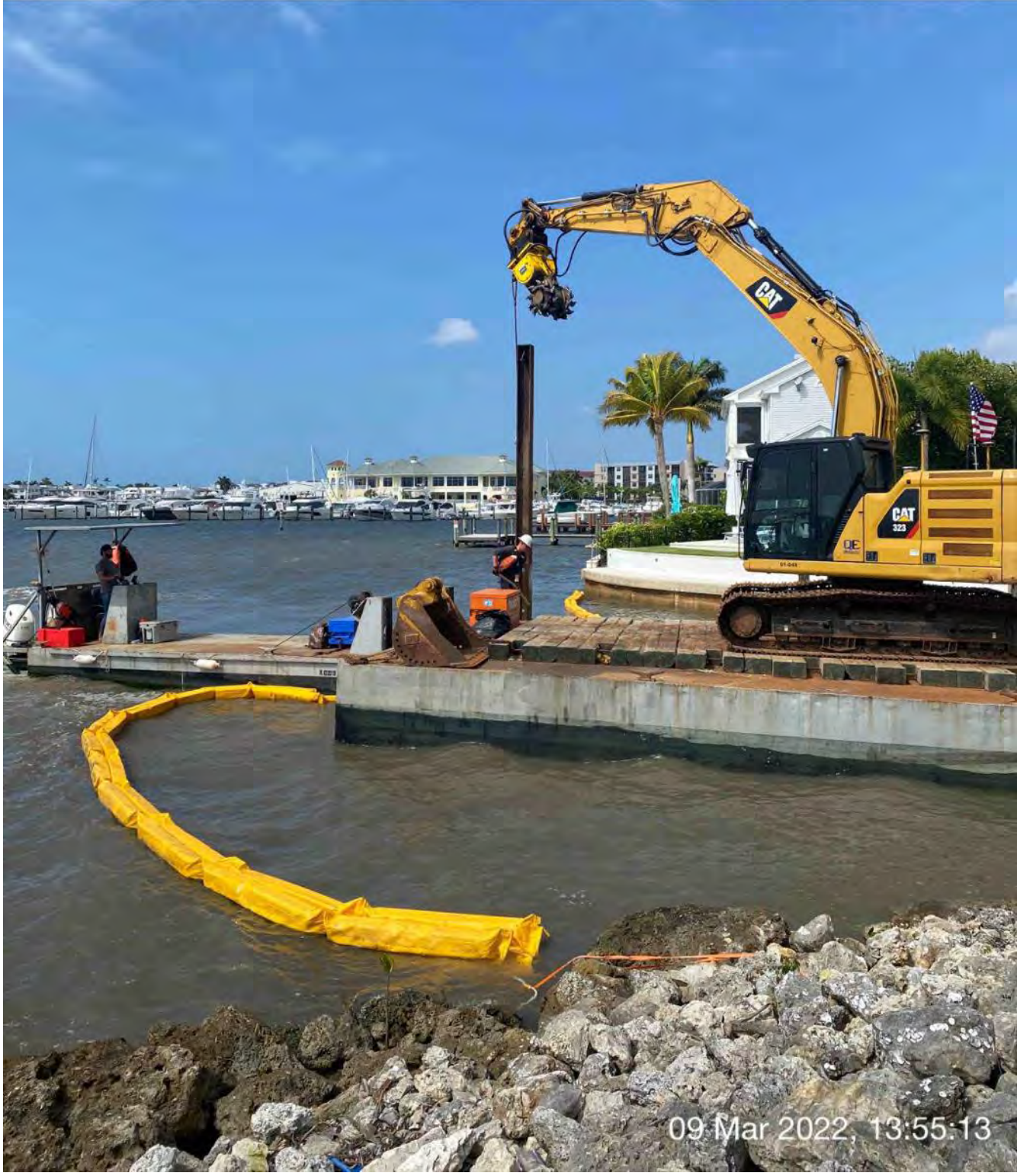
323 excavator lifting spud to allow push boat to mobilize barge at station 1+25
