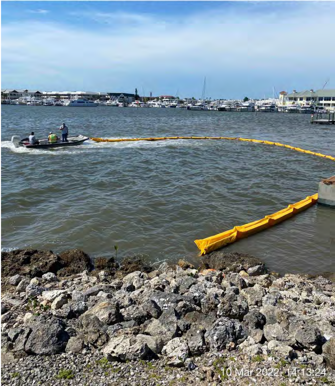
Support boat being used to open the turbidity curtain
