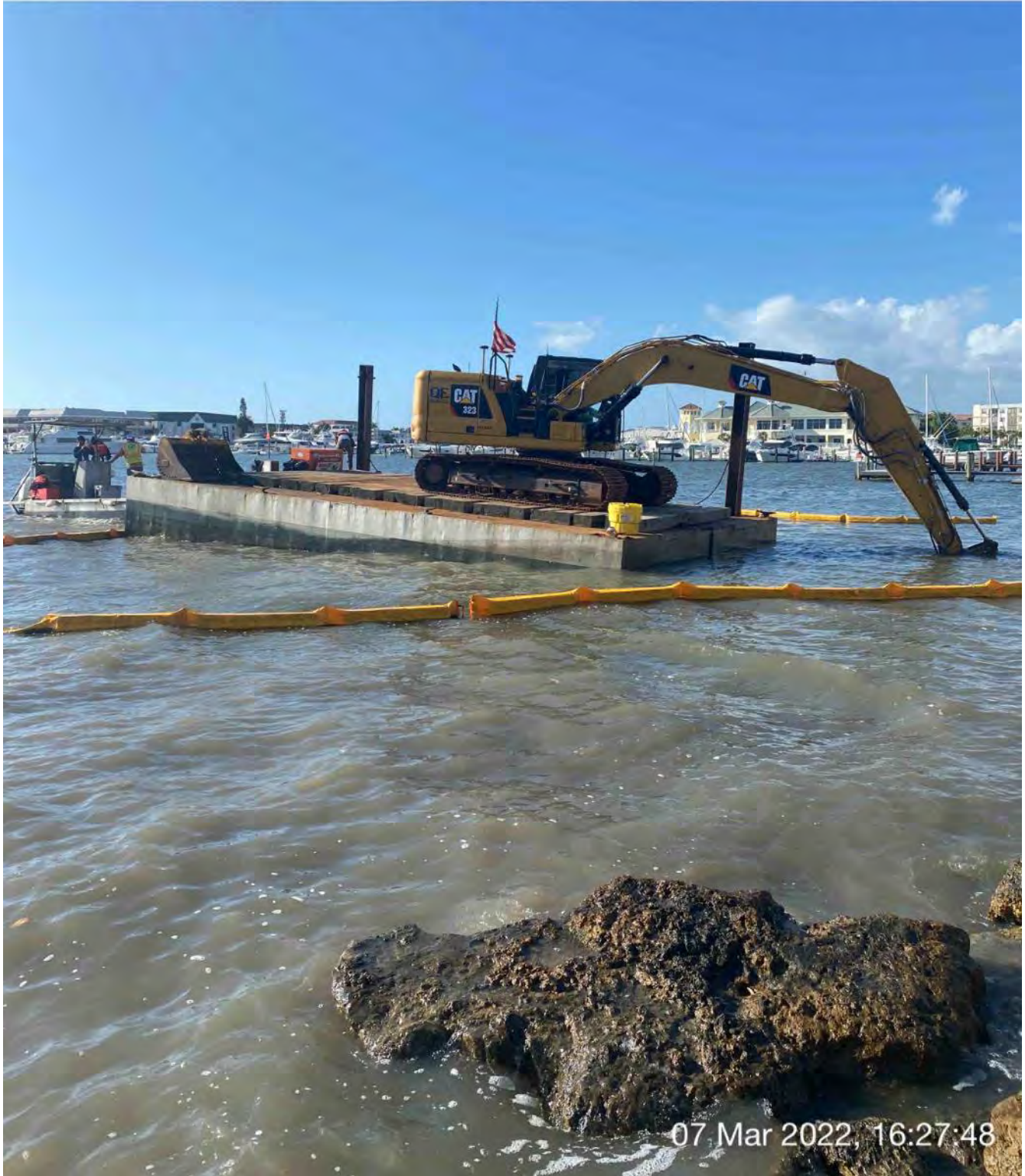
323 excavator grinding rock at station 0+50
