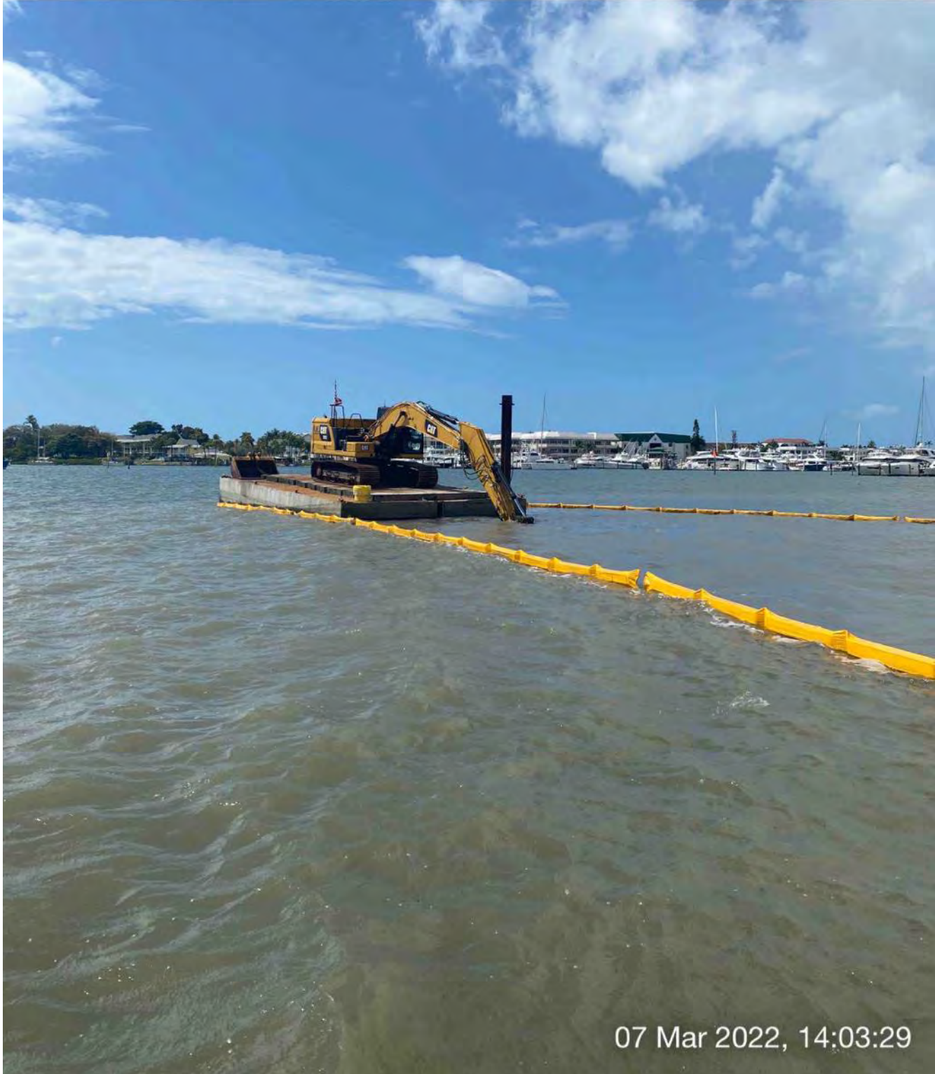
323 excavator grinding rock at station 0+00
