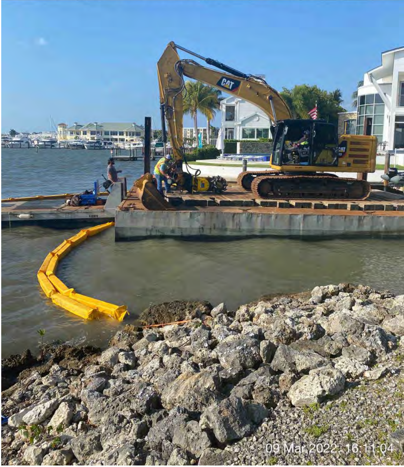
Contractor hammering pin back into place on 323 excavator
