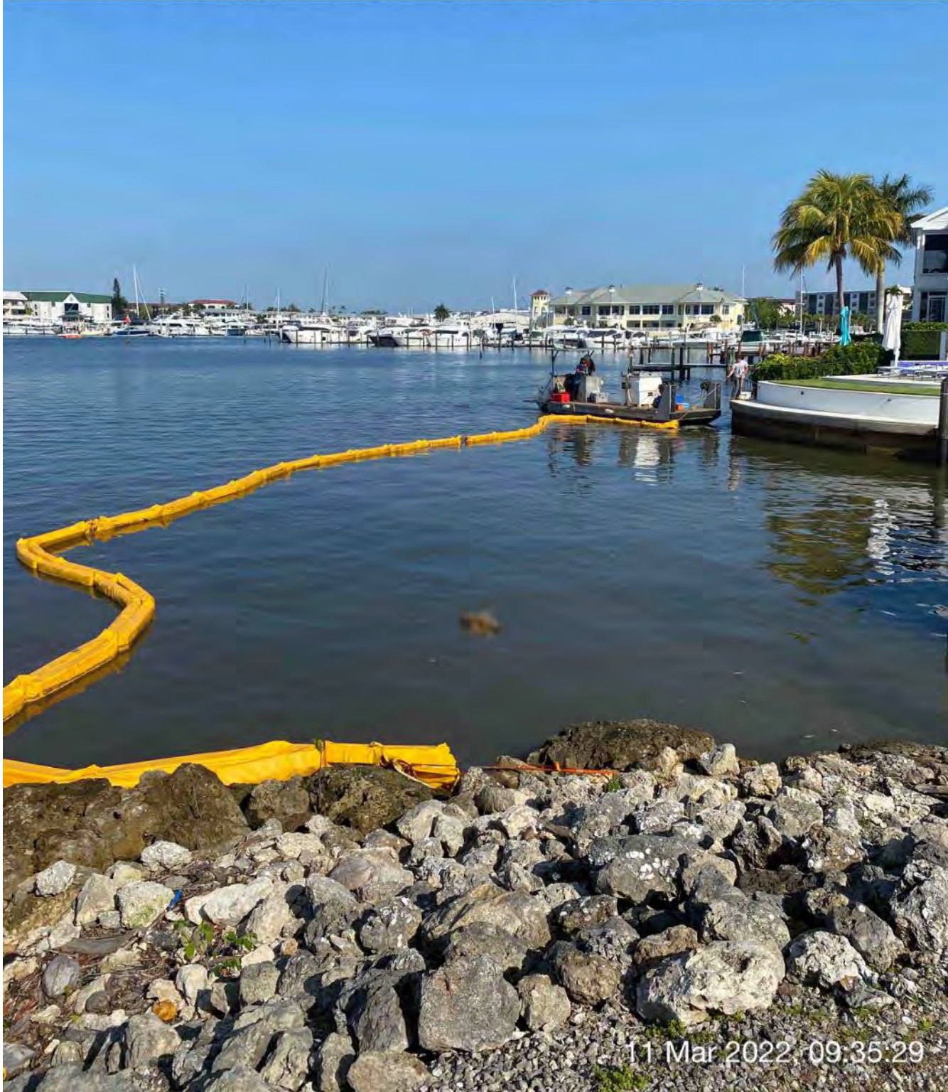
Installing turbidity curtain across the mouth of Canal BB-BB
