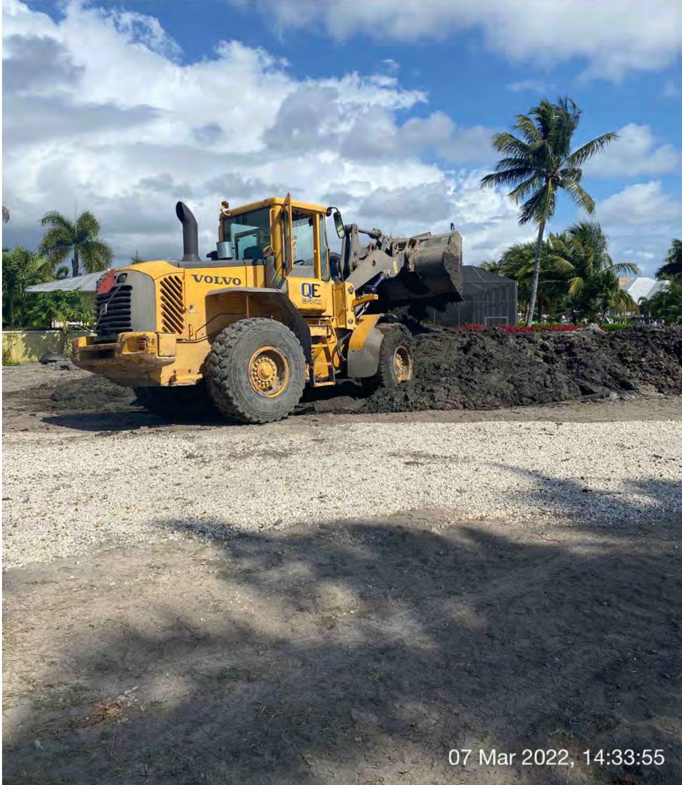
Front end loader redistributing removed material at the dewatering site at 1300 Curlew Avenue
