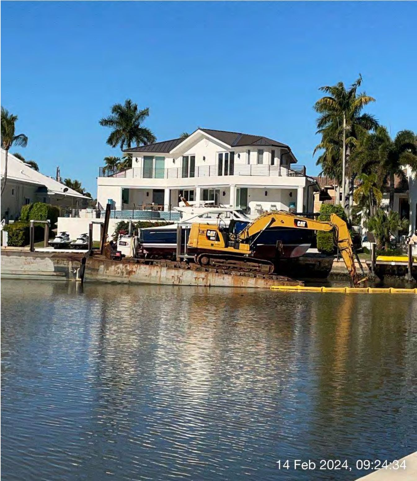
323 excavator grinding rock at station 4+00 in Canal A-A.
