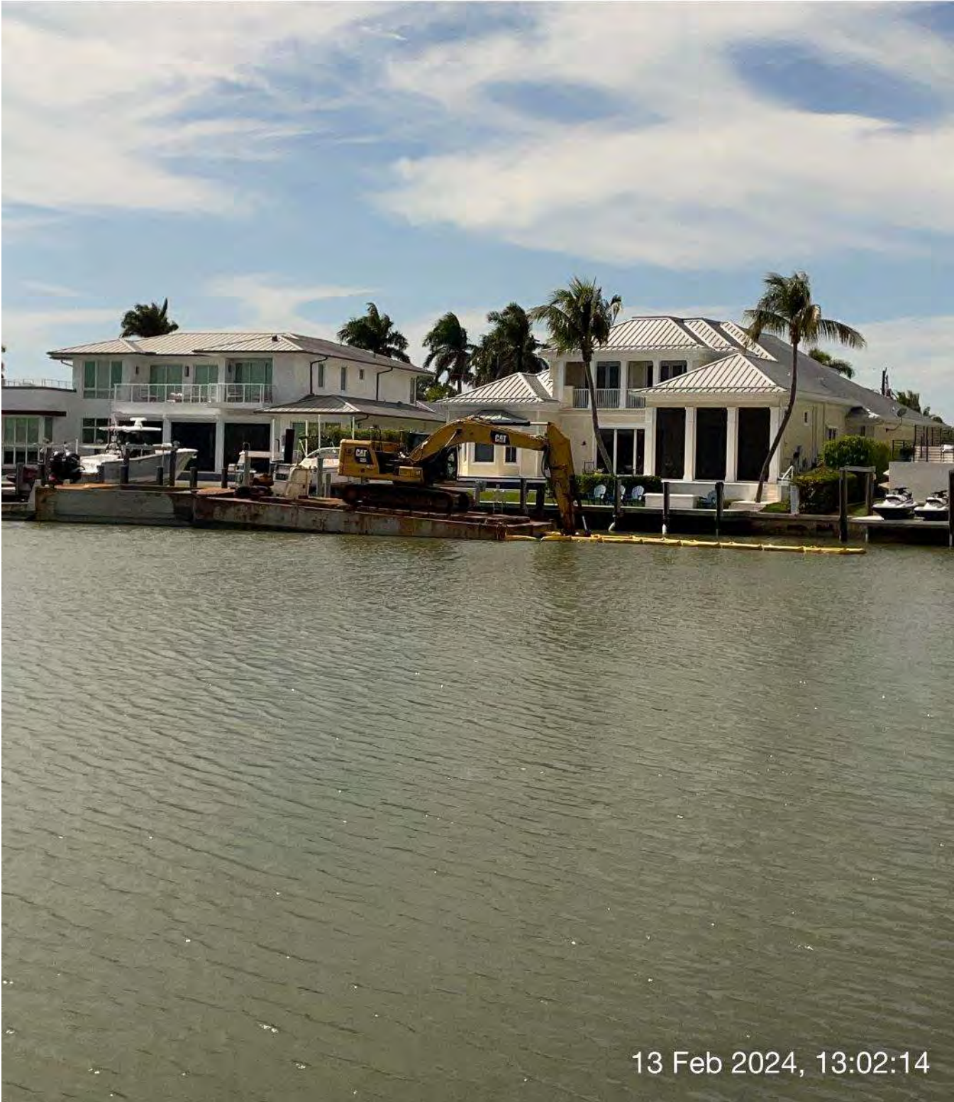
323 excavator grinding rock at station 2+75 in Canal A-A.
