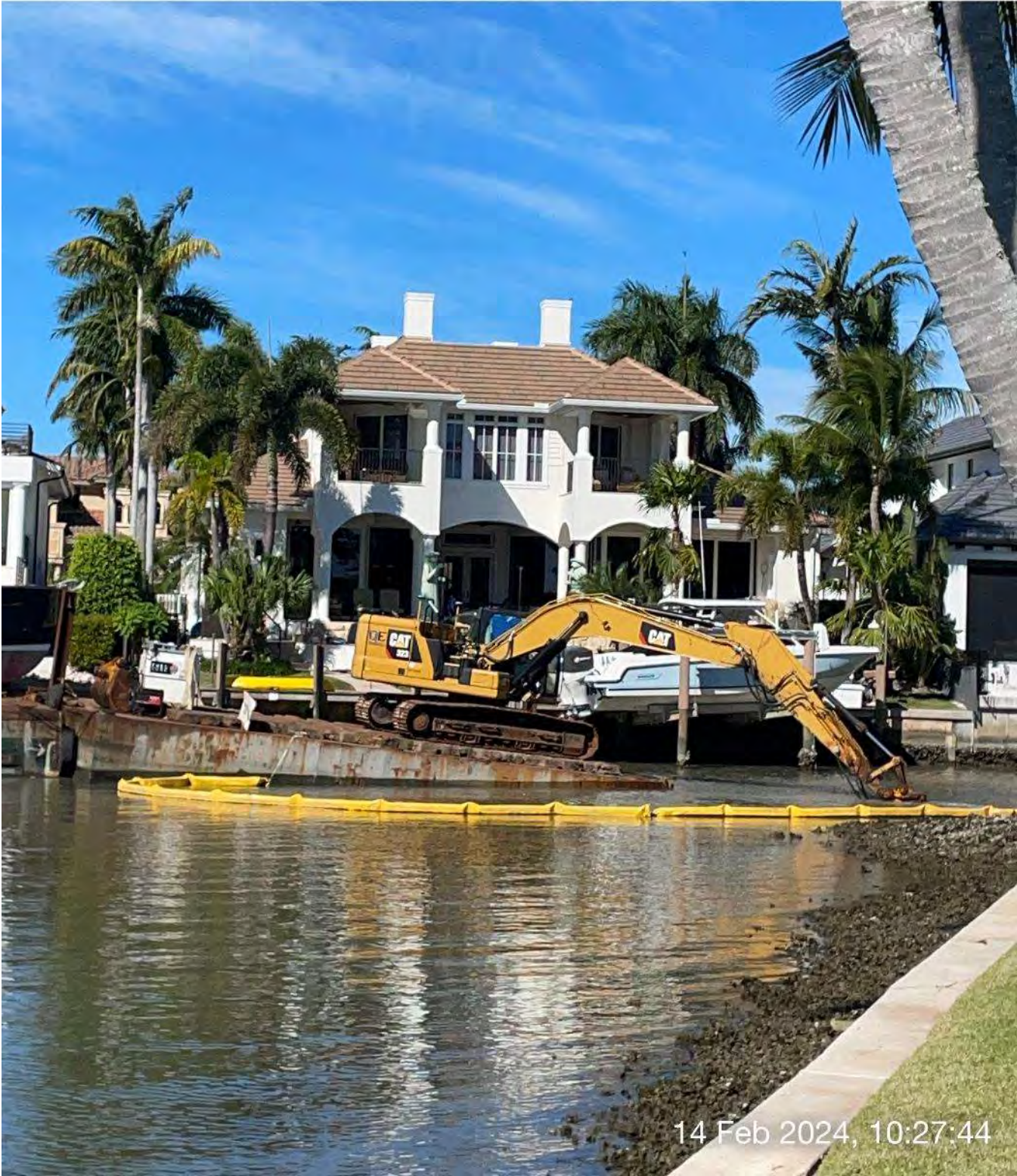
323 excavator grinding rock at station 4+50 in Canal A-A.
