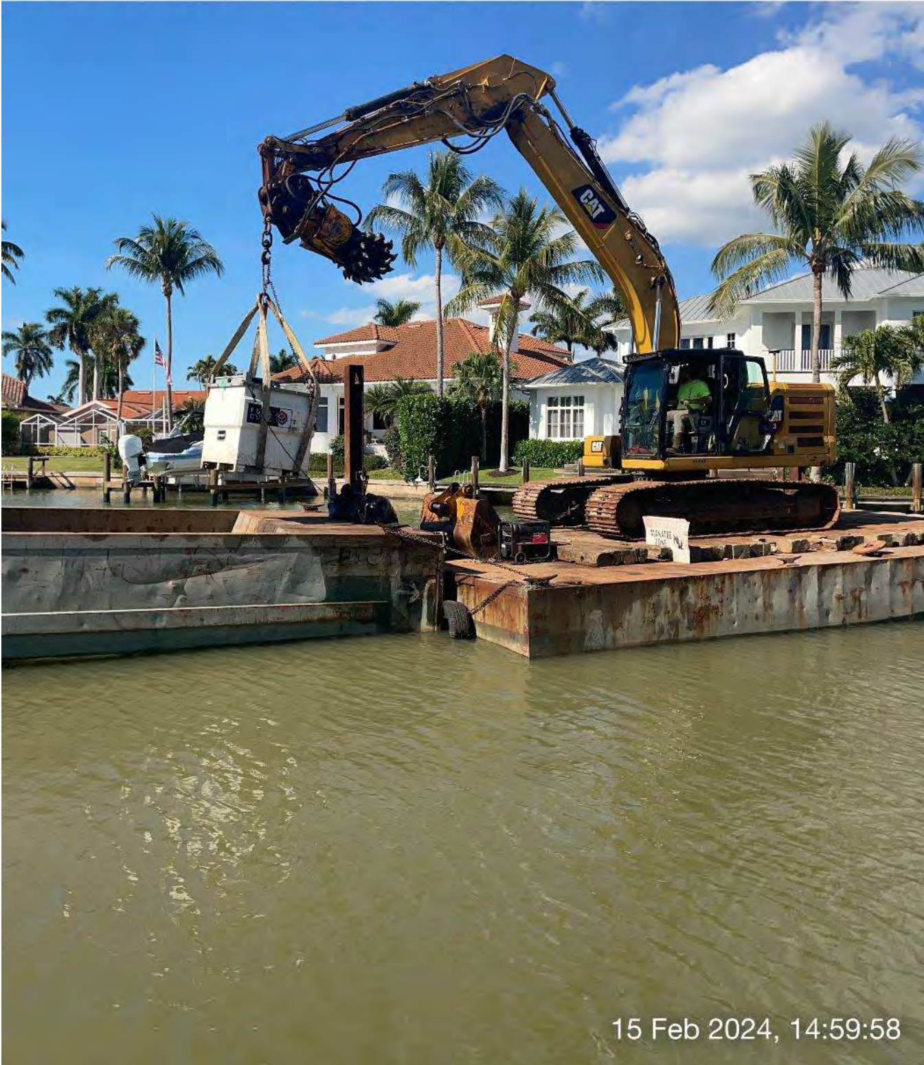
323 excavator loading fuel cube into hopper.
