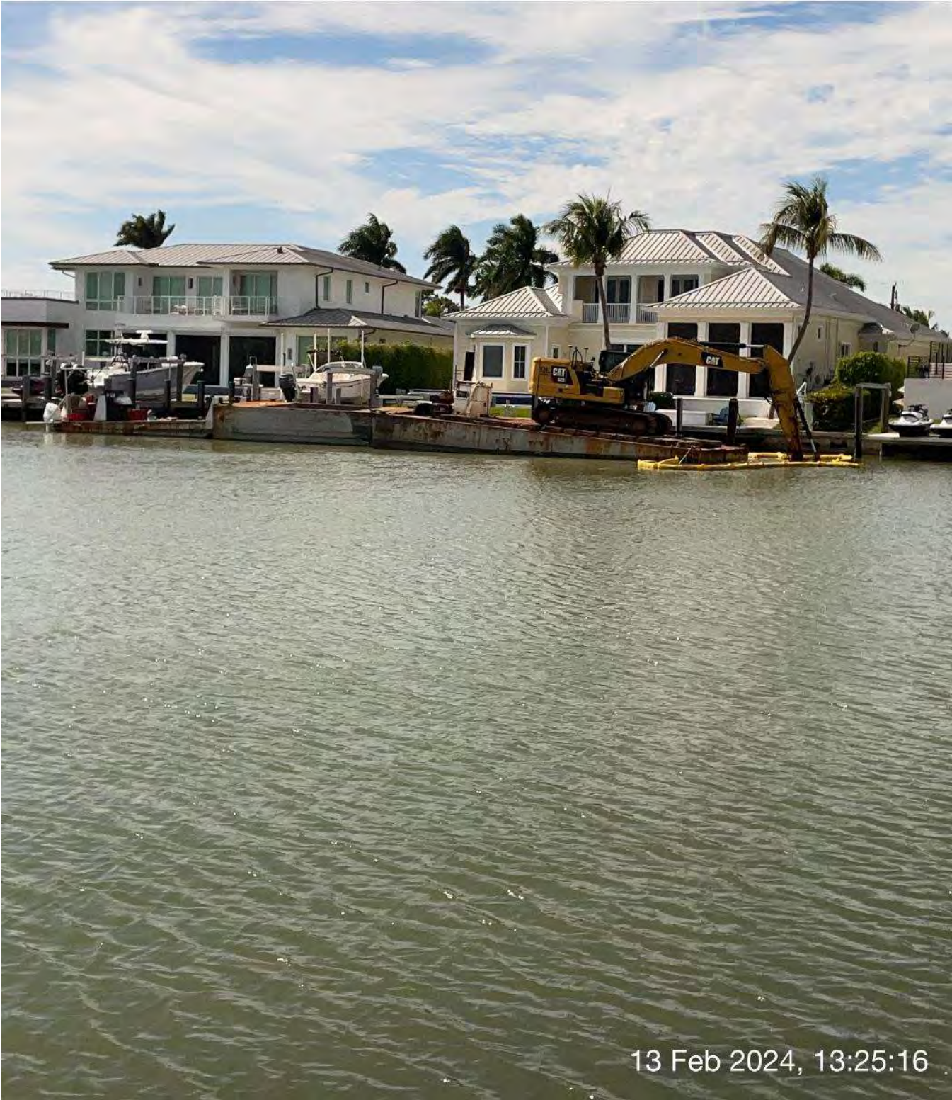
323 excavator grinding rock at station 3+00 in Canal A-A.
