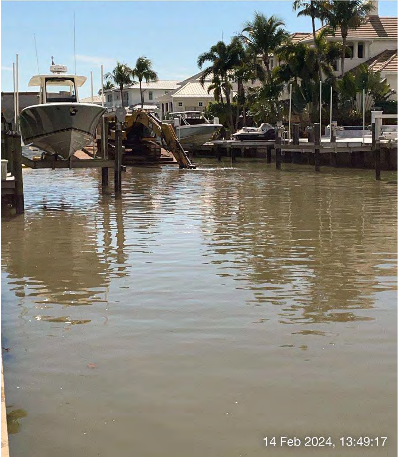
323 excavator grinding rock at station 5+00 in Canal A-A.
