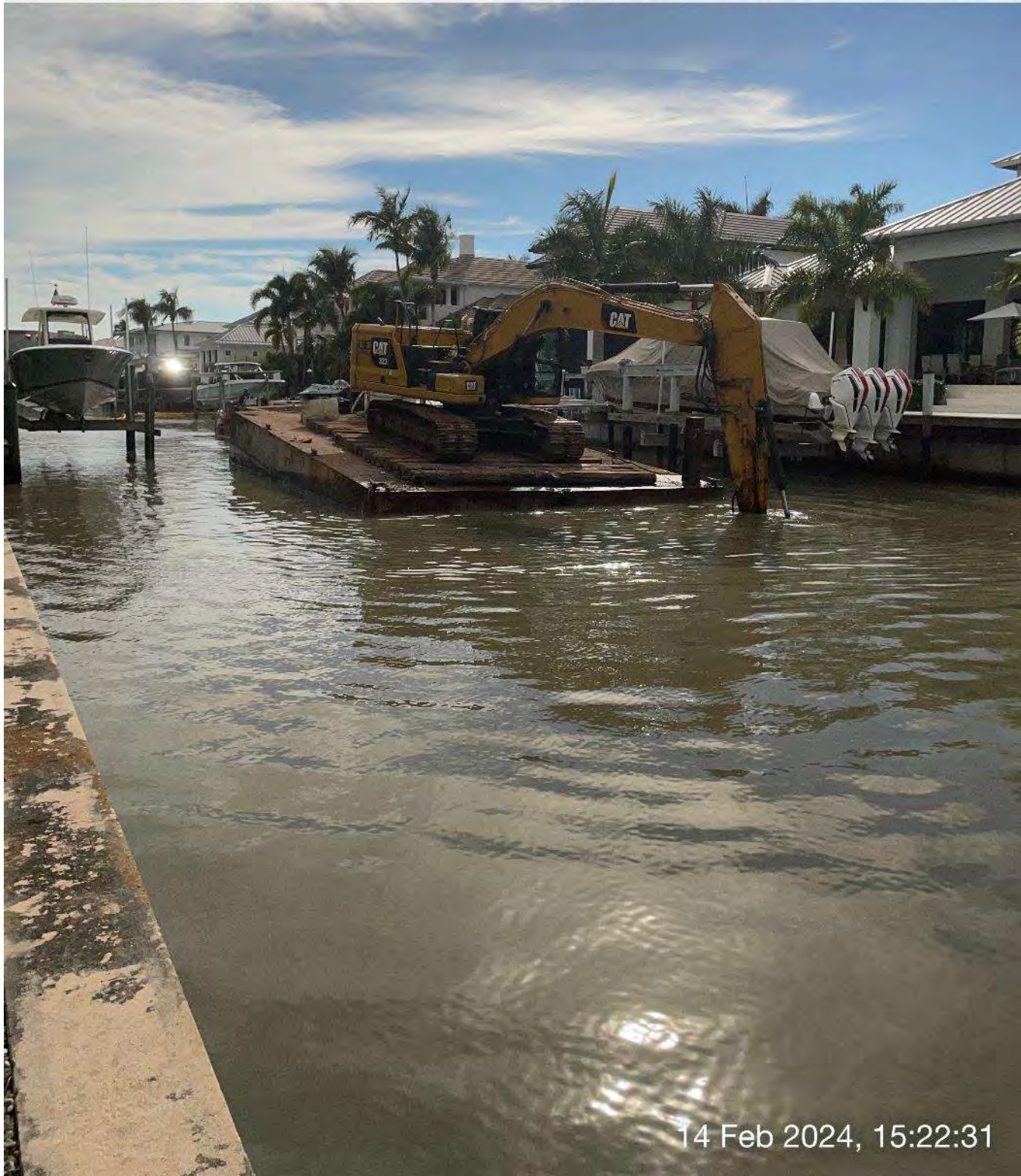
323 excavator grinding rock at station 5+50 in Canal A-A.
