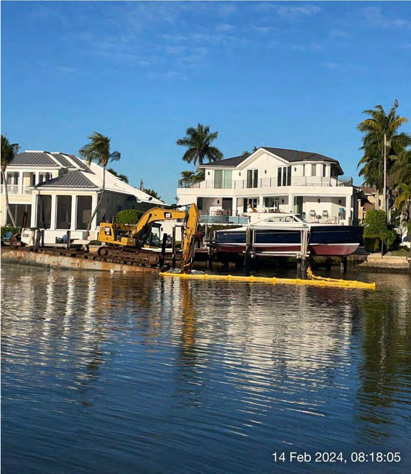
323 excavator grinding rock at station 3+50 in Canal A-A.
