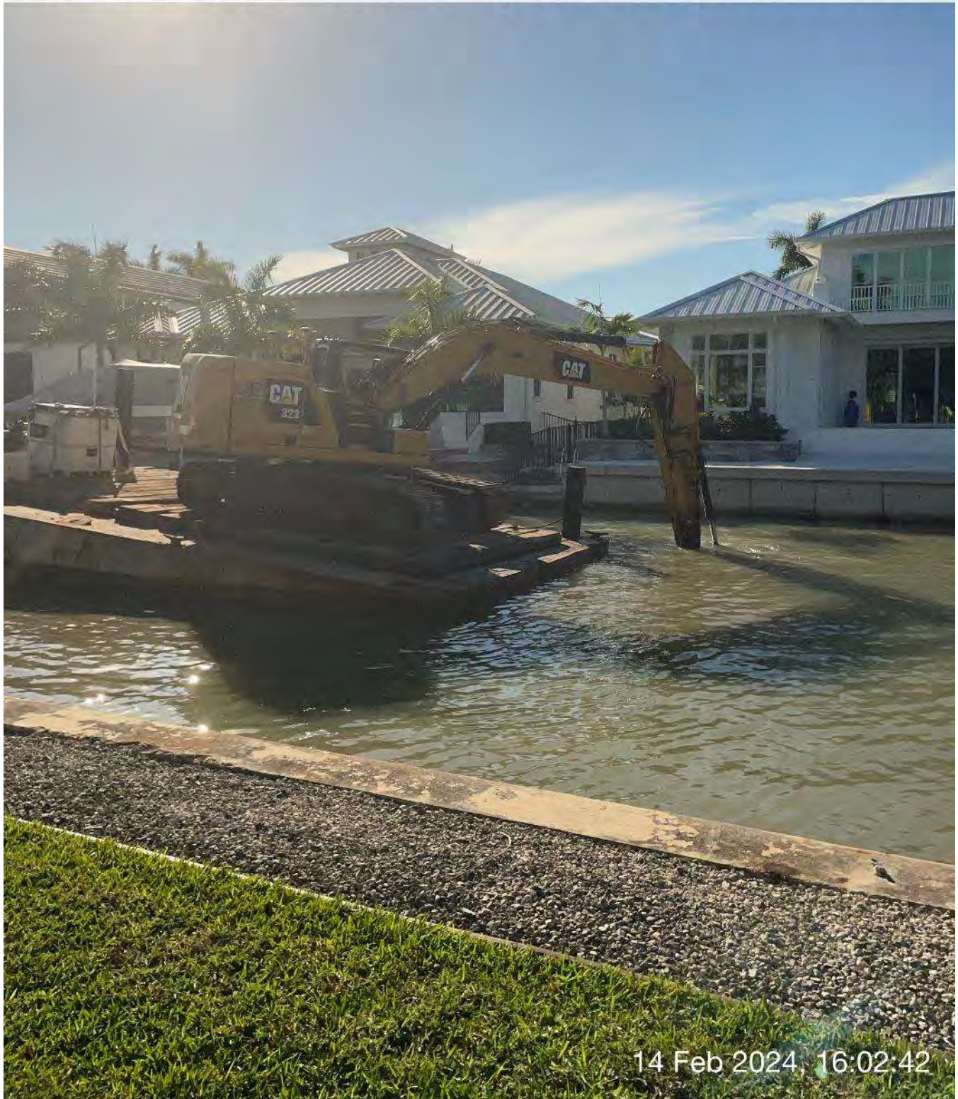
323 excavator grinding rock at station 6+00 in Canal A-A.
