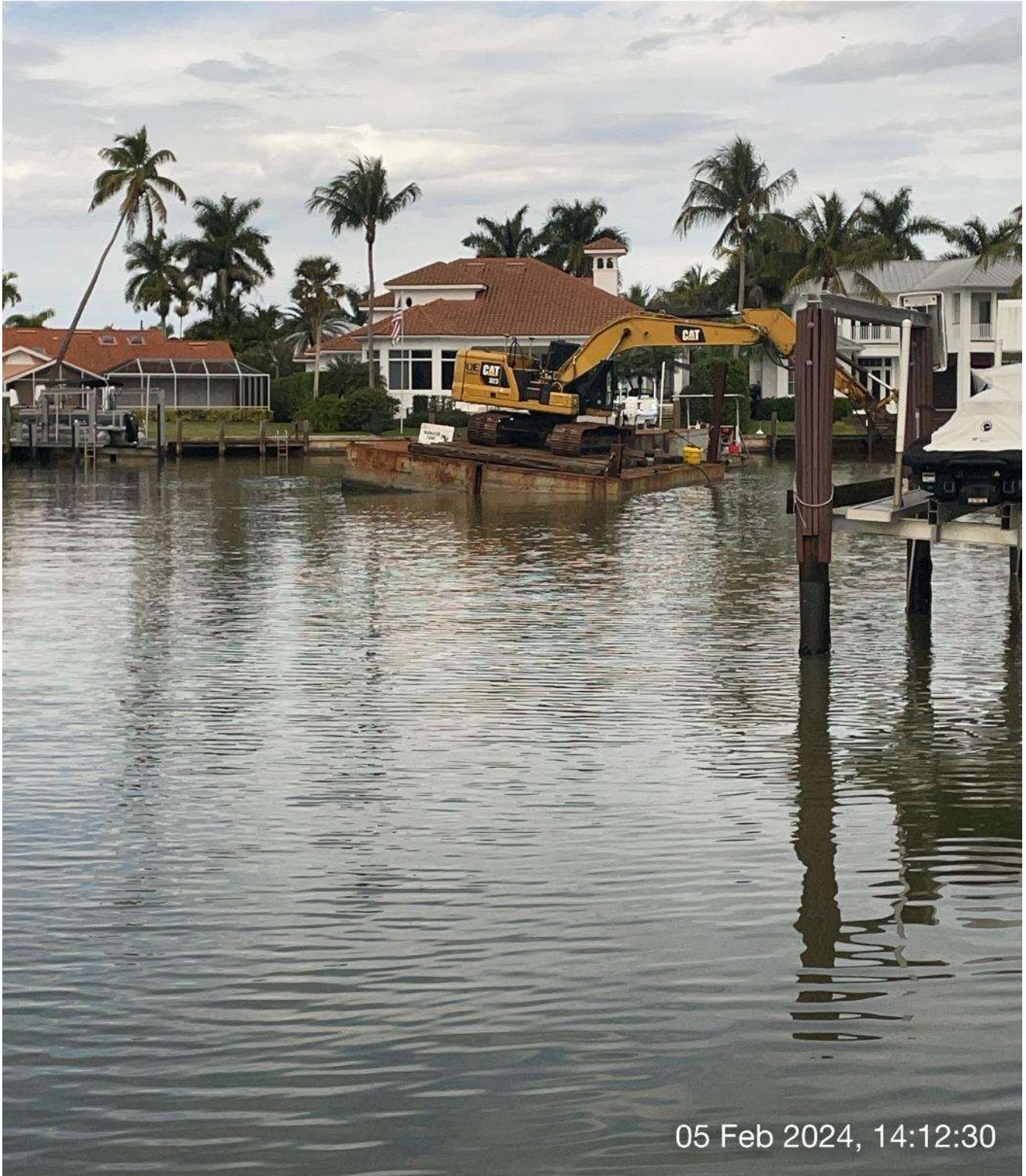
323 excavator grinding rock at station 12+50 in Canal A-A.
