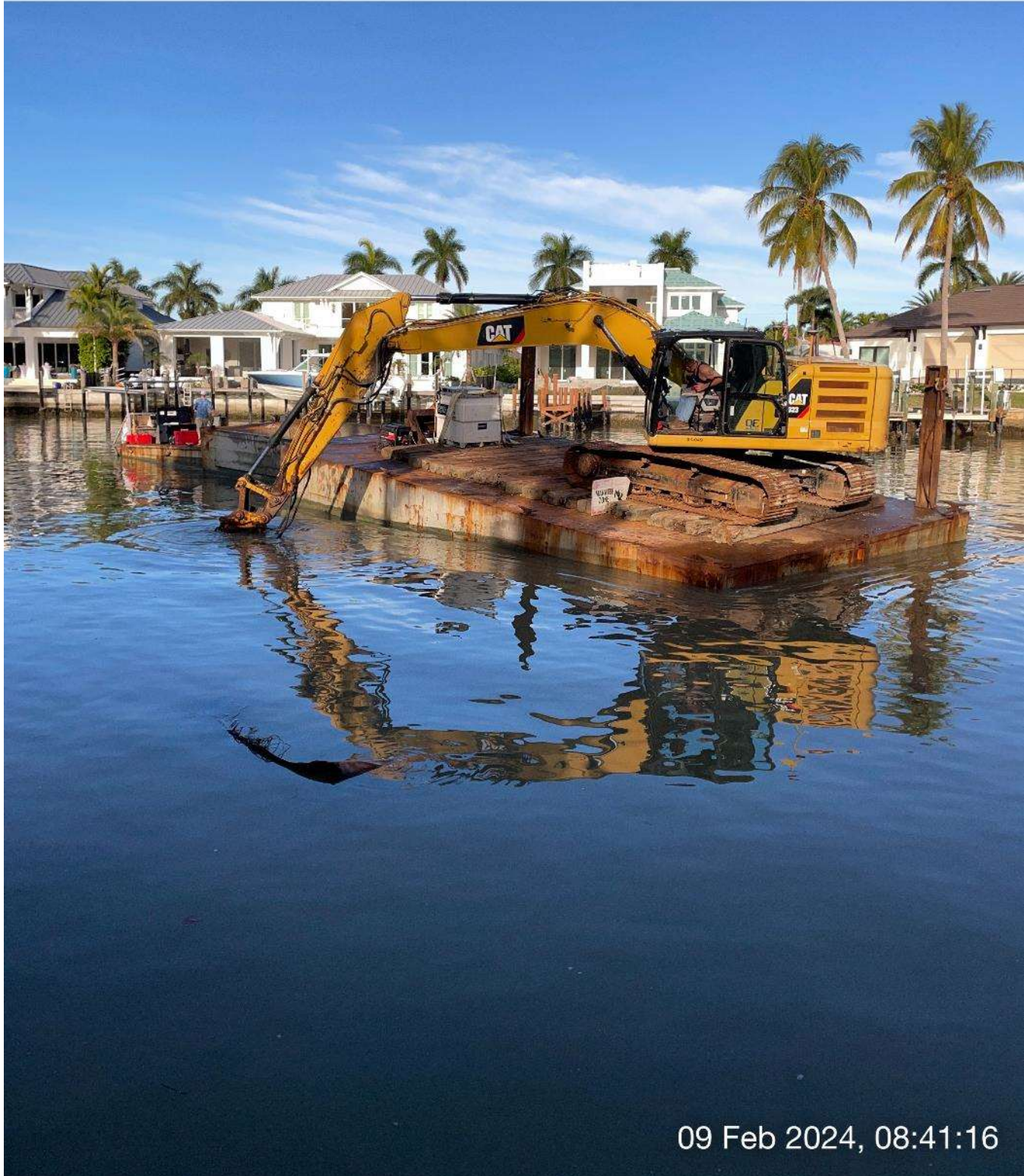
323 excavator grinding rock at station 12+75 in Canal A-A.
