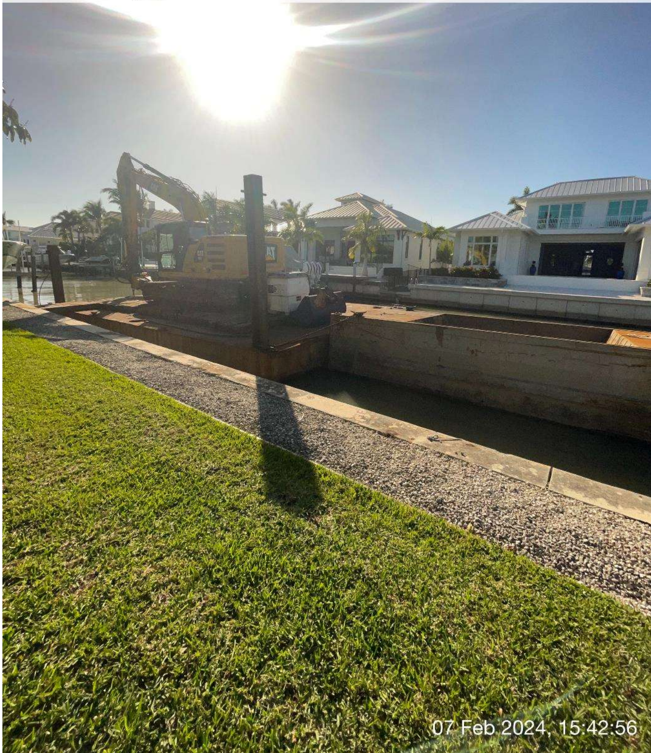
Equipment staged at station 6+00 in Canal A-A.
