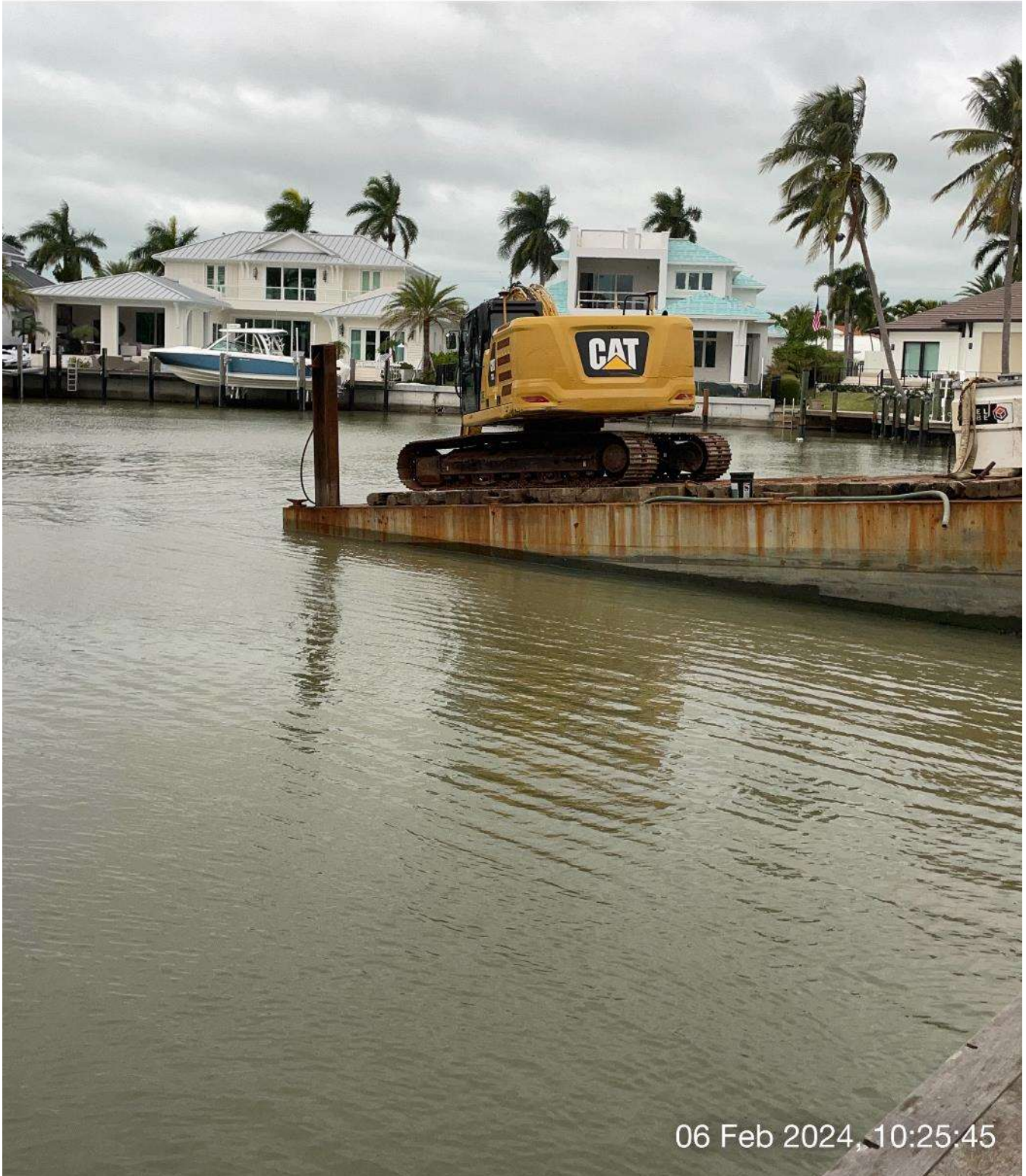
323 excavator grinding rock at station 13+00 in Canal A-A.
