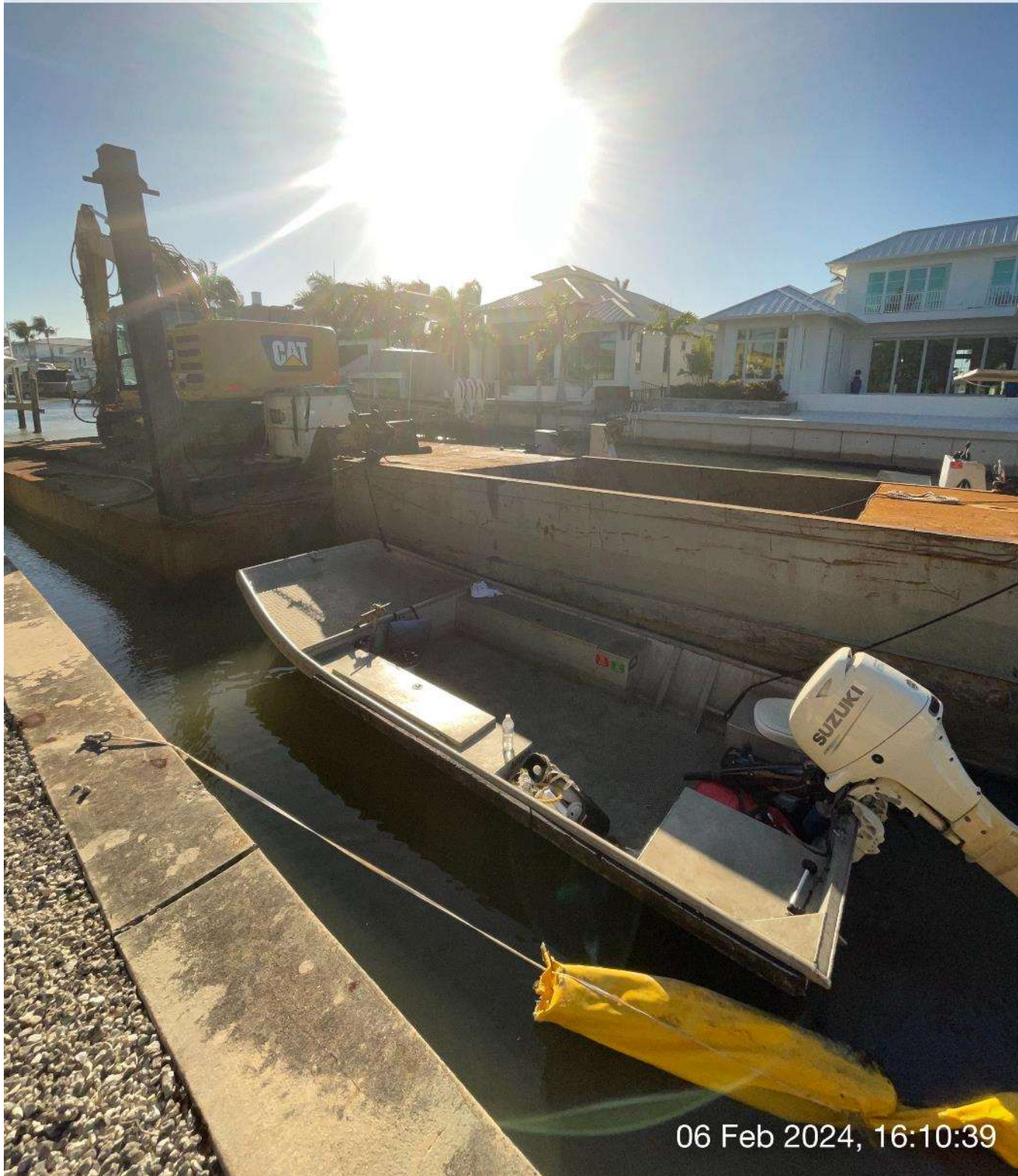
Equipment staged at station 6+00 in Canal A-A.
