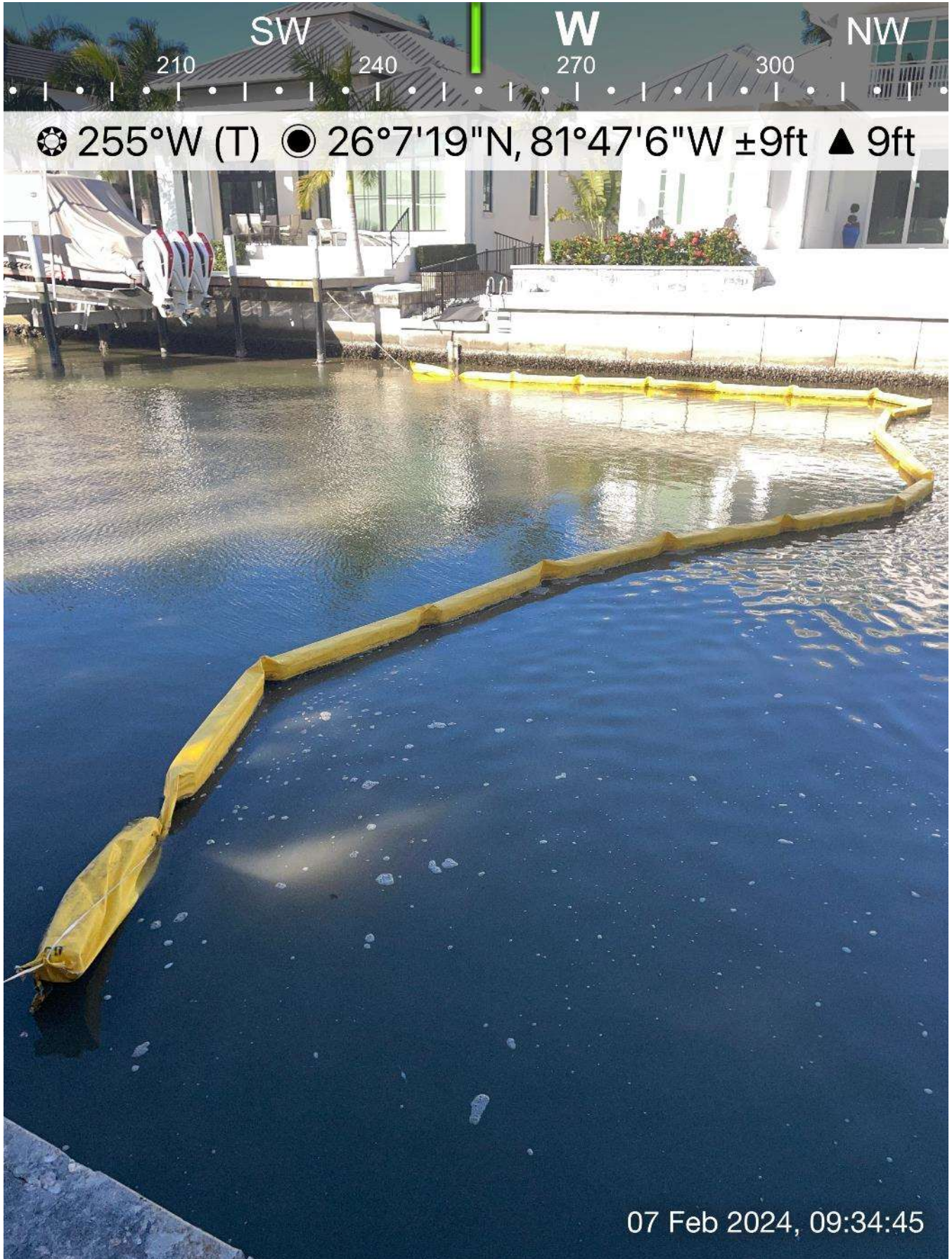
Turbidity curtain in place at station 6+00 in Canal A-A.
