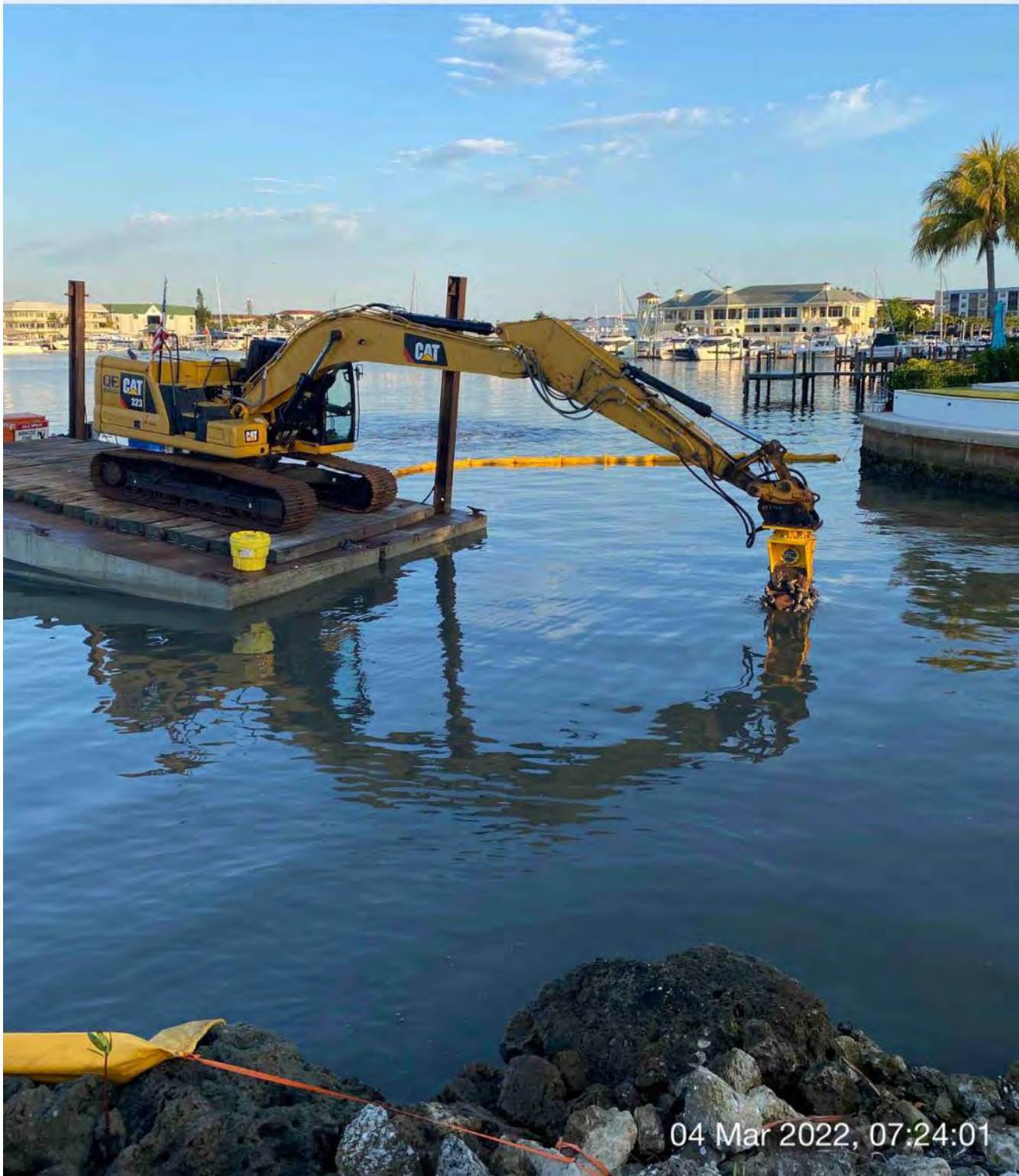
323 excavator grinding rock at station 0+00
