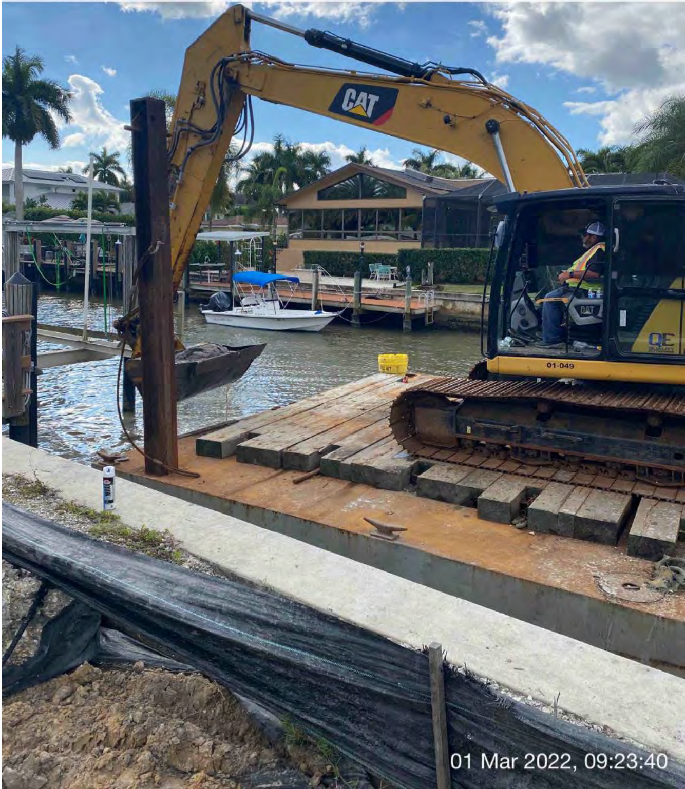
323 excavator removing material from station 2+50 and transferring to hopper
