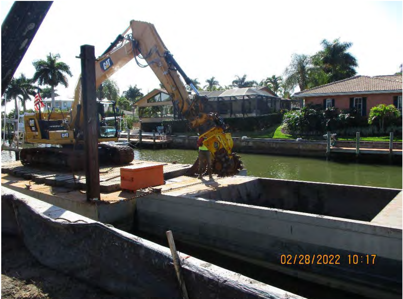
323 excavator on barge with Epiroc grinder at station 2+50
