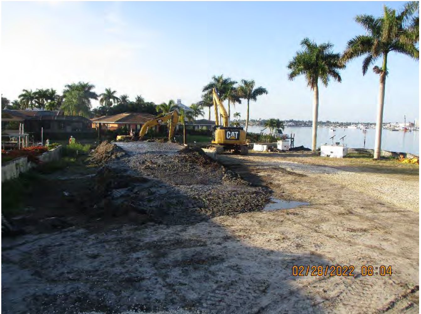
Removed material at dewatering site at 1300 Curlew Avenue
