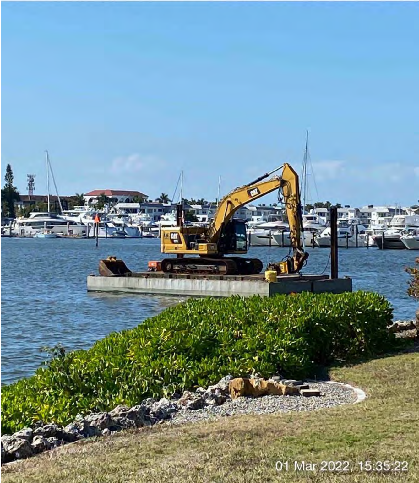
323 excavator and barge in Canal BB-BB at station 0+00
