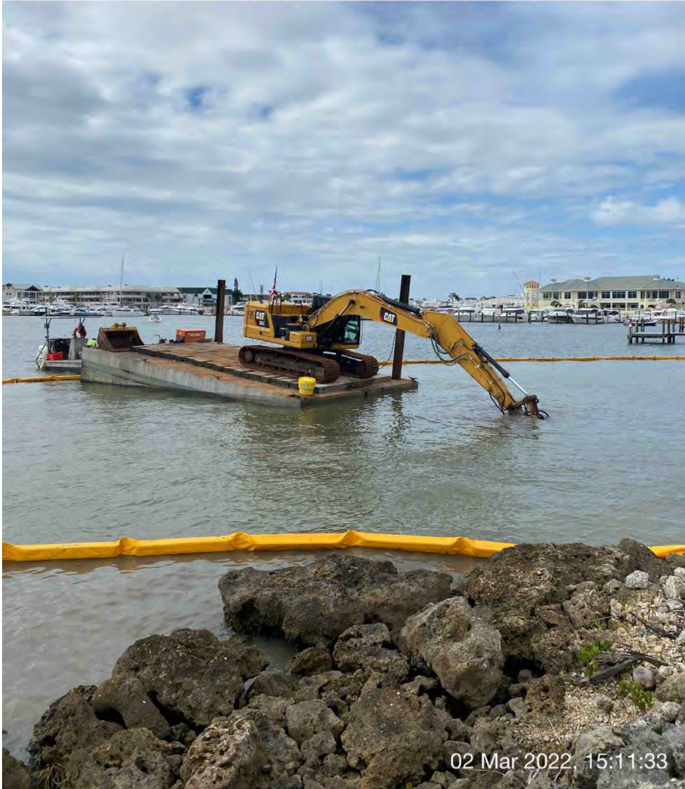
323 excavator grinding rock at station 1+00
