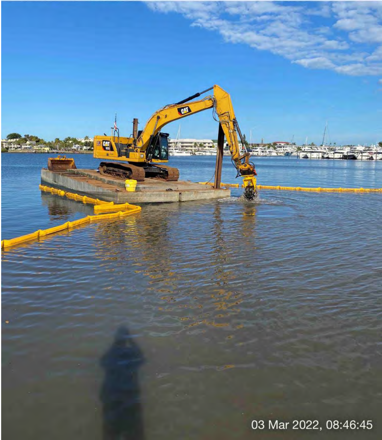
323 excavator grinding rock at station 0+50
