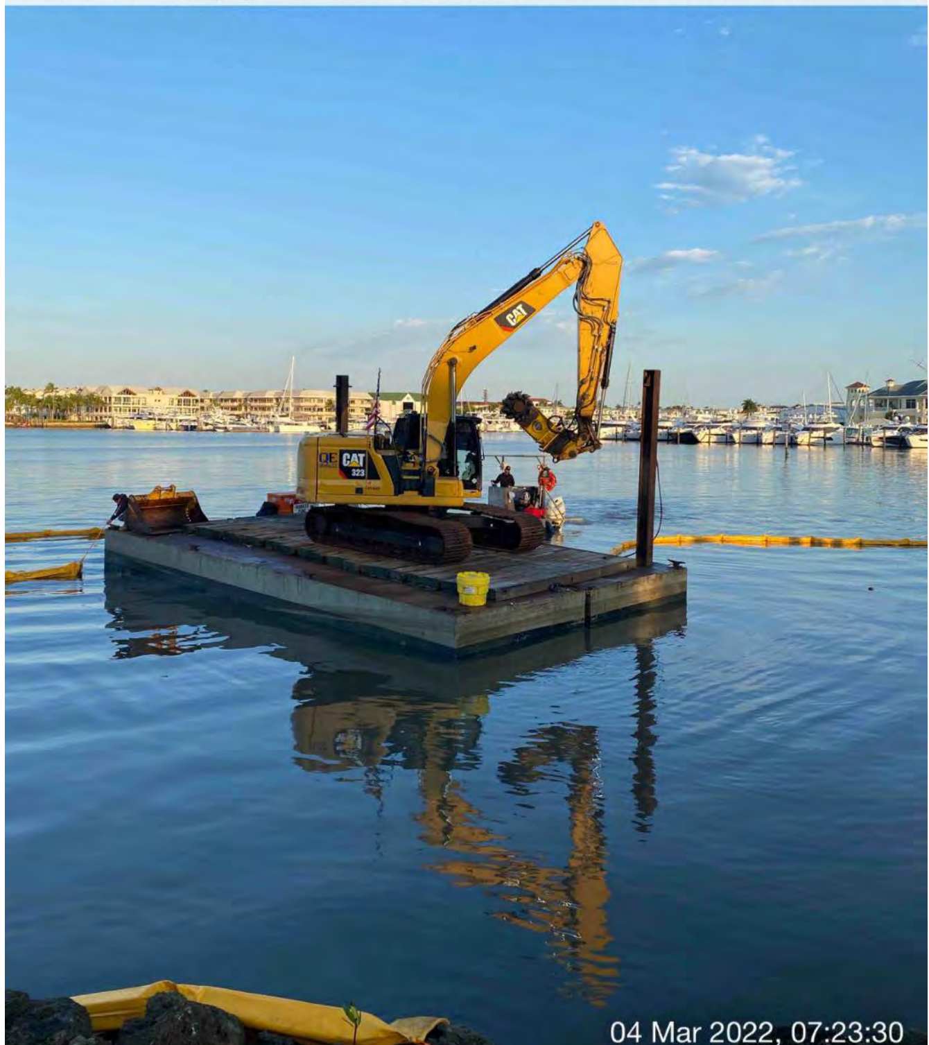
323 excavator with Epiroc grinder on barge at station 0+50
