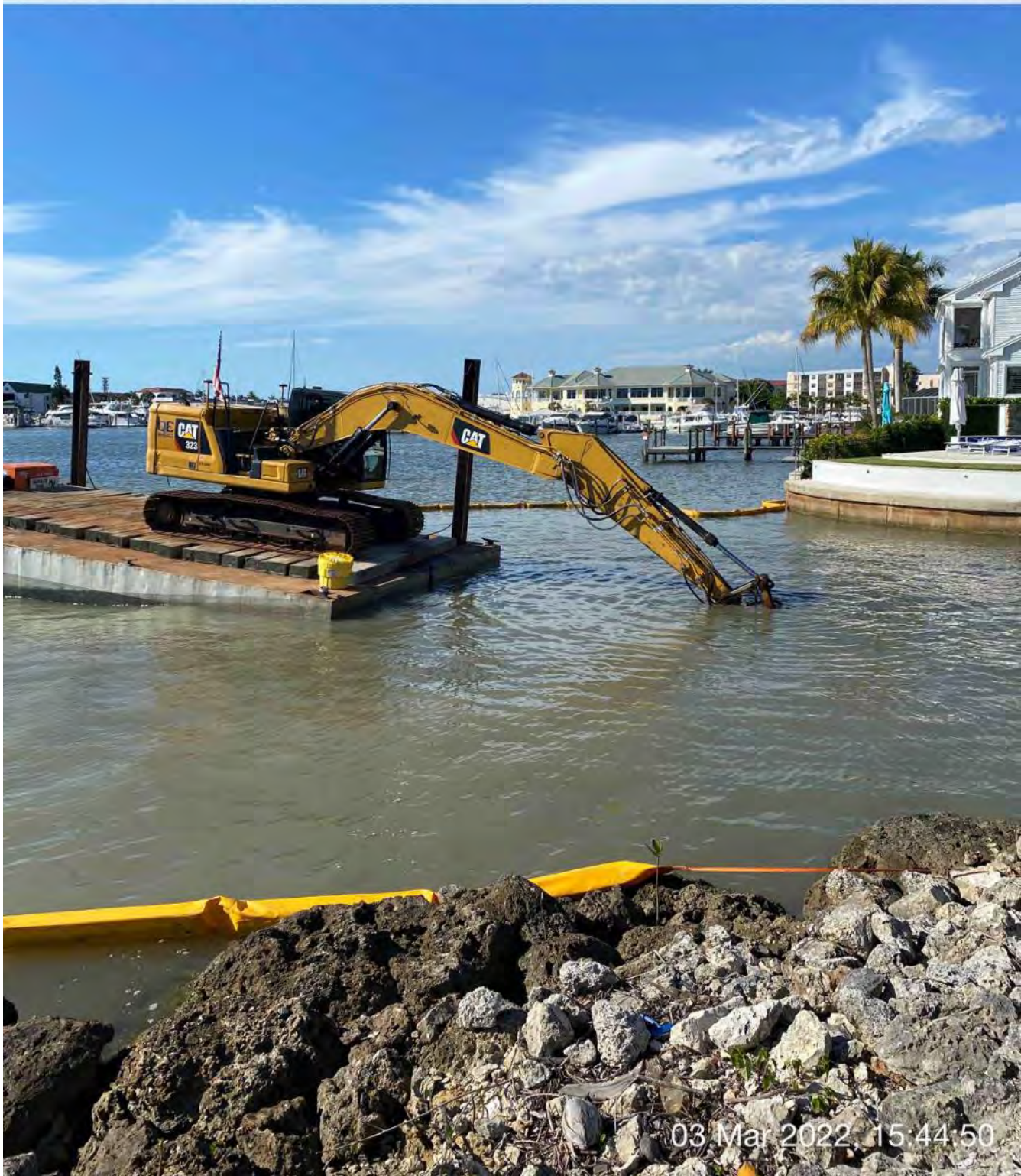
323 excavator grinding rock at station 1+00
