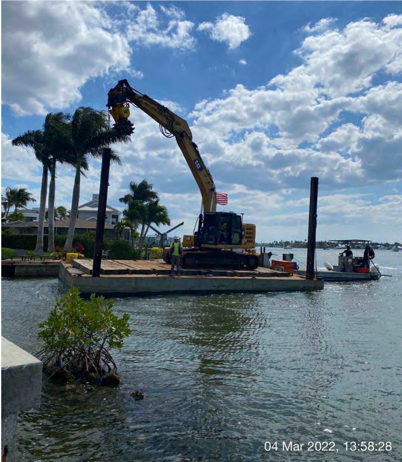
Push boat transporting barge and 323 excavator from Canal BB-BB to Canal CC-CC
