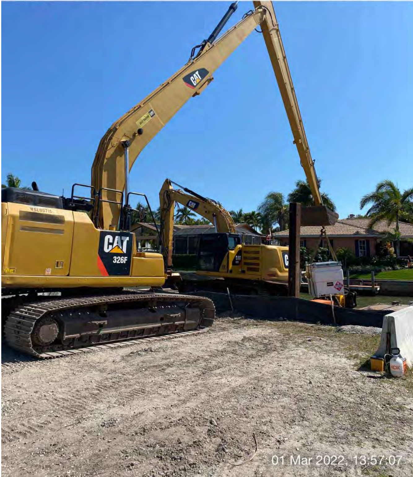
326 excavator transferring fuel cube to barge for refueling 323 excavator
