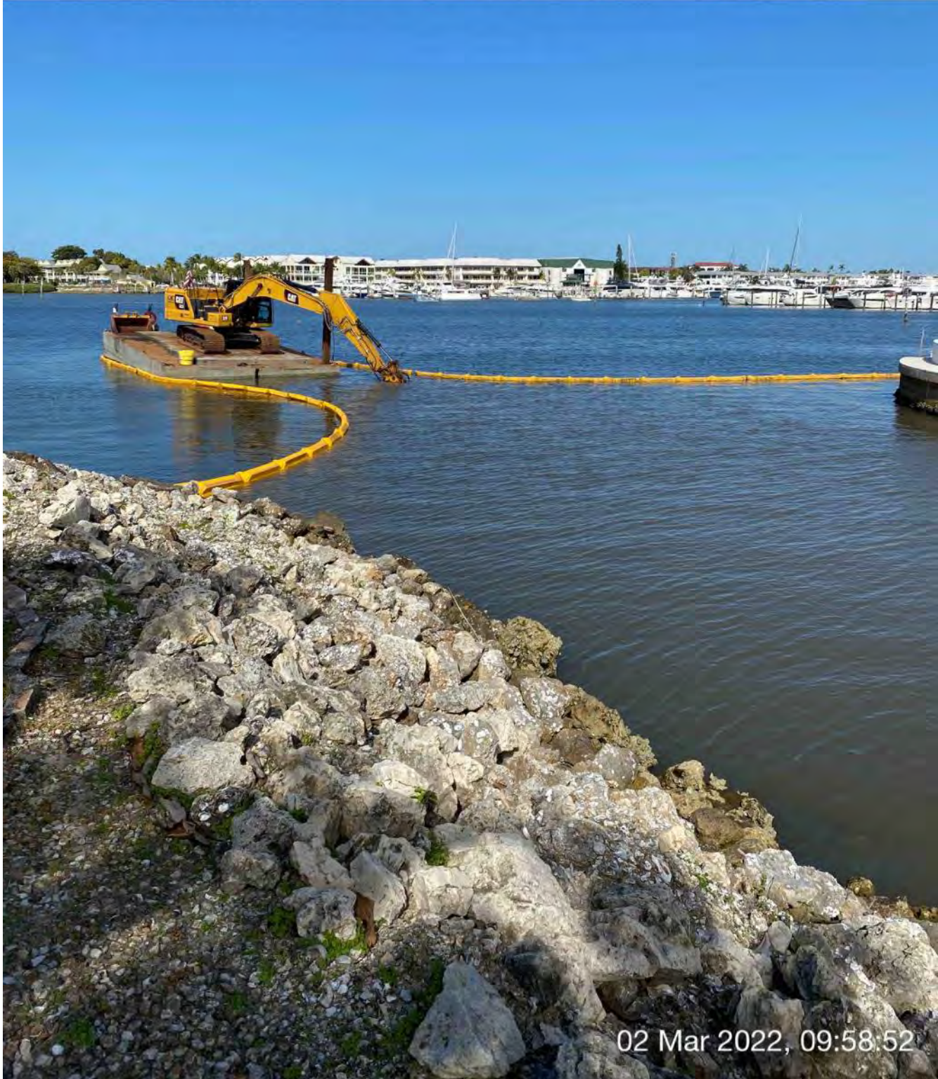
323 excavator grinding rock at station 0+00
