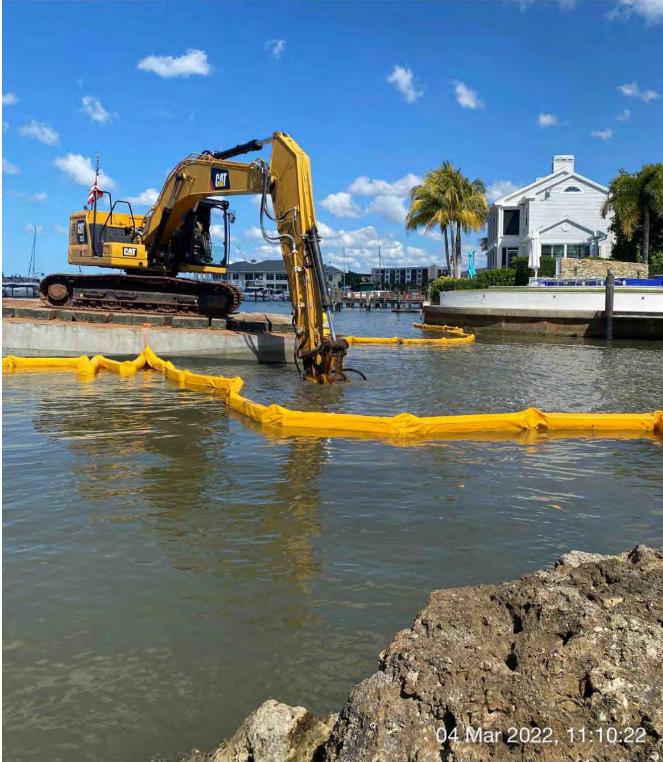
323 excavator grinding rock at station 1+00
