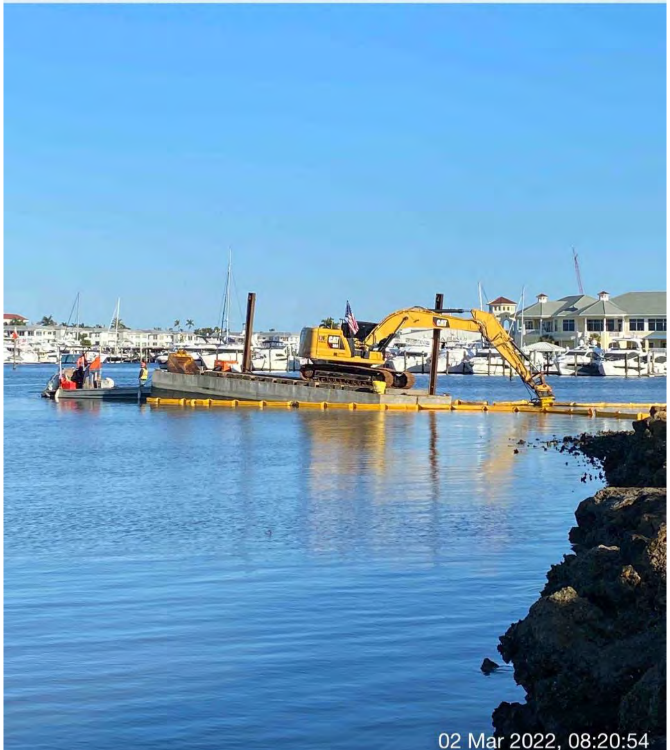
323 excavator grinding rock at station 0+00
