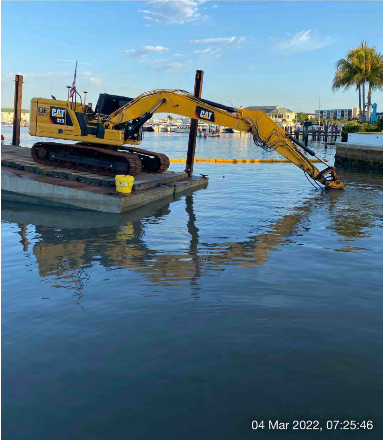
323 excavator grinding rock at station 0+00
