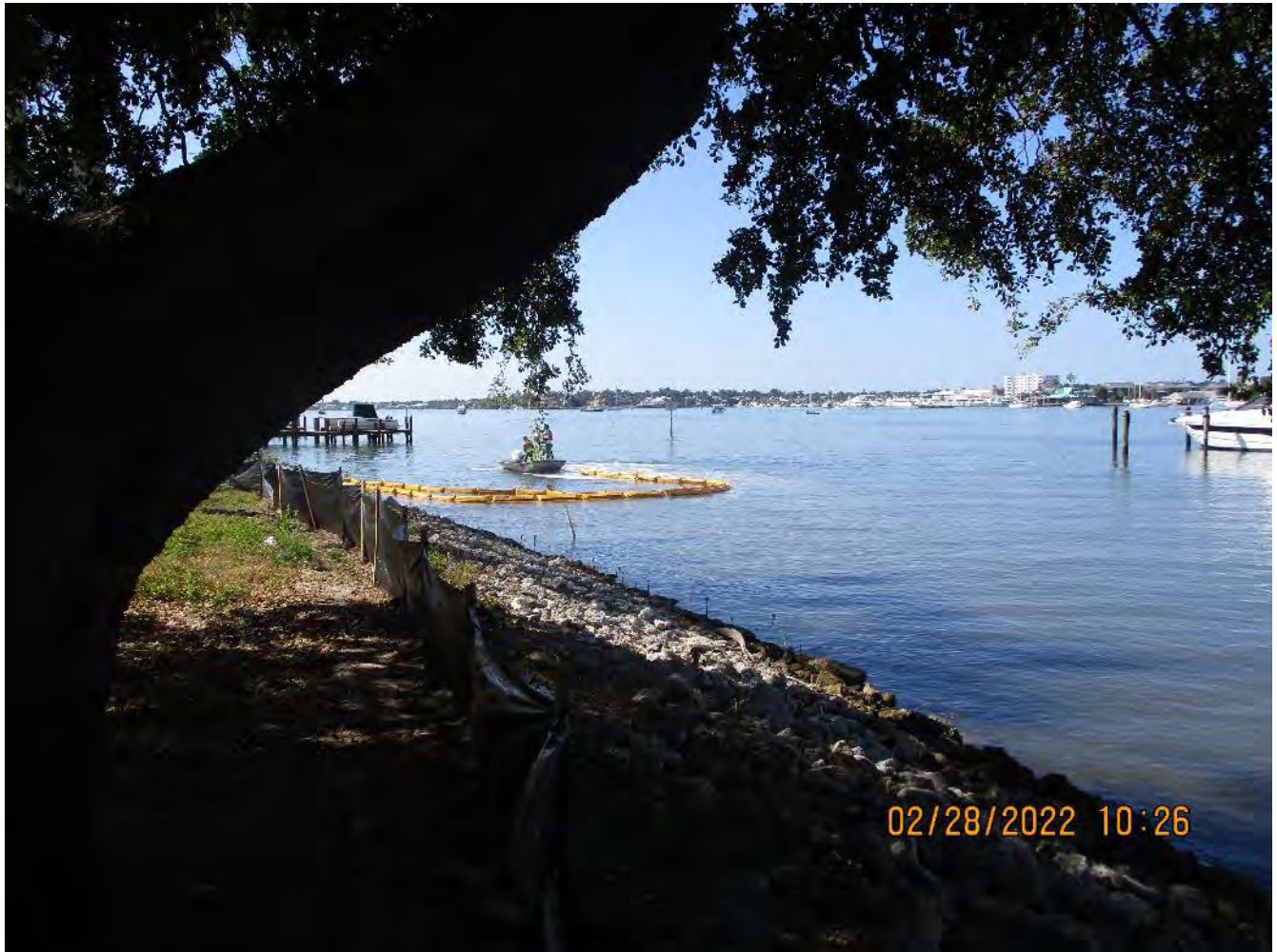
Installing turbidity curtain across the mouth of Canal CC-CC
