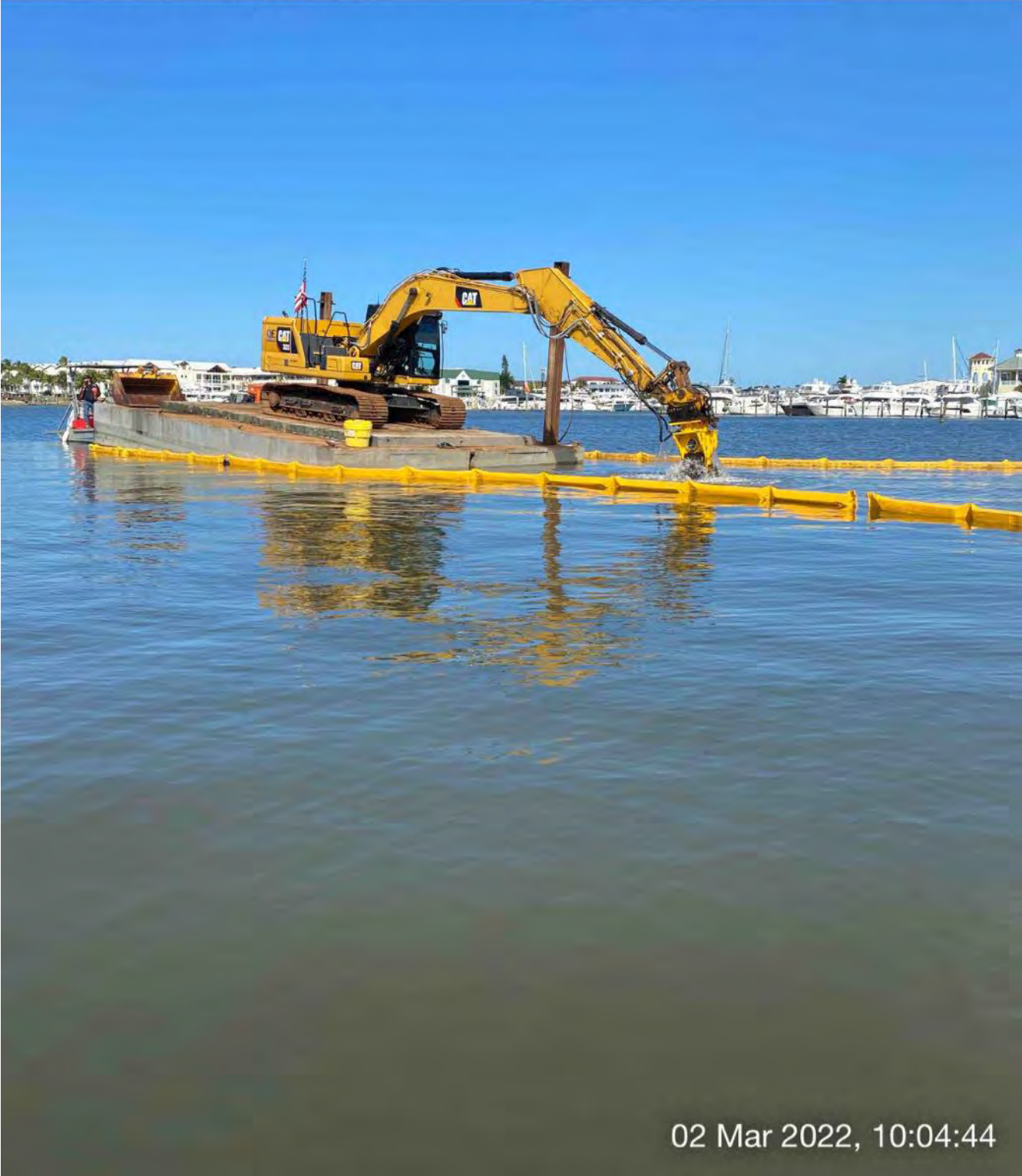
323 excavator grinding rock at station 0+50
