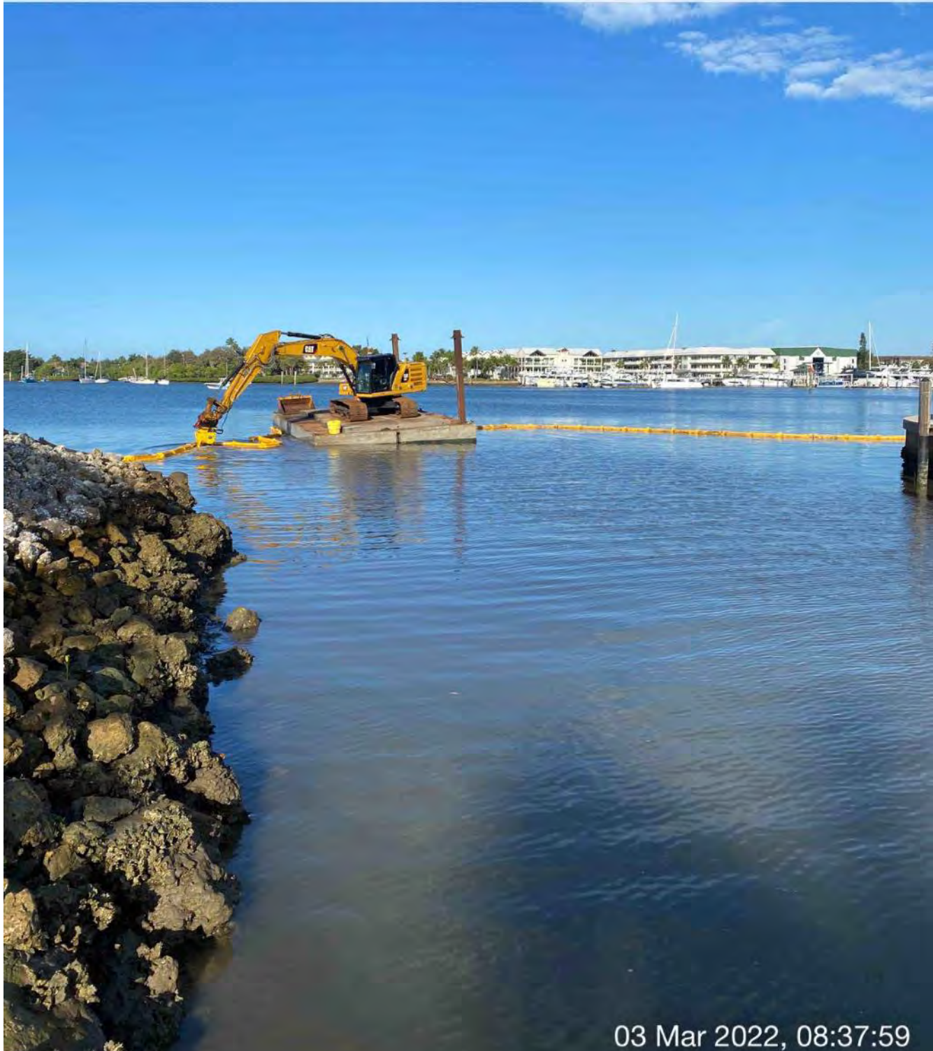
323 excavator grinding rock at station 0+50
