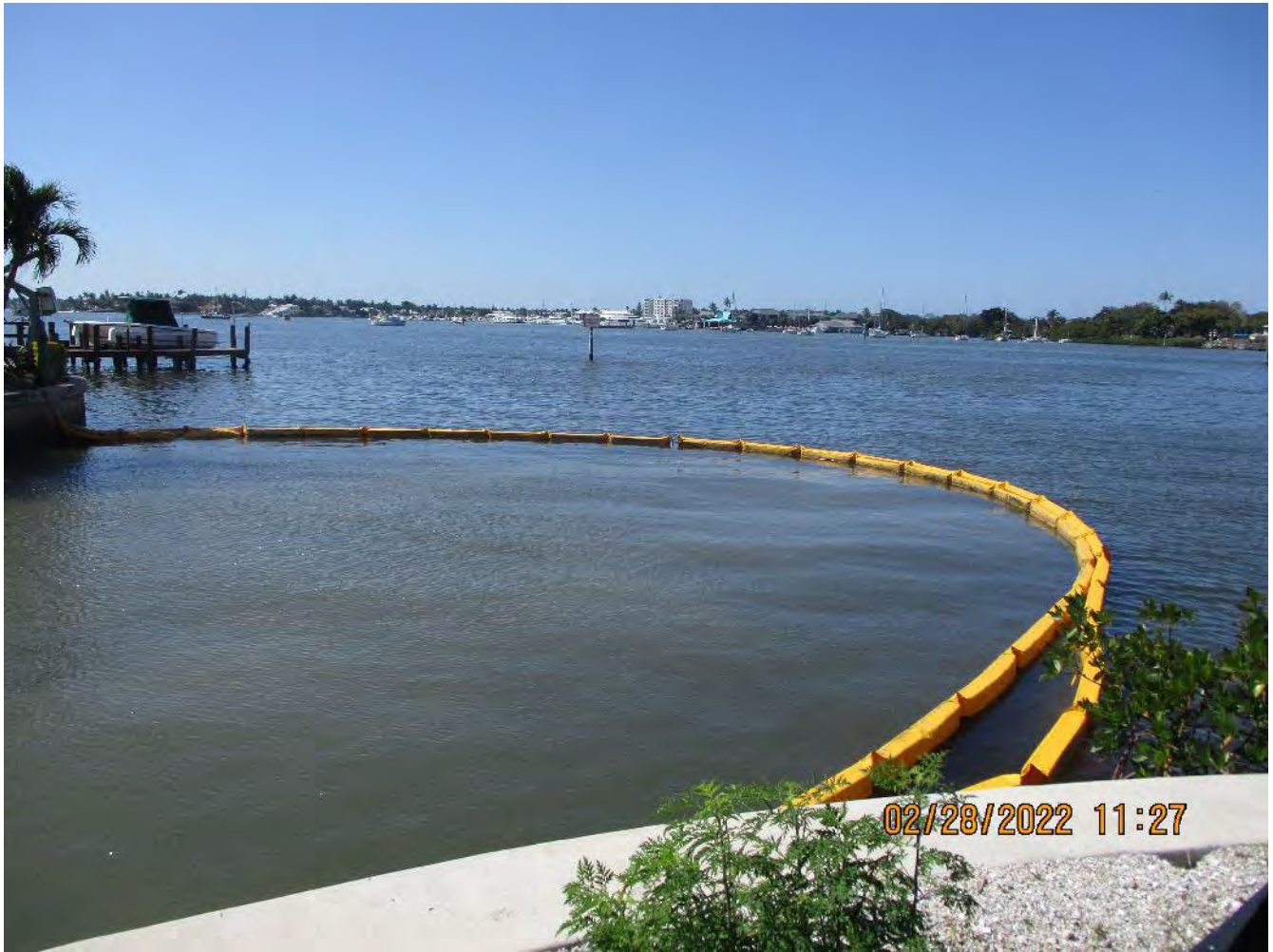
Turbidity curtain across the mouth of Canal CC-CC
