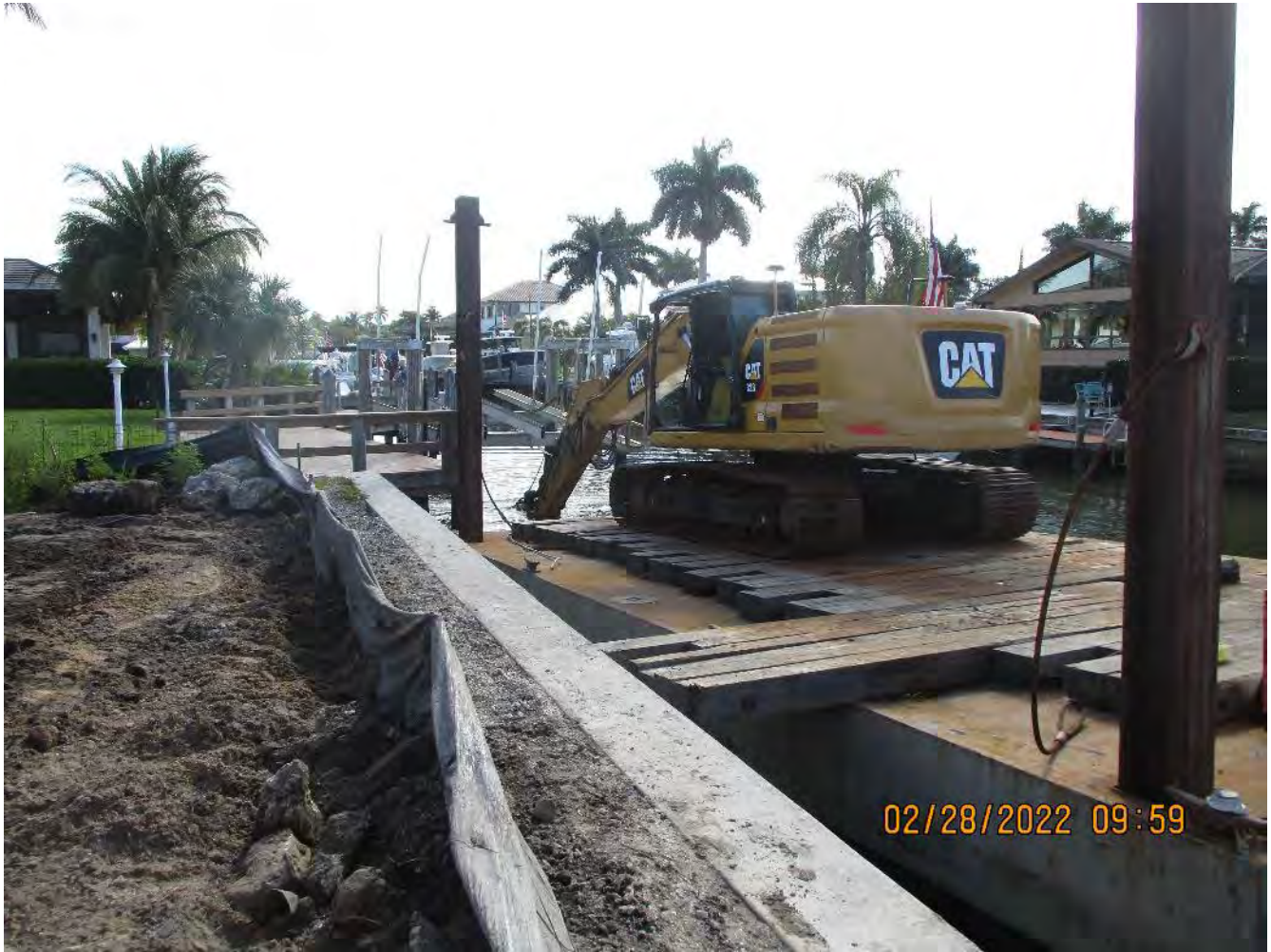
323 excavator grinding rock at station 2+75
