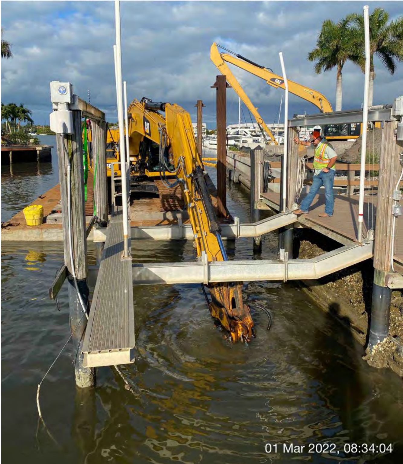
323 excavator grinding rock at station 2+75
