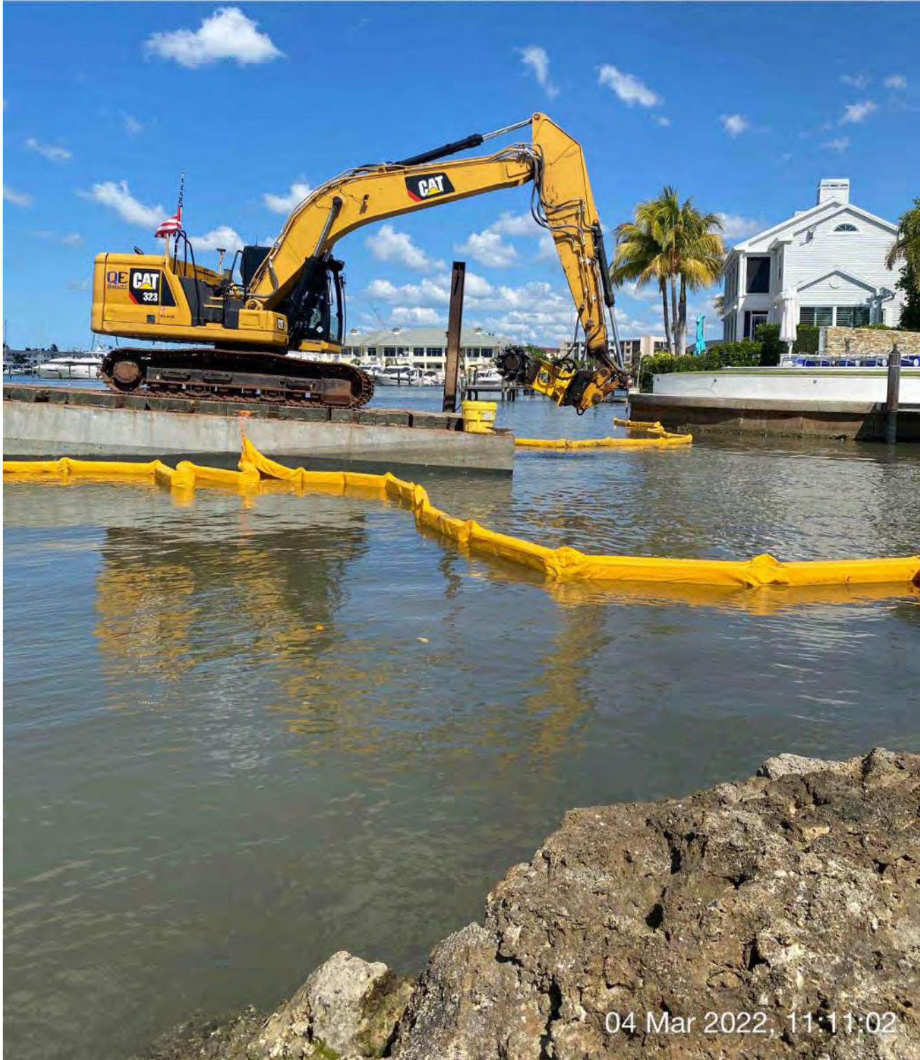
323 excavator with Epiroc grinder on barge at station 1+00
