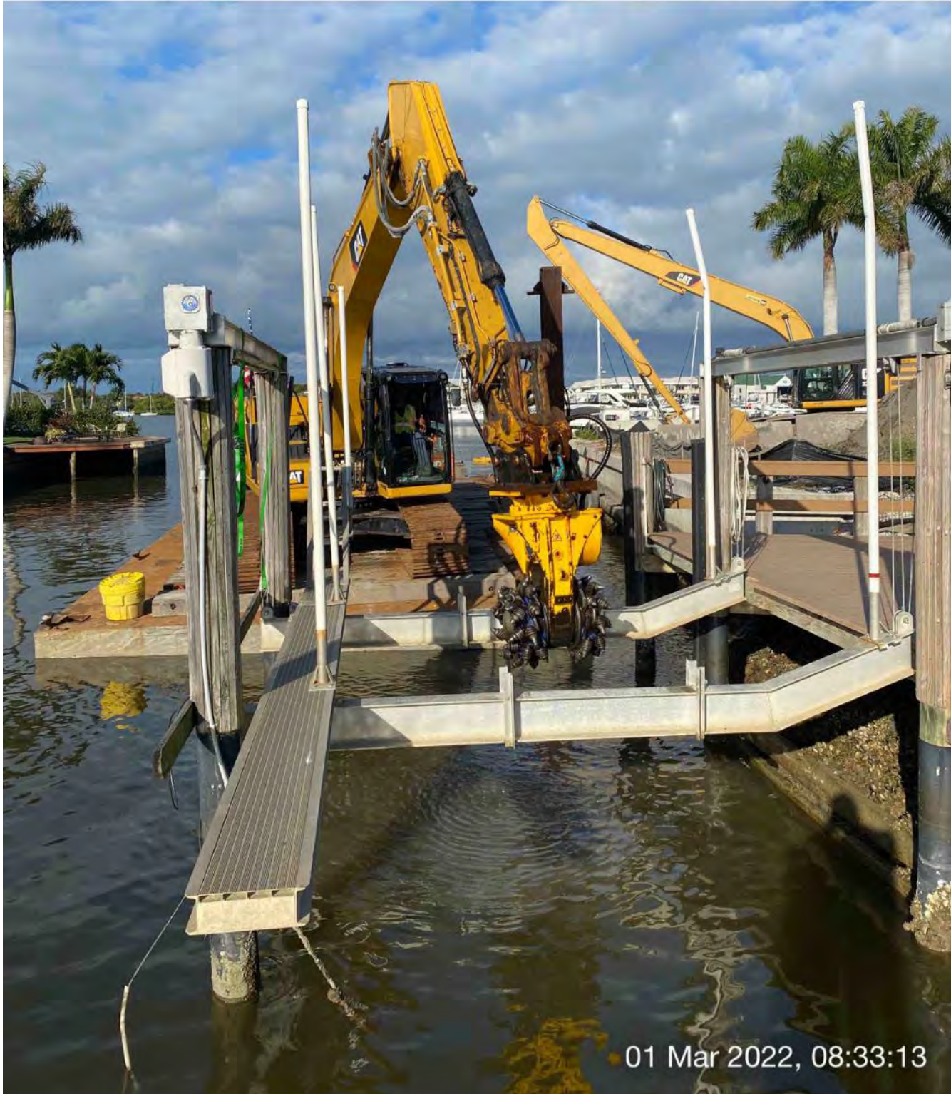
323 with Epiroc grinder at station 2+75
