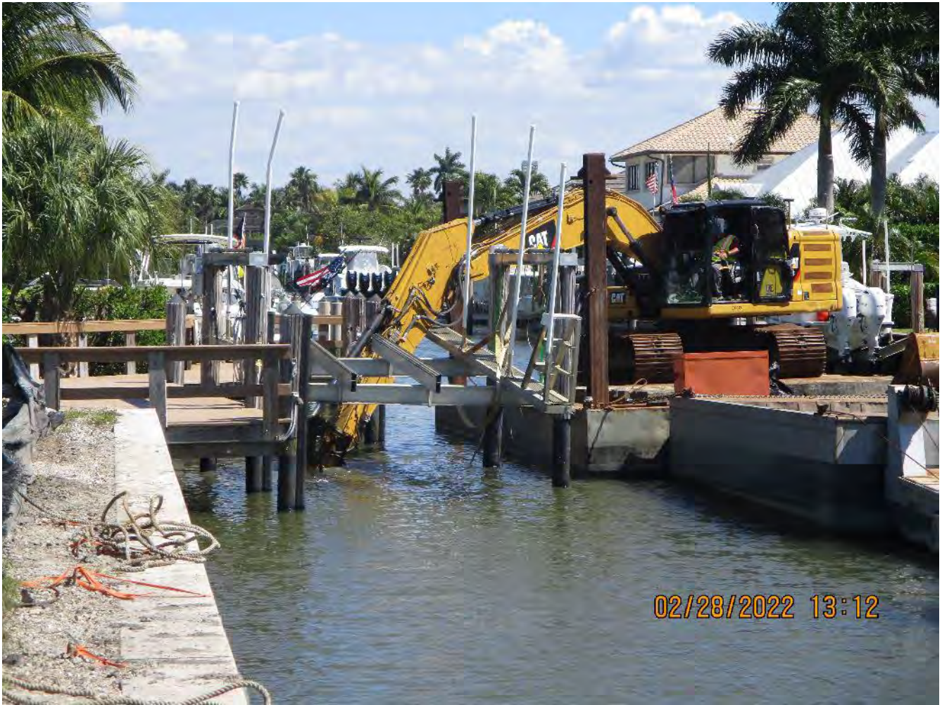
323 excavator grinding rock at station 2+75
