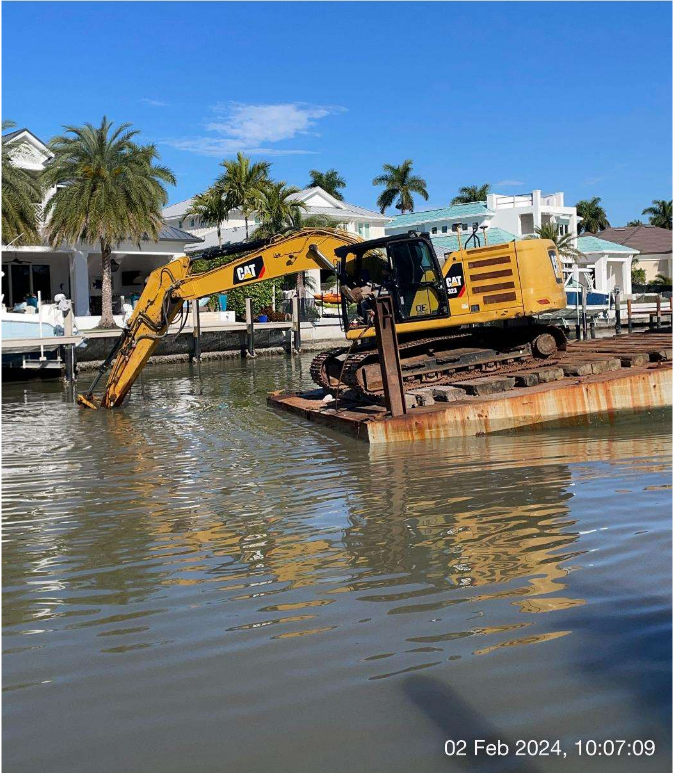
323 excavator grinding rock at station 10+00 in Canal A-A.
