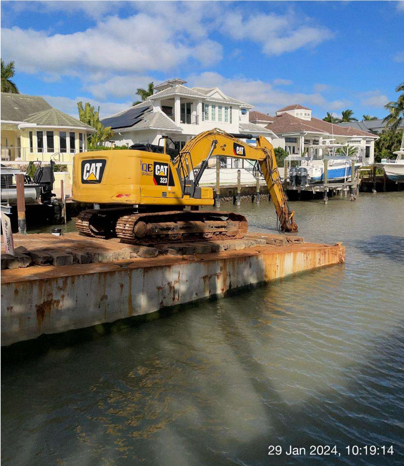
323 excavator grinding rock at station 8+75 in Canal A-A.
