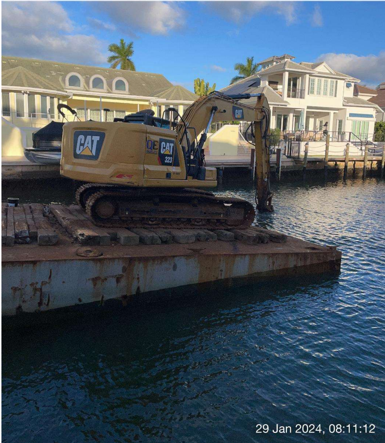
323 excavator grinding rock at station 8+50 in Canal A-A.
