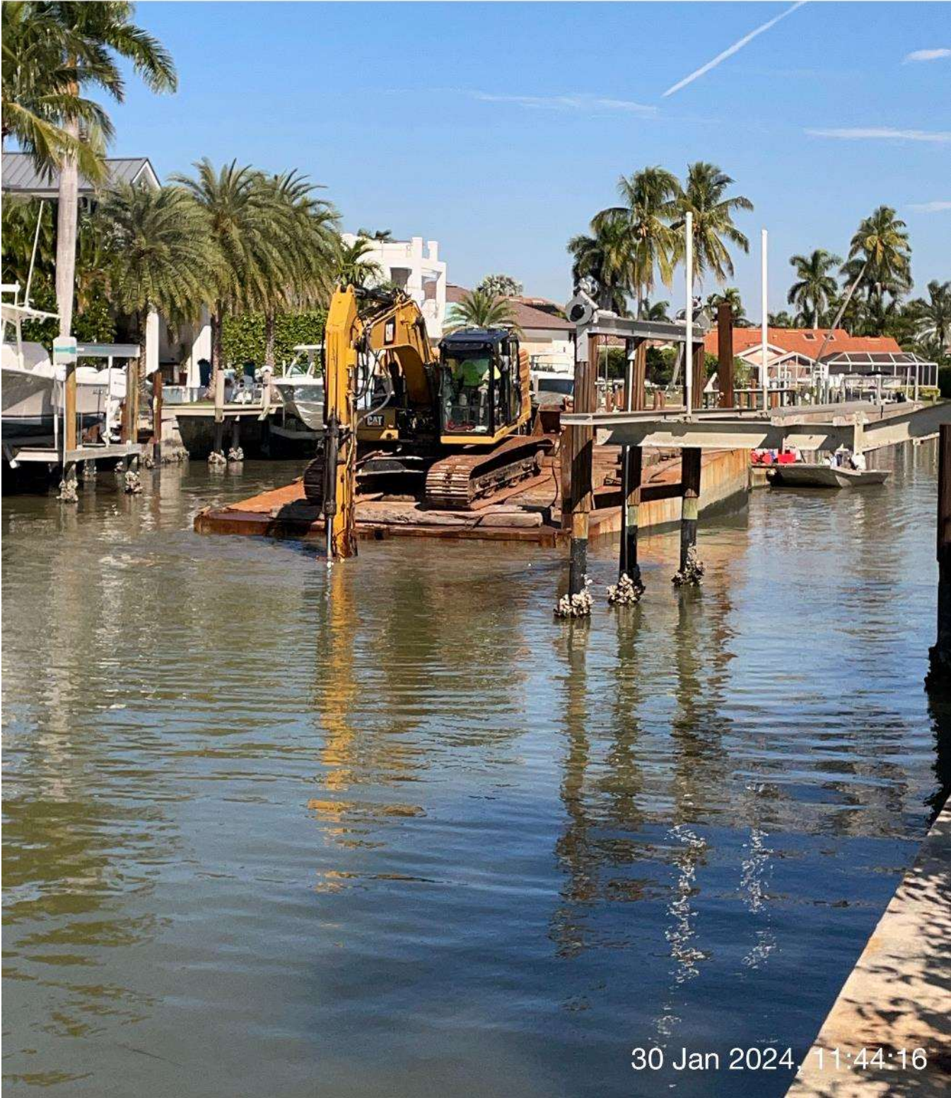
323 excavator grinding rock at station 9+00 in Canal A-A.
