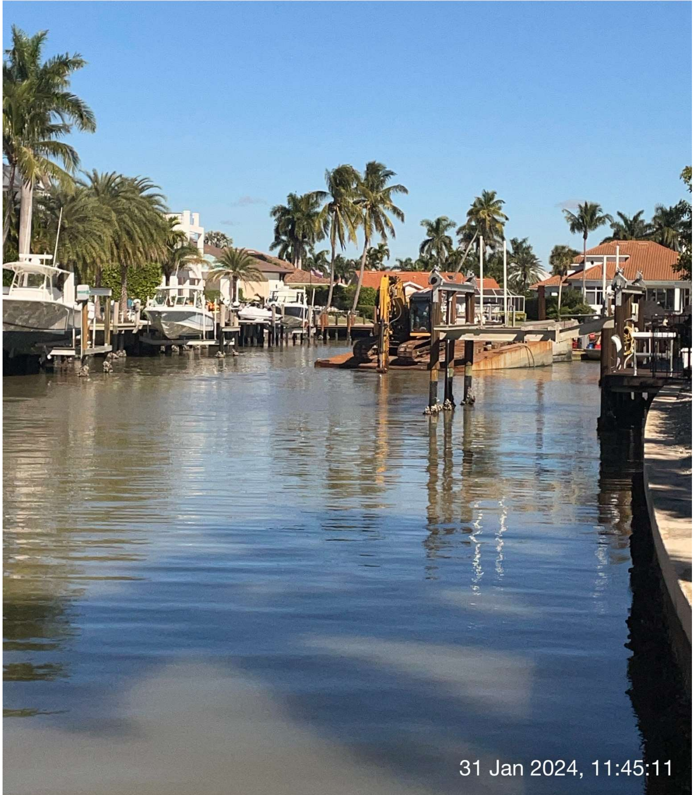
323 excavator grinding rock at station 9+50 in Canal A-A.
