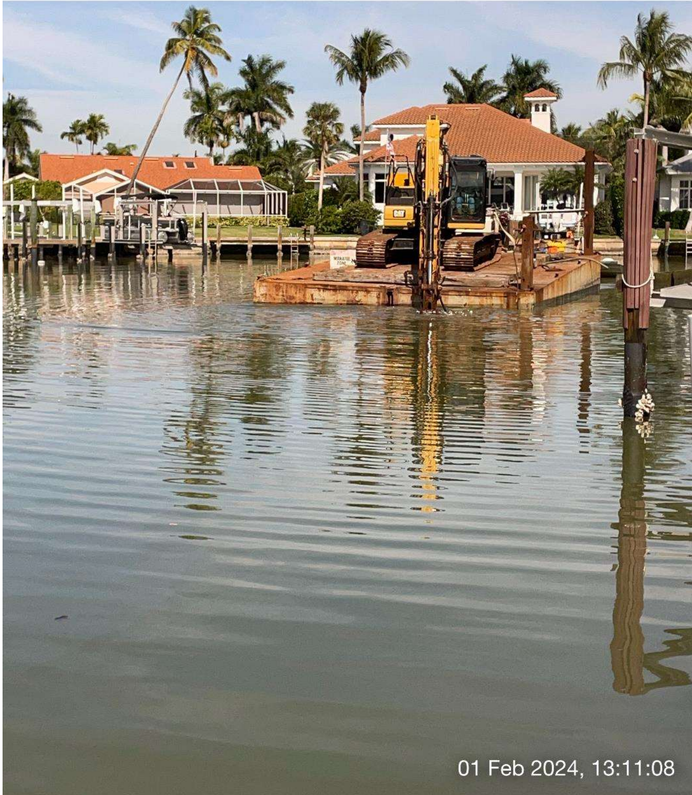
323 excavator grinding rock at station 10+50 in Canal A-A.
