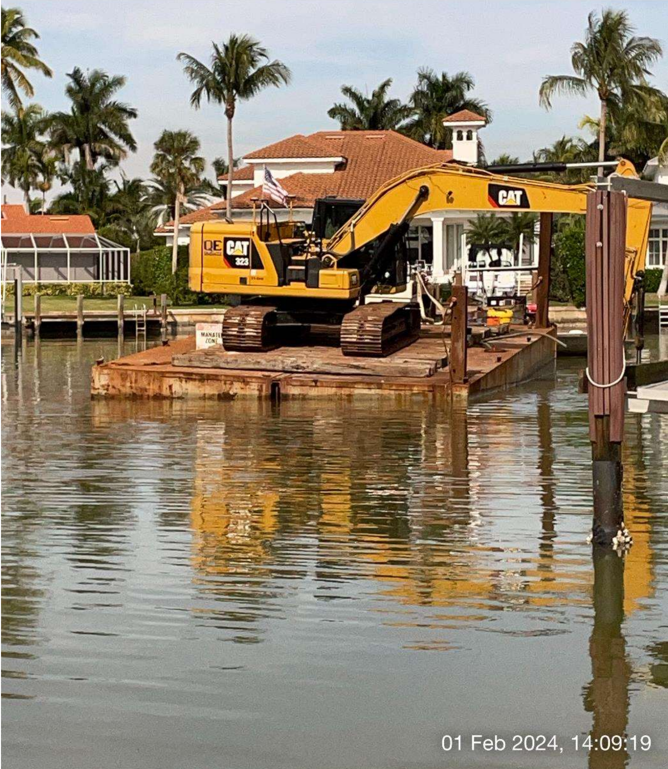
323 excavator grinding rock at station 11+50 in Canal A-A.
