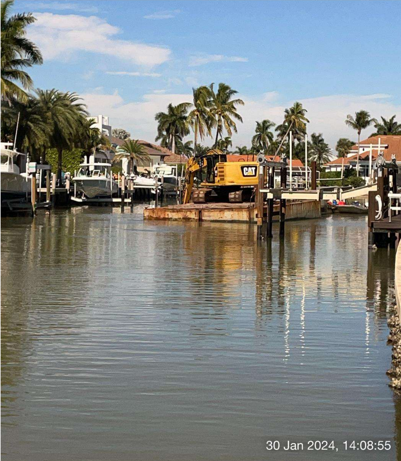
323 excavator grinding rock at station 9+25 in Canal A-A.
