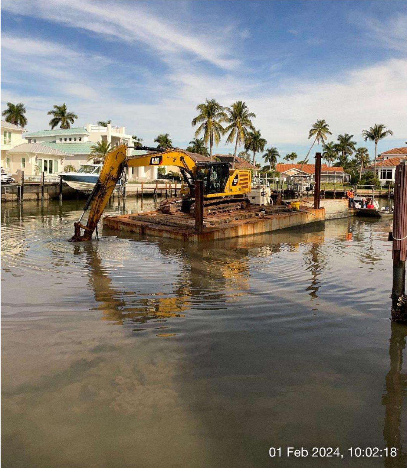
323 excavator grinding rock at station 9+75 in Canal A-A.
