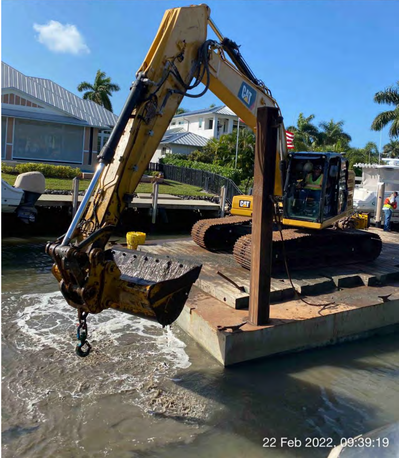
323 excavator removing material from station 5+25 and transferring to hopper
