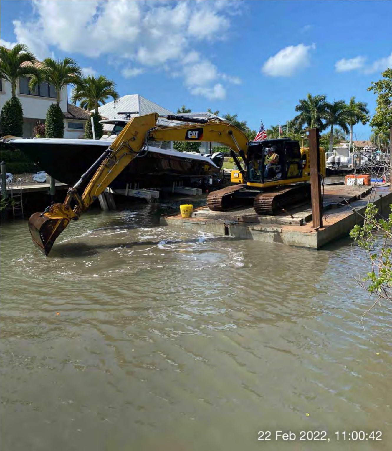
323 excavator removing material from station 7+00 and transferring to hopper
