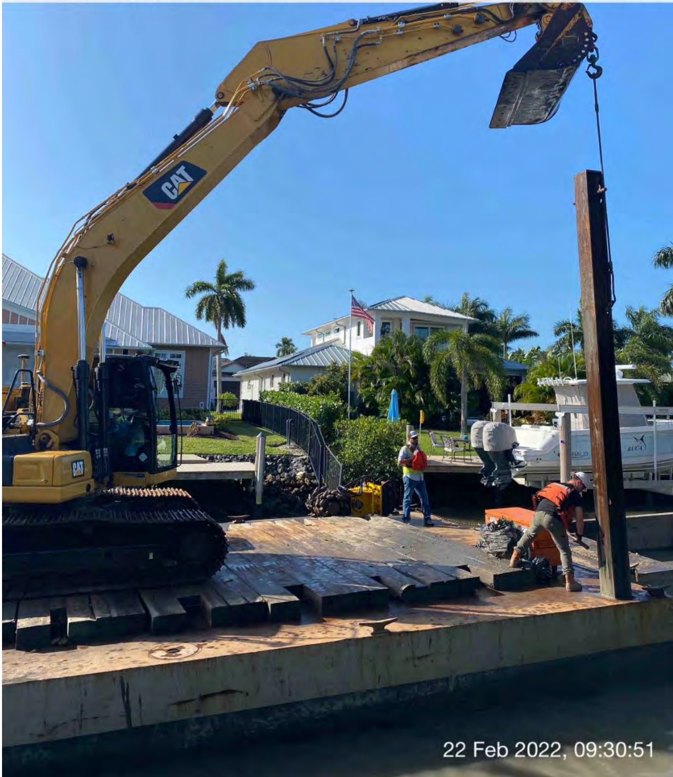
323 excavator lifting spud to allow push boat to mobilize barge at station 5+00
