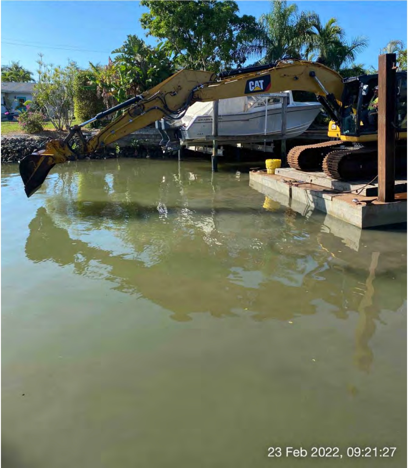
323 excavator removing material from station 13+00 and transferring to hopper
