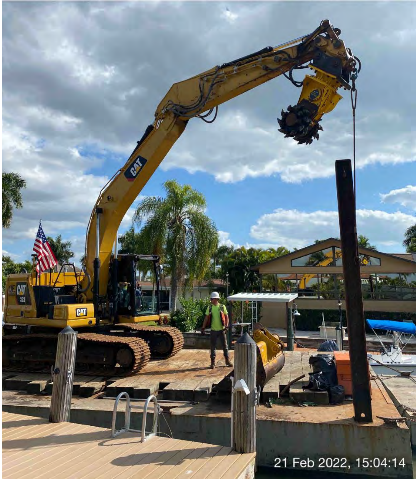
323 excavator lifting spud to allow push boat to mobilize barge at station 2+50
