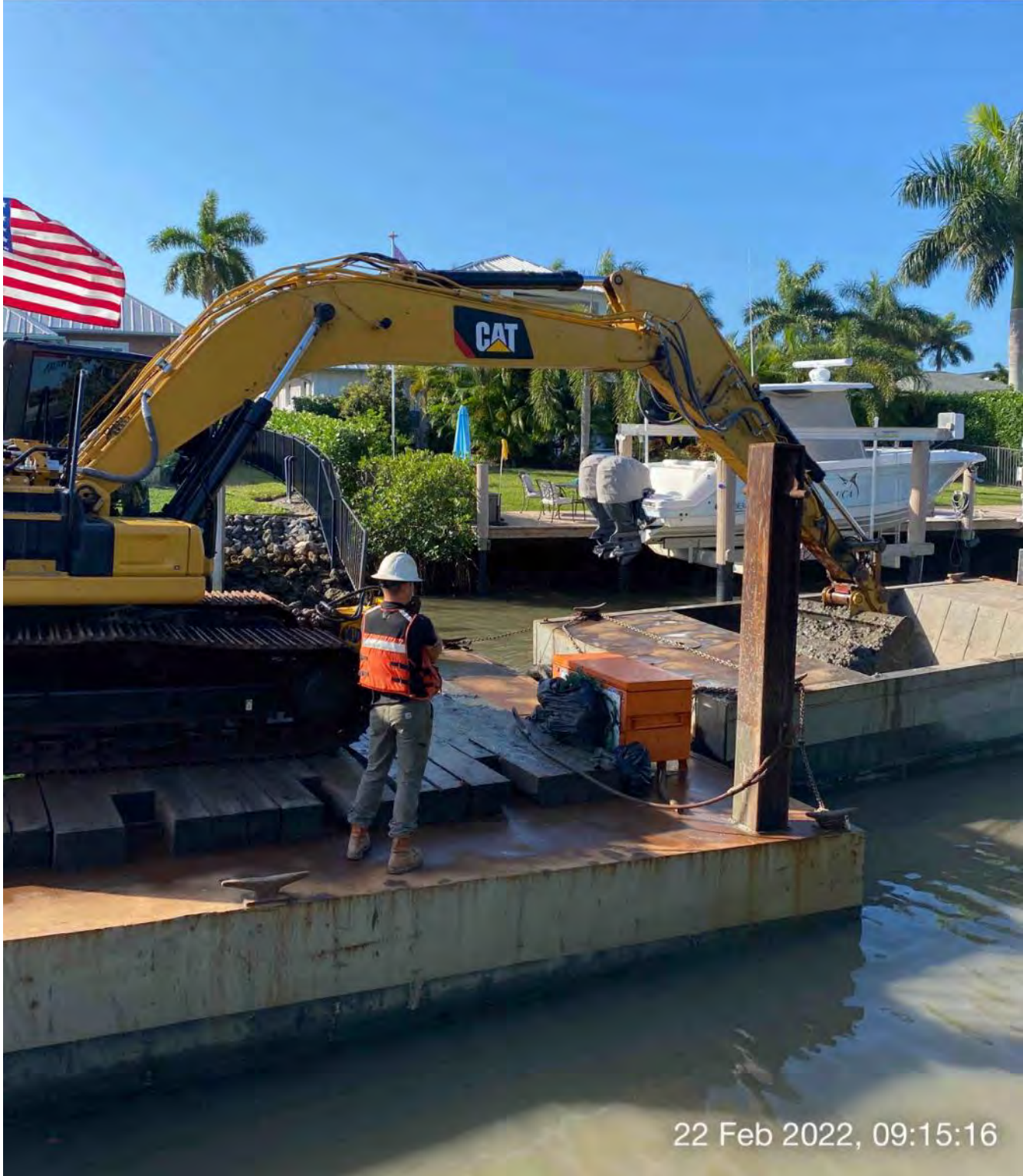
323 excavator removing material from station 5+00 and transferring to hopper
