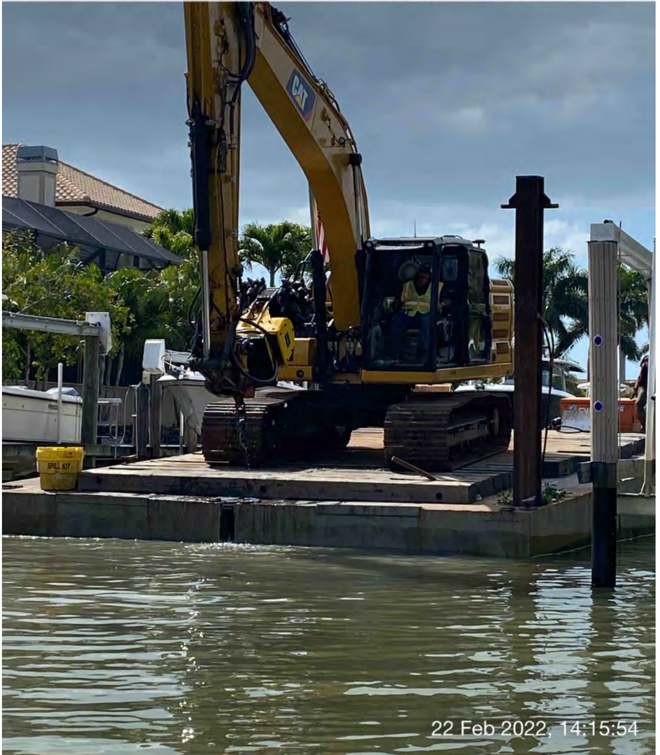
323 excavator with Epiroc grinder on barge at station 8+50
