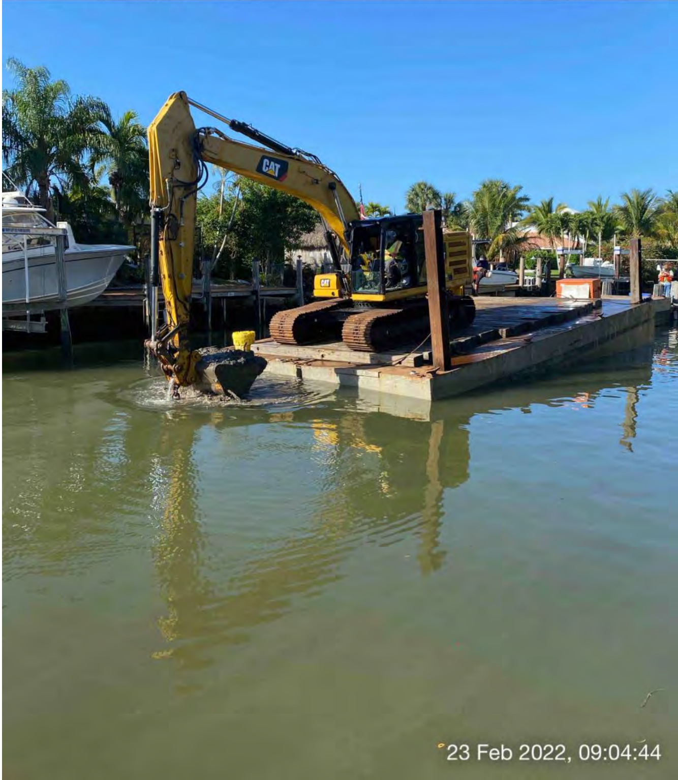
323 excavator removing material from station 12+00 and transferring to hopper
