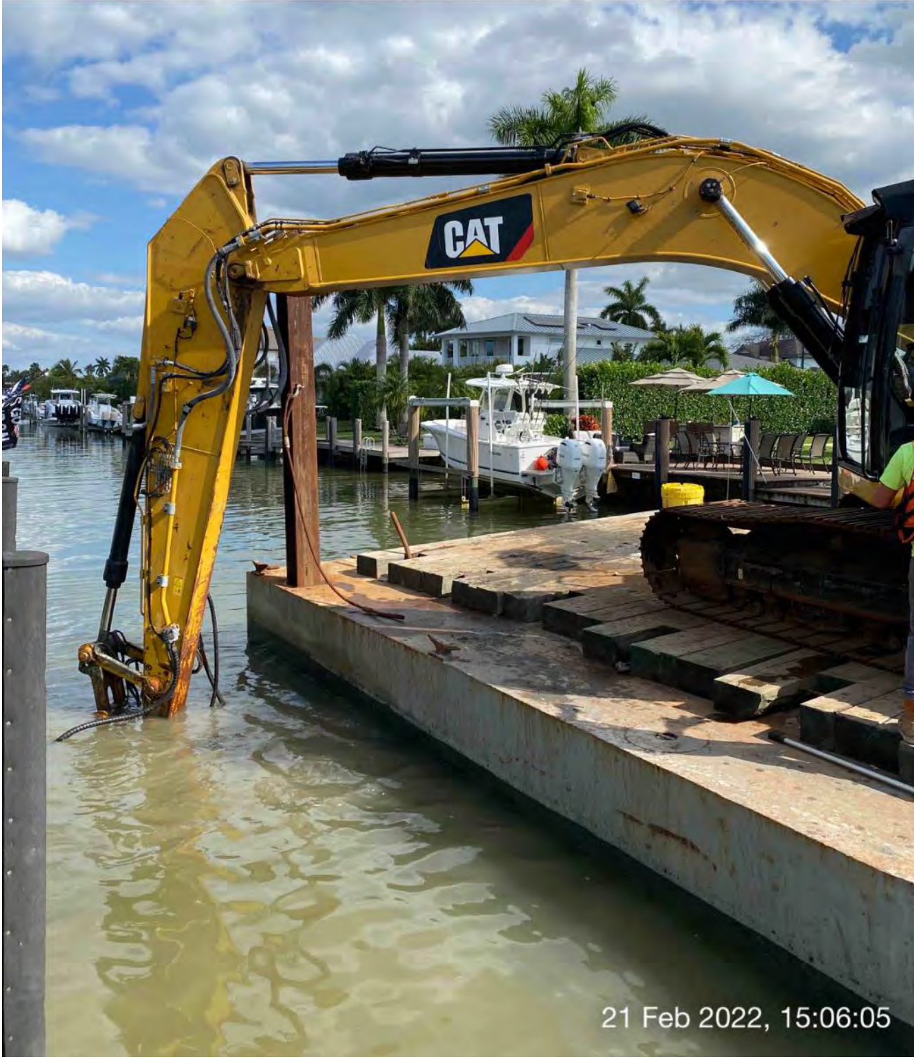
323 excavator grinding rock at station 3+25
