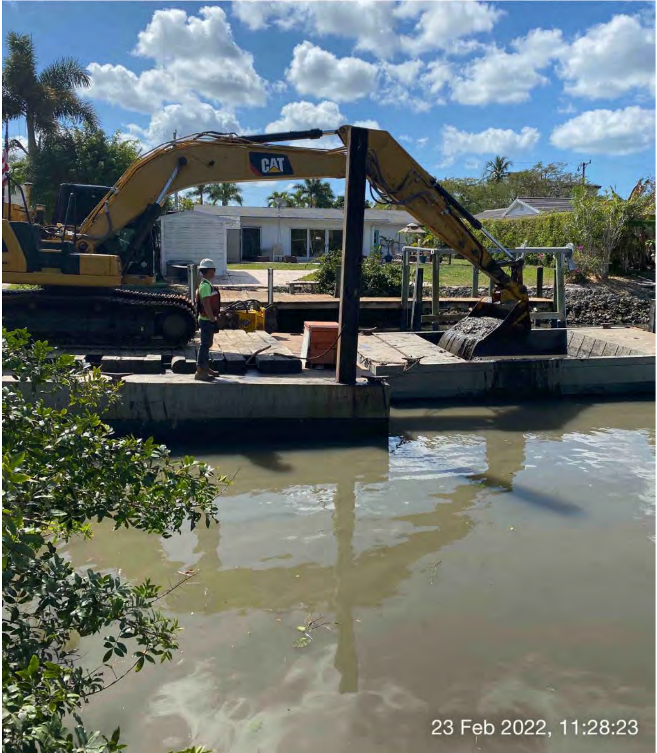
323 excavator removing material from station 13+50 and transferring to hopper
