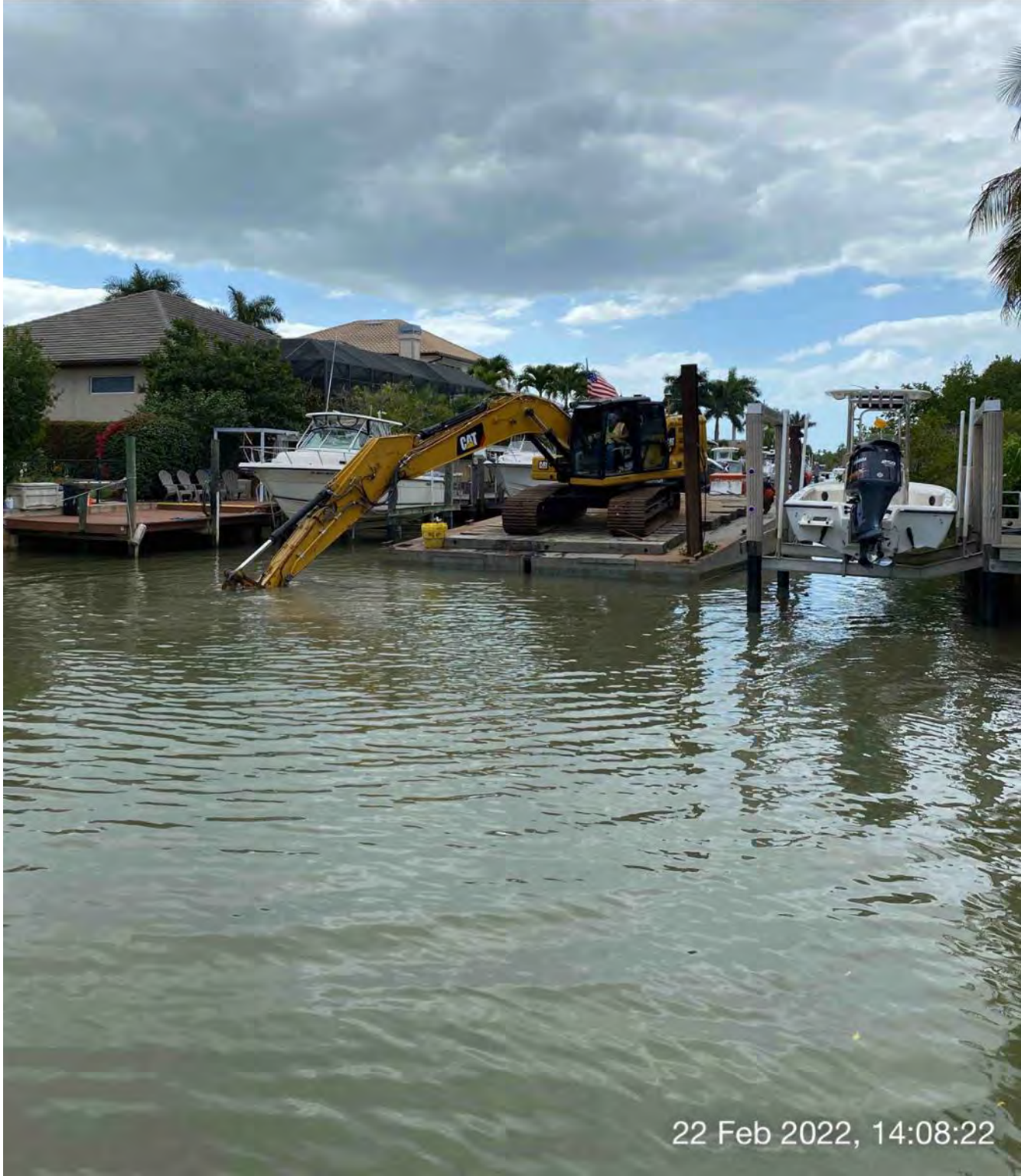
323 excavator grinding rock at station 8+50
