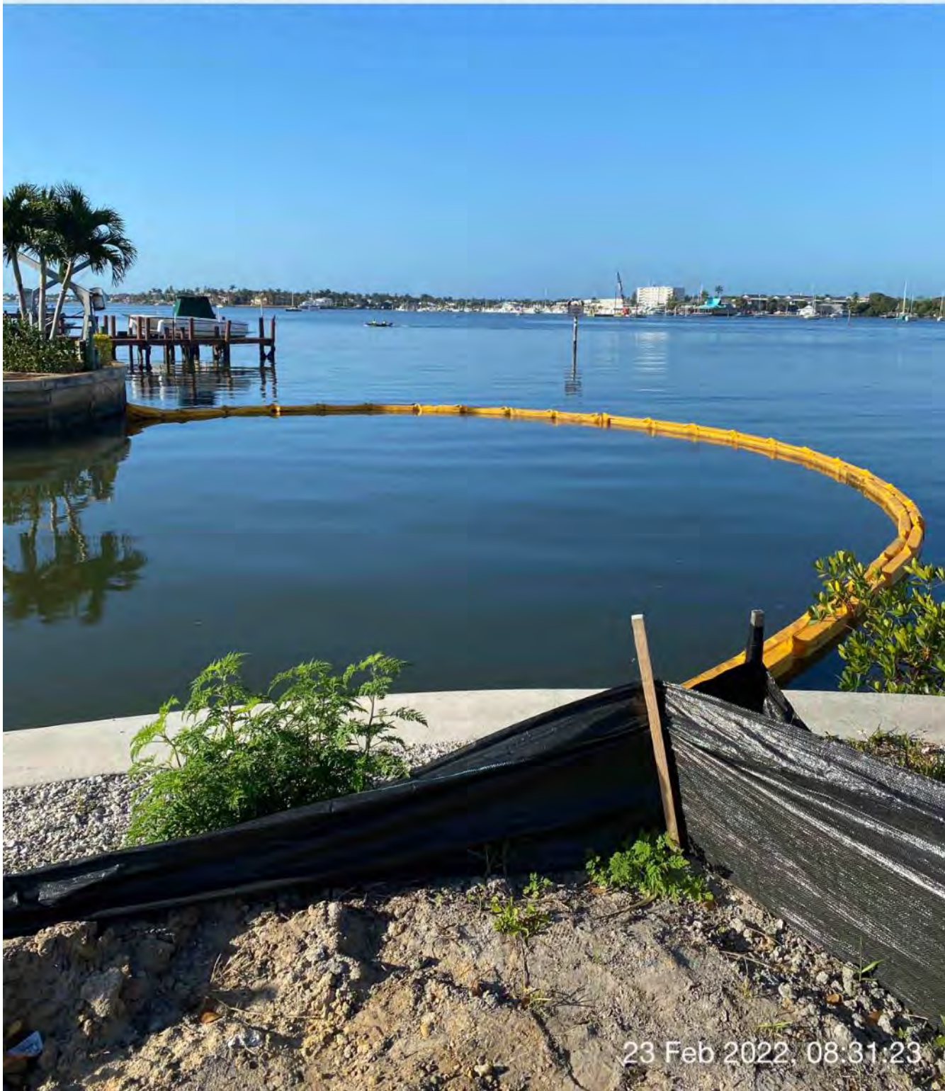
Turbidity curtain across the mouth of Canal CC-CC
