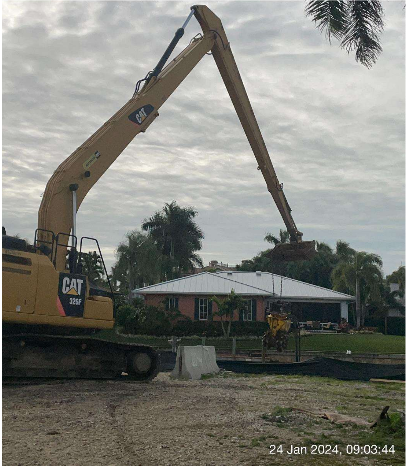
Contractor loading Epiroc grinder into hopper.
