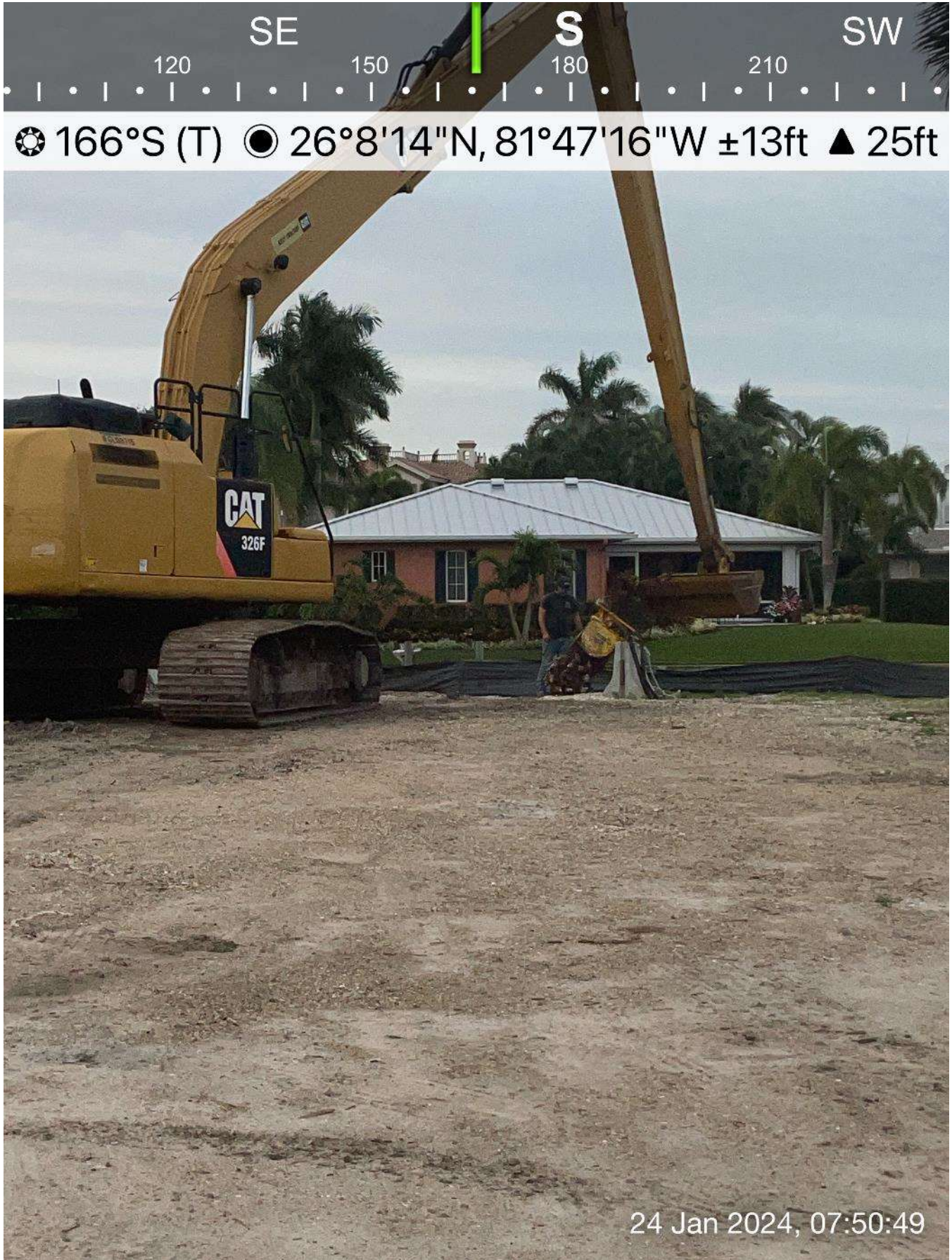
Epiroc grinder arriving on site.
