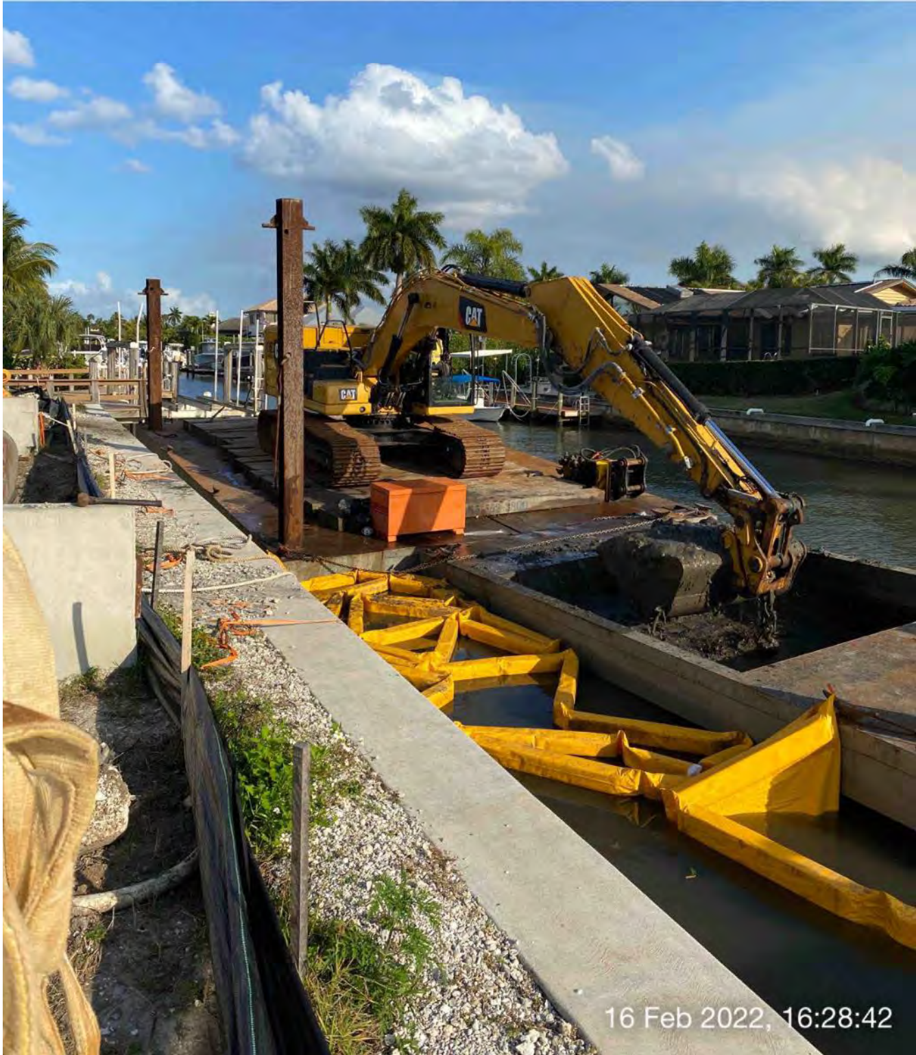
323 excavator transferring material from hopper to dewatering site at 1300 Curlew Avenue
