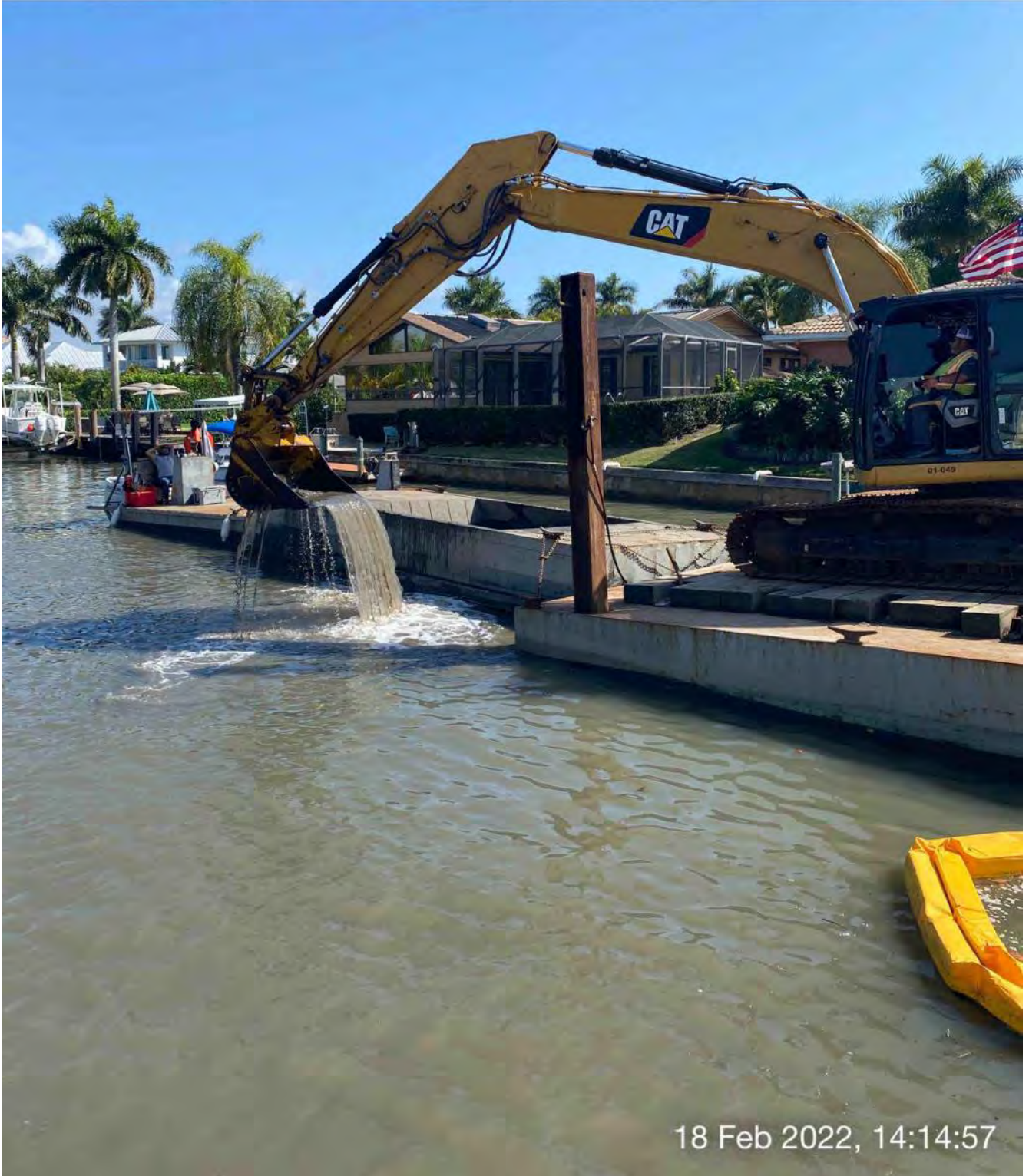
323 excavator removing material from station 1+50 and transferring to hopper
