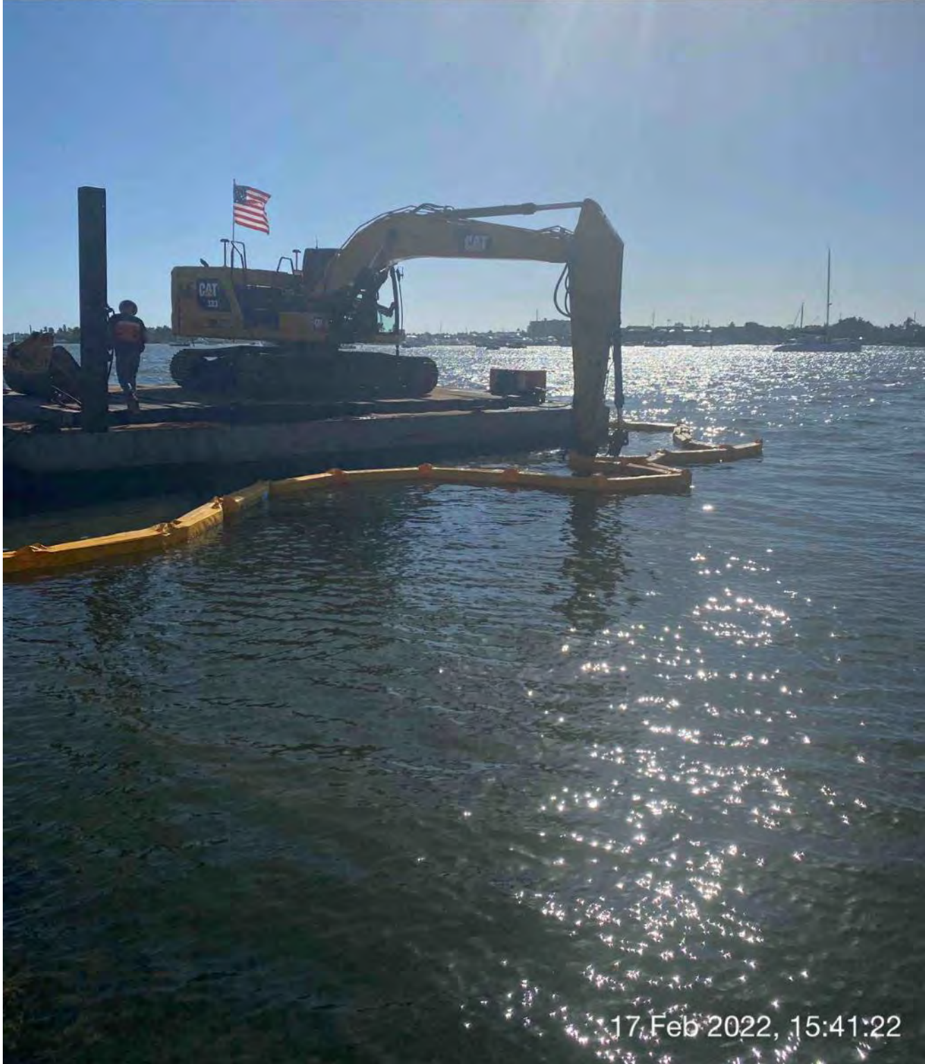
323 excavator grinding rock at station 0+50
