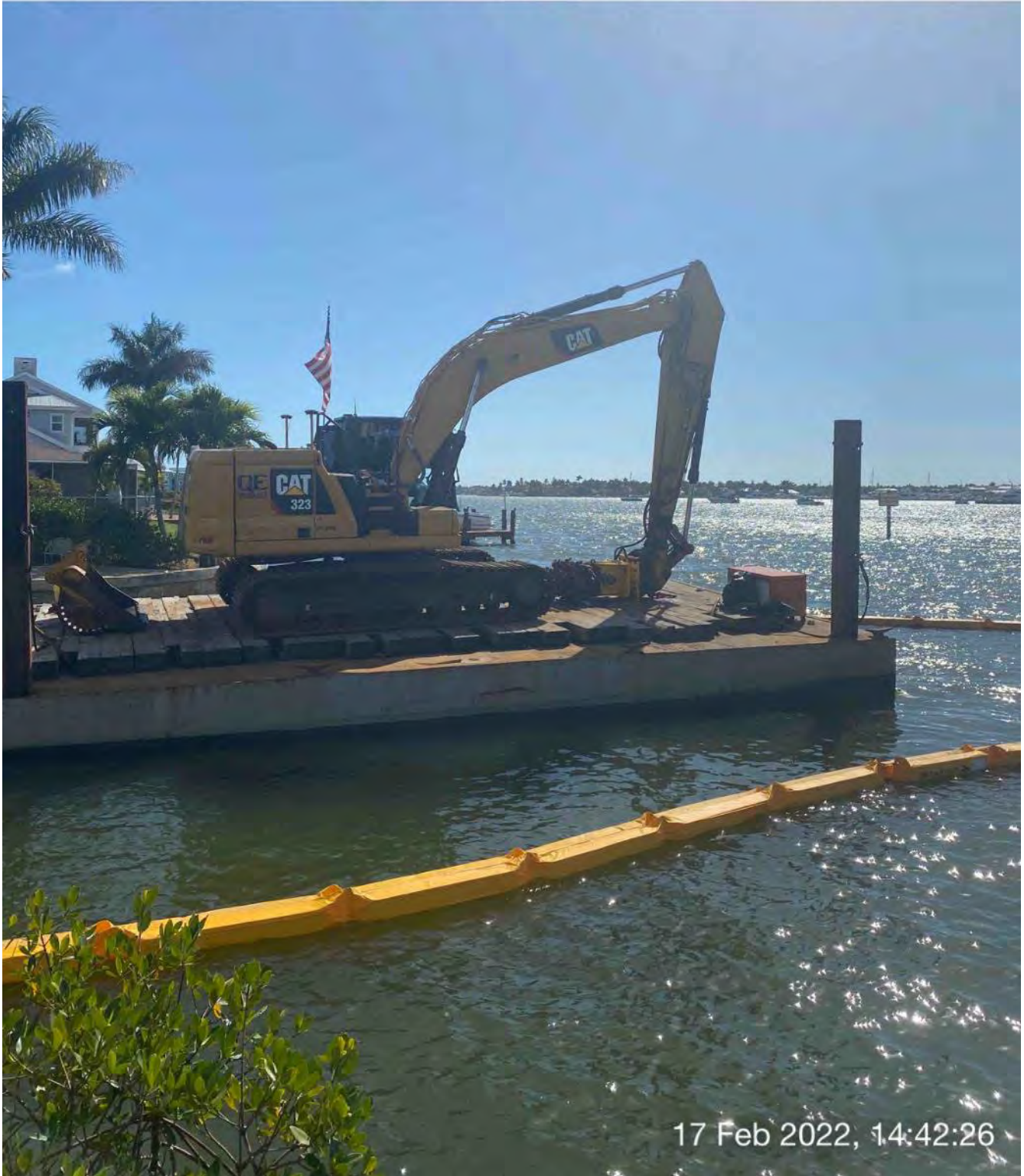
323 excavator with Epiroc grinder on barge at station 0+75
