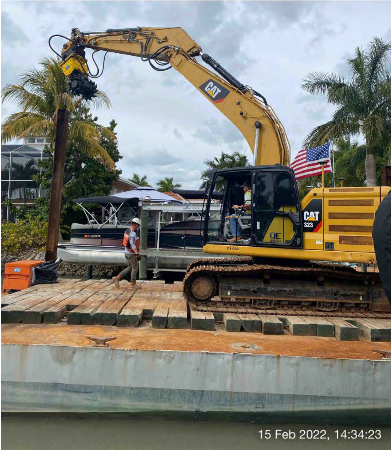
323 excavator lifting spud to allow push boat to mobilize barge at station 10+25
