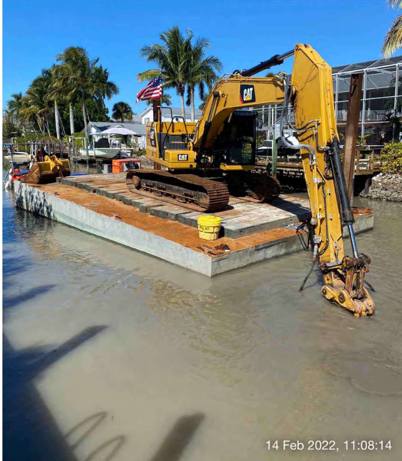
323 excavator grinding rock at station 9+50
