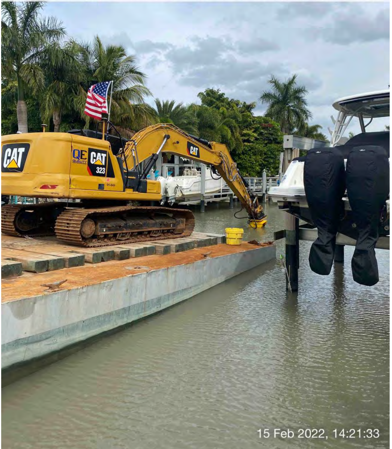
323 excavator grinding rock at station 10+25
