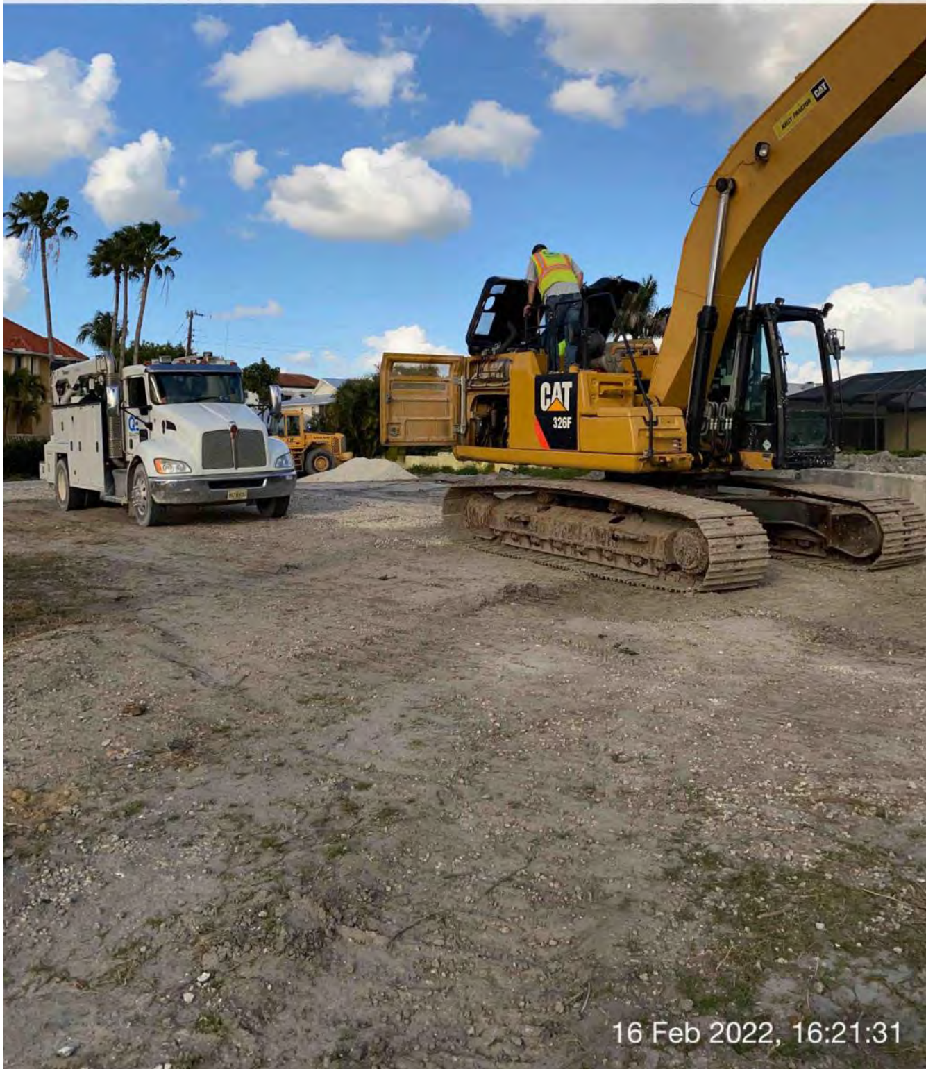
Mechanic inspecting 326 excavator
