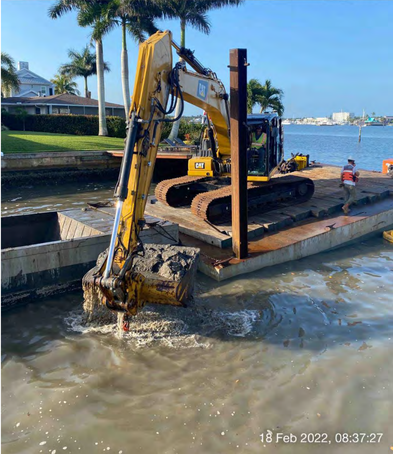
323 excavator removing material from station 1+00 and transferring to hopper
