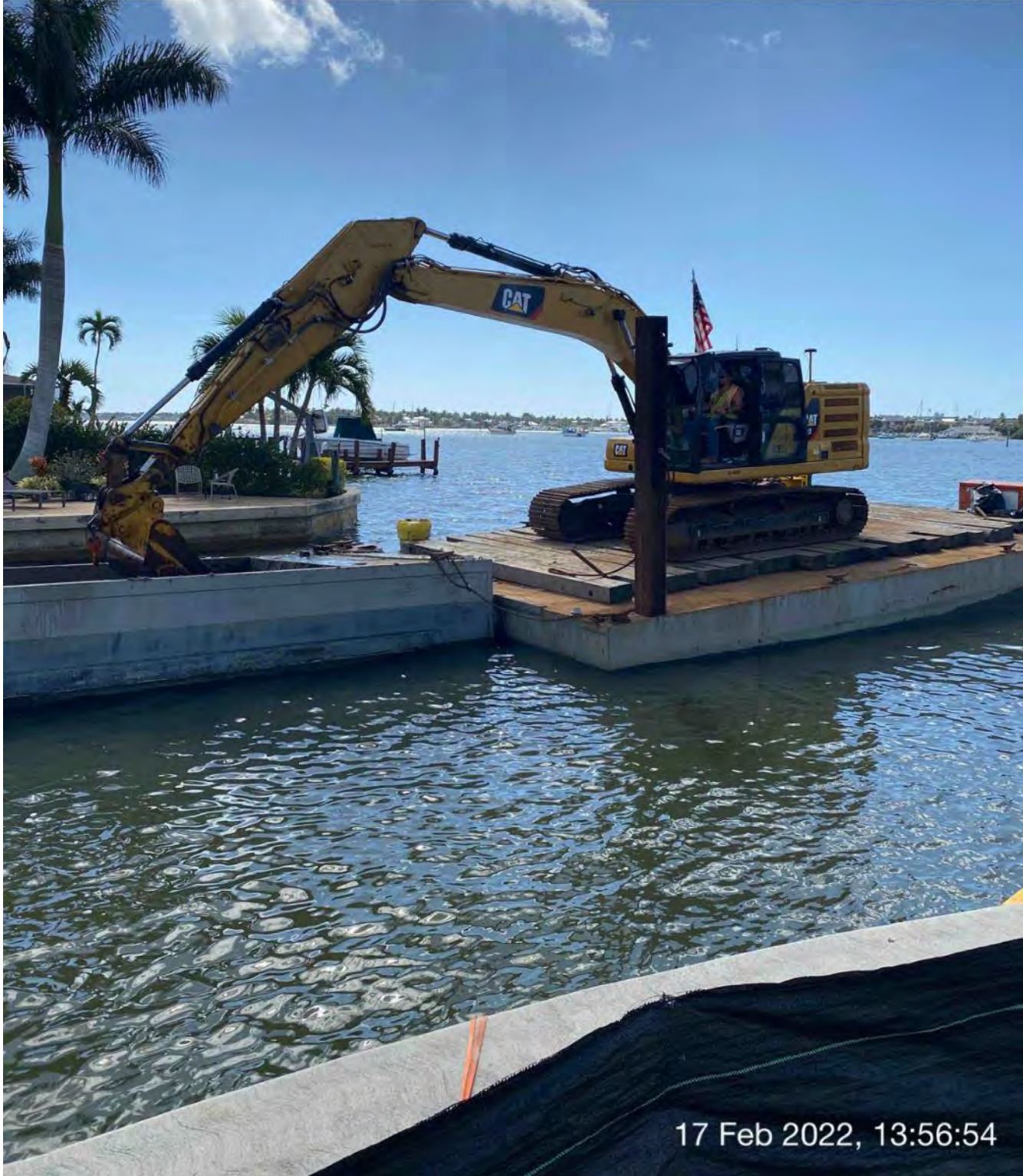
323 excavator removing material from station 0+50 and transferring to hopper
