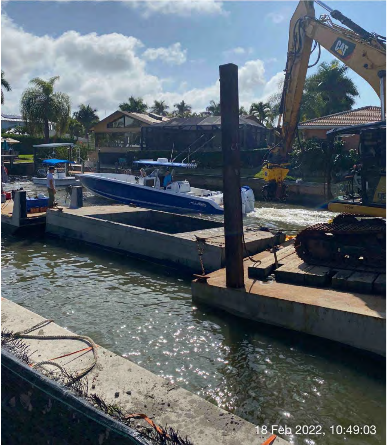
Canal CC-CC resident entering the canal
