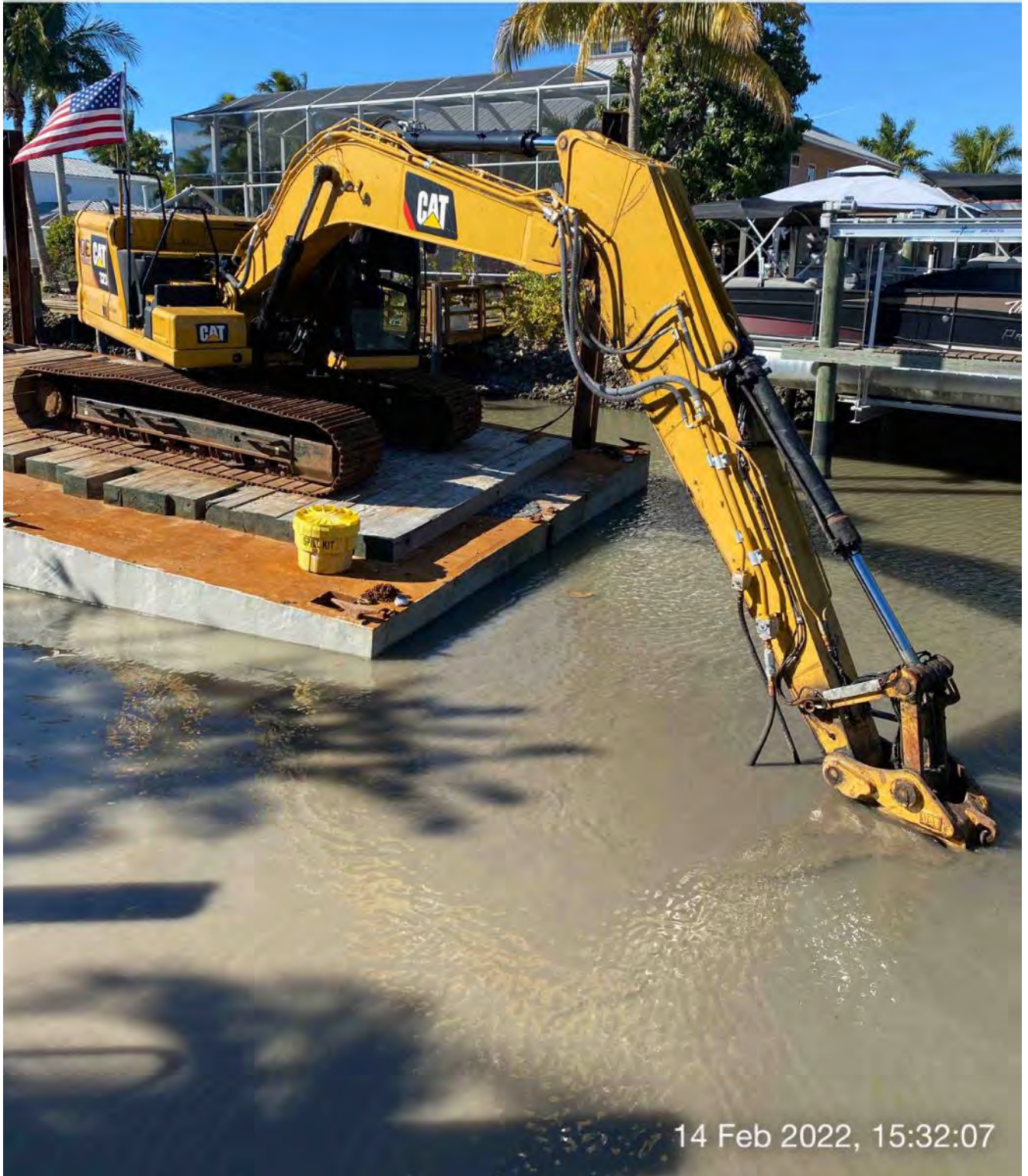
323 excavator grinding rock at station 9+75
