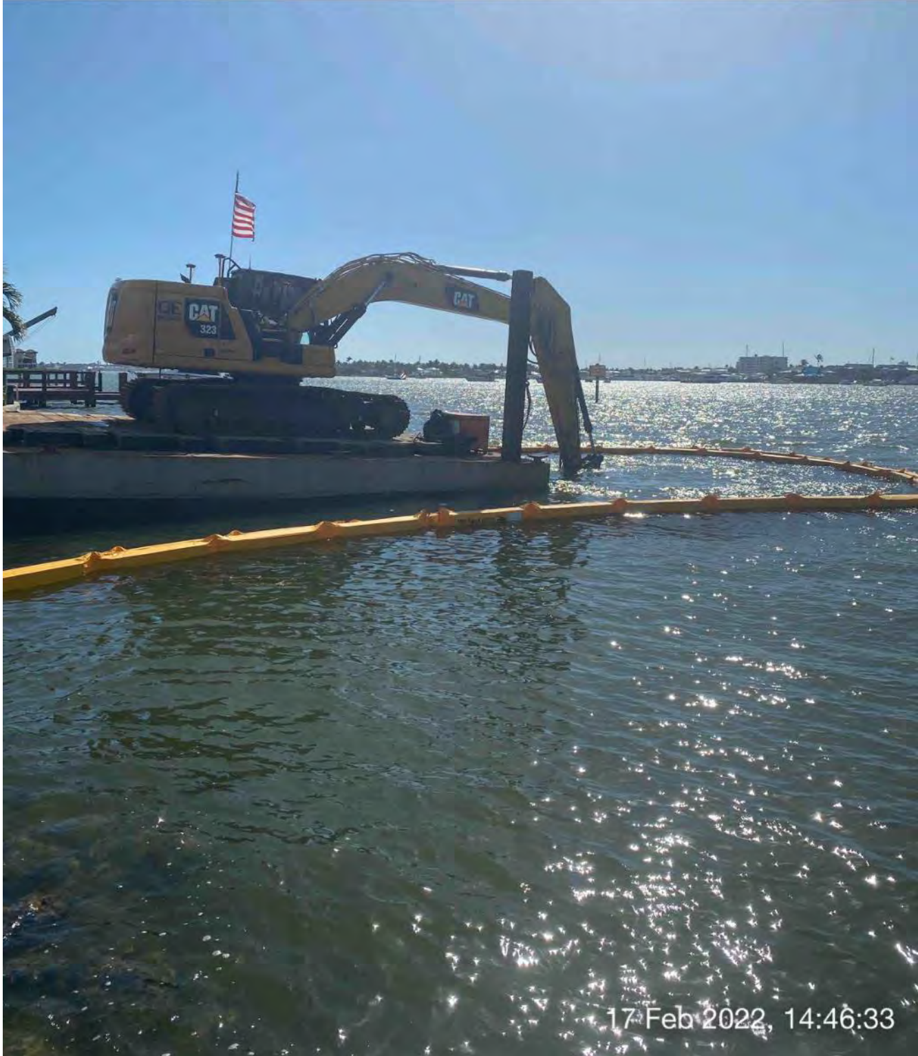
323 excavator grinding rock at station 0+50
