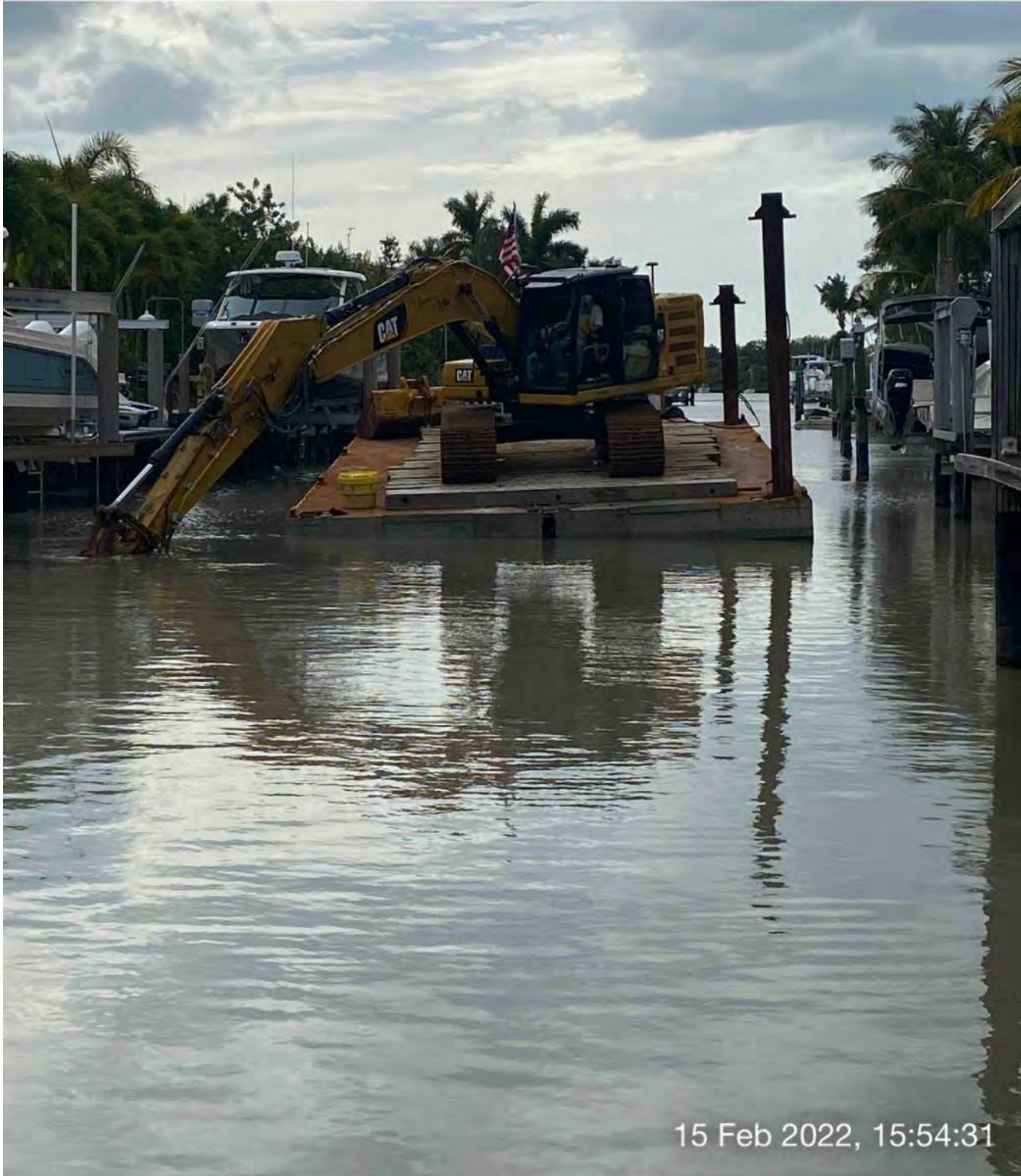
323 excavator grinding rock at station 11+00
