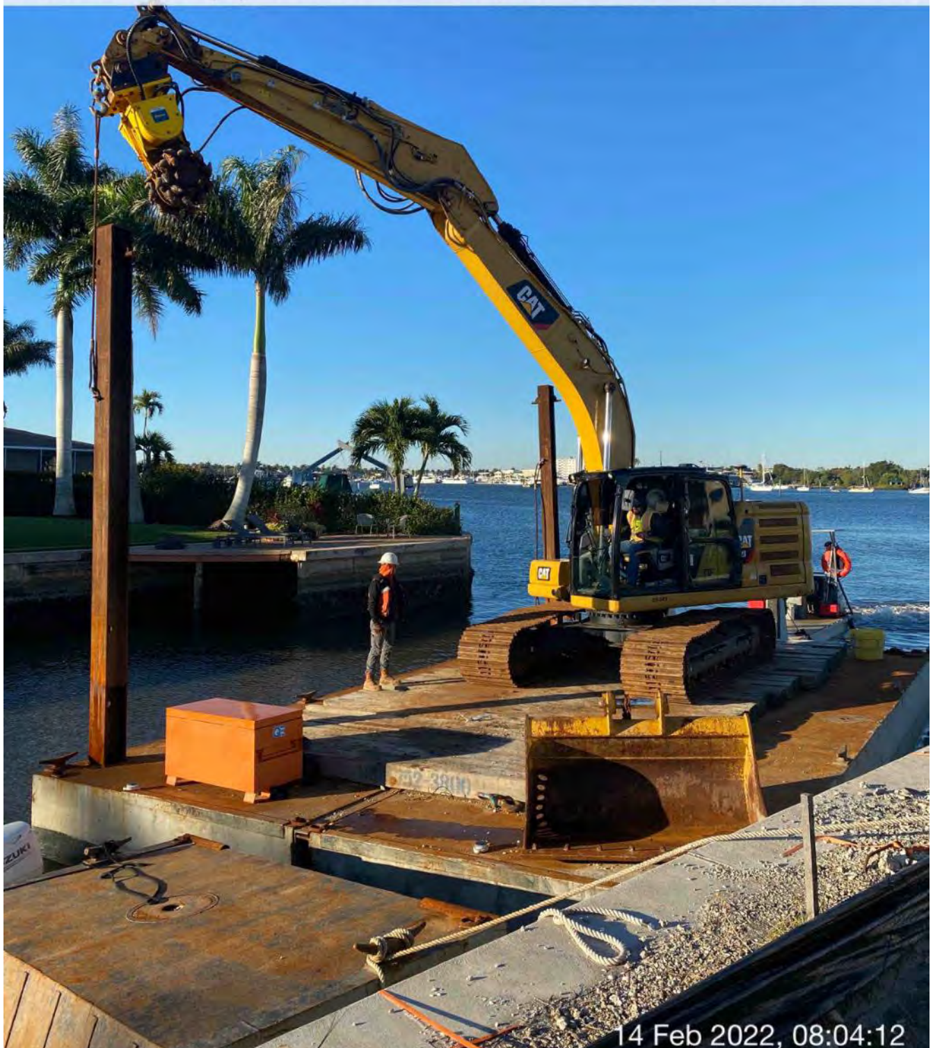
323 excavator lifting spud to allow push boat to mobilize barge at station 1+50 in Canal CC-CC
