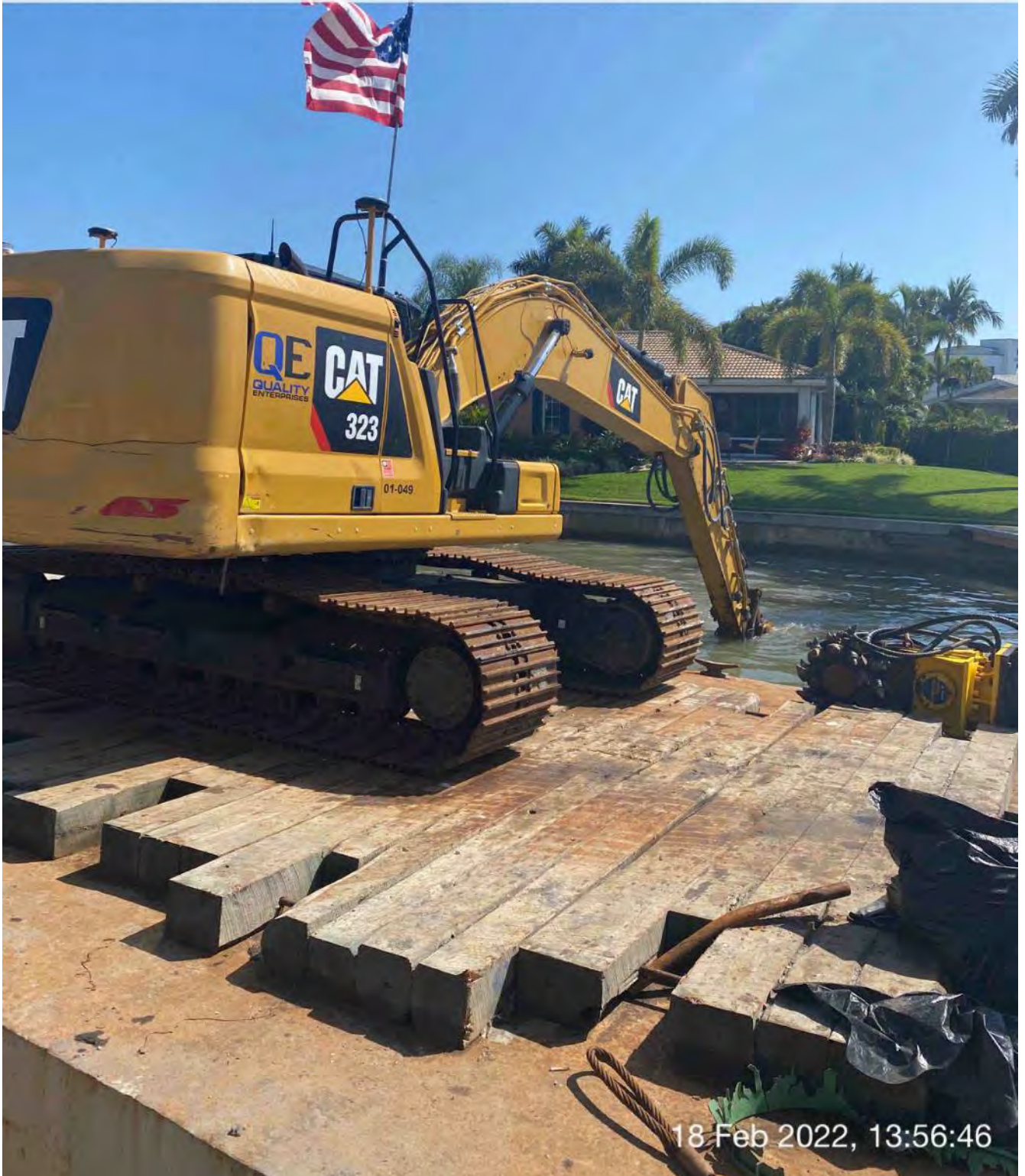
323 excavator grinding rock at station 1+00
