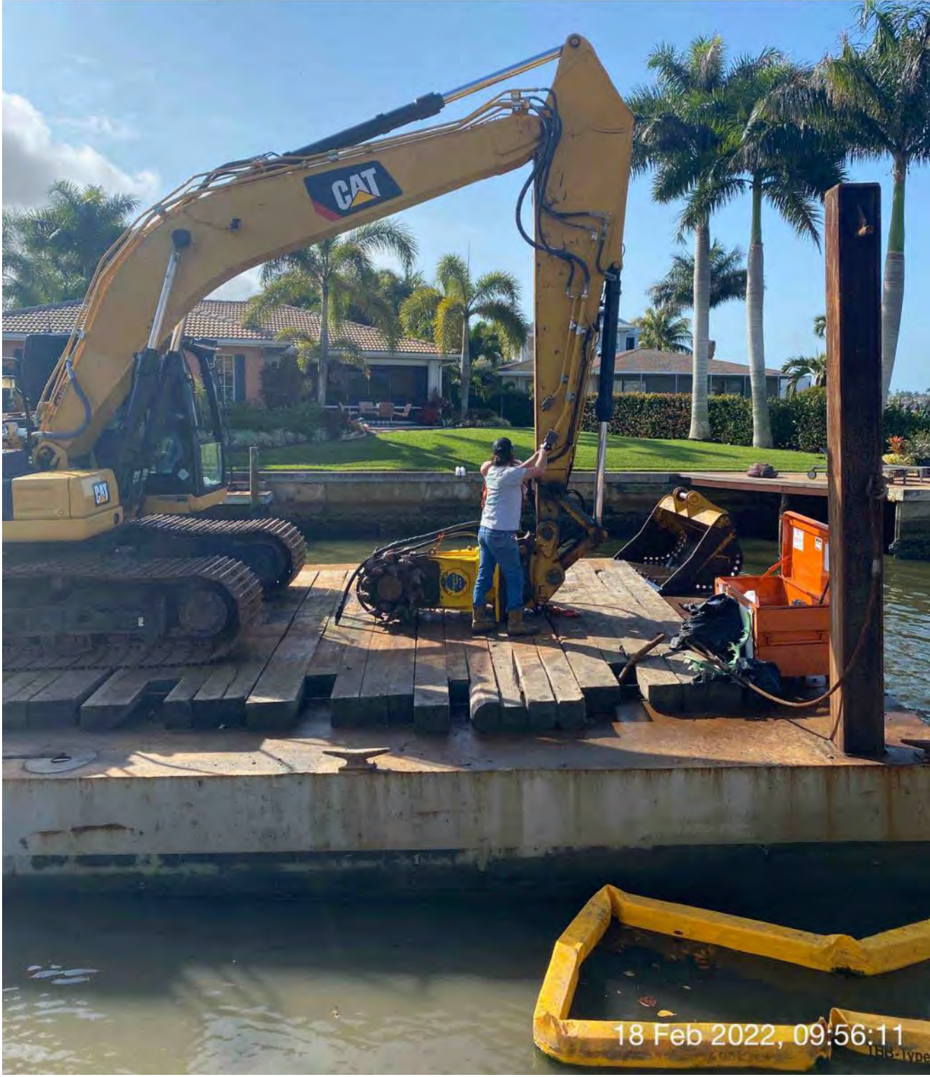
Changing attachment from bucket to Epiroc grinder on the 323 excavator at station 1+50
