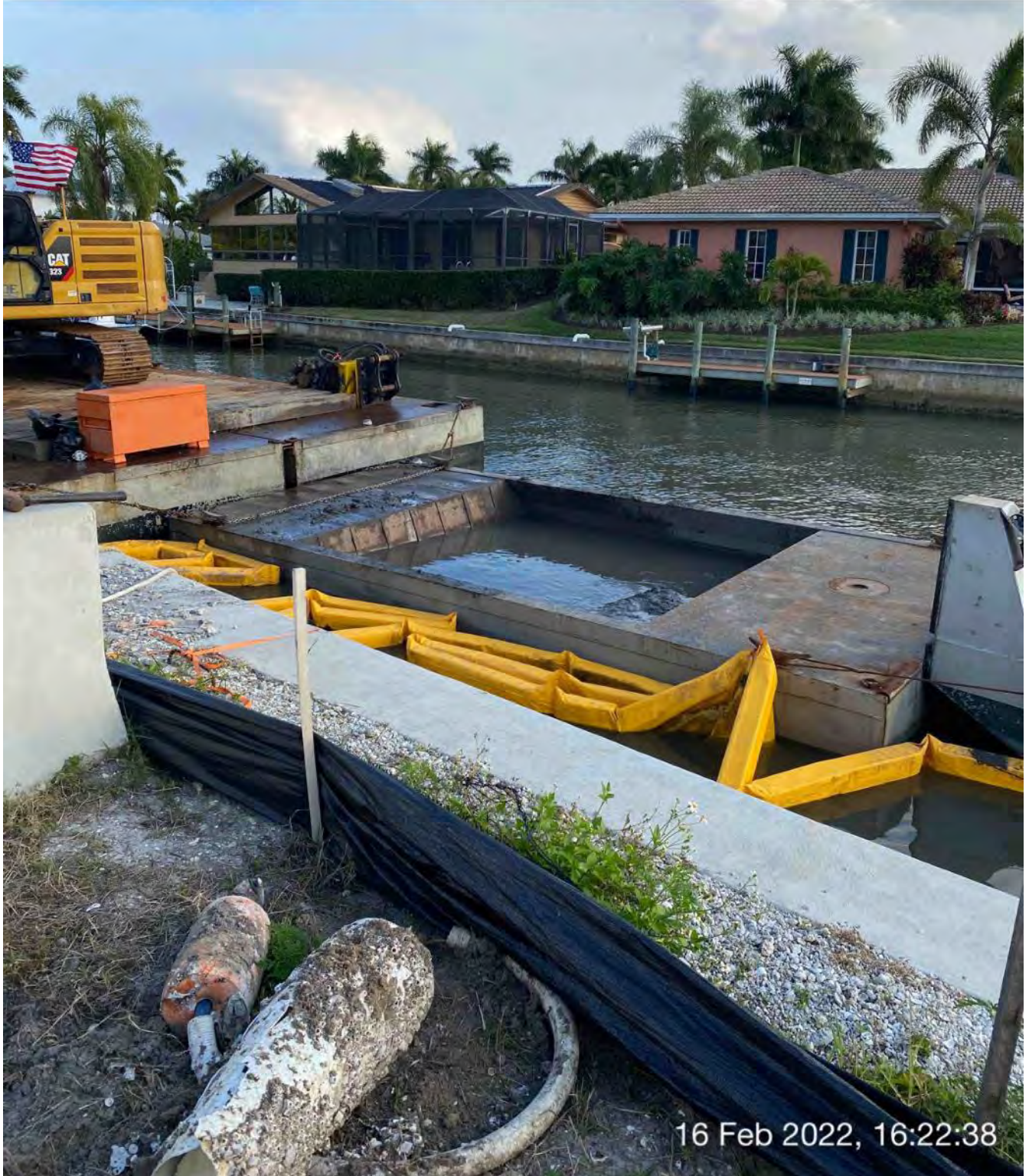
Hopper full of removed material from Canal CC-CC
