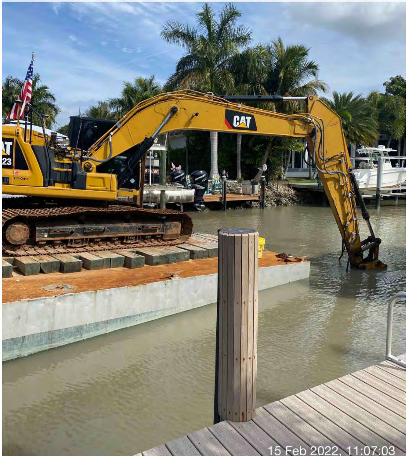
323 excavator grinding rock at station 10+00
