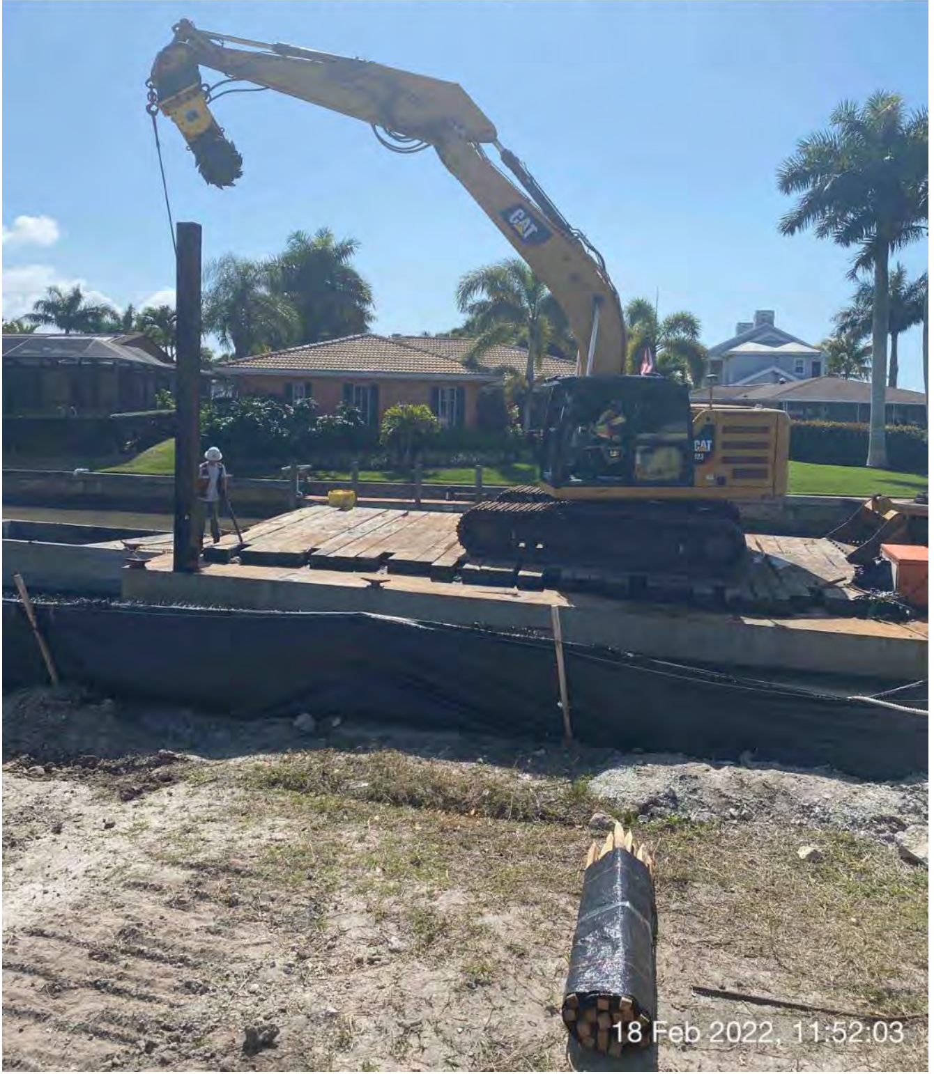
323 excavator lifting spud to allow push boat to mobilize barge at station 1+50
