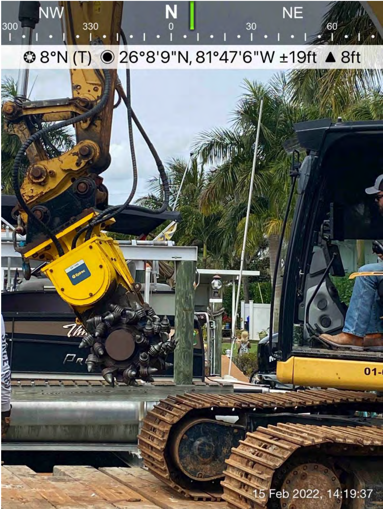
Epiroc grinder on 323 excavator
