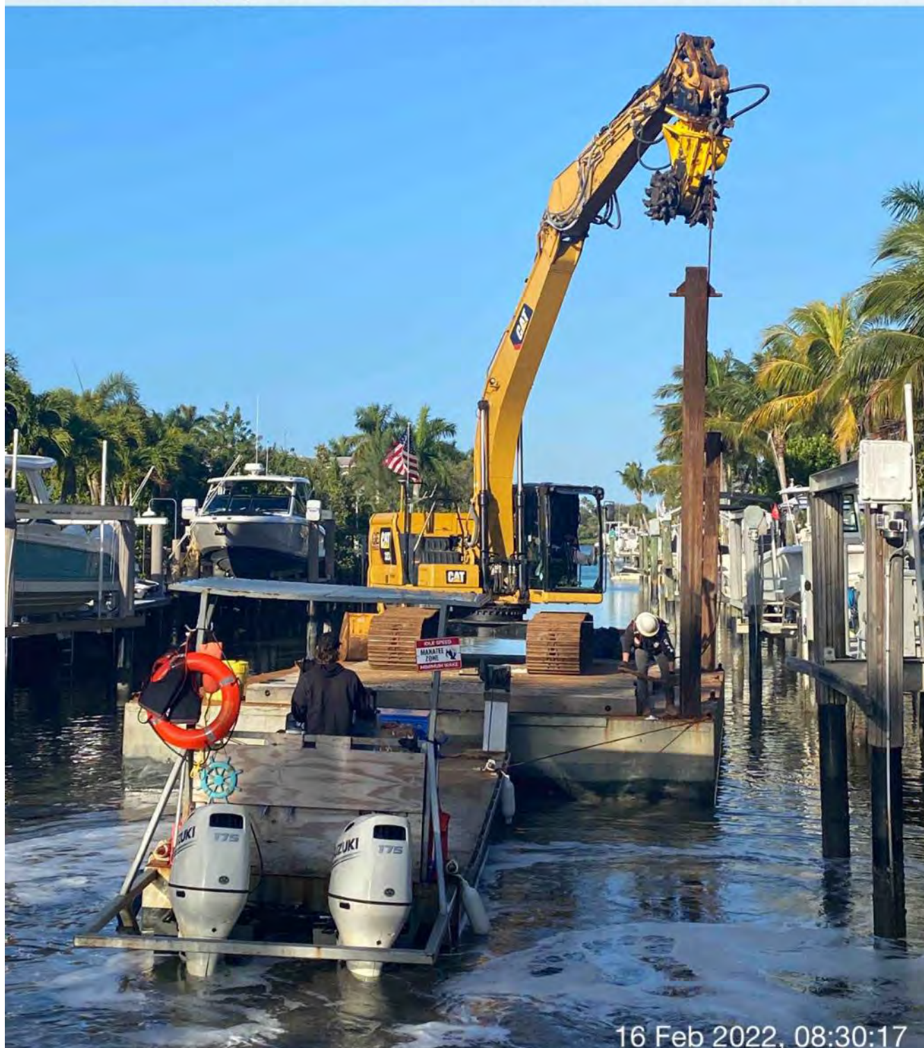
323 excavator lifting spud to allow push boat to mobilize barge at station 11+00 in Canal BB-BB
