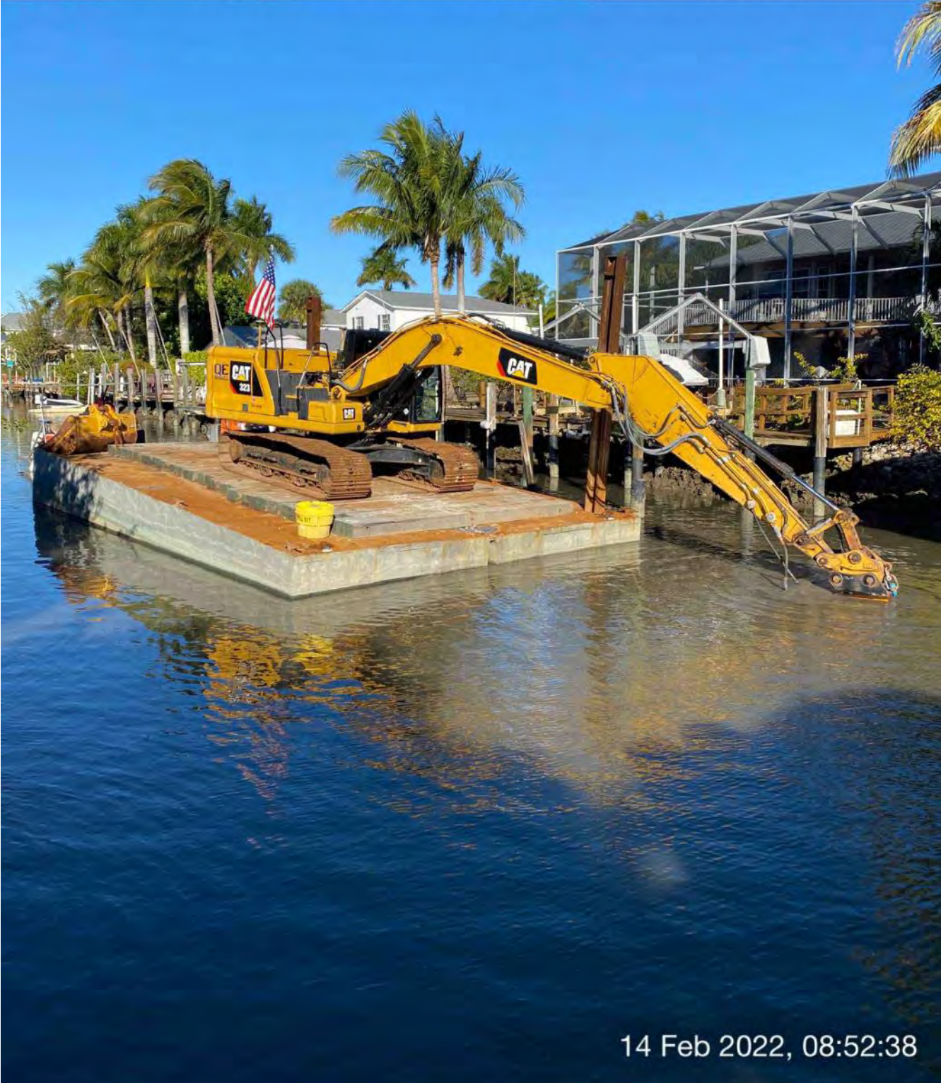
323 excavator grinding rock at station 9+50
